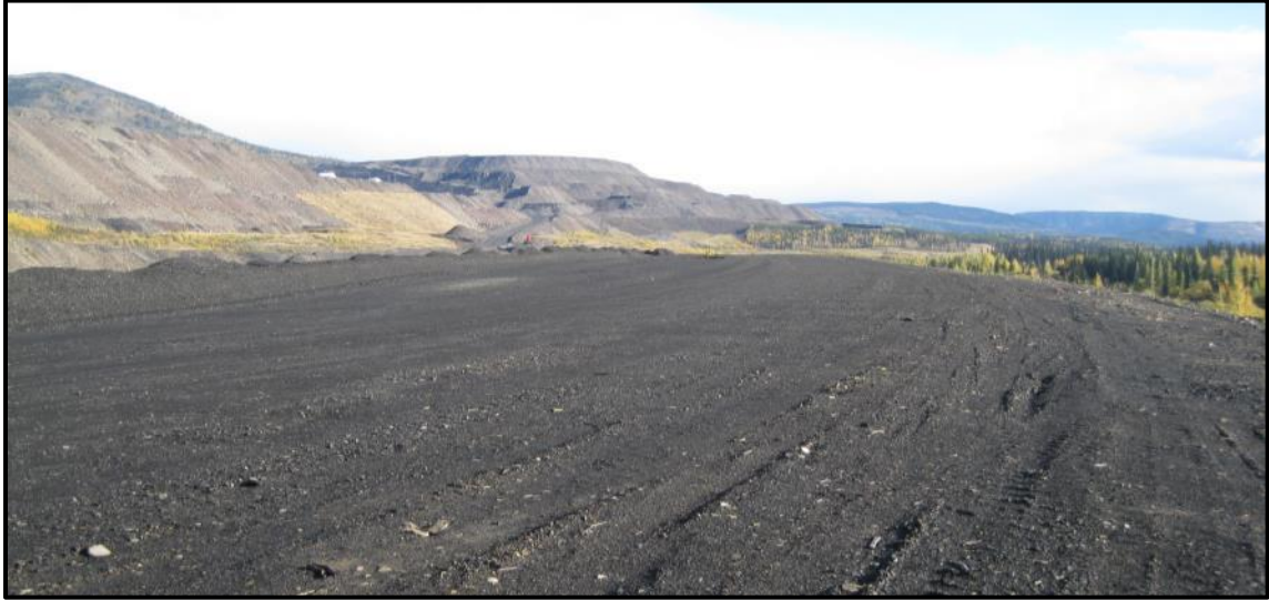
Photo 3: Crest area of the main embankment (looking northeast).
