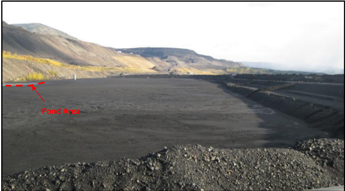
Photo 13: Tailings beach with edge of pond on far left (looking north).
