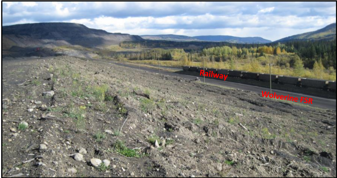
Photo 7: Reclamation on the main embankment downstream slope (looking northeast)
