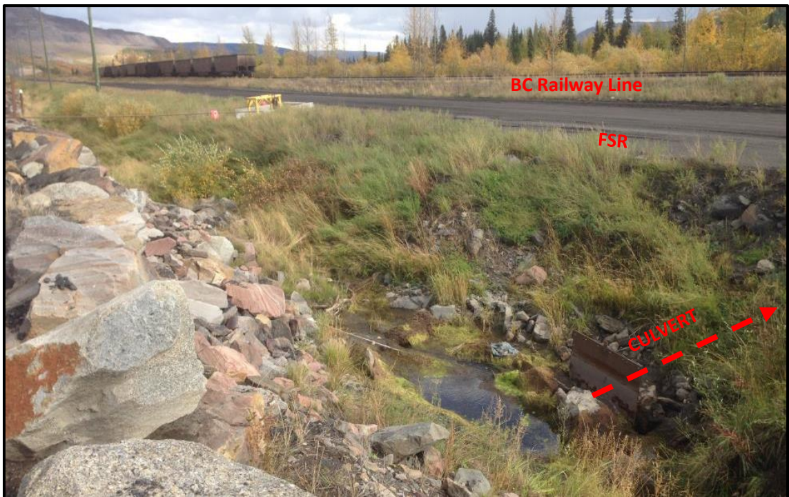
Photo 12: Toe drain ditch at approx. Station 7+00 (looking northeast). Minor flow (< 0.5 l/s, clear) observed coming from the toe drain and directly into the culvert.
