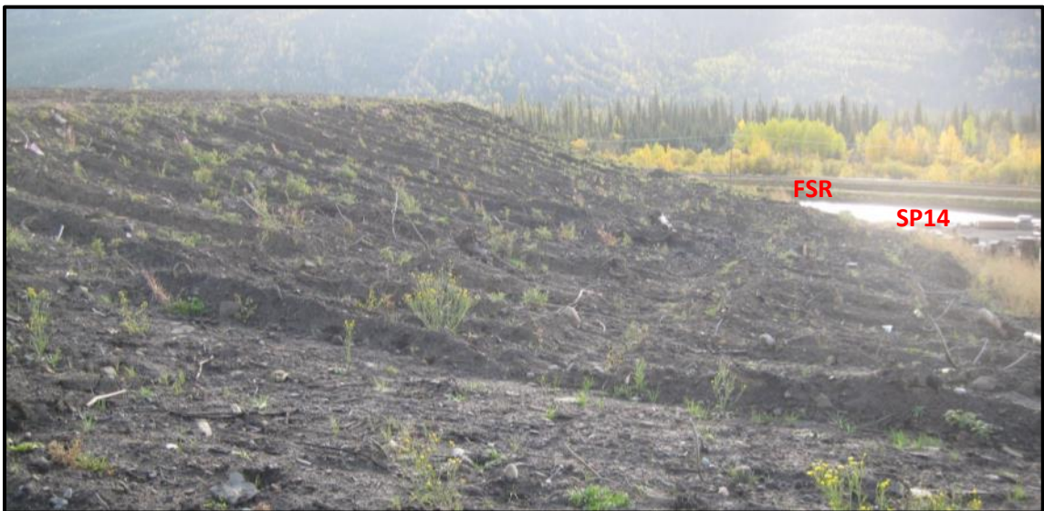
Photo 6: Reclamation material placed on the southern embankment downstream slope (looking east).
