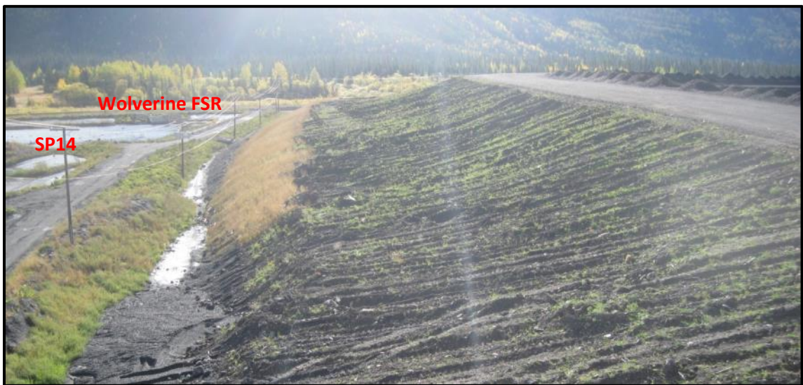
Photo 8: Reclamation on the northeastern embankment downstream slope (looking southeast)
