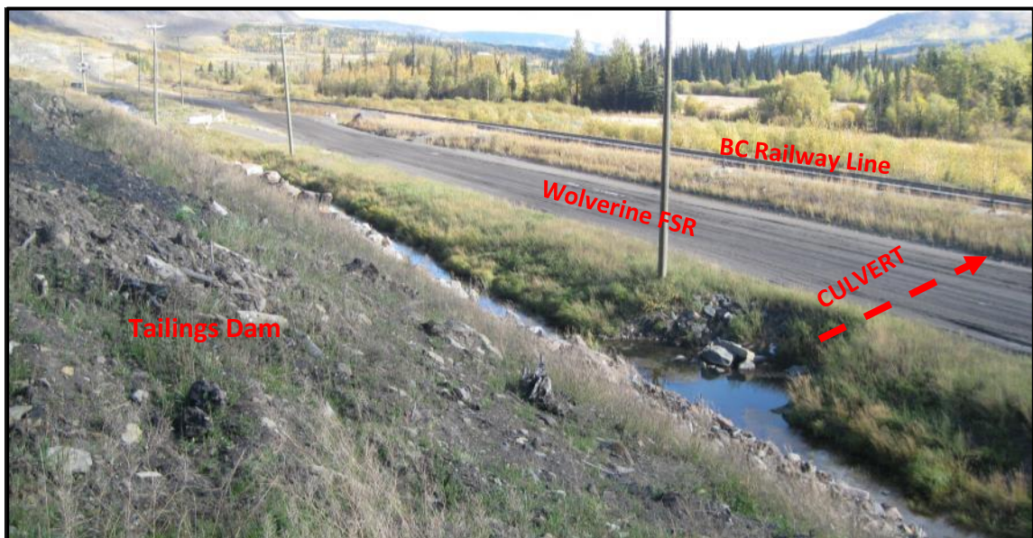
Photo 10: Toe drain ditch at approx. Station 3+00 (looking northeast). Water ponding between approx. Stations 3+00 and 4+50 due to plugged culverts at time of inspection. Culverts have since been opened up.
