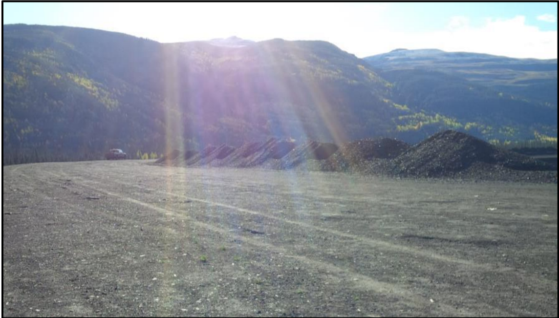
Photo 5: Crest area of the northern embankment (looking southeast).
