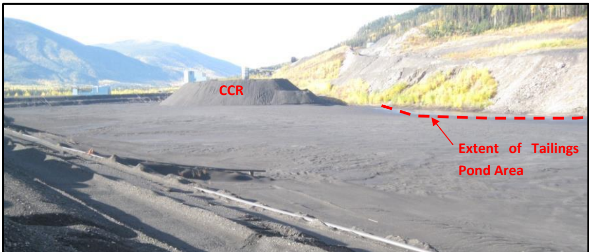
Photo 14: Winter CCR Temporary Stockpile (looking southwest) with tailings pond on right side.
