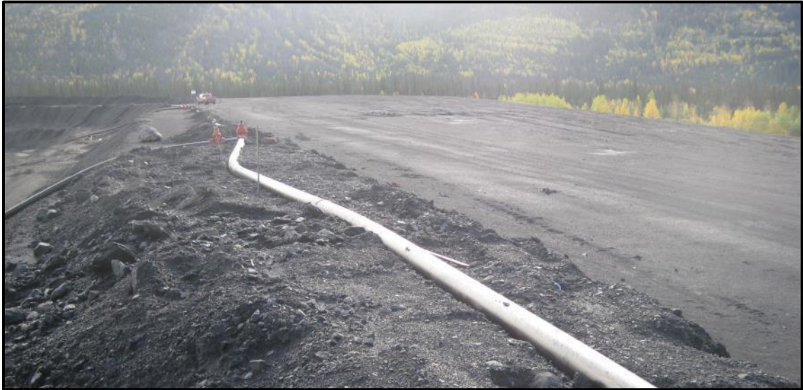
Photo 2: Crest area of the south embankment (looking east).
