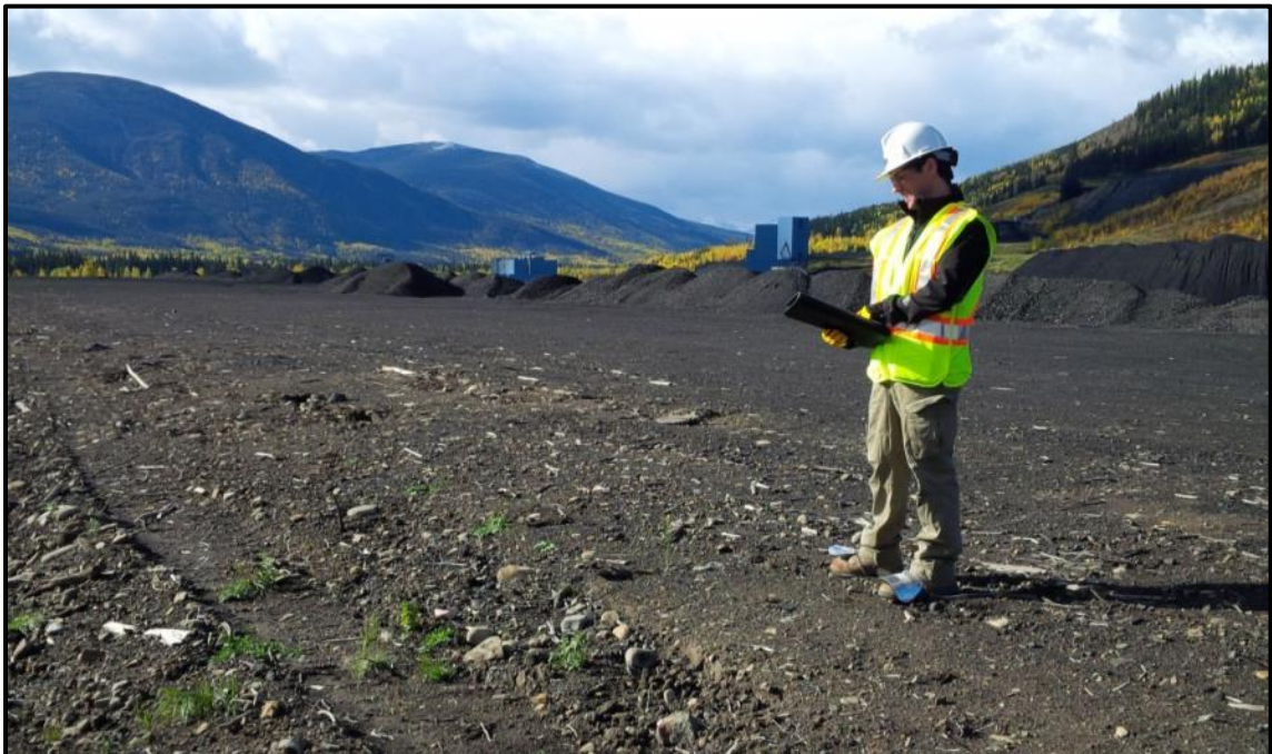
Photo 4: Crest area of the main embankment (looking southwest).
