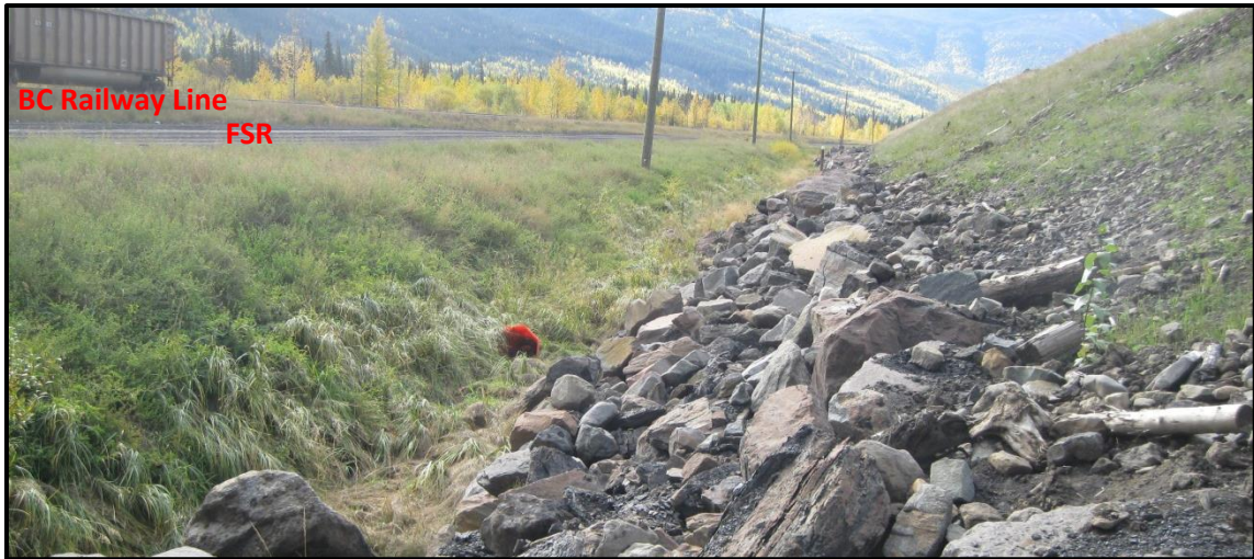
Photo 11: Toe drain ditch between Stations 4+00 and 5+00 (looking south). Ditch is generally dry from this point heading south.
