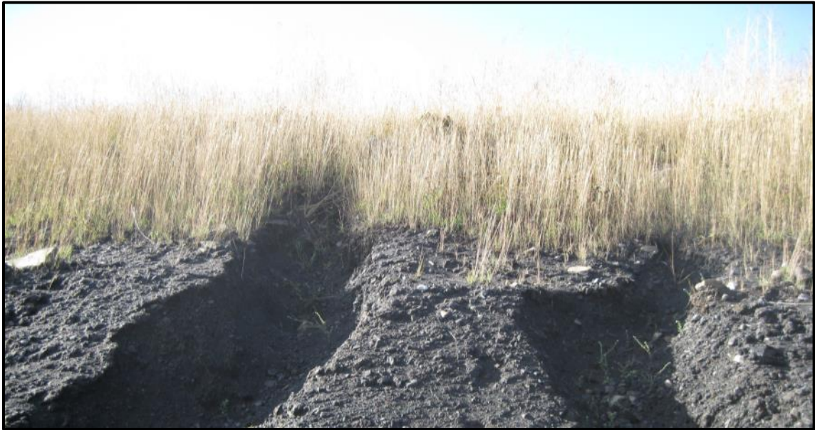
Photo 9: Reclamation on the northeastern embankment downstream slope. Further erosion has been minimized due to the presence of established vegetation.
