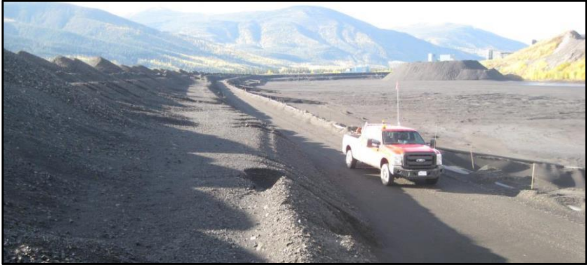
Photo 1: Upstream slope of the main embankment (looking southwest).
