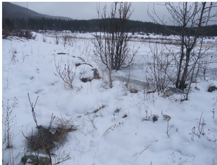
Photo 1: Upstream view of spillway inlet at TSF 1 (October 28/14)
