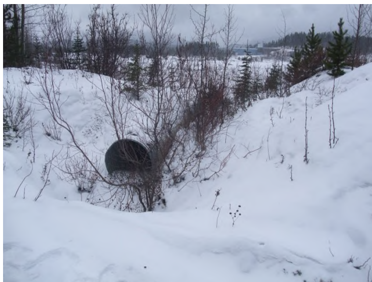
Photo 3: Incomplete culvert installation at south end of TSF 1 (October 28/14)
