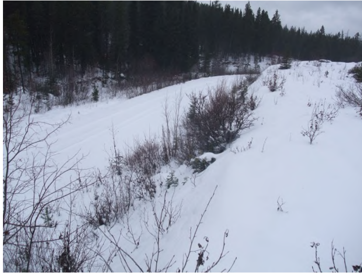
Photo 4: Oversteep section of berm along west side of TSF 1 (October 28/14)
