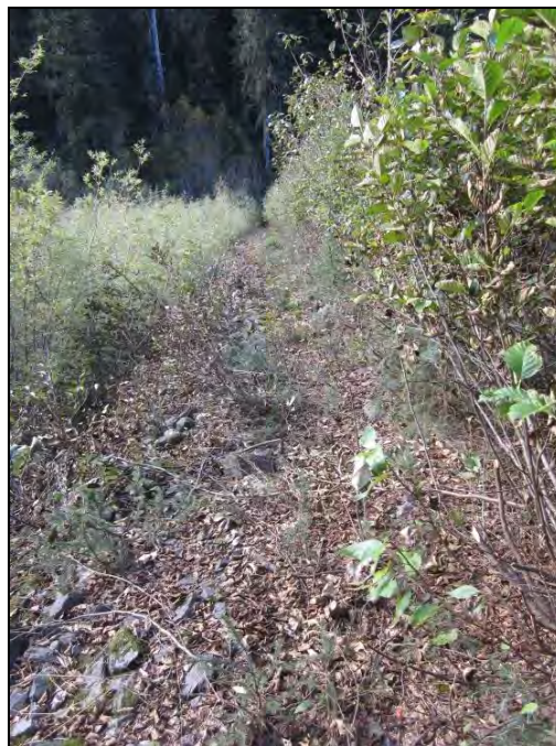
PHOTO 26 – Dyke 3 – Clear upstream crest of dyke at intersection with the downstream face of Dyke 3.
