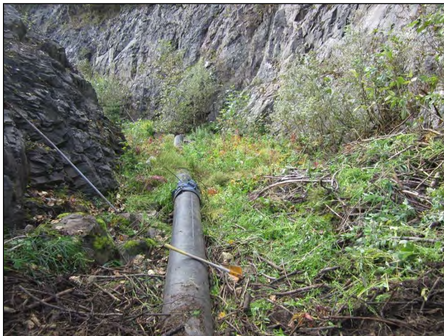
PHOTO 15 – Spillway - Side slopes and beaver protection pipe.
