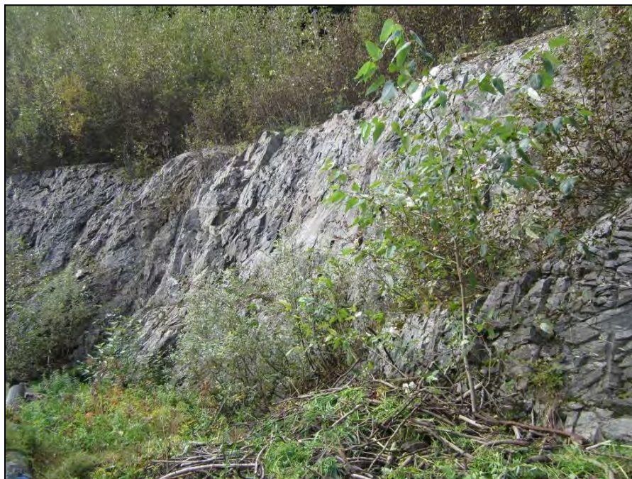
PHOTO 17 – Spillway – rock cut side slopes.
