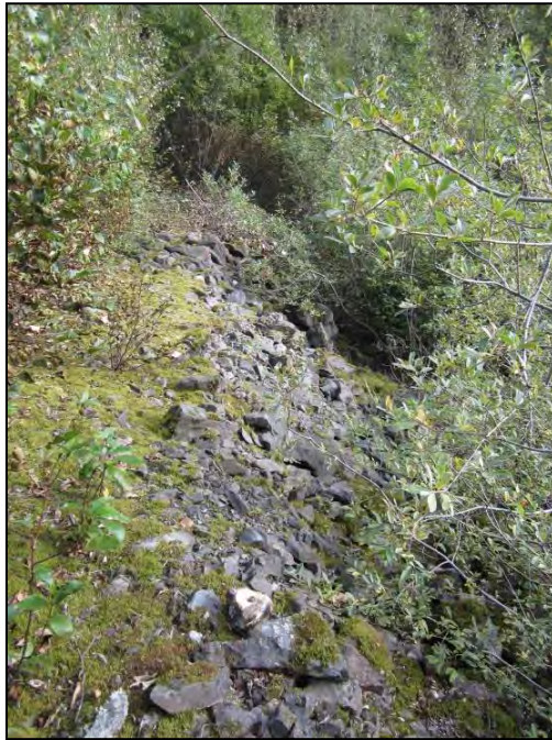
PHOTO 27 – Dyke 3 – Upstream face riprap.
