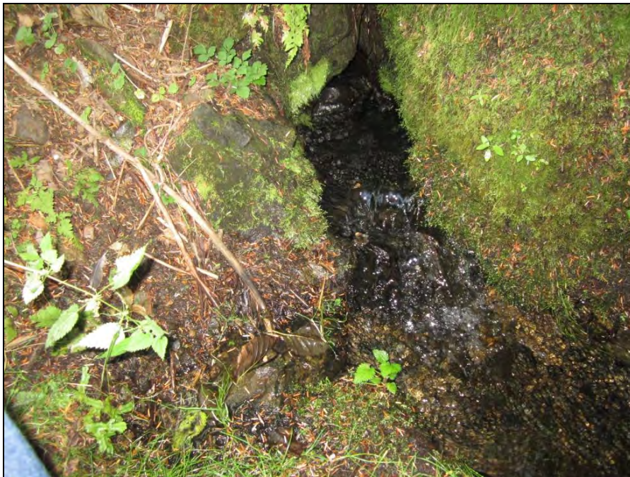
PHOTO 30 – Dyke 3 seepage – clear estimated flow rate 1 to 1.5 l/sec.
