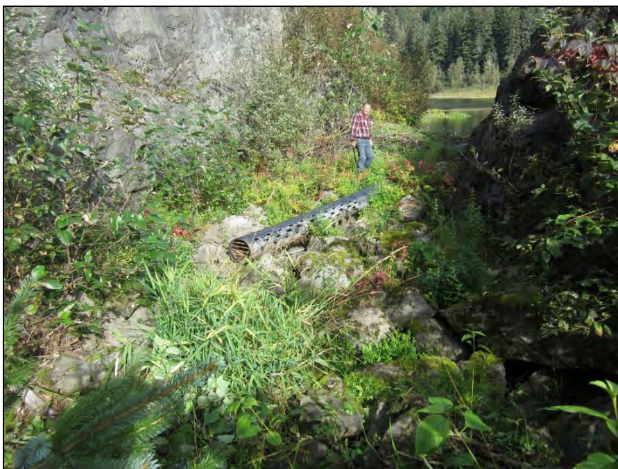
PHOTO 16 – Spillway - Side slopes and beaver protection pipe outlet.
