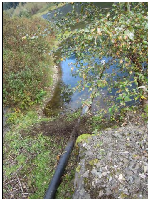
PHOTO 14 – Spillway entrance – site fabricated beaver protection pipe.
