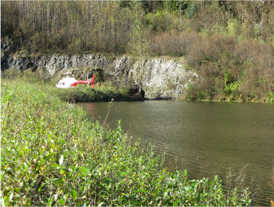
Photograph 3: Spillway Inlet, October 1, 2014
