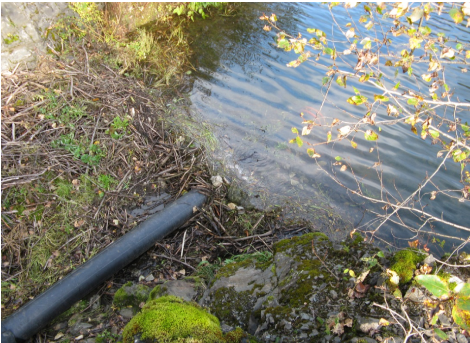
Photograph 4: Beaver Dam in Spillway with bypass pipe in center of spillway, October 1, 2014
