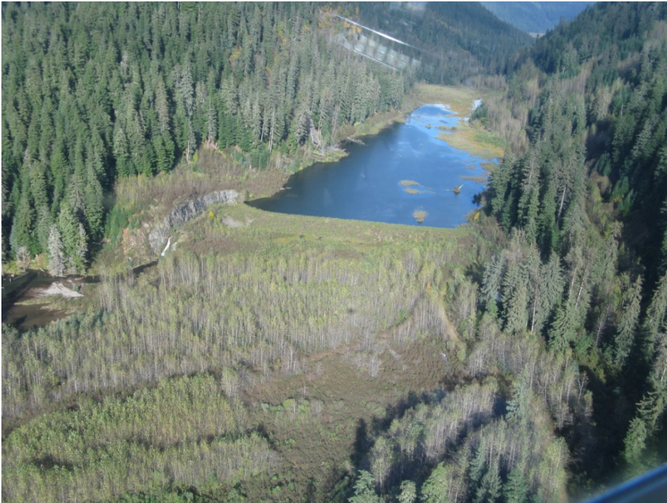
Photograph 1: Site Overview - Dyke 1 In Foreground, October 1, 2014
