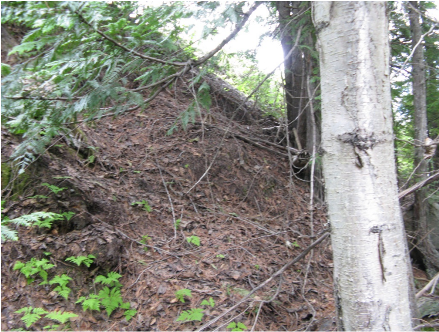
Photograph 3: Downstream slope Pond 1 from toe area – tree covered
