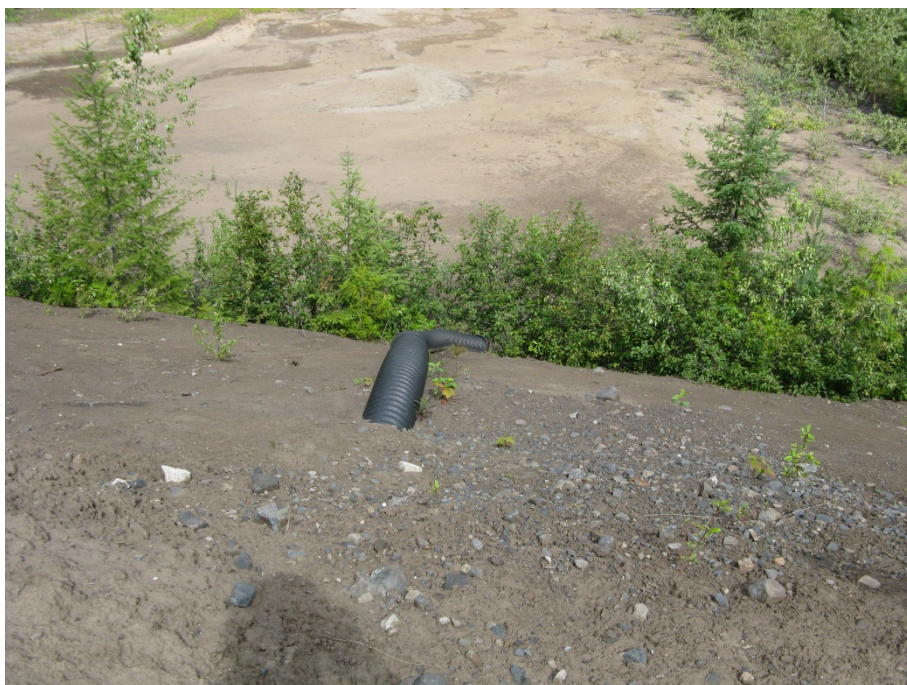
Photograph 6: Downstream Face of Pond 1 – Pond 1 overflow pipe on slope to Pond 2
