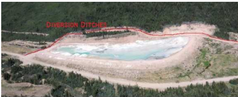
Figure 1 - TSF#1 Aerial view diversion channels
