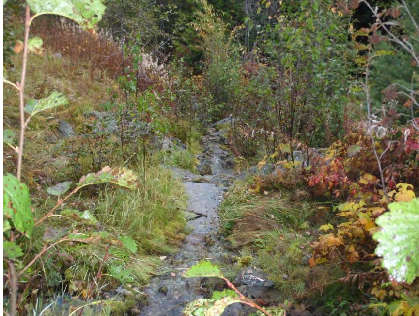
Photo 5. View looking down rediversion from just above first weir below junction of diversion and rediversion.
