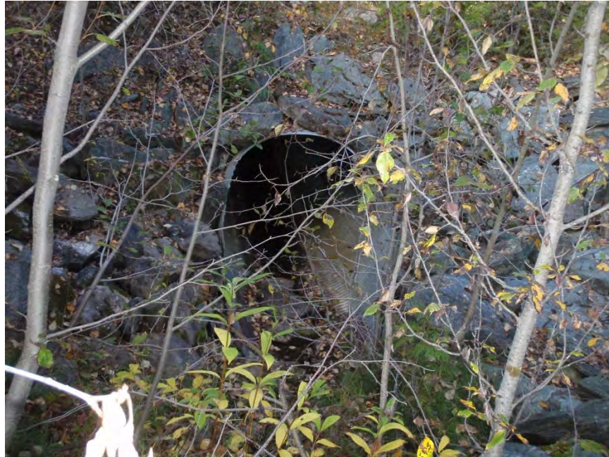
Photo 25. View of the inlet to the culvert under Johnson Lake Road at the bottom of Segment X. Alder saplings are becoming established and should be removed to prevent a buildup of debris.
