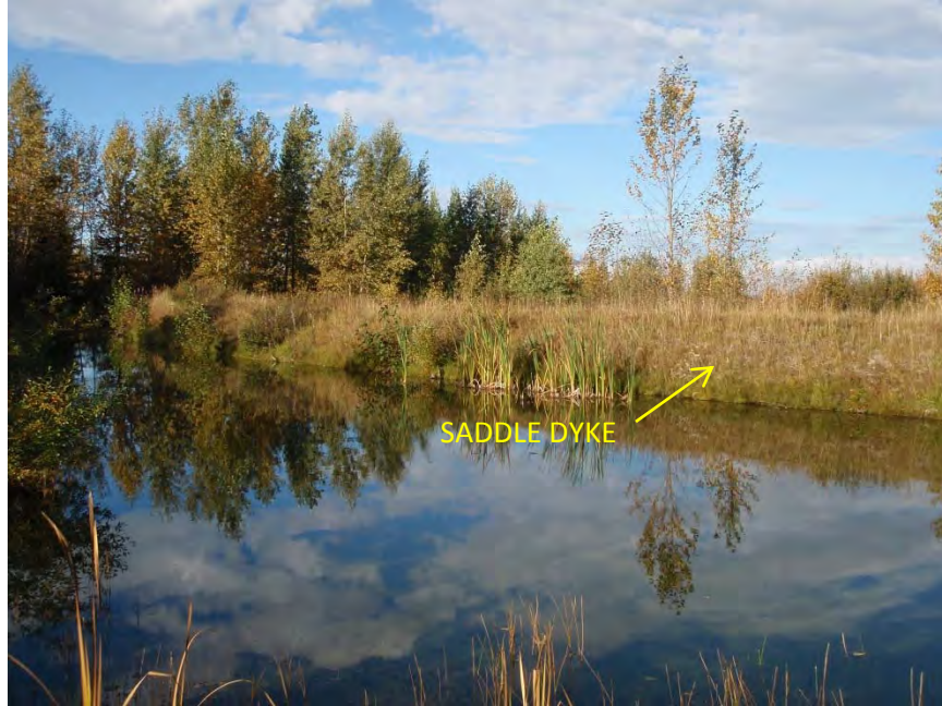
Photo 17. View of approach channel from just downstream of inlet and log boom. Note well vegetated upstream face of Saddle Dyke.
