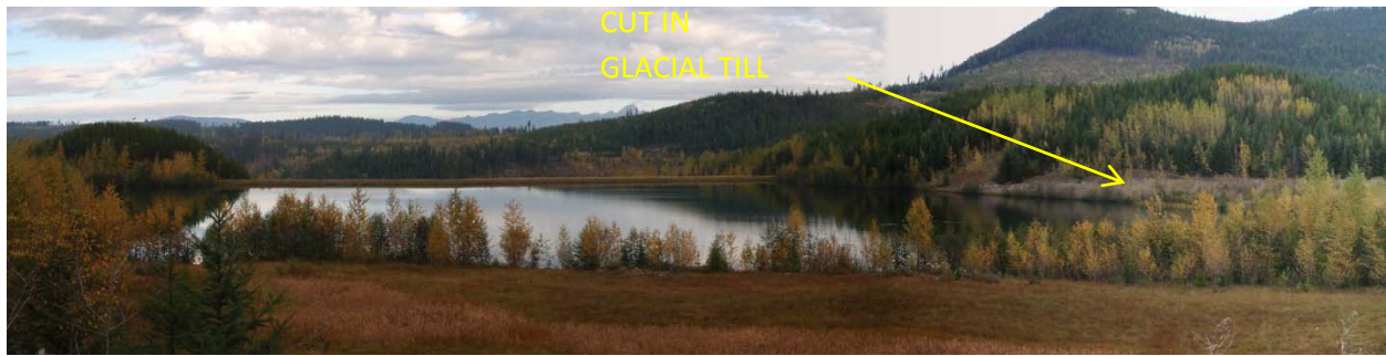
Photo 9. View of tailings storage facility from the point where redirection discharges into impoundment. Note exposed glacial till on the northwest shore on the right side of the photo. No evidence of instability or significant erosion. No work warranted at this time.
