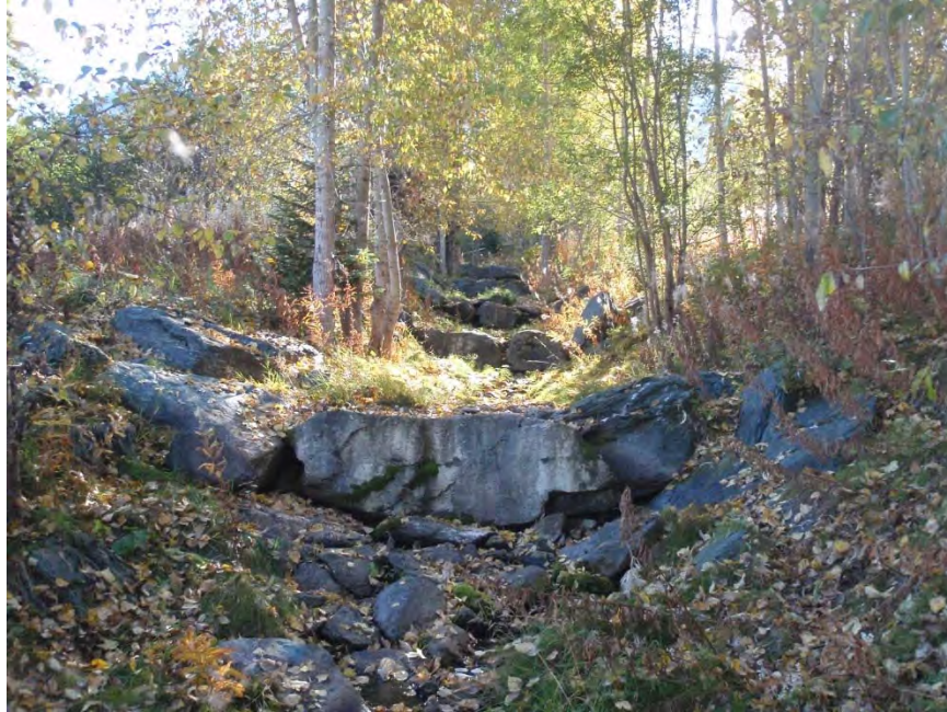
Photo 19. View looking up Segment VII about 100m below the spillway. Note the cleared channel.
