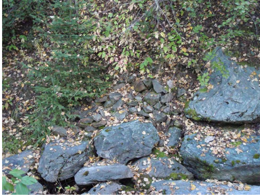
Photo 23. View of hand placed armour on right bank of Segment X. No erosion evident at any of the three locations of hand-placed armour.
