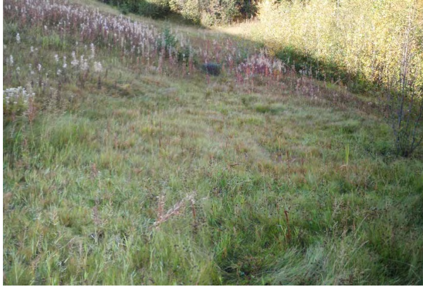
Photo 15. View of historic seepage zone at toe of tailings dam in vicinity of drainage blanket. Spongy ground and minor ponded water was noted at surface in this area. No work warranted.
