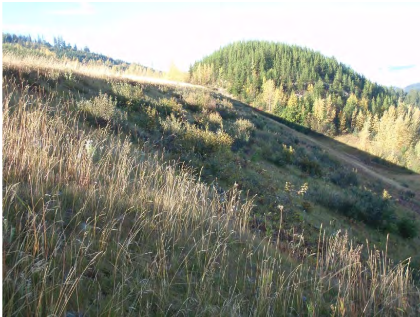
Photo 12. View looking along downstream face of tailings dam from the right abutment.
