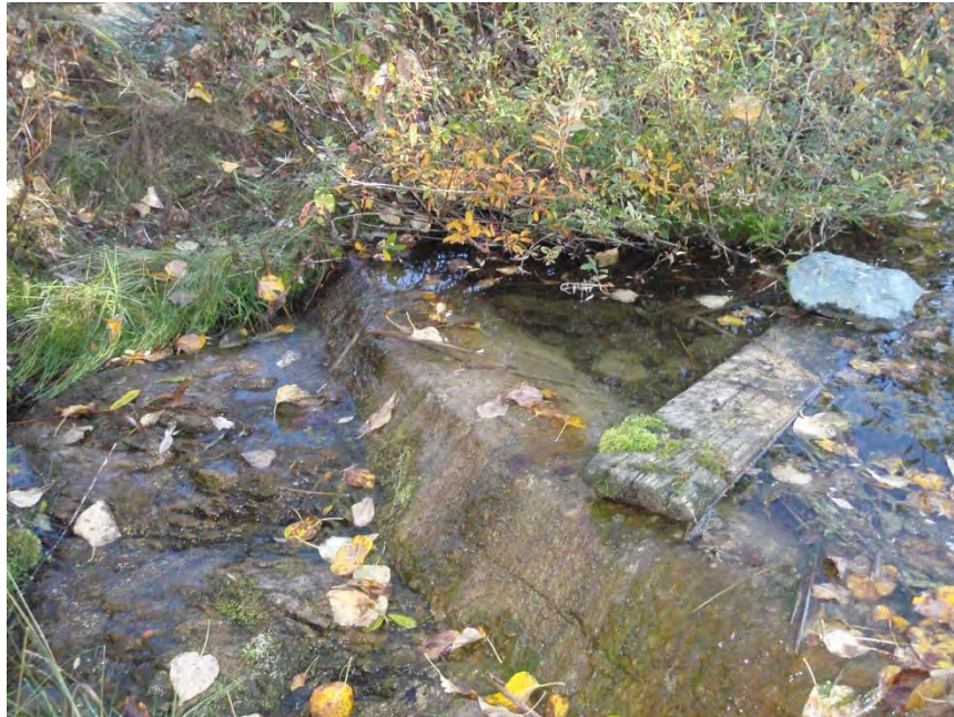
Photo 18. View of spillway weir. Note the water flowing over the crest of the weir.
