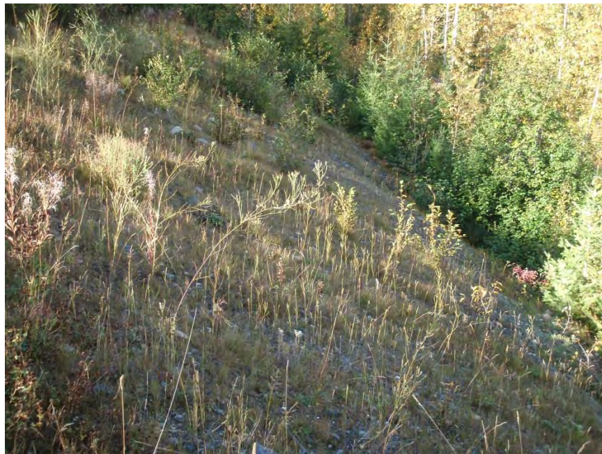
Photo 26. View of portion of resloped area of slope instability noted during previous inspections. Pulled back slope is performing well.
