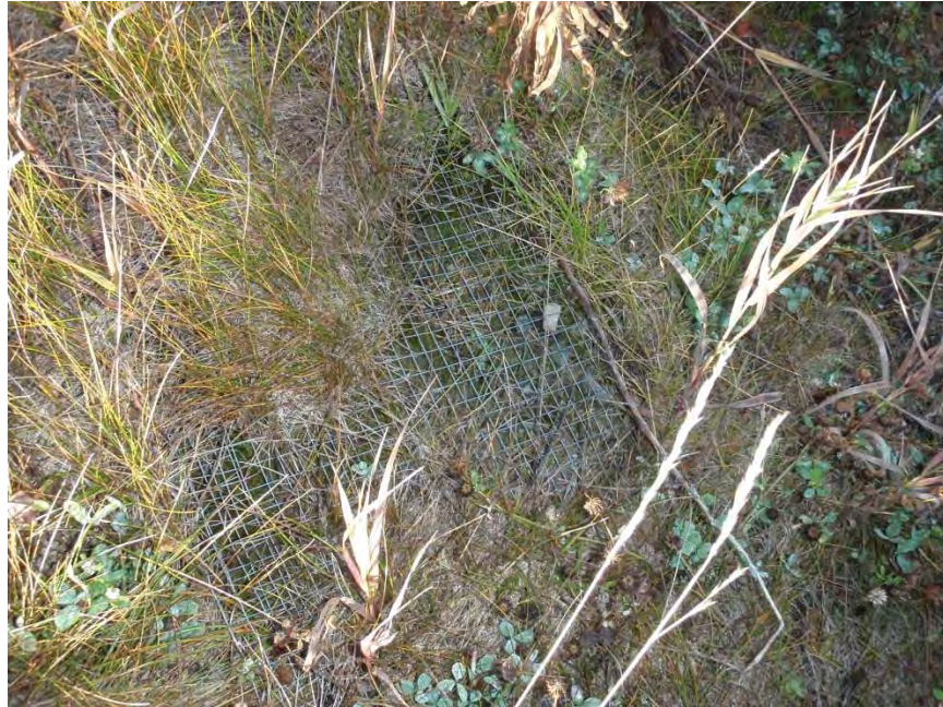
Photo 13. View of a portion of the galvanized mesh placed on upstream and downstream crest to help prevent gophers from burrowing into dam.
