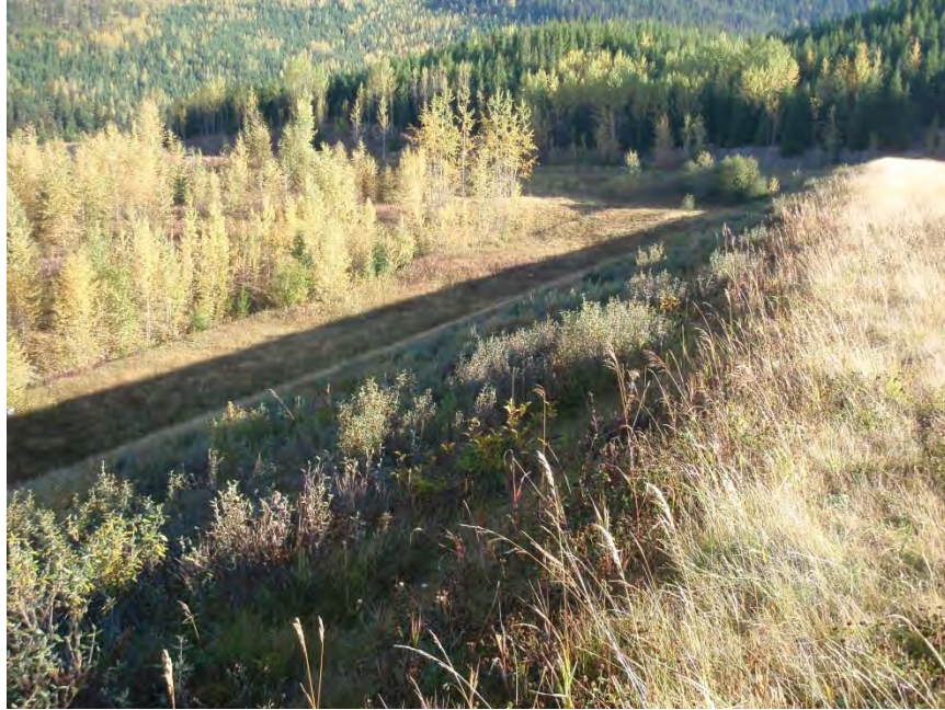
Photo 11. View looking along downstream crest and downstream face from the left abutment towards the right abutment. Note the Buffalo Berry bushes on the face. As noted during past inspections, these shrubs pose a limited risk and do not impede the ability to conduct a visual inspection of the dam. No work warranted.
