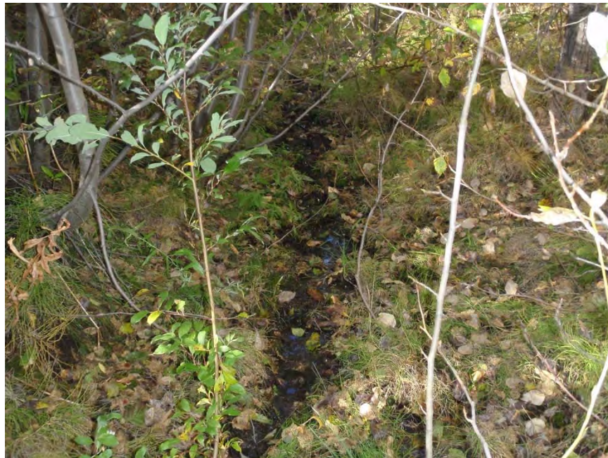
Photo 28. View of ponded water in seepage collection ditch below toe of tailings dam.
