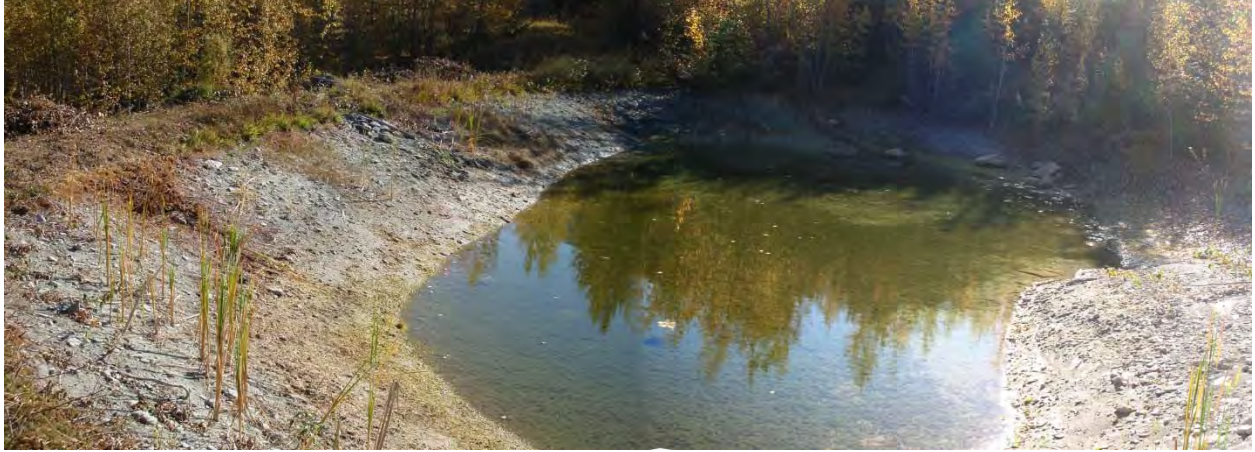
Photo 27. View of plant site sedimentation pond. No significant change since last inspection, except vegetation on dyke has been removed.
