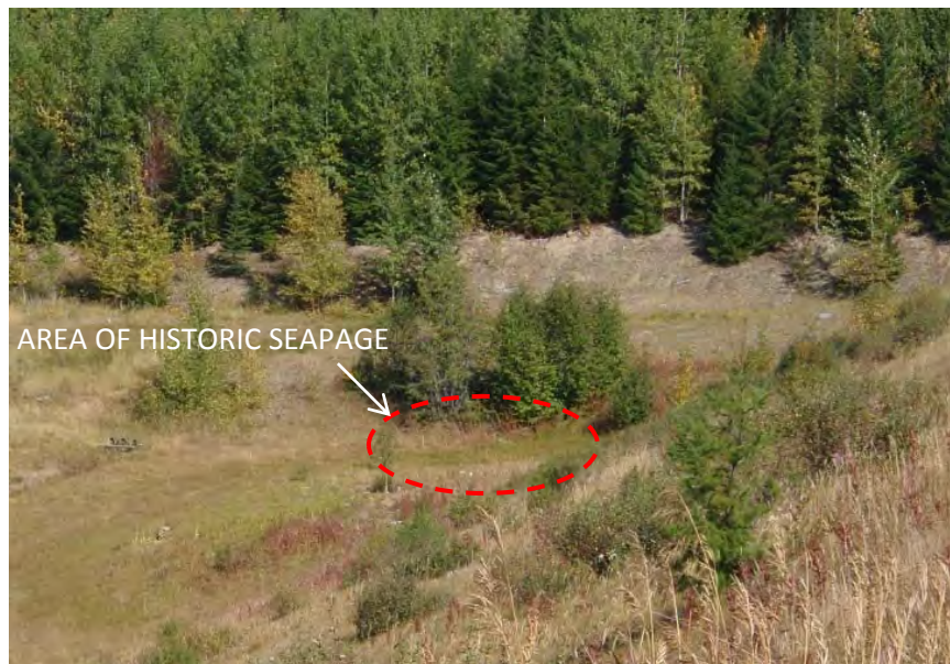
Photo 14. View of area of historic seepage and rutting on right abutment. No work warranted.
