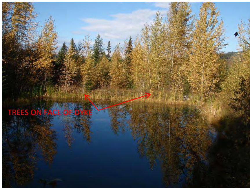
Photo 30. View of the water quality pond dyke. Note large saplings near waterline on upstream face of dyke that pose limited hazard to dyke stability and do not impede visual inspection. Removal of saplings not warranted at this time.
