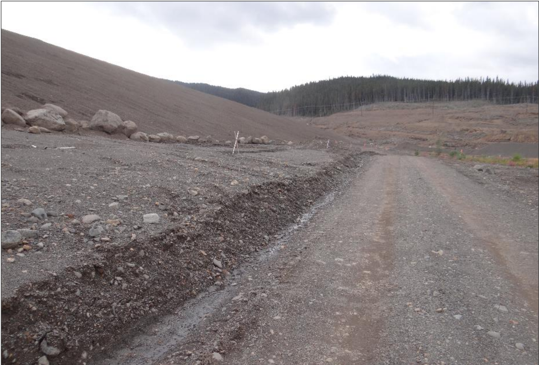
Toe of NSD, looking west towards the left abutment. Drainage blanket adjacent to access road. Seepage in the ditch along the road visually estimated at less than 0.1 litres/sec.
