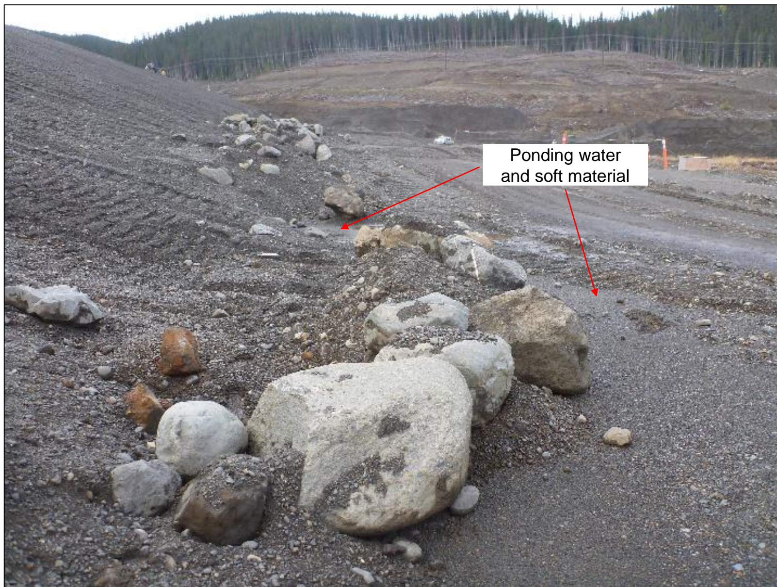
Chainage 0+325: Ponding water and saturated material at toe of dam, not visibly flowing. Appears wet for ~5 m where downstream toe meets blanket drain. Footsteps appear wet once stepped on. Looking west.
