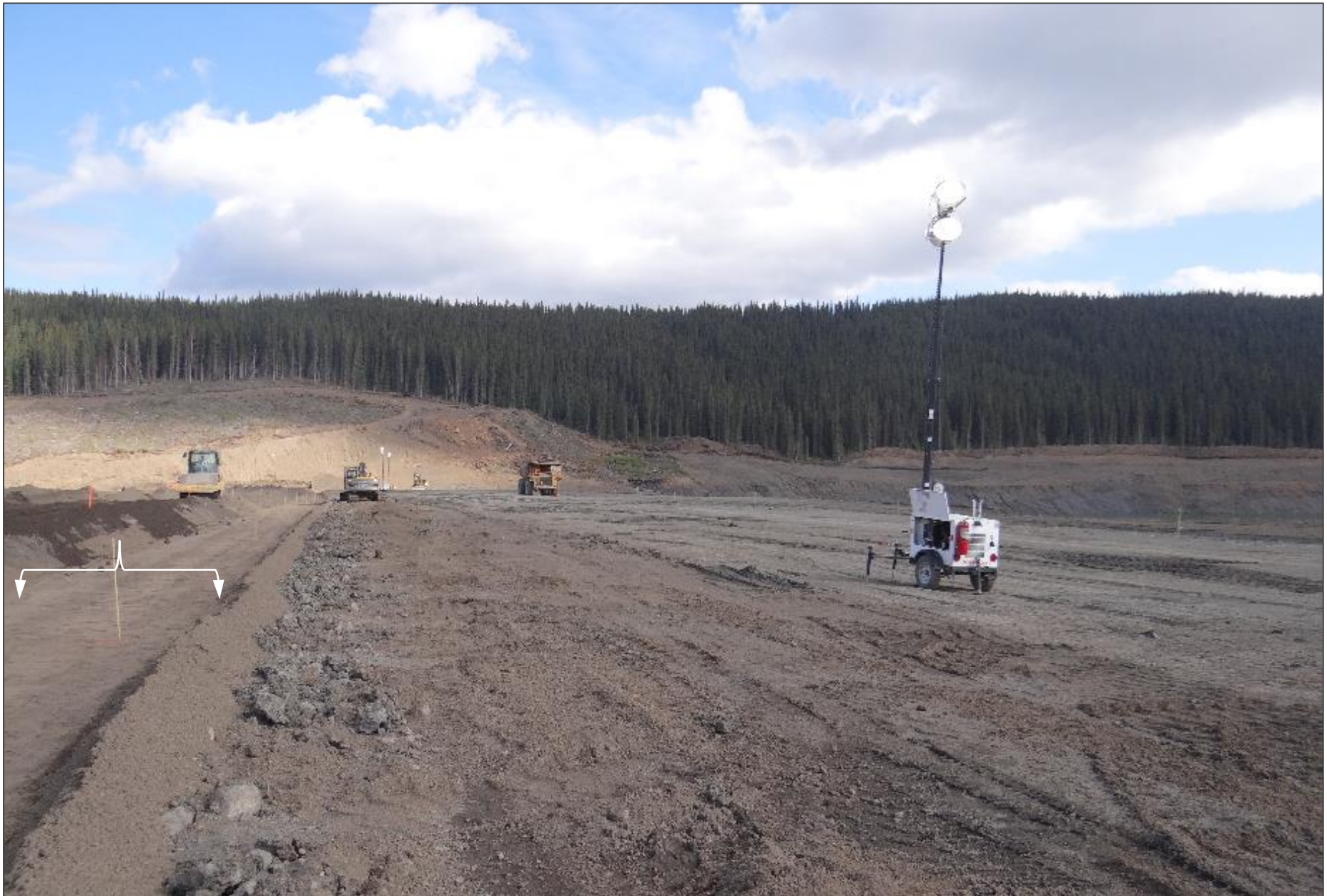
Crest of the NSD. Smooth drum vibratory roller working on Zone 3 b chimney. Bracket indicates Zone 3A chimney filter. Light plant situated on Zone 1 till core.
