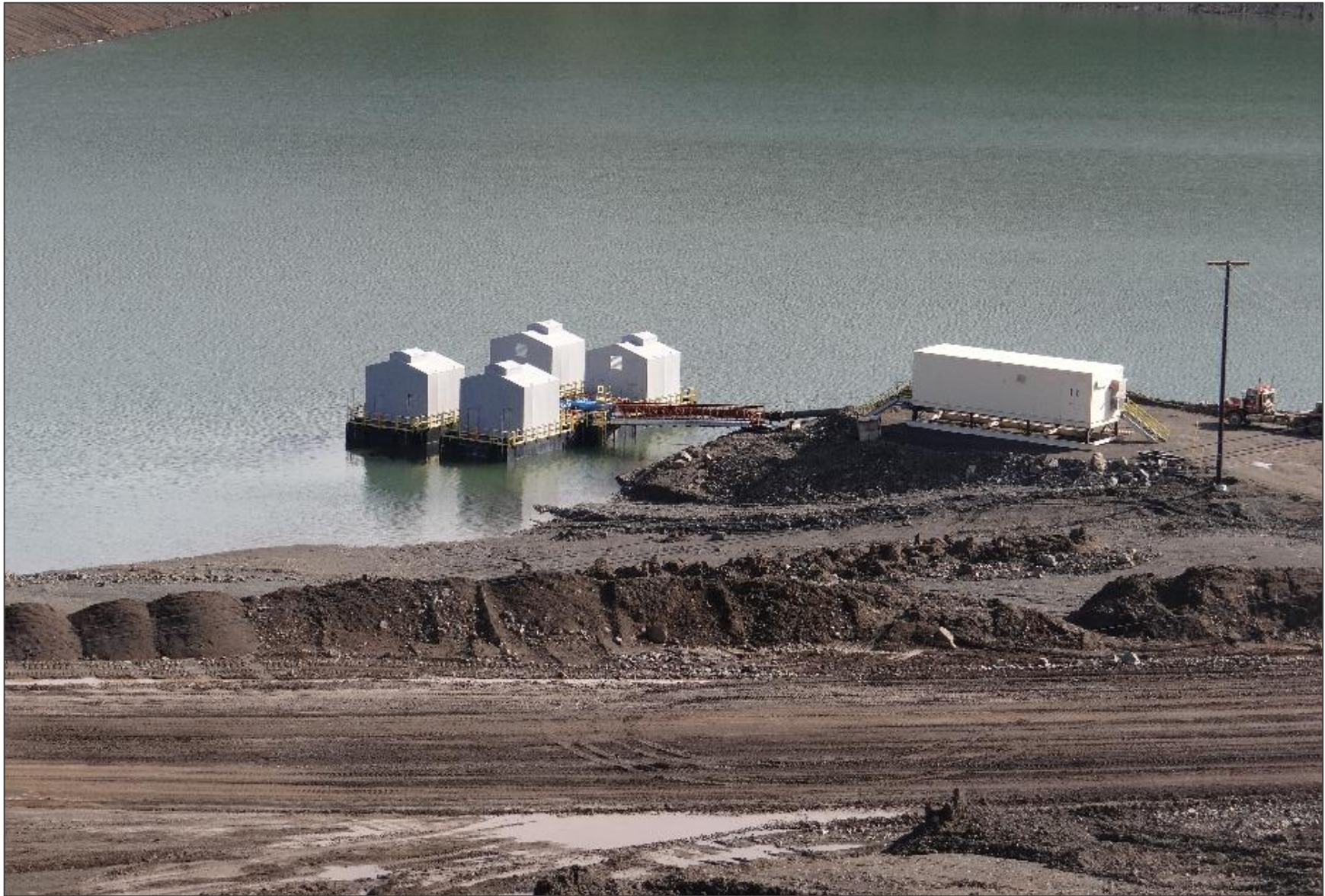
NSD reclaim and surplus water discharge pump barges. Not in operation at the time of the dam inspection.
