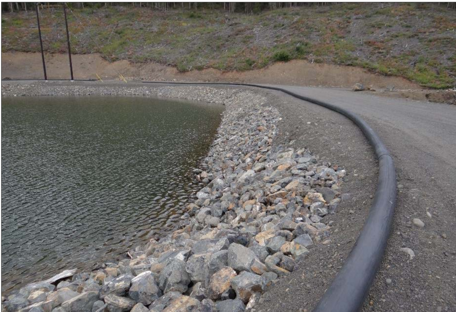
Looking west along the NRD crest and upstream slope, towards the left dam abutment. Pipeline is for pumpback from the NRD reservoir to the NSD reservoir. No indications of upstream slope instability or crest settlement. No indications of riprap instability.
