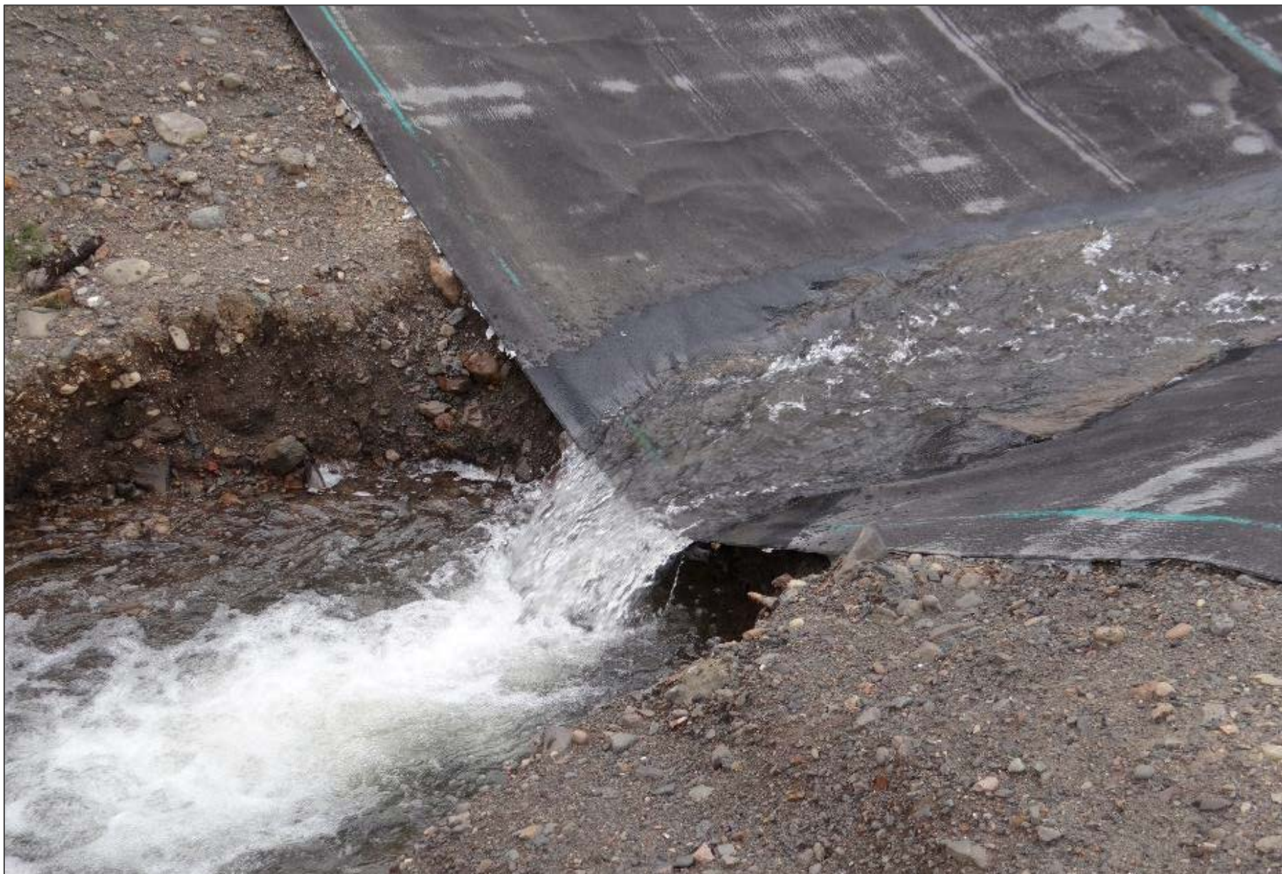
Outlet of the NRD spillway channel. The channel outfall and outlet structure has not yet been constructed, with the result that there is scour occurring and the geomembrane is being undermined. These works need to be completed and the existing scour repaired.
