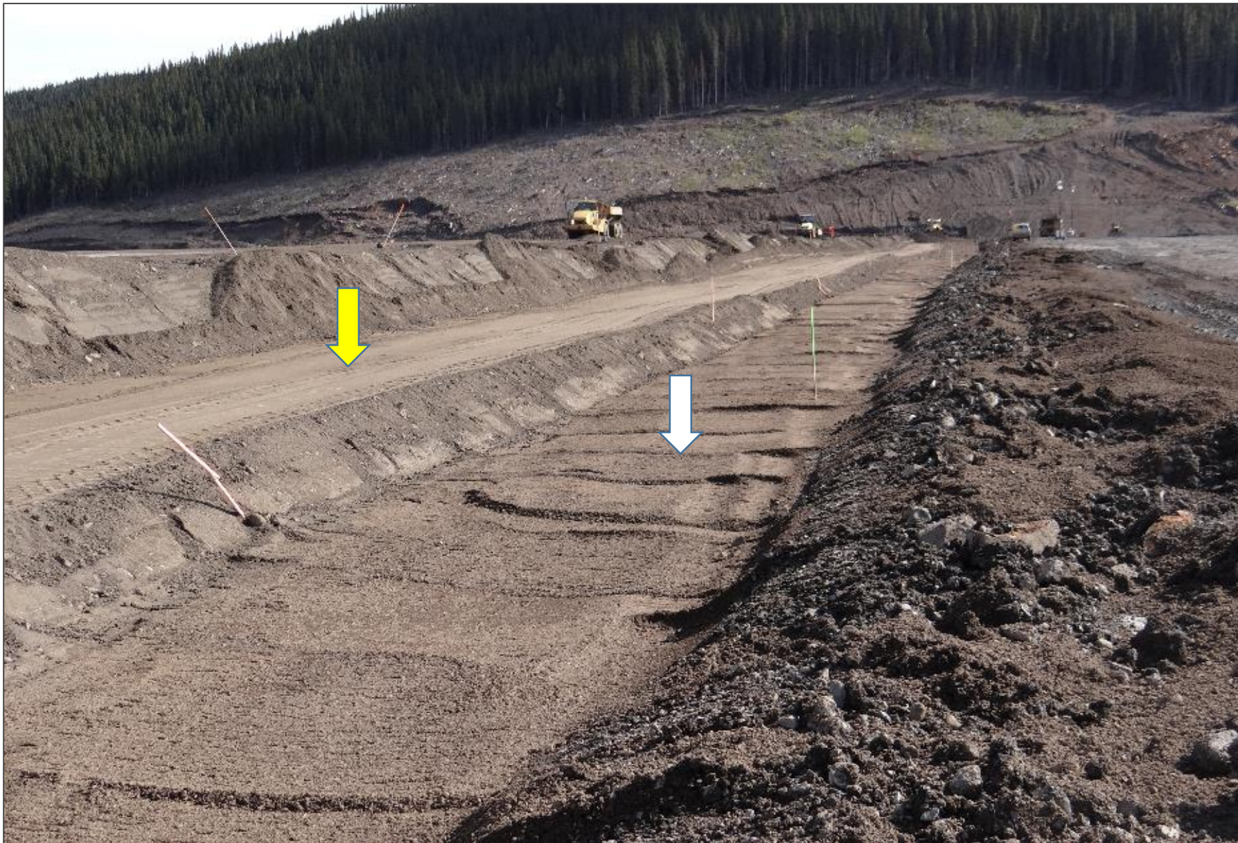
Crest of the NSD, looking east towards the right abutment. Zones 3A and 3B indicated by white and yellow arrows respectively. Waste/spoil on the core (to the right of 3A) will require removal prior to core preparation for additional till placement.
