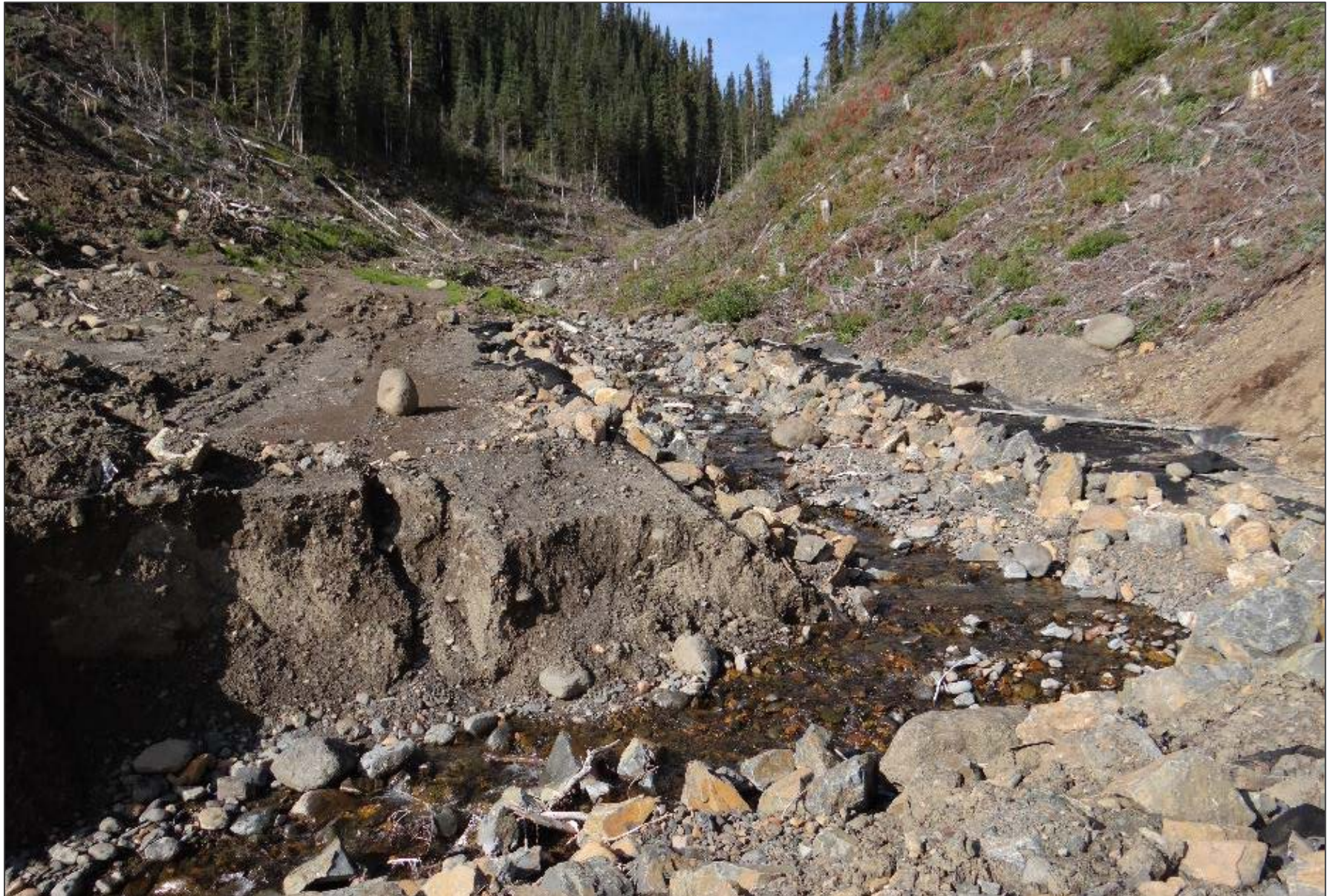
Breached diversion embankment in Beaver Creek, to allow flows to discharge into the NSD reservoir.
