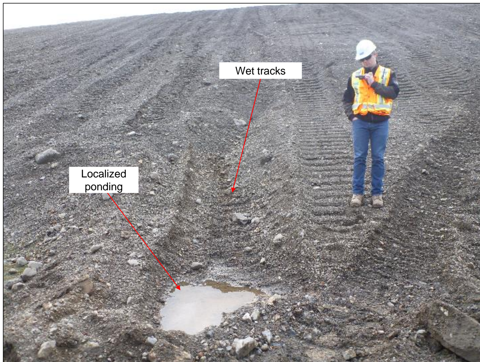
Chainage 0+470: Localized ponding (noted in Photo 2) with visibly wet track marks above. Track mark appeared wetter than others in the area. No flowing water visible. Photo taken at dam toe, looking south.
