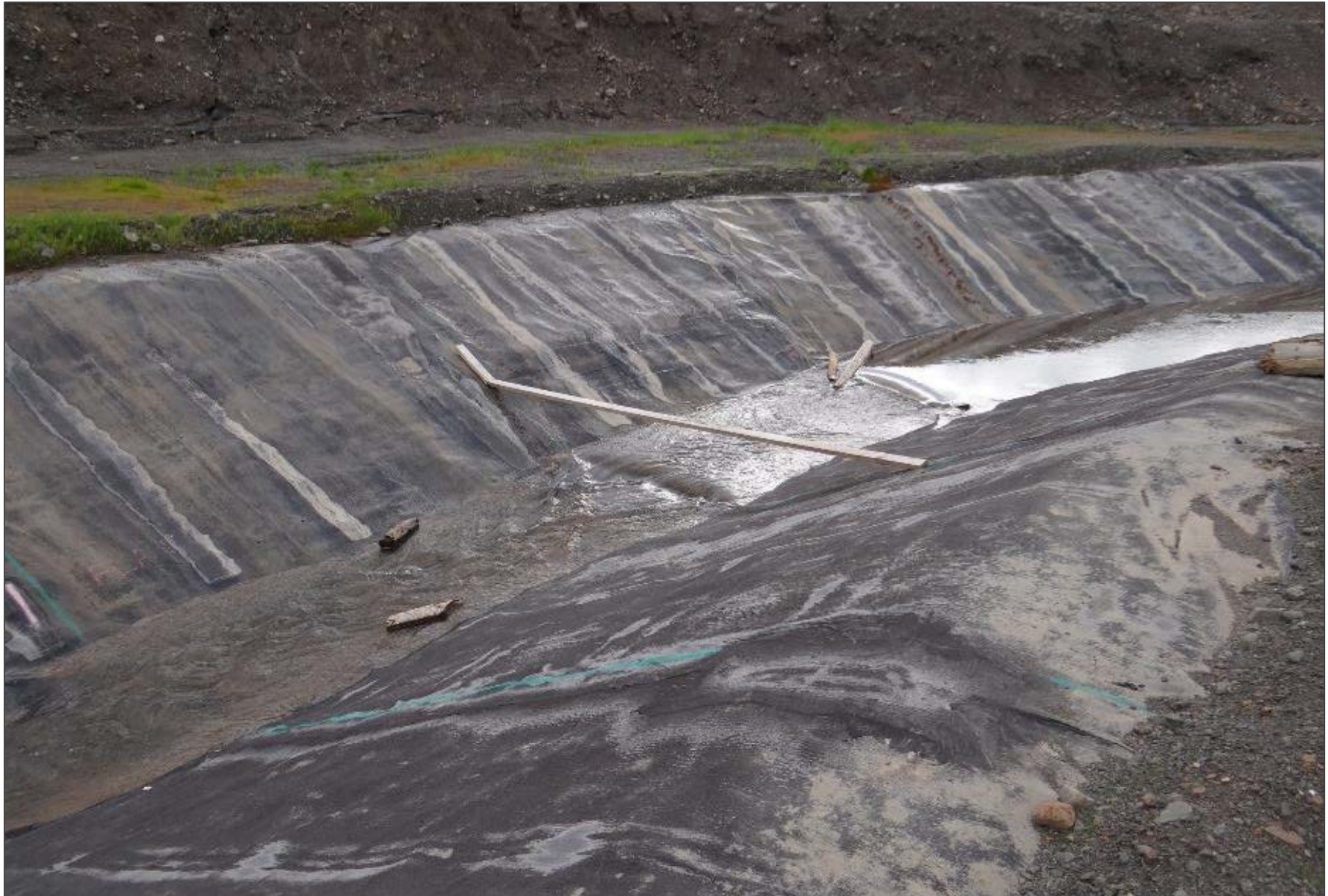
Open channel spillway from the NRD reservoir. Flow rate from the NRD reservoir is monitored continually by RCDC using a datalogger.
