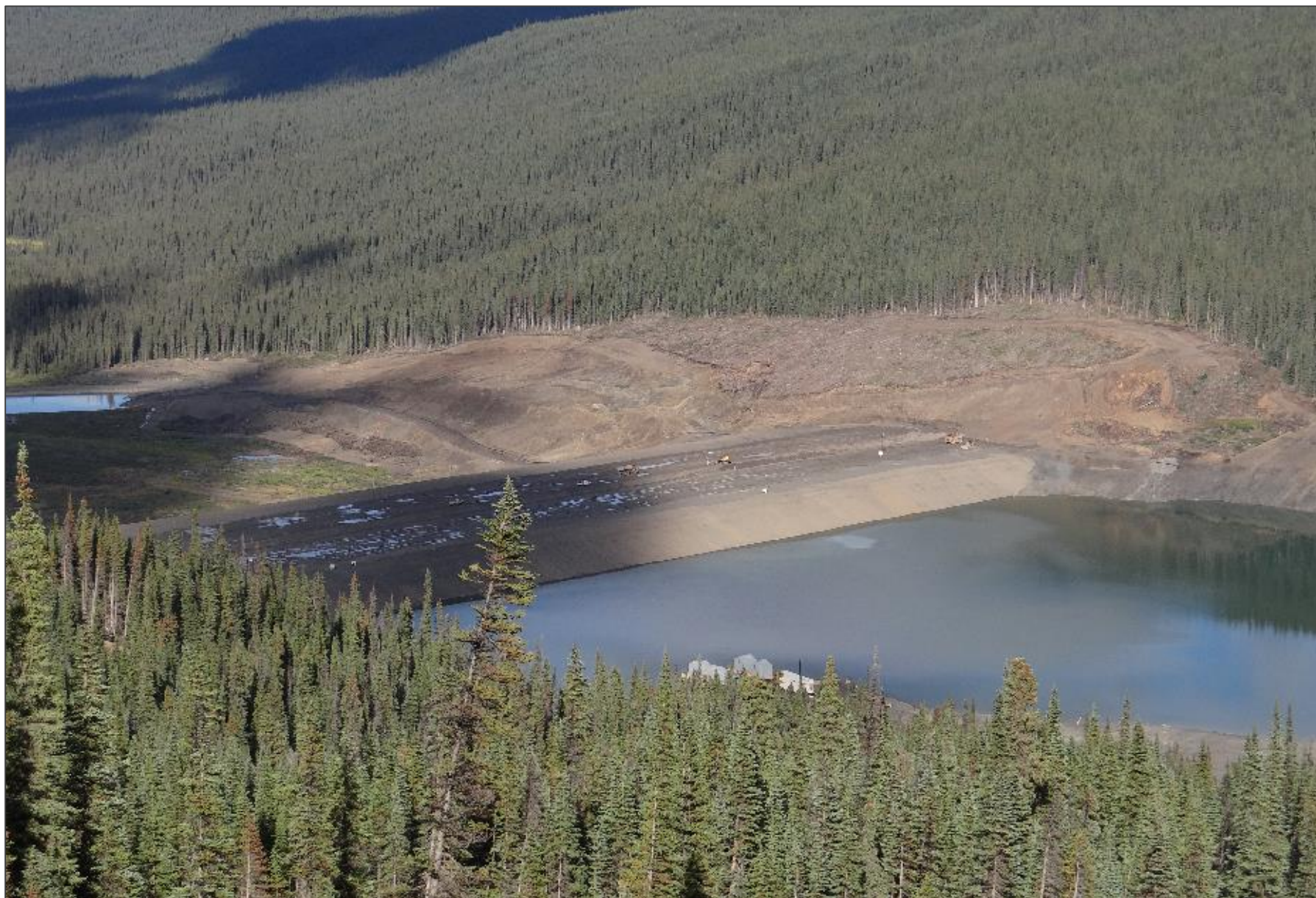
View of the crest and upstream face of the NSD, looking northwest, from vantage point on the TSF access road. Note ponds on dam surface due to recent rainfall.
