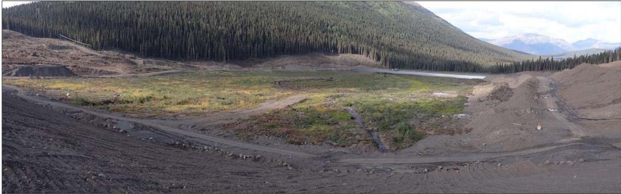
Panorama from crest of NSD near the right abutment, looking downstream towards the toe of the NSD (left), the area of groundwater discharge between the NSD toe and the NRD, and the NRD reservoir.
