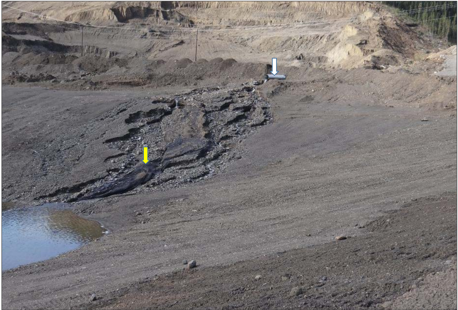
Looking west from the crest of the NSD. Discharge from the culvert (white arrow) represents Beaver Creek flow and pumpback from the NRD reservoir. Note that the discharge has caused erosion damage to the upstream till seepage reduction blanket. Attempt to arrest erosion with geotextile (yellow arrow) has been of limited effectiveness..
