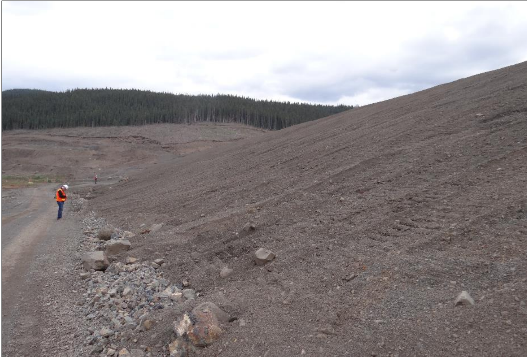
Toe of NSD looking east towards the right abutment. No indications of erosion or instability of the downstream slope of the dam. No indications of elevated seepage discharges on the dam face.
