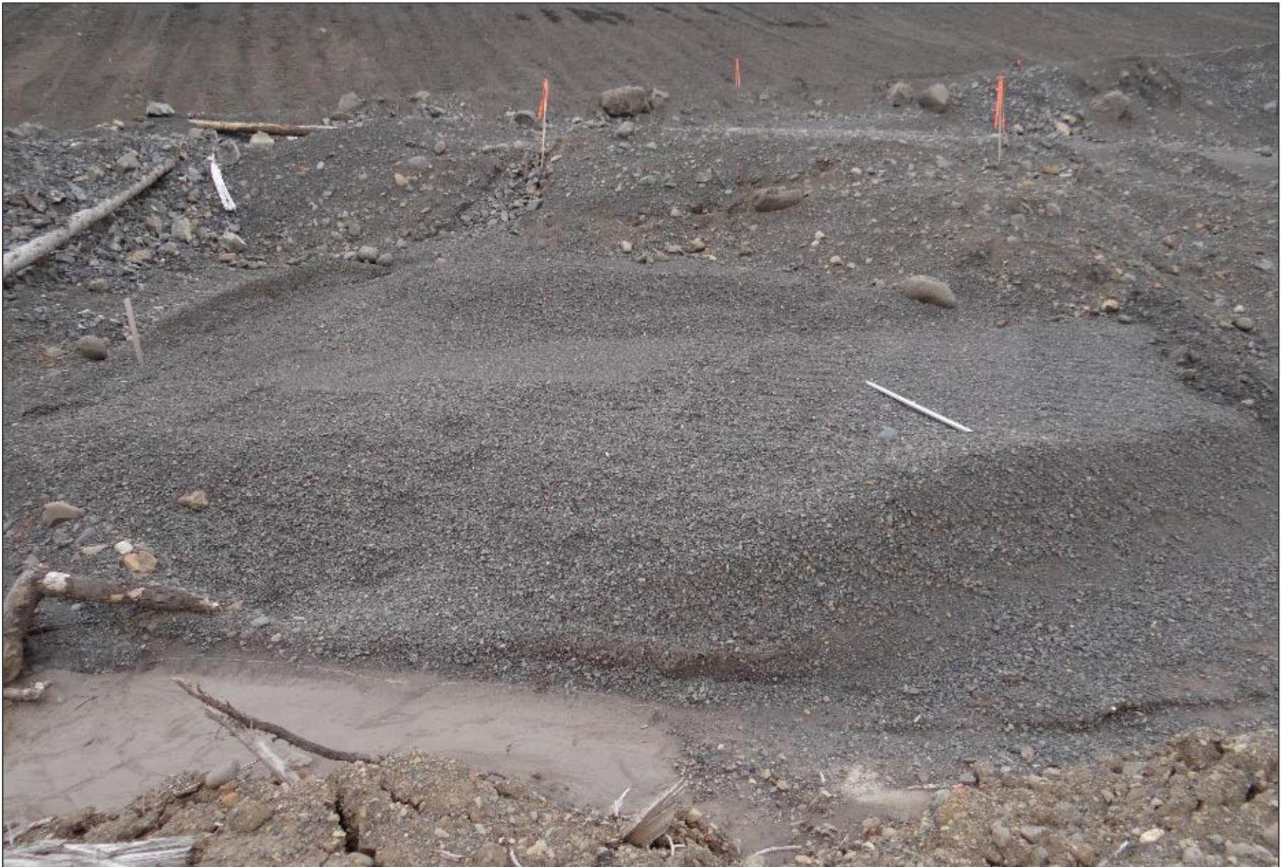
Finger drain 0+500 at toe of NSD near the left abutment.
