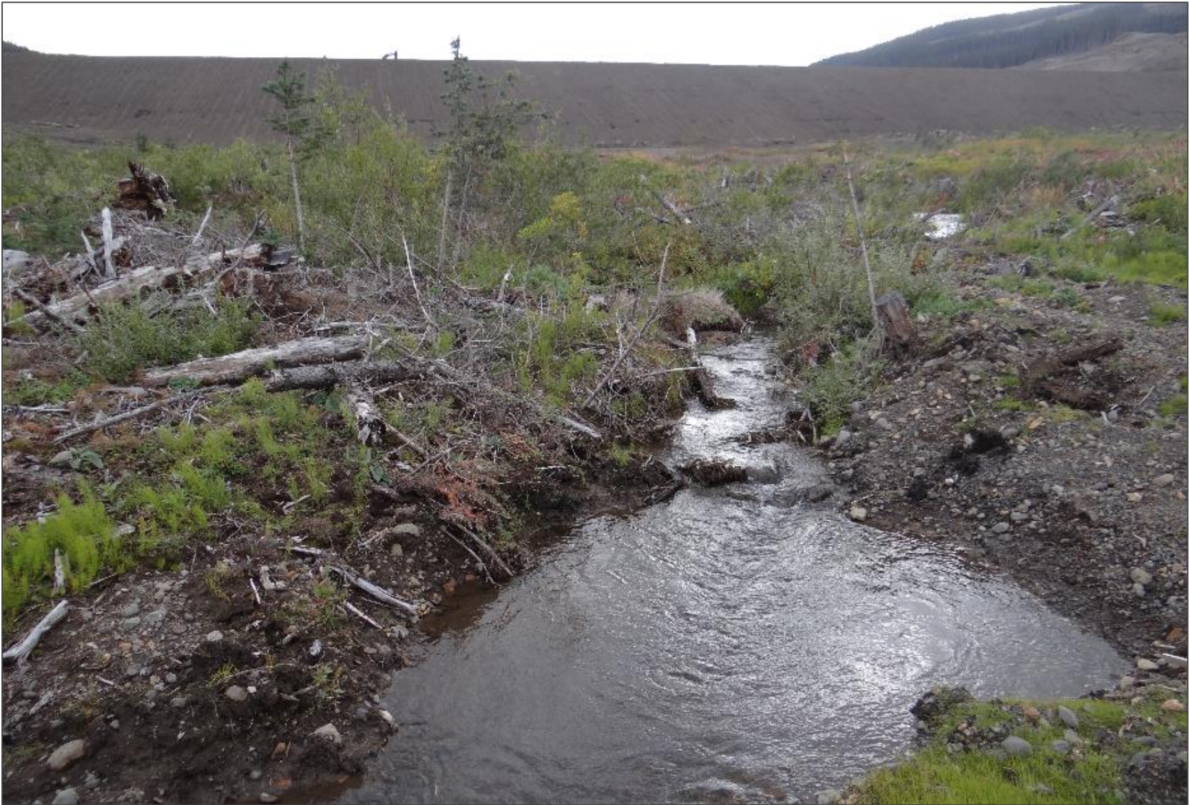
Looking south towards downstream slope of the NSD, again noting increased flows due to groundwater discharge in the area between the NSD and the NRD.
