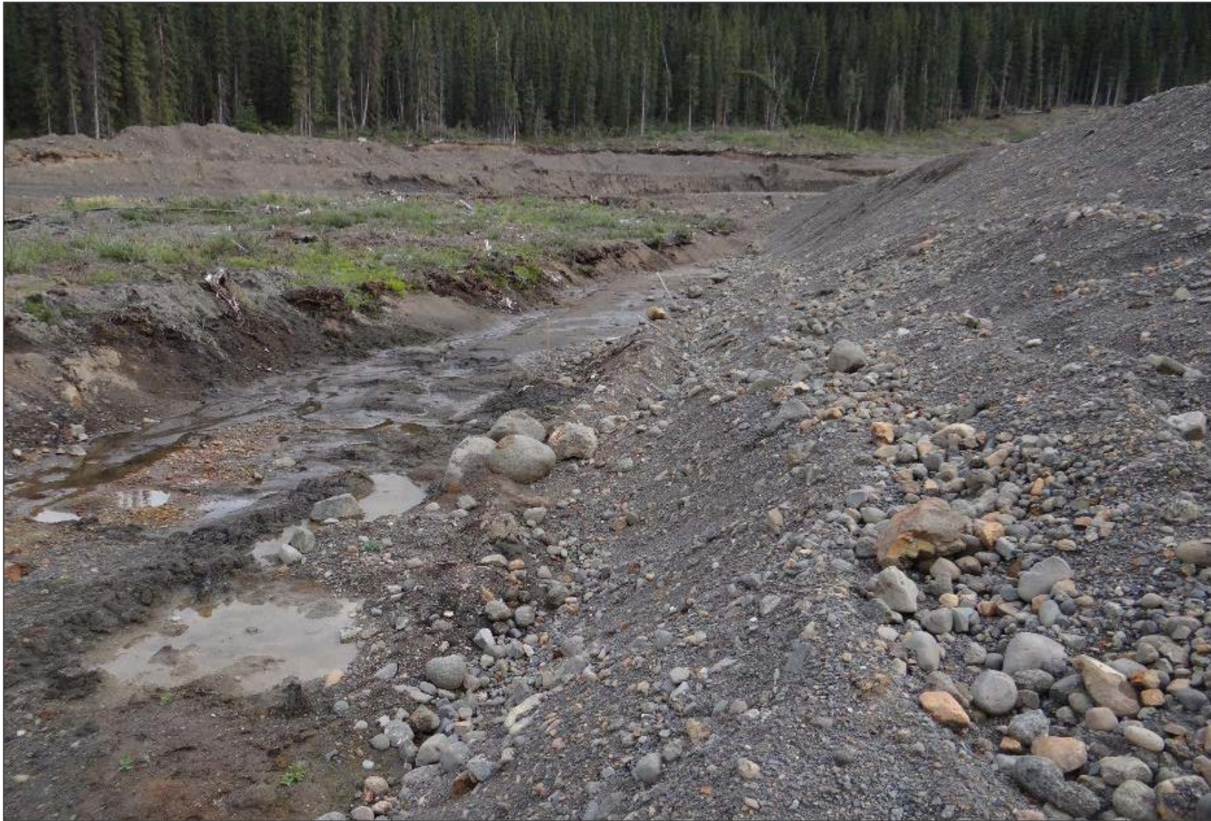
Looking east along the NRD toe and downstream face, towards the right dam abutment. Note wet toe conditions.
