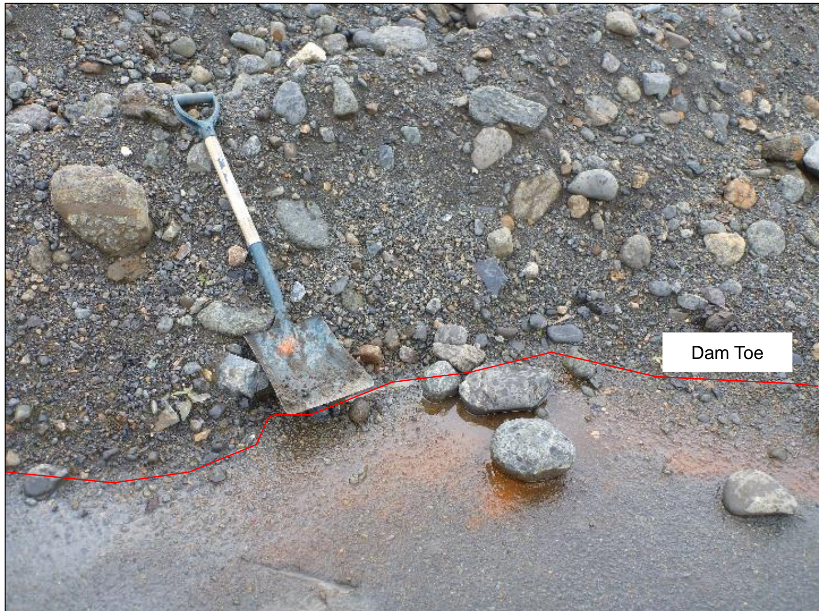
Chainage 0+080: Water observed trickling from dam toe. Orange staining in location of seepage.
