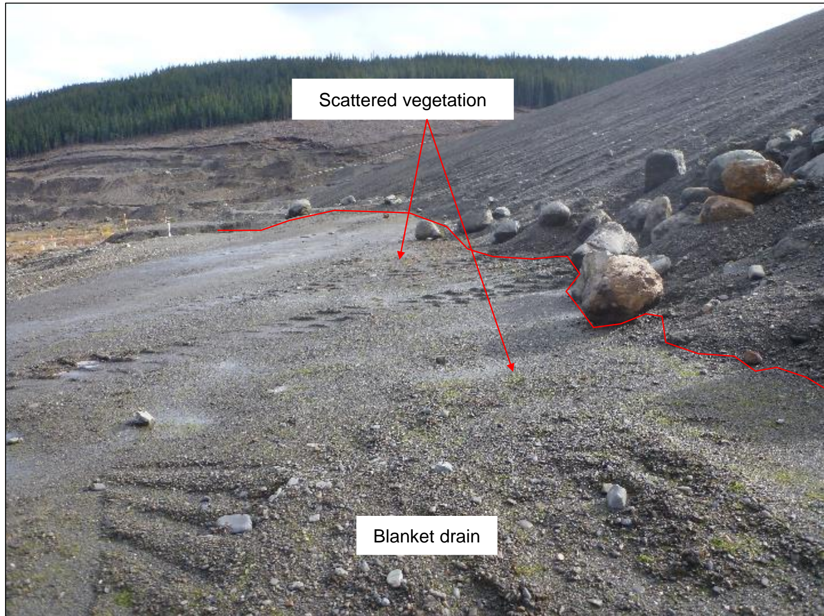
Chainage 0+420: Blanket drain that extends beyond downstream toe appears wet on surface. Small vegetation visible. No flowing water observed. Looking east.
