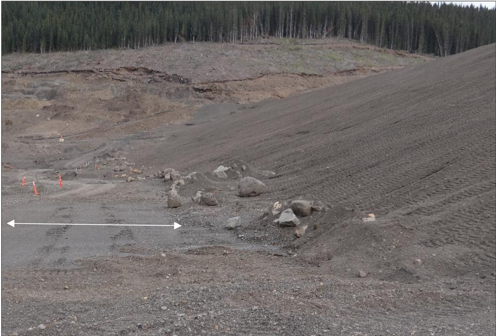
Toe of NSD looking east towards the right abutment. Minimal seepage indicated at the toe of the dam. No indications of erosion or slope instability. Drainage blanket indicated by arrow.
