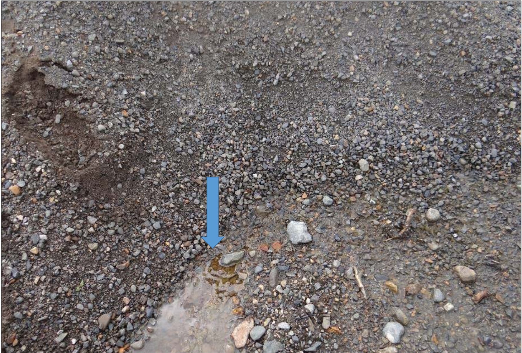
Arrow indicates upwelling seepage at the toe of the NRD – to be remediated via a filter blanket.
