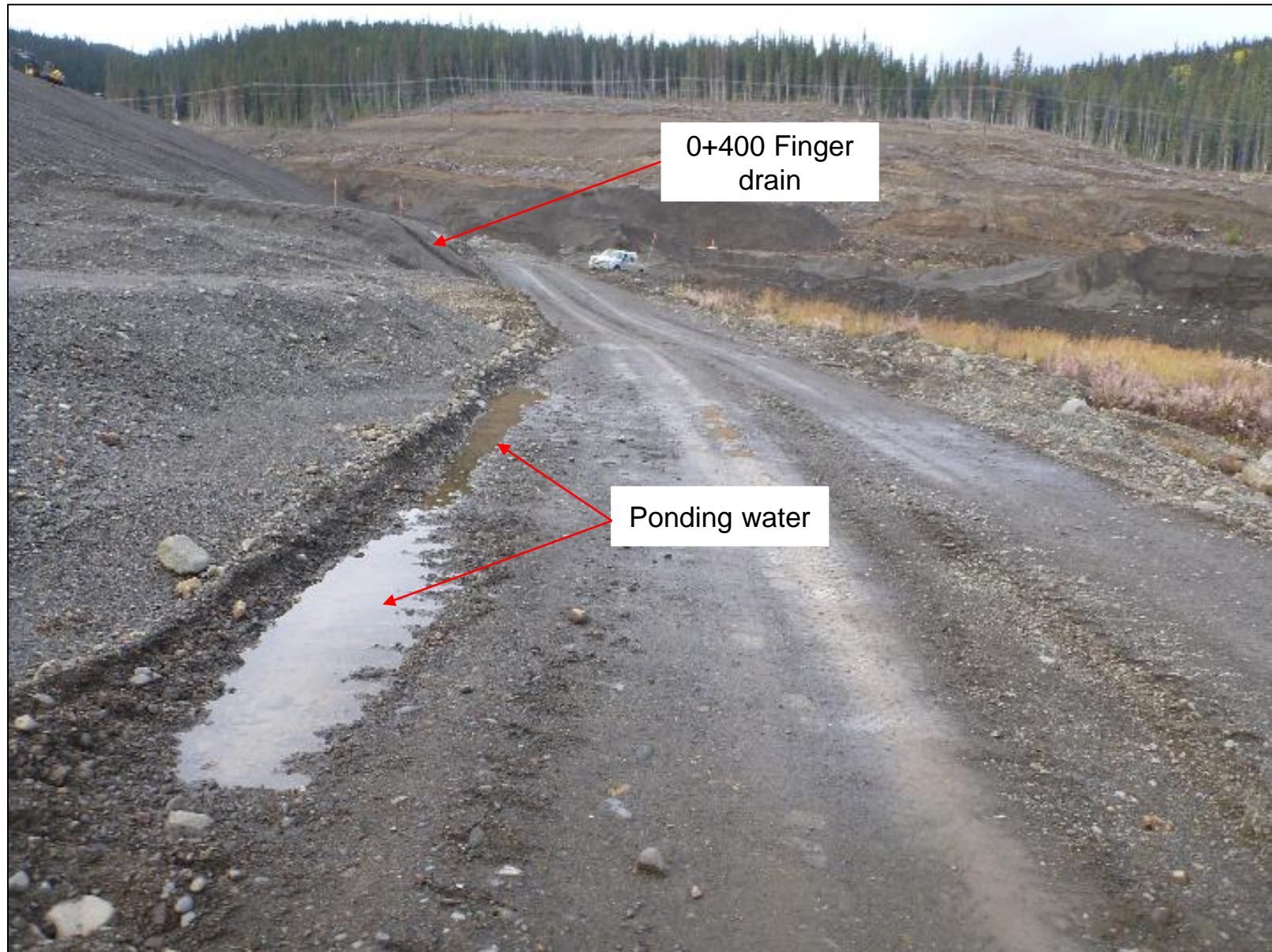
Chainage 0+390: Ponding water at toe of NSD east of finger drain. Extends approximately 8 m along toe. No flowing water observed. Looking west.
