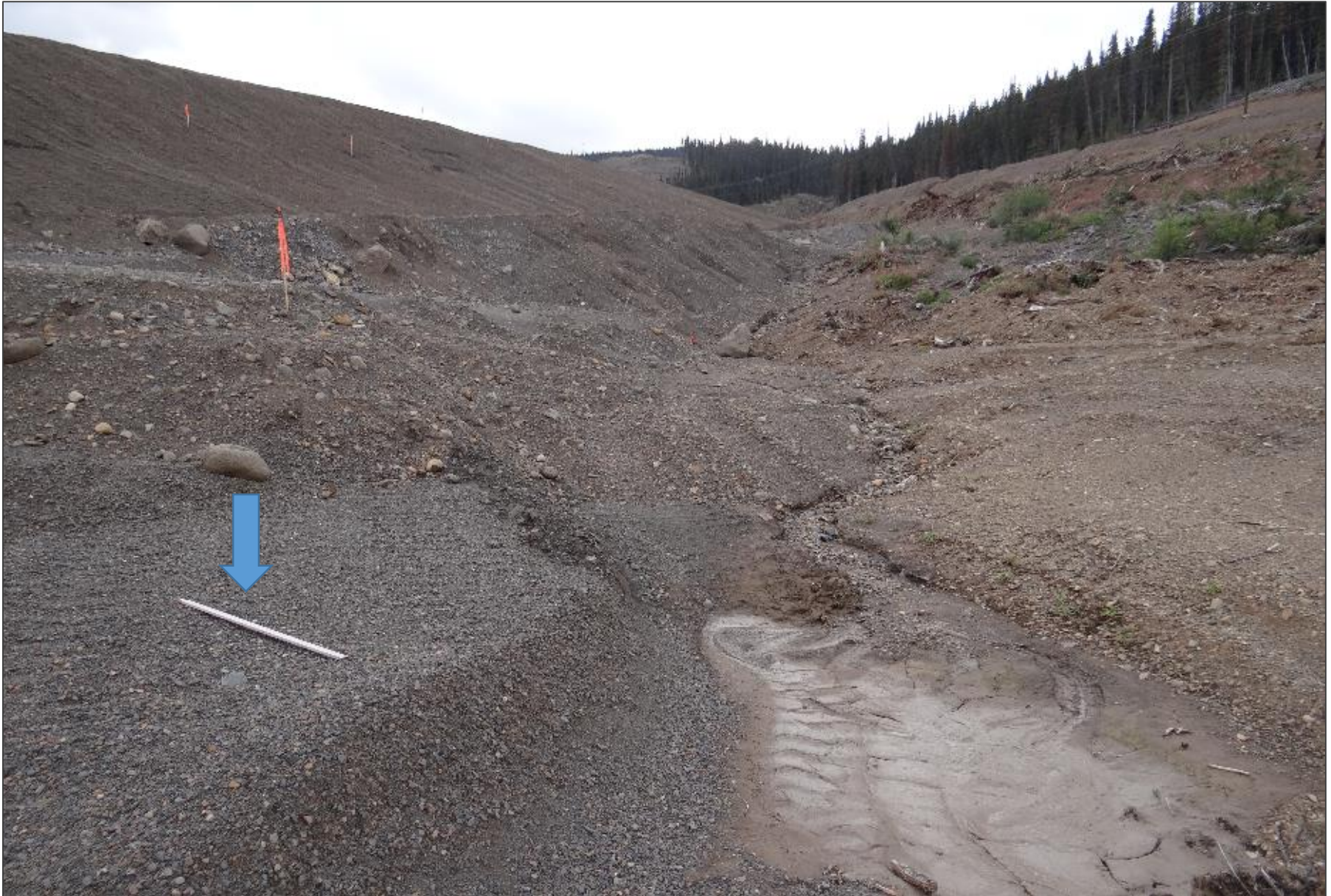
Toe of NSD looking up the left abutment. Finger drain 0+500 indicated by the arrow. Evidence of minor runoff erosion down the abutment, but no visible seepage discharge from the dam.
