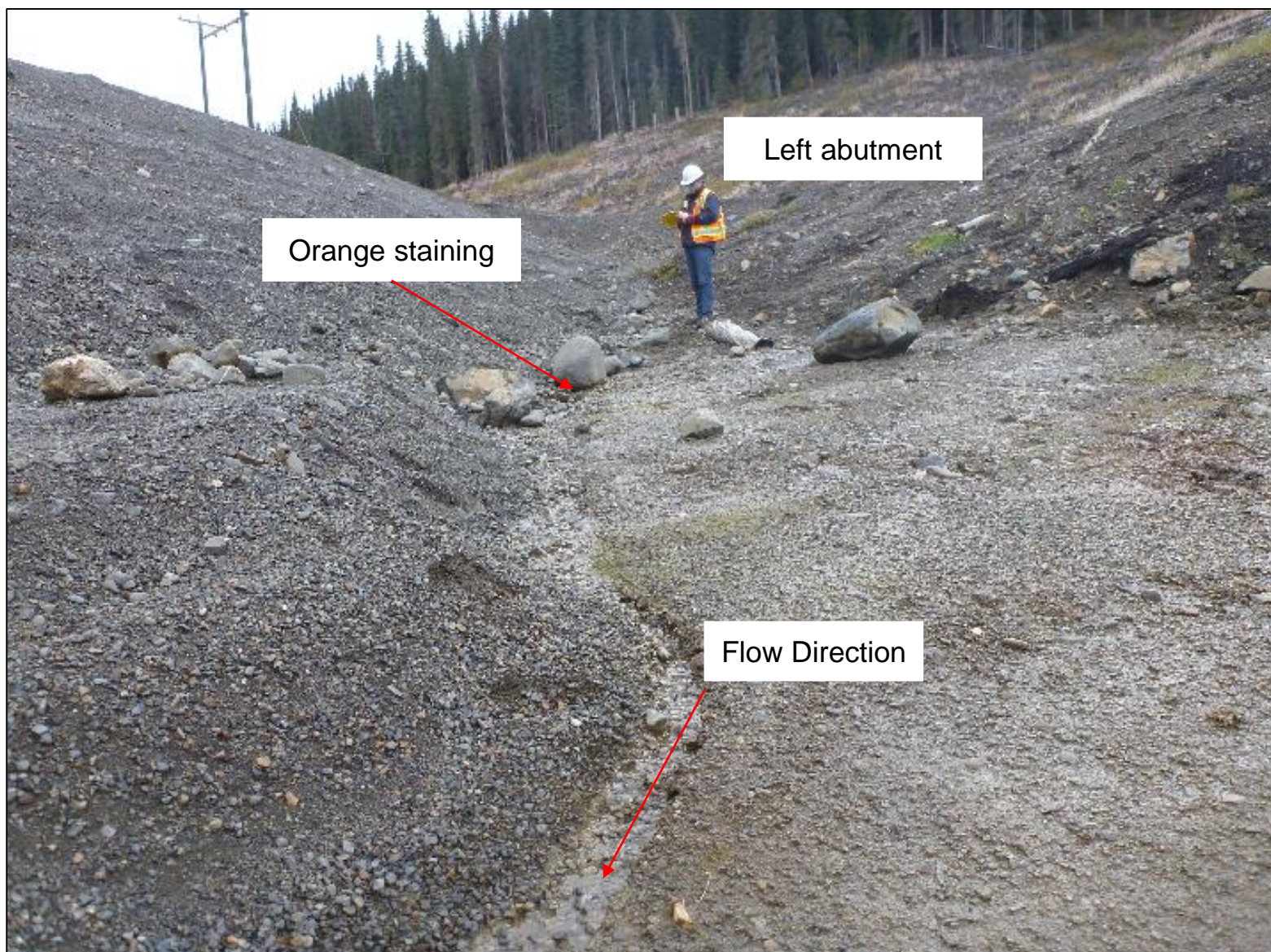
Chainage 0+290: Seepage originating from left abutment, visibly flowing along toe for approximately 50 m. Likely some seepage contribution from toe. Water is clear. Seepage elsewhere not visibly flowing but soil is damp nearby. Orange staining in location of seepage. Looking west.
