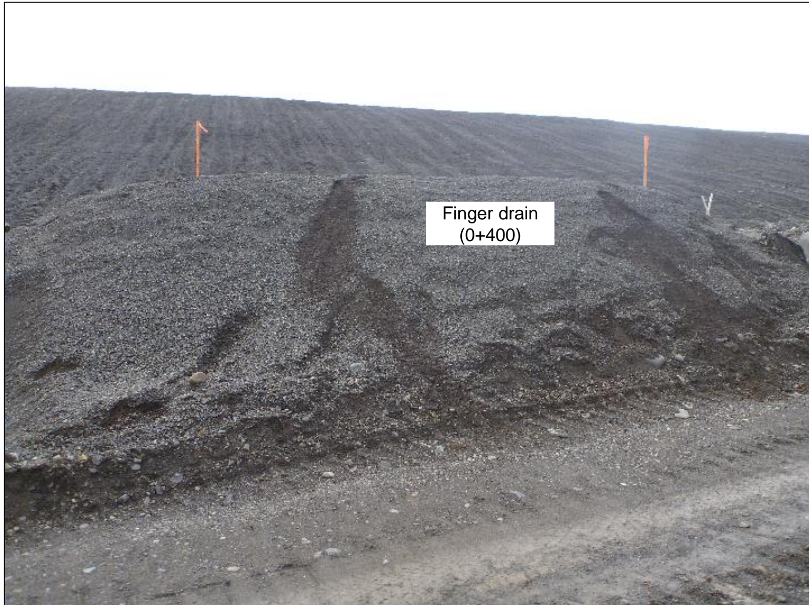
Chainage 0+400: Finger drain with no visible seepage or ponding water. Looking south from access road below NSD toe.
