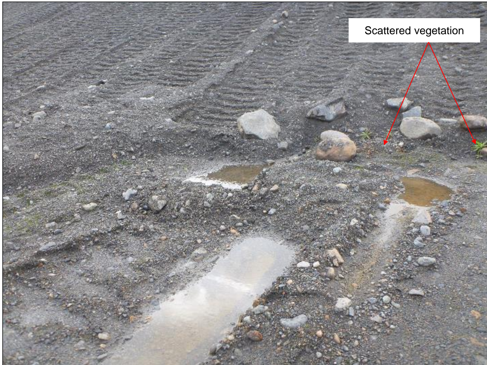
Chainage 0+250: Ponded water where downstream slope meets blanket drain. Footsteps appear wet once stepped on. Looking south toward the downstream toe from blanket drain.
