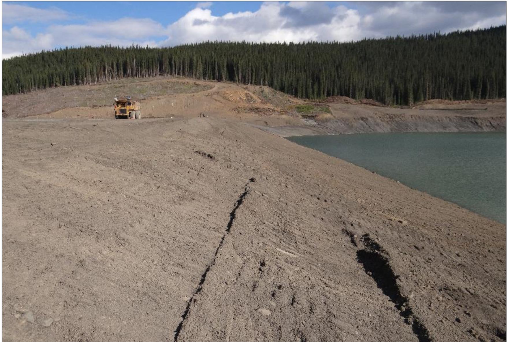
NSD upstream facing, looking east towards the right abutment. No indications of erosion or slope instability.
