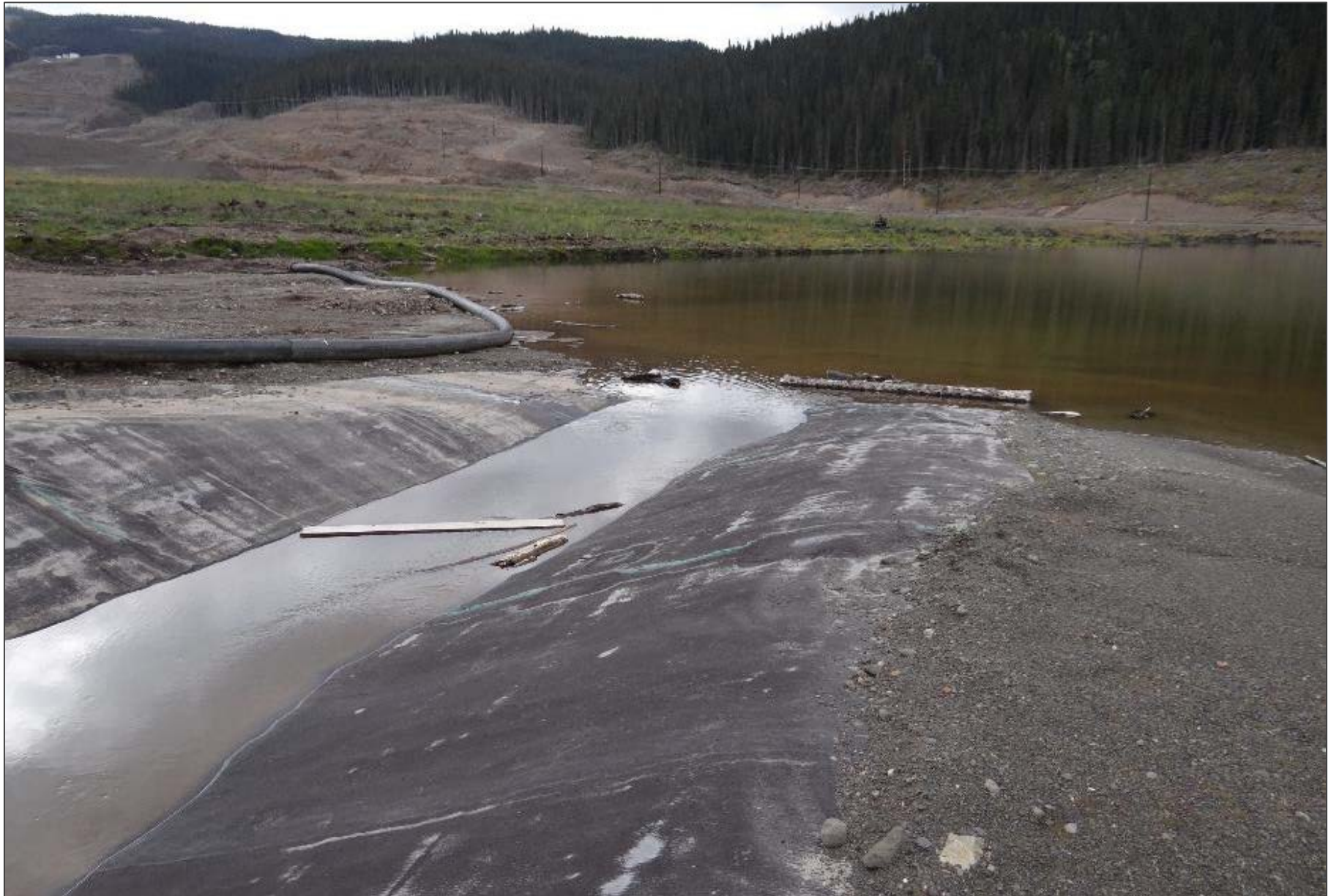
Inlet to the bituminous geomembrane-lined open channel spillway from the NRD reservoir. Note floating wood debris in the reservoir and in the channel. This material needs to be cleared.
