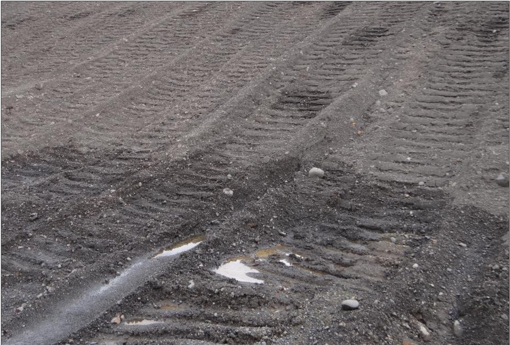
Seepage at toe of NSD, at about Sta. 0+250 m, where slope of the dam meets the drainage blanket. No flow rate discernible. No indications of fines in seepage discharge.
