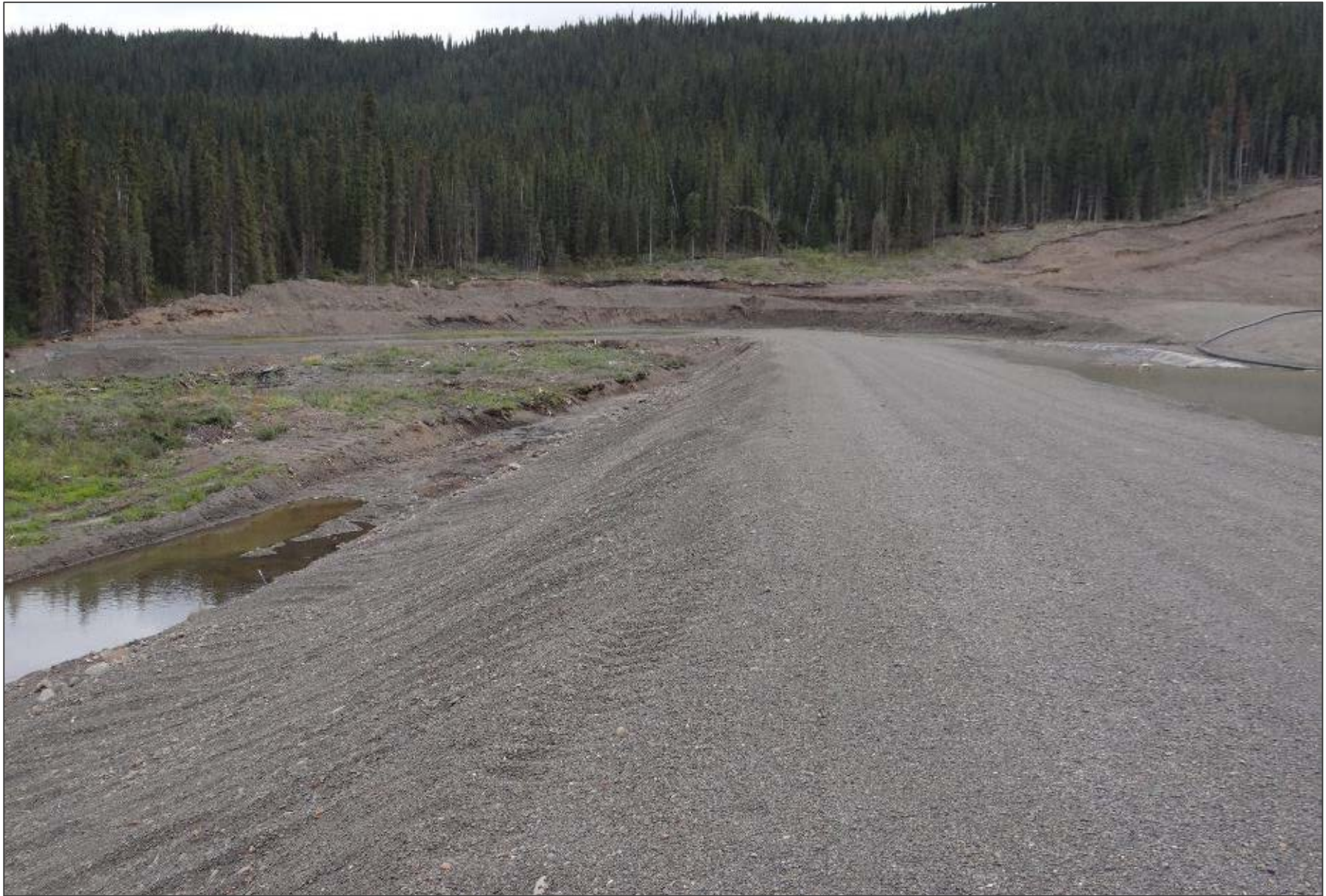
Looking east along the NRD crest and downstream slope, towards the right dam abutment and overflow spillway. Note ponding water and wet conditions along the downstream toe.
