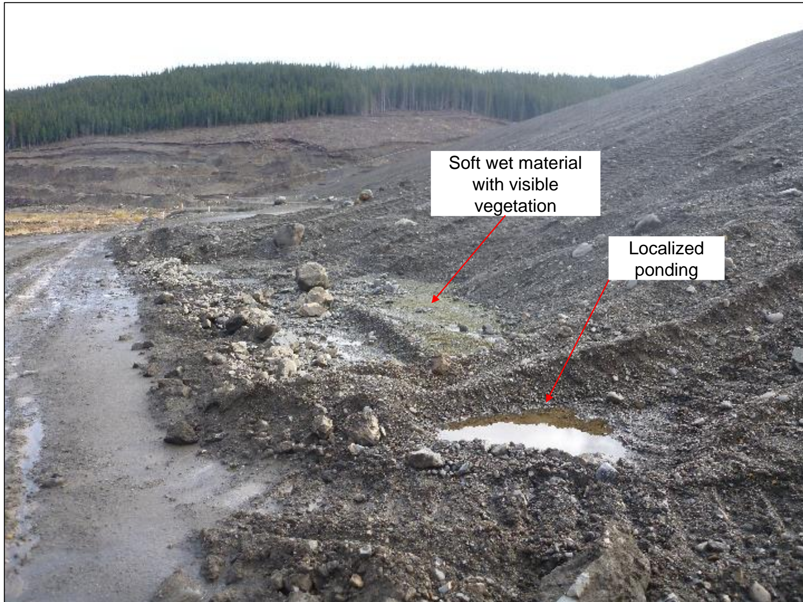
Chainage 0+470: Localized ponding and wet material at toe of NSD. No flowing water observed. Looking east.
