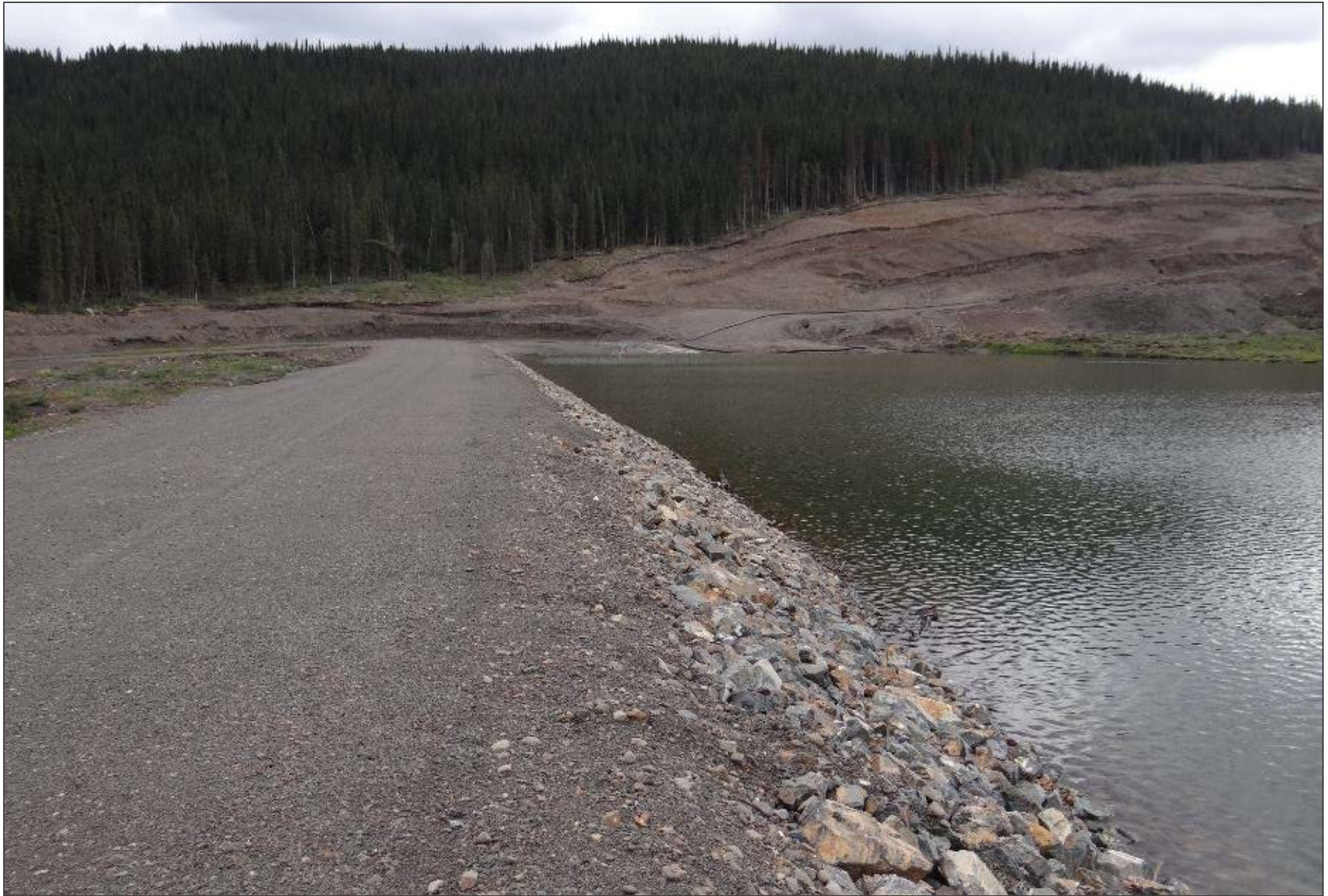
Crest of the NRD, looking east towards the right abutment. No indications of crest settlement, and no indications of upstream slope instability. Riprap on upstream face appears stable.
