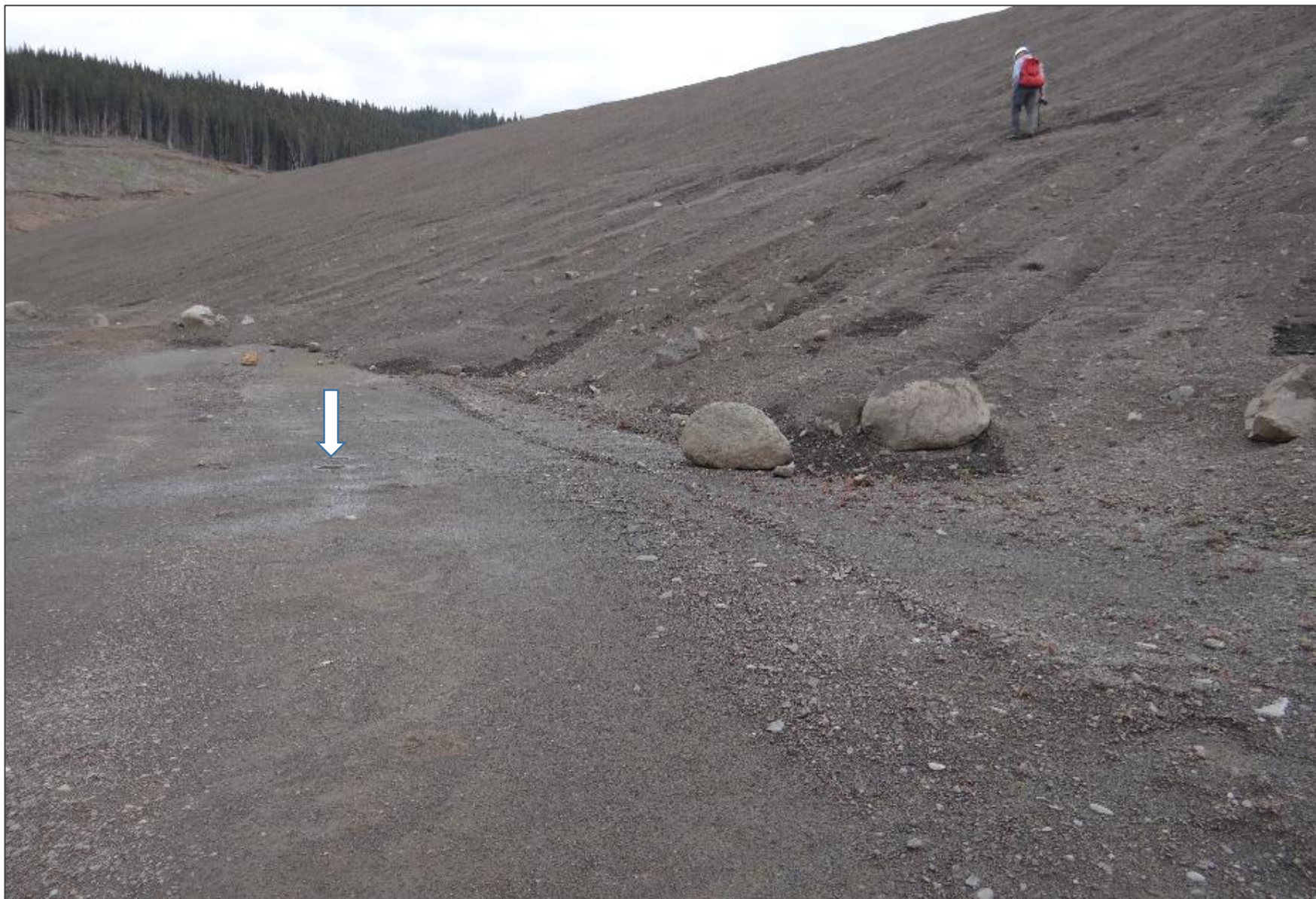
Toe of NSD looking east towards the right abutment. Wet patches on dam face judged to represent lagged discharge of infiltration from recent rains preceding the site visit. Minimal seepage indicated at the toe of the dam. Note wet spots on the surface of the drainage blanket (see arrow).
