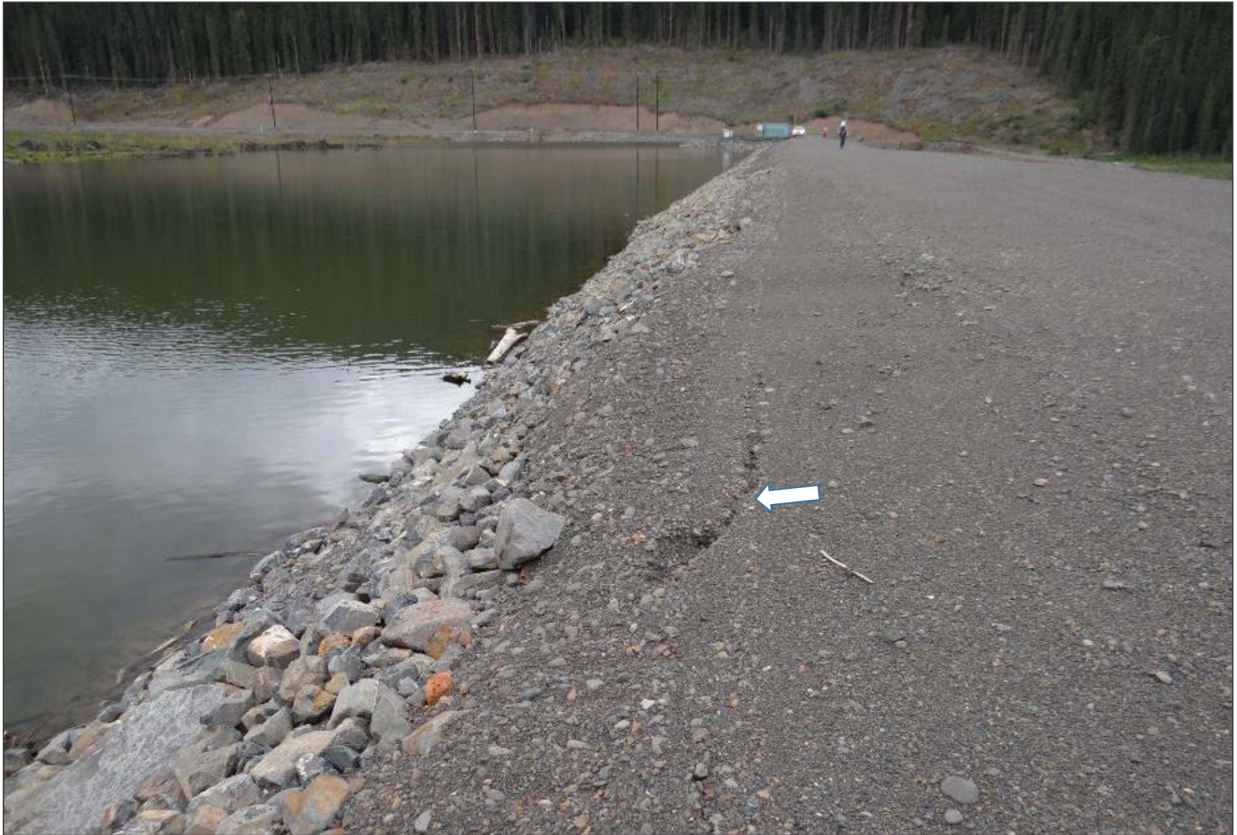
Looking west along the NRD crest and upstream slope, towards the left dam abutment. Apparent crack indicated by arrow appears to be the result of granular road surfacing eroding into the underlying riprap. No indications of upstream slope instability or crest settlement. No indications of riprap instability.
