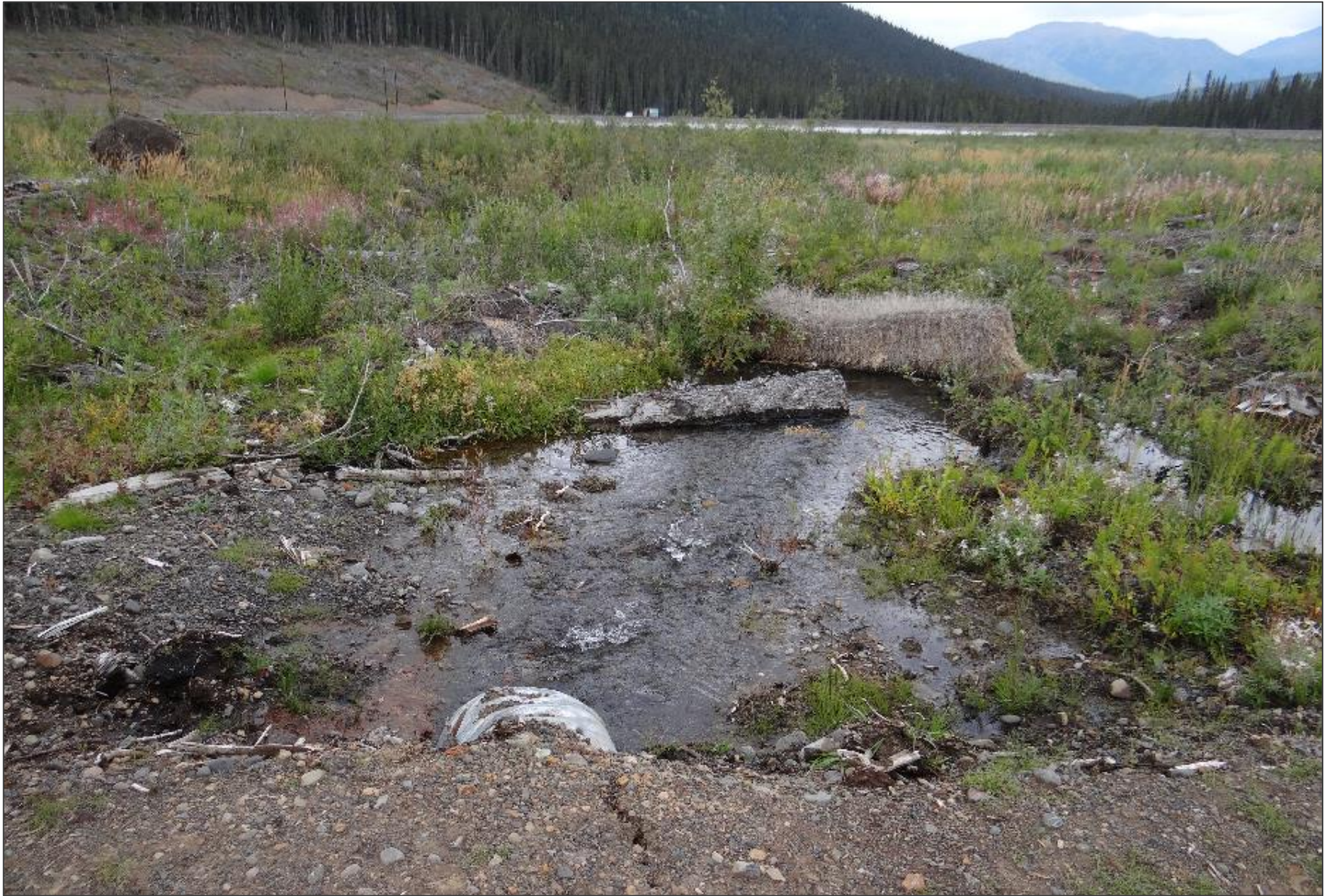
Looking north towards the NRD. Flow rates continuing to increase moving towards the NRD reservoir from the NSD toe.
