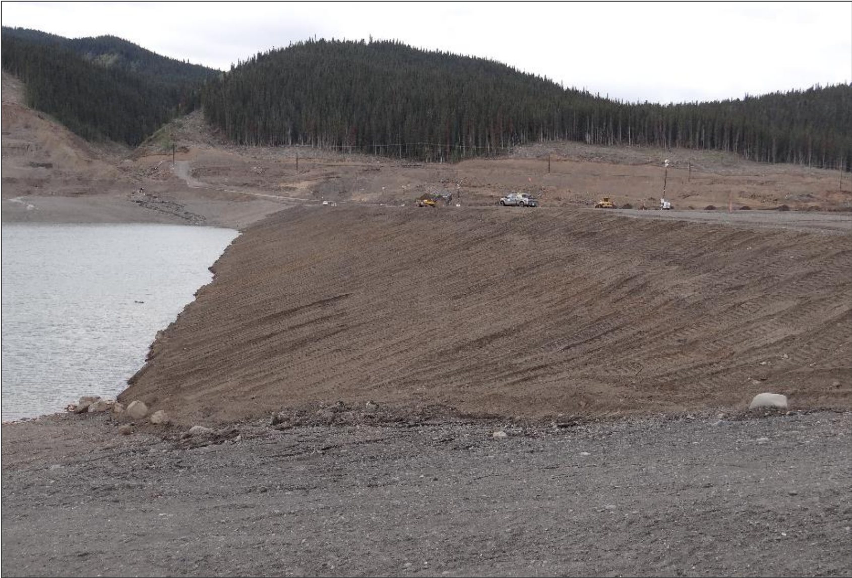
NSD upstream facing, looking west towards the left abutment. No indications of erosion or slope instability.
