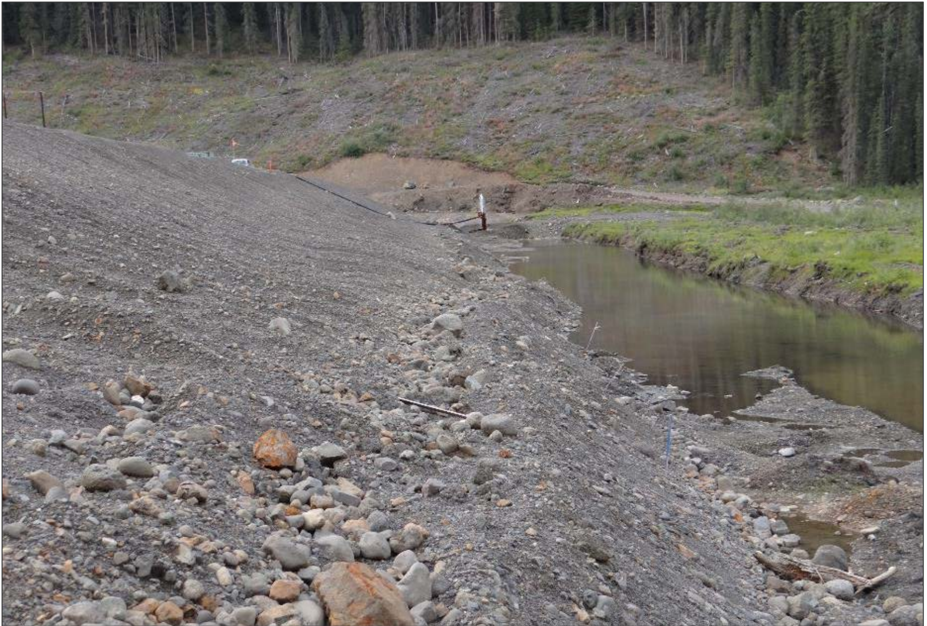
Looking west along the NRD toe, towards the left dam abutment. Discharge from artesian groundwater well 11-NPW2, and upwelling seepage, resulting in water ponding at the toe of the dam. A filter blanket is to be constructed at the toe of the dam to reduce potential for internal erosion of foundation soils.
