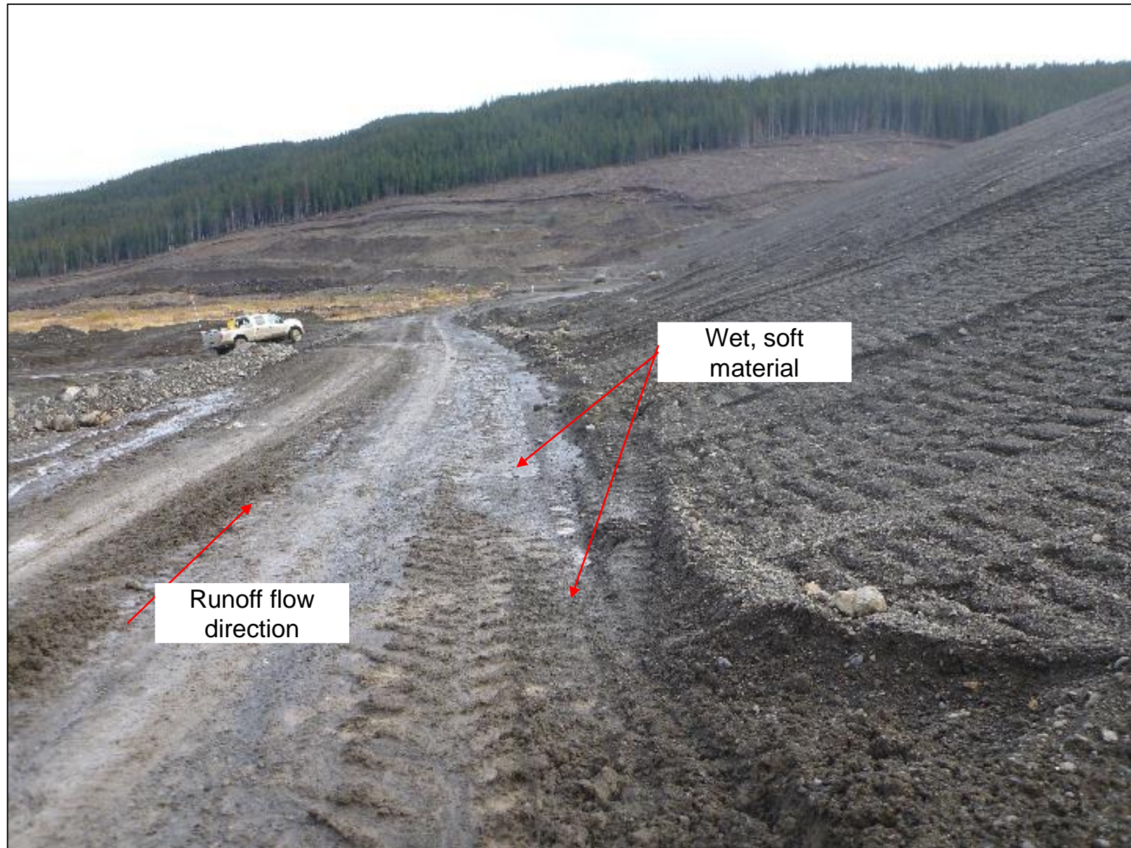
Chainage 0+472: Wet, soft material and ponding water observed at toe of dam. Runoff from access road observed on left (north).
