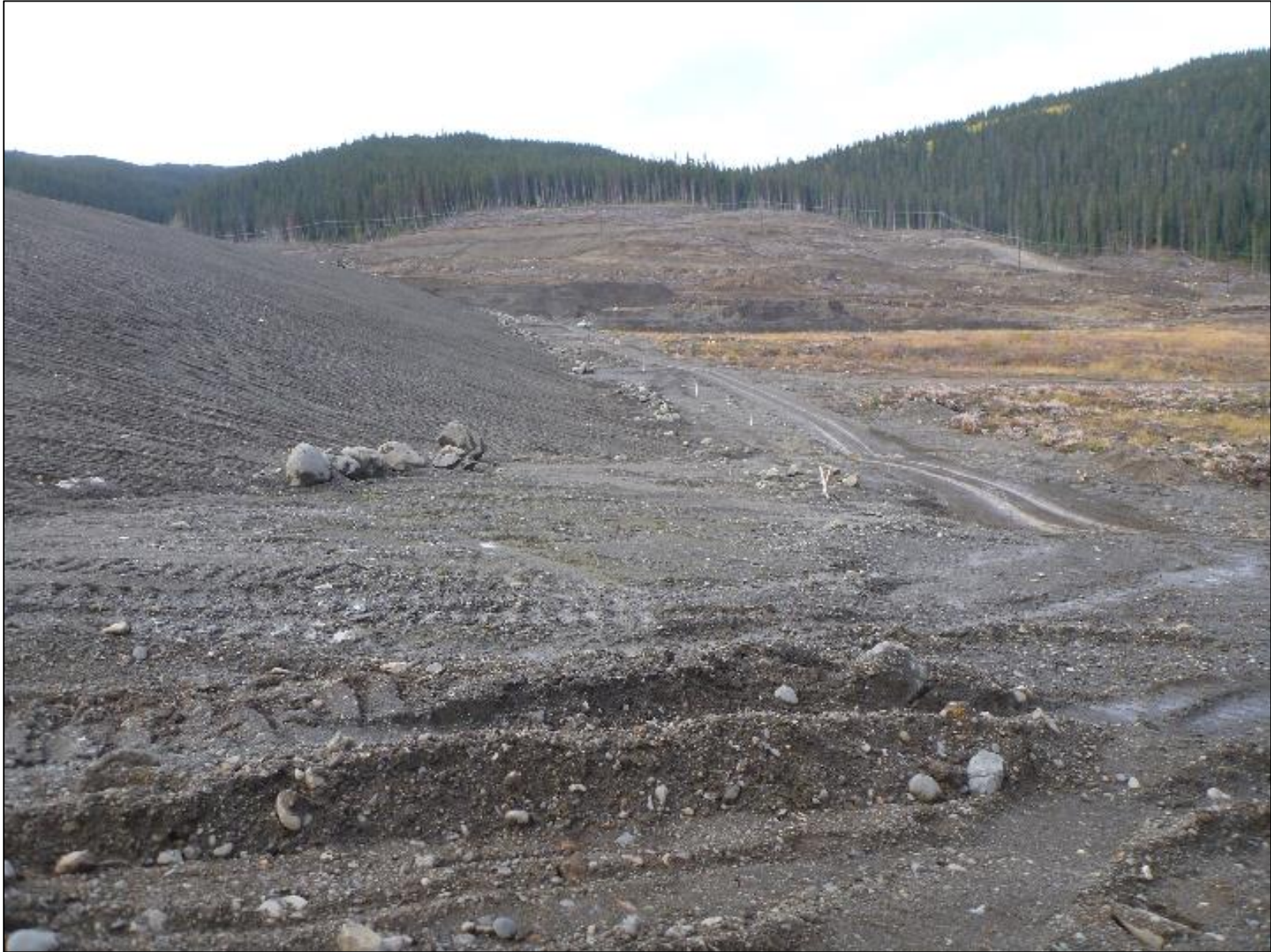
Chainage 0+135: No seepage noted at elevations higher than this point. Ponding water observed in ruts. Looking west.
