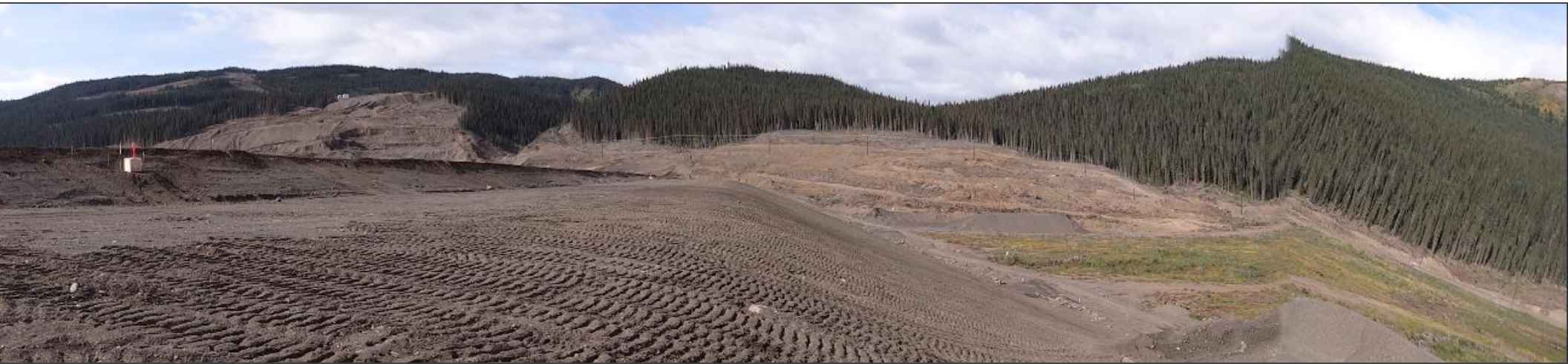
NSD crest and downstream slope (2.5H:1V), looking west towards the left abutment. No indications on slope of instability, erosion, seepage break-out.
