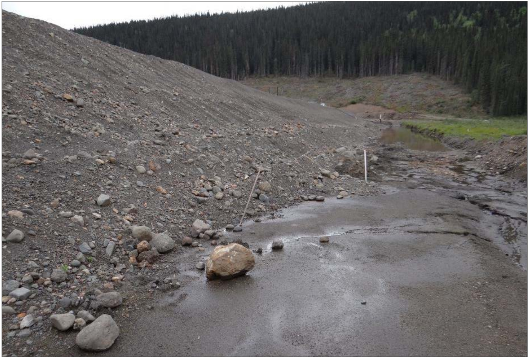
Looking west along the NRD toe, towards the left dam abutment. Note wet conditions owing to this being a groundwater discharge area. No indications of internal erosion, but clear indications of upwelling seepage. A sand and gravel drainage blanket is recommended for construction in the toe area, to protect against potential internal erosion.
