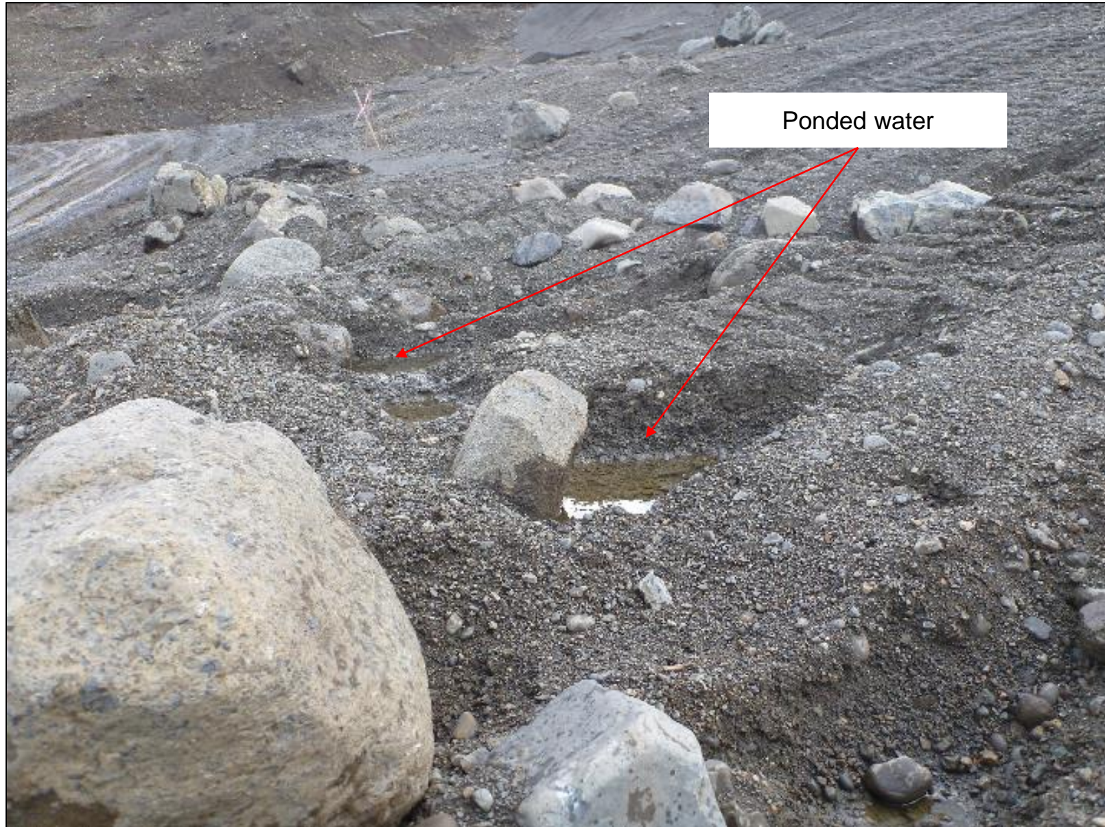
Chainage 0+195: Ponded water observed in depressions caused by side cast rocks from the 1118 Bench above. Looking east.
