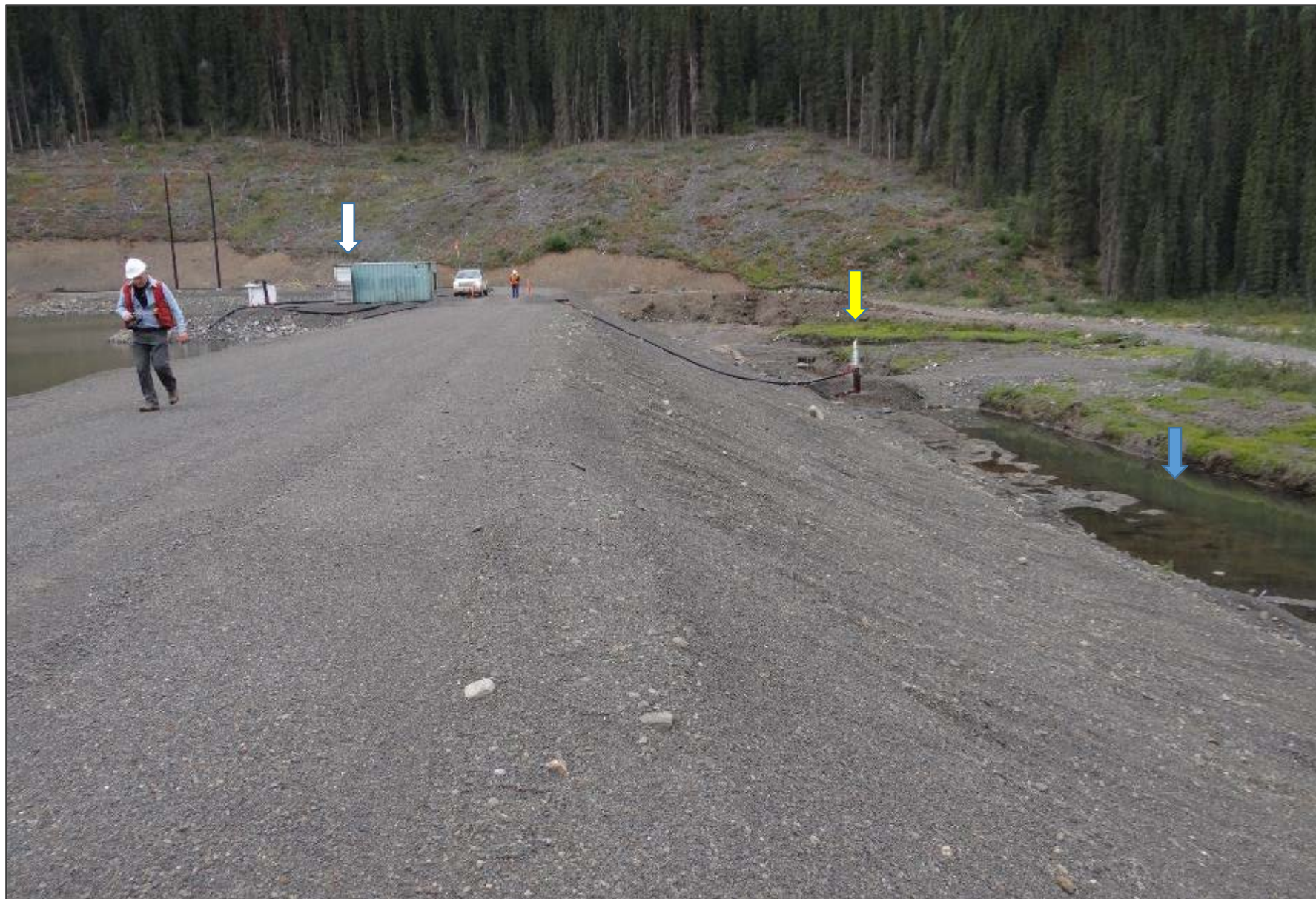
Looking west along the NRD crest, towards the left dam abutment. Pumphouse indicated by the white arrow. Artesian groundwater well 11-NPW2 indicated by the yellow arrow. Discharge from this well is ponding at the downstream toe of the NRD (blue arrow). Downstream slope shows no indications of instability or erosion.
