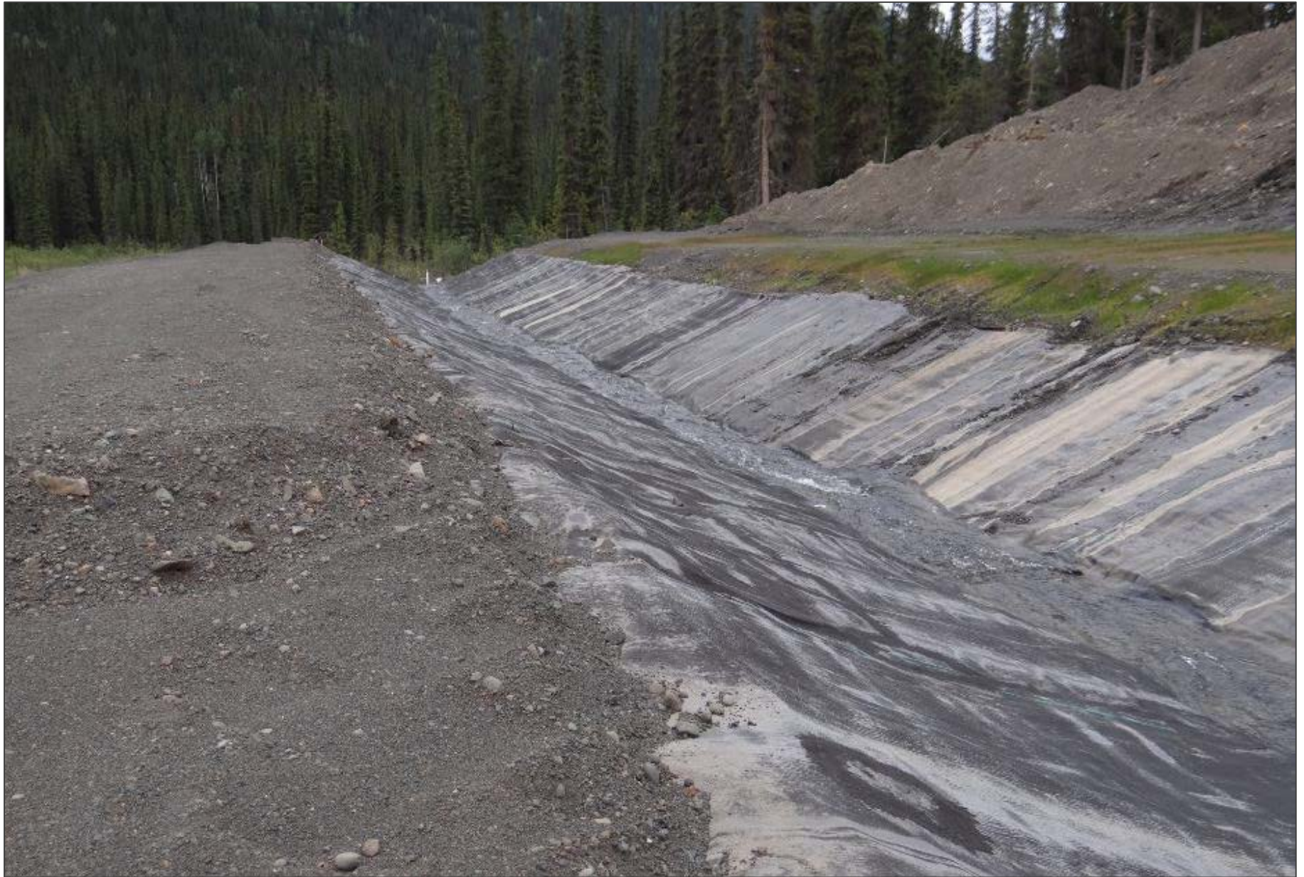
Open channel spillway from the NRD reservoir, looking downstream towards the outlet.
