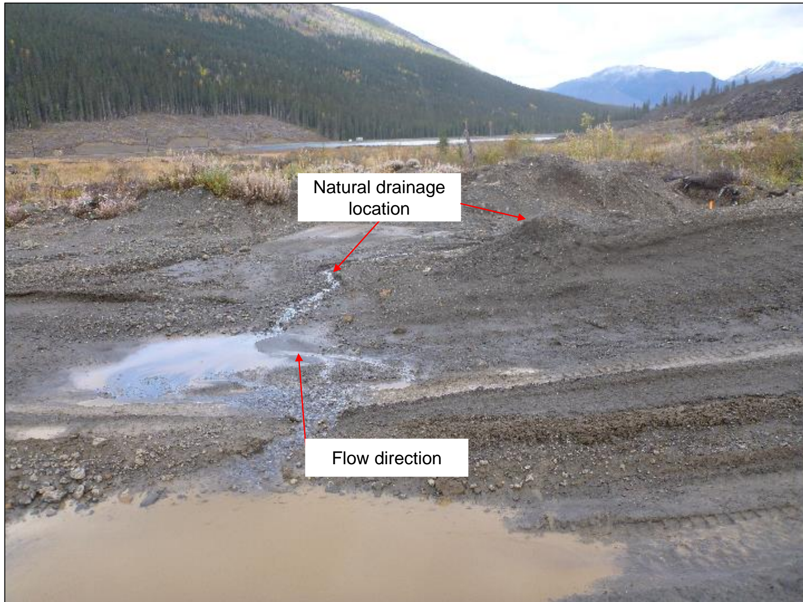
Chainage 0+215: Trickling water on access road below NSD; this location is a low point on the downstream toe and blanket drain near where a natural creek flowed before dam construction. Looking north from NSD toe.
