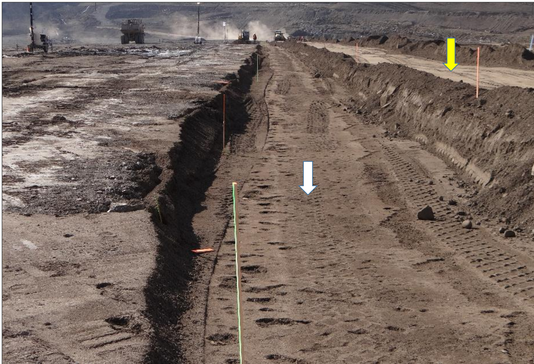
Crest of the NSD. Zone 3A chimney filter (white arrow) and Zone 3B chimney filter (yellow arrow) under construction. Survey stakes in place to control the construction. Zone 1 till core (no 2014 construction on the core prior to the inspection visit) to the left of Zone 3A.
