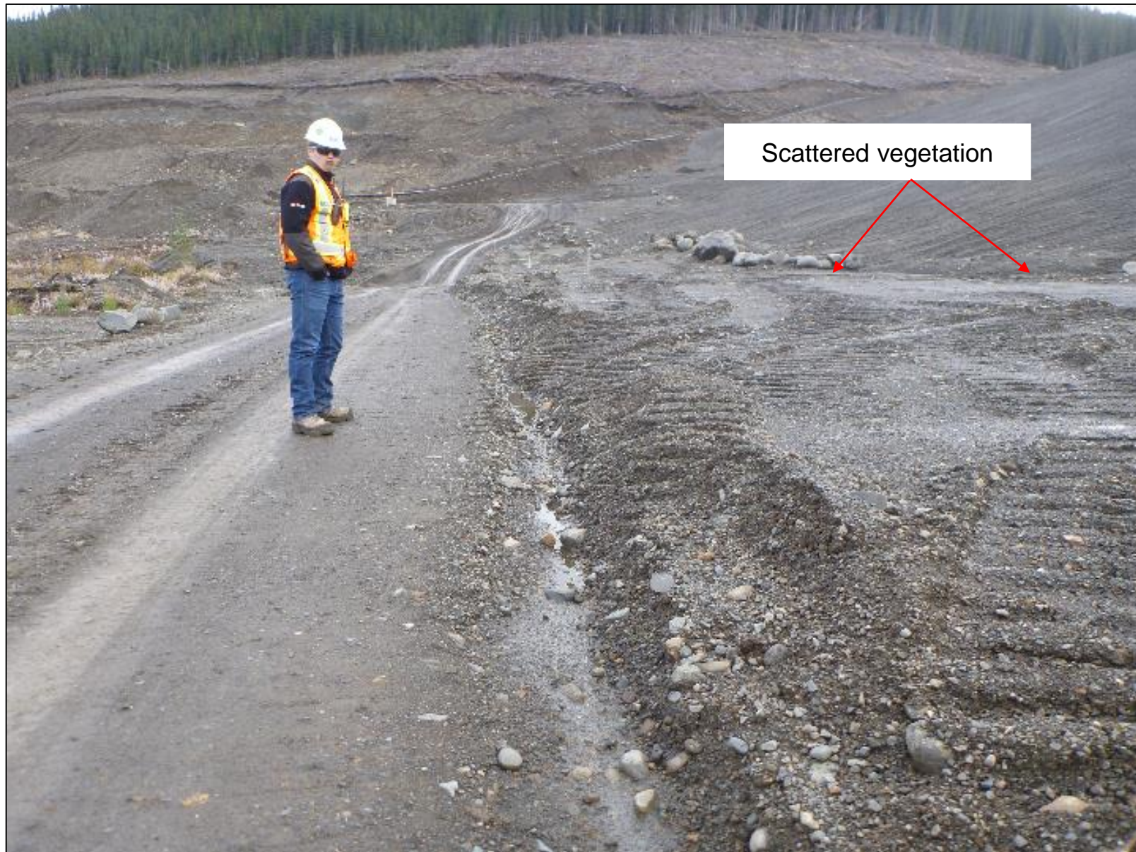
Chainage 0+270: Blanket drain appears wet at surface with scattered vegetation. Drainage ditch along toe. Looking east.
