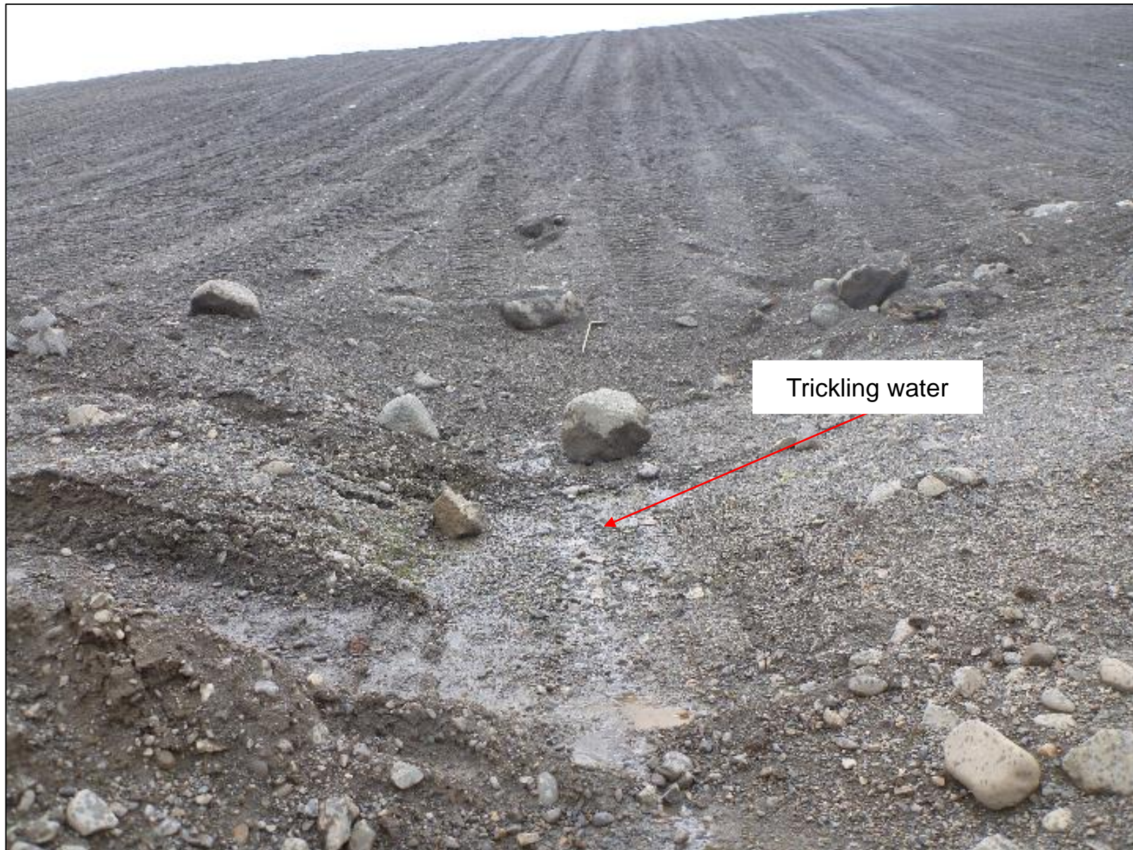
Chainage 0+215: Trickling water noted on the blanket drain; this location is a low point on the downstream toe and blanket drain near where a natural creek flowed before dam construction. Looking south from NSD toe.
