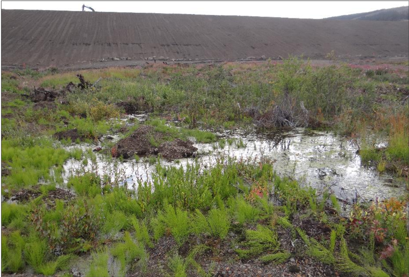
Looking south towards downstream slope of the NSD. Increased flows and springs/ponds moving progressively downstream from NSD to NRD. Note again moist spots at consistent elevations on the downstream face of the dam, representing lagged discharge of rainfall infiltration to the downstream shell of the dam, rather than seepage from the NSD reservoir. No discernible flow at any of these locations.
