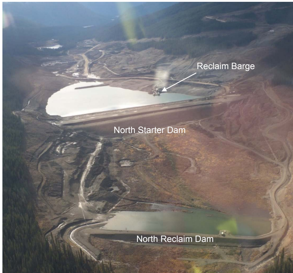
Figure 1. Aerial view of the Red Chris TSF looking south (October 2014). The North Reclaim Dam is approximately 300 m long and the North Starter Dam approximately 600 m long.
