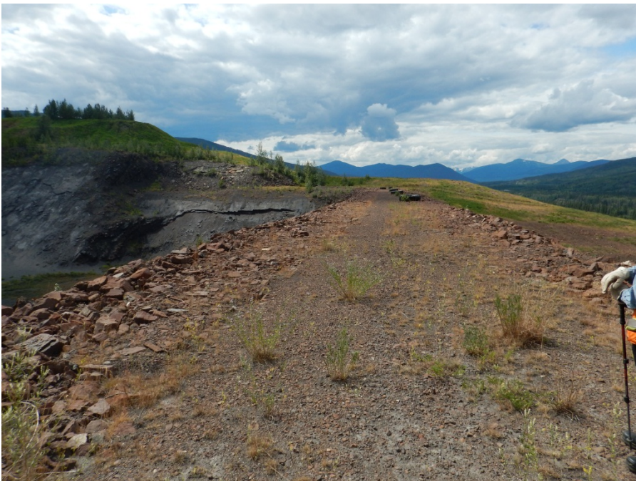
Photo I-13 Overview of NSTD dam crest. No signs of movement or settling (e.g. sinkholes, cracks, slumping) observed. (NSTD-2014-02)
