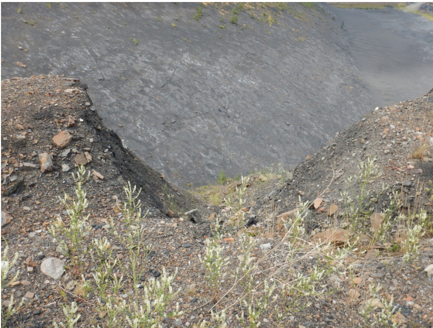
Photo I-3 Erosion of the upslope crest of the Southern Basin Wall near the access road where flow is concentrated through openings in the roadside perimeter berms. No significant observed changes since 2013 DSI. (NSTD-2014-13)
