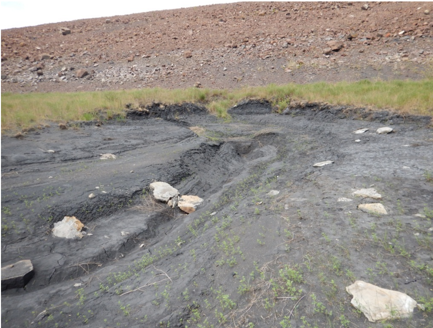
Photo I-17 Drainage channel from the existing pond to the upstream face of the NSTD to promote seepage was unobstructed and dry. (NSTD-2014-07)
