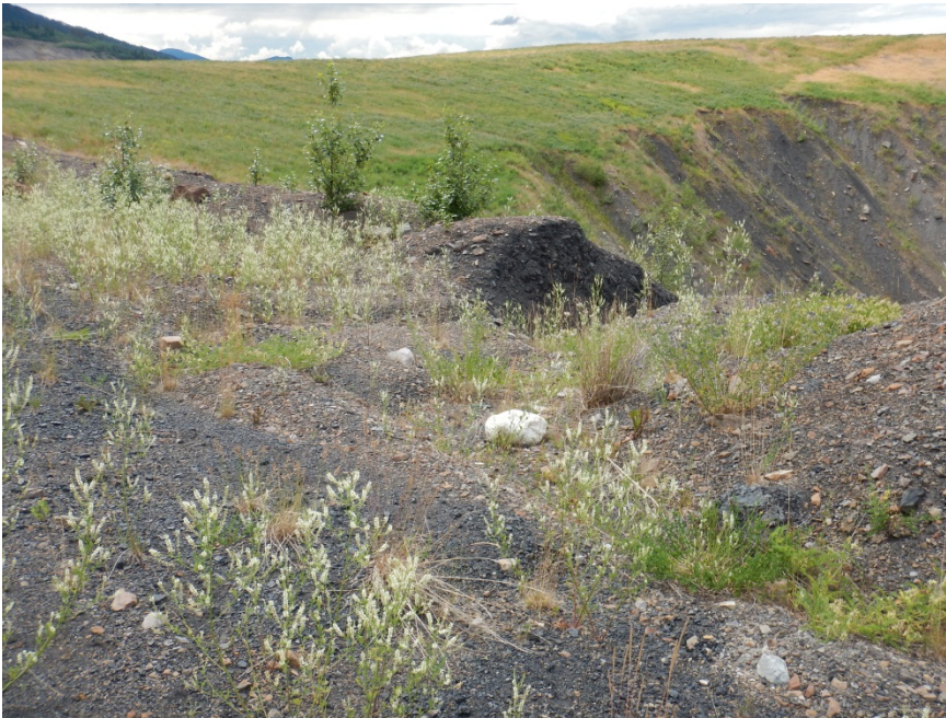
Photo I-4 Erosion shown in Photo I-3 is encroaching on the access road (offset approximately 4 m). Safety berms constructed to the Code are recommended between the access road and erosion features. No significant observed changes since 2013 DSI. (NSTD-2014-13)
