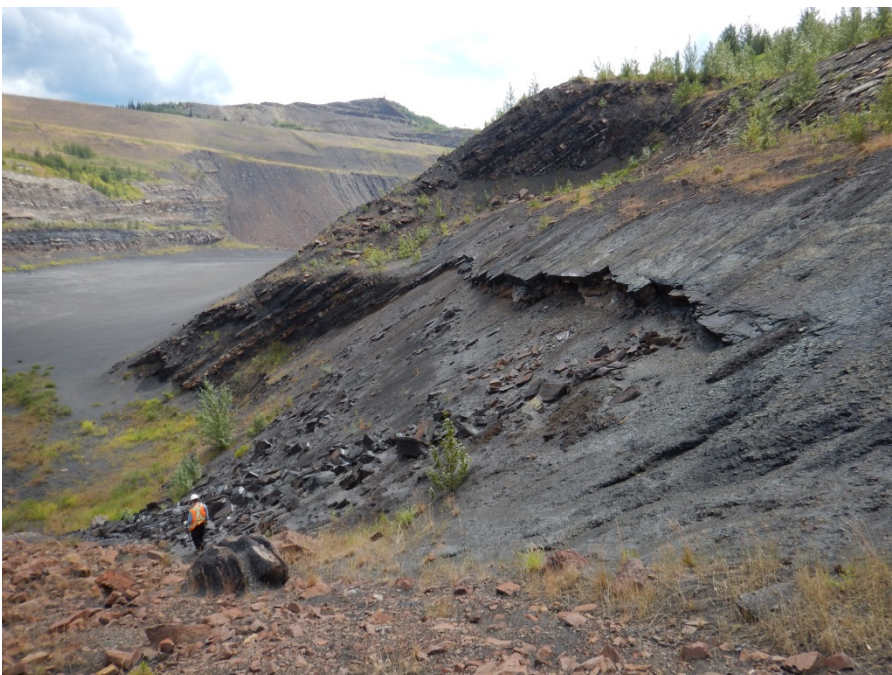
Photo I-20 Ravelling of the exposed rock face upstream of the west abutment caused by weathering of alternating beds of sandstone and shale. No significant change from 2013 DSI.
