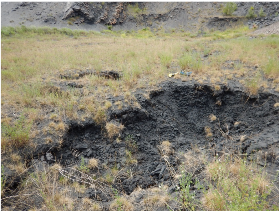
Photo I-16 Sinkholes observed on tailings beach, refer to Section 5 of main text. (NSTD-2014-05)
