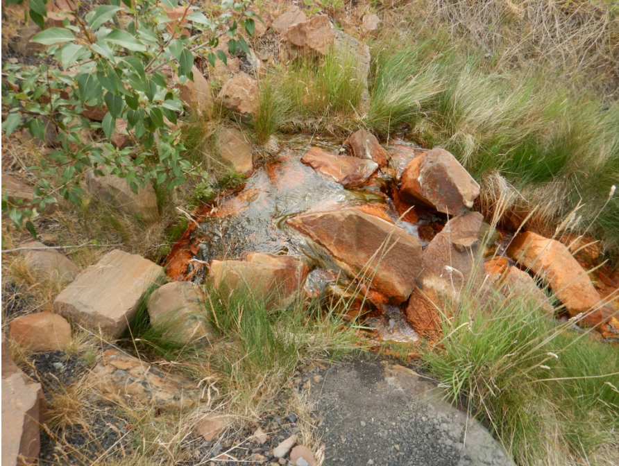
Photo I-6 Seepage discharge from low level outlet downstream of dam. (NSTD-2014-11)
