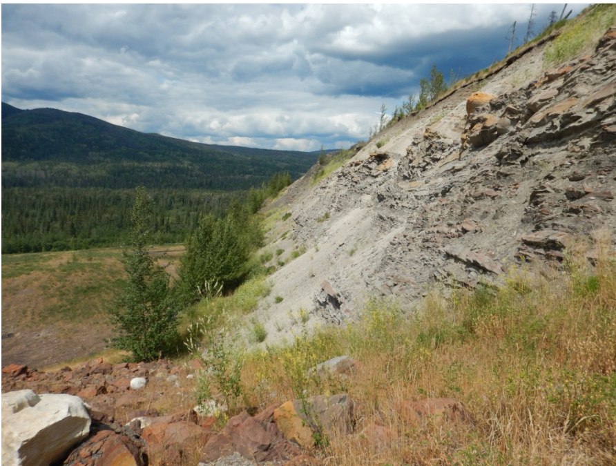
Photo I-11 No Signs of recent movement or settling along the pit wall downstream of the NSTD or at the east abutment contact. (NSTD-2014-02)
