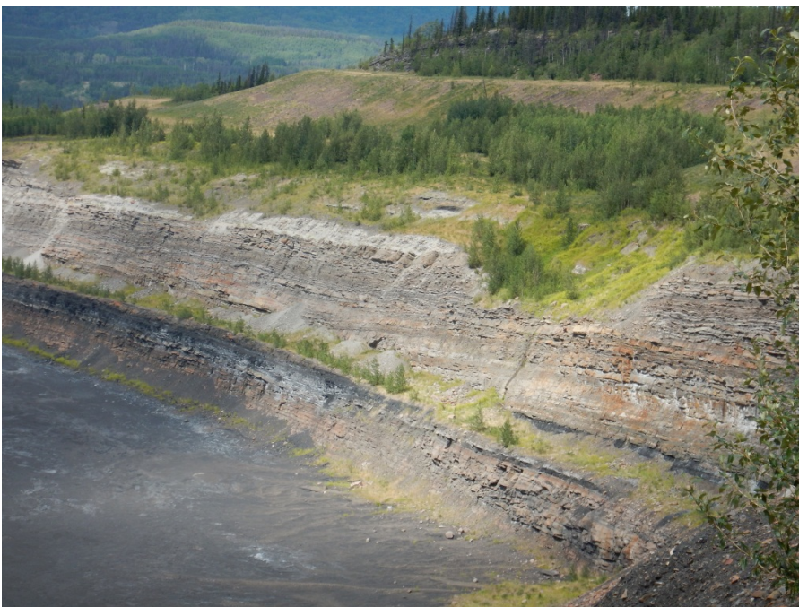
Photo I-5 View of historic slumping failure on the Eastern Basin Wall. No significant observed changes since 2013 DSI. (NSTD-2014-13)
