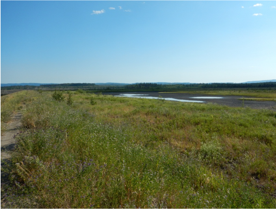
Photo I-12 Ponded water in northwest corner of impoundment. Ponding was noted in this area noted during 2012 and 2013 DSI. (PS-2014-13)
