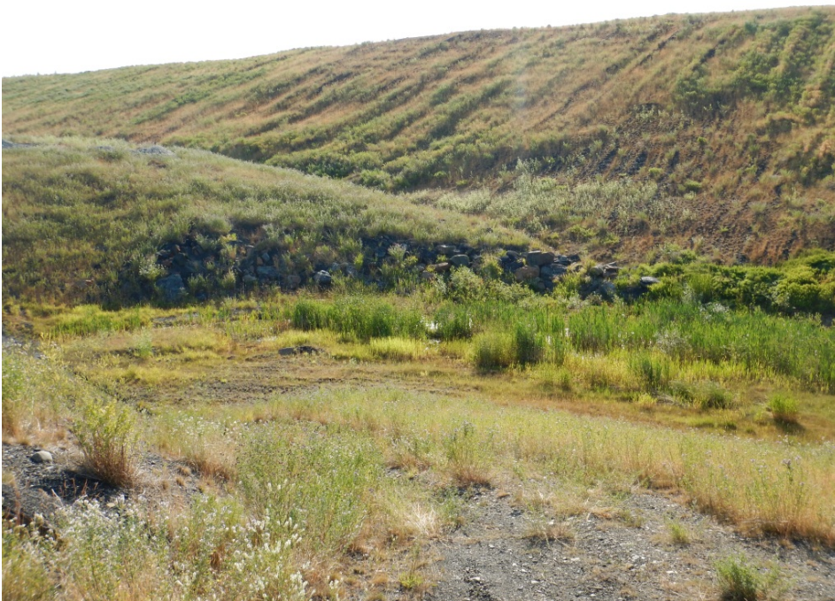
Photo I-3 Riprap (partially overgrown) along outer edge at the sharp bend in spillway channel. (PS-2014-02)
