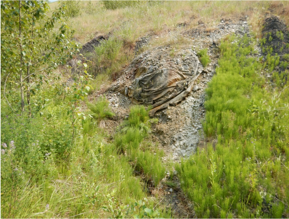
Photo I-16 Typical underdrain daylighting at toe of dam slope. Low rate of seepage visible from underdrain, approximately Sta. 1+150. (PS-2014-35)
