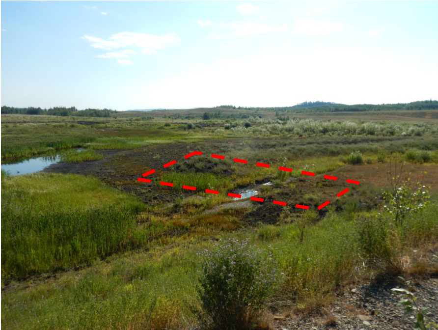
Photo I-6 Inlet to the spillway channel (red dashed area) which is clear with no obstructions. (PS-2014-08)
