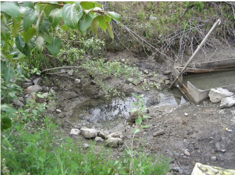
Photo I-18 North Dam Toe east weir. Flow ~ 10 L/s.
