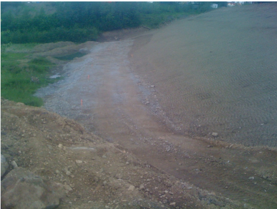
Photo I-8 Cross Dyke: Fine Filter Blanket Drain overbuilt, but can be remediated since site visit.
