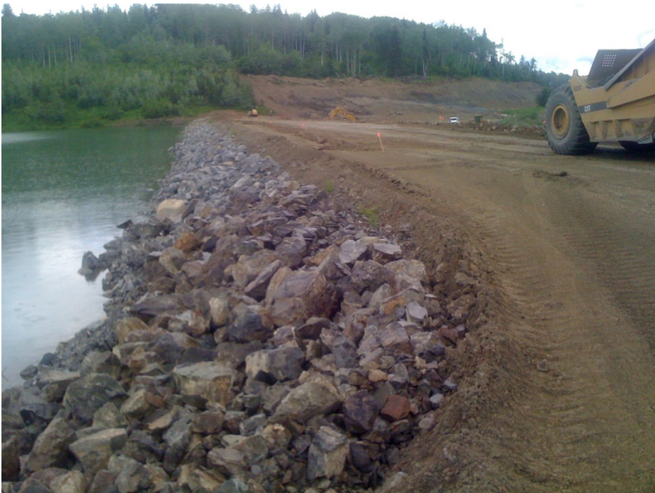
Photo I-6 Cross Dyke: Upstream Face in area where armouring is complete.
