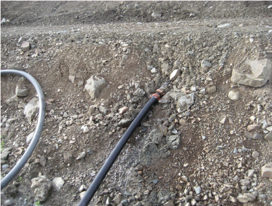
Photo I-15 North Dam Seepage Return pipe leaking at Upper Bench.
