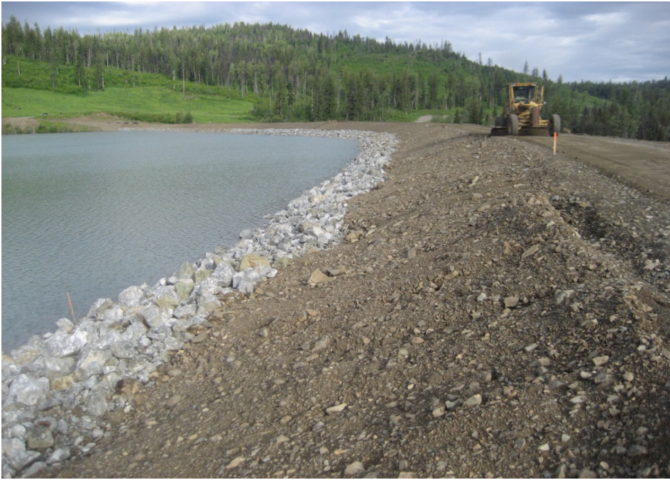
Photo I-13 North Dam Upstream Face, Armouring incomplete at time of site visit
