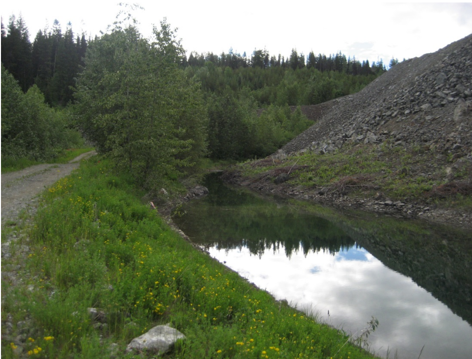
Photo I-20 Seepage Collection Pond (toe of North Dam). Note rockfill slope appears oversteepened.
