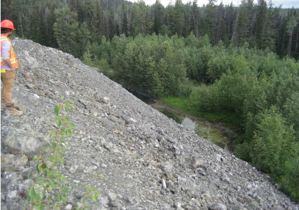
Photo I-10 North Dam Downstream Face. Appears oversteepened. Slope will be confirmed with as-constructed survey.
