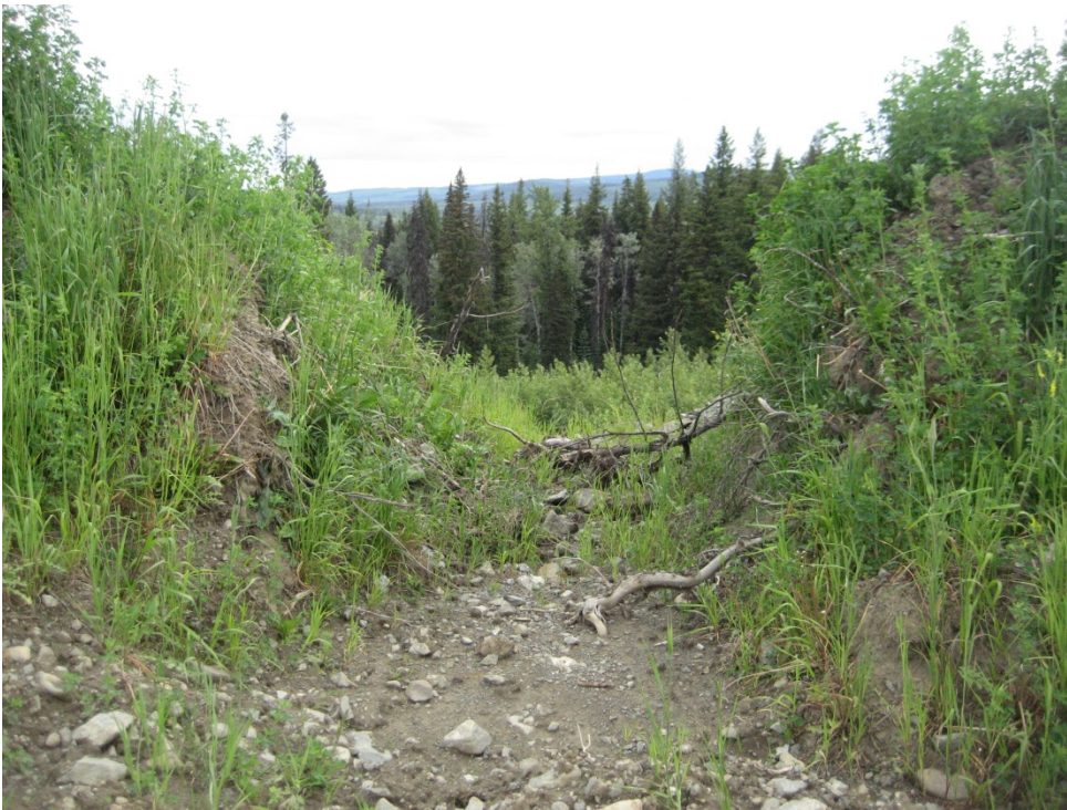
Photo I-21 East Diversion Ditch. Overgrown but generally clear of major debris. Channel dry at the time of the site visit.
