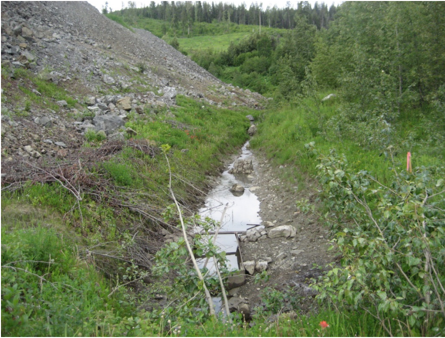
Photo I-17 North Dam Toe. Seepage weir functions but should be kept clear of debris.
