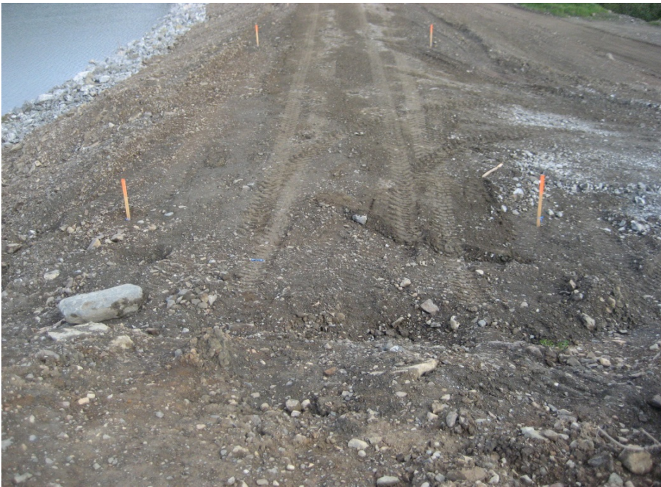
Photo I-11 North Dam Crest. Right abutment material was loose and uncompacted at time of site visit. Has since been remediated.
