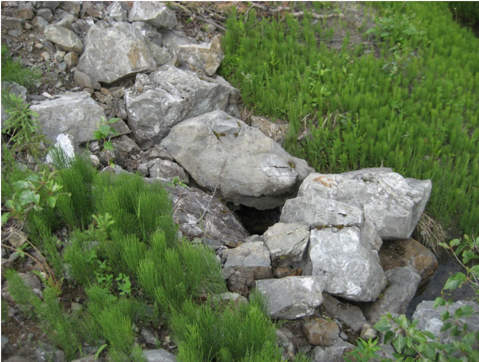
Photo I-19 North Dam Rock Drain Outlet (Flow ~ 8 L/s)
