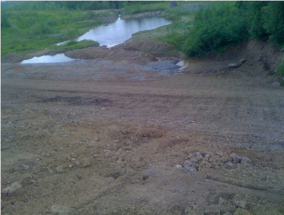
Photo I-7 Cross Dyke Downstream Face. Seepage face observed partway down slope during DSI site visit has since dried.
