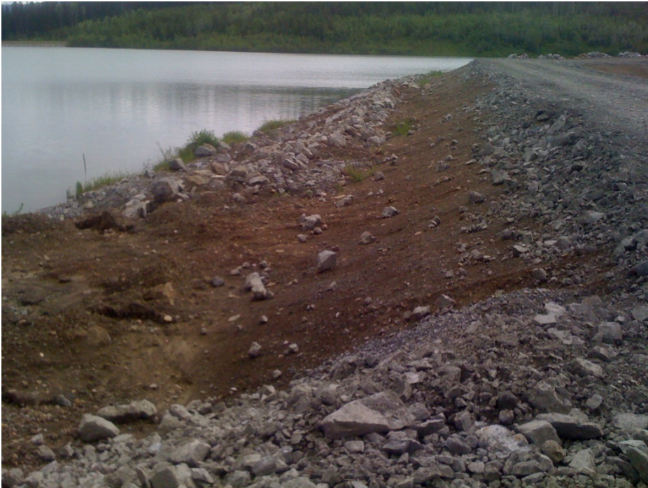
Photo I-3 Cross Dyke: Upstream Slope, Armouring incomplete at the time of site visit.
