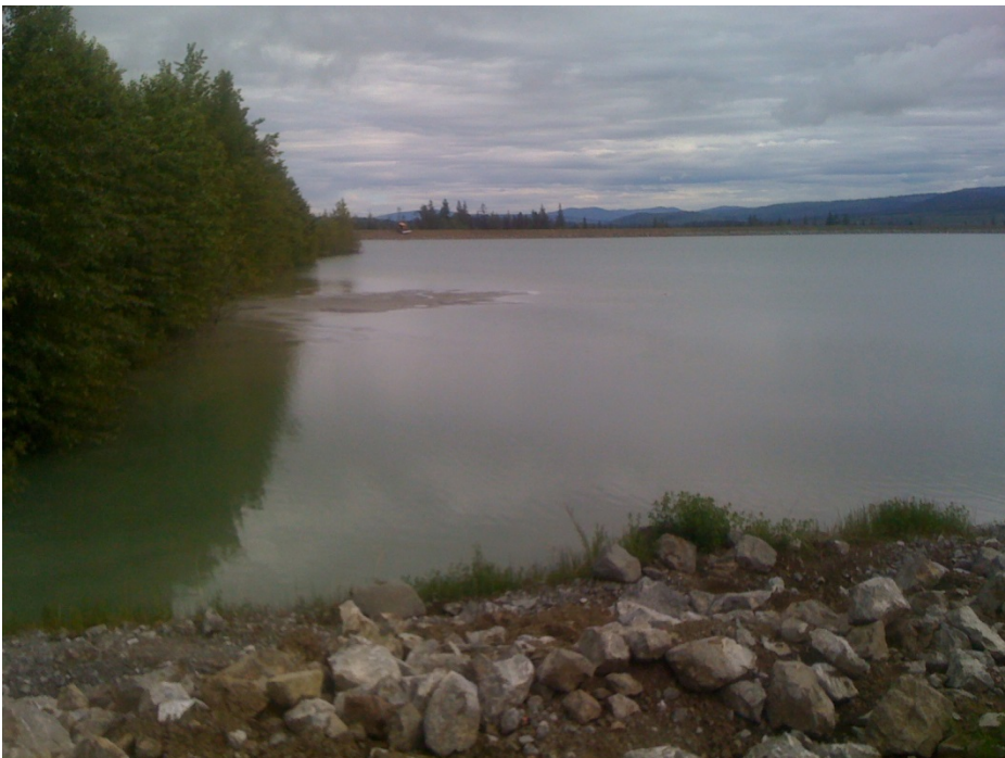
Photo I-4 Tailings Beach on West Side of Impoundment. Heavy vegetation on slope above beach.
