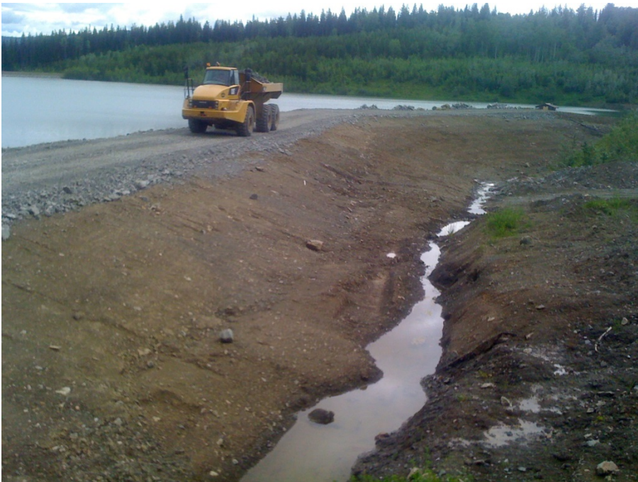
Photo I-2 Cross Dyke: Toe Ditch from Right Abutment to French Drain.
