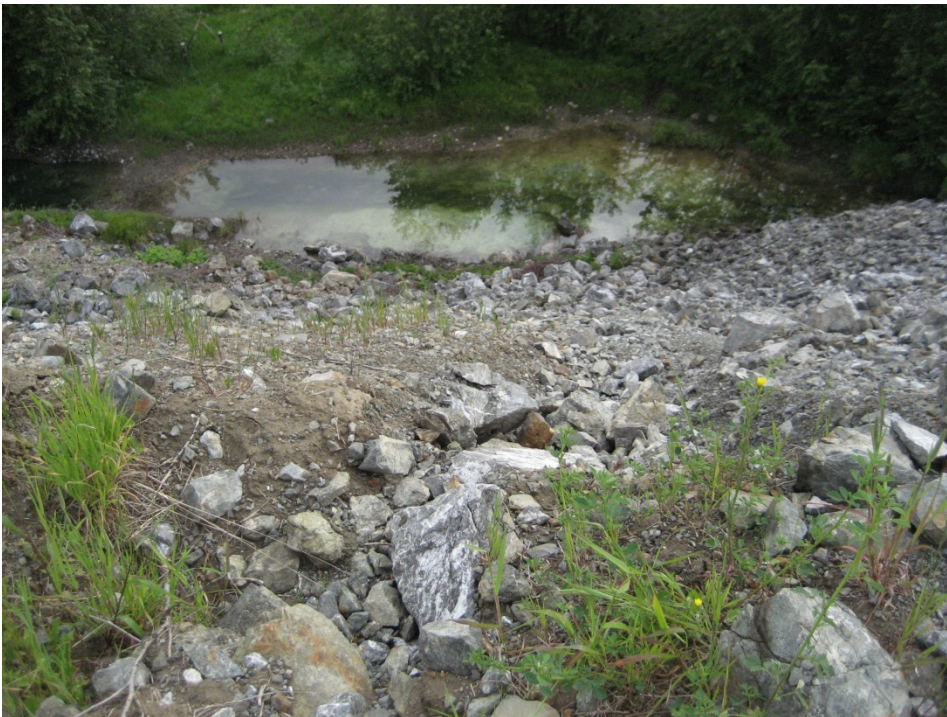
Photo I-16 North Dam downstream rockfill face and seepage collection pond.
