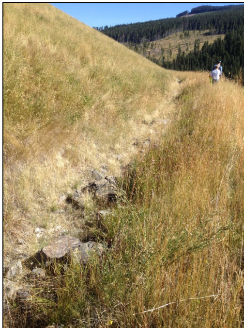
PHOTO 6 – Embankment bench area on downstream slope (eastern side).
