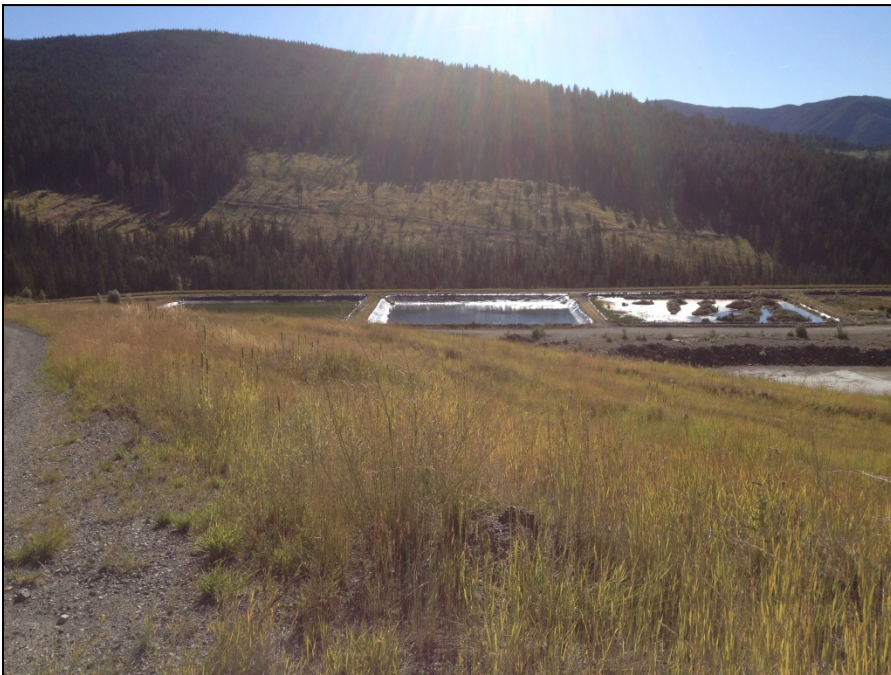
PHOTO 2 – Lined ponds on tailings surface (northeast end of facility).
