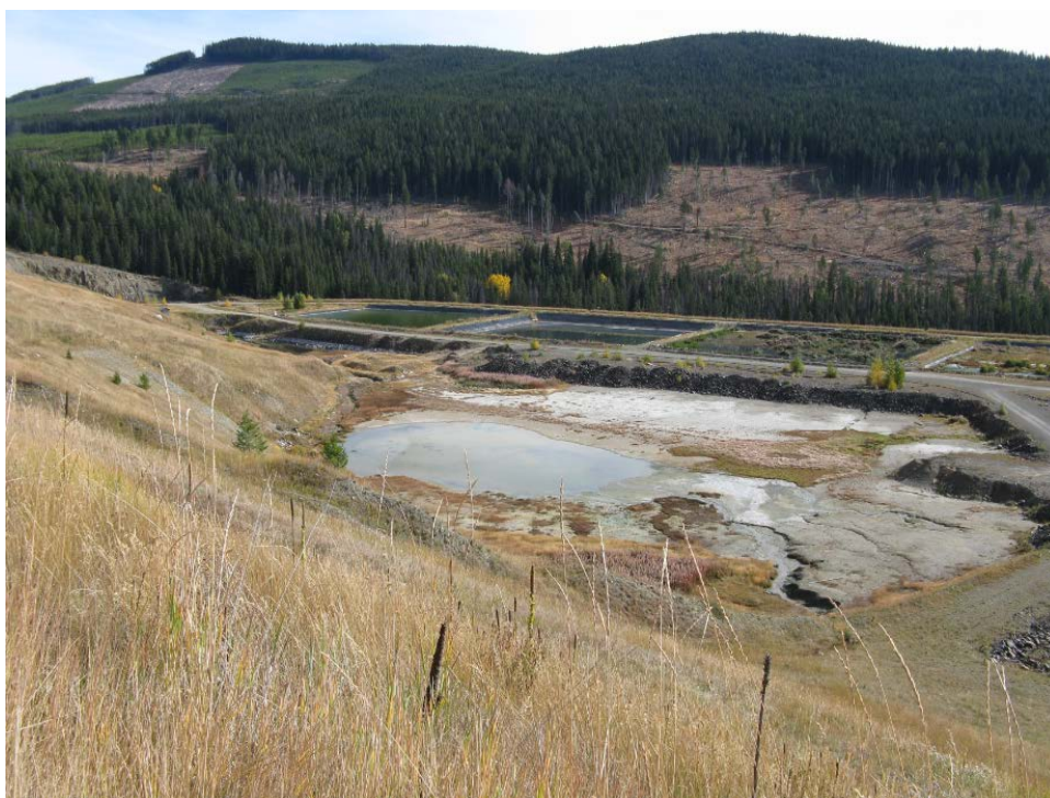
Photograph 2: Lined Pond and Contingency Pond at North End of Tailings Facility, October 9, 2014
