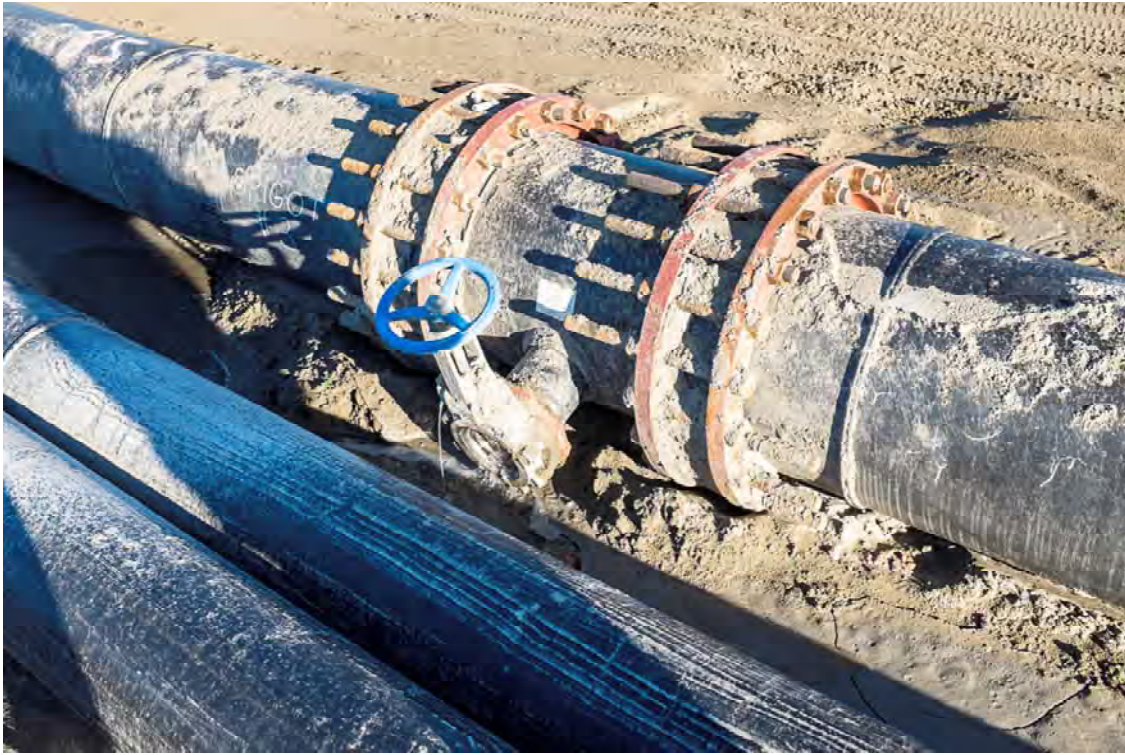
Photo DC07: View of spigot 3 on Dam C looking northwest. Note leaking valve.
