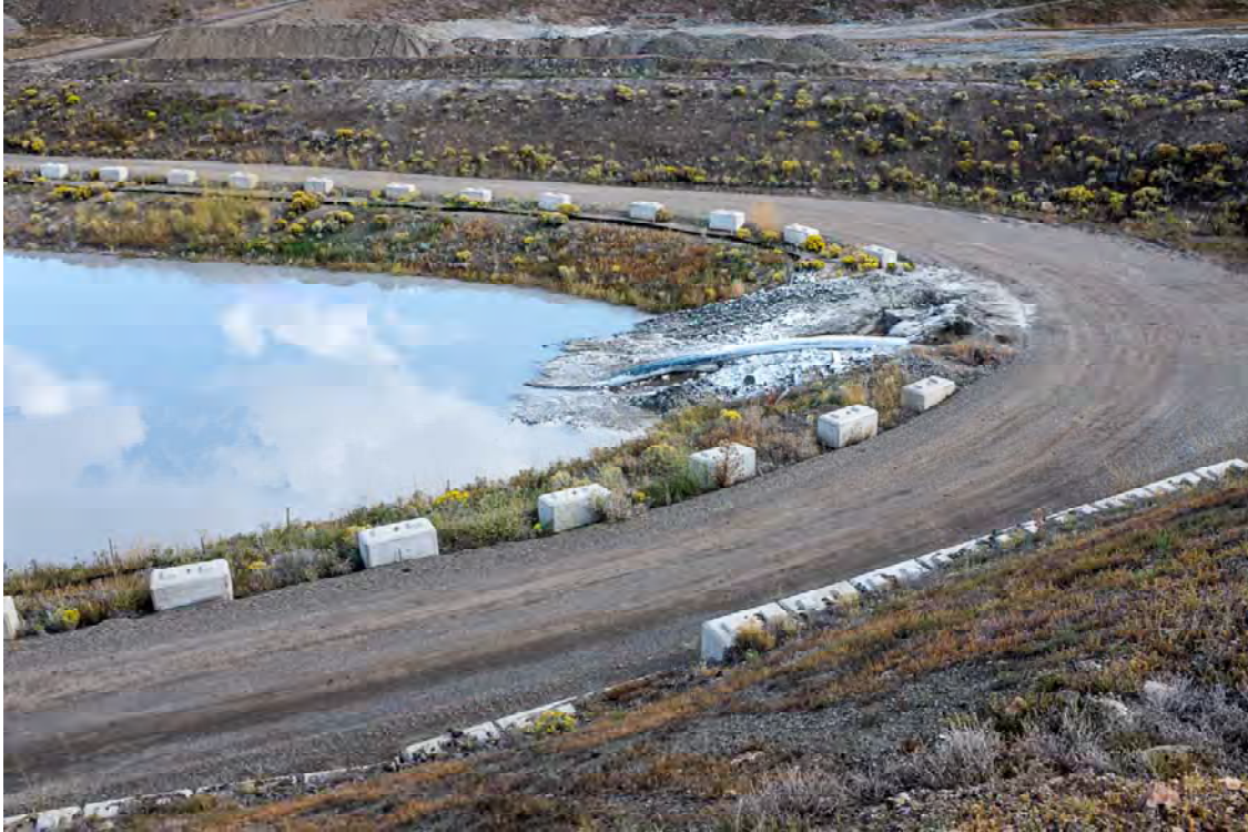
Photo TL13: View of Spill Pond from top of hill adjacent to ore stockpile looking east. Note water level inlet line.
