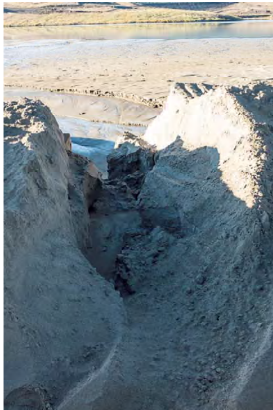
Photo DC10: View of erosion in upstream sand cell berm due to leaking valve at spigot 3 looking south.
