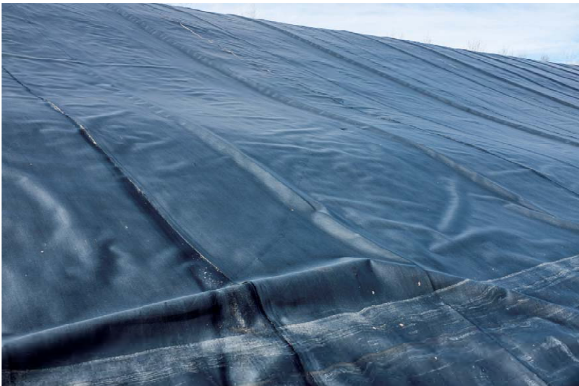
Photo PD08: View of punctures and abrasion damage on the upstream face of the Pothook Dam mid-way between the first dogleg and the tailings pipeline ramp.
