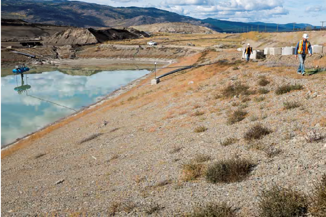
Photo S305: View of the west and north sides of Seepage Pond 3 from the north east corner looking west.
