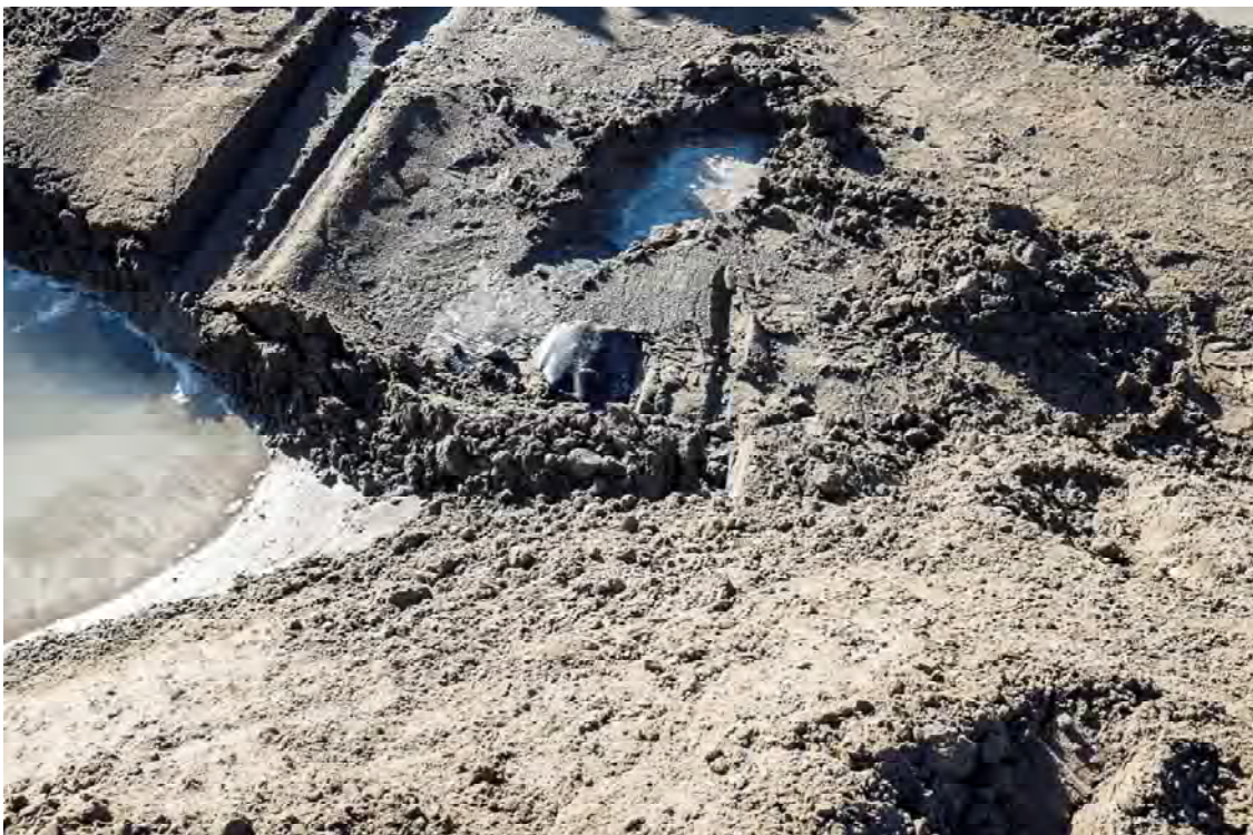
Photo DC18: View looking south at tear in liner adjacent to anchor trench at approximately sta. 0+500 m. Damage done during liner exposure to be repaired if upstream of seaming to liner raise.
