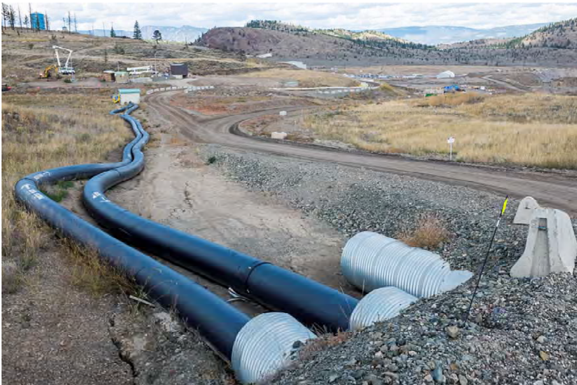
Photo TL04: View of cracking on tailings line right of way on road to TSF just upstream of turn-off to Teck TSF. Note transition from HDPE to steel pipeline in background. Note crew straightening power poles in background left of photo.
