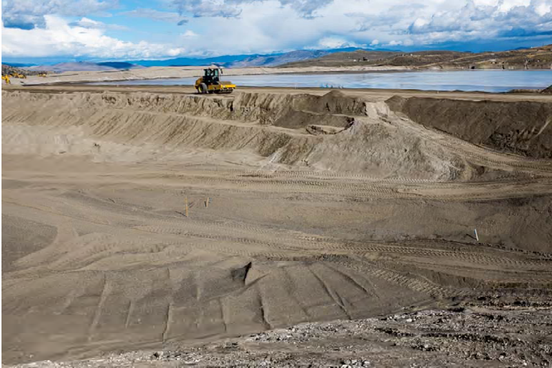
Photo DB03: View looking northeast at Dam B downstream face and toe from the left abutment downstream toe at boundary with Dam A. Dam C visible in the background.
