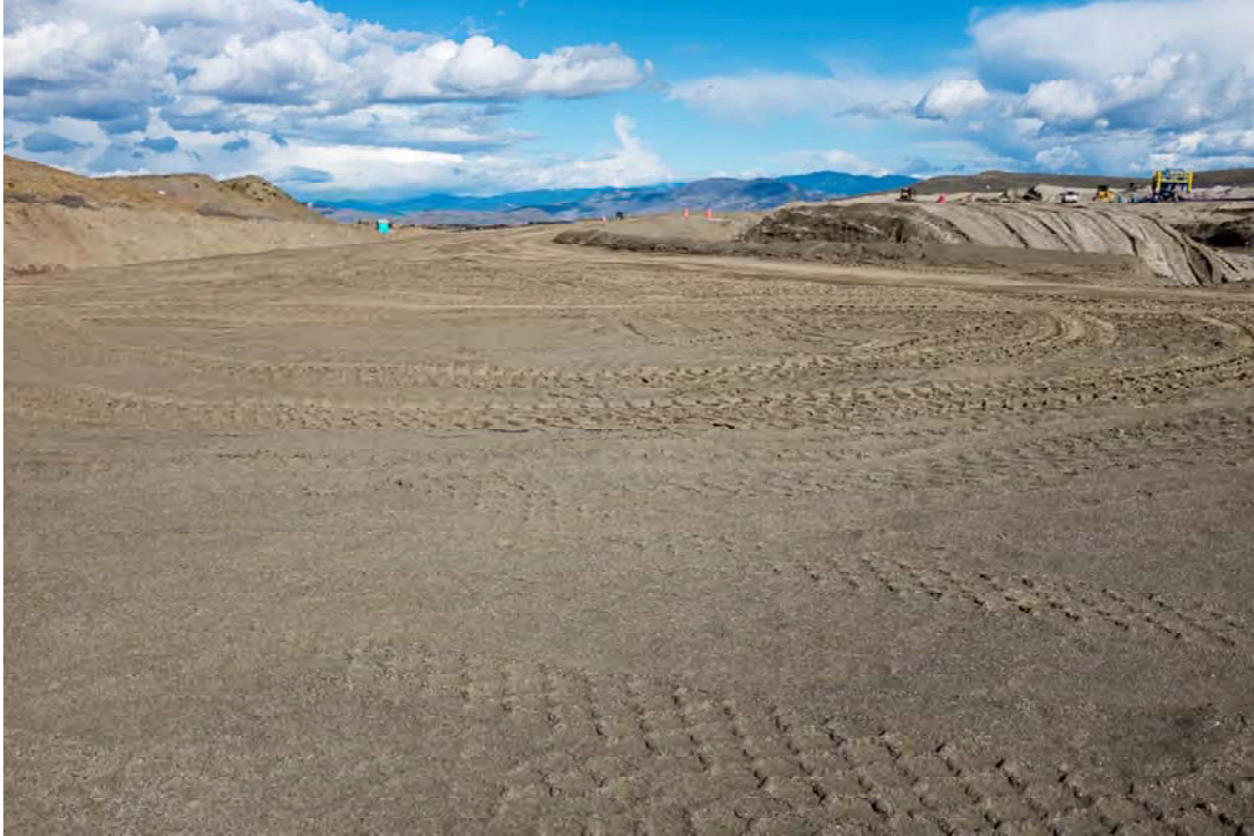
Photo DB09: View looking northeast at right abutment of Dam B from downstream toe. Left abutment of Dam C visible at top right of photo.
