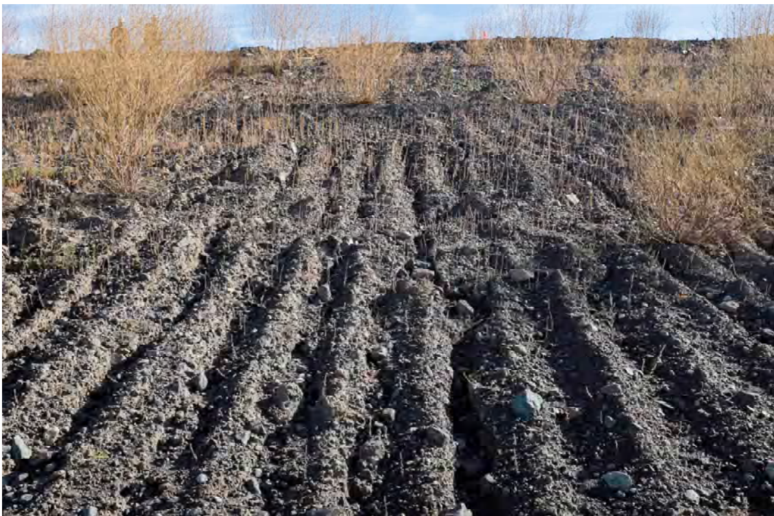
Photo S106: View of downstream face and crest from downstream toe looking east. Note rilling of dam face.
