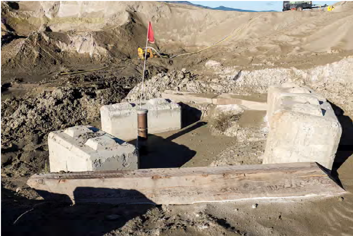
Photo DC35: View looking south west at instrumentation protected by Lock-Blocks on crest at right abutment of Dam C. Note pump used to manage ponded water in background.
