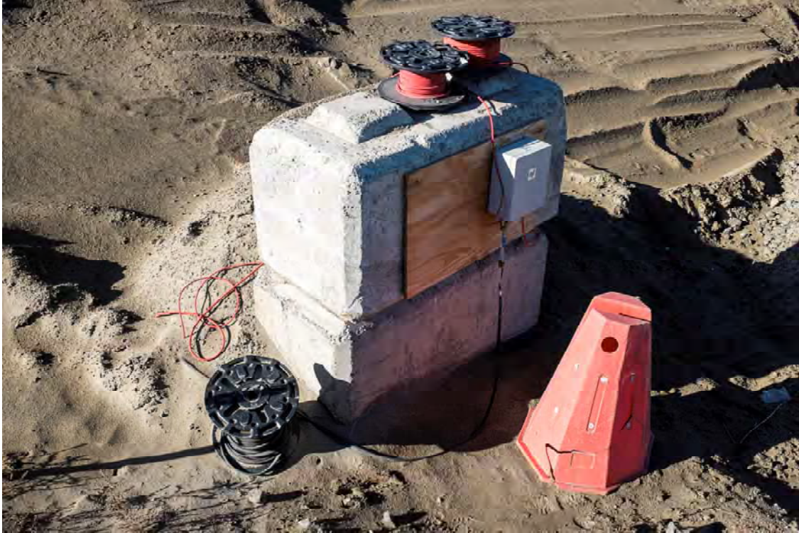
Photo DC37: View looking southwest at instrumentation reporting to datalogger mounted on Lock-Blocks at downstream toe at right abutment of Dam C.
