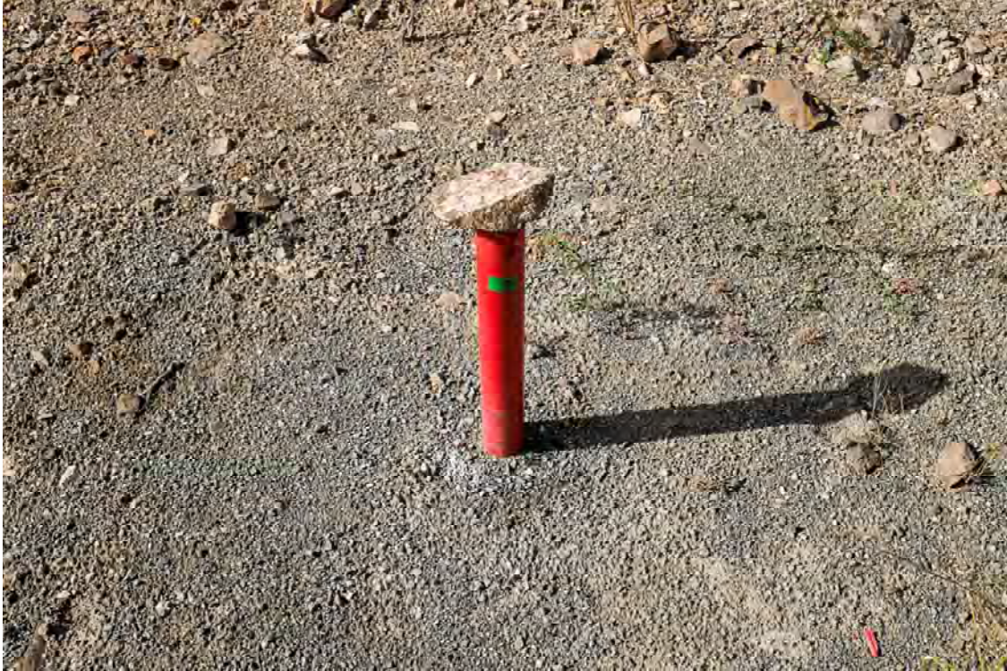
Photo PD27: View of inclinometer casing on downstream side of crest of Pothook Dam adjacent to and north of tailings pipeline ramp.
