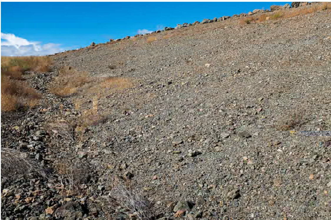
Photo WD14: View of the downstream face and right abutment of the West Dam from the downstream toe.
