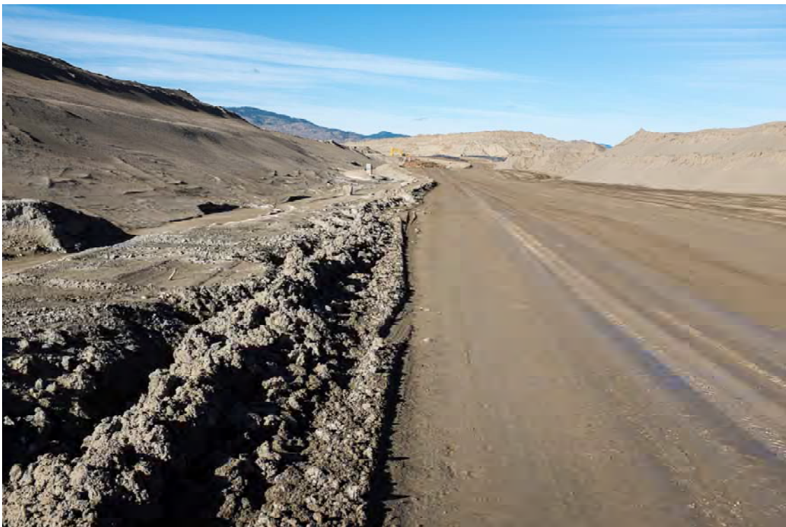
Photo DC26: View looking west from downstream toe of Dam C at approximately sta. 0+600 m.
