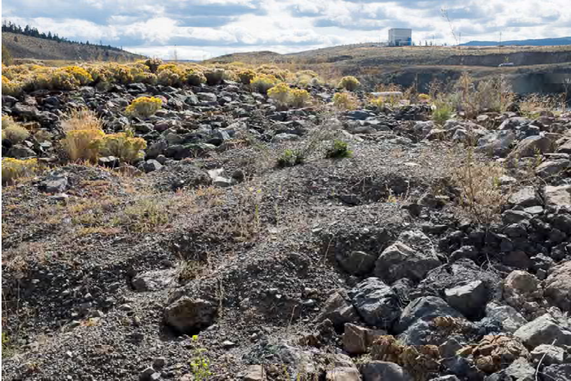
Photo PD39: View of riprap in Pothook Emergency Spillway looking south from spillway. Primary cyclone visible in background.
