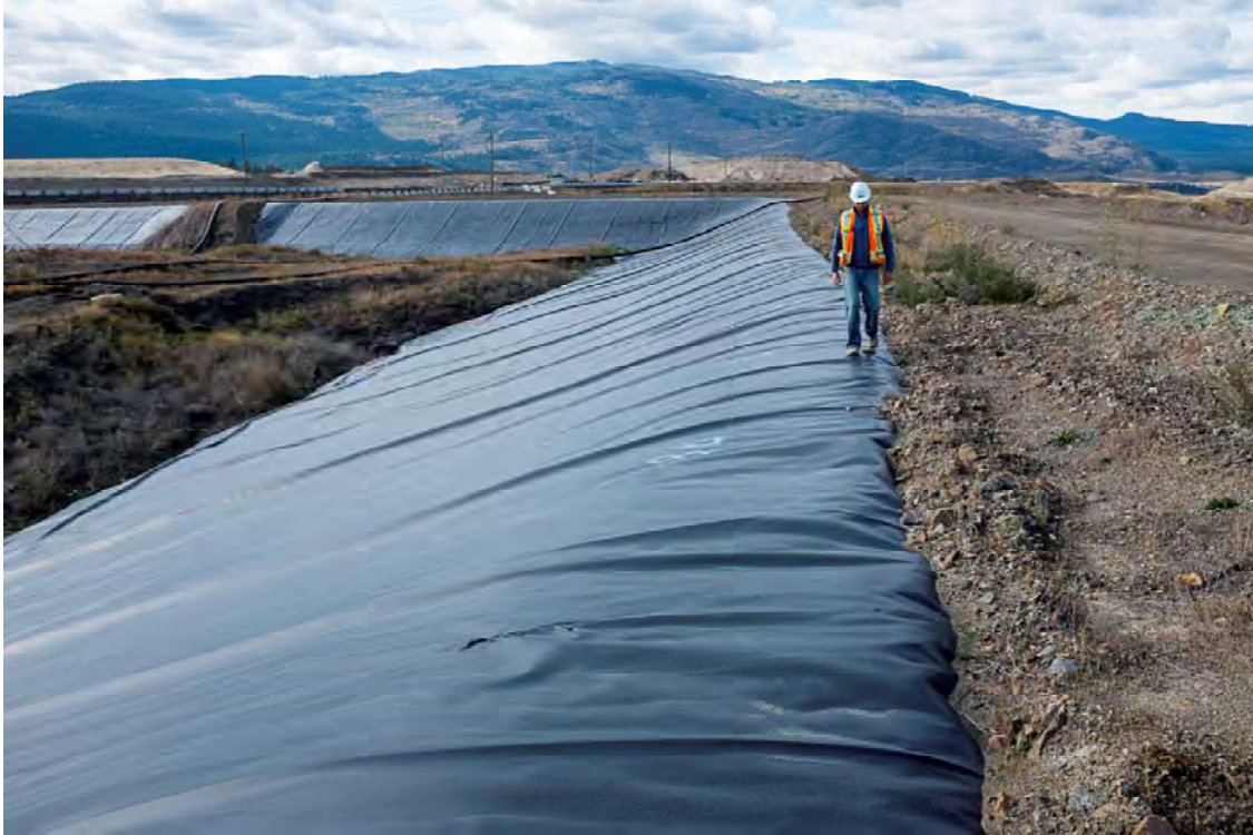
Photo PD31: View of the upstream face and crest of the Pothook Dam from the crest at the right abutment.
