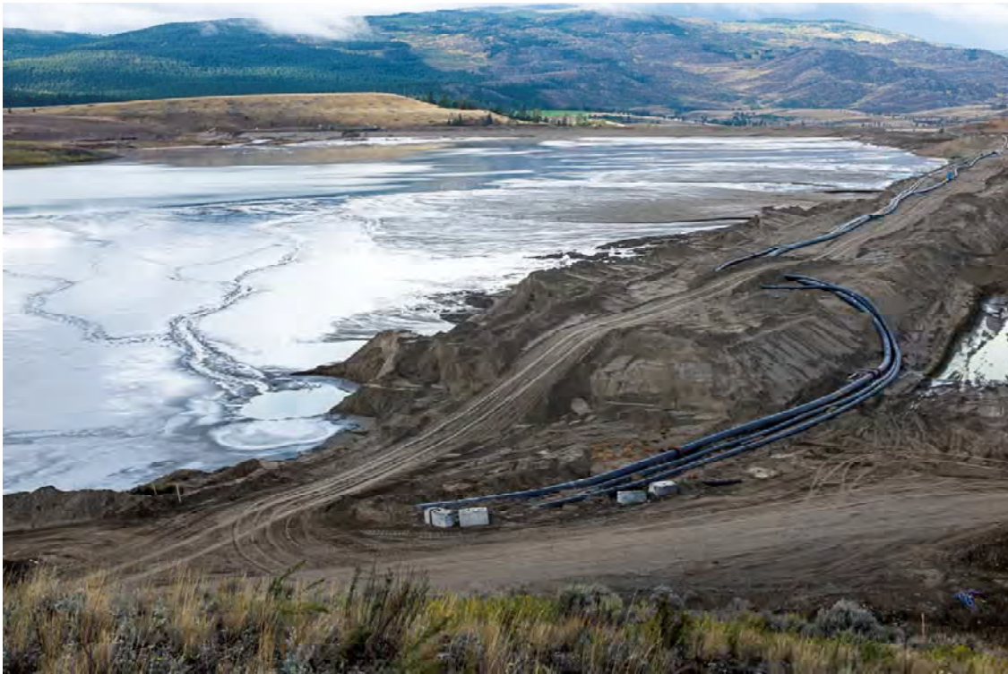
Photo DC03: View of Dam C upstream sand cells and beach looking southwest from survey shed above right abutment.
