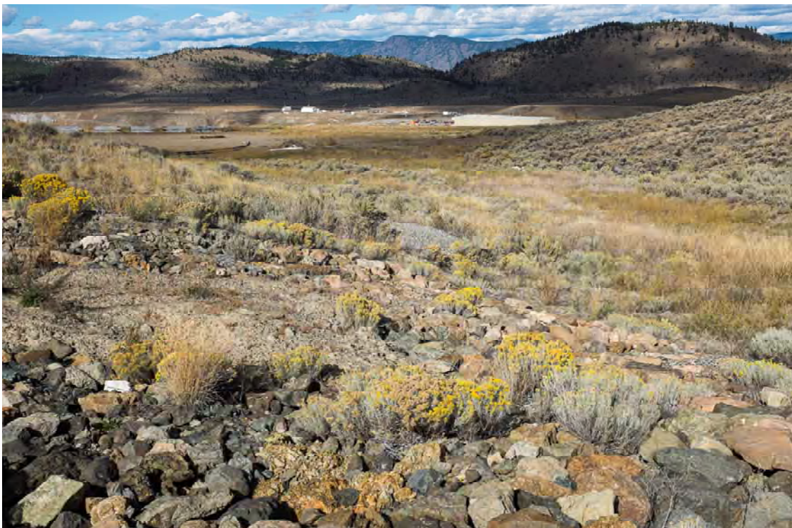
Photo PD38: View looking northwest at outlet of Pothook Pit Emergency Spillway. Afton Open Pit visible in background.
