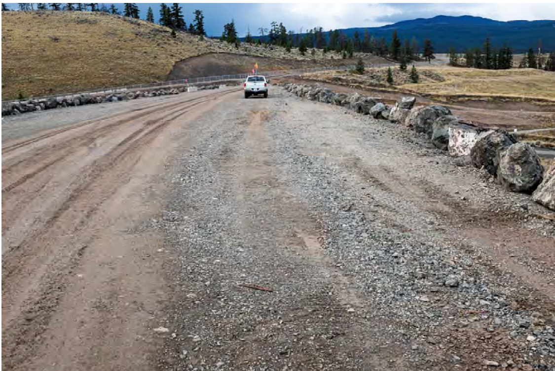
Photo SD10: View of right abutment of South Dam from near left abutment on crest.
