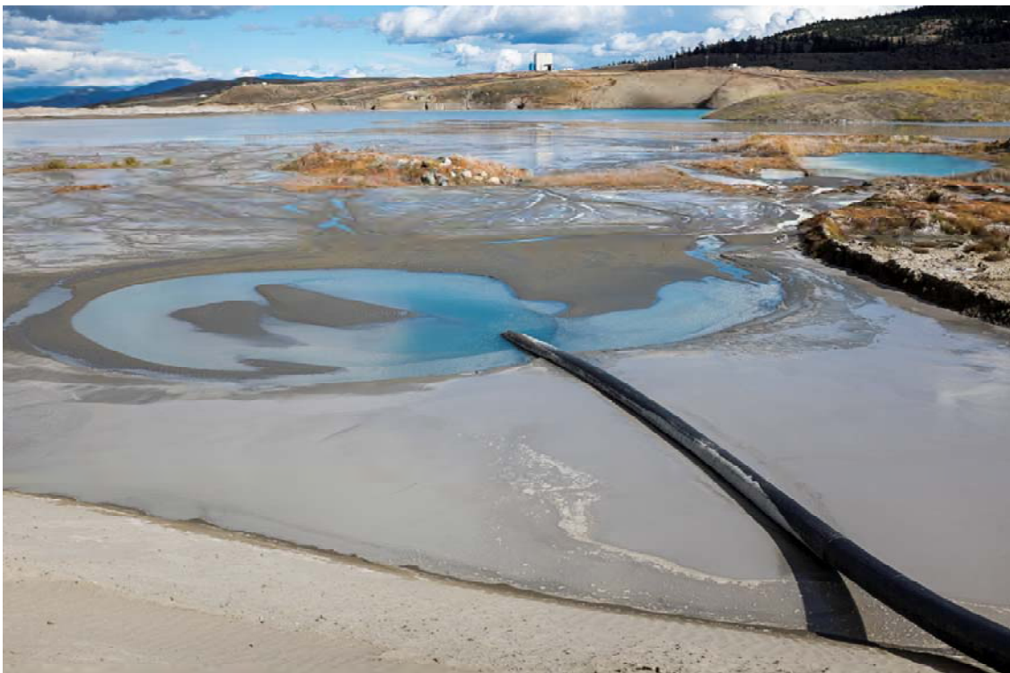
Photo DB16: View looking east at secondary overflow discharge line on beach upstream of sand cell at left abutment of Dam B. Dam C and South Dam visible in the top left and right of photo, respectively.
