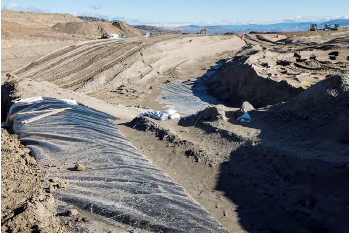
Photo DB21: View looking northeast at exposed liner at right abutment of Dam B and left abutment of Dam C. Note damage to liner caused during excavation to expose liner to be repaired.
