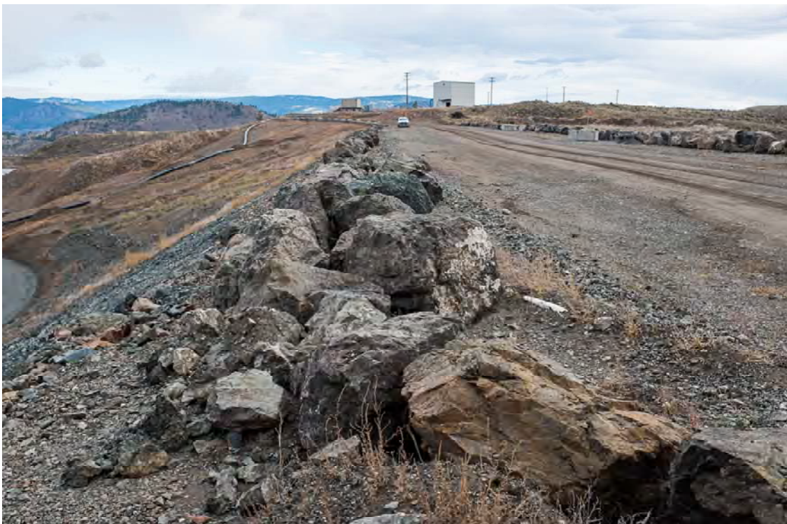
Photo SD08: View of South Dam upstream face and crest from right abutment looking toward left abutment. Primary cyclone visible in background.
