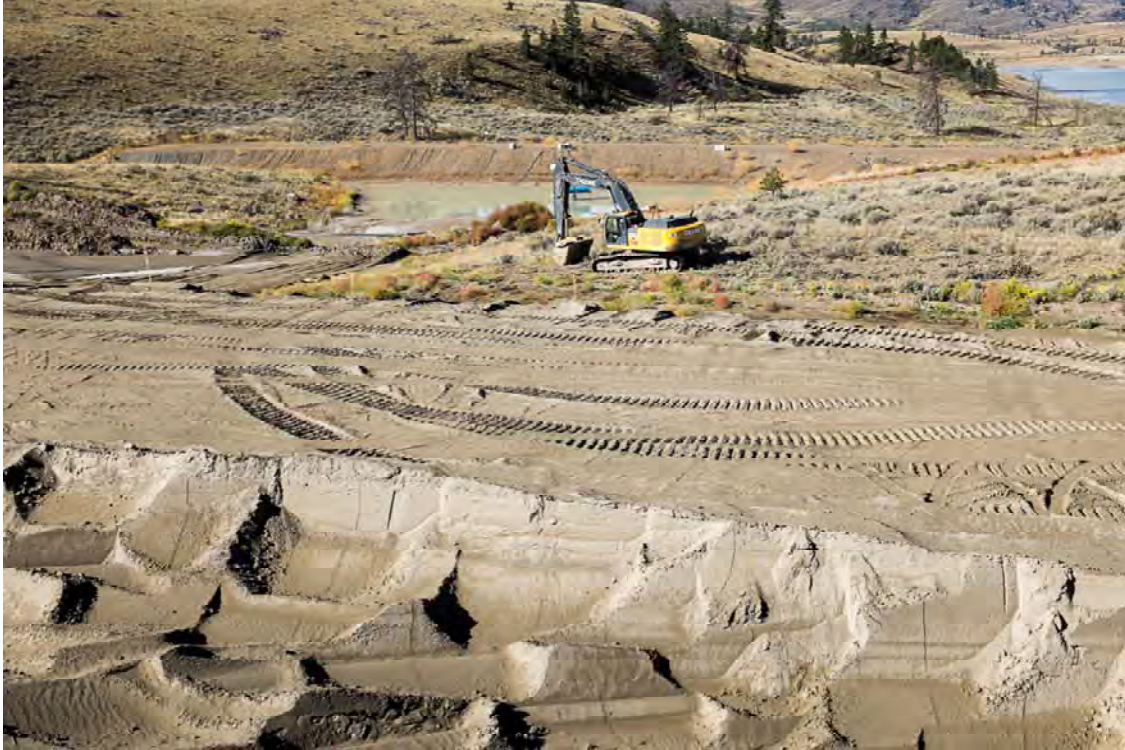
Photo DA15: View looking west at downstream toe of Dam A and Seepage Pond 1. Teck TSF visible in upper right of photo.
