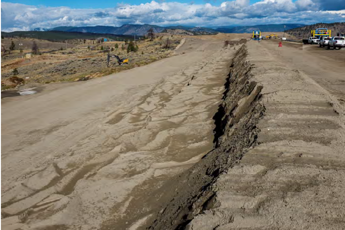
Photo DA21: View looking north at Dam A downstream slope and crest from left abutment looking toward right abutment. Note stepped downstream slope from mining of hydraulically placed sand.
