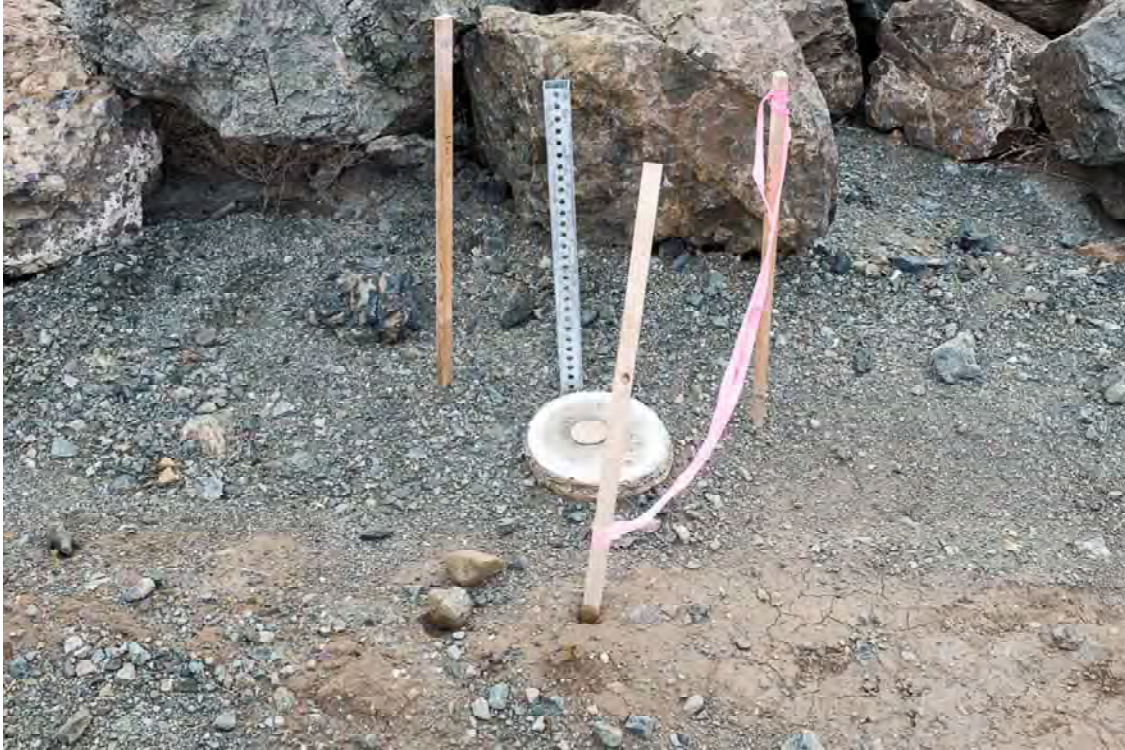
Photo SD25: View of survey monument on the downstream crest of the South Dam near the mid-point of the dam looking east. Note lack of Lock-Block protection.
