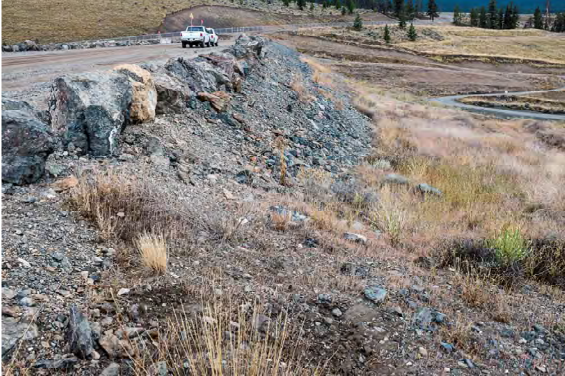
Photo SD01: View of South Dam upstream face and toe from left abutment looking toward right abutment.
