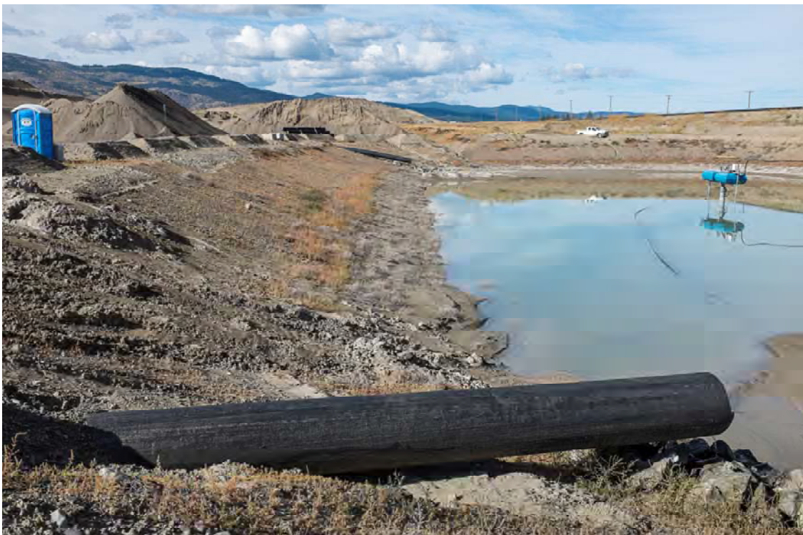
Photo S308: View of south and west sides of Seepage Pond 3 from south east corner. Filter stockpiles visible in background left of photo.
