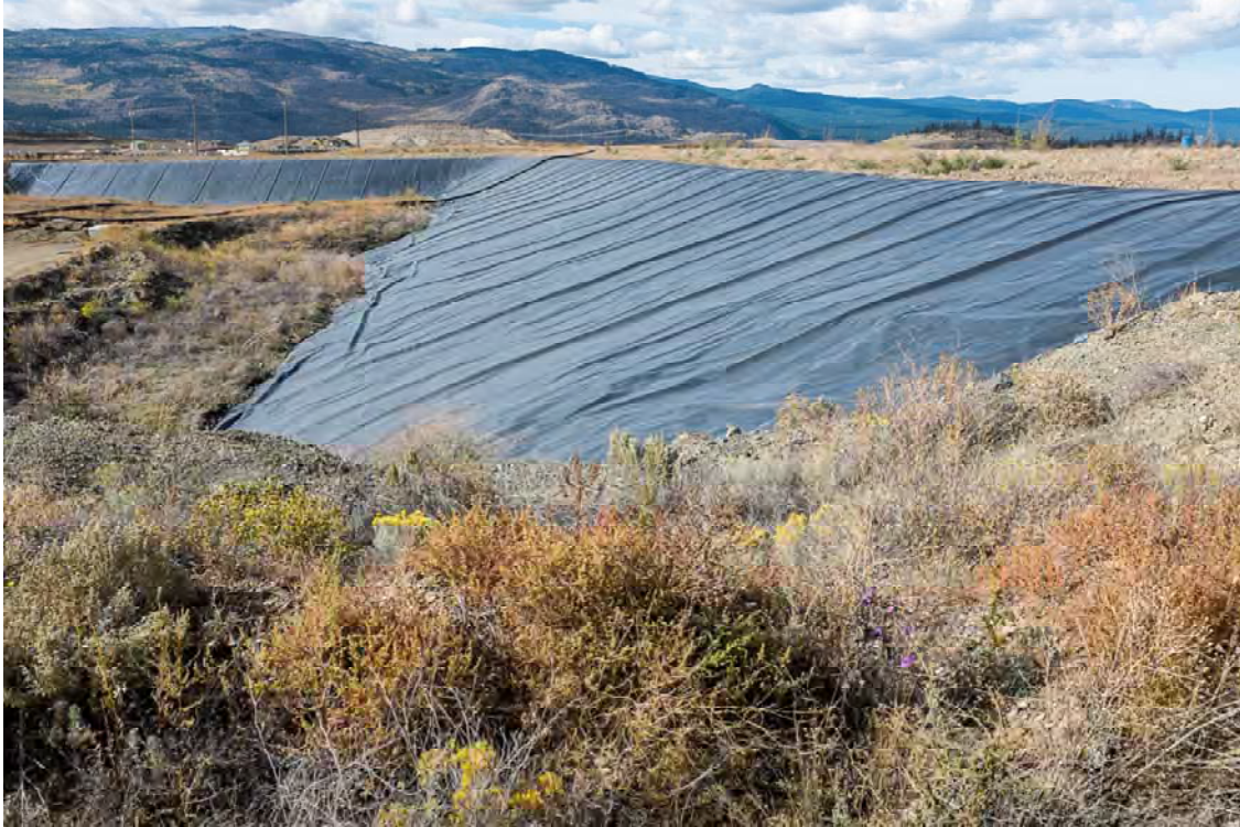
Photo PD03: View of the upstream face and toe of the Pothook Dam at the right abutment. Note pipeline draped down the upstream face of the dam over liner in the background.
