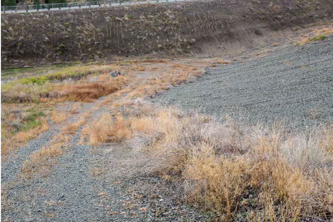
Photo SD19: View of the downstream toe and downstream face of the South Dam from the mid-point of the left abutment.
