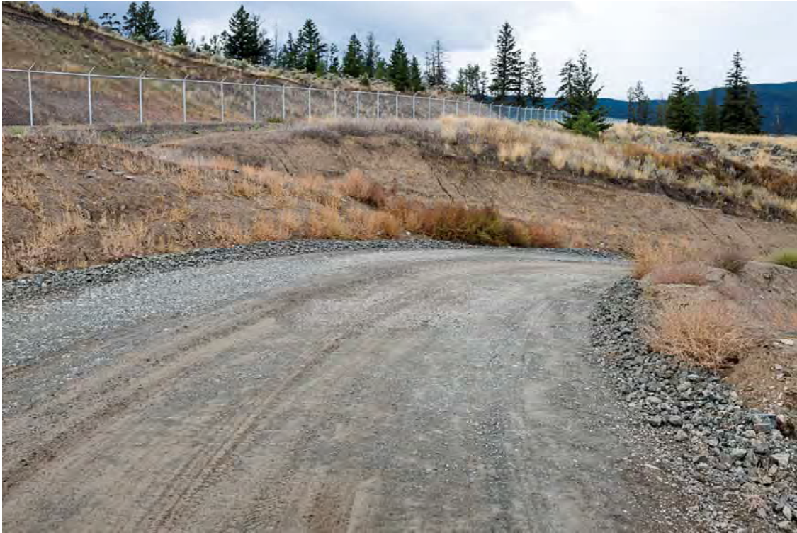
Photo SD09: View of right abutment of South Dam from right abutment crest looking south.
