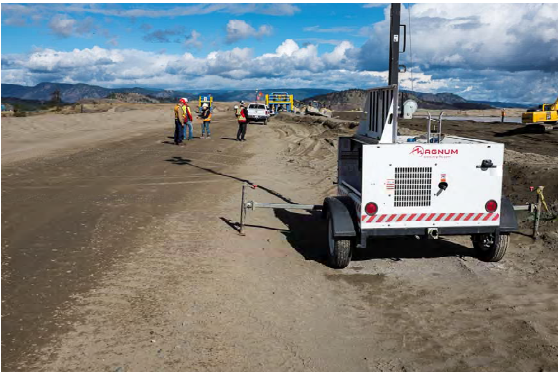
Photo DA22: View looking north at crest of Dam A and upstream sand cell. Dam C visible at top right of photo.
