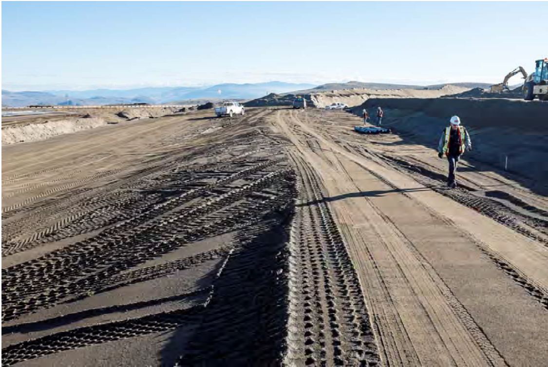
Photo DC23: View looking northeast at crest of Dam C from adjacent to left abutment of Dam C.
