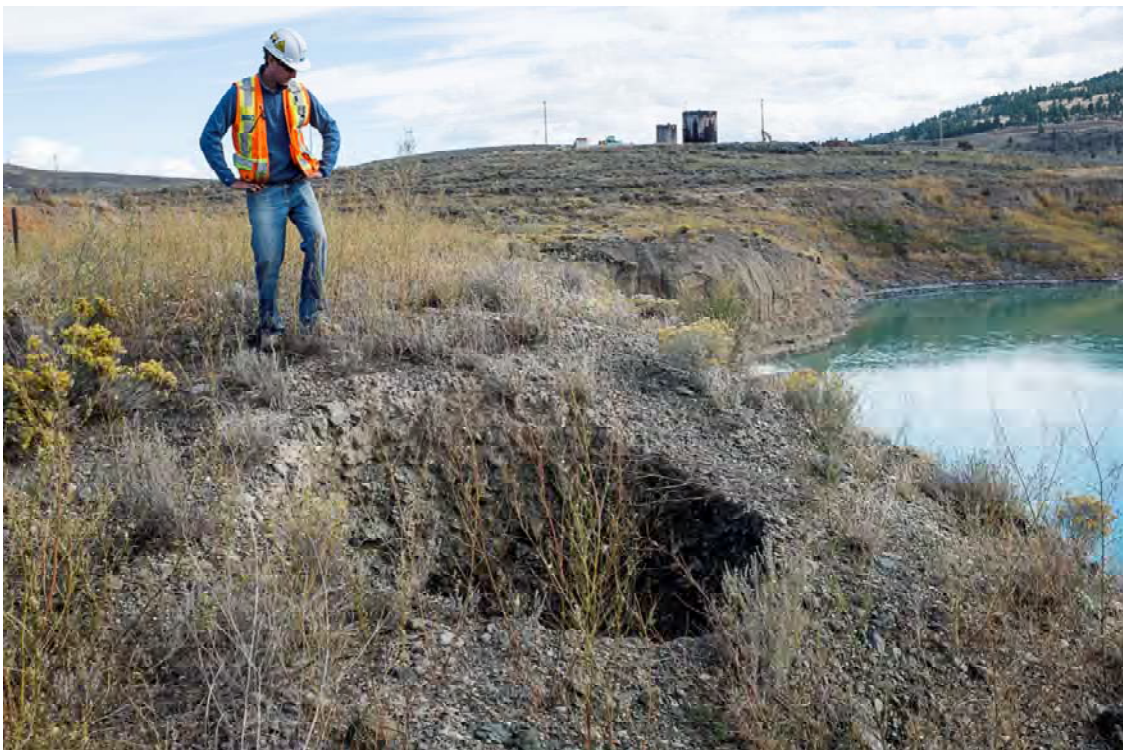
Photo PD34: View looking east at sinkholes in till along the north rim of the Pothook Pit between the Pothook Dam and the Emergency Spillway. Source of water likely pipelines from Afton Pit.
