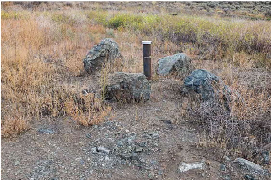
Photo SD26: View of monitoring well monument at the downstream toe of the South Dam looking northeast.
