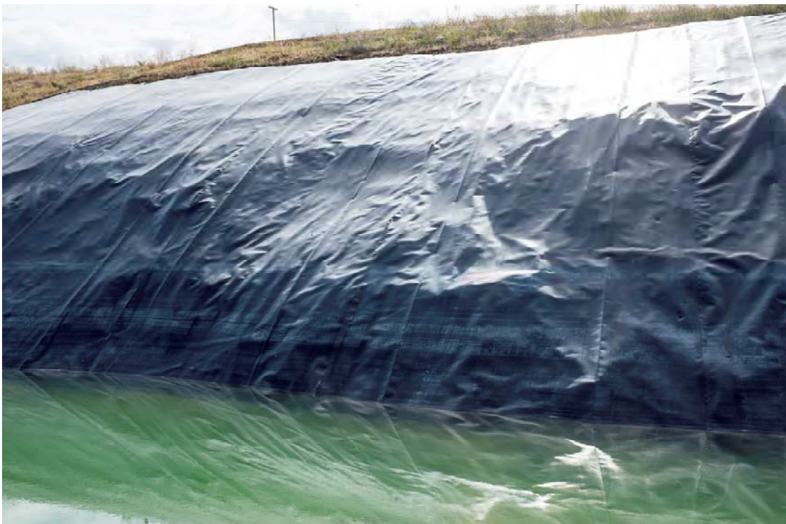
Photo PD14: View of the liner on the upstream face of the Pothook Dam adjacent to the left abutment looking south. Note various punctures across the entire liner.
