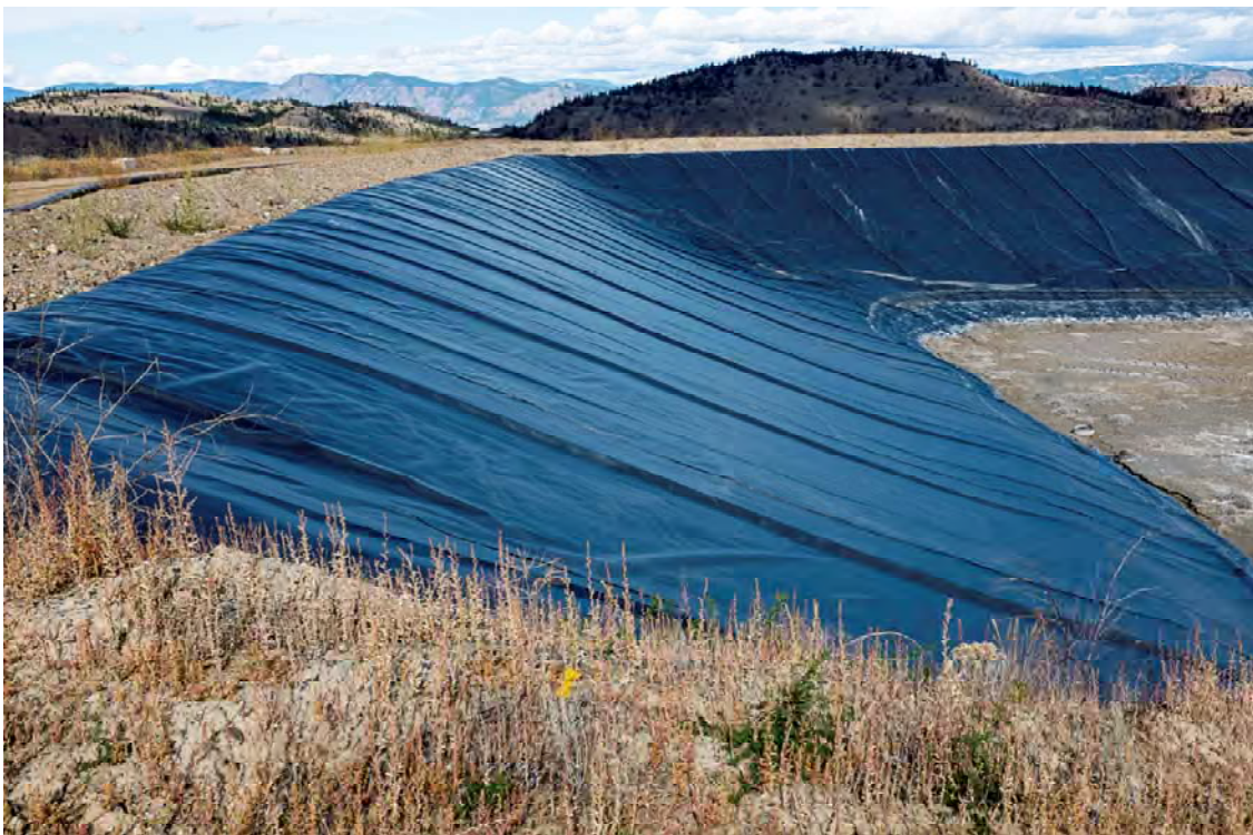
Photo PD22: View of upstream face of Pothook Dam at first dogleg from the tailings pipeline ramp looking north. Note high water mark on liner at upstream toe.
