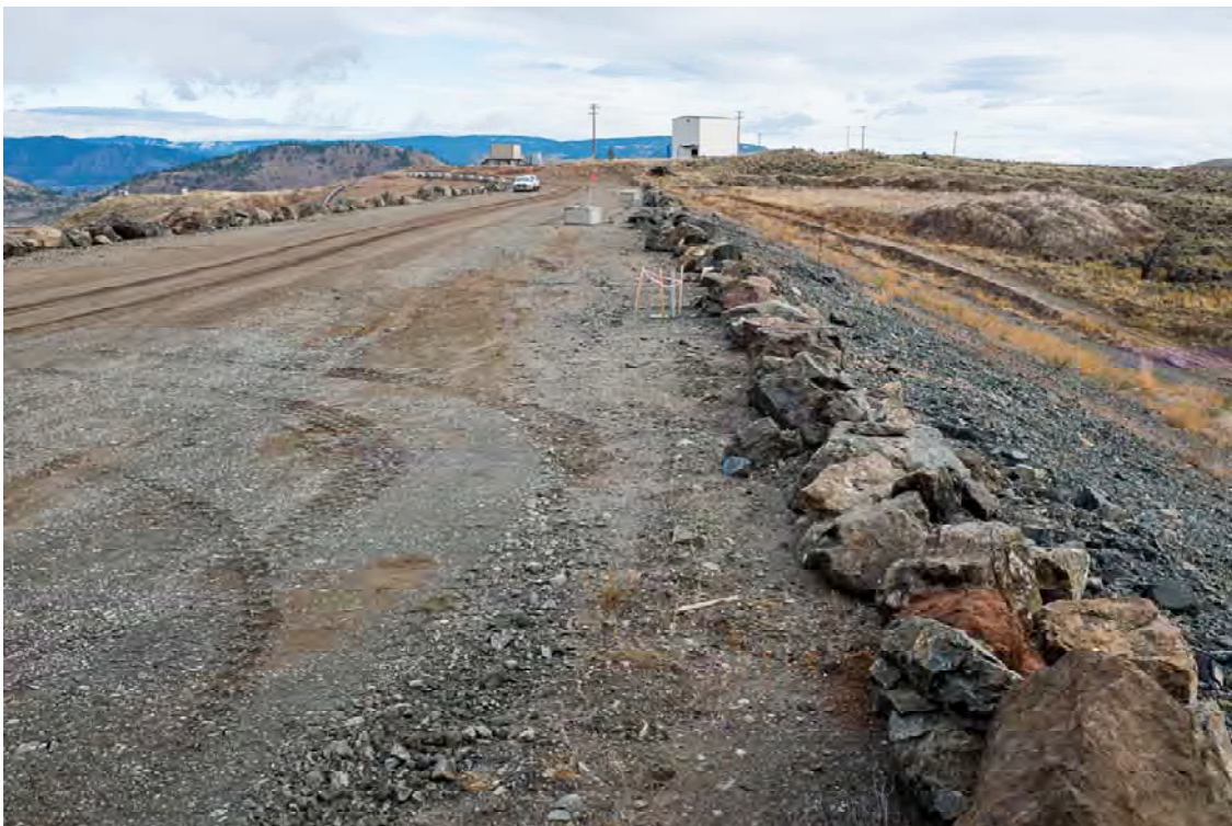
Photo SD12: View of crest and the downstream face of the South Dam from the right abutment.
