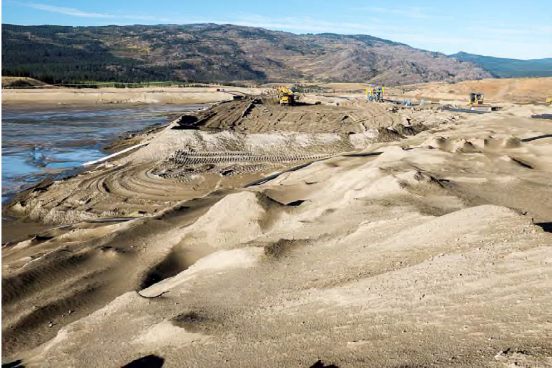
Photo DC11: View of Upstream sand cells of Dam C looking west. Dam B visible in the background. Note mining of cyclone sand for mechanical placement elsewhere on Dam C.
