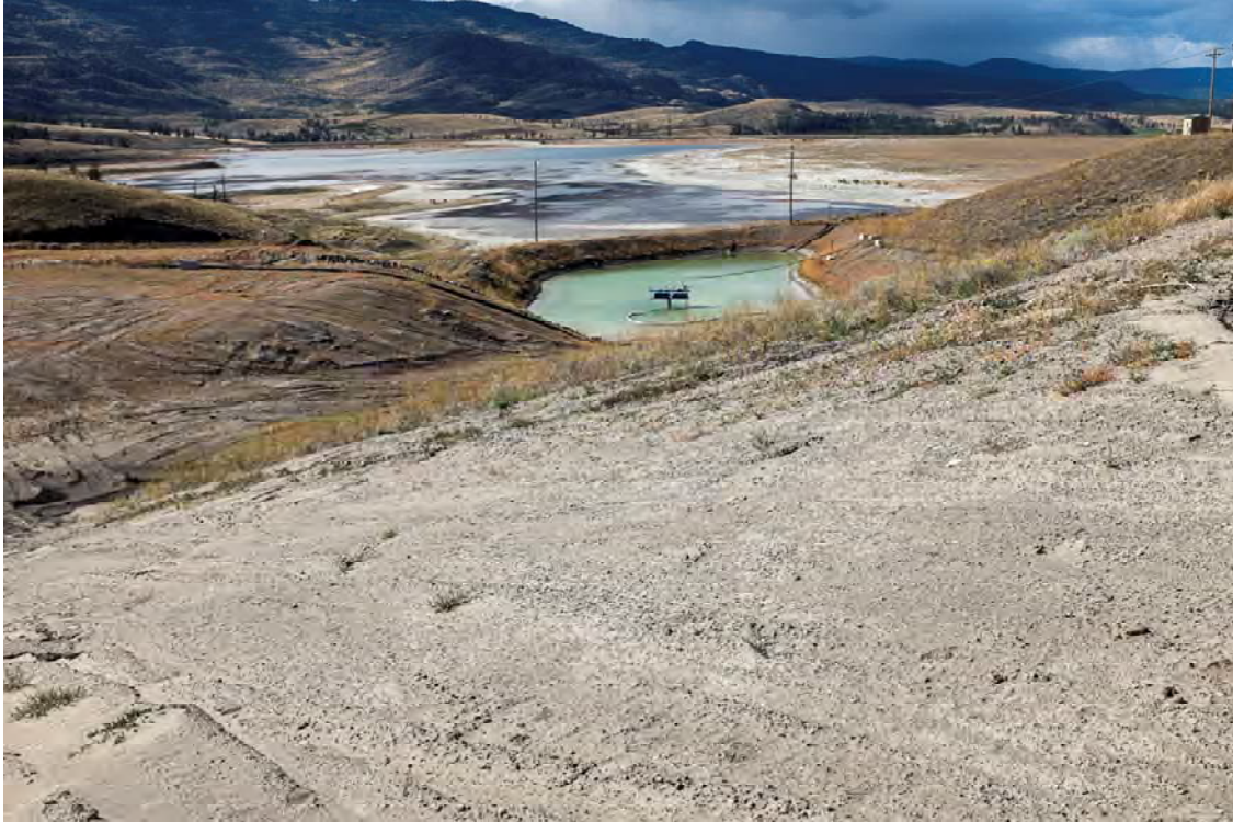
Photo S201: View looking west at Seepage Pond 2 from the downstream face of Dam B. Teck TSF visible in the background.
