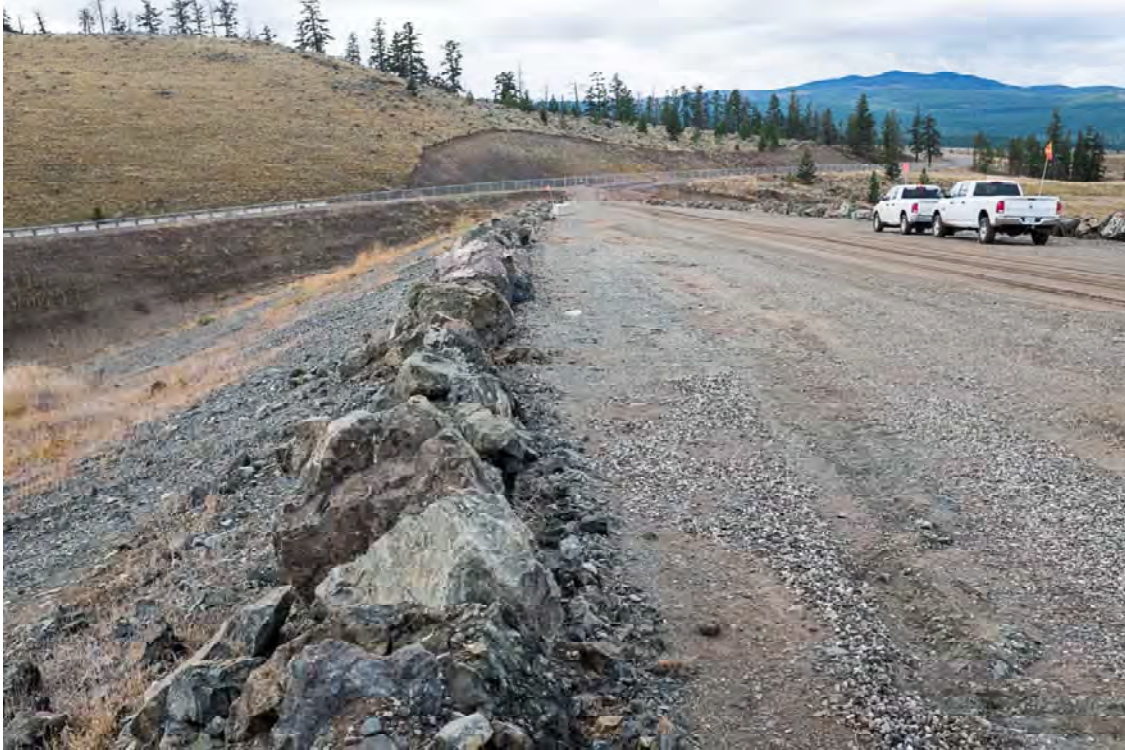
Photo SD21: View of the crest and downstream face of the South Dam from the left abutment crest looking toward the right abutment.
