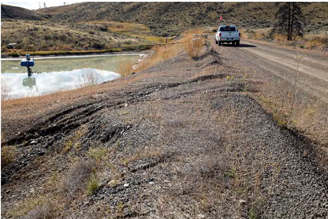
Photo S102: View of Seepage Pond 1 Dam crest and upstream face from right abutment.
