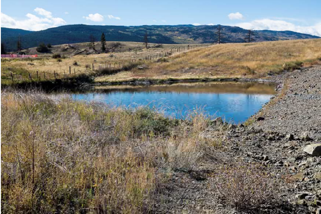
Photo WD15: View of ponding at the downstream toe of the West Dam from just east of the downstream toe looking west.
