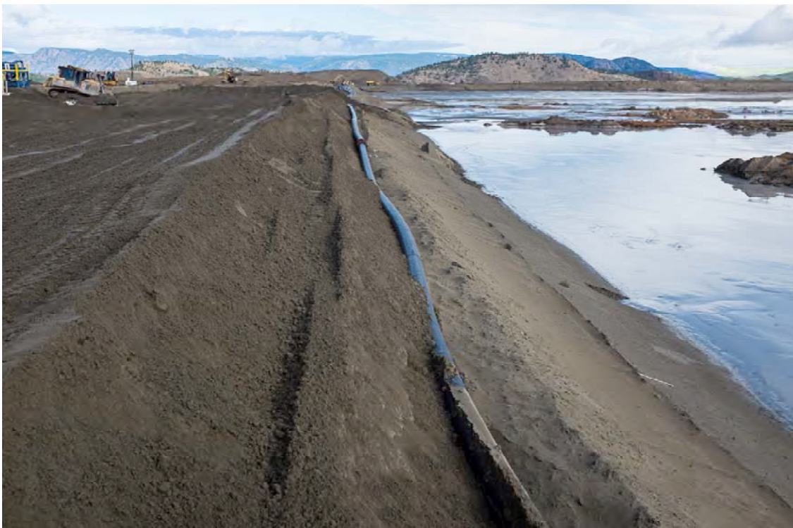
Photo DA04: View looking north at upstream end of sand cell and tailings beach on Dam A. Dam C visible in background right of photo.
