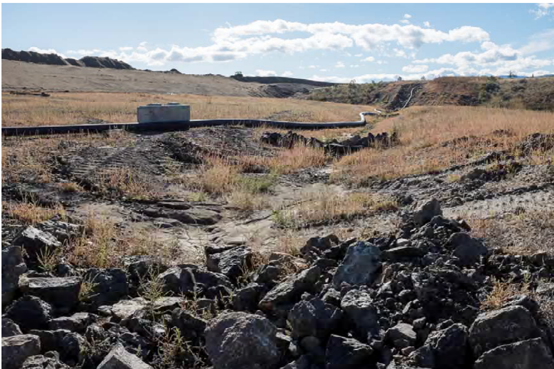
Photo S202: View of the inlet channel and check berms upslope of Seepage Pond 2 looking southwest. Dam B visible in the background.
