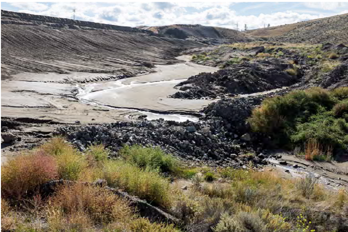
Photo S112: View of downstream toe of Dam A from immediately upstream of Seepage Pond 1. Note accumulation of sediment at toe of dam.
