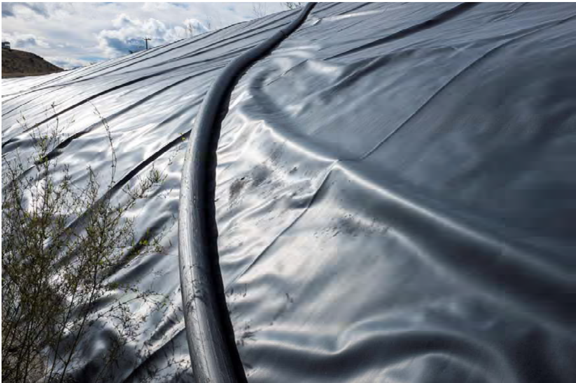
Photo PD10: View of abrasion damage and punctures in liner on upstream face of the Pothook Dam due to a waterline draped over liner south of the tailings pipeline ramp.
