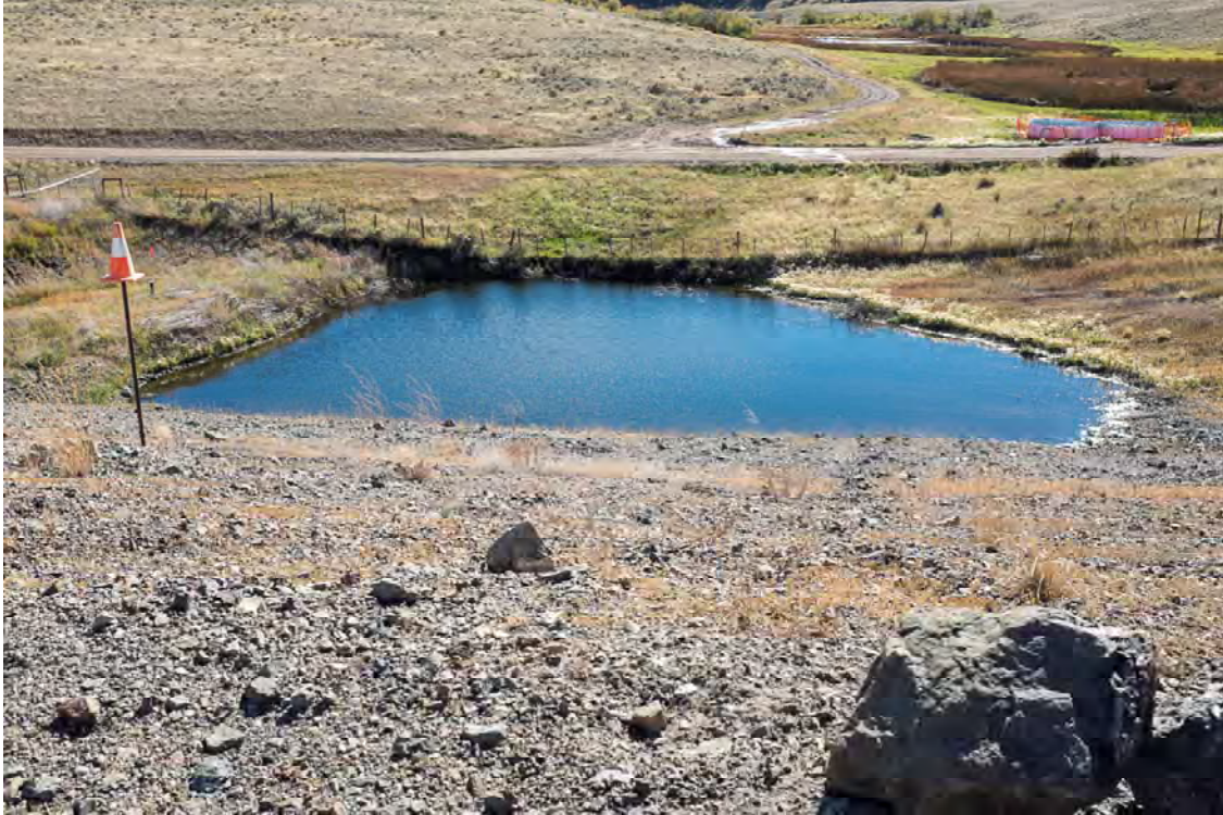
Photo WD19: View of ponding at the downstream toe of the West Dam from the crest at the mid-point the West Dam. Note settlement plate riser pipe and monitoring well monument at the middle left of the photo.
