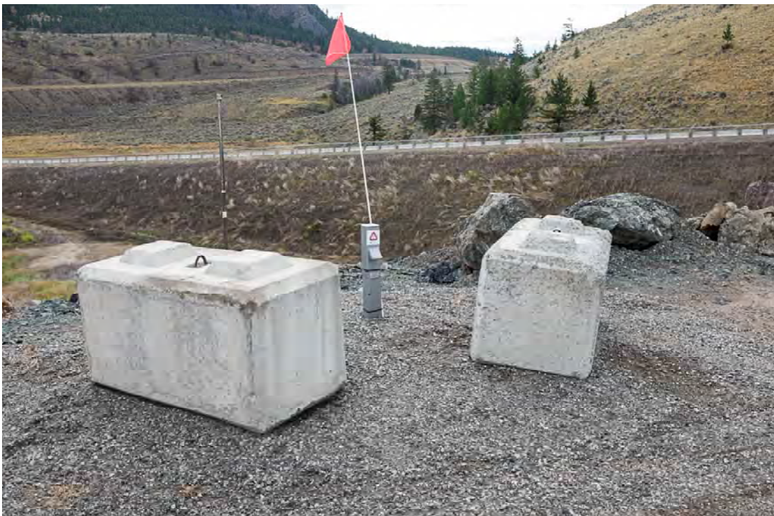
Photo SD24: View of Lock-Block protection around inclinometer monument on downstream crest looking east near mid-point of South Dam. Settlement plate riser pipe visible in background.
