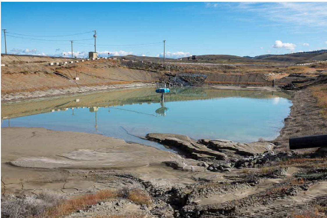
Photo S310: View of north and east sides of Seepage Pond 3 from south west corner. Tailings line visible in background of the photo.
