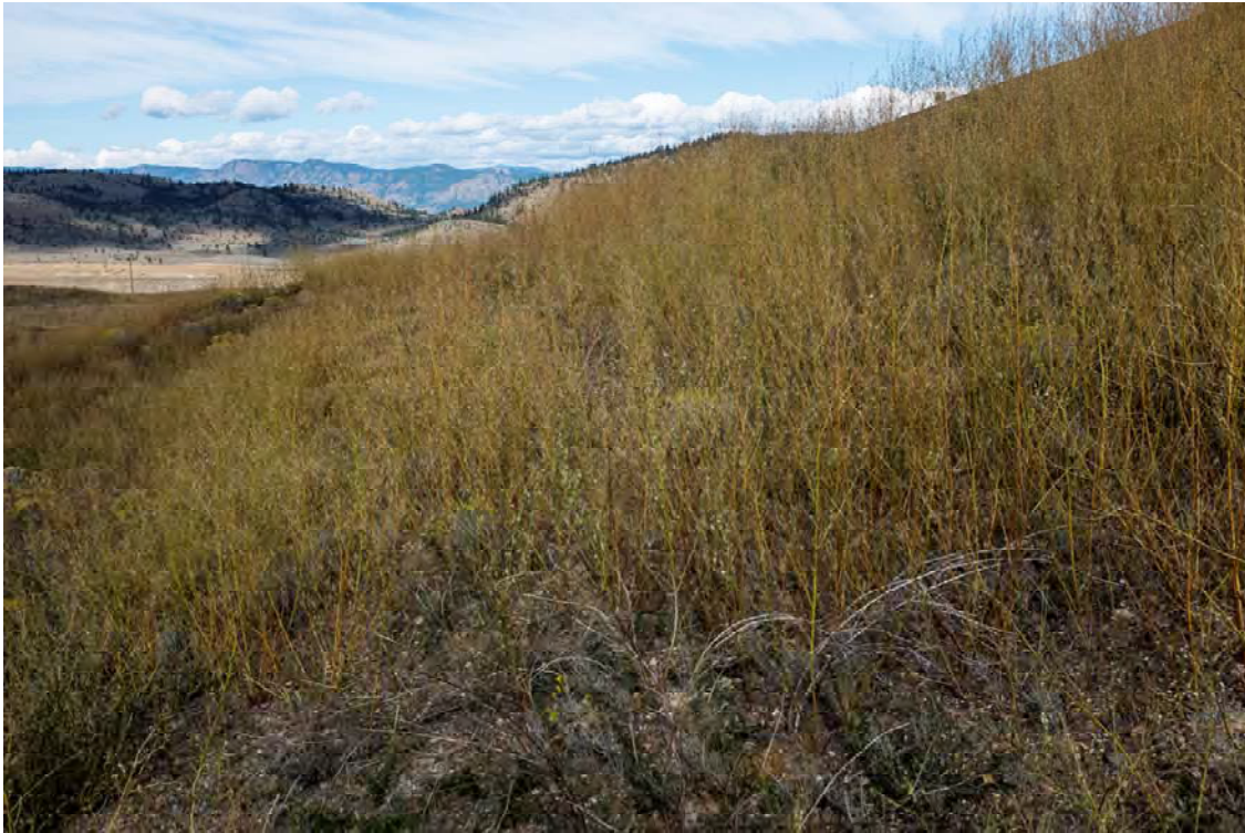
Photo PD29: View looking north at downstream face of Pothook Dam north of the tailings pipeline ramp.
