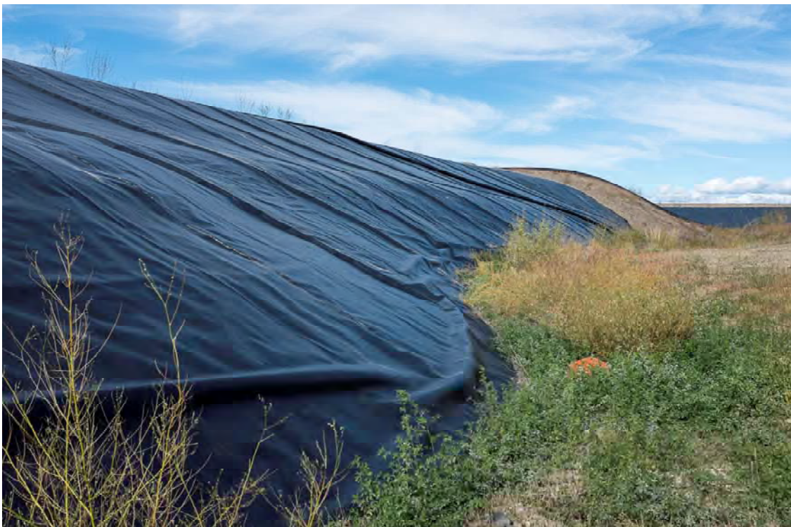
Photo PD12: View of the upstream face and toe of the Pothook Dam from the upstream toe just south of the tailings pipeline ramp looking north.
