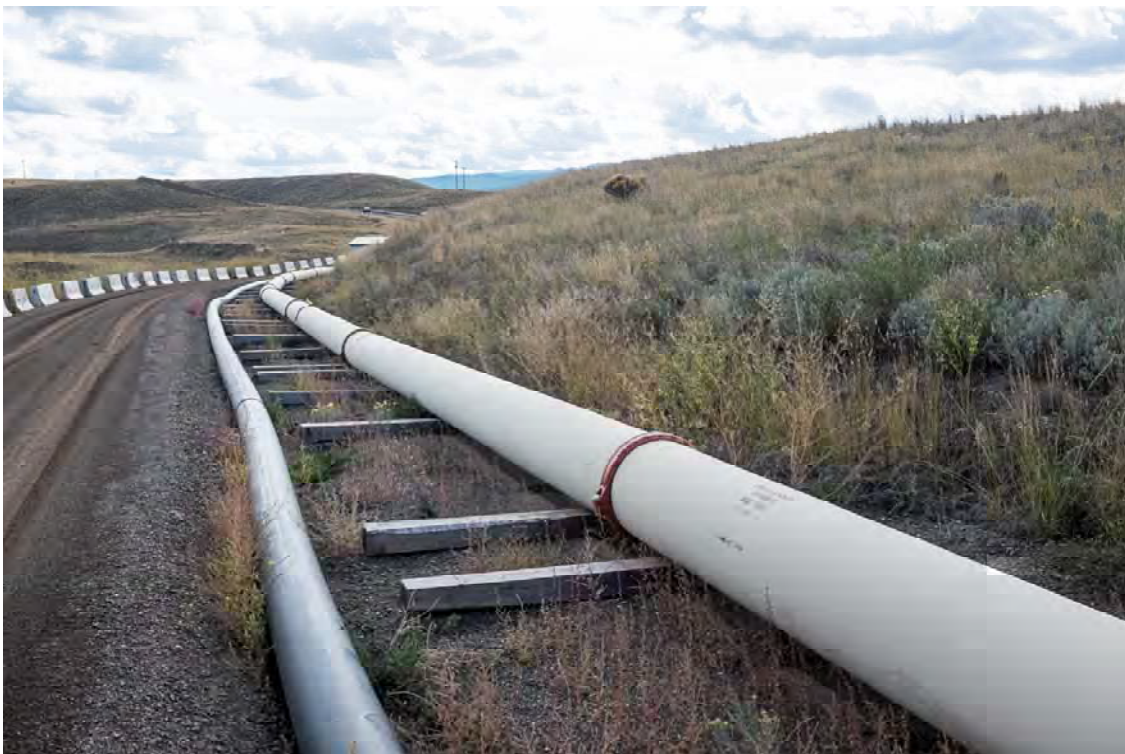
Photo TL06: View looking southeast along steel portion of tailings line from just upslope of mill.
