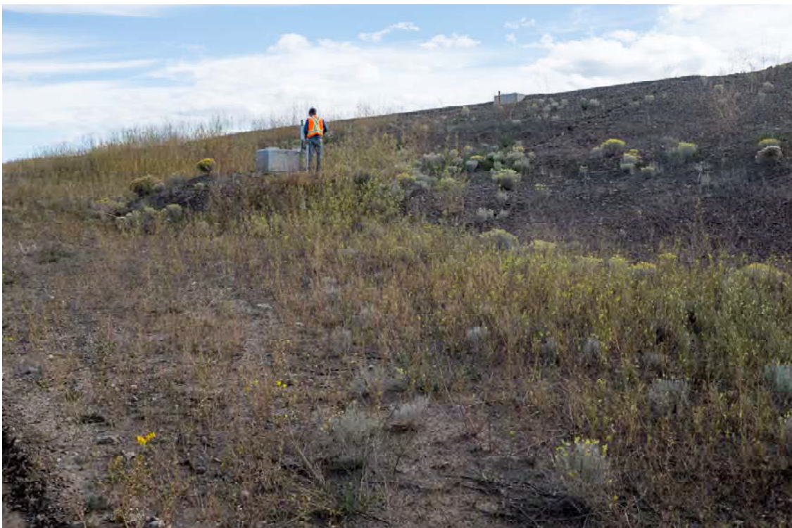
Photo PD30: View looking southeast at instrumentation on the downstream face and toe of the Pothook Dam just east of the first dogleg.
