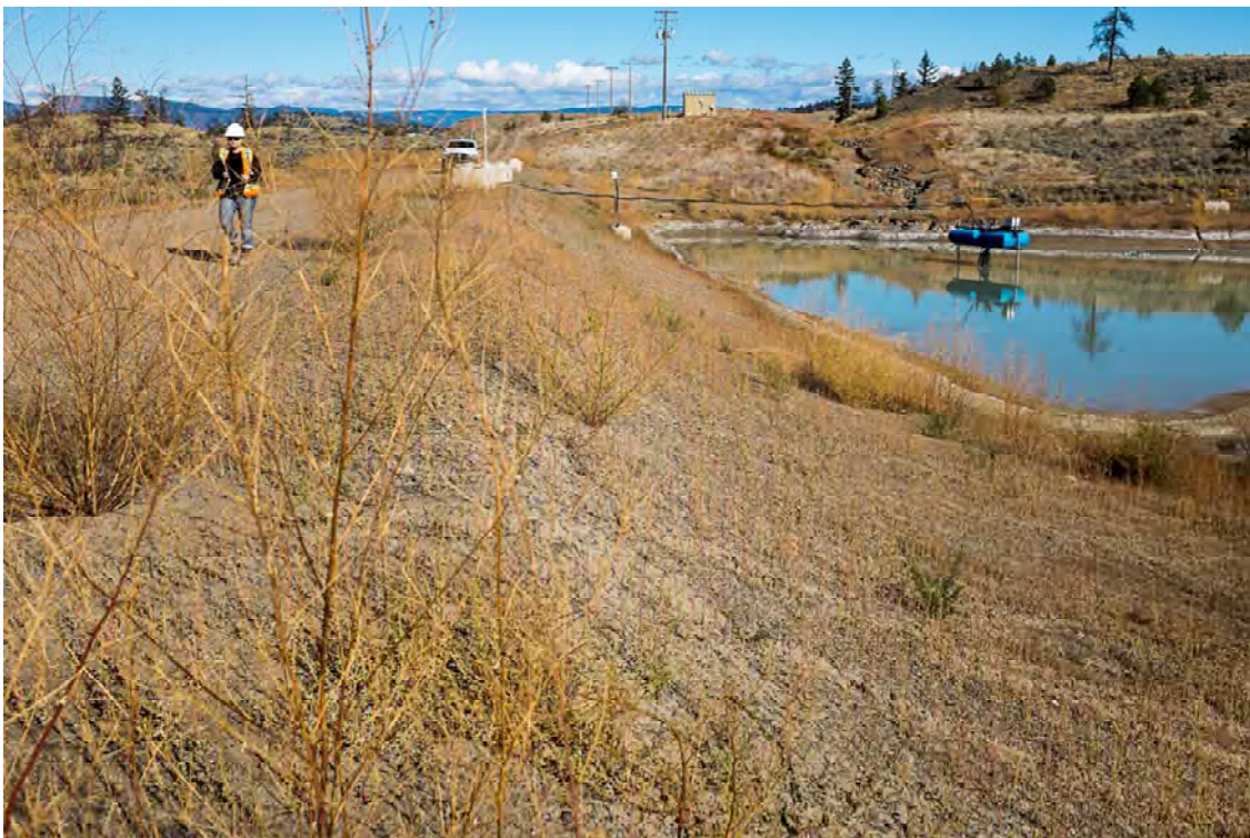
Photo S110: View of upstream face and crest of Seepage Pond 1 Dam crest from left abutment.
