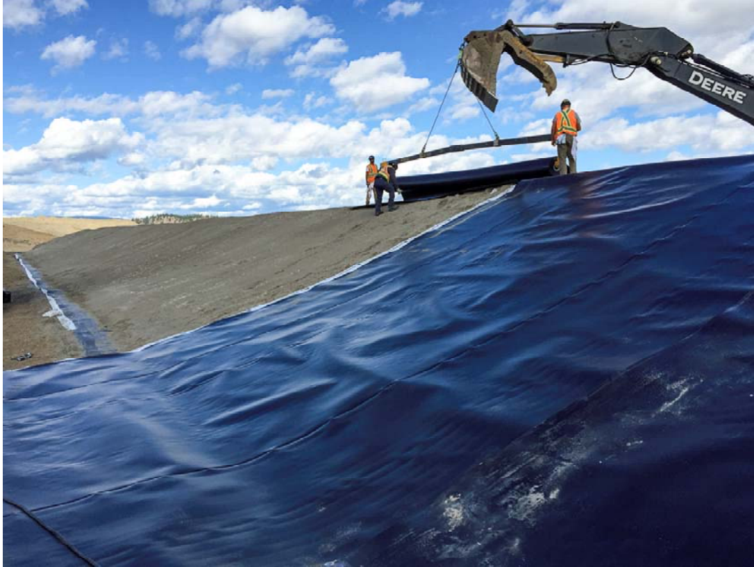
Photo DB23: Liner being placed on Dam B at approximately sta. 1+375 m. View looking northeast.
