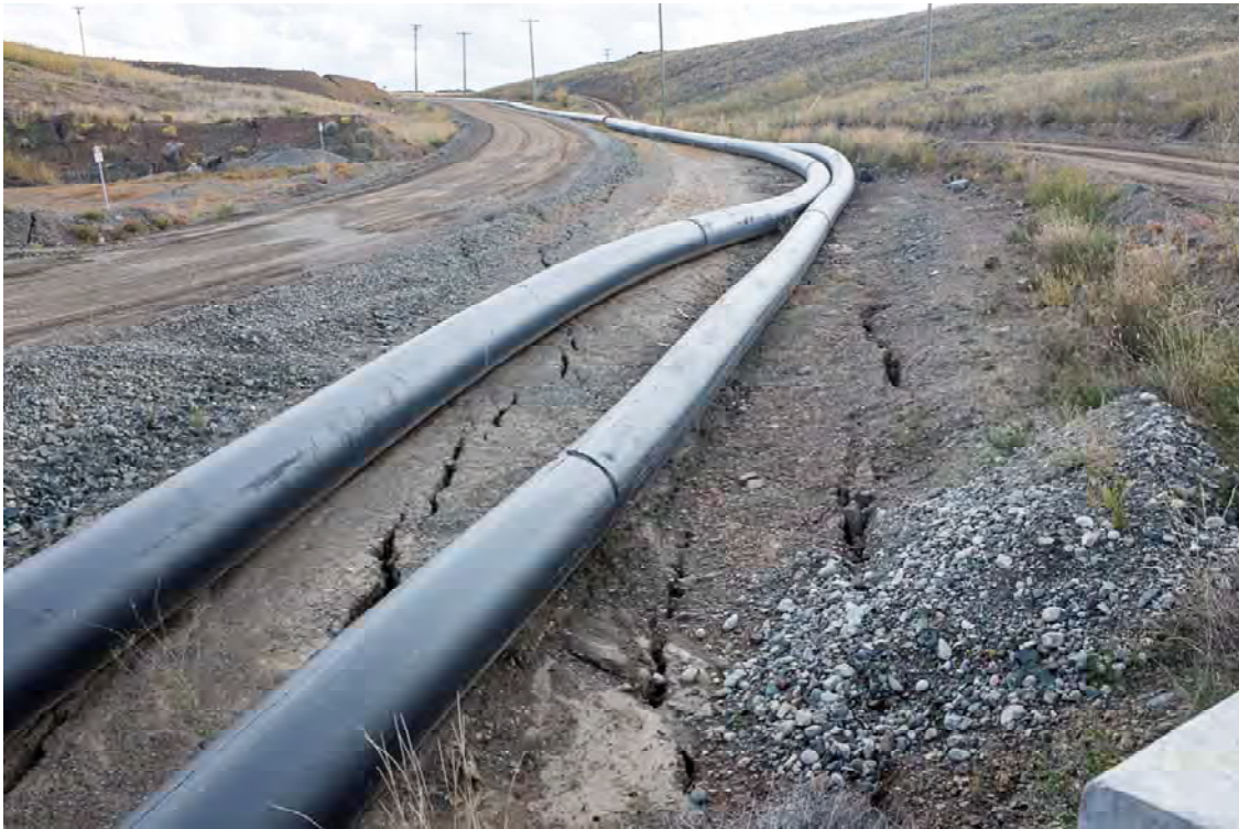
Photo TL03: View looking east at cracking from block cave subsidence along road to tailings facility just upstream of turn-off to Teck TSF. Cracking more pronounced than previous year.
