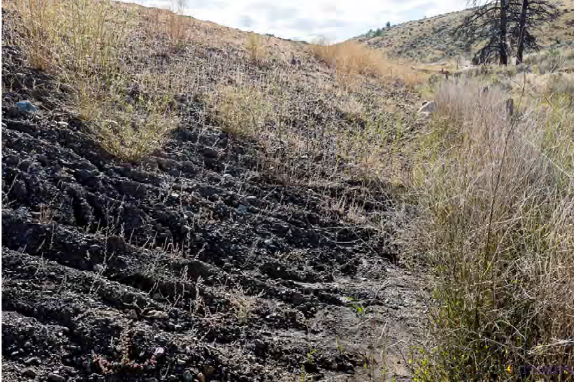
Photo S107: View of downstream face from downstream toe of Seepage Pond 1 Dam looking toward left abutment. Note rilling and vegetation on dam face.
