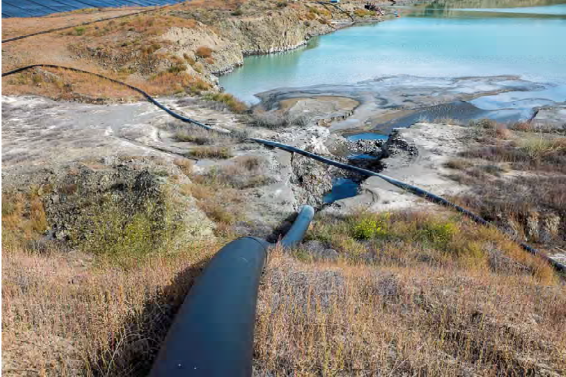
Photo PD21: Tailings pipeline discharge at base of tailings pipeline ramp on upstream face of Pothook Pit adjacent to first dogleg looking east.
