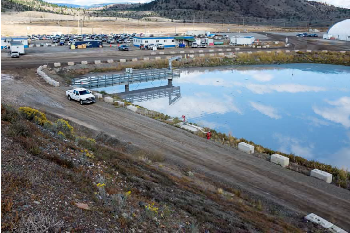
Photo TL11: View of Spill Pond from top of hill adjacent to ore stockpile looking north. Note water level relative to inlet culverts and algae rafts on pond surface at top right of photo.
