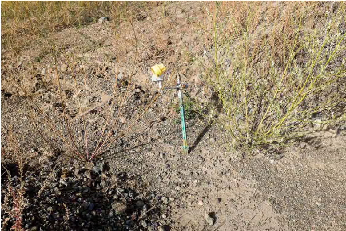
Photo PD25: View of damaged survey prism at the downstream crest of Pothook Dam at the first dogleg.
