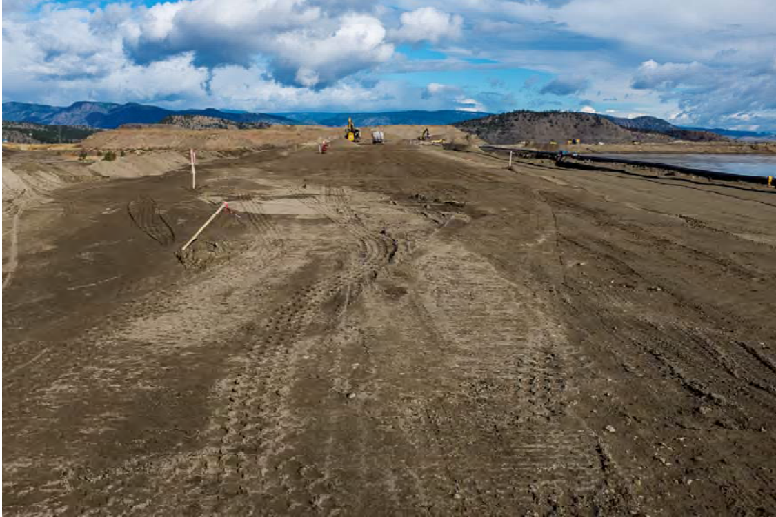
Photo DA09: View looking north at right abutment of Dam A toward Dam B from crest at approximately sta. 1+700 m.
