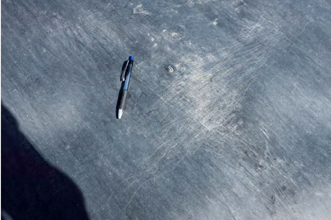
Photo PD05: View of abraision and liner bedding protrusion damage on the liner on Pothook Dam at the downstream toe one third of the way between the right abutment and the first dogleg of the dam.
