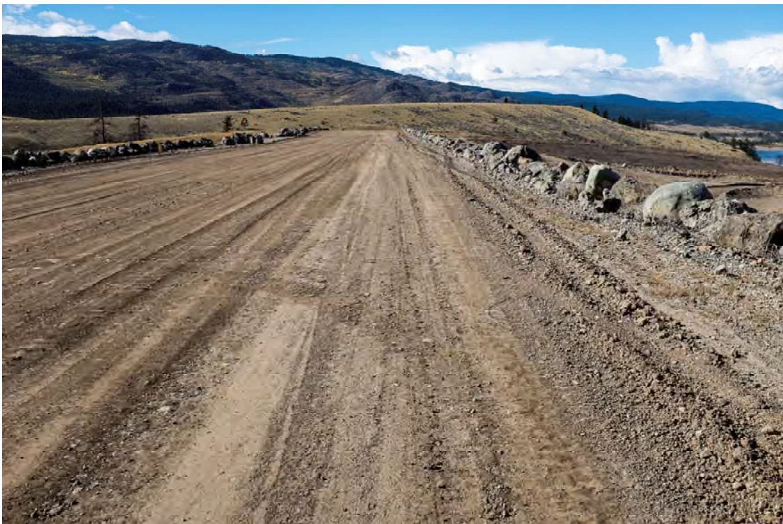
Photo WD02: View looking west at crest of West Dam toward right abutment from left abutment.
