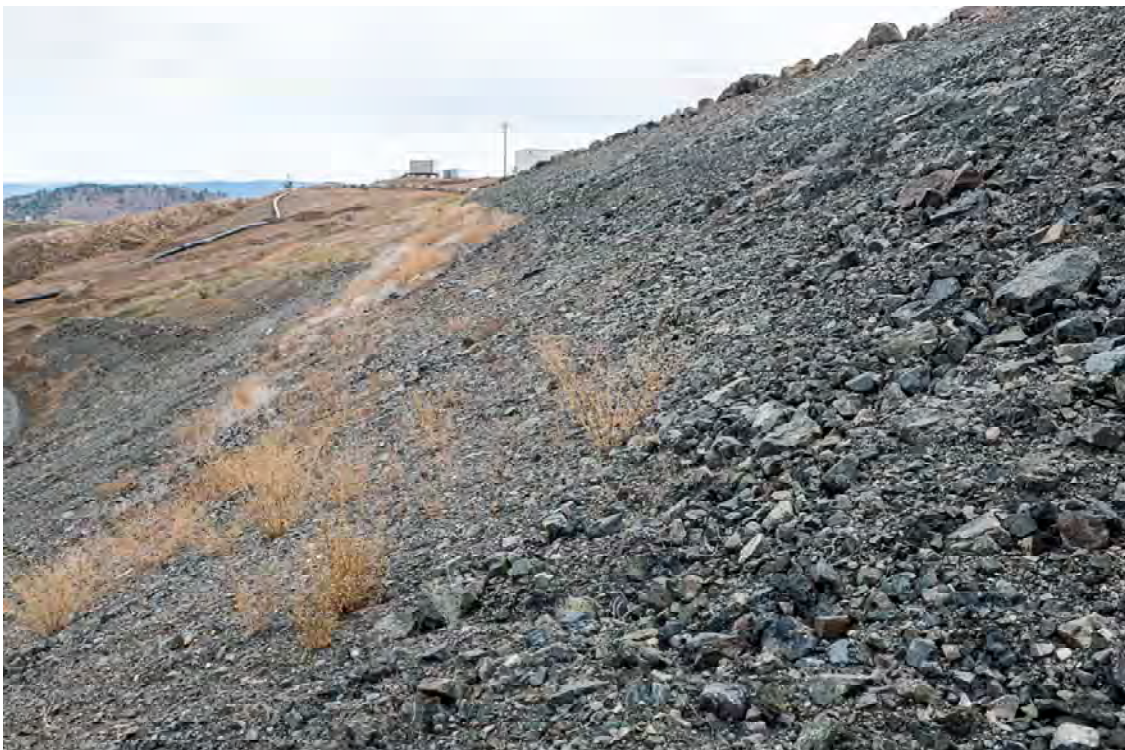
Photo SD06: View of South Dam upstream face and left abutment from mid-way down the slope on right abutment.
