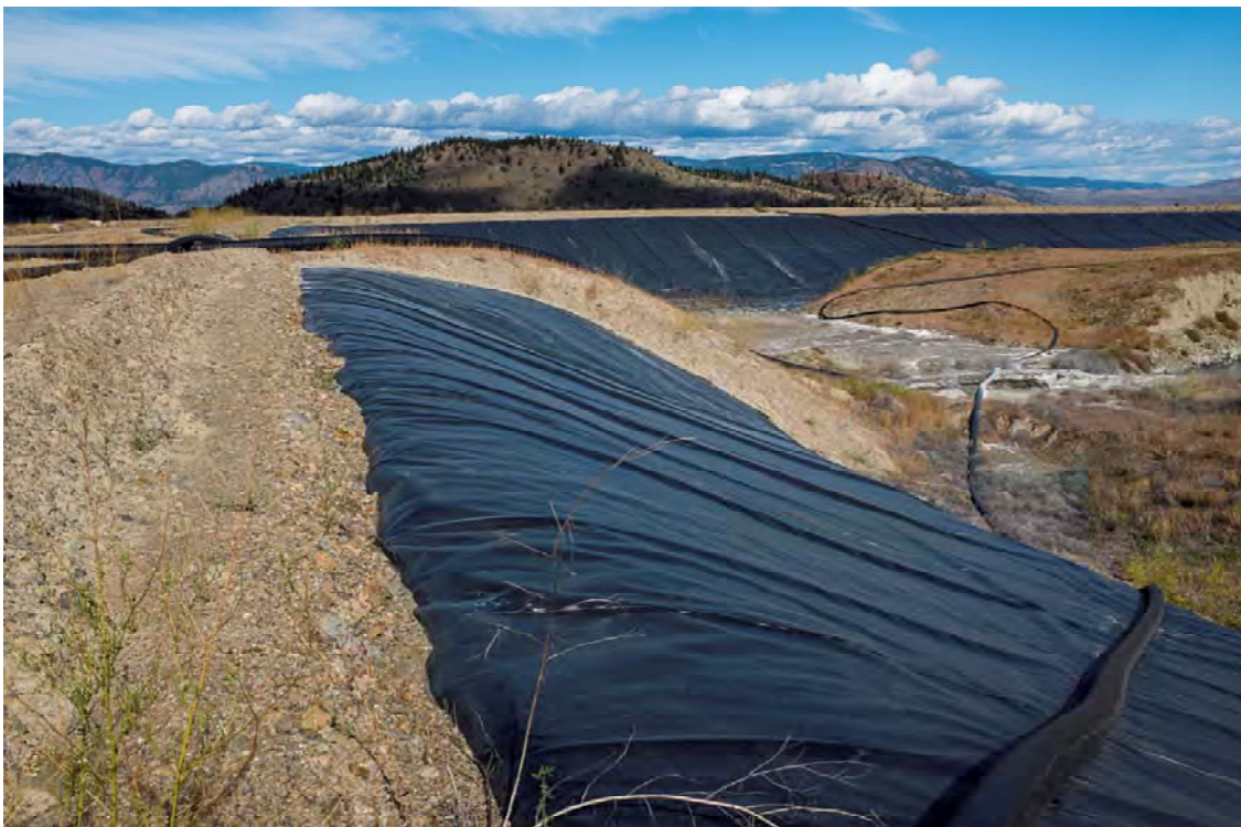
Photo PD20: View of tailings pipeline ramp on upstream face of Pothook Dam adjacent to first dogleg looking north from crest. Note several pipelines on liner on upstream face of dam.
