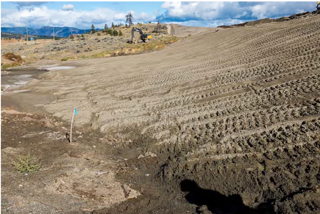
Photo DA18: View looking north at right abutment and downstream face and toe of Dam A from mid-slope of left abutment. Note uniform downstream face and change in slope toward downstream toe. Soft saturated sand at toe of dam.
