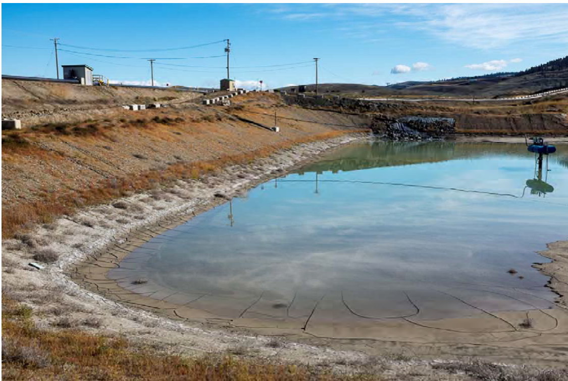
Photo S302: View of the north and east sides of Seepage Pond 3 from the west side.
