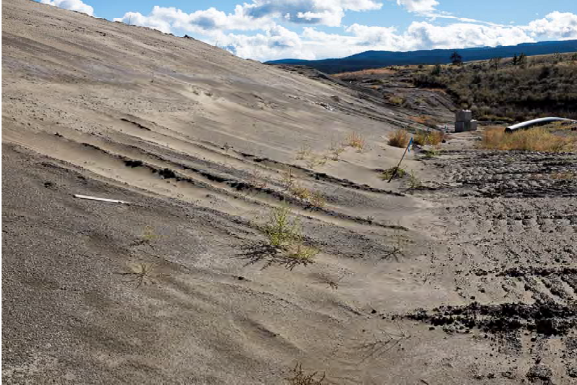
Photo DB07: View looking south at the downstream face of Dam B from the downstream toe at approximately sta. 1+350 m.
