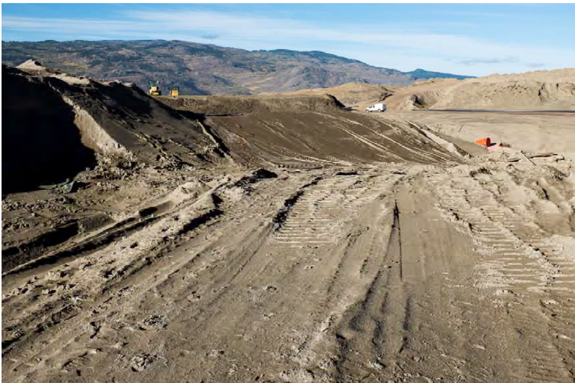
Photo DC22: View looking west toward bend in Dam C at sta. 0+900 m. Note exposed liner at mid-left of photo.
