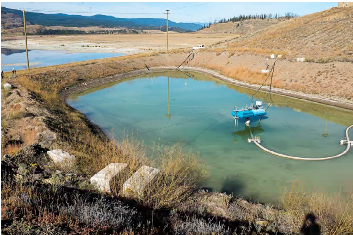
Photo S204: View looking west at Seepage Pond 2 from the inlet channel above impoundment. Teck TSF visible in background. Note erosion on slope between truck and impoundment.
