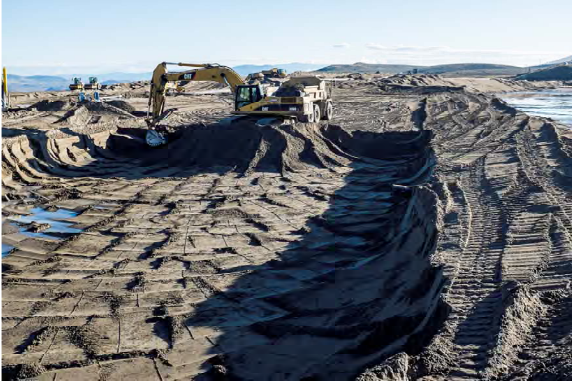
Photo DC13: View of excavation of hydraulically placed sand for use in Dam C construction looking east. Note sand cell decant pipe visible on middle right of photo.
