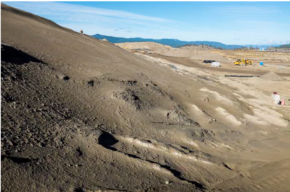
Photo DC24: View looking west from right abutment at downstream face and toe of Dam C. Note uniform downstream slope and filter stockpiles at top right of photo. Downstream face has been sprayed with polymer to prevent dusting.
