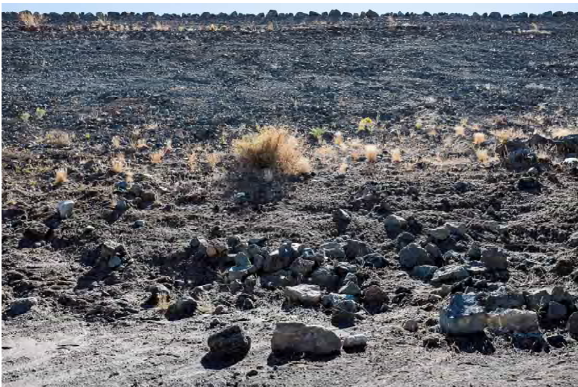
Photo WD08: View of the upstream face of the West Dam from the upstream toe.
