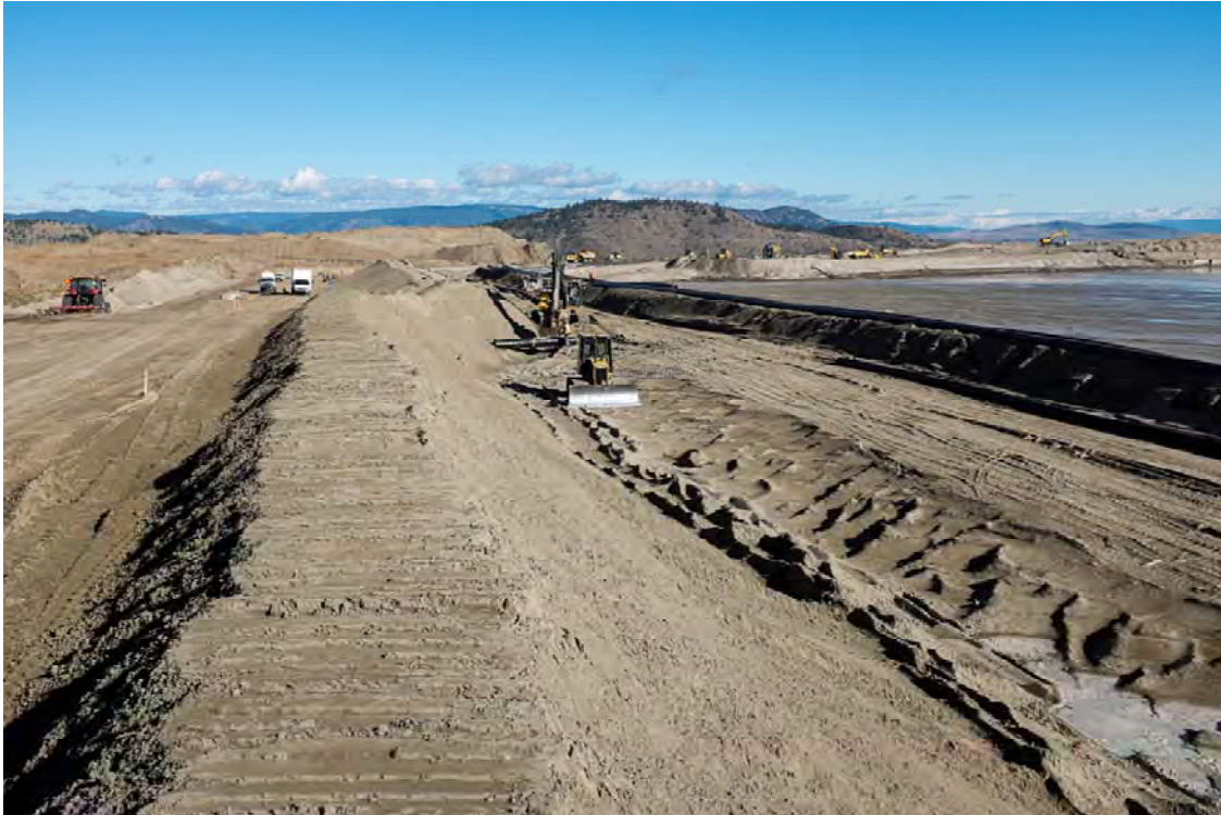
Photo DB19: View looking north at upstream sand cells and crest of Dam B from approximately sta. 1+475 m. Transition between lined and unlined section of Dam B visible in crest offset with lined portion in background.
