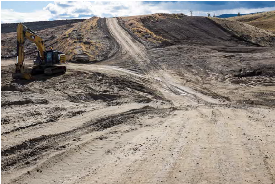
Photo DA02: View looking south at left abutment of Dam A. Dam alignment follows road alignment. Note stakes on middle right of photo denoting downstream edge of till core to be placed as part of the 2014 construction season.
