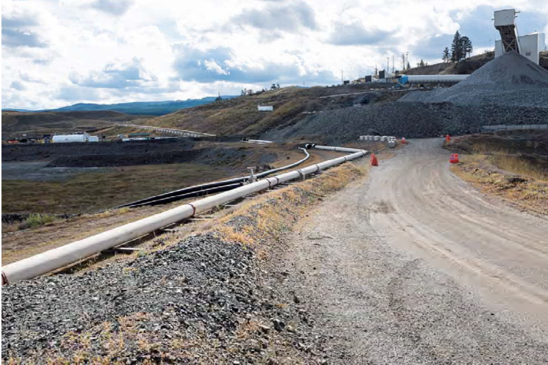
Photo TL07: View looking southwest at steel tailings line adjacent to ore stockpile. Note sections in culverts, and drain line to spillpond.
