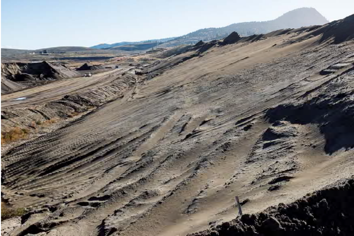
Photo DC29: View looking east toward right abutment of Dam C from downstream toe at approximately sta. 0+950 m.
