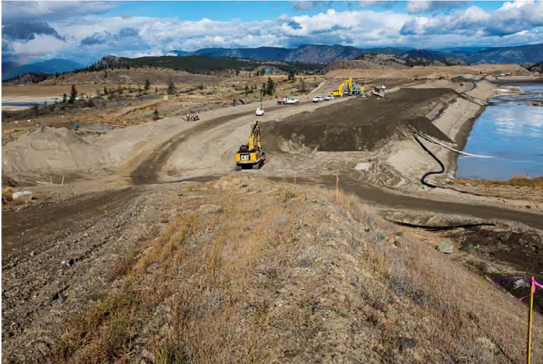
Photo DA01: View looking north from above left abutment of Dam A. Teck TSF and Seepage Pond 1 visible at top left of photo. Note upstream sand cell preparation. Dam B and Dam C visible at top right of photo.
