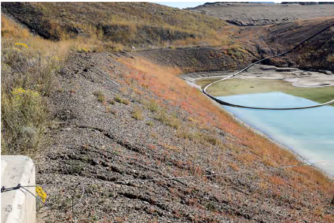
Photo S208: View of north perimeter of impoundment and inlet of Seepage Pond 2. Note minor rilling of impoundment slope in foreground. Dam B visible in background right of photo.
