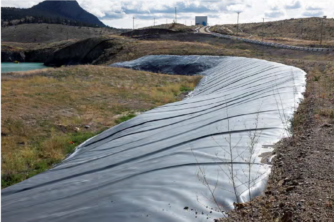
Photo PD19: View of the left abutment and second dogleg of Pothook Dam looking southeast from crest. Primary cyclone and tailings line visible in background of photo. Note reclaim barge in Pothook Pit in upper left of photo.
