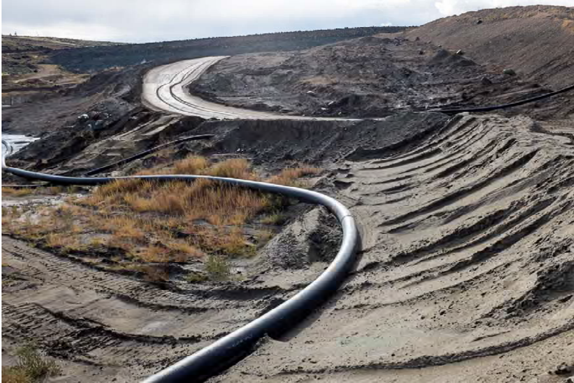
Photo DA03: View looking south at left abutment of Dam A from upstream limit of upstream sand cell at left abutment. West Dam visible at top of photo.
