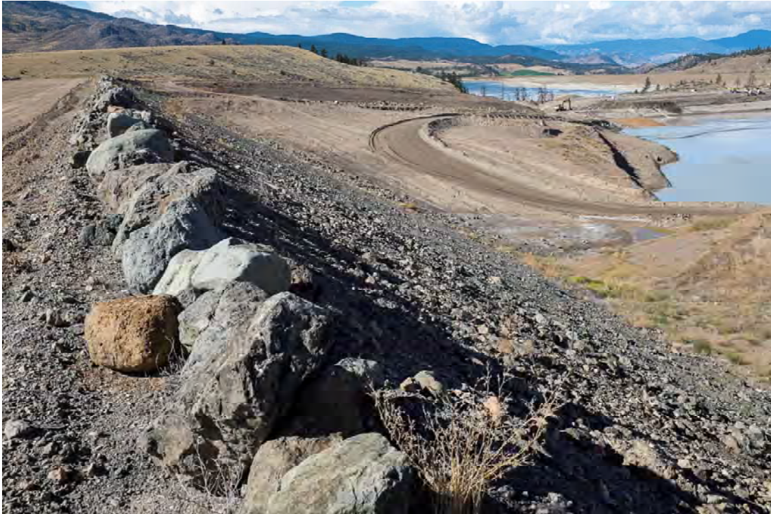
Photo WD03: View of upstream face and toe of West Dam from left abutment. Dam A and Teck TSF visible in upper right of photo. Note location of tailings and pond relative to the upstream toe of the West Dam.
