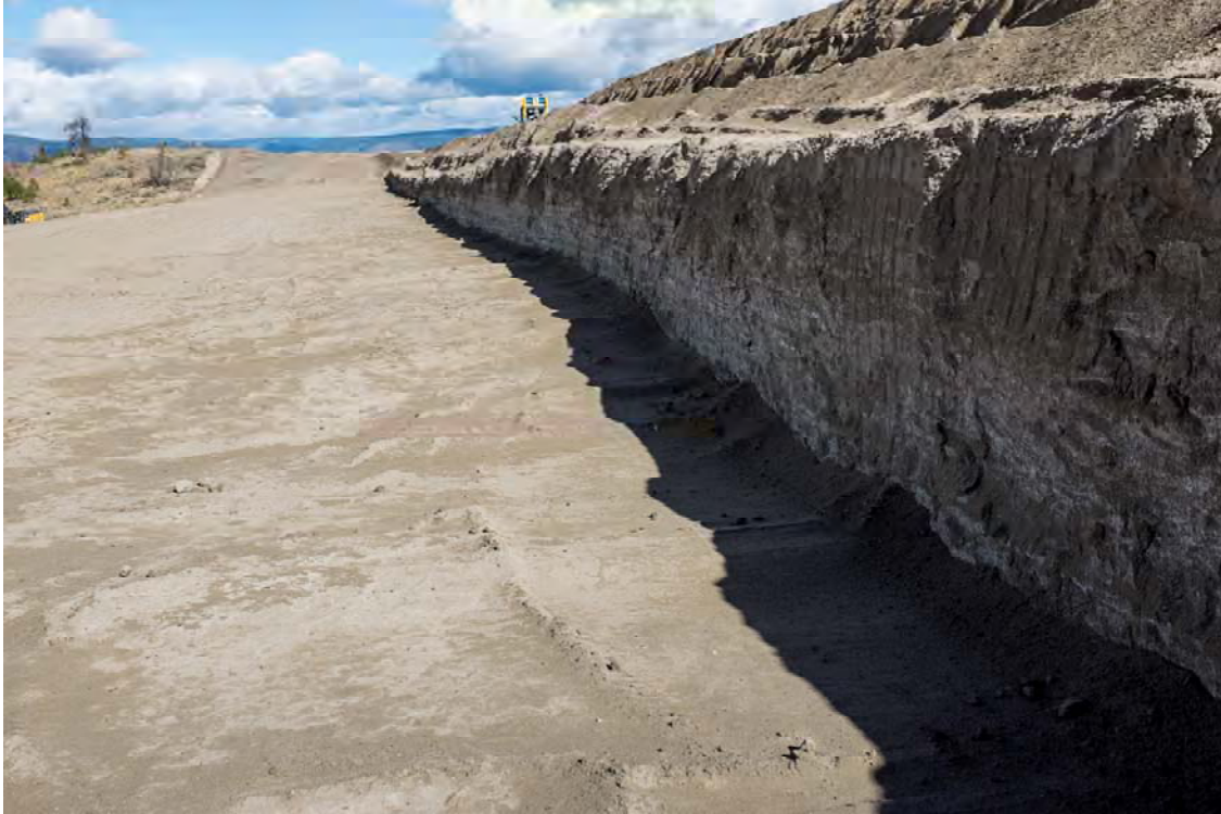
Photo DA19: View looking north of downstream slope of Dam A from close to left abutment. Bench and stepped face due to mining of hydraulically placed sand.
