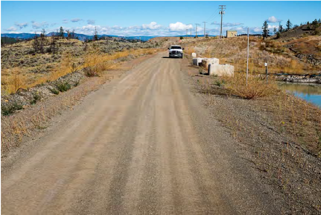
Photo S111: View of crest of Seepage Pond 1 Dam from left abutment.
