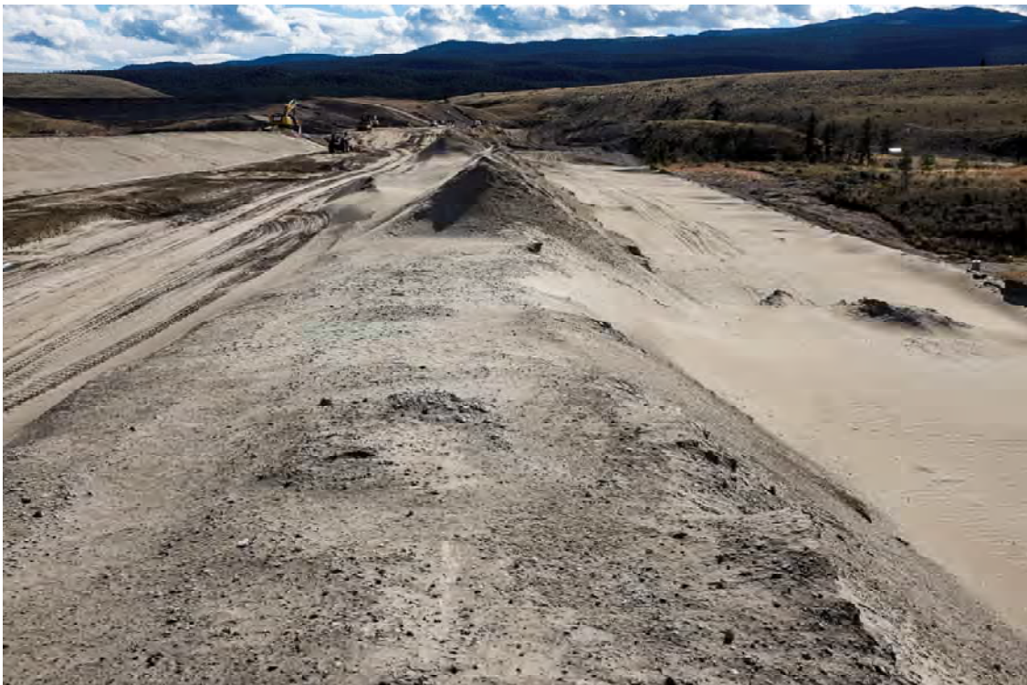
Photo DB10: View looking south at crest and downstream face of Dam B from right abutment. Note liner exposed on left side of photo and prepared bedding surface in anticipation of liner raise. West Dam visible at top left of photo.
