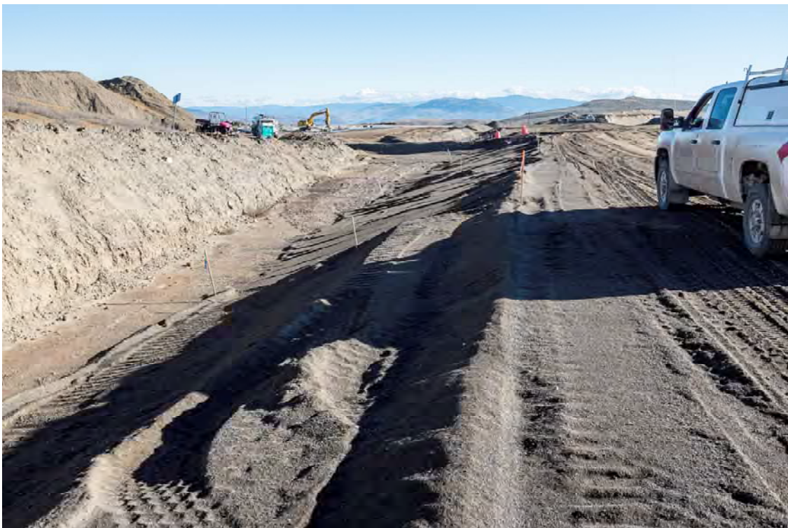
Photo DC32: View looking northeast at downstream toe from left abutment of Dam C.
