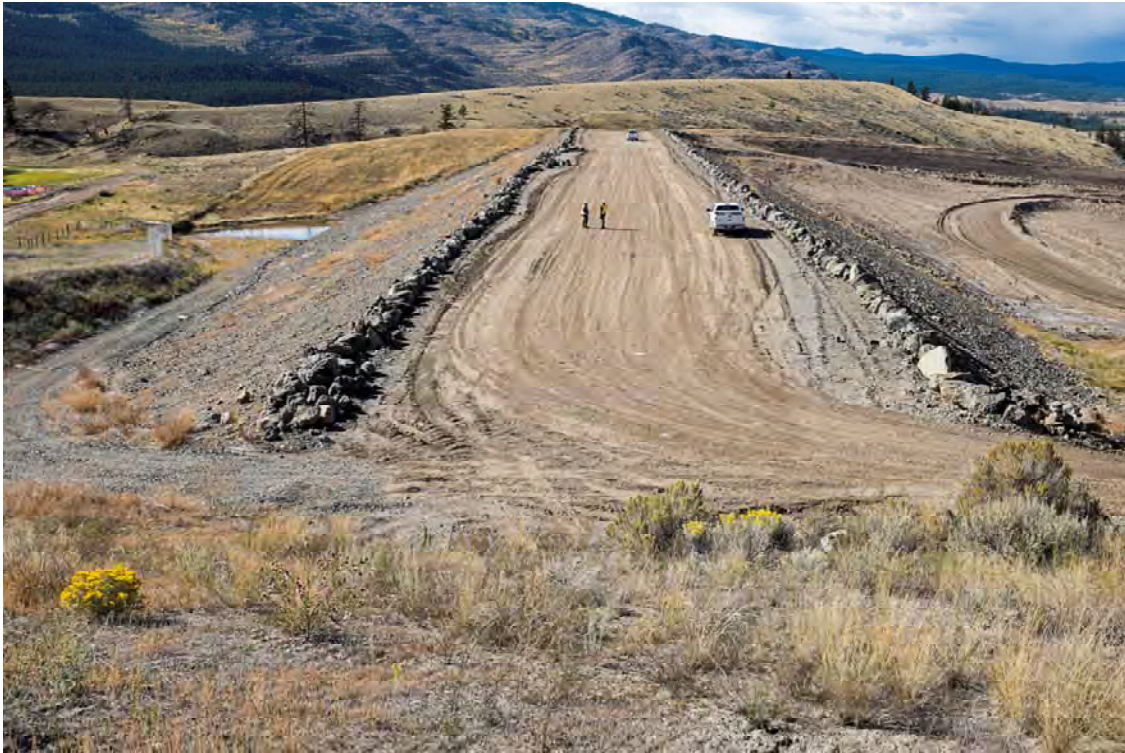
Photo WD01: View looking west at West Dam from above left abutment.
