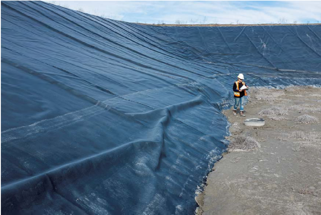
Photo PD07: View of the first dogleg in the Pothook Dam from the upstream toe.
