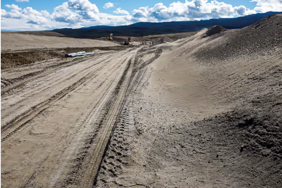
Photo DB11: View looking south at crest of Dam B from right abutment. Note liner exposed on left side of photo and prepared bedding surface in anticipation of liner raise.
