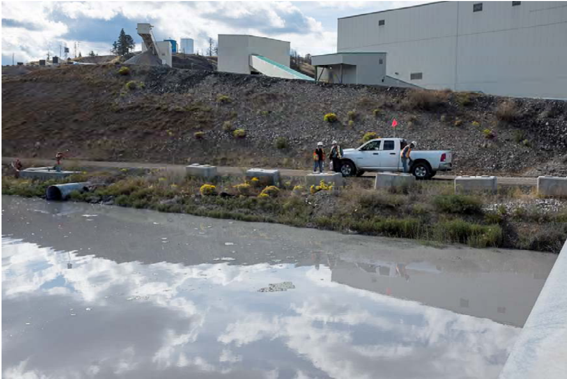
Photo TL09: View of Spill Pond adjacent to mill. Note water level relative to inlet culverts and algae rafts.
