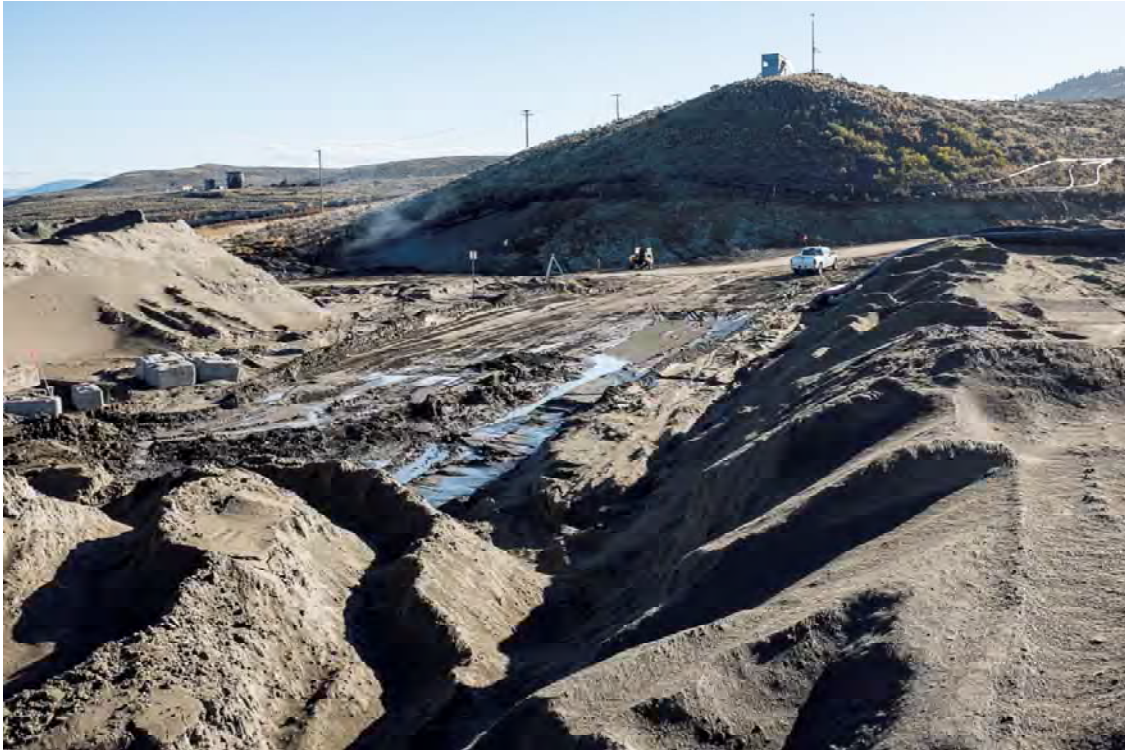
Photo DC17: View of right abutment of Dam C from downstream edge of upstream sand cell looking east. Note ponding on crest and Lock-Block protection around instrumentation installed in Dam C starter dam.
