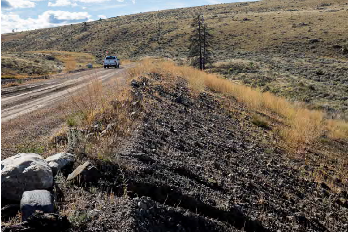
Photo S103: View of Seepage Pond 1 Dam crest and downstream face from right abutment. Note rilling and minor erosion in foreground. Note vegetation on downstream face.
