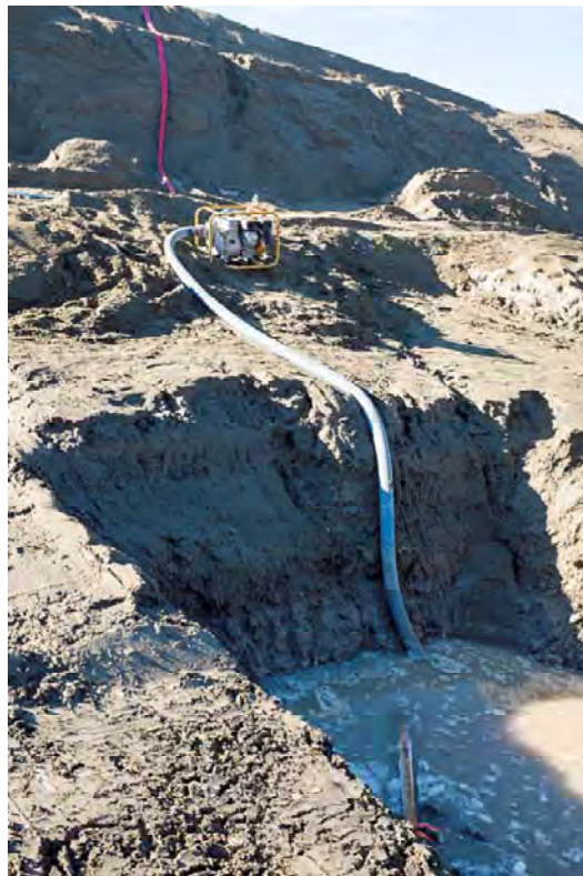
Photo DC20: View looking southwest at sump and pump managing ponded water on Dam C crest at approximately sta. 0+750 m. Pump is cycled on and off as needed.
