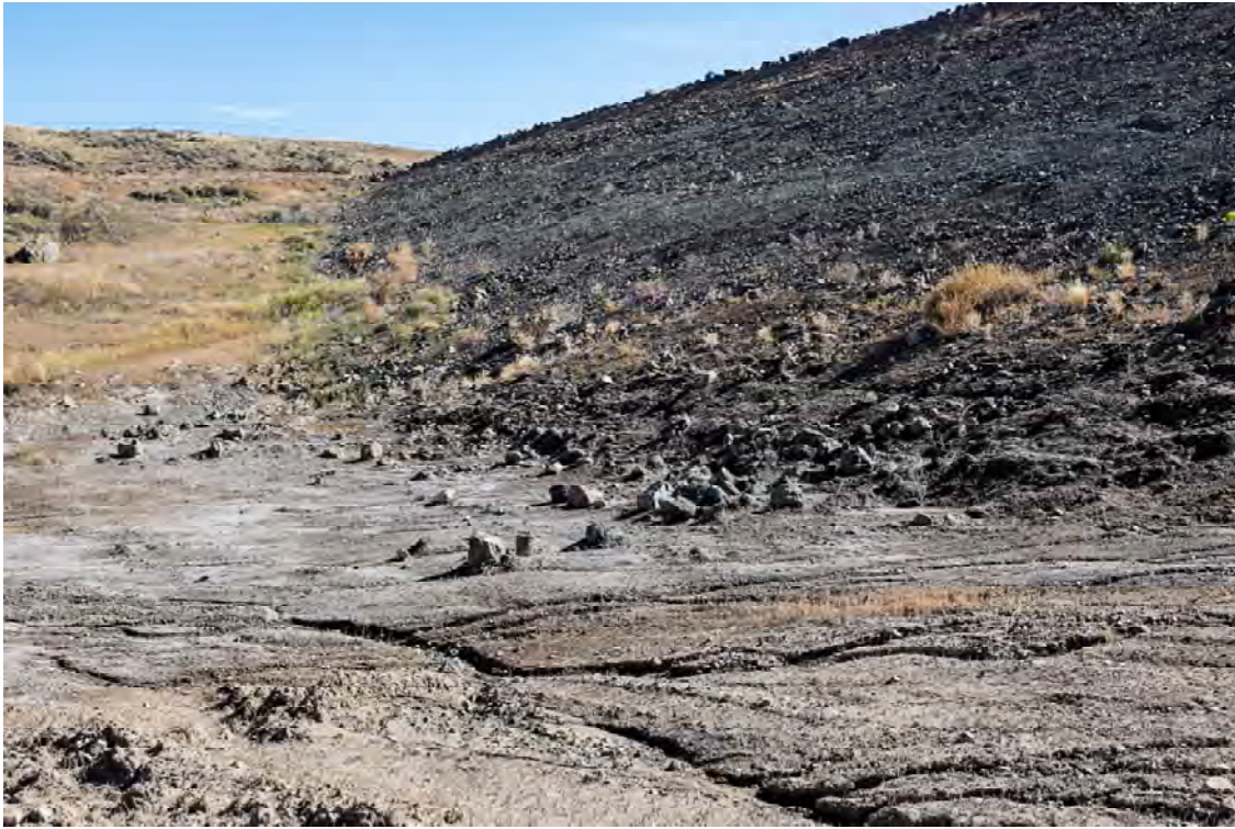
Photo WD07: View of the upstream face and left abutment of the West Dam from the upstream toe.
