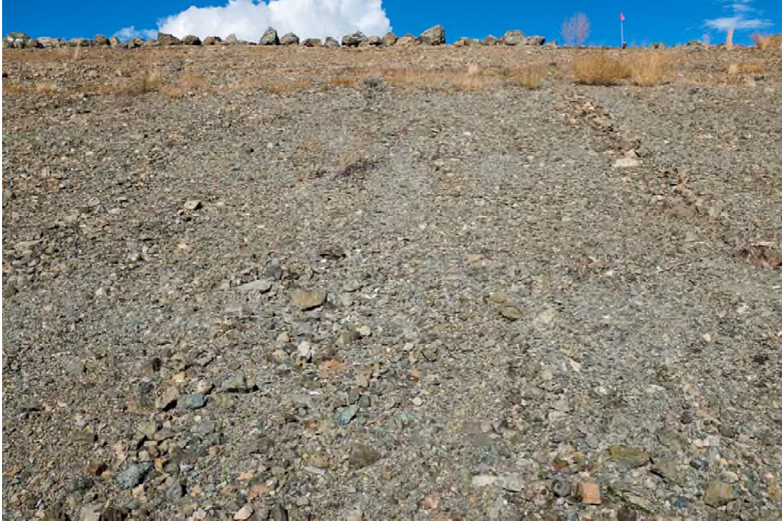
Photo WD13: View of the downstream face of the West Dam downstream toe. Note uniform slope and minimal vegetation.
