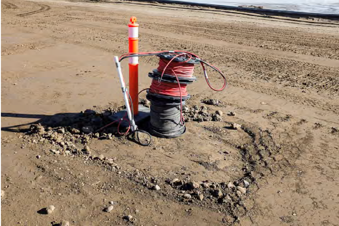
Photo DA23: Veiv of instrumentation leads on crest of Dam A looking northeast at approximately 1+700 m.
