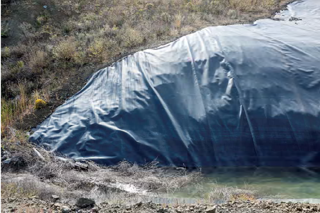
Photo PD15: View of the left abutment of the Pothook Dam from the left abutment upstream toe looking south.
