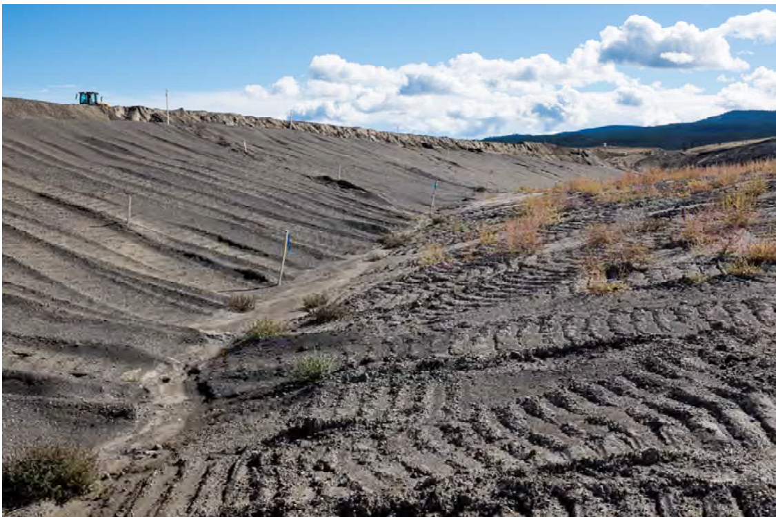
Photo DB06: View looking south at the downstream face and left abutment of Dam B from the downstream toe at approximately sta. 1+450 m.
