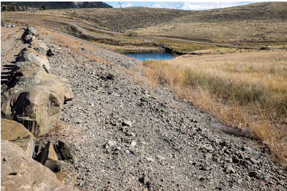
Photo WD16: View of the downstream face and toe of the West Dam from the crest at the right abutment. Note ponding at the downstream toe.
