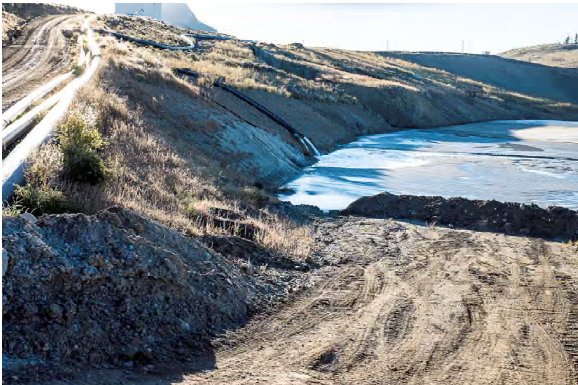
Photo DC04: View of water discharge from Pothook Pit upstream of Dam C. Looking south from right abutment of Dam C.
