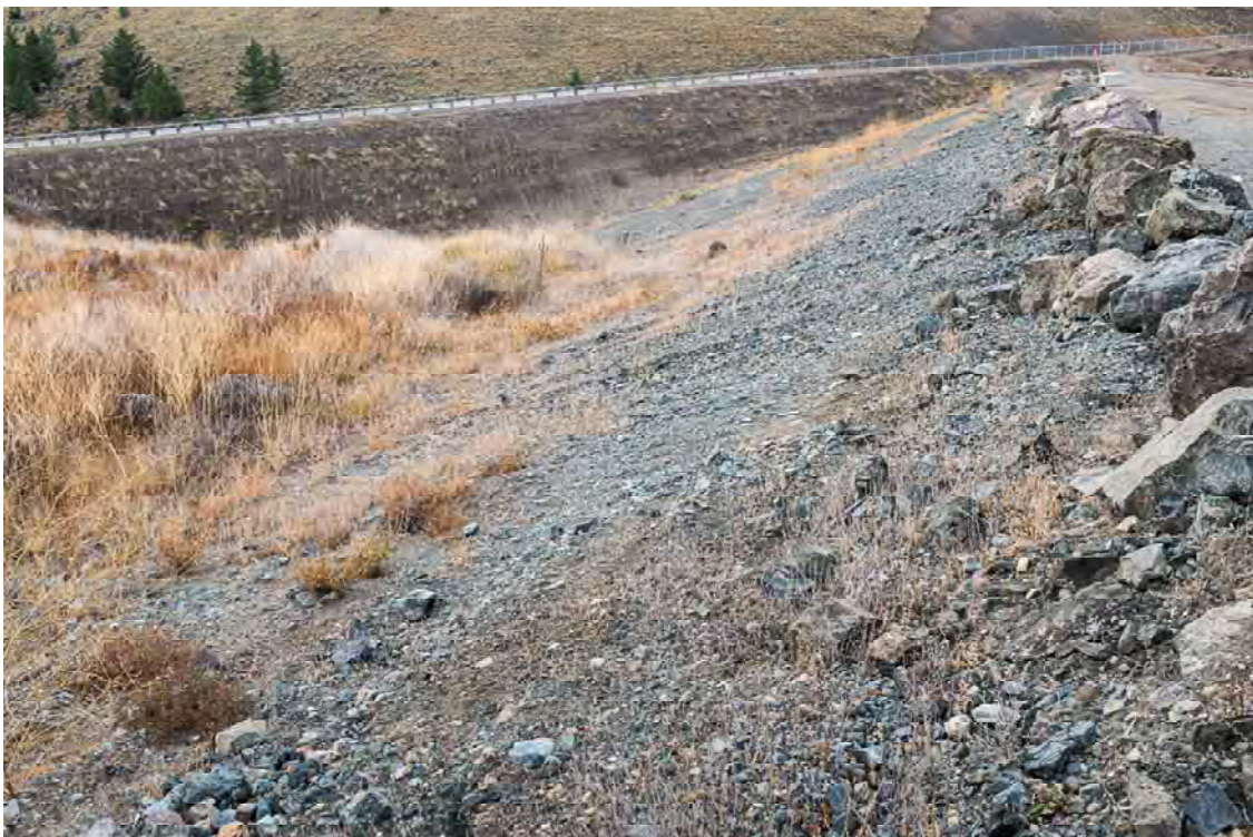
Photo SD20: View of the downstream face and toe from the left abutment crest of the South Dam.
