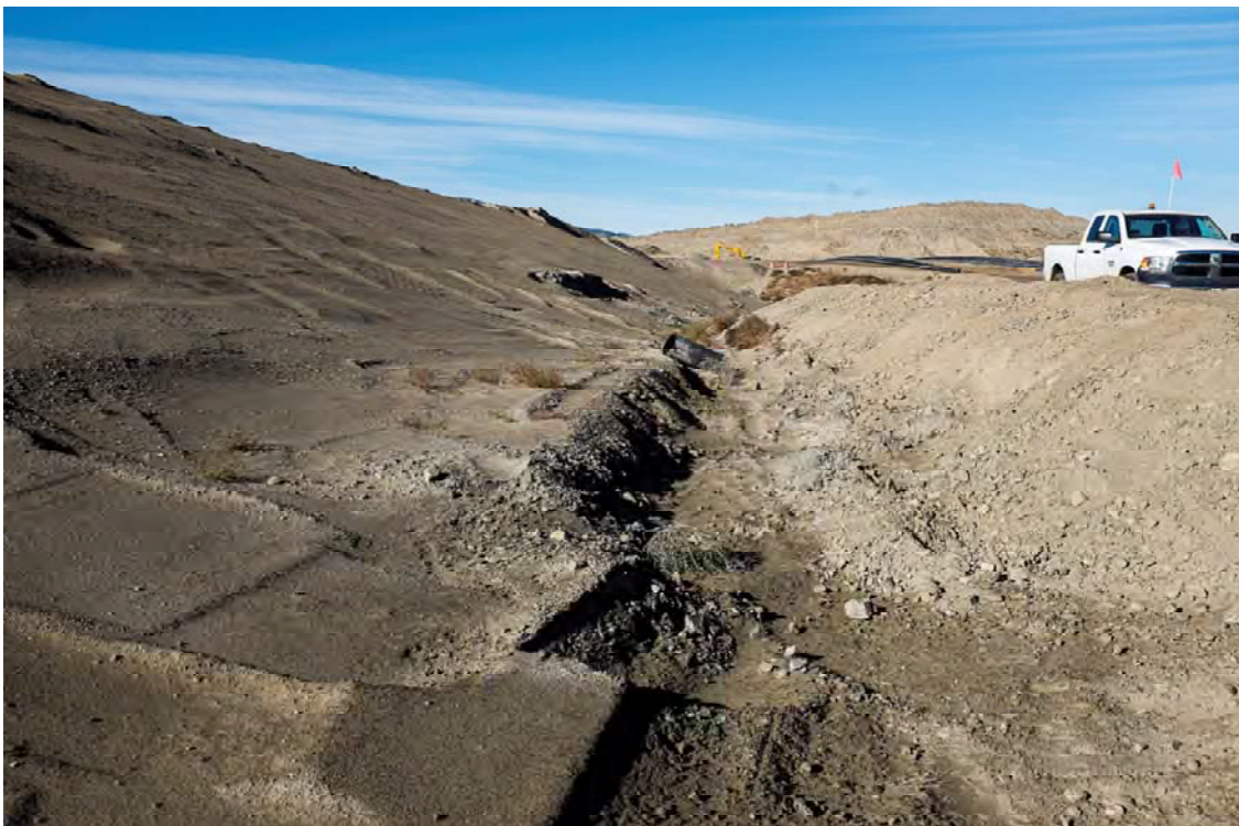
Photo DC28: View looking west from downstream toe of Dam C at approximately sta. 0+850 m. Note till stockpile in background at excavator.
