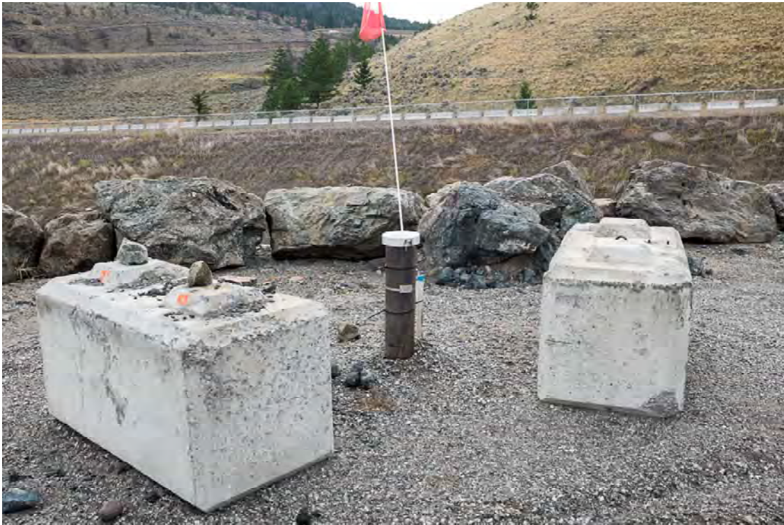
Photo SD23: View of Lock-Block protection around vibrating wire monument on downstream crest looking east at mid-point of South Dam.
