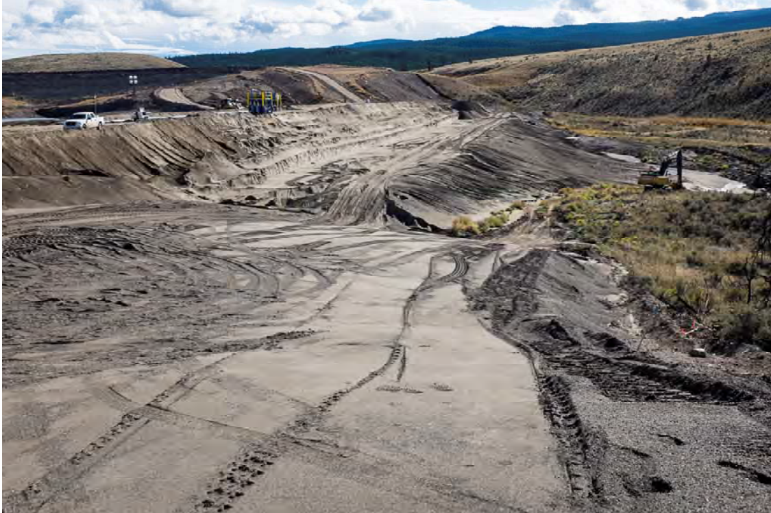
Photo DA13: View looking south from downstream toe of Dam A at boundary with Dam B. West Dam visible at top left of photo. Note change in downstream slope at toe near excavator, and stepped slope closer to dam crest.
