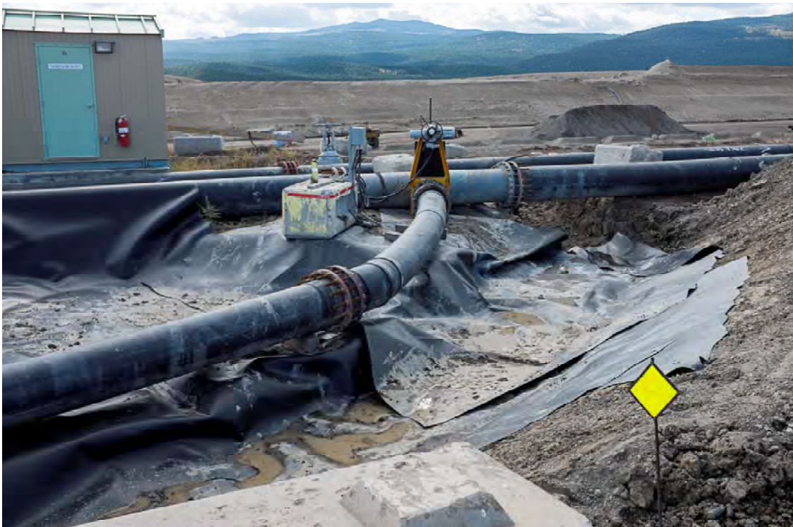
Photo TL02: View looking south at valve and liner placed and yet to be seamed to contain and direct potential spills to Seepage Pond 3. Location of previous valve leak.
