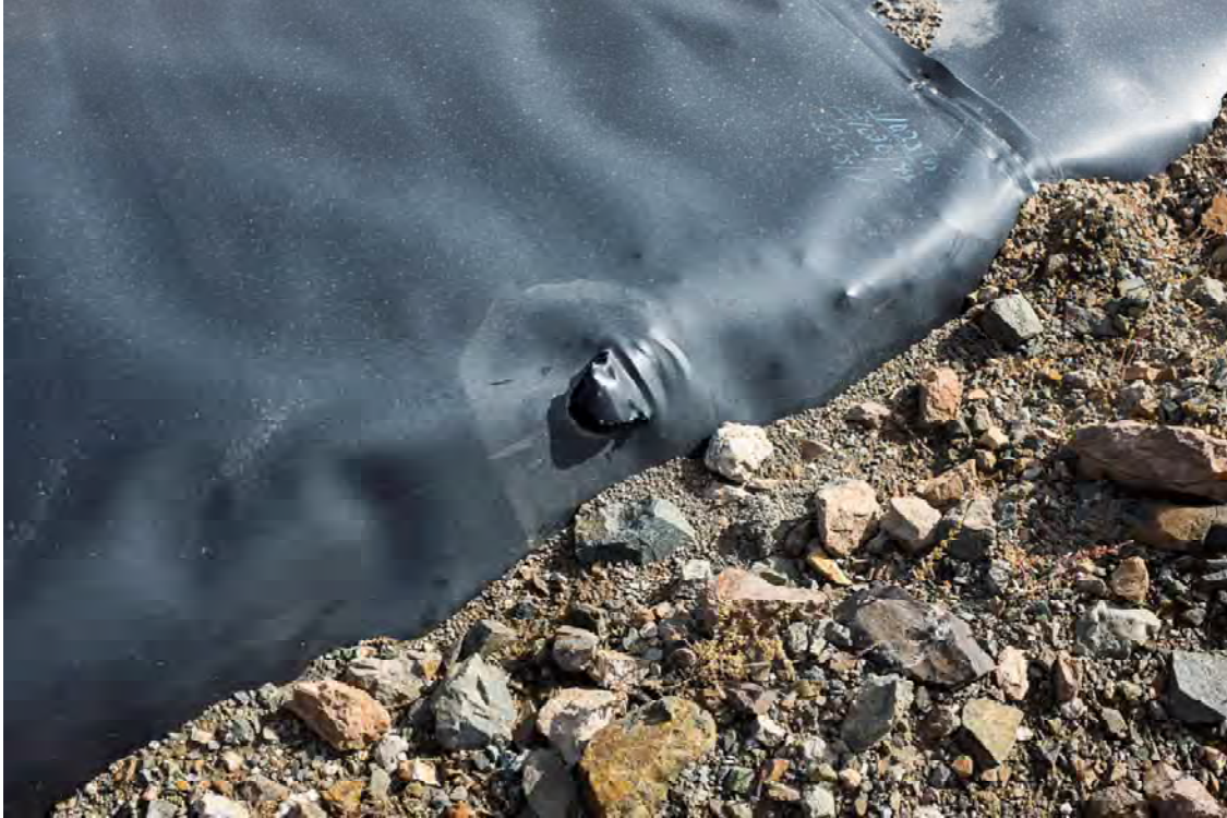
Photo PD23: Note tear in liner at anchor trench just north of the tailings pipeline ramp. Defect identified for repair in 2013 annual inspection report.
