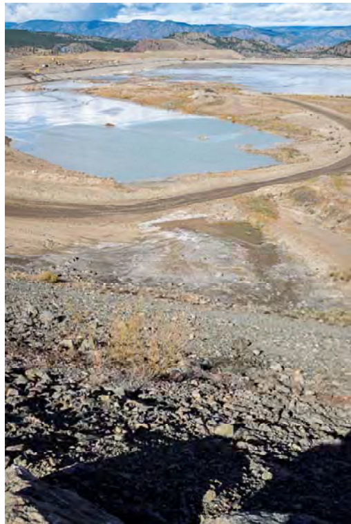
Photo WD04: View of the upstream toe of the West Dam from the crest at the mid-point of the dam looking north. Dam B and C visible in the background. Note ponding at the upstream toe of the West Dam.
