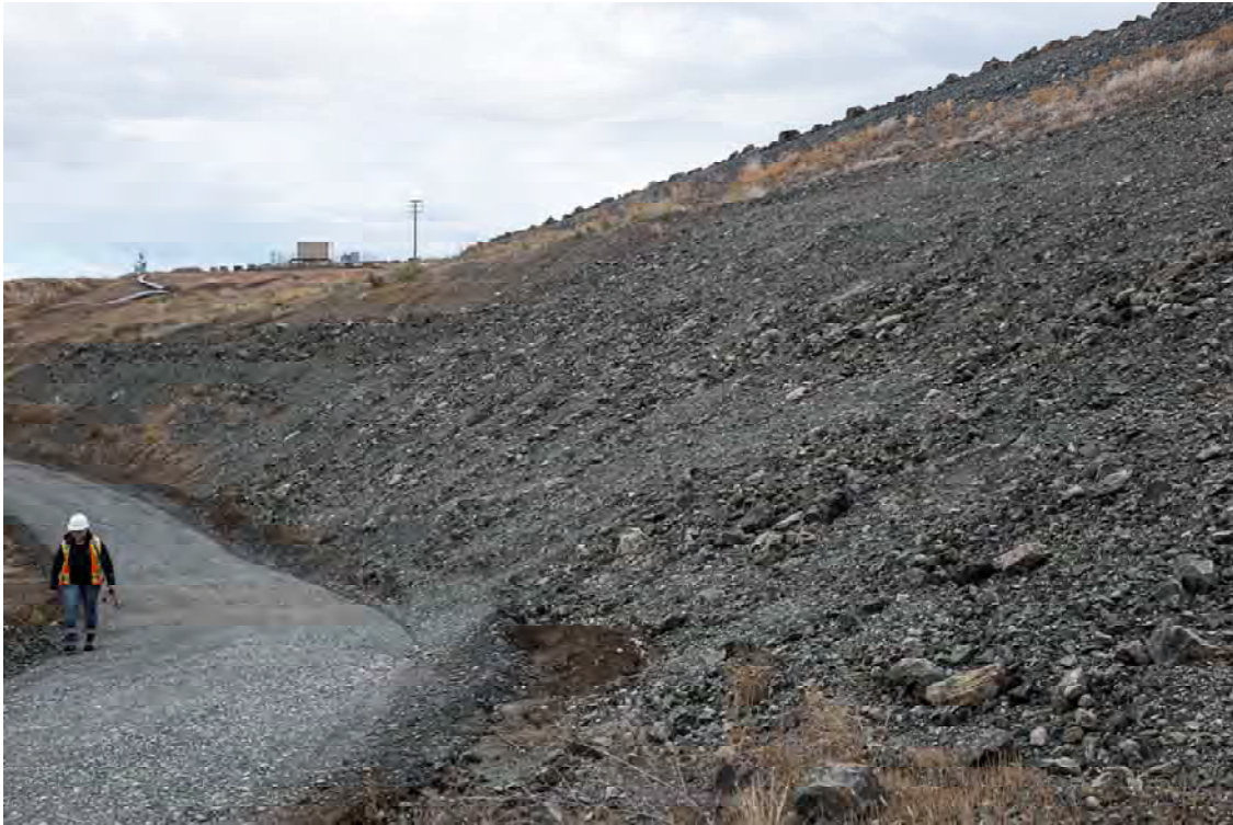
Photo SD05: View of left abutment and upstream face of South Dam from upstream toe.
