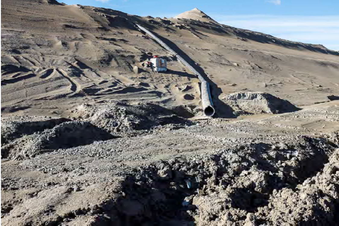
Photo DC25: View looking southwest at instrument leads and decant pipe on downstream face of Dam C at approximately sta. 0+600 m.
