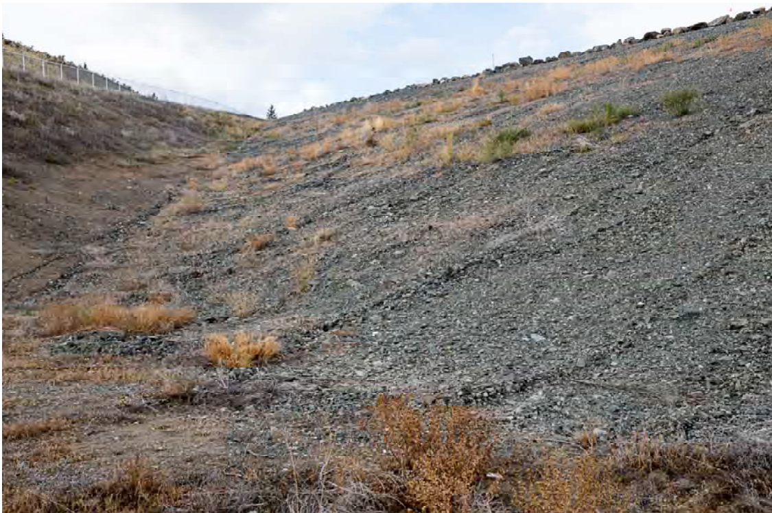
Photo SD16: View of the right abutment and downstream face of the dam from the downstream toe of the South Dam.
