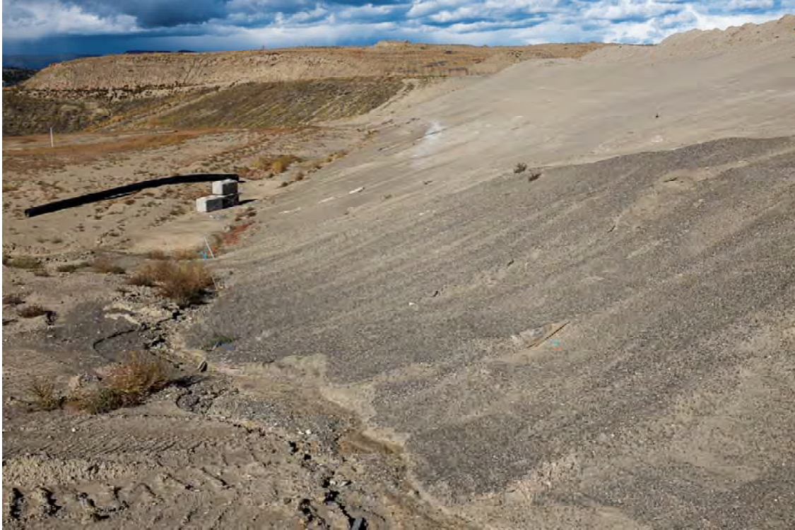
Photo DB05: View looking north at the downstream face and right abutment of Dam B from the downstream toe at approximately sta. 1+450 m.
