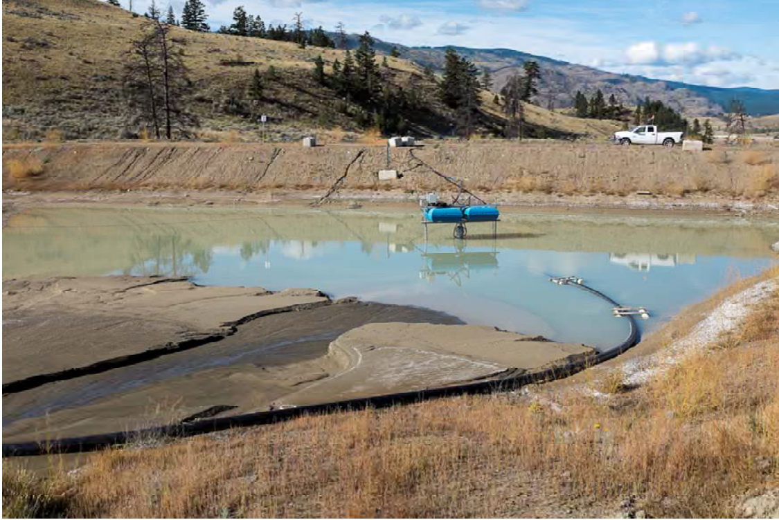
Photo S113: View of Seepage Pond 1 and Dam from upstream end of impoundment. Note minor erosion of dam face and sediment collecting in pond. High water mark visible on face of dam.
