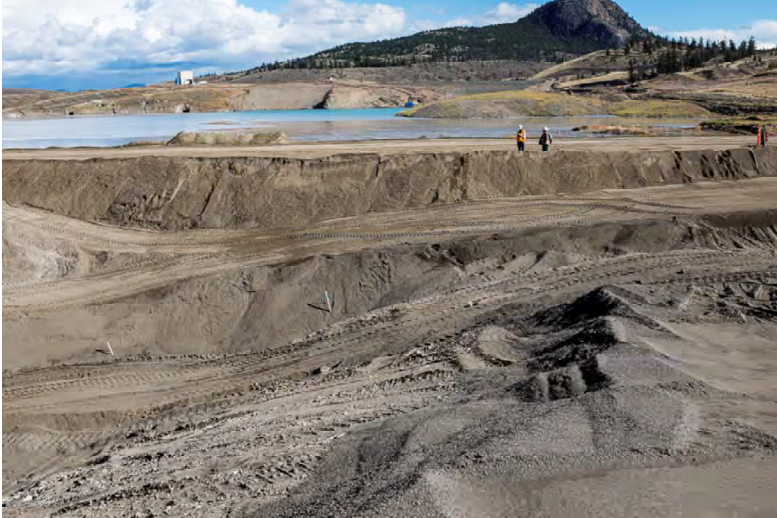
Photo DA11: View looking east from downstream toe of Dam A at boundary with Dam B. South Dam and reclaim barge visible in upper mid-right of photo. Primary cyclone visible in upper left of photo.
