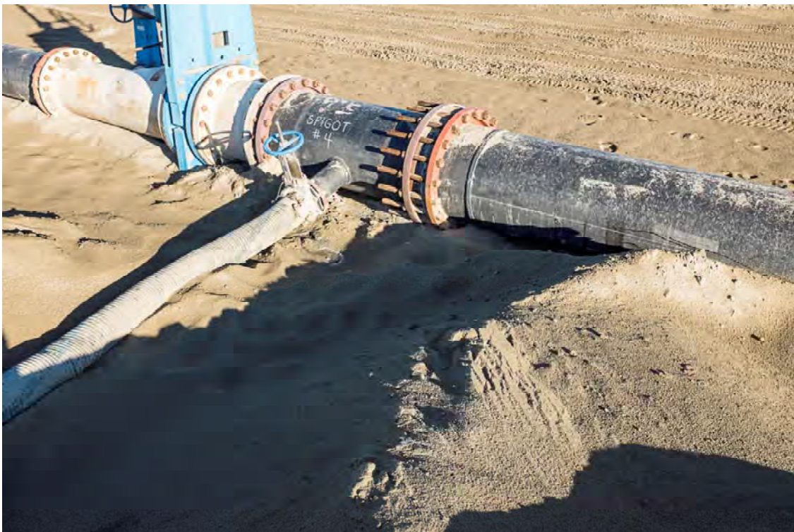
Photo DC08: View of spigot 4 on Dam C looking northwest. Note leaking connection at valve.
