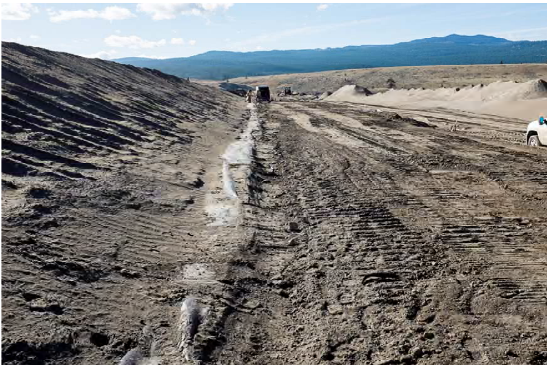
Photo DB20: View looking south at exposed liner on Dam B crest near right abutment. Note damage to liner caused by excavation to expose liner in the process of being repaired in anticipation of liner raise.
