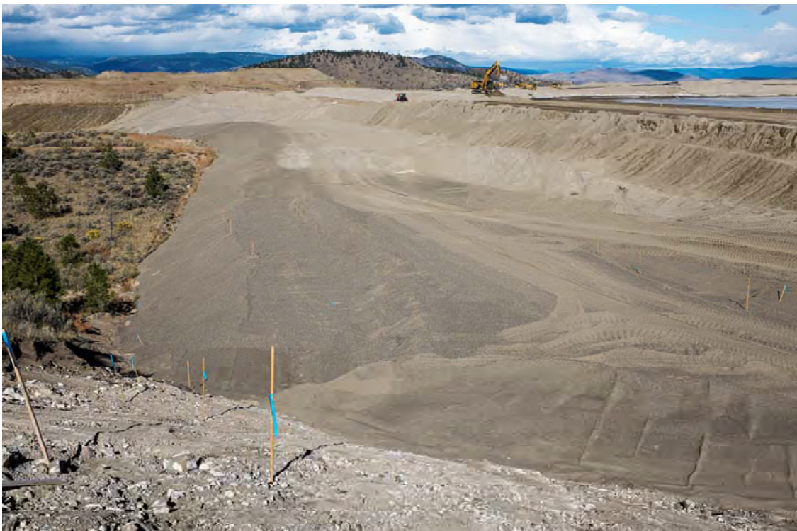
Photo DB02: View looking north at Dam B downstream face and toe from the left abutment downstream toe at boundary with Dam A. Note stepped downstream face, and extent of filter at downstream toe.
