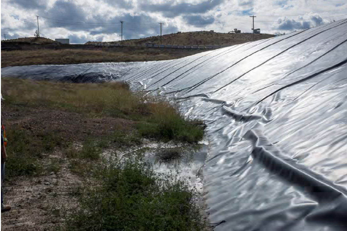
Photo PD11: View of upstream face and toe of the Pothook Dam between the tailings pipeline ramp and the second dogleg in the dam looking south. Primary cyclone visible in the background left of photo.
