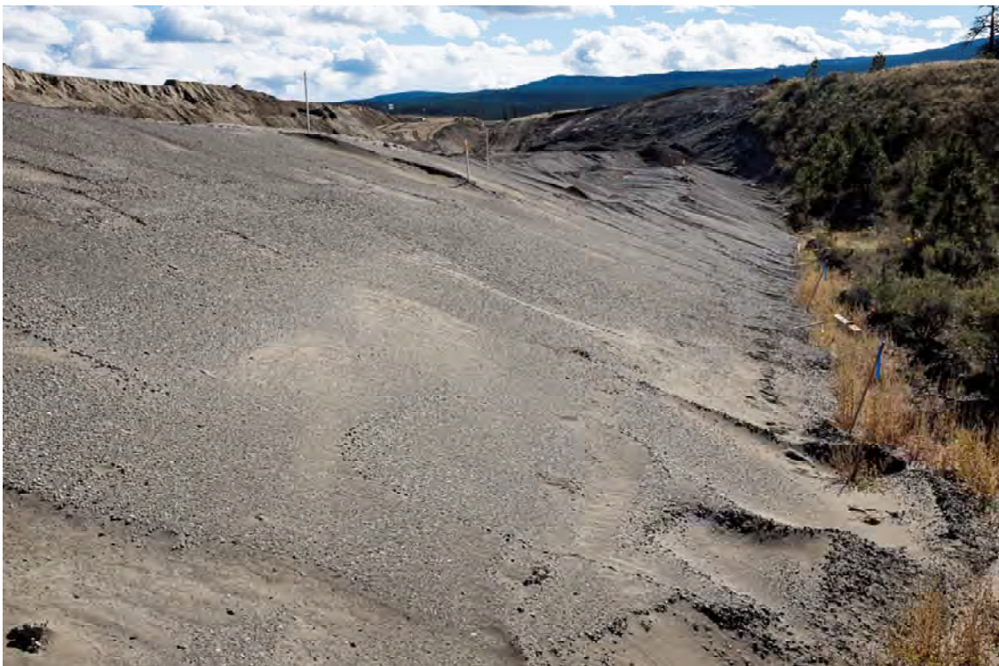
Photo DB04: View looking south at the downstream face and left abutment of Dam B from the downstream toe at approximately sta. 1+500 m.
