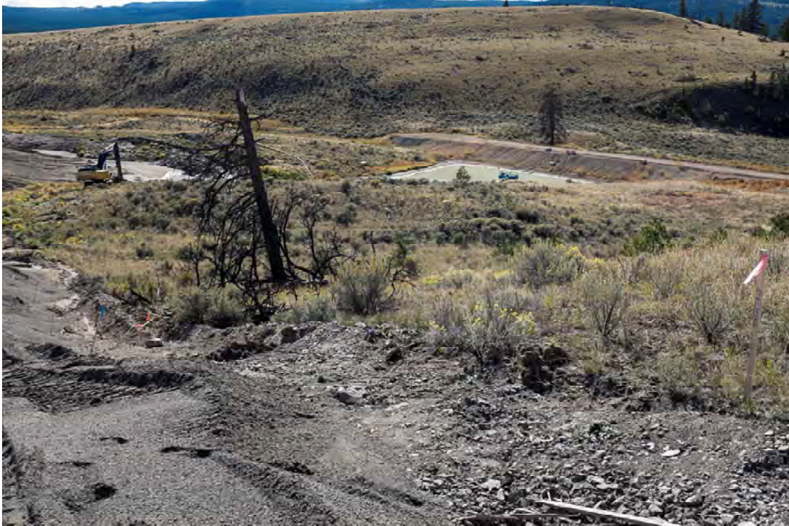
Photo S101: View looking southwest at Seepage Pond 1 from boundary between Dam A and Dam B at downstream toe. Downstream toe of Dam A visible at top left of photo.
