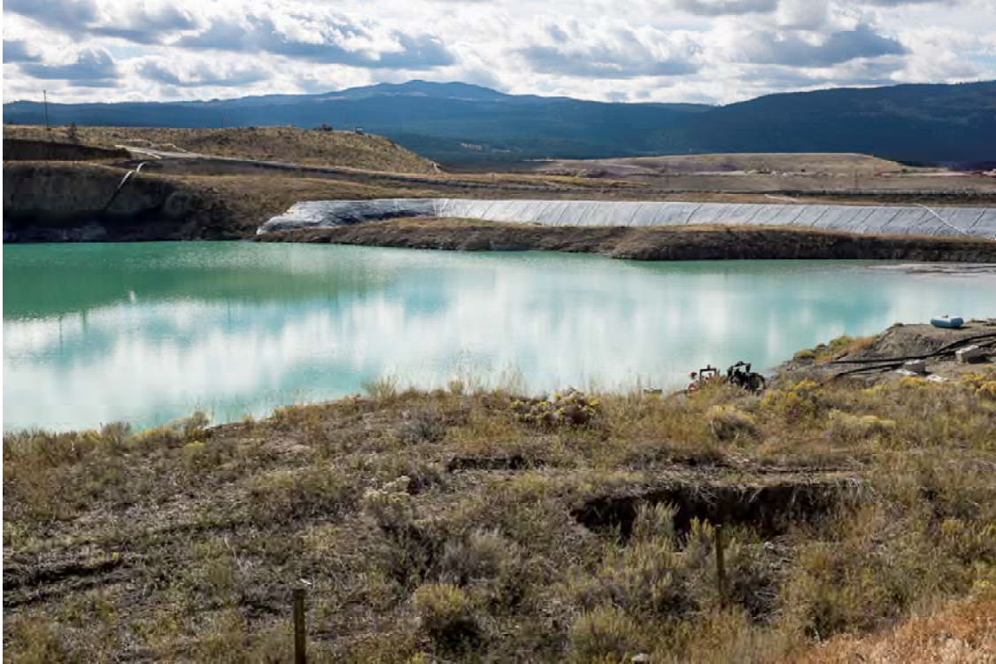
Photo PD41: View of south rim of Pothook Pit and left abutment of Pothook Dam from west of Emergency Spillway looking south.
