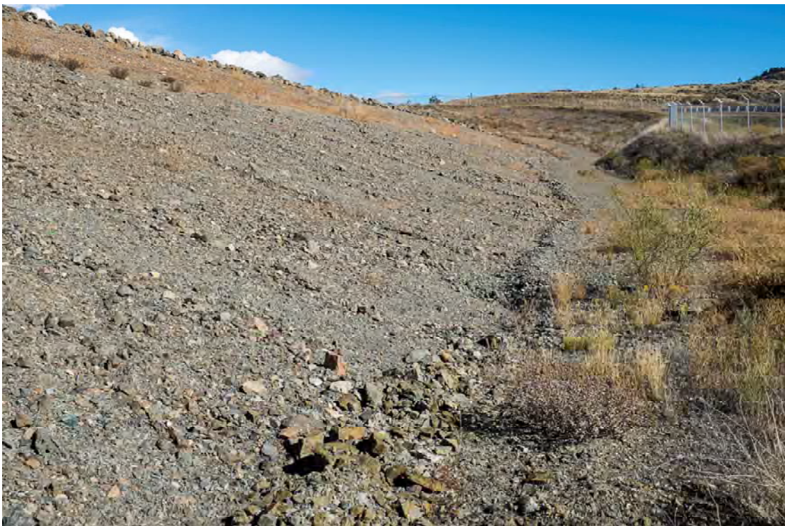
Photo WD12: View of the downstream face and left abutment of the West Dam from the downstream toe.
