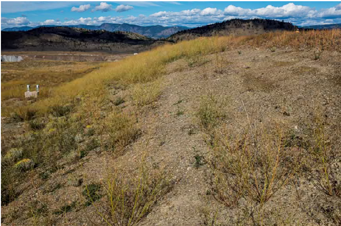
Photo PD26: View of the downstream face of the Pothook Dam looking north from south of the first dogleg at mid-slope on the downstream face. Note air quality station at toe of dam.
