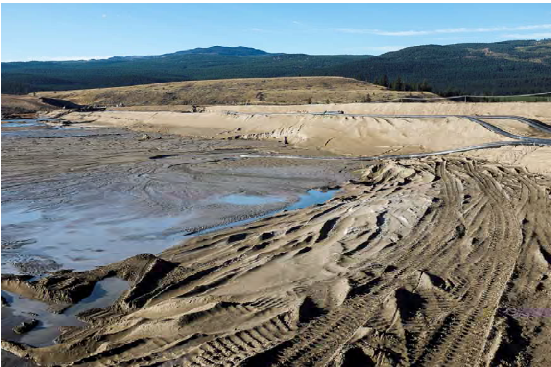
Photo DC12: View of left abutment of Dam C and the right abutment of Dam B from the upstream sand cell of Dam C looking southwest.
