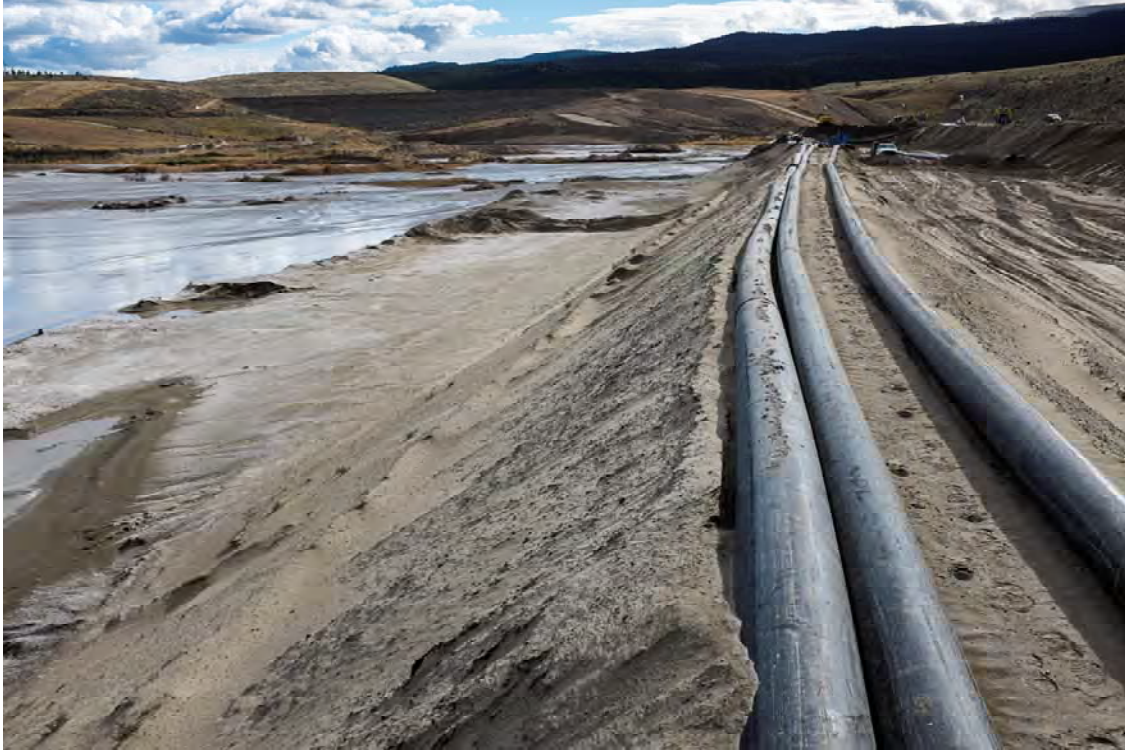
Photo DB15: View looking south at upstream limit of upstream sand cell from left abutment of Dam B toward Dam A. Sand cells being prepared for hydraulic sand placement.
