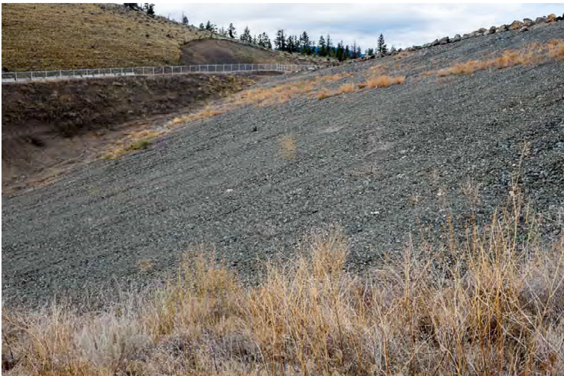
Photo SD18: View of the downstream face and right abutment from the left abutment at the mid-height of the slope of the South Dam.
