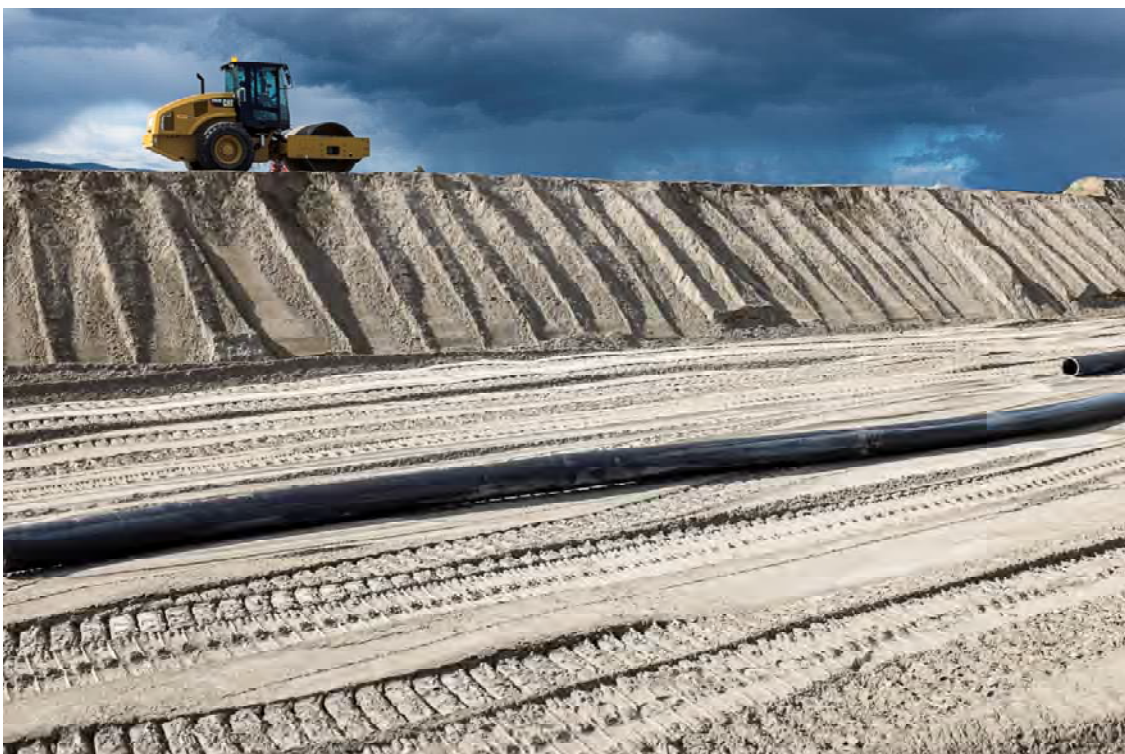
Photo DB14: View looking west at downstream limit of prepared upstream sand cell on Dam B.
