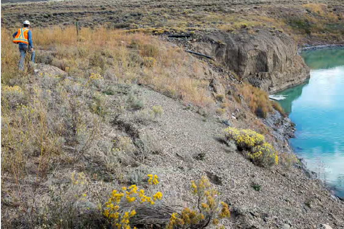
Photo PD35: View of scarps and tension cracks in till along the north rim of Pothook Pit adjacent to the Emergency Spillway looking east
