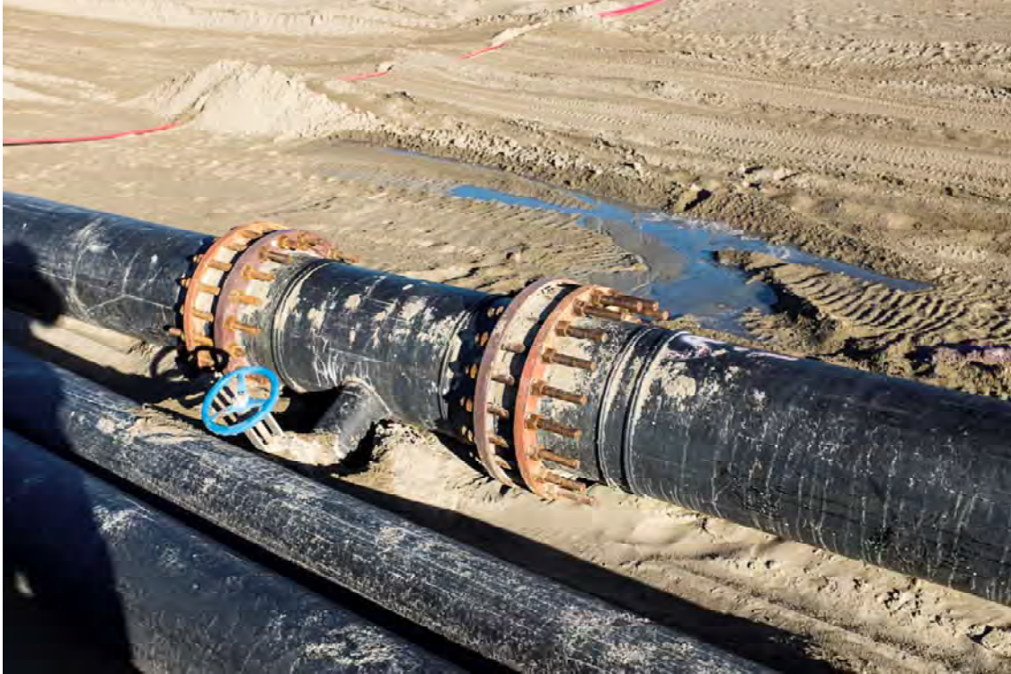
Photo DC09: View of spigot 6 on Dam C looking northwest. Note leaking valve and ponded water downstream of header pipe.
