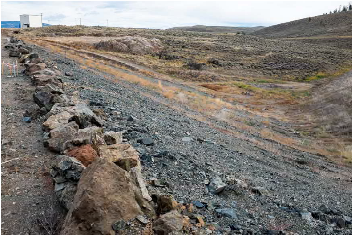
Photo SD13: View of the downstream face and toe from the right abutment crest of the South Dam.
