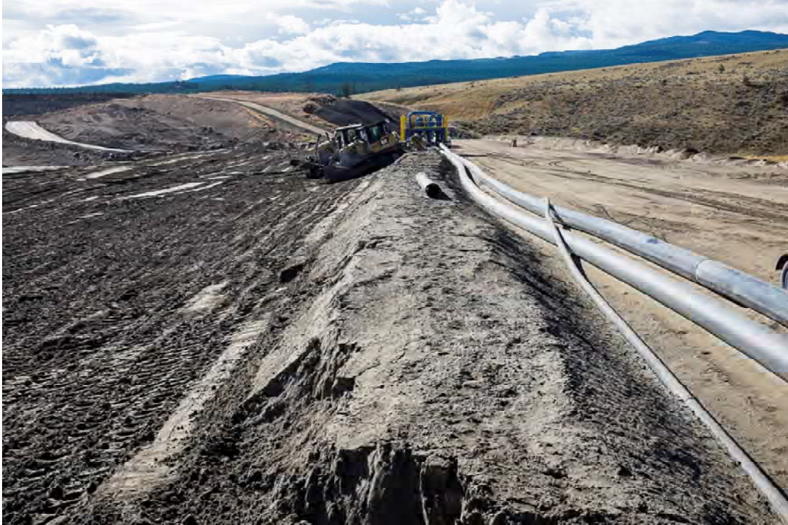
Photo DA07: View looking south toward left abutment of Dam A from approximately 1+700 m at boundary between upstream sand cell and core.
