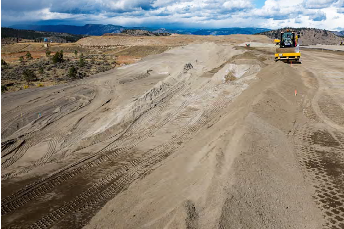
Photo DB01: View looking north at Dam B downstream face and toe from the left abutment crest at boundary with Dam A. Note stepped downstream face, and extent of filter at downstream toe.
