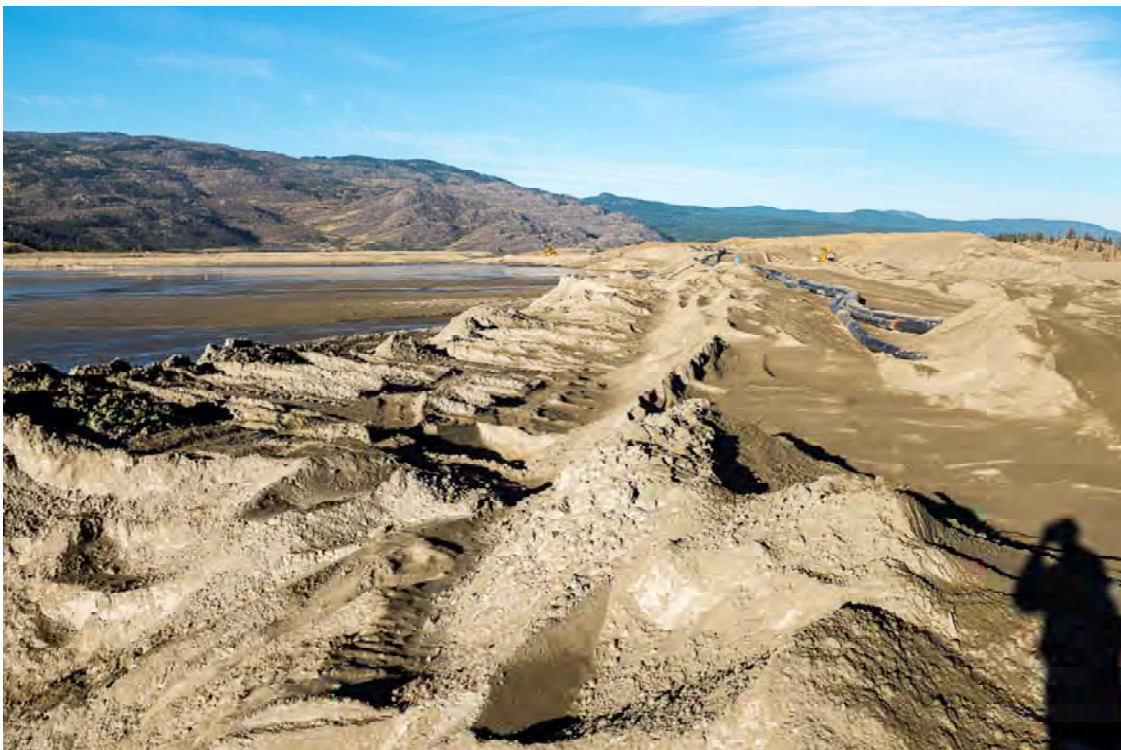
Photo DC06: View of upstream sand cells from right abutment of Dam C looking west. Note tailings that have been pushed into impoundment on left side of photo.
