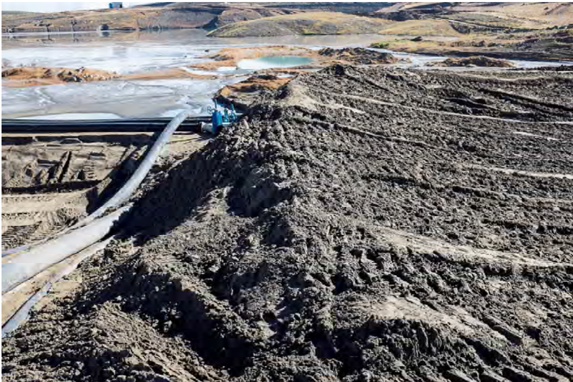
Photo DA08: View looking west at lateral boundary between upstream sand cells at approximately sta. 1+700 m. Primary cyclone visible in top left of photo.
