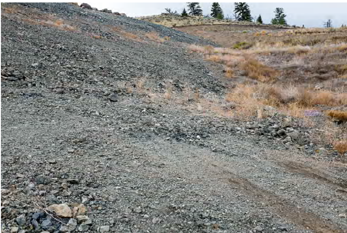
Photo SD04: View of right abutment and upstream face of South Dam from upstream toe.
