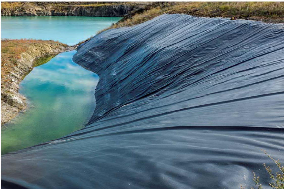
Photo PD18: view of the left abutment and upstream face of the Pothook Dam from the crest at the second dogleg looking east.
