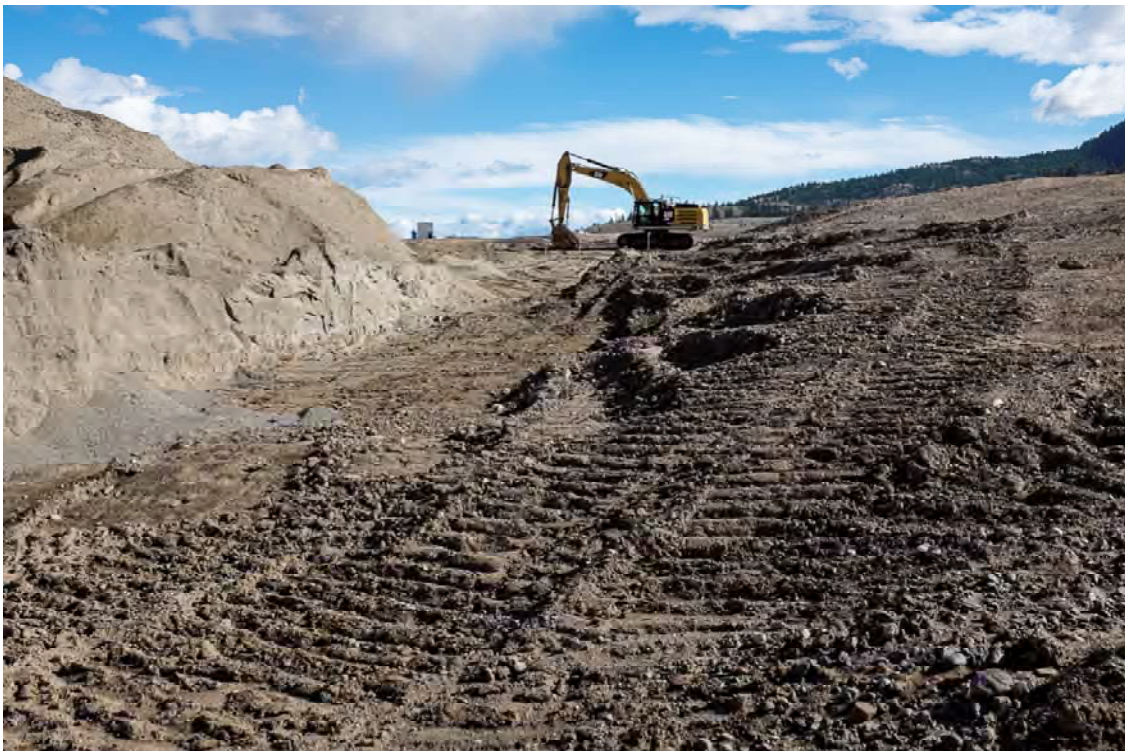
Photo DA20: View looking east at left abutment just downstream of crest of Dam A where dam bends toward West Dam. Staking denotes upper limit of till core to be placed as part of the 2014 construction season.
