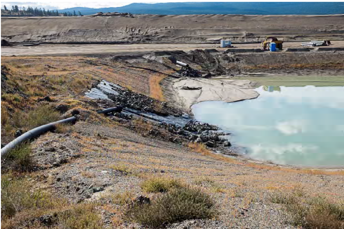
Photo S304: View of the east side of Seepage Pond 3 from the north side looking south. Note sediment accumulated at the decant pipe discharge.
