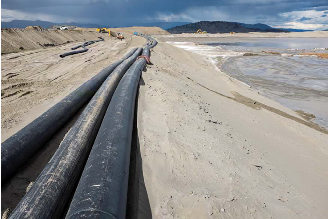
Photo DB13: View looking north at Dam B upstream limit of upstream sand cell from left abutment. Dam C visible at top right of photo.
