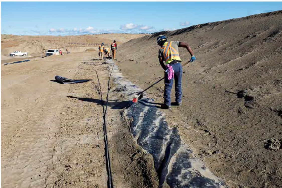
Photo DB22: View looking north at exposed liner being cleaned and repaired in anticipation of liner raise. At approximately sta. 1+375 m on Dam B crest.
