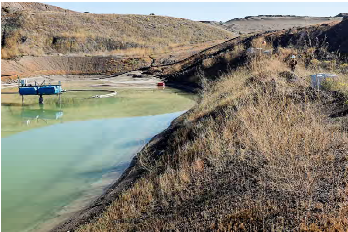
Photo S206: View looking east at inlet of Seepage Pond 2. Note sediment in impoundment. Dam B visible in the background right of the photo.
