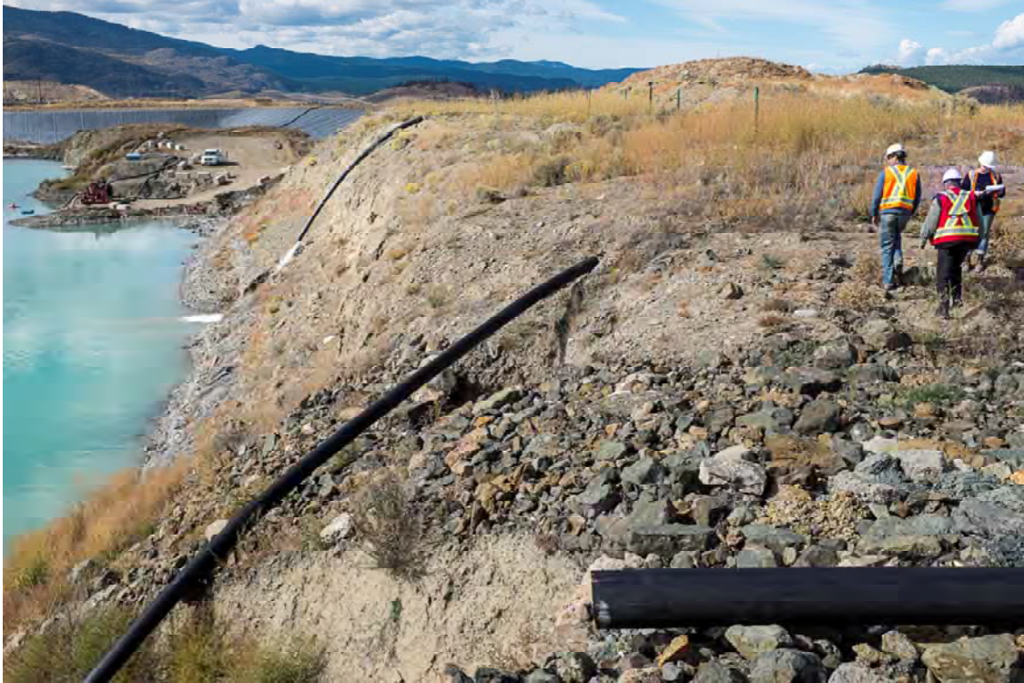
Photo PD37: View of tension cracks in the upper till unit along the north rim of Pothook Pit from the inlet to the Emergency Spillway looking west
