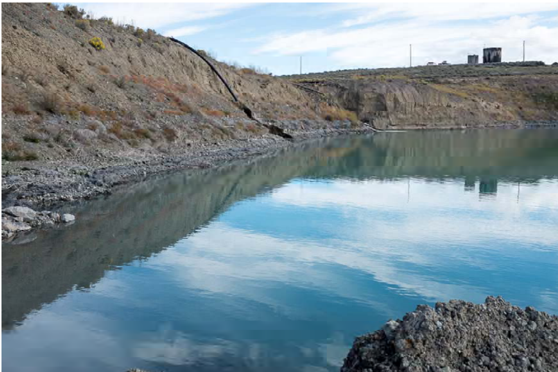
Photo PD32: View of the slope between the right abutment of the Pothook Dam and the Pothook Emergency Spillway on the north side of the Pothook Pit looking east from the pump ramp in the pit. Note erosion from pipeline discharge of water from the Afton Pit.
