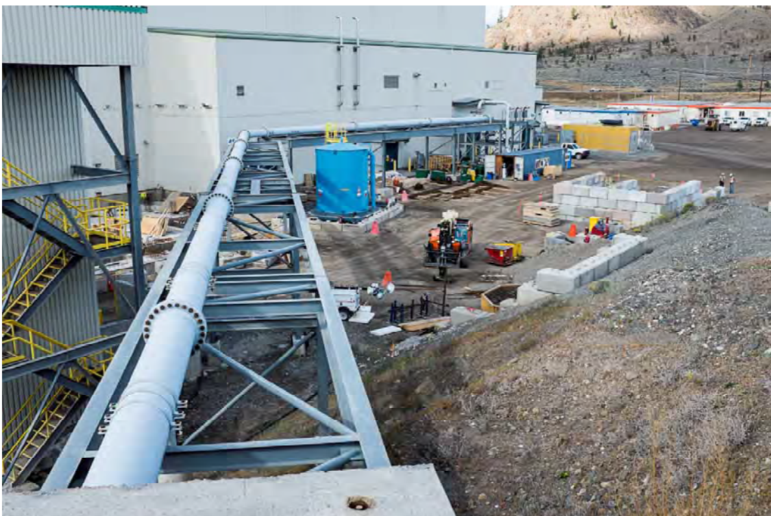
Photo TL08: View of steel tailings line where it enters the mill.
