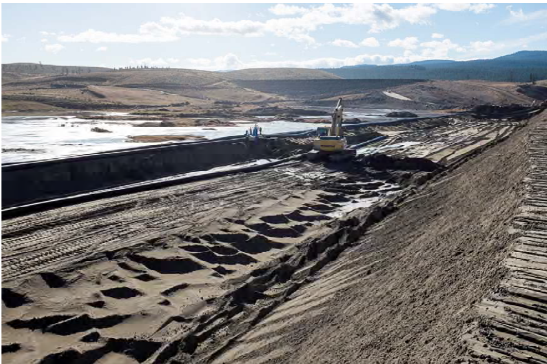
Photo DB18: View looking southeast at upstream sand cells being prepared on upstream face of Dam B at approximately sta. 1+450 m. West Dam visible in background.
