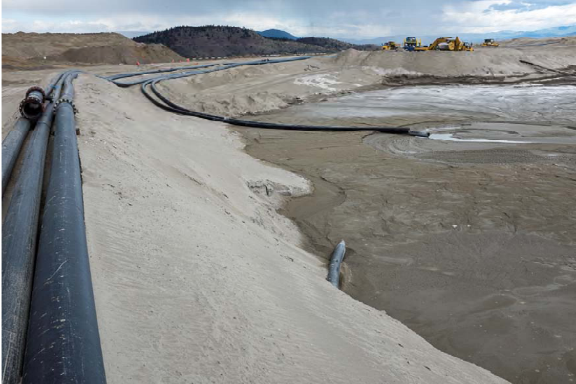
Photo DB17: View looking north at upstream limit of upstream sand cell from right abutment of Dam B toward Dam C.
