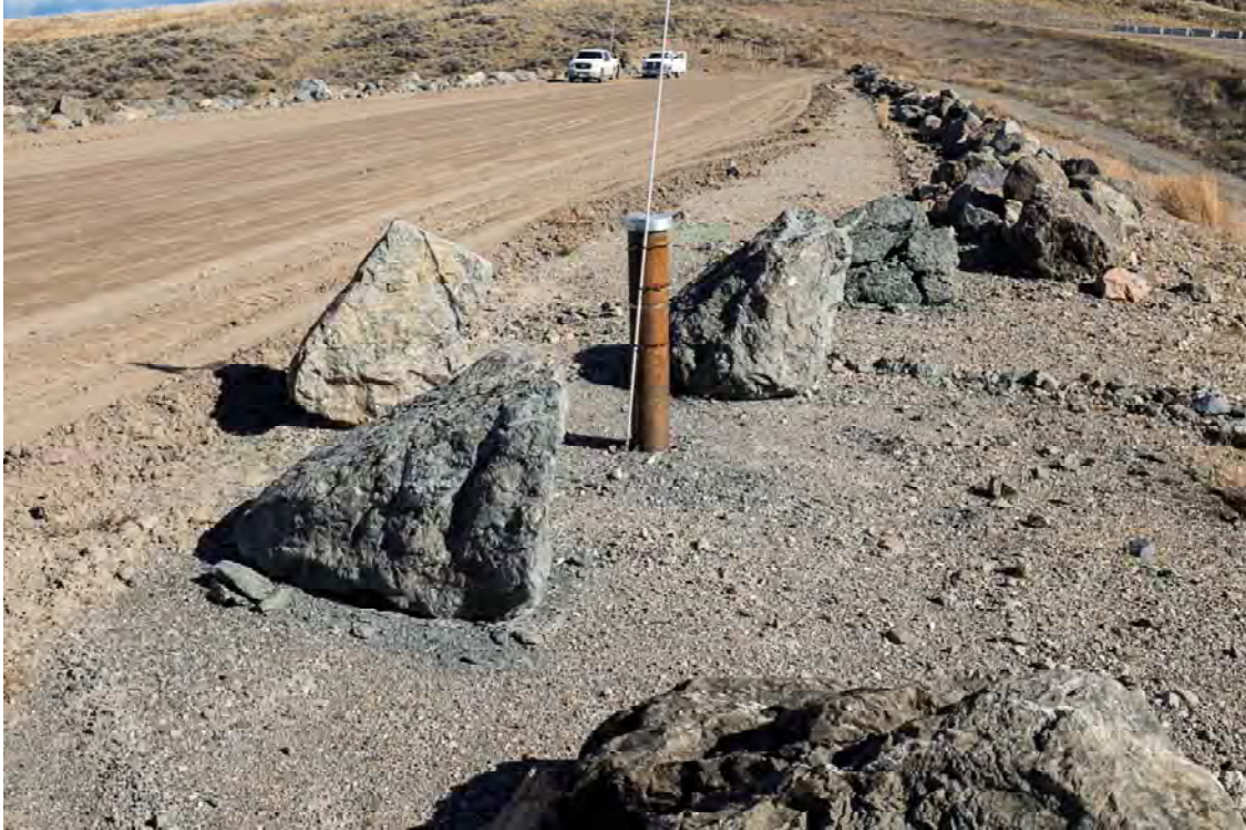
Photo WD21: View of vibrating wire monument installed on the downstream side of the crest at the mid-point of the West Dam. Note rock protection around instrument housing.
