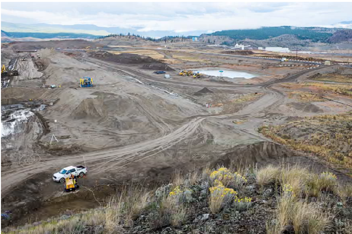
Photo DC02: View of Dam C from survey shed above right abutment looking northwest. Note Seepage Pond 3 to the upper right of the photo.
