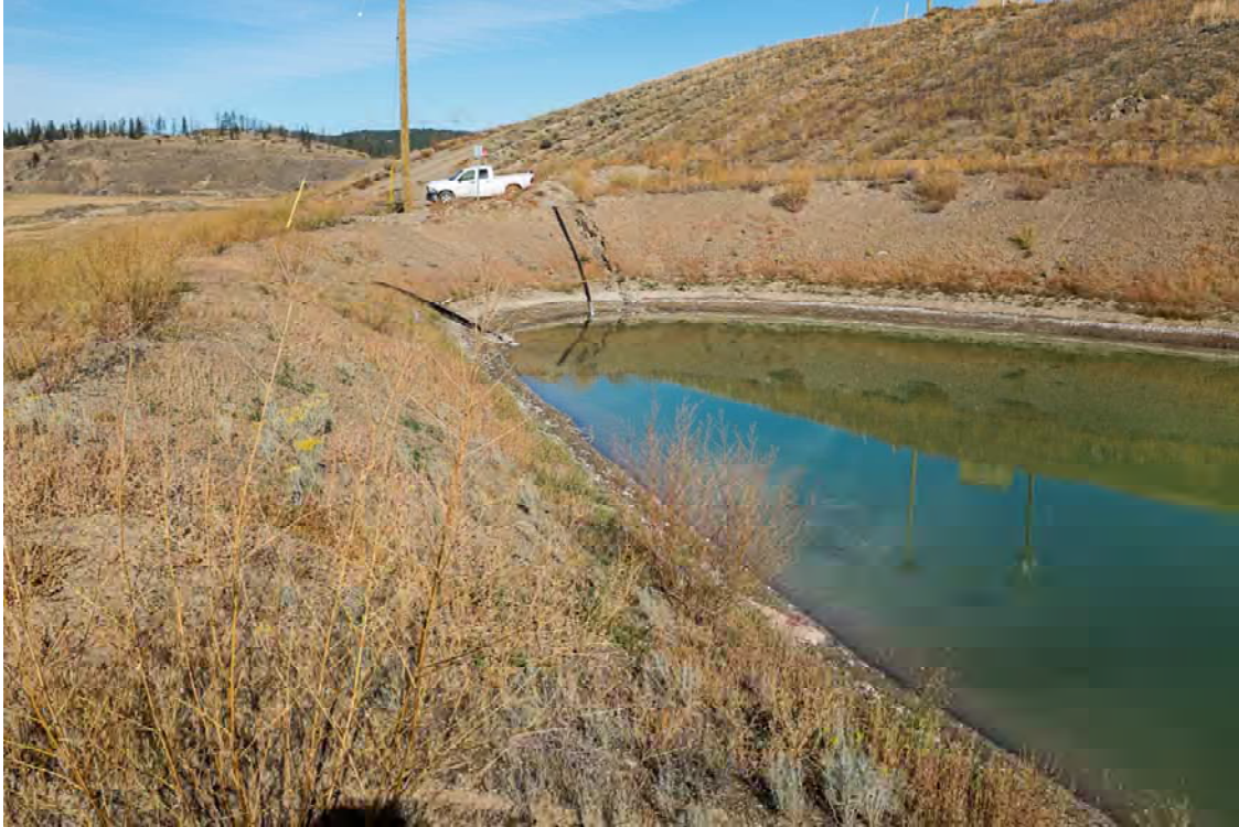
Photo S207: View looking north at northwest end of Seepage Pond 2. Note erosion of slope between truck and impoundment where inlet channel reports to impoundment. Teck TSF visible at top left of photo.
