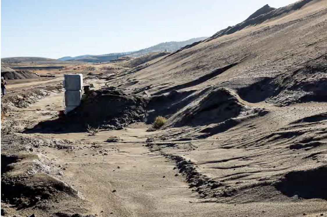
Photo DC27: View looking east toward right abutment of Dam C from downstream toe at approximately sta. 0+800 m. Note instrumentation leads at toe of dam mounted on Lock-Blocks.
