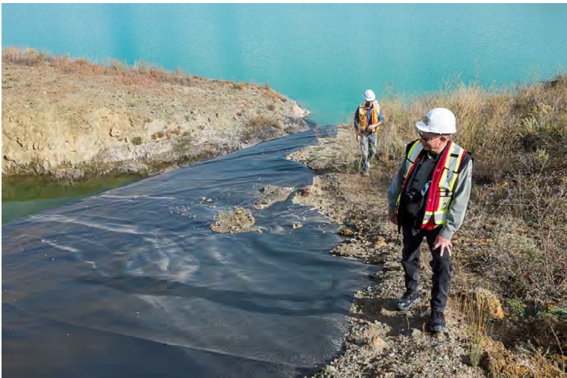
Photo PD16: View of the left abutment and upstream toe of the Pothook Dam from the crest looking north.
