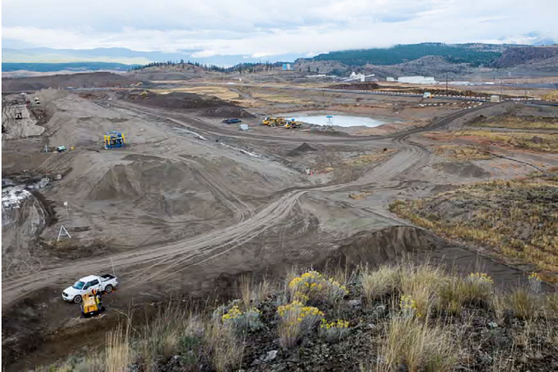
Photo S301: View looking northwest at Seepage Pond 3 from above the right abutment of Dam C adjacent to the survey shed. Dam C visible on the left side of the photo.
