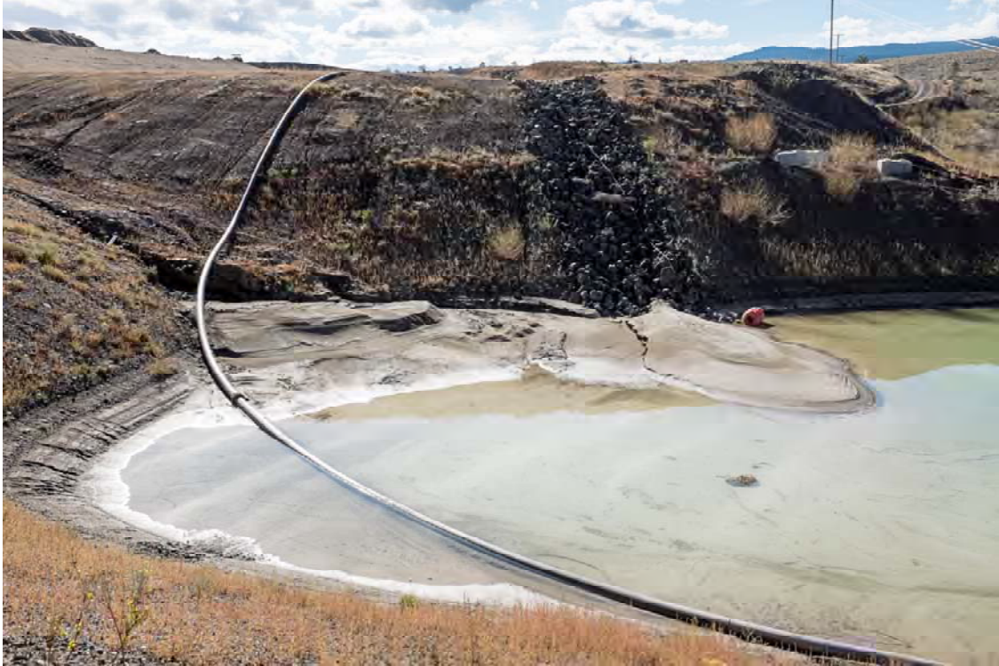
Photo S203: View of the inlet channel and erosion protection looking southwest from the north perimeter of Seepage Pond 2. Note sediment in pond and erosion at inlet from Dam B.
