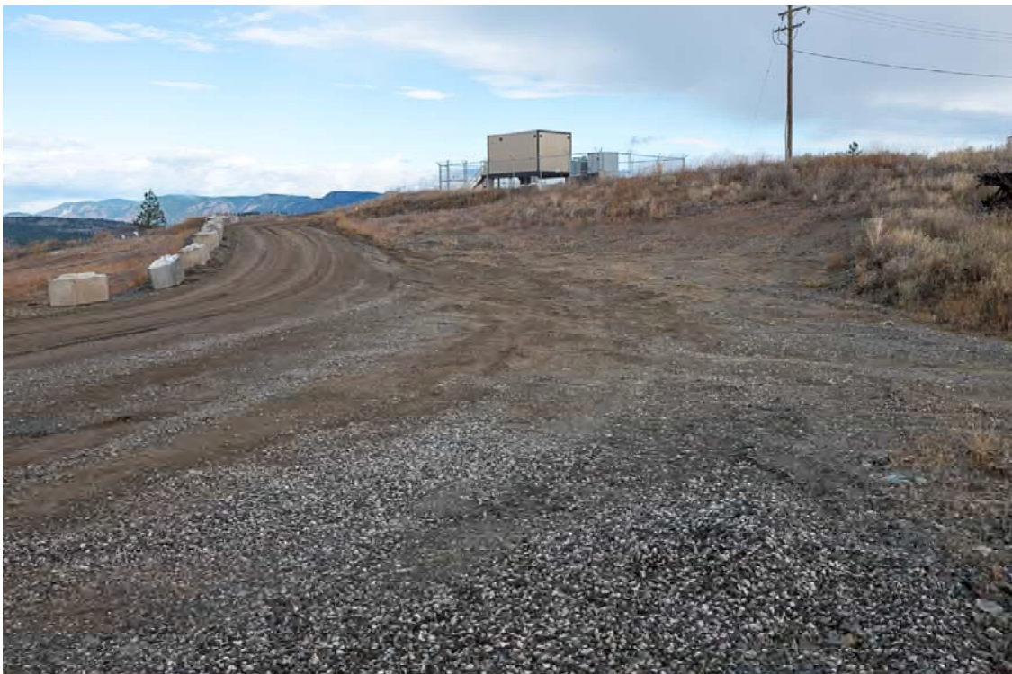
Photo SD22: View of the left abutment and the primary cyclone from the left abutment of the South Dam looking north.
