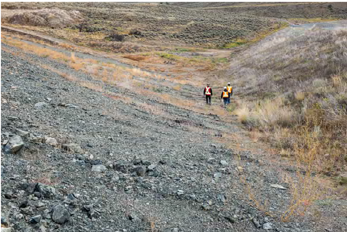
Photo SD14: View of the downstream right abutment and toe from mid-way down the slope.
