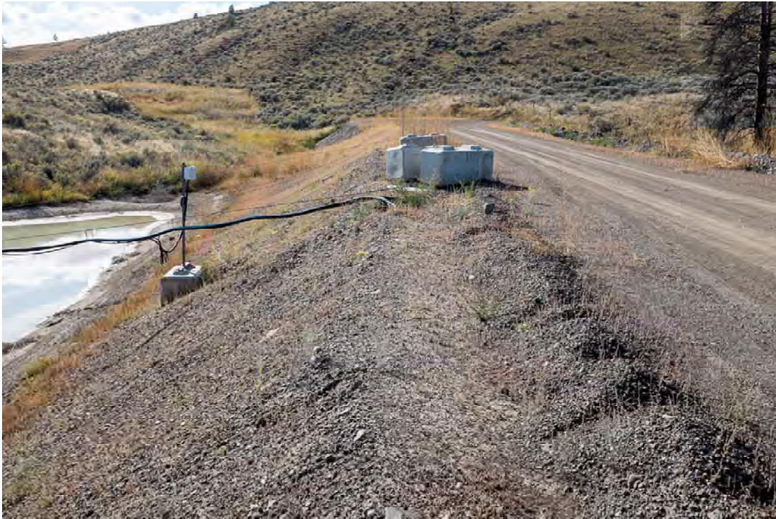
Photo S209: View looking south at western perimeter of Seepage Pond 2. Note uniform slope.
