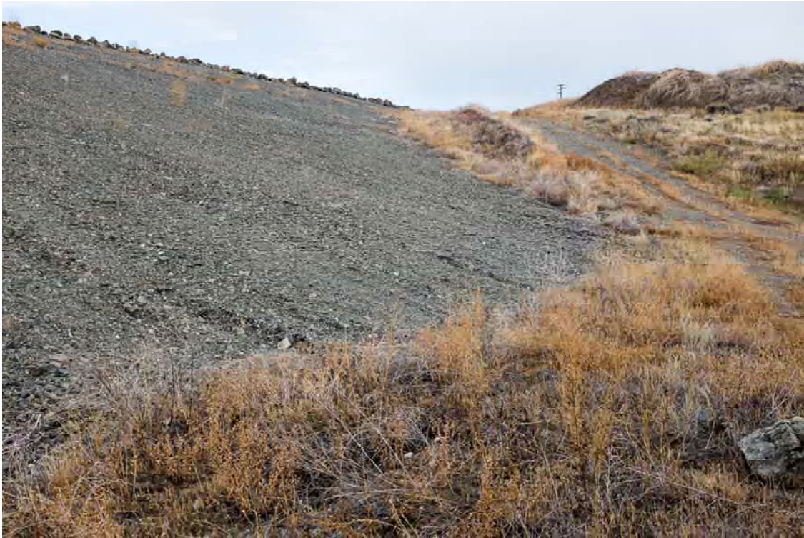
Photo SD17: View of the left abutment and downstream face from the downstream toe of the South Dam.
