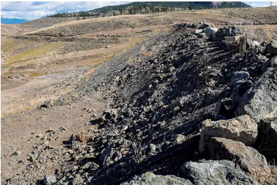
Photo WD06: View of the upstream face and toe from the right abutment of the West Dam looking toward the left abutment.
