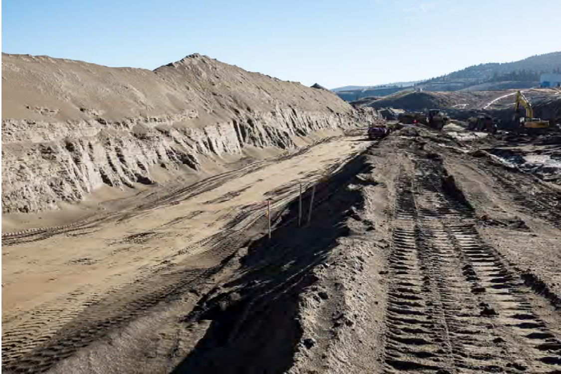
Photo DC21: View looking east toward right abutment of Dam C of crest and limit of downstream sand cell.
