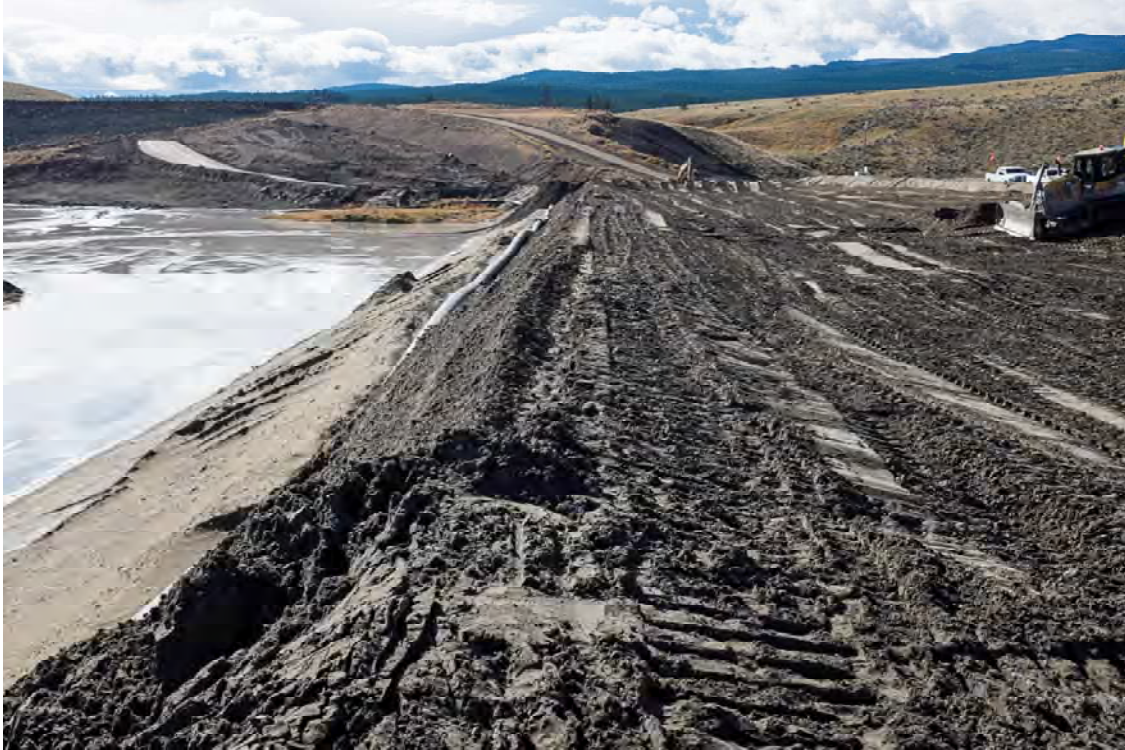
Photo DA05: View looking south at left abutment of Dam A from upstream limit of upstream sand cell. West Dam visible at top left of photo.
