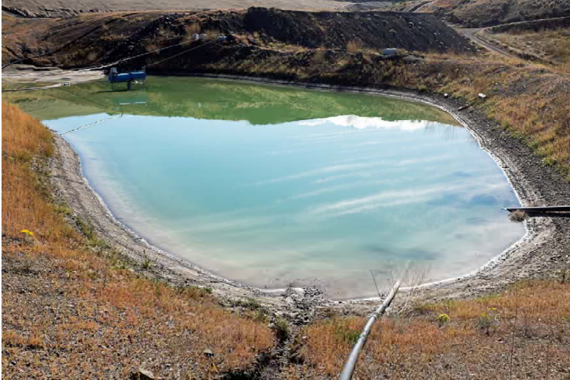
Photo S205: View of Seepage Pond 2 from northwest end of impoundment. Dam B visible in the background. Note erosion on slope in foreground.
