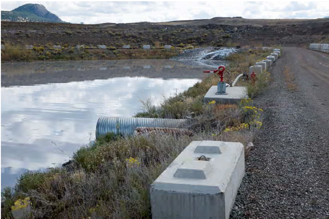
Photo TL10: View looking south at the Spill Pond where the inlet line enters the pond. Note the water level relative to the inlet culvert level.
