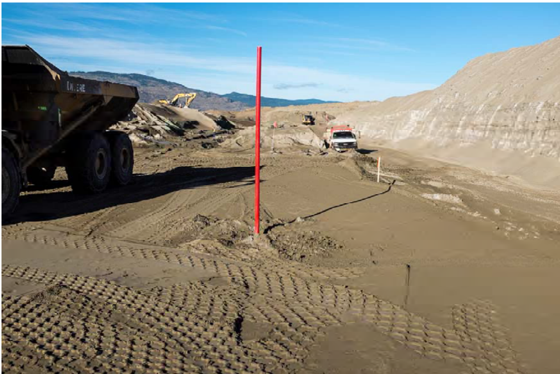
Photo DC36: View looking west at inclinometer riser pipe recently installed on the crest of Dam C at approximately sta. 0+700 m. Note tire tracks from articulated trucks around inclinometer casing. Vibrating wire piezometer leads flagged in the background behind inclinometer casing.
