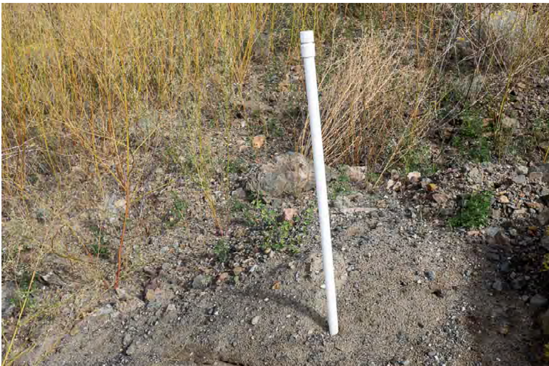
Photo PD28: View of standpipe piezometer casing at downstream toe of Pothook Dam north of the tailings pipeline ramp.
