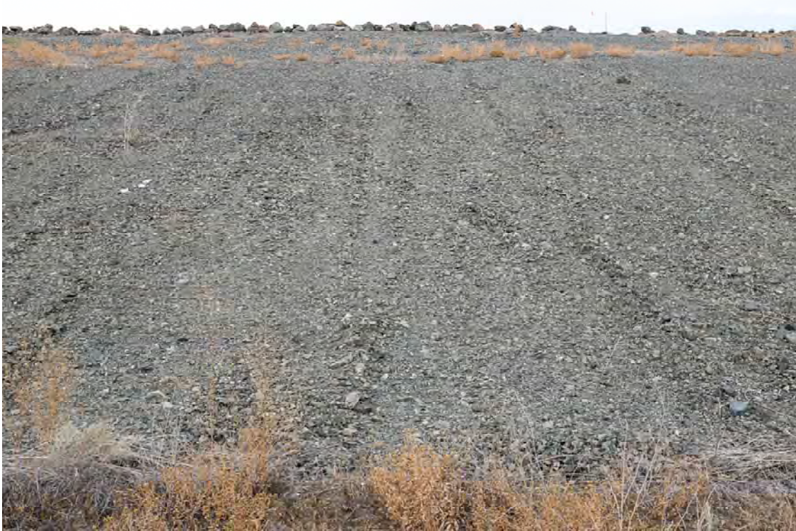
Photo SD15: View of the downstream face from the downstream toe of the South Dam. Note uniform slope and minimal vegetation.
