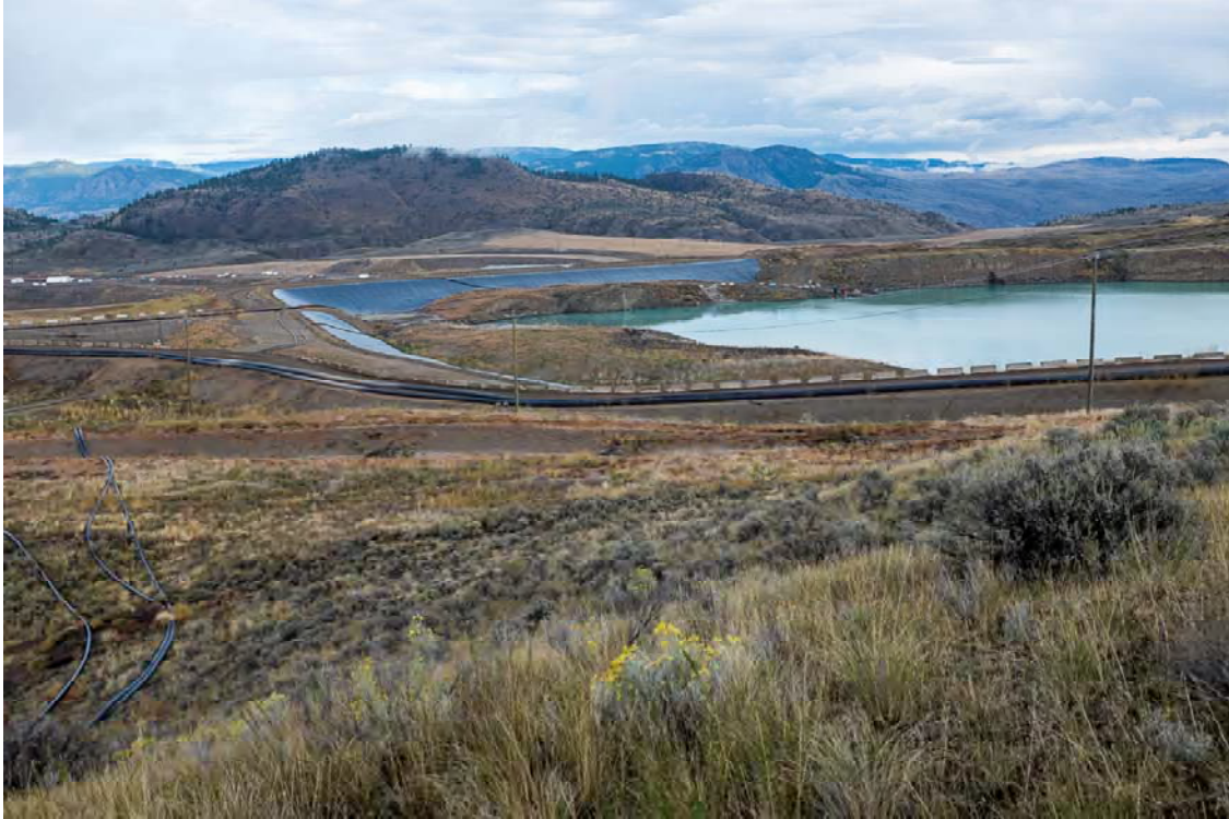
Photo PD01: View of the Pothook Dam and Pothook Pit from the survey shed above the right abutment of Dam C looking north.
