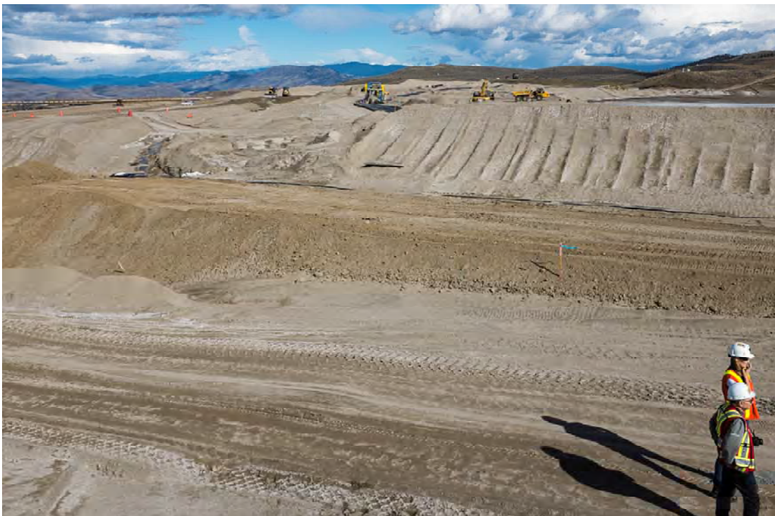
Photo DB12: View looking northeast at right abutment and crest of Dam B from downstream side of crest. Dam C visible at top right of photo. Note exposed liner and prepared slope for liner raise.
