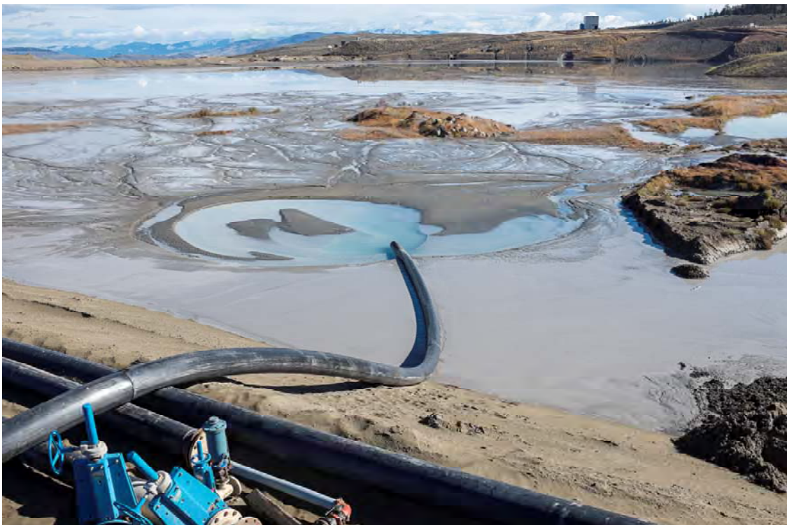
Photo DA06: View looking northeast along secondary overflow spigot line on upstream sand cell on Dam A at approximately 1+700 m.
