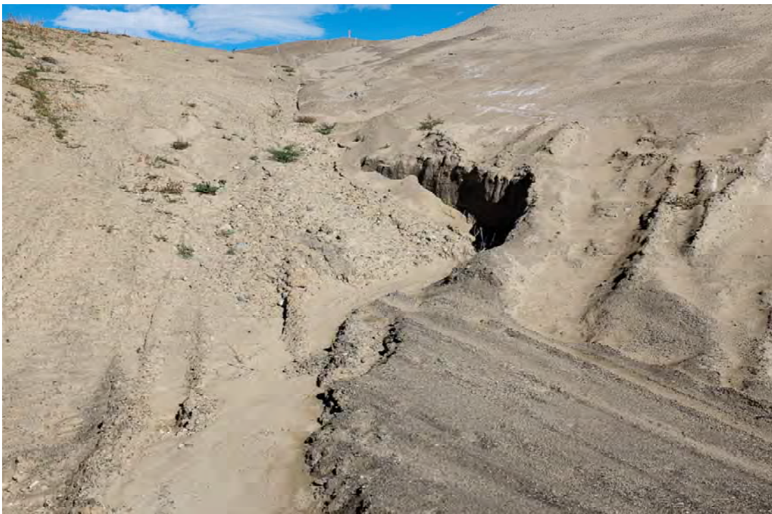
Photo DB08: View looking northeast at the downstream toe at approximately sta. 1+300 m. Note erosion of downstream toe.
