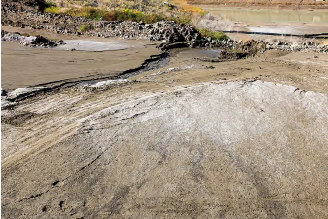
Photo DA17: View looking west at downstream toe of Dam A. Note loose saturated sand deposited at the toe of the dam immediately upstream of Seepage Pond 1 visible at top right of photo.
