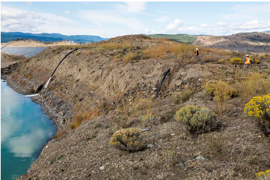
Photo PD36: View of tension cracks in the upper till unit along the north rim of Pothook Pit adjacent to the Emergency Spillway looking west
