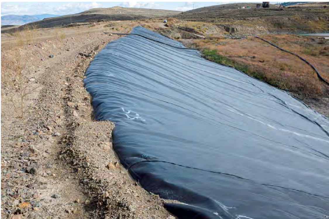
Photo PD24: View of the upstream face and right abutment of the Pothook Dam from the crest at the first dogleg looking east.
