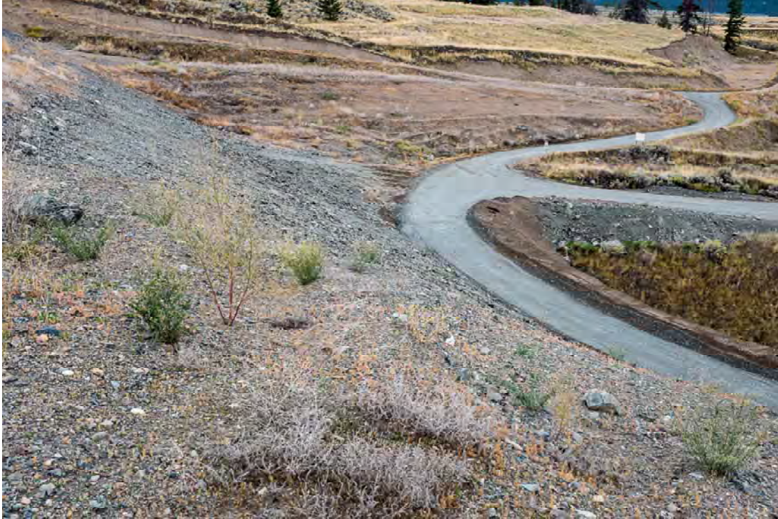
Photo SD03: View of South Dam upstream toe from mid-way down the slope on left abutment looking toward upstream toe.
