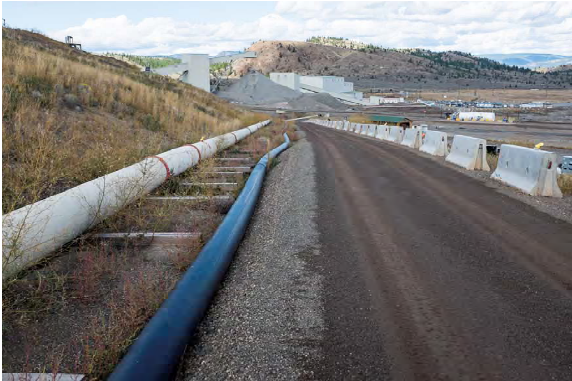
Photo TL05: View of steel tailings line just upslope of mill. Note survey prisms strapped to tailings line. In some locations along line, cribbing used to elevate line where subsidence has occurred along right of way.
