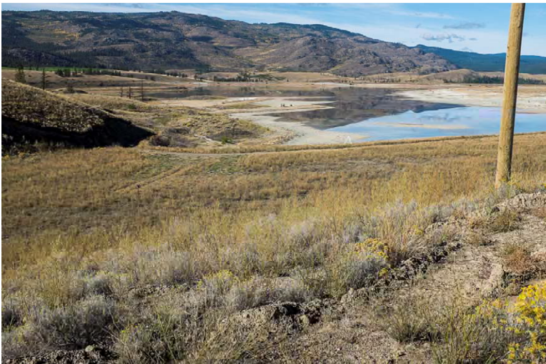
Photo S210: View looking west at downstream slope from Seepage Pond 2 and Teck TSF from western limit of Seepage Pond 2.
