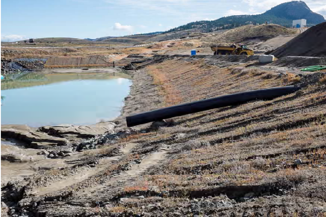
Photo S309: View of south and east sides of Seepage Pond 3 from the south west corner. Primary Cyclone visible in top right of photo.
