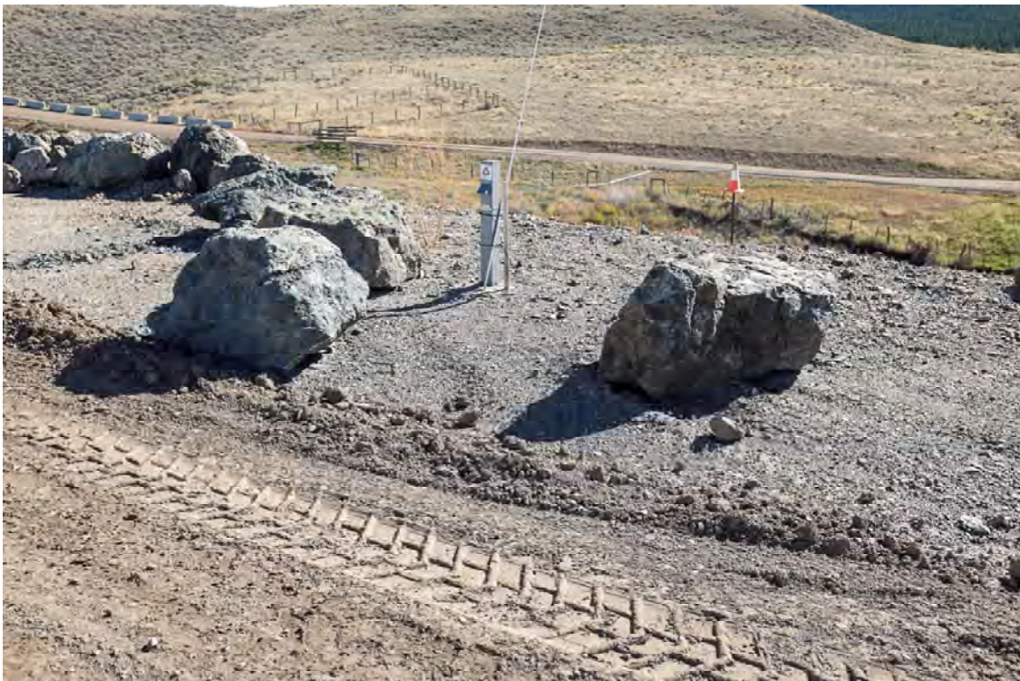
Photo WD18: View looking south at inclinometer monument installed on the downstream crest at the mid-point of the West Dam. Note rock protection. Settlement plate riser pipe on the downstream face of the dam visible in the background.
