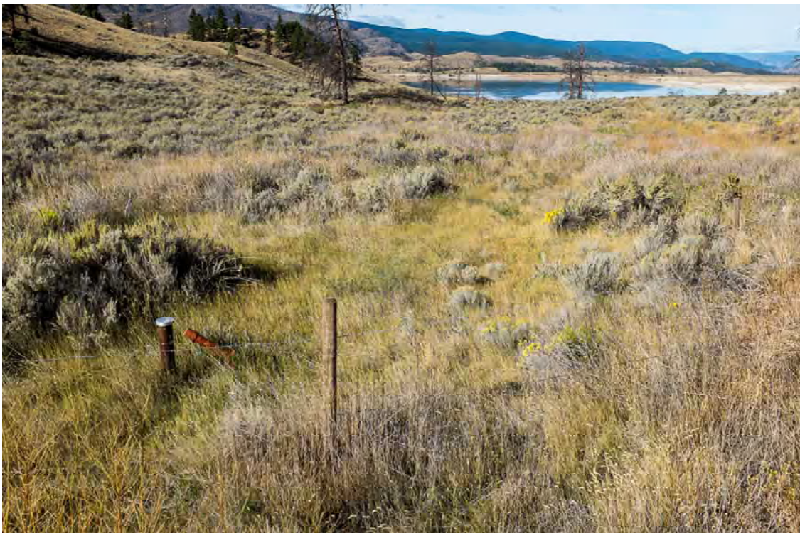
Photo S108: View of monitoring well looking west from downstream toe of Seepage Pond 1. Teck TSF visible in background.
