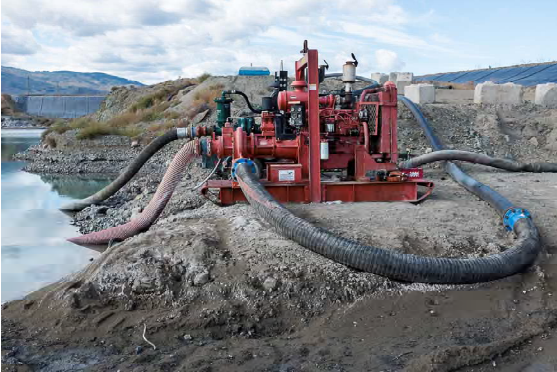
Photo PD33: View of pump station in the Pothook Pit upstream of the right abutment of the Pothook Dam looking west.
