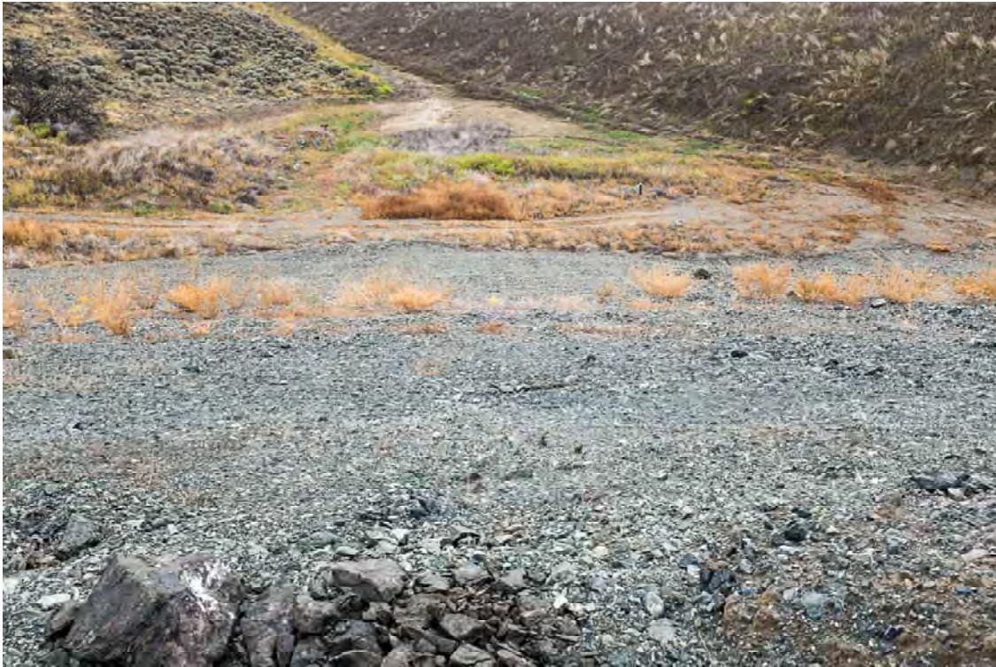
Photo SD11: View of downstream toe of South Dam from mid-point of dam crest.
