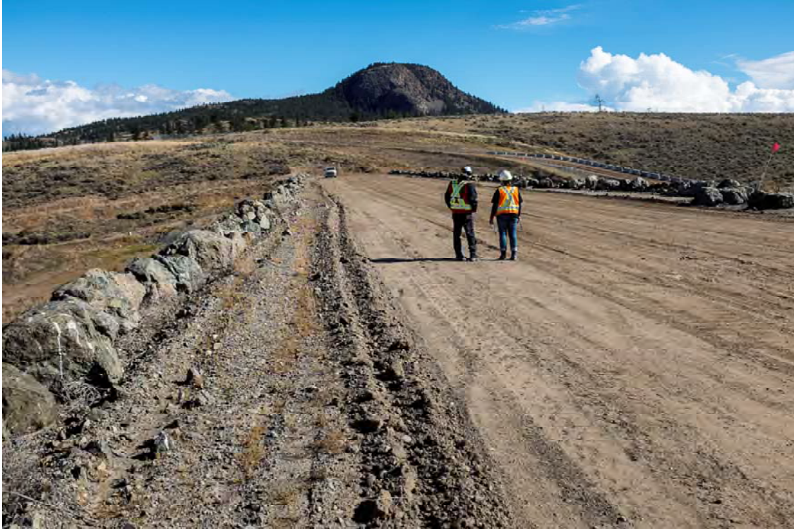
Photo WD05: View of the crest and left abutment of the West Dam from the mid-point of the dam at the upstream side of the crest.
