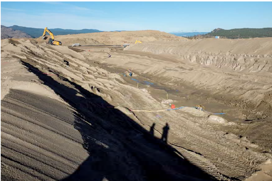
Photo DC16: View looking west along Dam C crest. Pounded water directed to sump and pumped to TSF impoundment.
