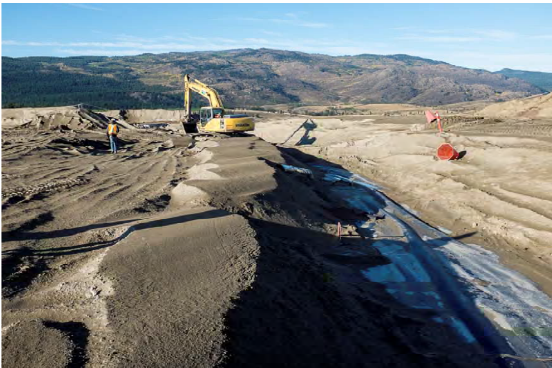
Photo DC14: View of LLDPE liner exposed near left abutment of Dam C looking west. Note tears in liner from excavation and exposure of liner. All damage to liner upstream of seamed liner raise to be repaired.
