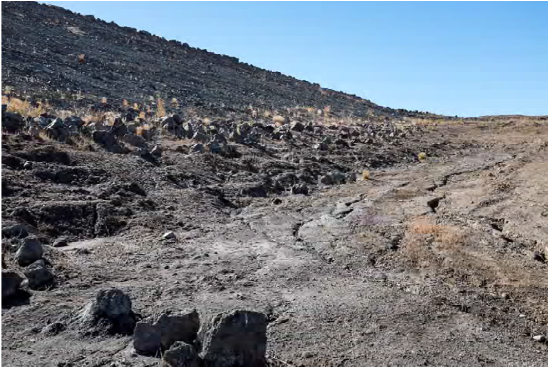
Photo WD09: View of the upstream face and right abutment of the West Dam from the upstream toe.
