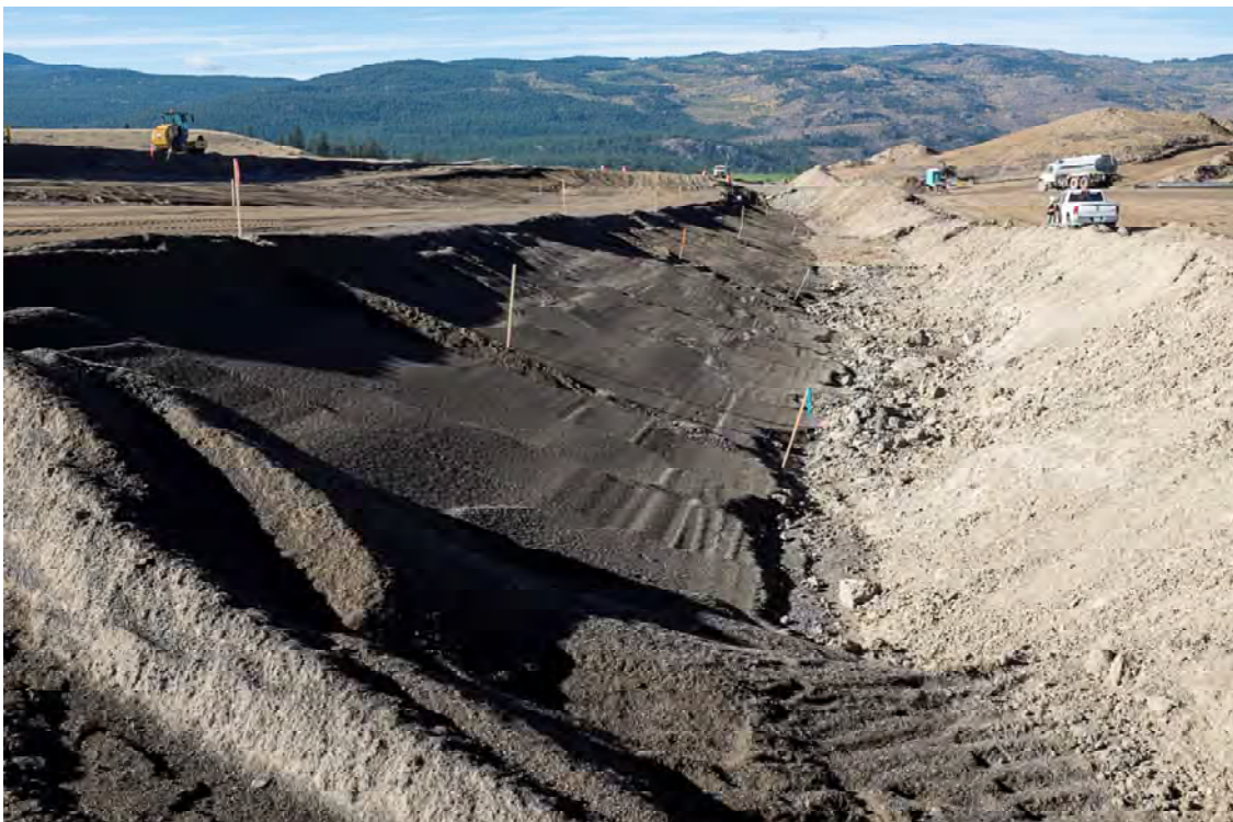
Photo DC30: View looking southwest at downstream toe of Dam C from sta. 1+100 m. Right abutment of Dam B visible in background.
