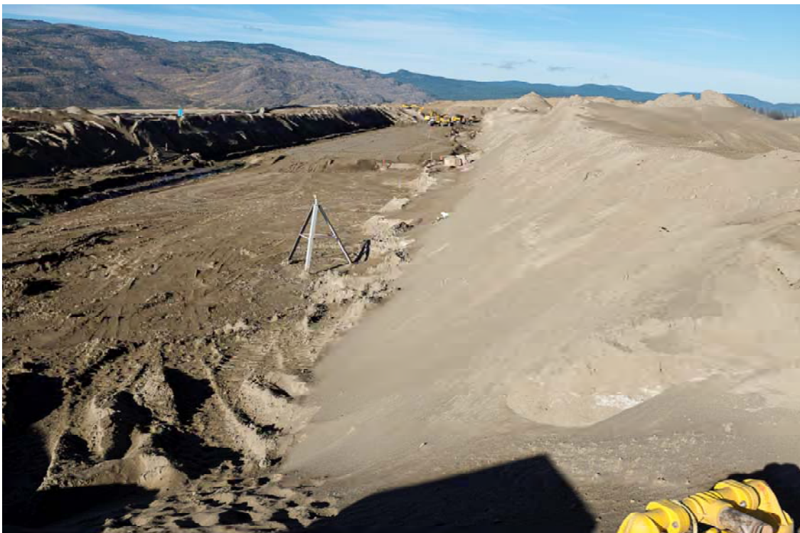
Photo DC34: View looking west from crest at right abutment of Dam C. Note survey tripod, and slope inclinometer protected by Lock-Blocks on downstream side of crest.
