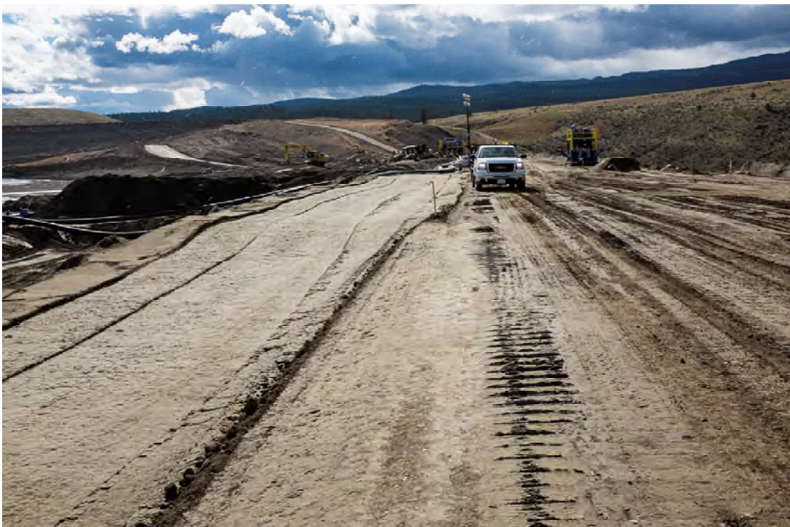
Photo DA10: View looking south toward left abutment of Dam A from upstream side of crest at approximately sta. 1+700 m.
