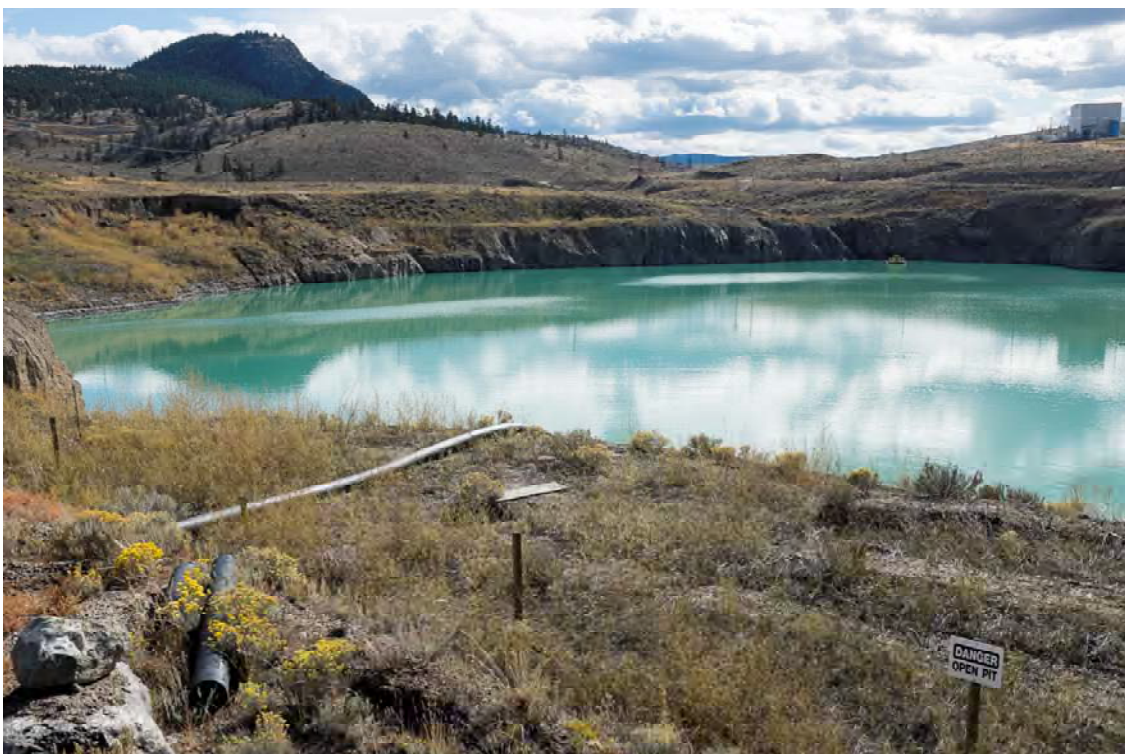
Photo PD40: View of eastern rim of Pothook Pit from west of Emergency Spillway looking southeast.
