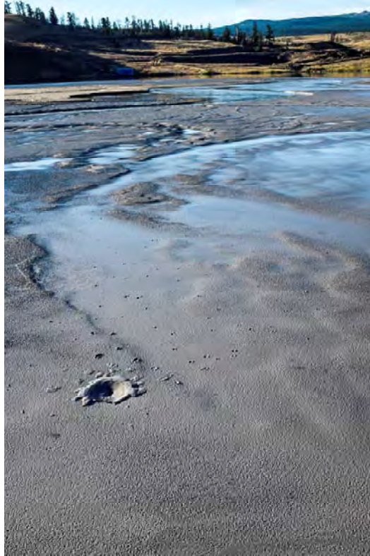
Photo DC05: View of tailings immediately upstream of Dam C looking south. Note crater in beach from rock thrown into tailings.
