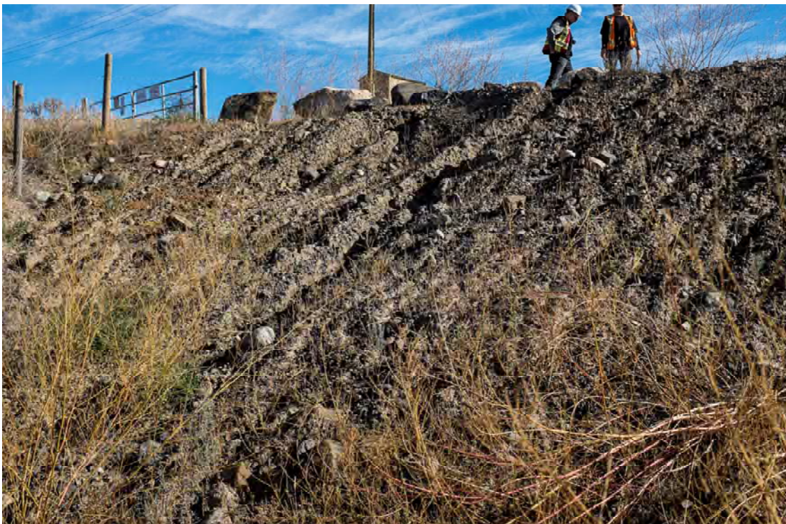
Photo S104: View of downstream face of Seepage Pond 1 Dam at right abutment. Note erosion and rilling of dam face.
