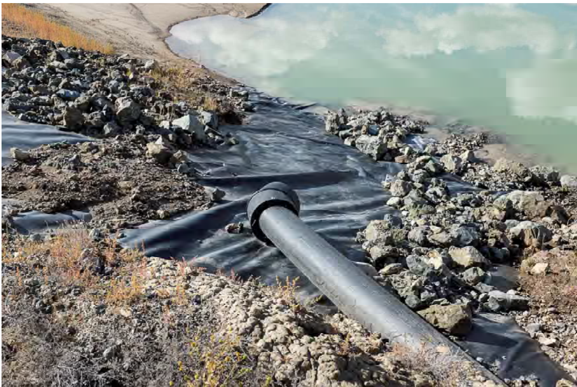
Photo S306: View of pipe outlet and liner slope protection on the west side of Seepage Pond 3.
