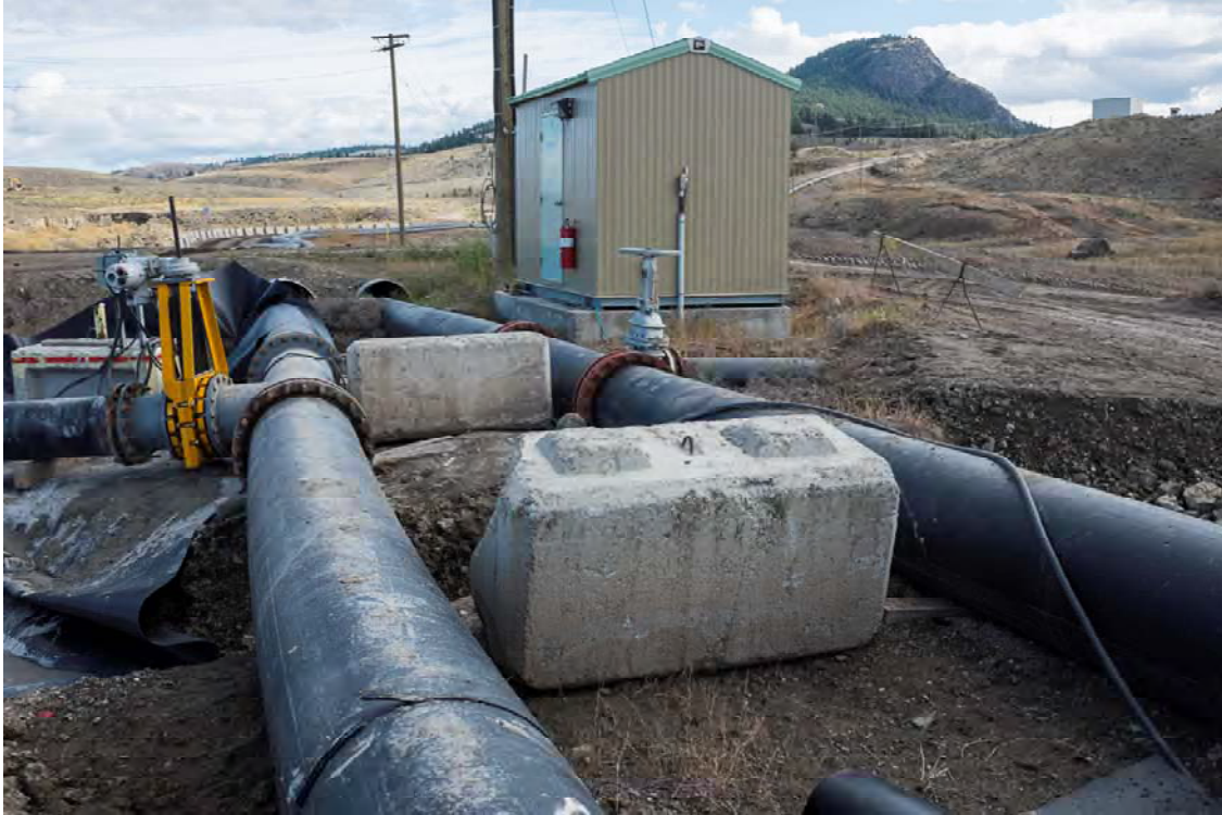
Photo TL01: View looking east along tailings line from Seepage Pond 3 E-House upstream to Primary Cyclone on top right of photo.
