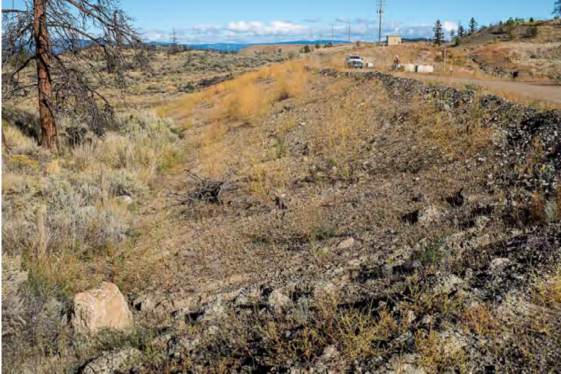
Photo S109: View of downstream face and crest of Seepage Pond 1 Dam from left abutment. Note vegetation on downstream face.
