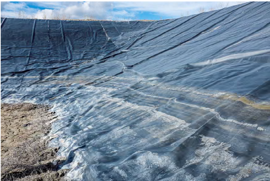
Photo PD06: View of first dogleg in the Pothook Dam from the upstream toe.
