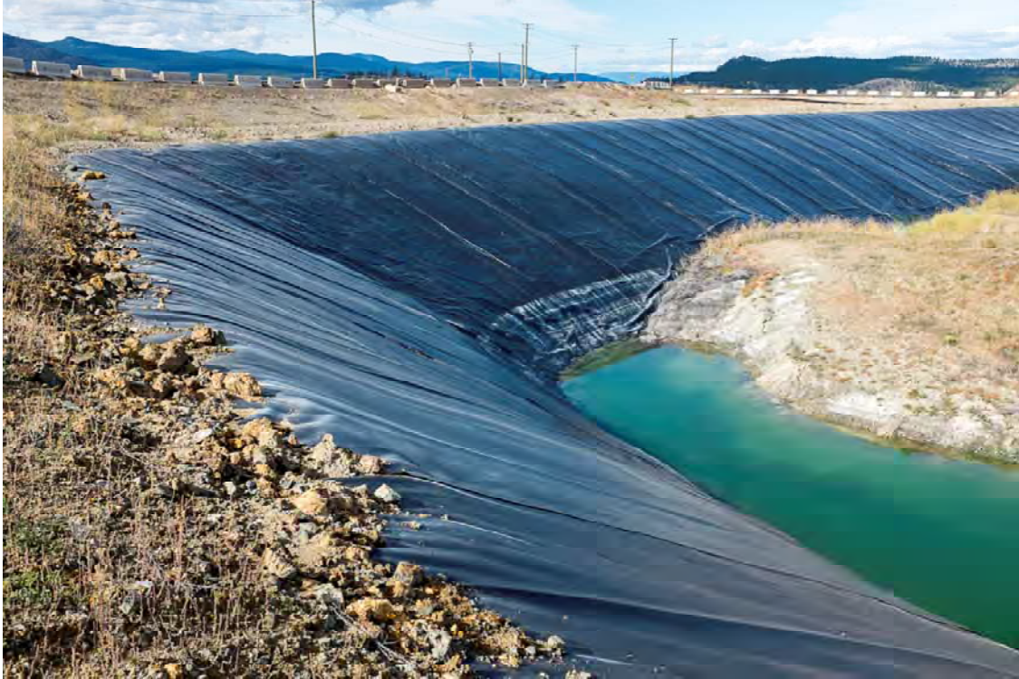
Photo PD17: View of the upstream face of the Pothook Dam from the crest looking west at the second dogleg. Note high water mark on the liner at the upstream toe.
