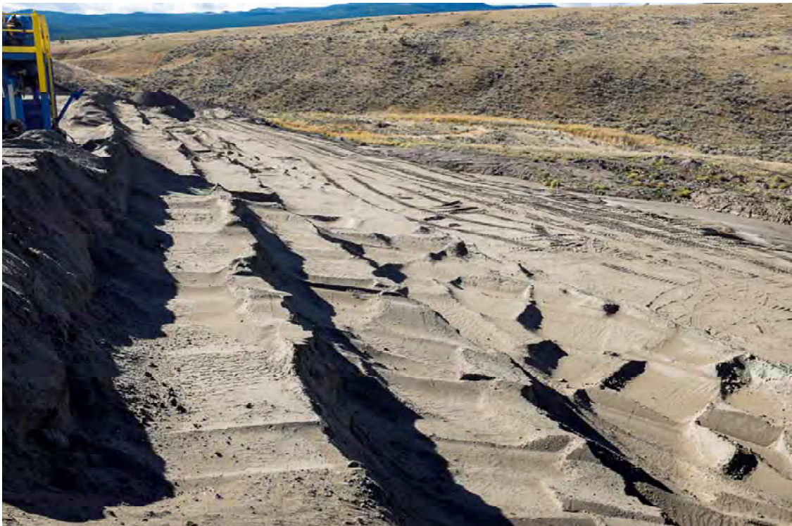
Photo DA14: View looking south at downstream face of Dam A from crest at approximate mid-point of dam. Note stepped downstream slope due to mining of hydraulically placed sand.
