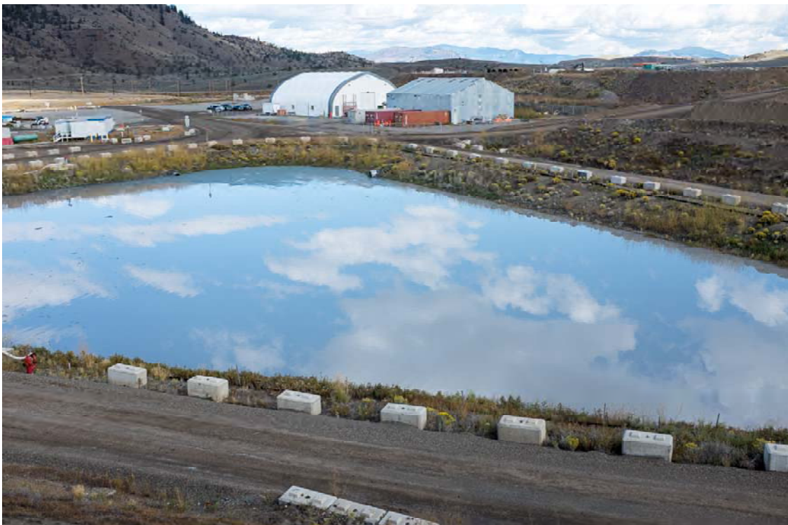
Photo TL12: View of Spill Pond from top of hill adjacent to ore stockpile looking northeast. Note water level relative to inlet culverts and algae rafts on pond surface at top right of photo.
