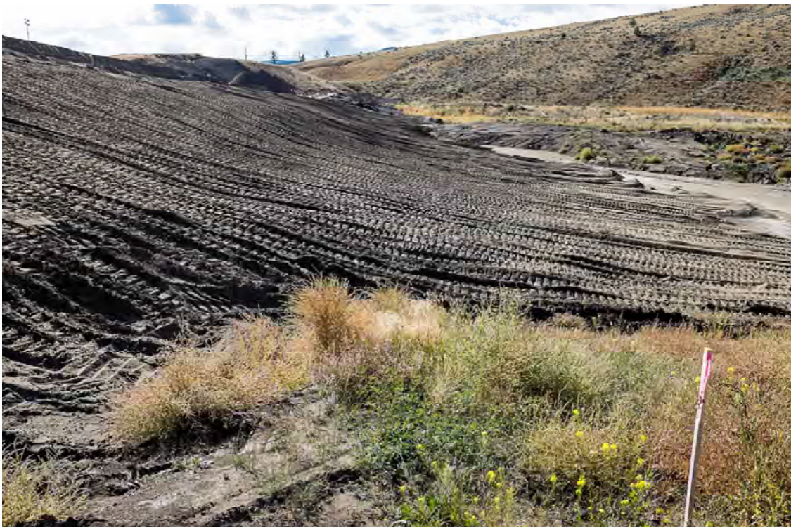
Photo DA16: View looking south at downstream toe and face, and left abutment of Dam A from downstream toe near mid point of dam. Note dressed downstream face.
