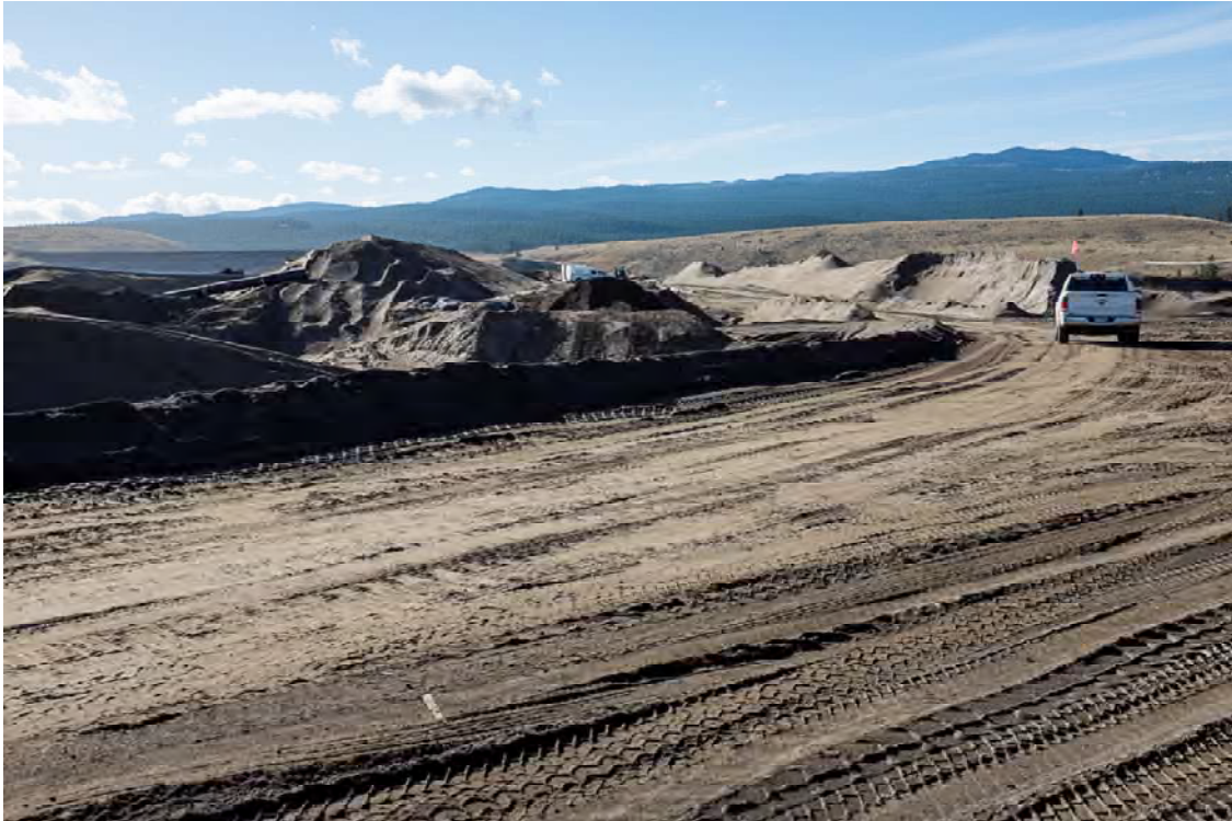
Photo DC33: View looking south at left abutment of Dam C and right abutment of Dam B from downstream toe of Dam C. Note liner raise being prepared on Dam B in middle background of photo where trucks and personnel visible.
