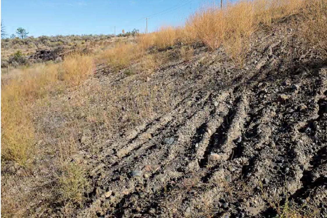
Photo S105: View of downstream face from downstream toe of Seepage Pond 1 Dam looking toward right abutment. Note rilling and vegetation on dam face.
