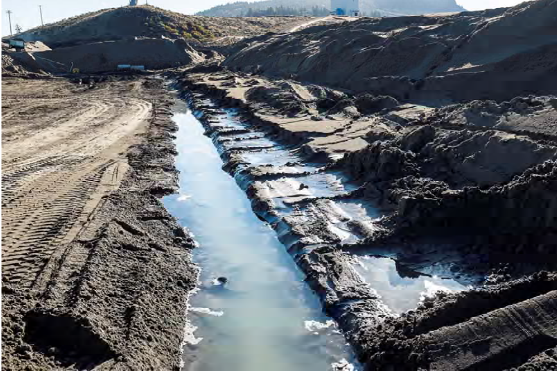
Photo DC19: View looking east at liner exposed along anchor trench on Dam C right abutment. Note tears in liner from excavation to expose liner. Damage to be repaired if upstream of seaming to liner raise.
