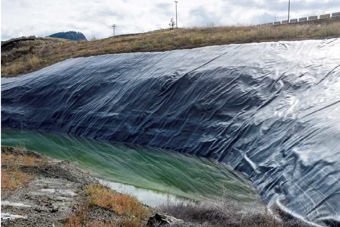
Photo PD13: View of the liner on the upstream face of the Pothook Dam at the left abutment looking south. Note punctures across the entire liner surface.
