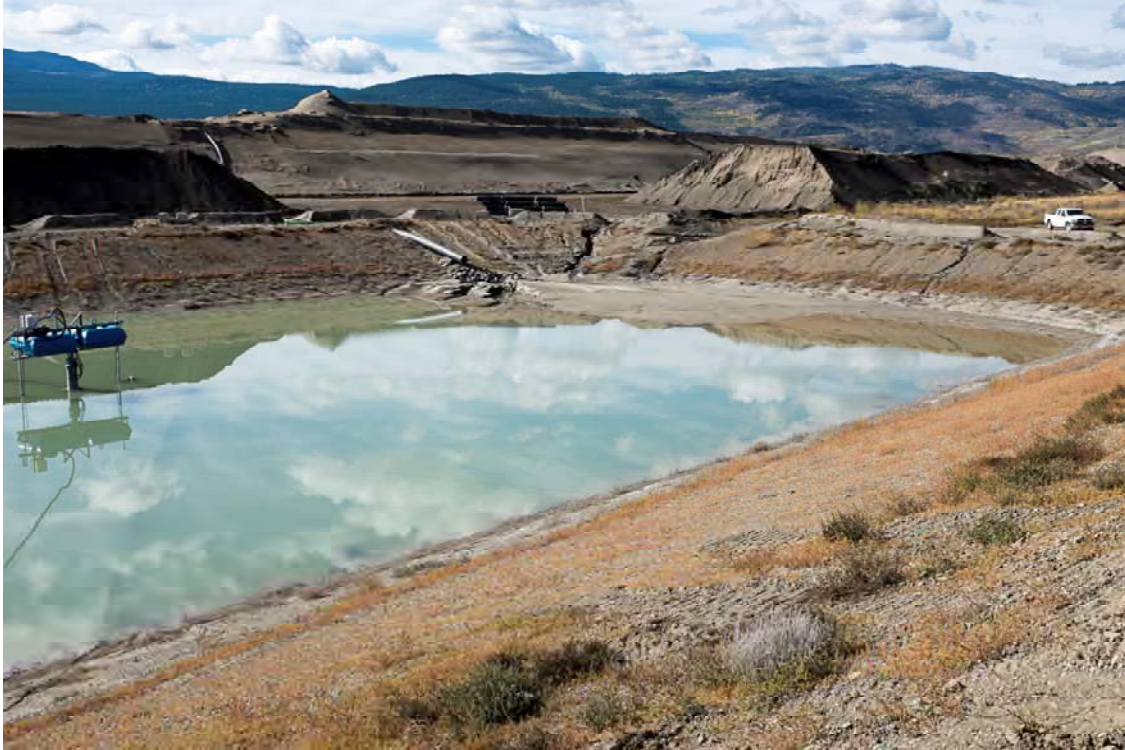
Photo S303: View of the west and south sides of Seepage Pond 3. Note erosion of slopes in the vicinity of the inlet channels, and sediment in the vicinity of the decant pipe discharge.
