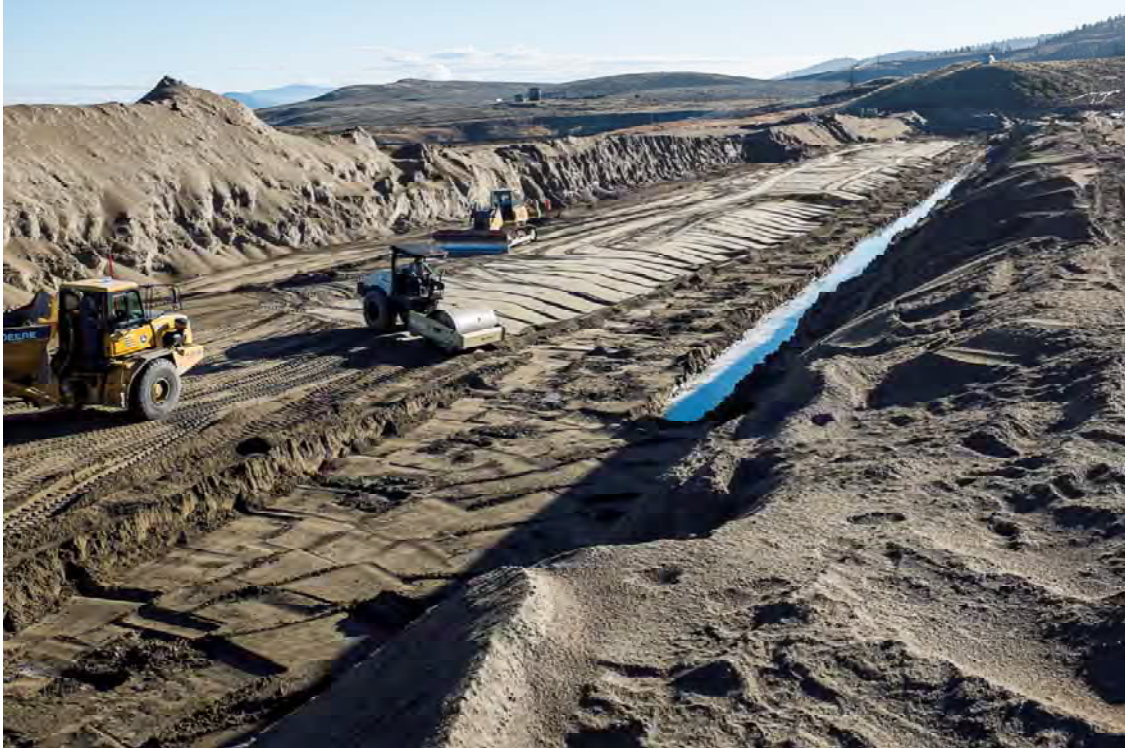
Photo DC15: View looking northeast of crest from mid-point of Dam C. Right abutment of Dam C visible in top right of photo. Pounded water visible along trench where liner is exposed along the crest of the Dam C starter dam.
