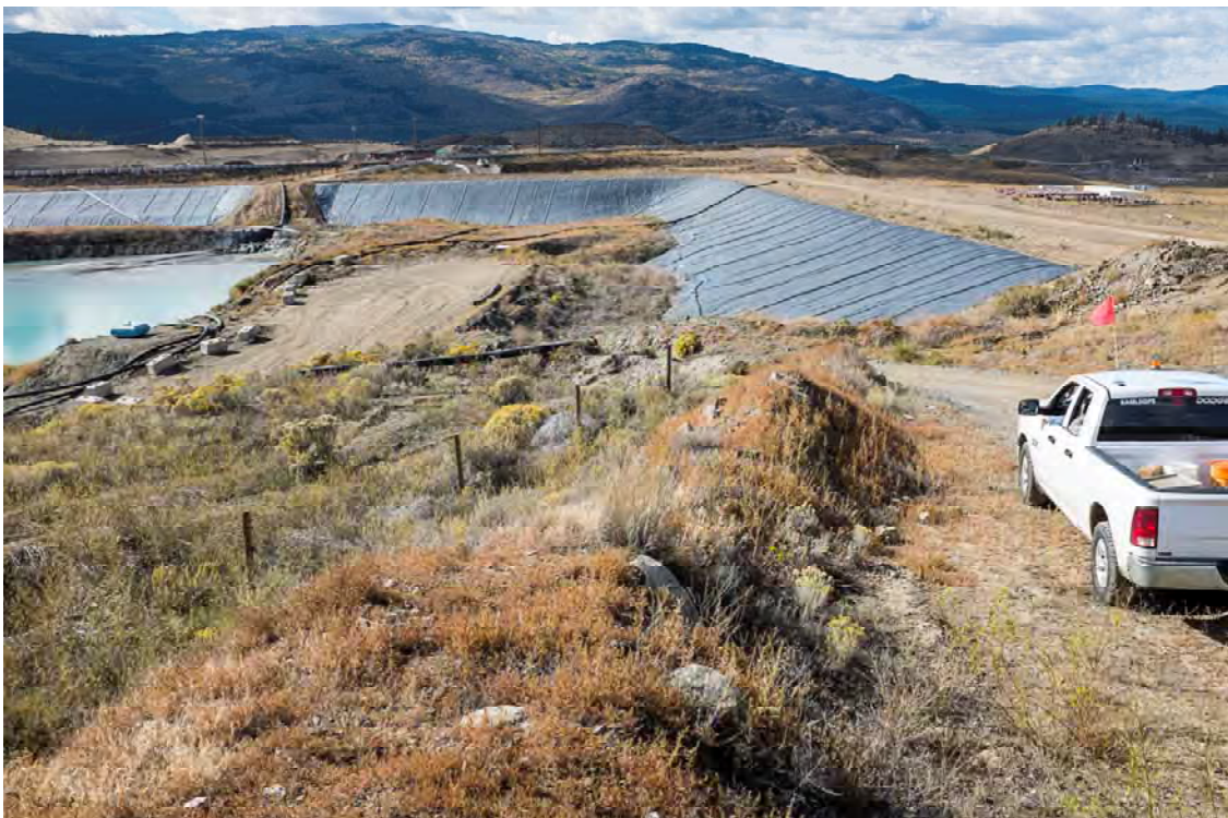
Photo PD42: View looking west at left abutment of Pothook Dam and first dogleg from west of the Emergency Spillway.
