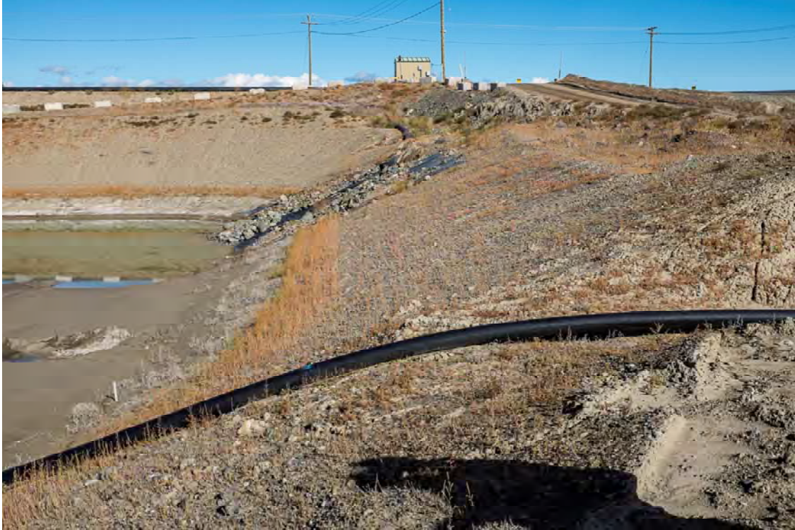
Photo S307: View of the west and north sides of Seepage Pond 3 from the south east corner. E-House and tailings line visible in background.
