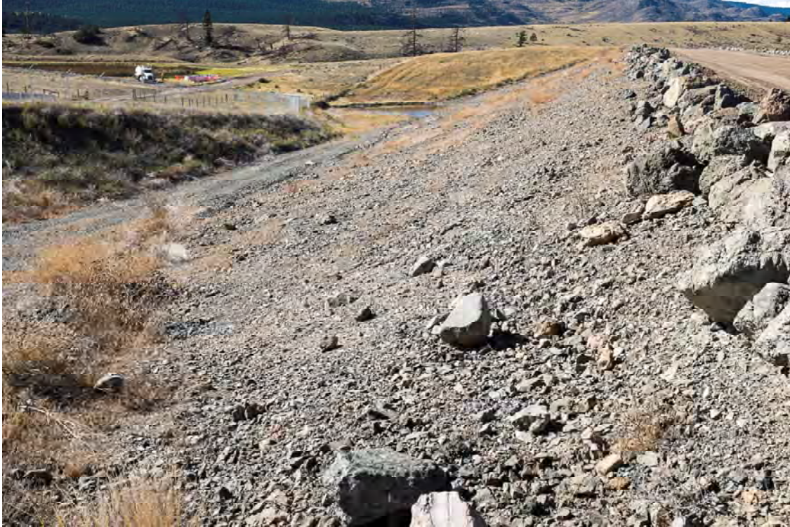
Photo WD11: View of the downstream slope and toe of the West Dam from the rest at the left abutment looking west.
