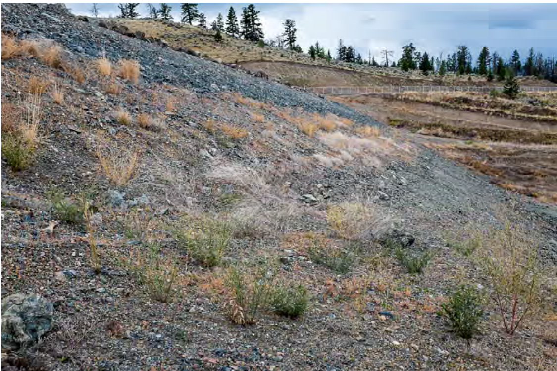
Photo SD02: View of South Dam upstream face and toe from mid-way down the slope on left abutment looking toward right abutment.
