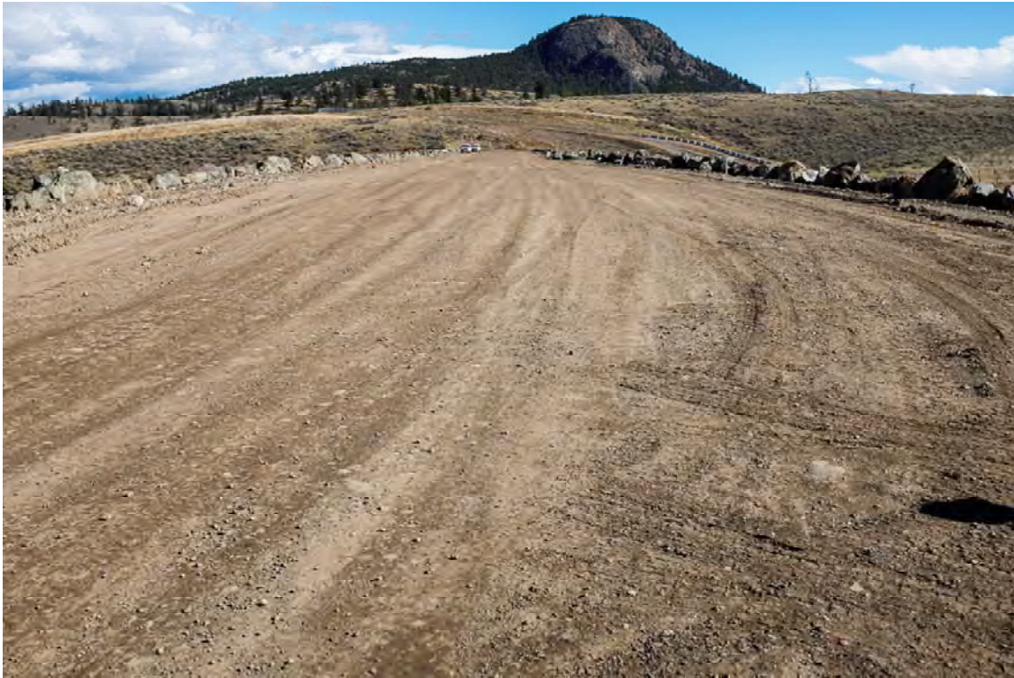
Photo WD17: View of the crest and left abutment of the West Dam from the right abutment.
