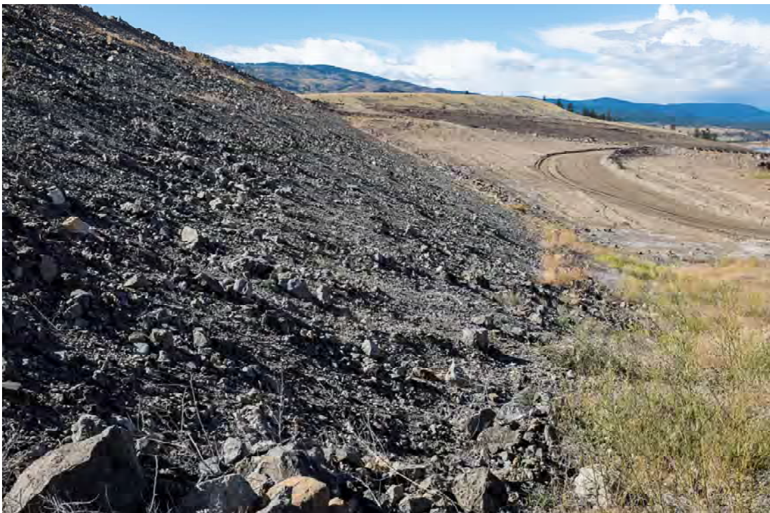
Photo WD10: View of the upstream face of the West Dam from mid-way up the upstream face on the left abutment looking west.
