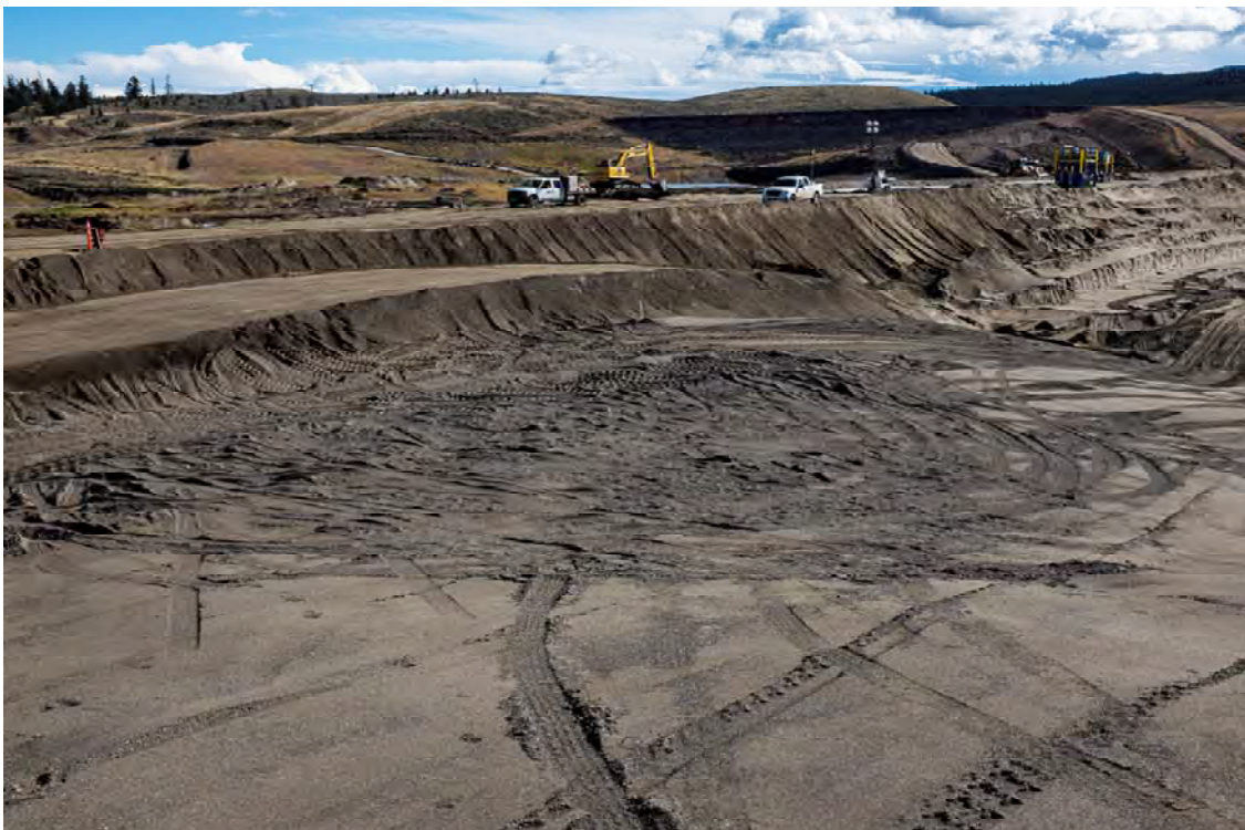
Photo DA12: View looking southeast at downstream face of Dam A from downstream toe of Dam A at boundary with Dam B. West Dam visible in upper right of photo.
