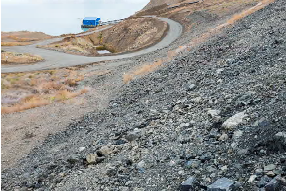
Photo SD07: View of reclaim barge and upstream toe of South Dam from mid-way up the right abutment on the upstream side. Note pond level relative to South Dam.
