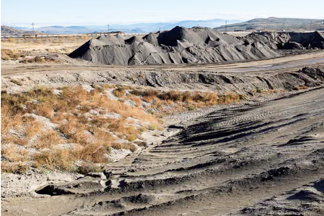
Photo DC31: View looking northeast at downstream toe of Dam C from approximately sta. 0+950 m. Note filter stockpiles and tailings pipeline in background.
