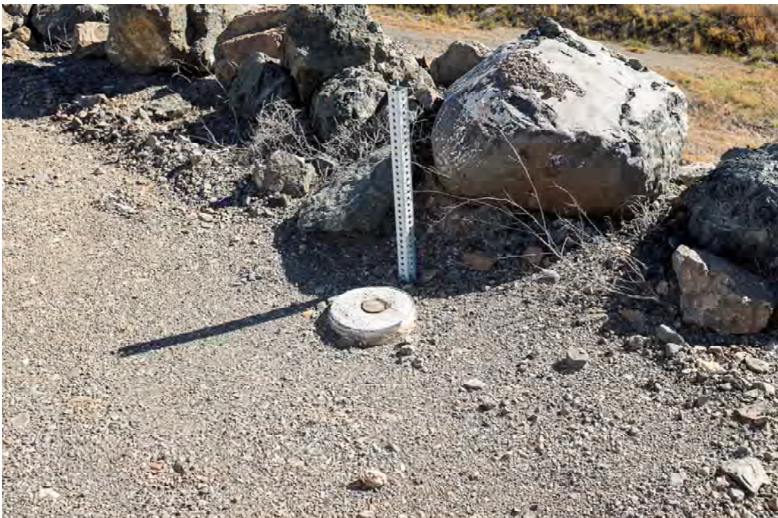
Photo WD20: View of survey monument on the downstream side of the crest of the West Dam near the mid-point of the dam.
