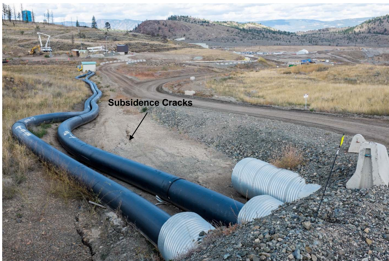
Figure 6-20. View looking north northwest at tailings line and water reclaim line. Tailings line is on the left and water reclaim line is on the right. Note subsidence cracks along pipeline corridor. October 1, 2014.
