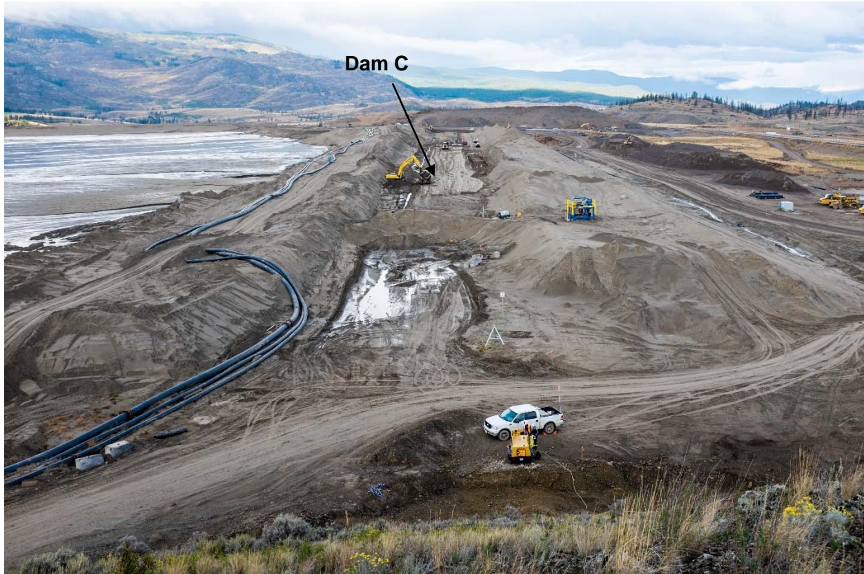
Figure 6-7. View looking west from approximately 75 m east of Dam C. Arrow pointing to mid-point of dam and till core at crest. September 30, 2014.
