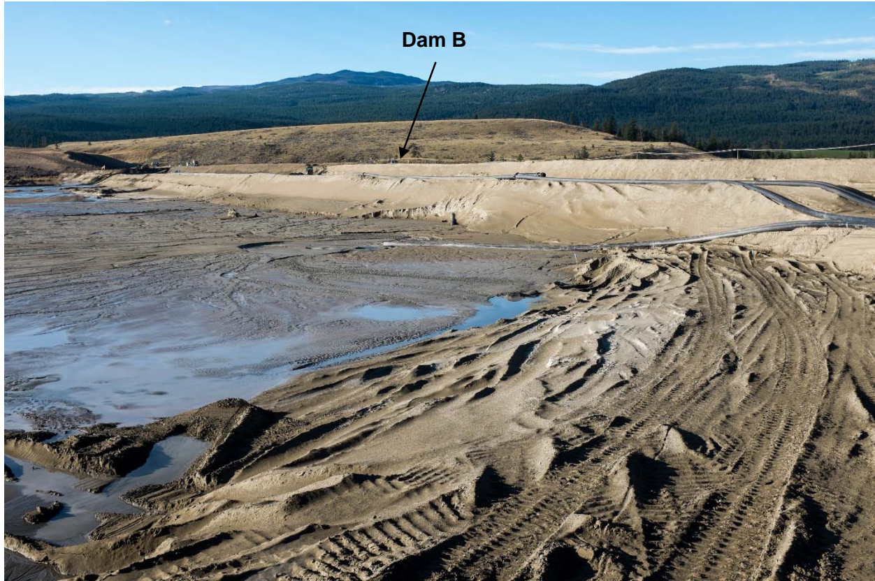
Figure 6-4. View looking north at Dam B from the upstream side of the left abutment of Dam C. Arrow pointing to mid-point of dam at upstream cyclone sand shell. October 1, 2014.
