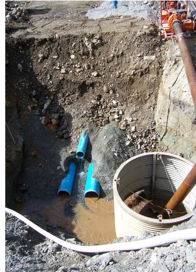
B) Outer drain conveyance pipes
