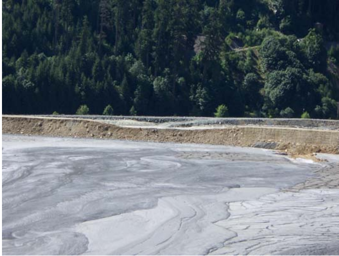
A) South paste berm with spillway swale
