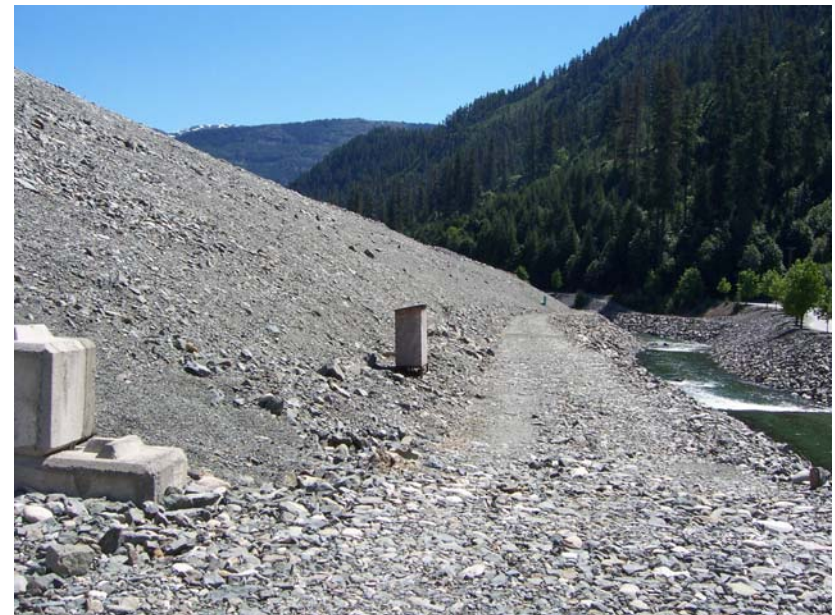
B) New TDF seismic upgrade berm slope 2:1
