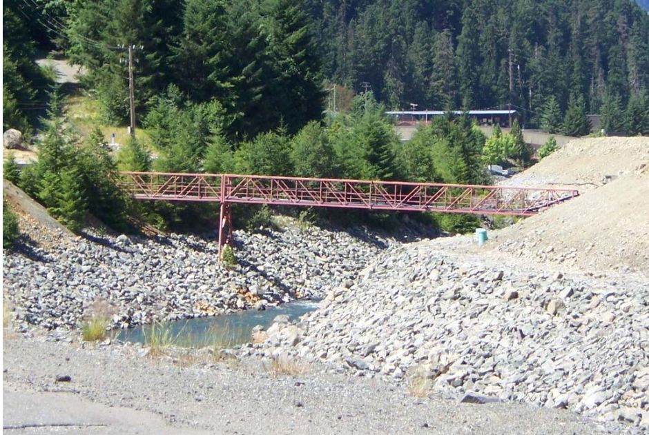
Red Pipe Bridge 0+1000 – conveys sand to backfill plant and overflow water from backfill plant to paste area.
