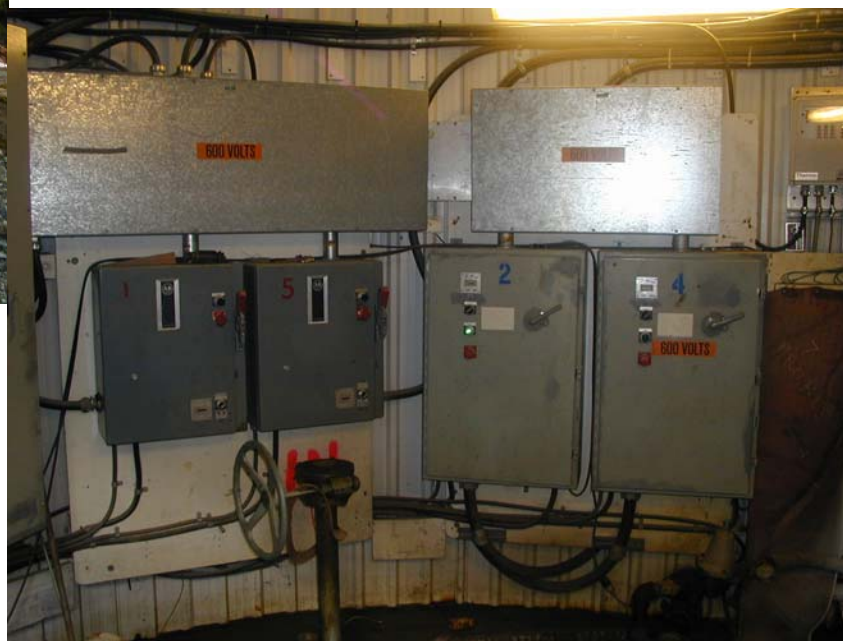
B) Inside No.4 Pumphouse – pump starter controls
