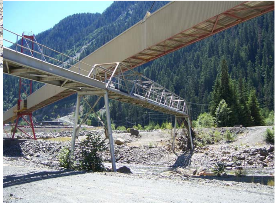
Grey Pipe Bridge 0-25 – conveys Super Pond discharge to Polishing Ponds and Sludge from Polishing Ponds to Paste Area during pond cleaning.
