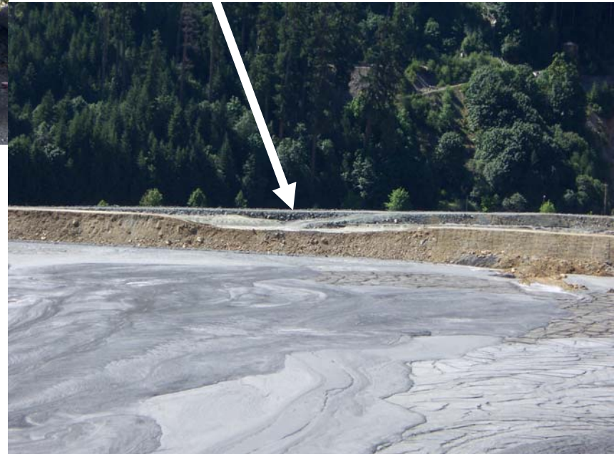
Paste Berm Spillway Swale
