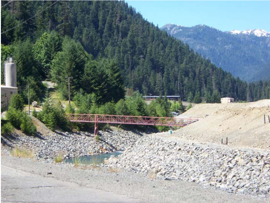
A) Riprap armouring for 1:1000 year flood protection
