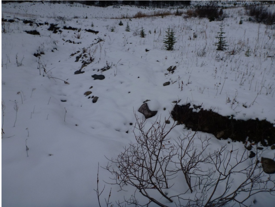
Photo 23 – Spillway channel erosion on downstream slope of TSF dam and on natural ground beyond downstream toe. Photo taken facing northeast.
