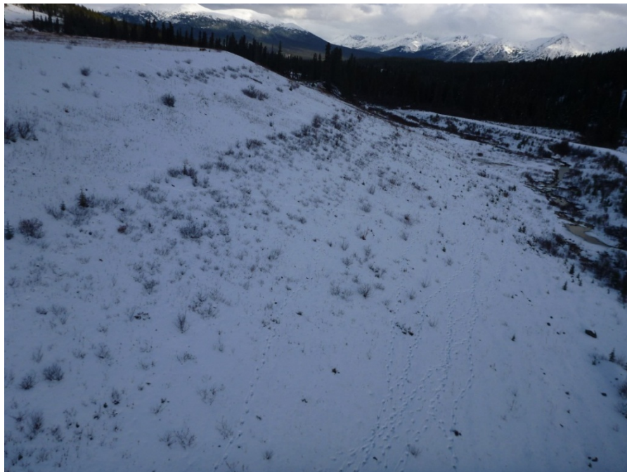
Photo 6 – View of downstream slope and crest of south limb of TSF dam at apex between south and north limbs. Photo taken facing north from helicopter. Note creek located beyond downstream toe of TSF dam.
