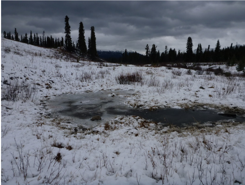
Photo 17 – Ponded water from seepage at toe of TSF dam. Photo taken facing north. This site is believed to be Seep-1 identified in the last inspection report (Piteau, 1997).
