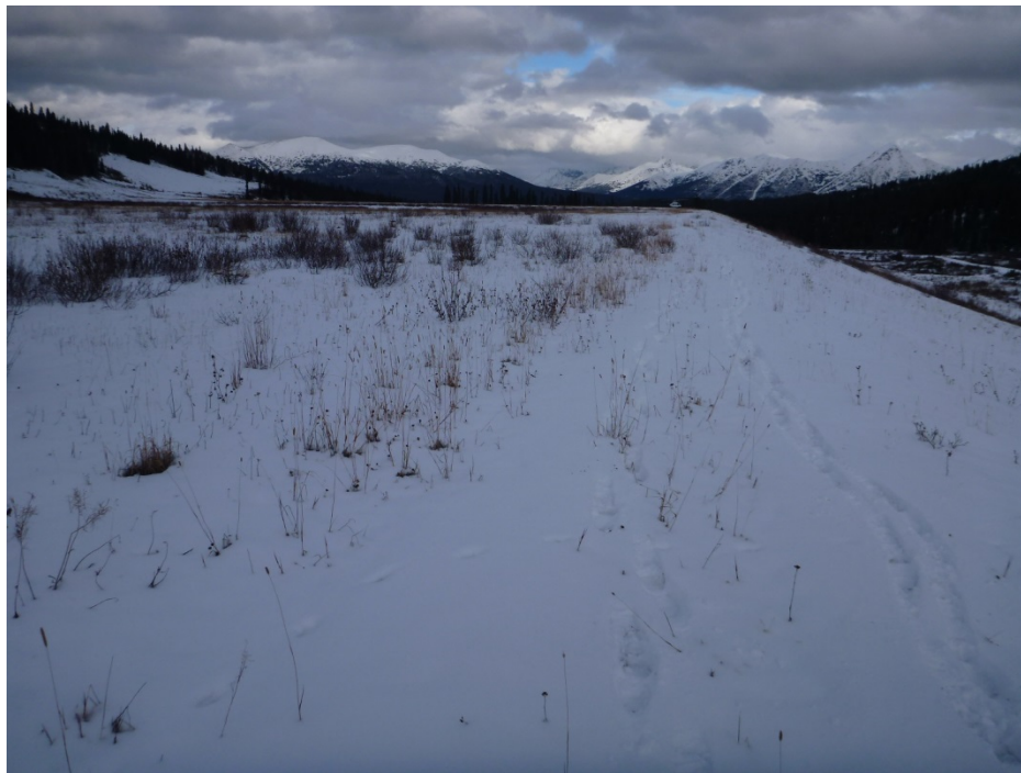
Photo 10 – Crest of south limb of TSF dam. Photo taken facing northeast.
