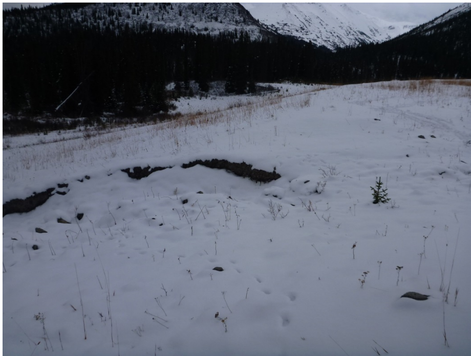
Photo 22 – Spillway channel erosion at downstream crest of dam. Photo taken facing southeast.
