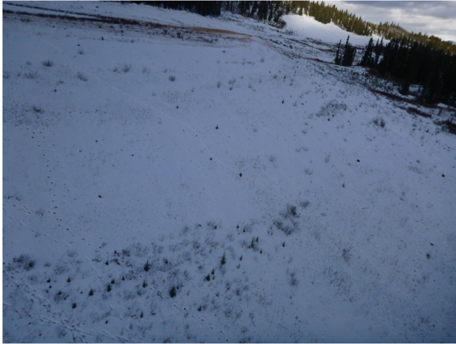
Photo 7 – Downstream slope at apex of south and north limbs of TSF dam. Photo taken facing northwest from helicopter.
