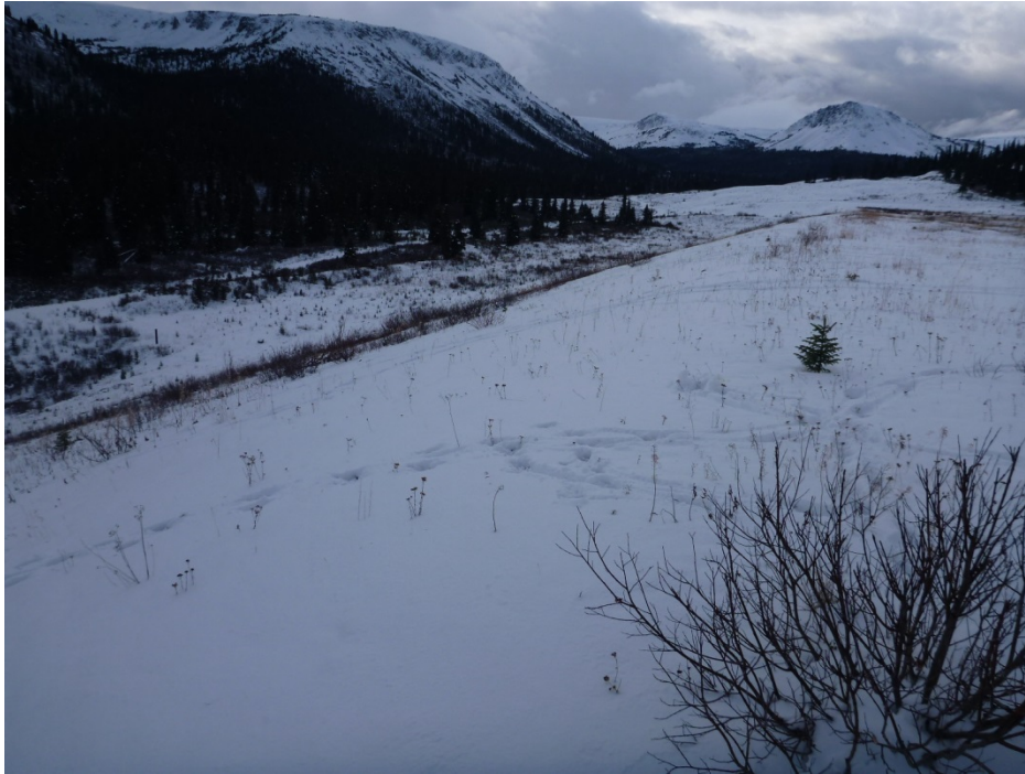
Photo 13 – Crest and downstream slope of south limb of TSF dam viewed from apex with north limb. Photo taken facing southwest.
