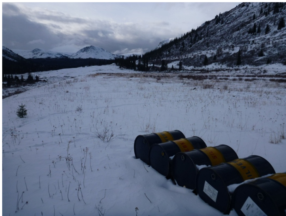
Photo 24 – Reclaimed tailings surface with depression in background. Photo taken facing southwest. Note density of vegetation is greater on top of reclaimed tailings surface than on dam slopes and crest. Fuel drums are for helicopter operations in the area.
