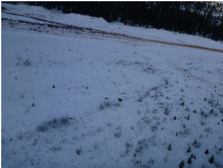
Photo 8 – Downstream slope and crest of north limb of TSF dam. Photo taken facing west from helicopter.
