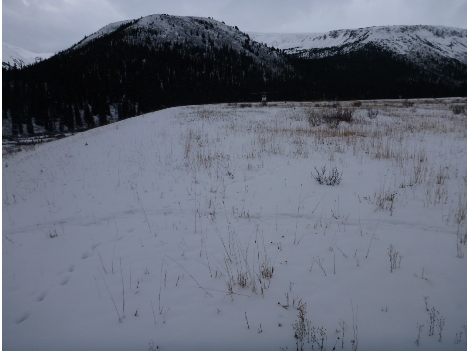
Photo 18 – Crest of north limb of TSF dam. Photo taken facing southeast.
