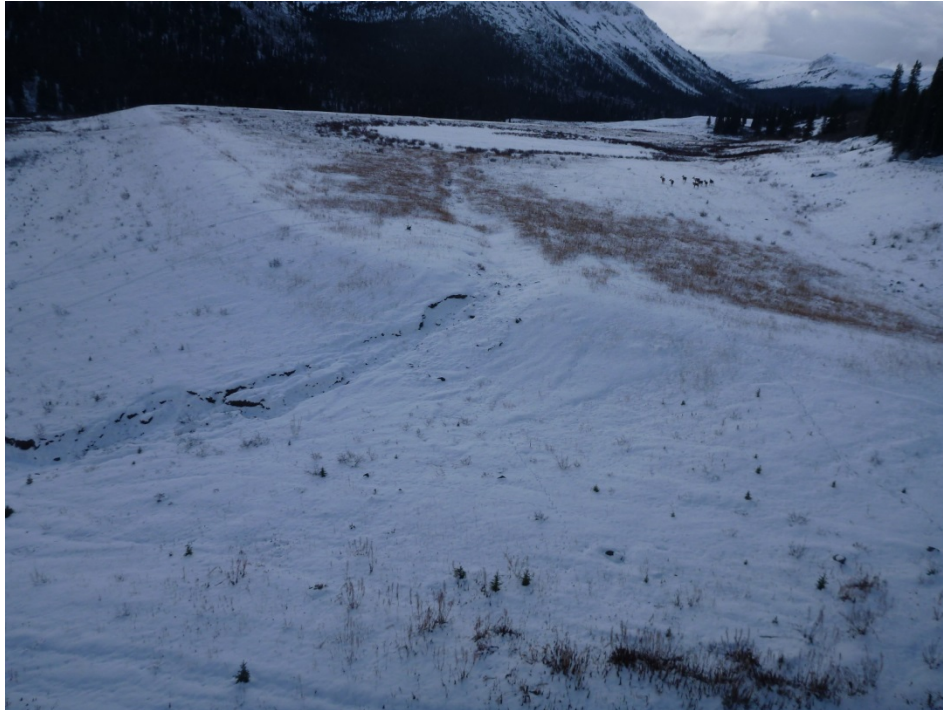
Photo 9 – Erosion at spillway channel extending up downstream slope of TSF dam to crest. Photo taken facing southeast from helicopter. Note caribou foraging on reclaimed tailings surface.
