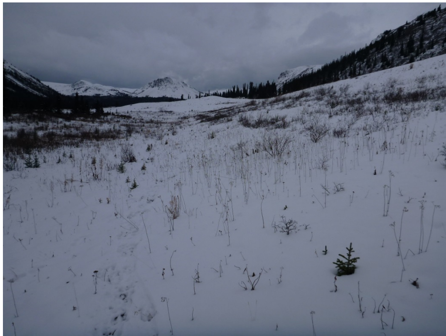
Photo 16 – Downstream slope of south limb of TSF dam. Photo taken facing southwest.
