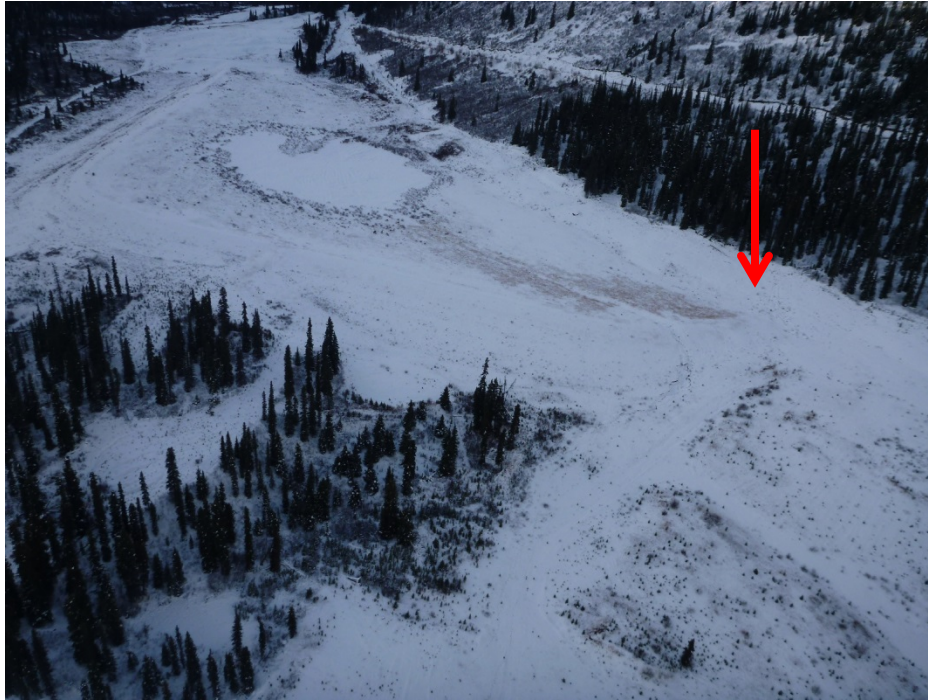
Photo 3 – North limb of TSF dam. Photo taken facing south from helicopter. Red arrow indicates location of spillway and channel.
