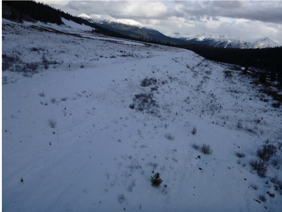
Photo 5 – View of downstream slope and crest of south limb of TSF dam. Photo taken facing northeast from helicopter.
