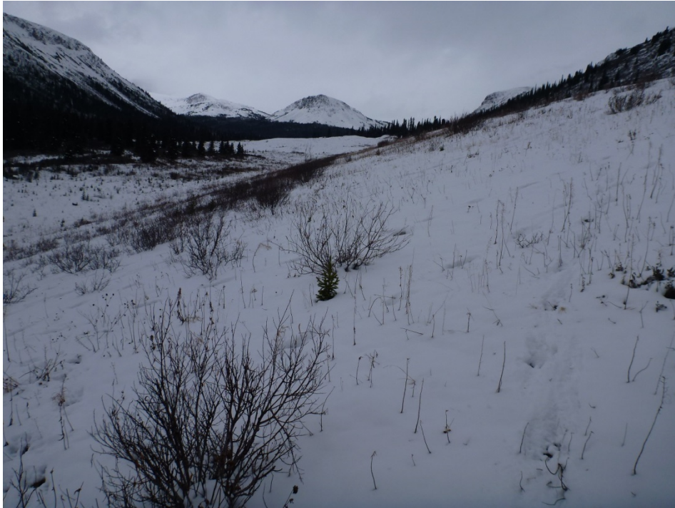
Photo 15 – Downstream slope of south limb of TSF dam. Photo taken facing southwest.
