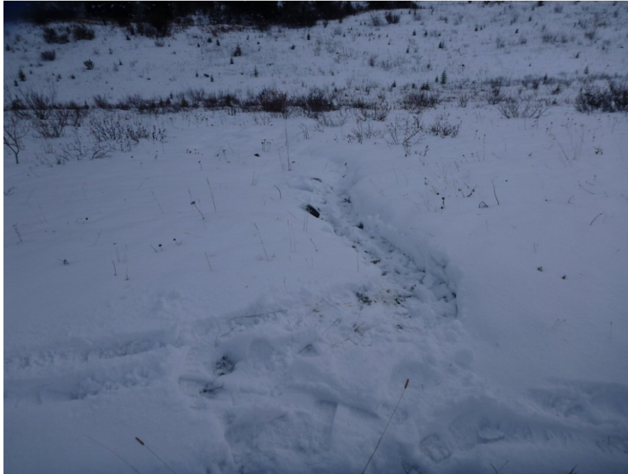
Photo 11 – Downstream slope of south limb of TSF dam near right abutment. Photo taken facing west. One of two erosion rills extending from crest to 1/3 embankment height at this location has been cleared of snow.
