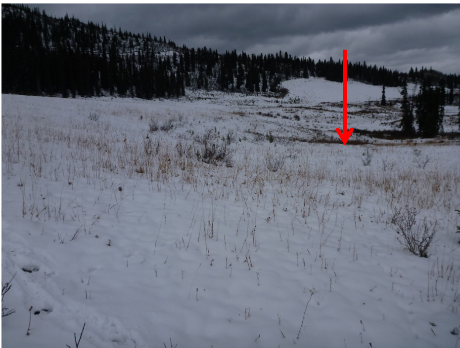
Photo 20 – Downstream slope of north limb of TSF dam. Photo taken facing northwest. Red arrow indicates natural high ground between apex of embankment and left abutment.
