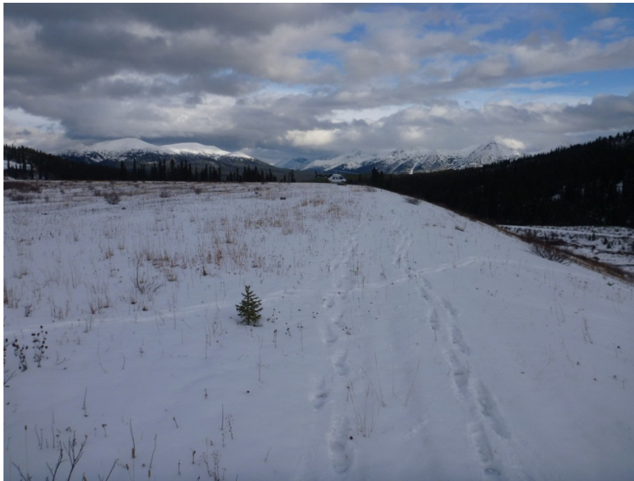
Photo 12 – Crest of south limb of TSF dam at approximate mid-point of limb. Photo taken facing northeast.
