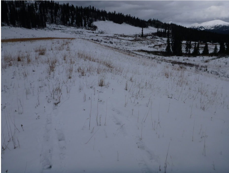
Photo 19 – Crest and downstream slope of north limb of TSF dam. Photo taken facing northwest.
