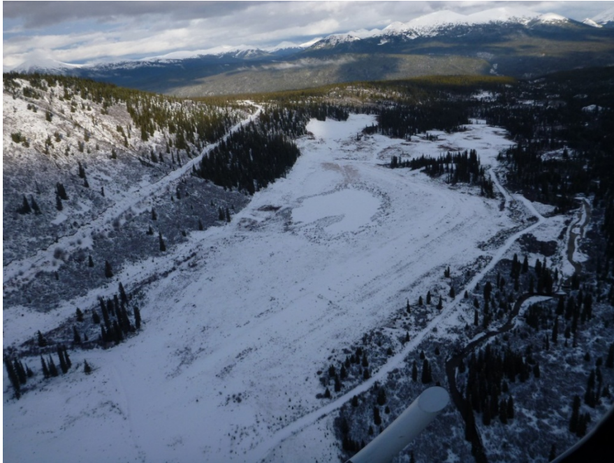
Photo 1 – Aerial oblique view of TSF facing north. Note depression in middle of reclaimed tailings surface.
