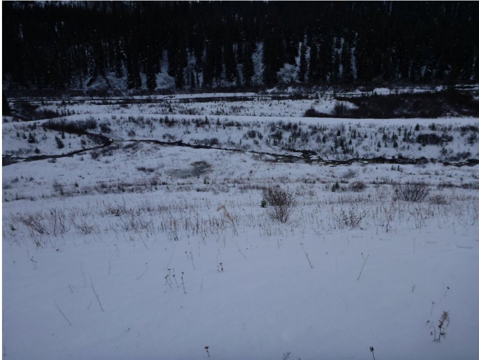
Photo 14 – Downstream slope of TSF dam at apex. Note creek of flowing water beyond toe area. Photo facing east.
