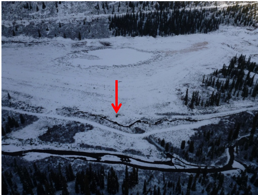
Photo 2 - Aerial oblique view of TSF facing west. Note former location of Lawyers Creek near toe of TSF and road embankment between realigned Lawyers Creek and toe of TSF. Red arrow indicates seepage pond location (Seep-1 identified by Piteau, 1997) beyond downstream toe of dam at apex between limbs.
