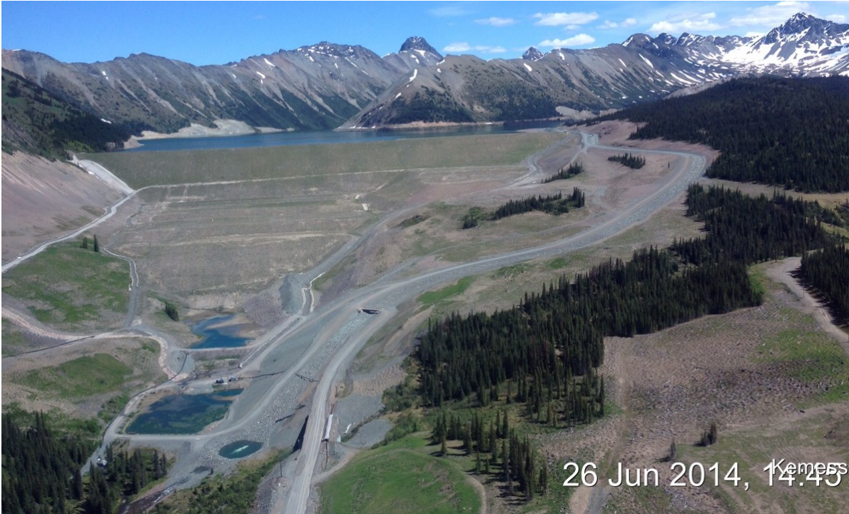
Photo: Main Dam of TSF Viewed toward the East. Completed spillway on RHS
