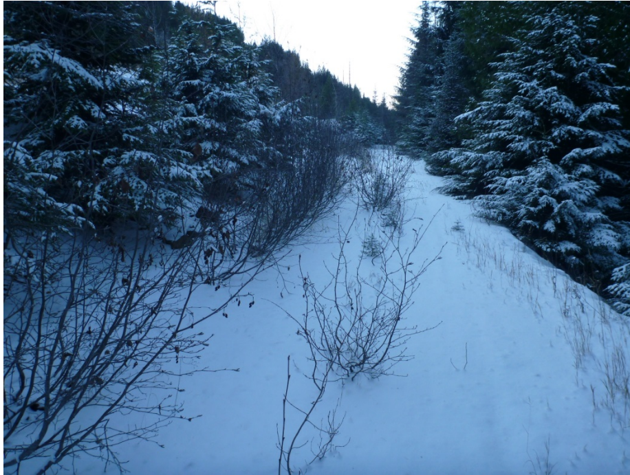
Photo 3 – Good Friday, West Limb of dam, downstream toe area. Photo taken facing south approximately 20 m past barricade entrance to toe access road. Natural slope downstream of dam, to left in photo) is heavily treed.
