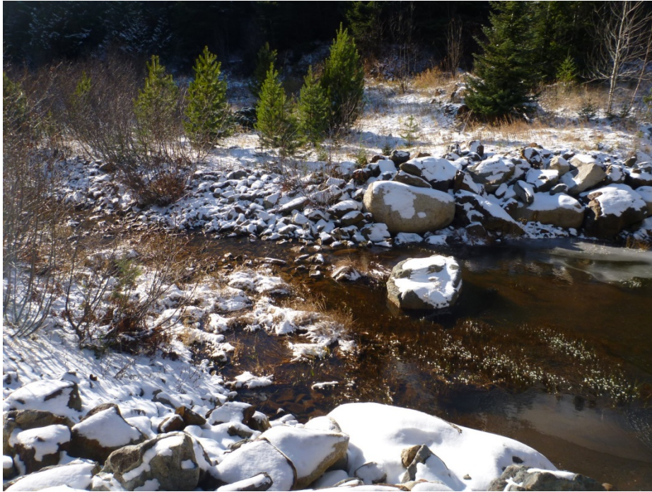
Photo 47 – Jumbo stilling basin outlet and discharge channel. Photo taken facing west. Rip rap is only visible at bottom of stilling basin near outlet.
