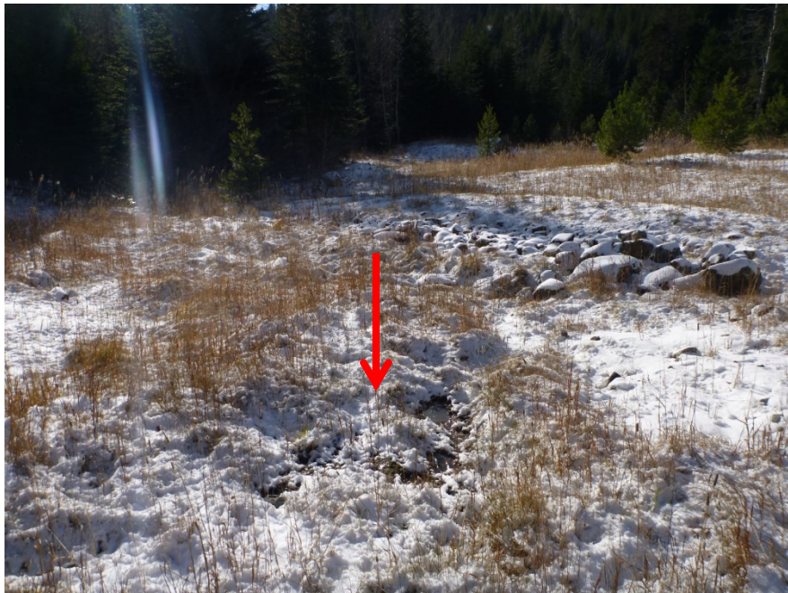
Photo 28 – Good Friday borrow area downstream of South Limb of Good Friday TSF. Photo taken facing south towards confluence of seepage area with flows from spillway. Red arrow indicates seepage flowing over ground surface towards rip rap lined seepage collection channel.
