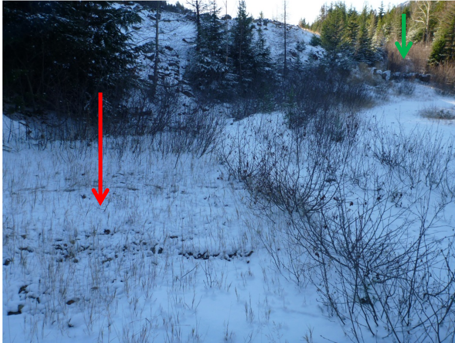
Photo 1 – Good Friday, right abutment area of West Limb dam. Photo taken facing south. Red arrow indicates seepage area melting thin cover of snow that fell the night before the inspection. Green arrow indicates boulder barricade of toe access road.
