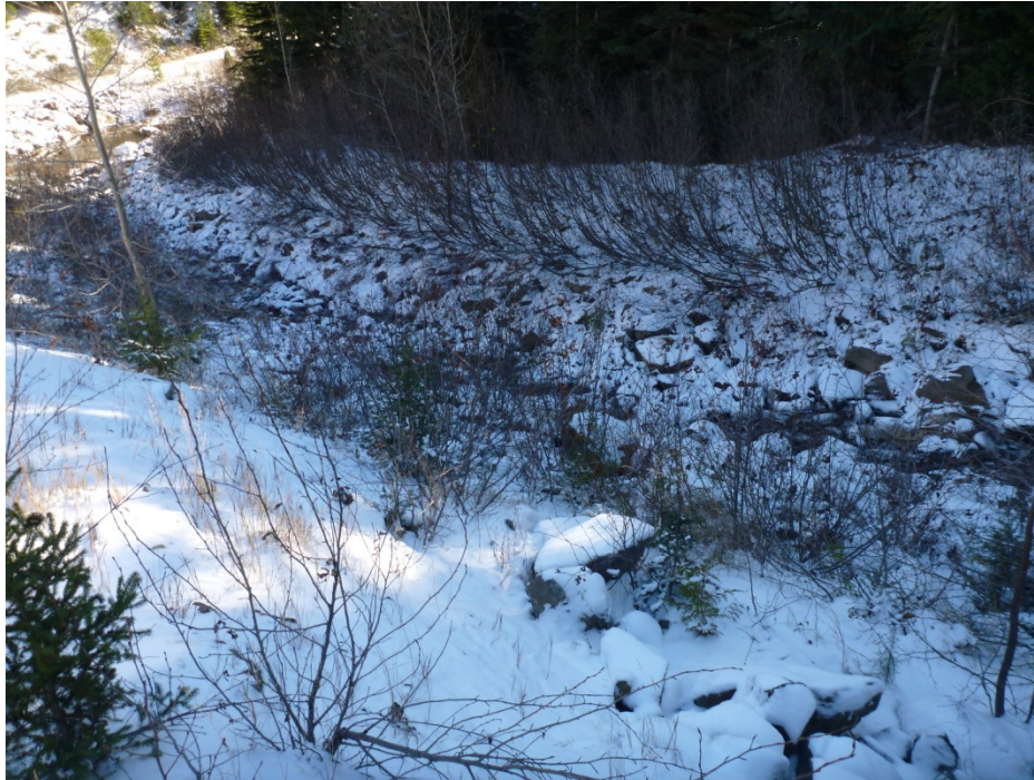
Photo 53 – Jumbo spillway channel approximately 20 m upstream of stilling basin. Photo taken facing south east. Note alders/willows growing on and near channel slopes.
