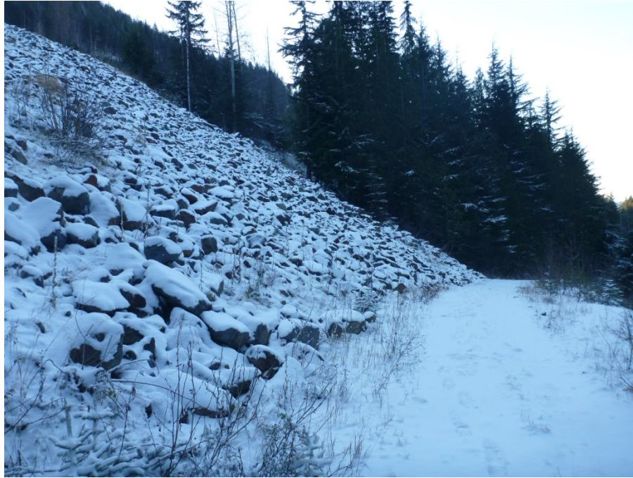
Photo 7 – Good Friday, downstream toe area. Photo taken facing south along access road from Hwy 3B of rockfill stabilized natural slope below South Limb of dam.
