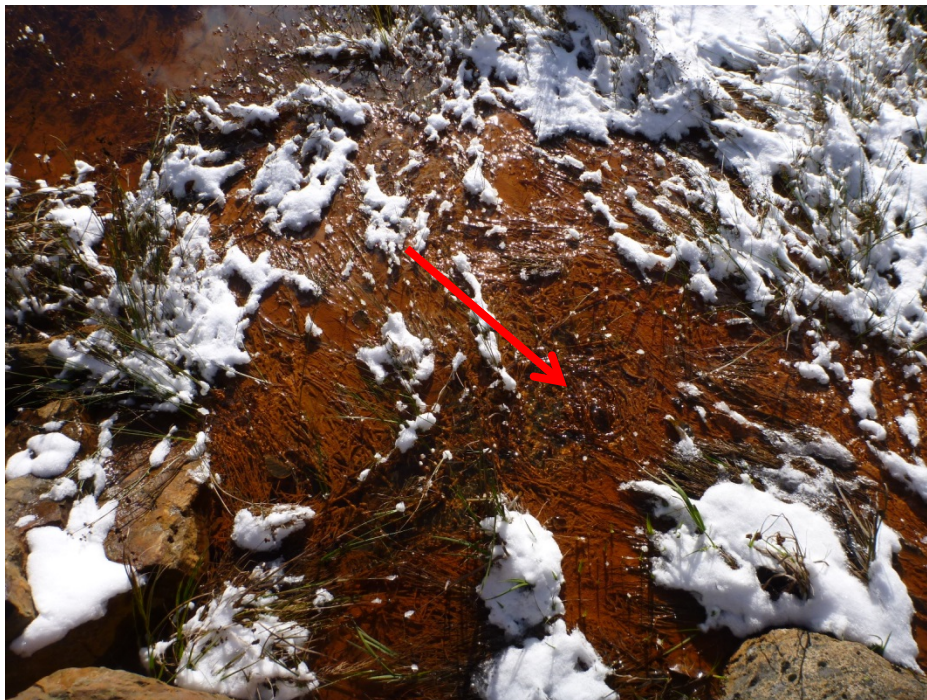
Photo 46 - Jumbo Spillway stilling basin. Seepage is entering stilling basin from the bottom and depositing red silt (believed to be tailings) over vegetation that is growing on surface of silt. Red arrow indicates one seepage discharge point. Seepage is clear.
