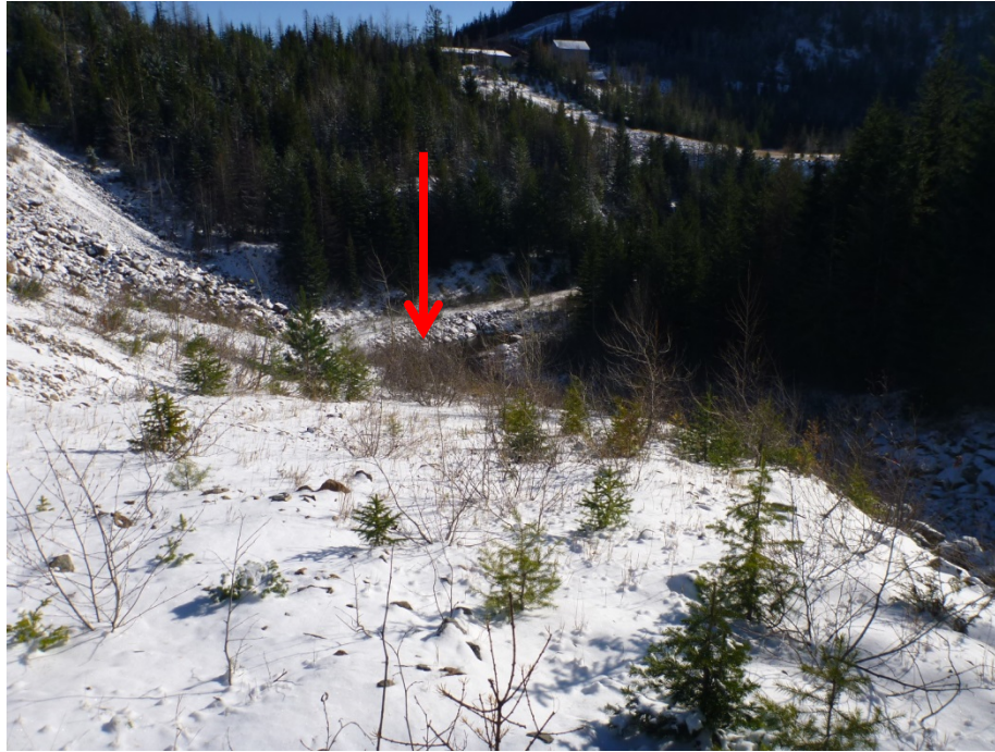
Photo 37 – Jumbo Dam, downstream slope and right abutment. Photo taken facing south east. Spillway is located at right abutment and along downstream toe of dam. Red arrow indicates general location of spillway stilling basin.
