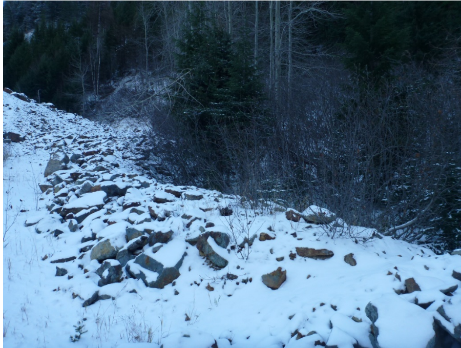
Photo 21 – Good Friday spillway at left abutment of dam. Photo taken facing north. Note trees growing in spillway channel and rockfill training berms to guide spillway discharge in channel.
