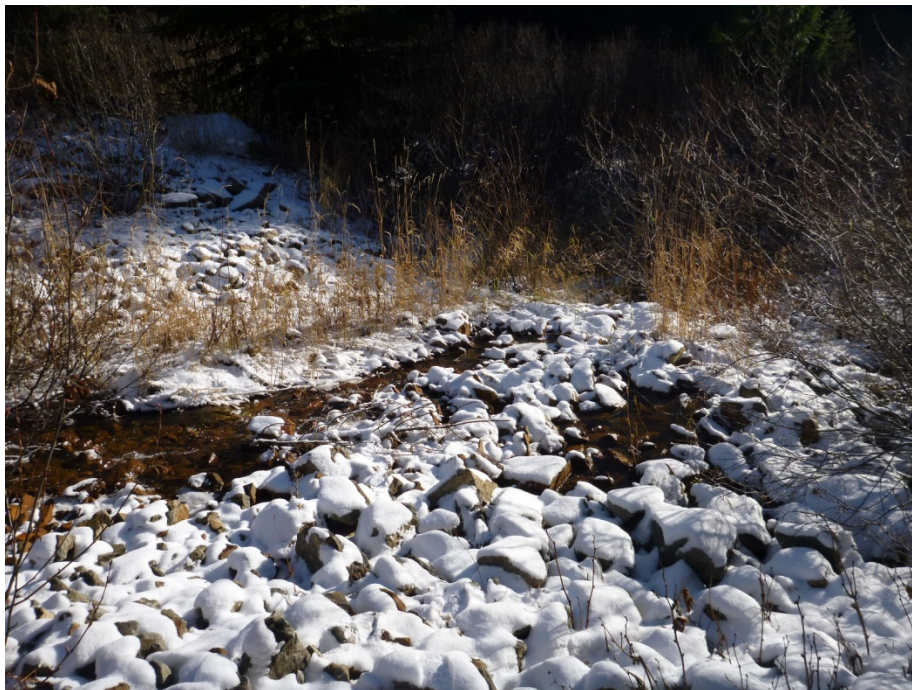
Photo 54 – Jumbo discharge channel sediment berm. Photo taken facing south downstream of stilling basin. The rip rap berm is not clearly defined and rip rap appears to have been dislodged with a channel being eroded through the berm.
