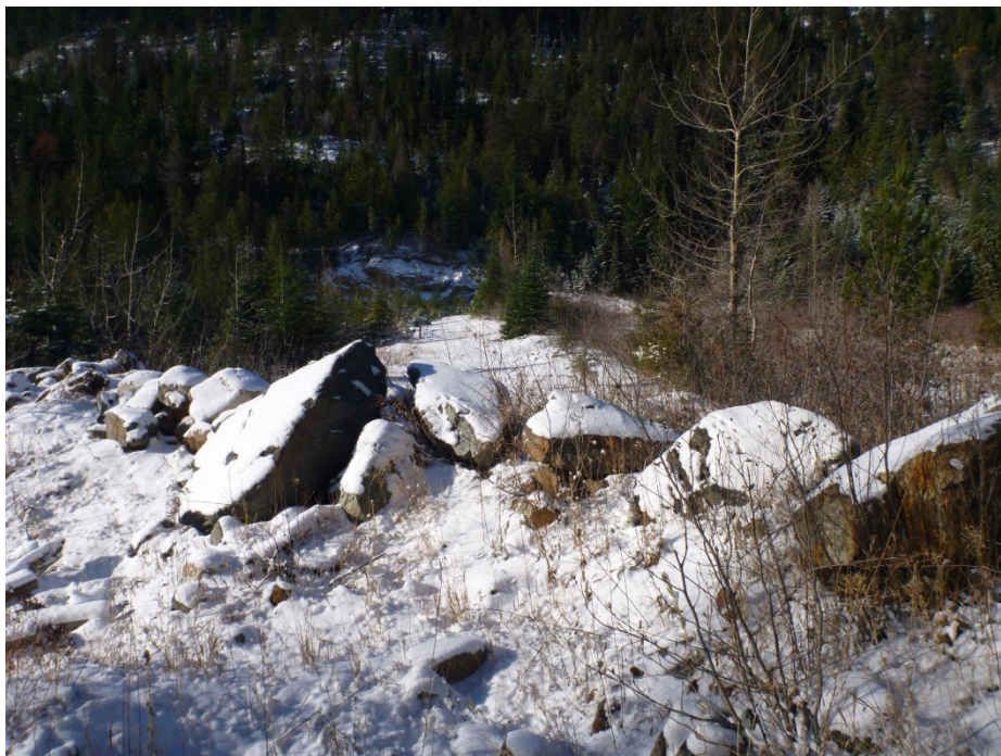
Photo 34 – Jumbo Dam crest. Photo taken from left abutment at access road. Note boulder barricade preventing vehicle access to dam crest or reclaimed tailings impoundment surface.
