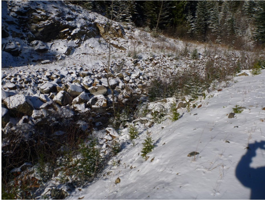
Photo 51 - Jumbo drainage channel entering spillway. Photo taken facing north west at crest of dam near right abutment. Note shrubs and alders/willows growing on channel slopes.
