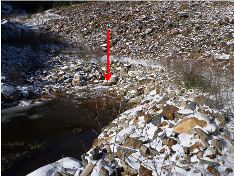
Photo 44 – Jumbo Spillway stilling basin. Photo taken facing north west. Red arrow indicates location of seepage and associated deposit of red silt with trace to some fine sand (believed to be tailings).
