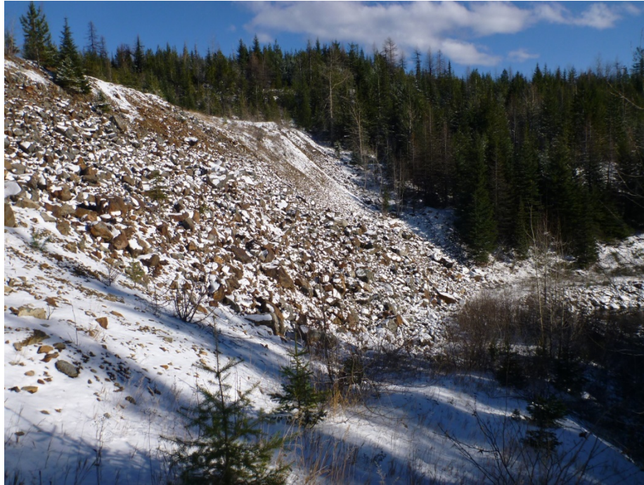
Photo 41 – Jumbo Dam downstream slope. Photo taken from access route located at downstream toe of dam at right abutment. Note uneven surface of dam fill on slope face which appears to be due to original grading of dam during initial construction.
