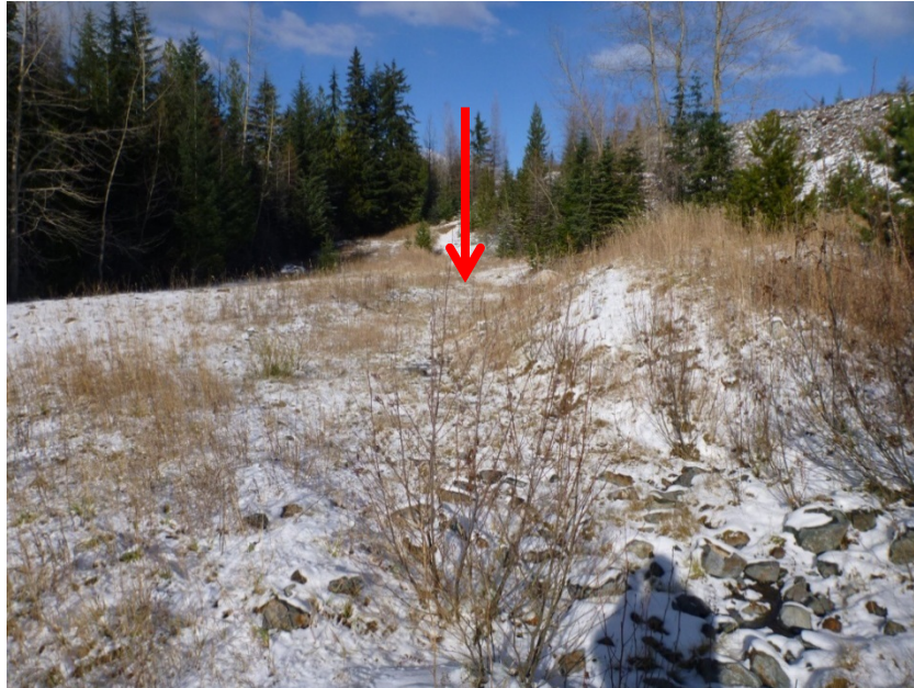
Photo 27 – Good Friday drainage swale from South Limb of dam. Photo taken facing north. A drainage swale with an earthen berm has been constructed to direct seepage from the dam toe through the borrow area. Red arrow shows where seepage was noted at the base of the swale 10 m beyond the downstream toe of the dam.
