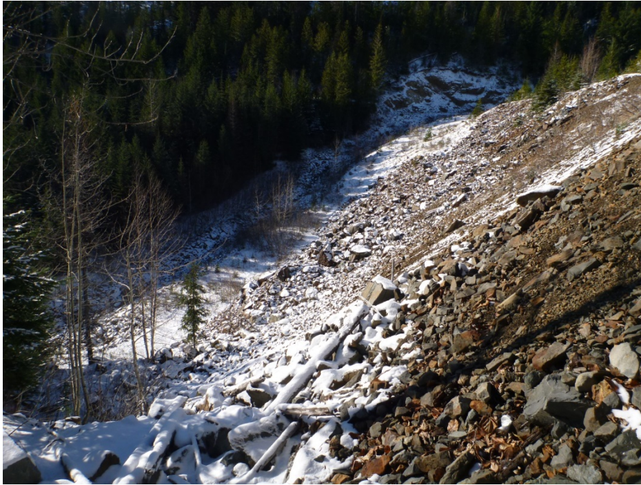
Photo 43 – Jumbo Dam downstream slope. Photo taken facing west from upper left abutment. Note uneven slope surface which is believed to be from original construction of dam.
