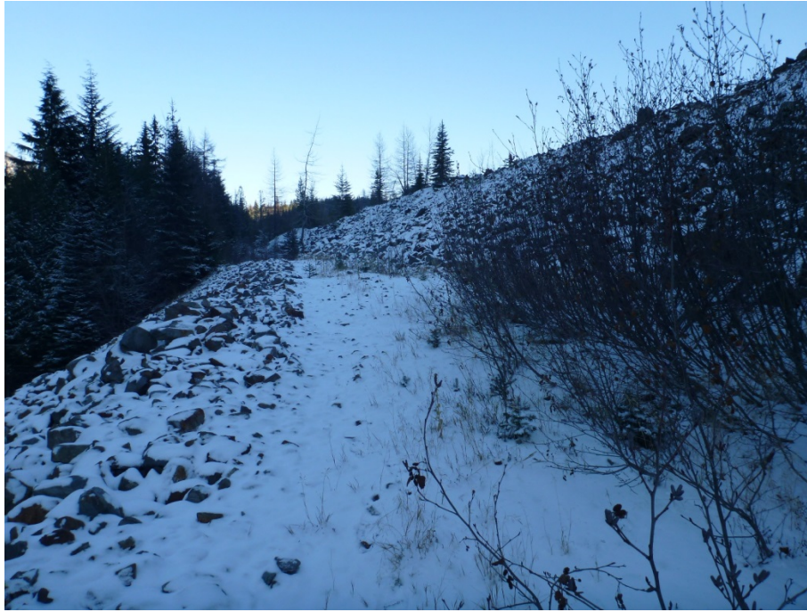
Photo 5 – Good Friday, downstream toe area. Rockfill buttress repair of natural slope instability exacerbated by an overtopping event prior to reclamation of tailings facilities. Downstream slope of South Limb of dam located to right of photograph.
