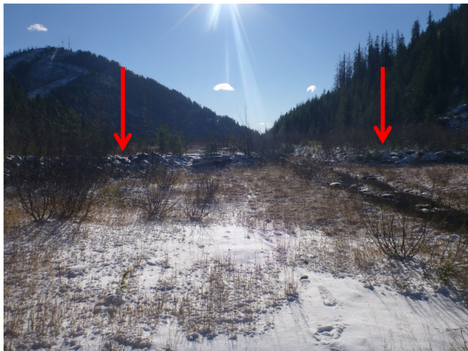
Photo 48 – Jumbo tailings impoundment near start of diversion channel over reclaimed tailings surface. Photo taken from start of tailings surface, facing south. Note guide berms to direct creek flow into drainage channel.
