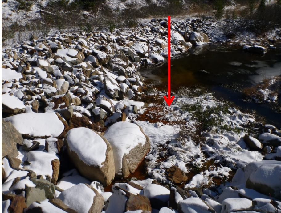
Photo 45 - Jumbo Spillway stilling basin. Photo taken facing south east. Red arrow indicates location of seepage and associated deposit of red silt with some fine sand (believed to be tailings).
