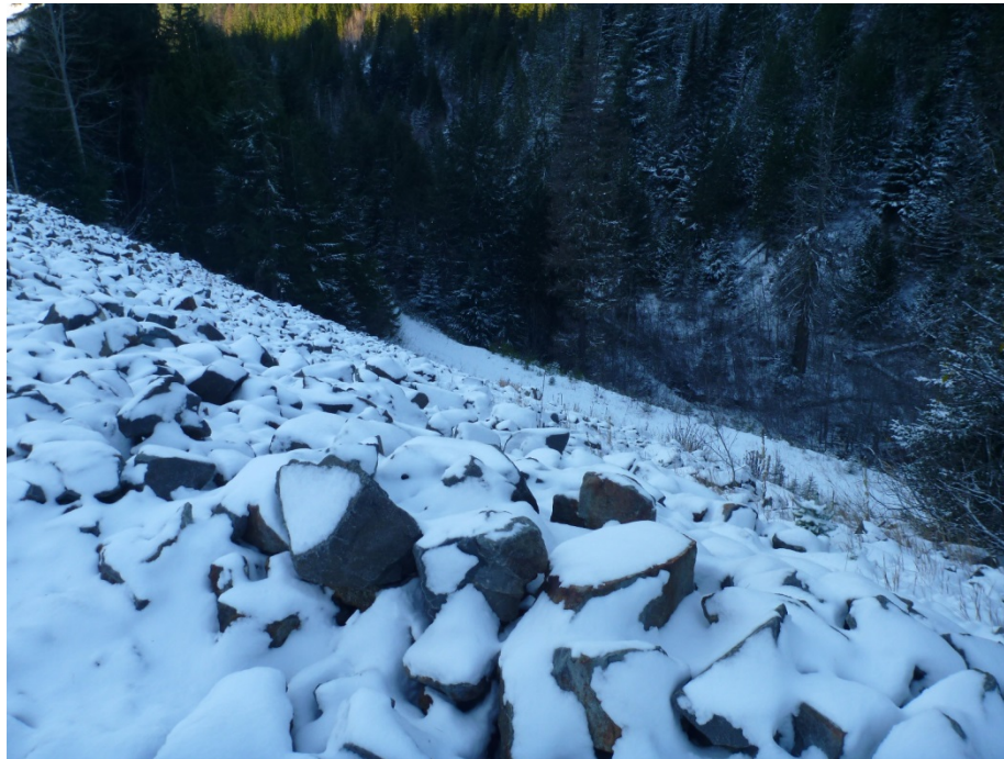
Photo 6 – Good Friday, downstream toe area. View looking downslope over rockfill buttress repaired natural slope above main access road from Hwy 3B. Photo taken facing south east.
