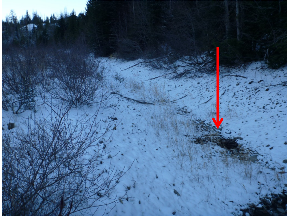
Photo 17 – Good Friday drainage channel. Photo taken facing north from approximate mid-point of channel length. Red arrow indicates surficial water flow, believed to be collected seepage from adjacent slope.
