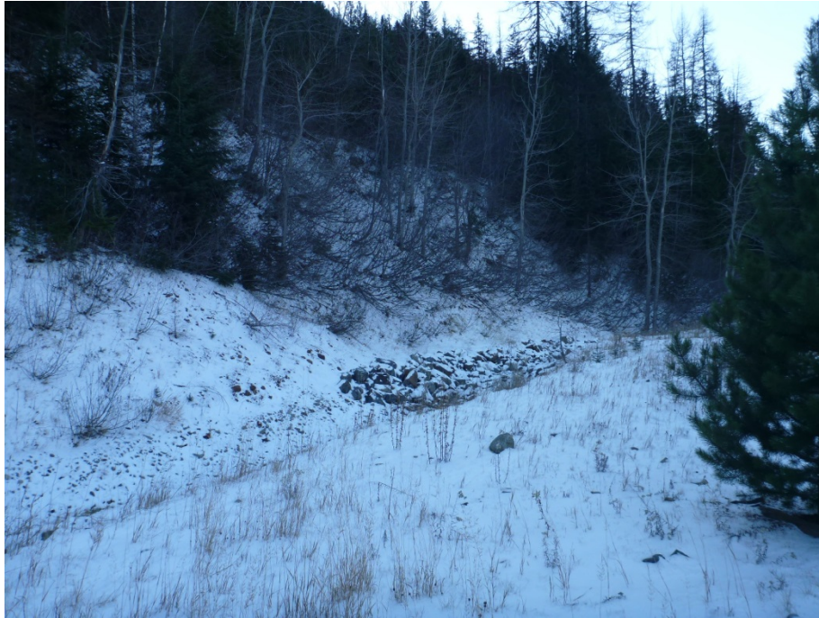
Photo 19 – Good Friday drainage channel and spillway at left abutment. Photo taken facing south east. Transition from drainage channel to spillway is indicated by change in size of channel armouring from gravel and cobbles to rip rap cobbles and boulders.
