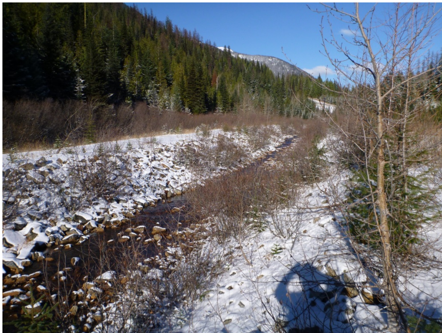
Photo 50 – Jumbo drainage channel on reclaimed tailings surface. Photo taken facing north approximately two thirds of channel length from entrance to channel shown in Photo 47. Note shrubs and alders/willows growing on channel slopes.
