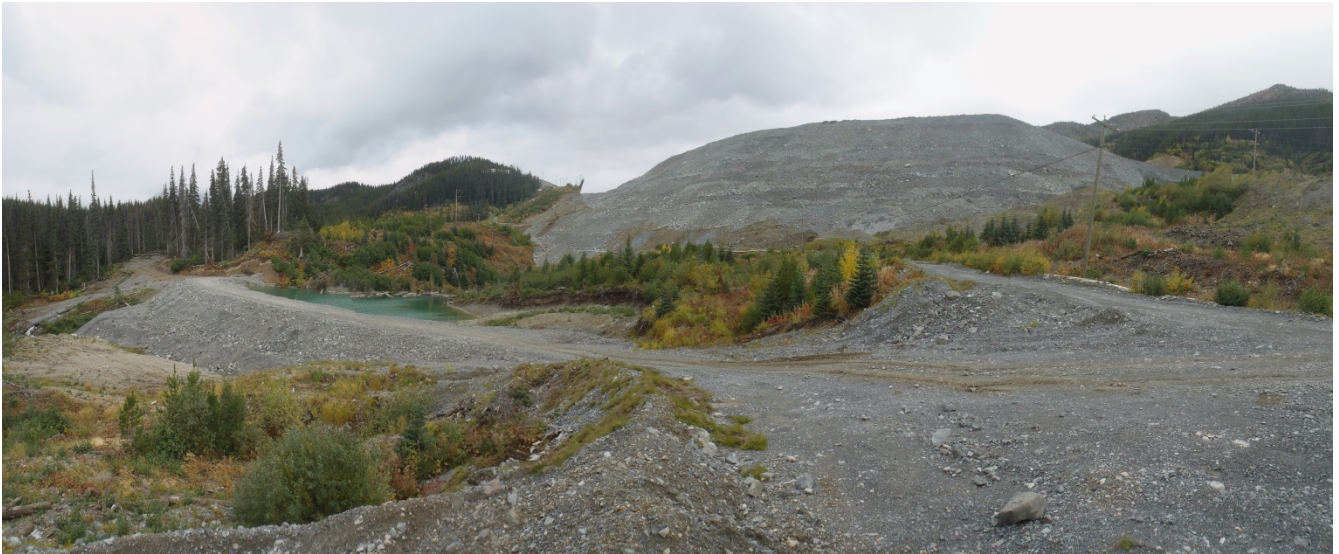
Photograph 7: East Pit Plug Dam Downstream Face and Seepage Collection Pond Looking North
