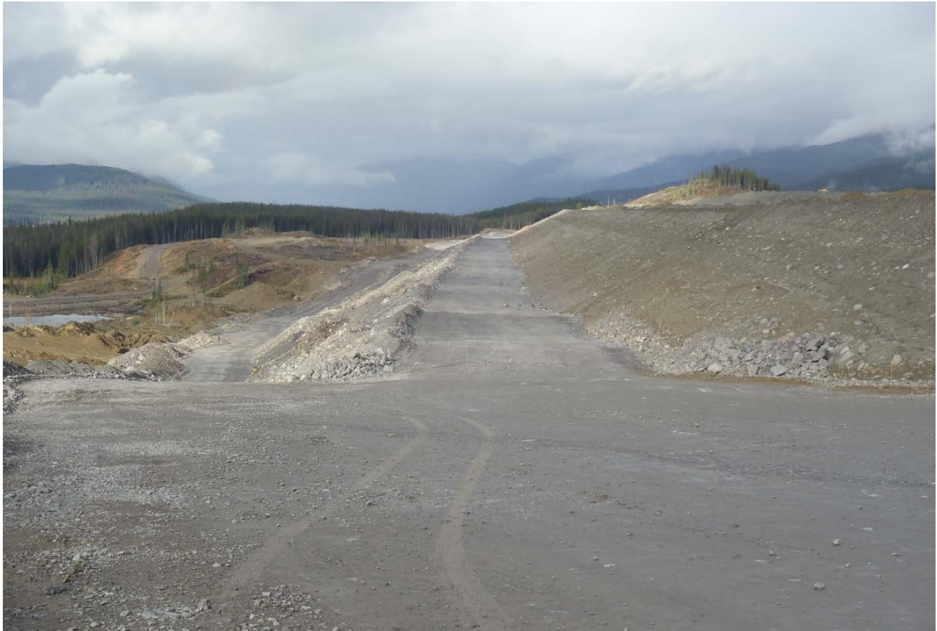
Photograph 14: TMF-3 Downstream Face (looking west)
