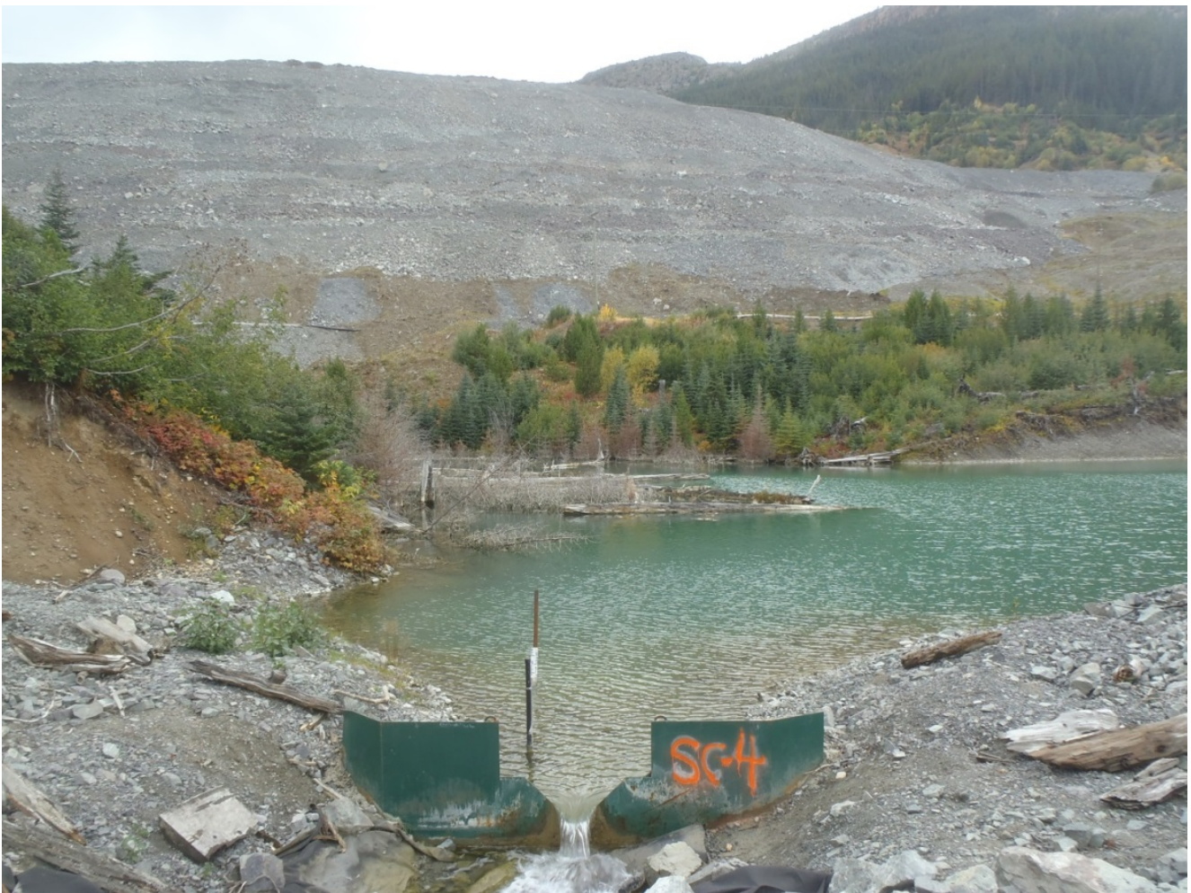
Photograph 8: East Pit Plug Dam Downstream Face (looking north east)
