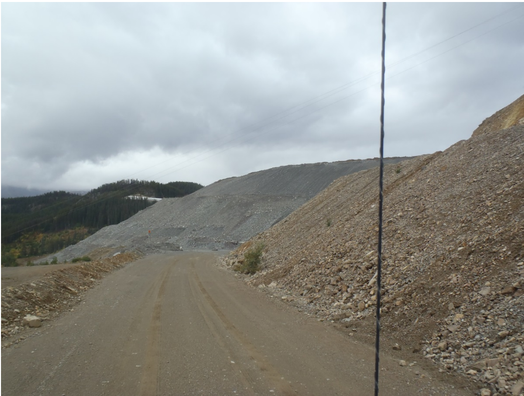
Photograph 6: East Pit Plug Dam Downstream Face (looking north west)
