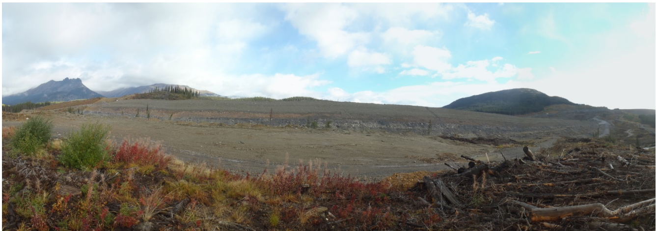
Photograph 15: TMF-3 Downstream Face (looking north)
