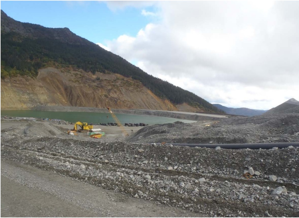
Photograph 5: East Zone Pit Impoundment (looking north-east)
