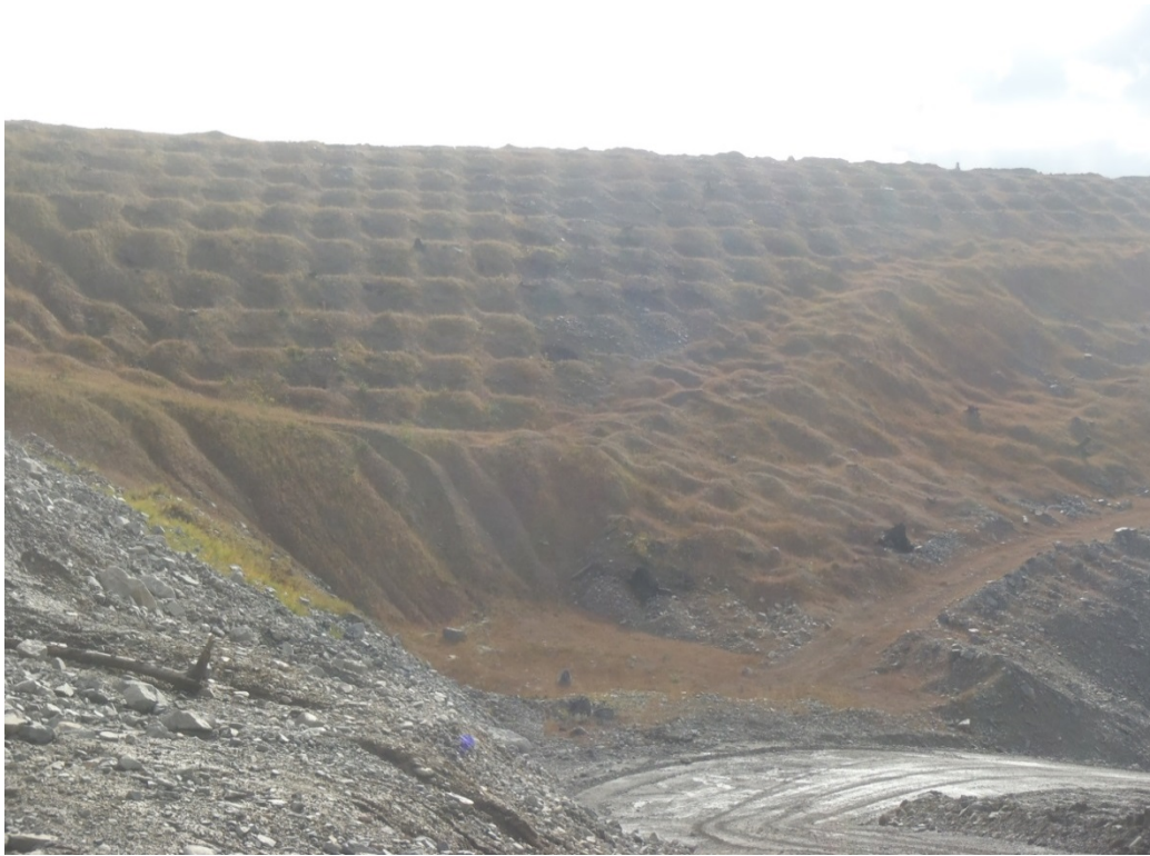
Photograph 3: TMF-2 Dam Downstream Slope Showing Reclamation (looking east)
