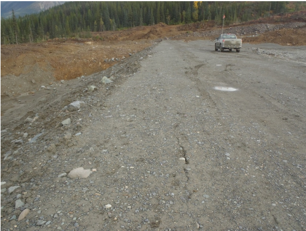
Photograph 17: TMF-3 Saddle Dam Tension Crack at Downstream Crest. The crack is above the pond level and does not present a dam safety concern provided that repairs are performed in advance of the pond level reaching the level of the crack.
