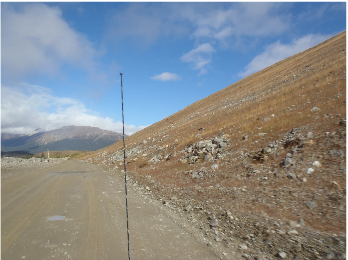
Photograph 2: TMF-2 Dam Downstream Face (looking west)
