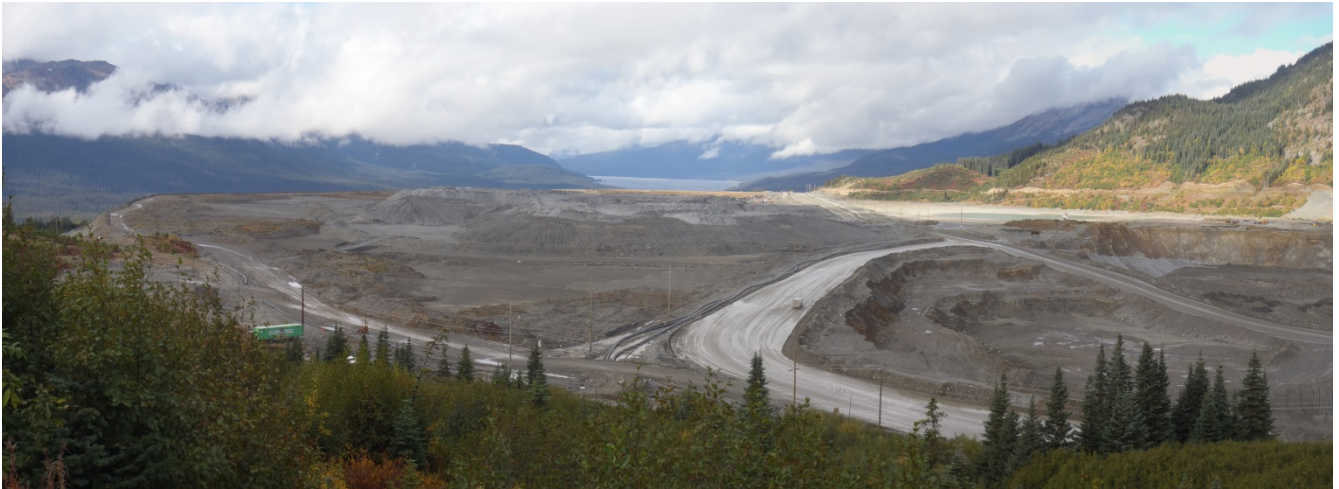
Photograph 1: TMF-2 Impoundment Overview (looking west)
