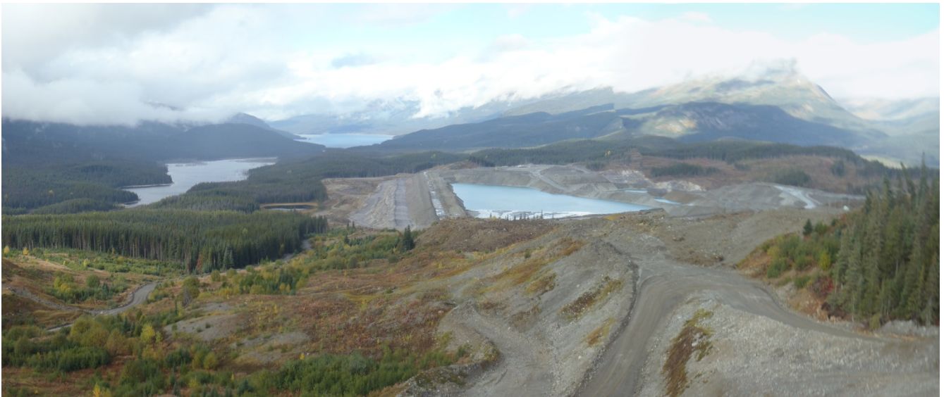
Photograph 12: TMF-3 (looking west)
