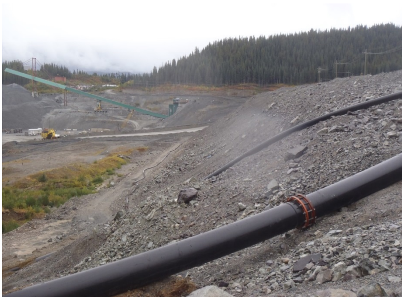
Photograph 11: East Dam Downstream Face (looking south)
