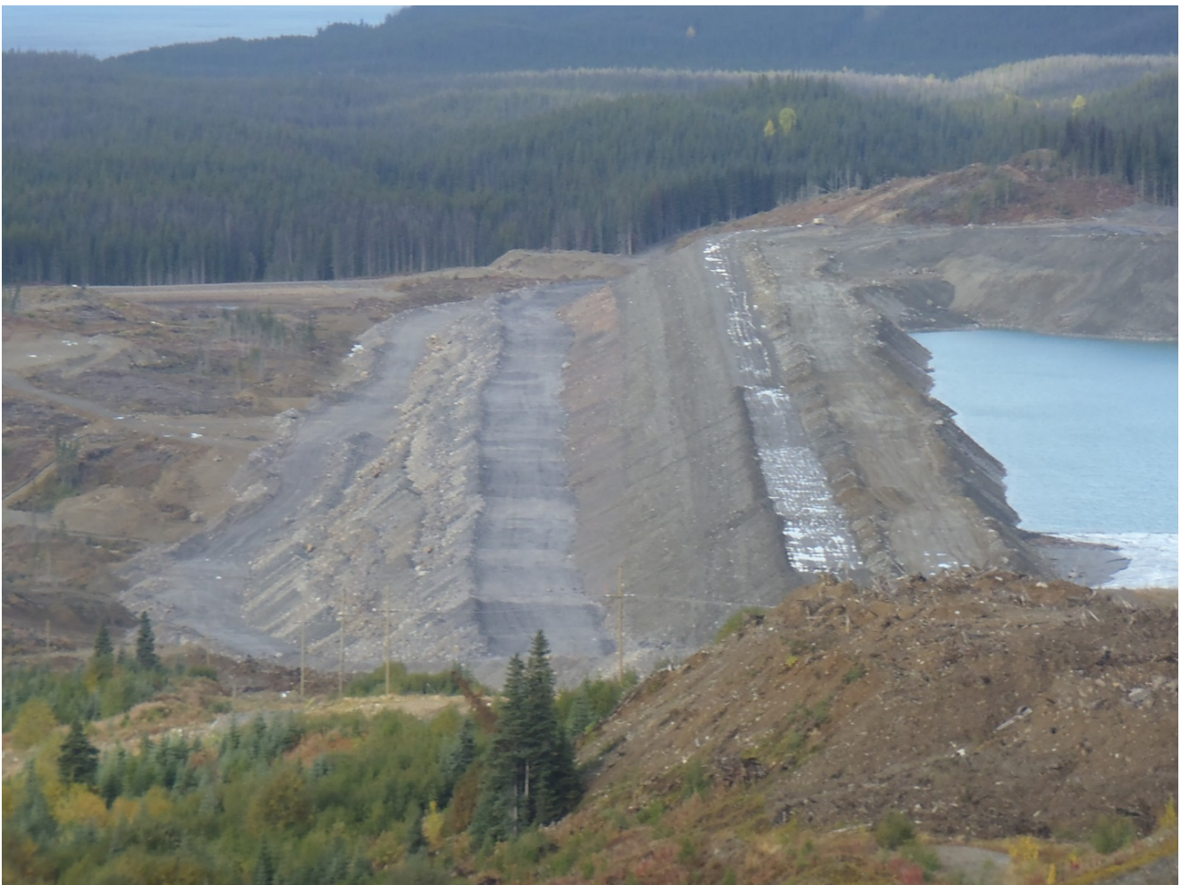
Photograph 13: TMF-3 Dam (looking west)
