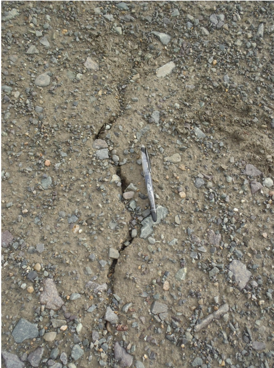
Photograph 18: TMF-3 Saddle Dam Tension Crack at Downstream Crest. The crack is above the pond level and does not present a dam safety concern provided that repairs are performed in advance of the pond level reaching the level of the crack.
