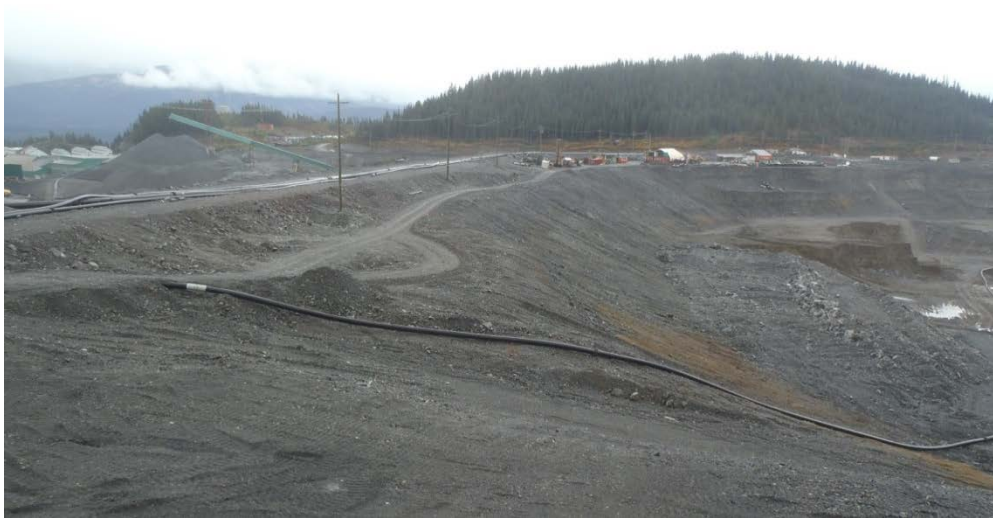
Photograph 10: East Dam Upstream Face (looking south)
