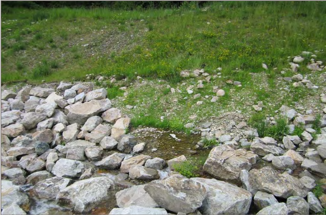
Photo 5: Spillway Channel – noted missing rip-rap protection on the right bank of channel (used for the slough repair)
