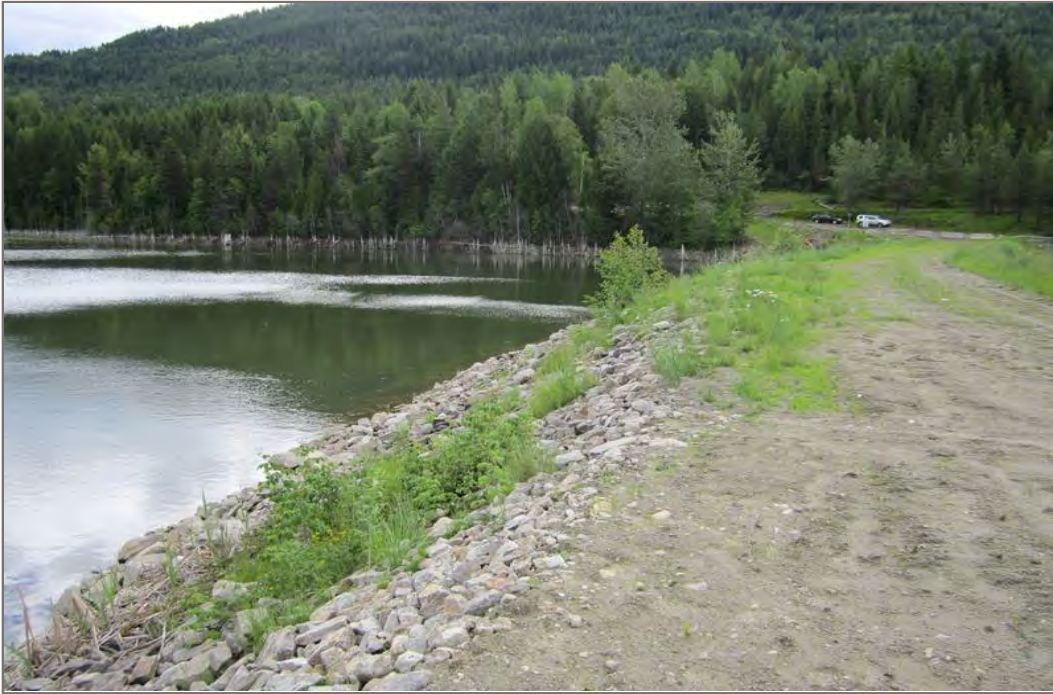
Photo 1: Crest of dam – observed rutting from vehicle traffic and minor animal activity
