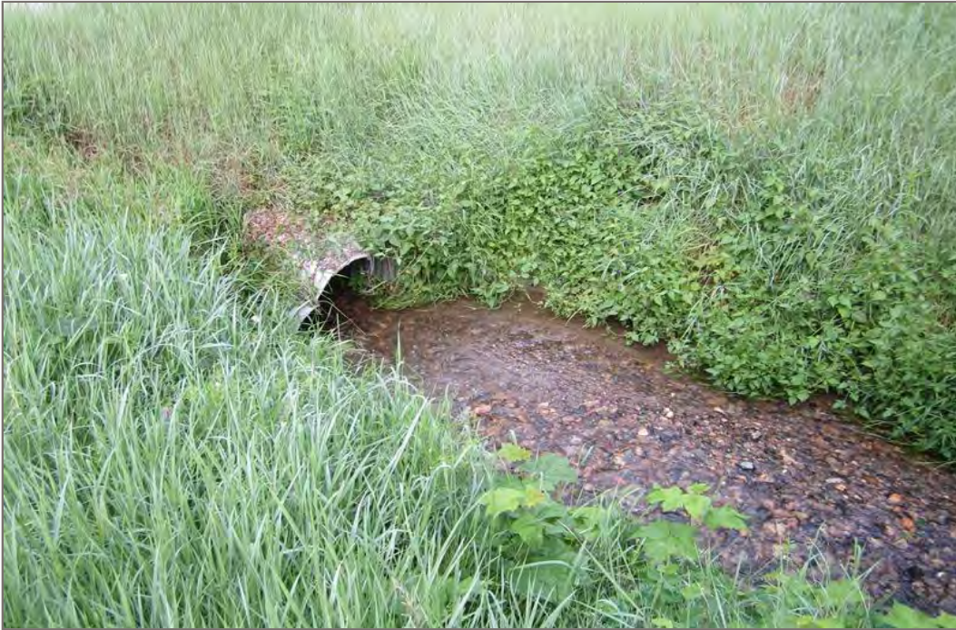
Photo 9: Dam outlet flows downstream under a culvert under Highway 3
