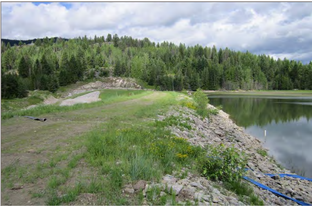
Photo 2: Upstream Face – vegetation/brush/tree growing on the upstream face of the dam
