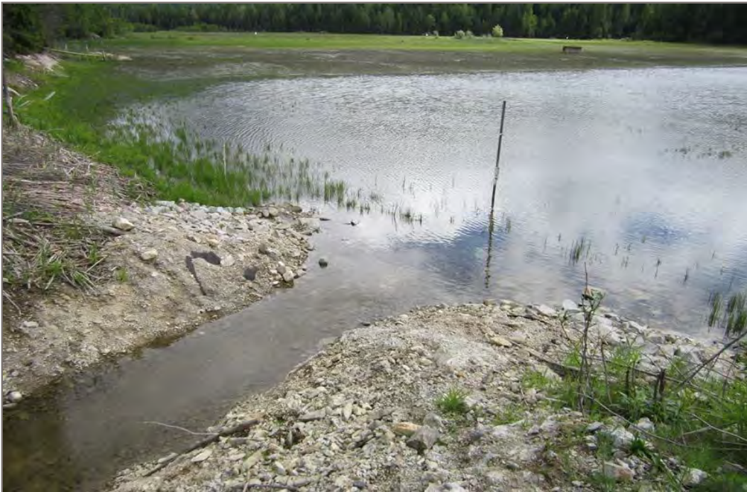
Photo 4: Spillway - bottom width measured to be 1.7 m
