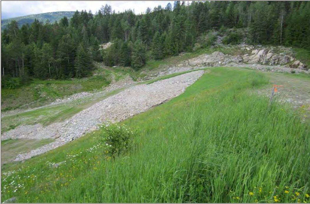
Photo 3: Downstream Face – observed new rock blanket at slough
