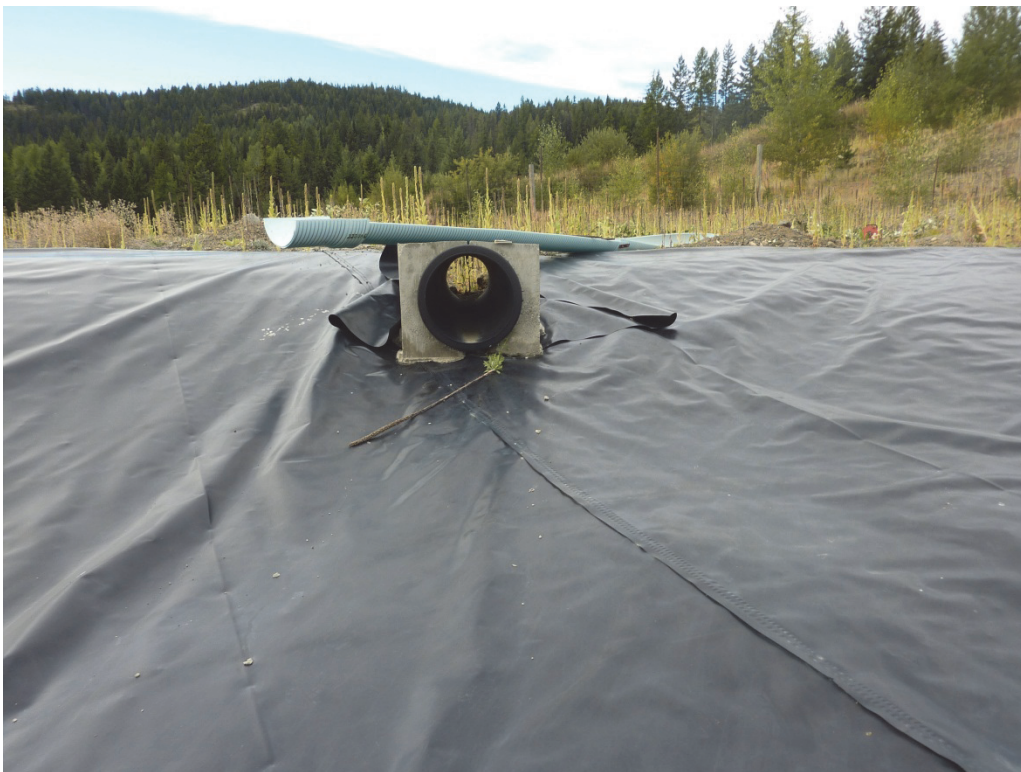
Photo III-6 – Tailings Pond – Surface Water Inlet Culvert at Southwest End of Dam Embankment
