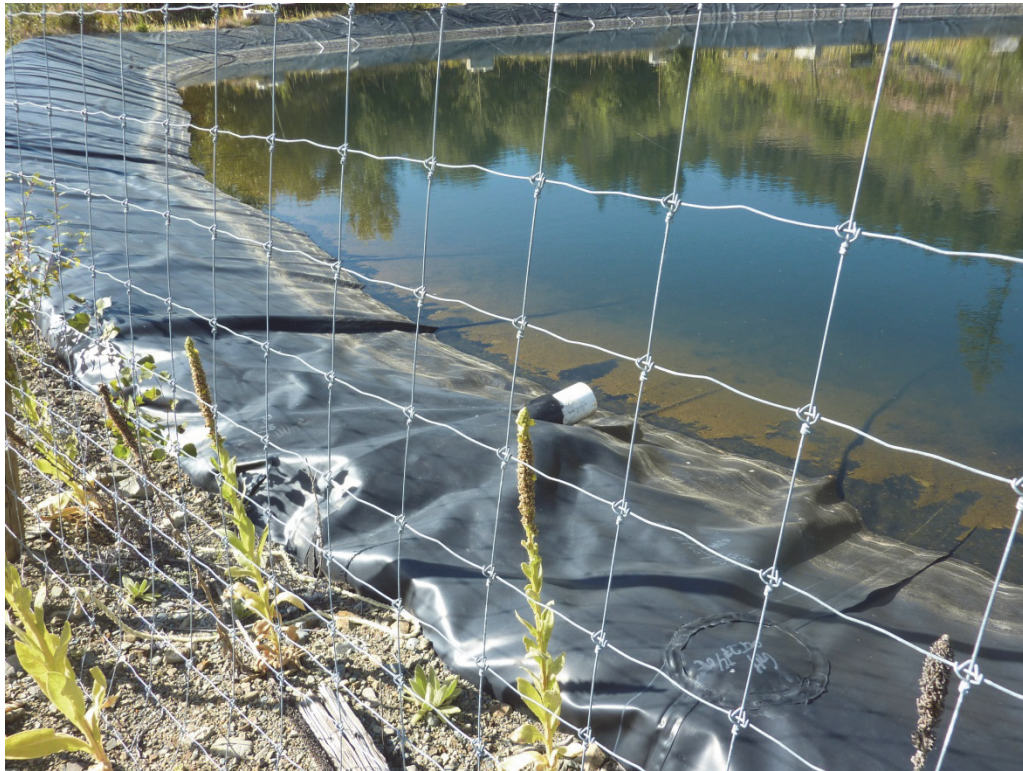
Photo III-3 – Emergency Water Pond - PVC Outlet Pipe
