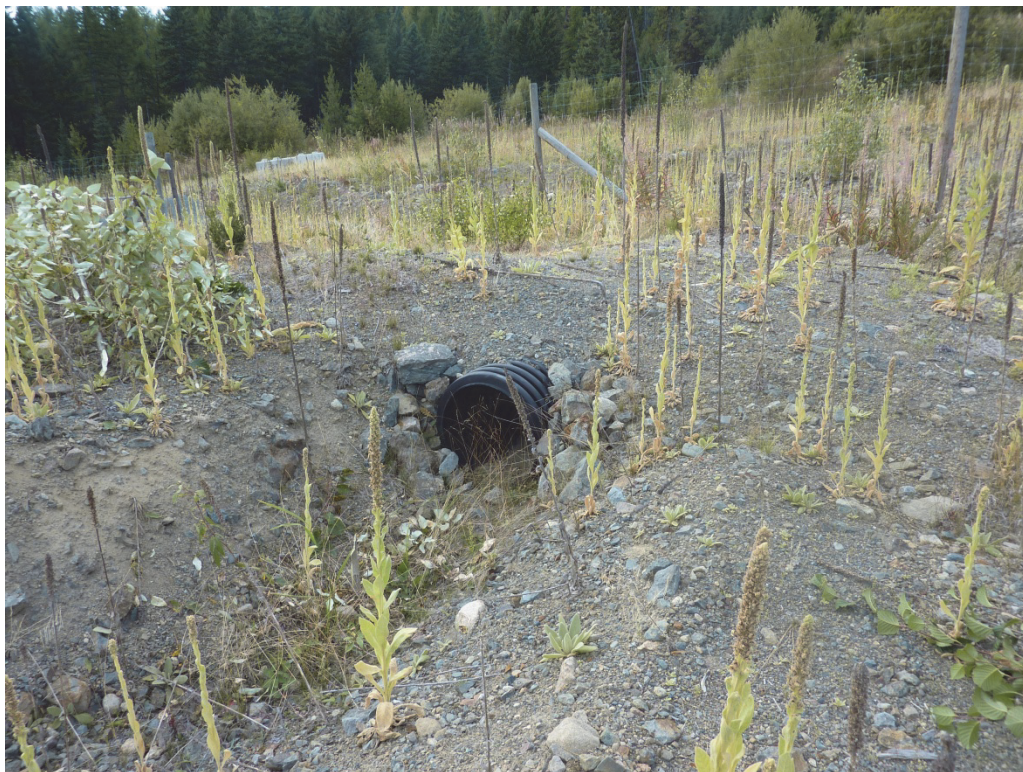
Photo III-8 – Tailings Pond – Bypass Channel and Culvert at Southwest End of Dam Embankment
