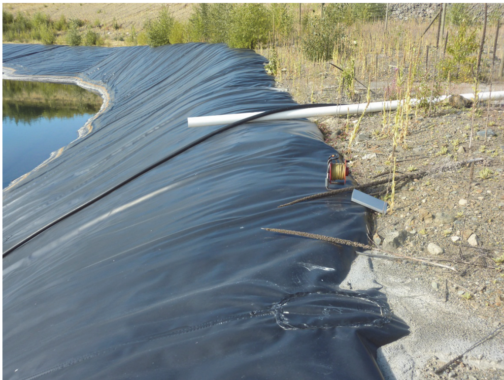
Photo III-4 - Emergency Water Pond - PVC Outlet Pipe Discharge at Tailings Pond
