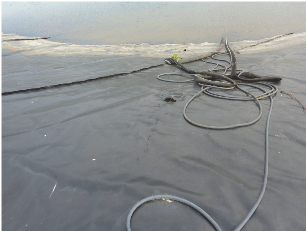
Photo III-12 – Tailings Pond – Small tears in geomembrane at SW corner. Note reclaim pump power cable and discharge hose are still present.
