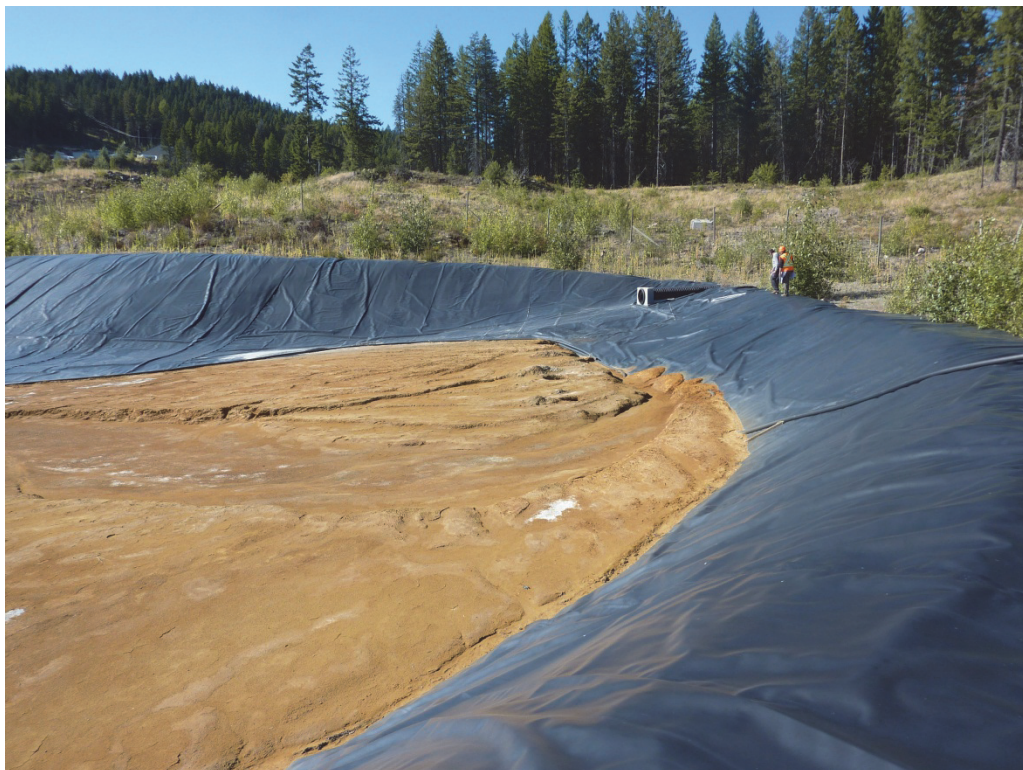
Photo III-16 – Tailings Pond – Tailings Beach Spigot Point in Northeast Corner
