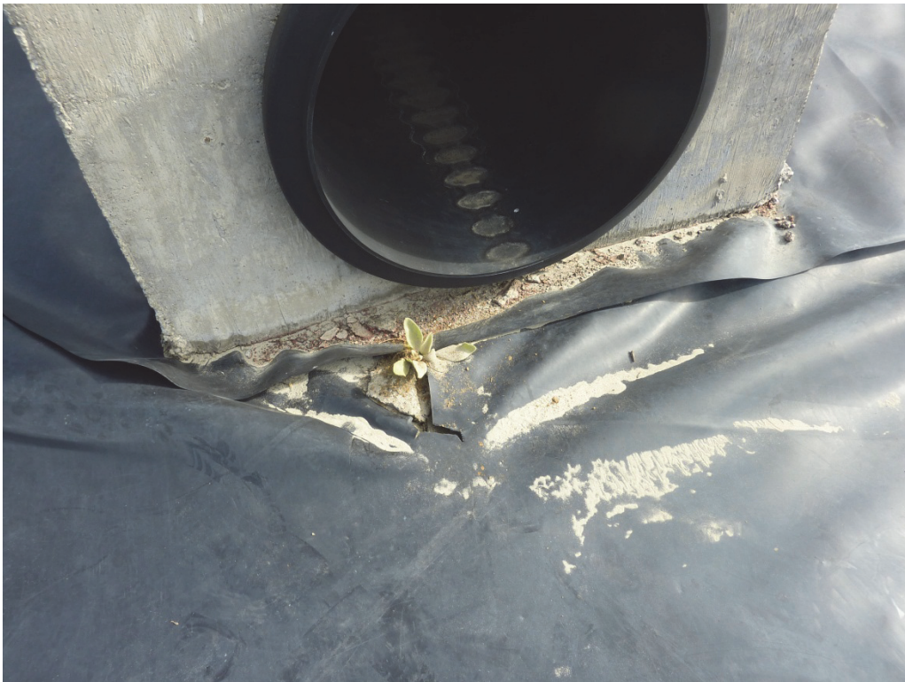
Photo III-14 – Tailings Pond – Tear in geomembrane liner at culvert inlet in northeast corner
