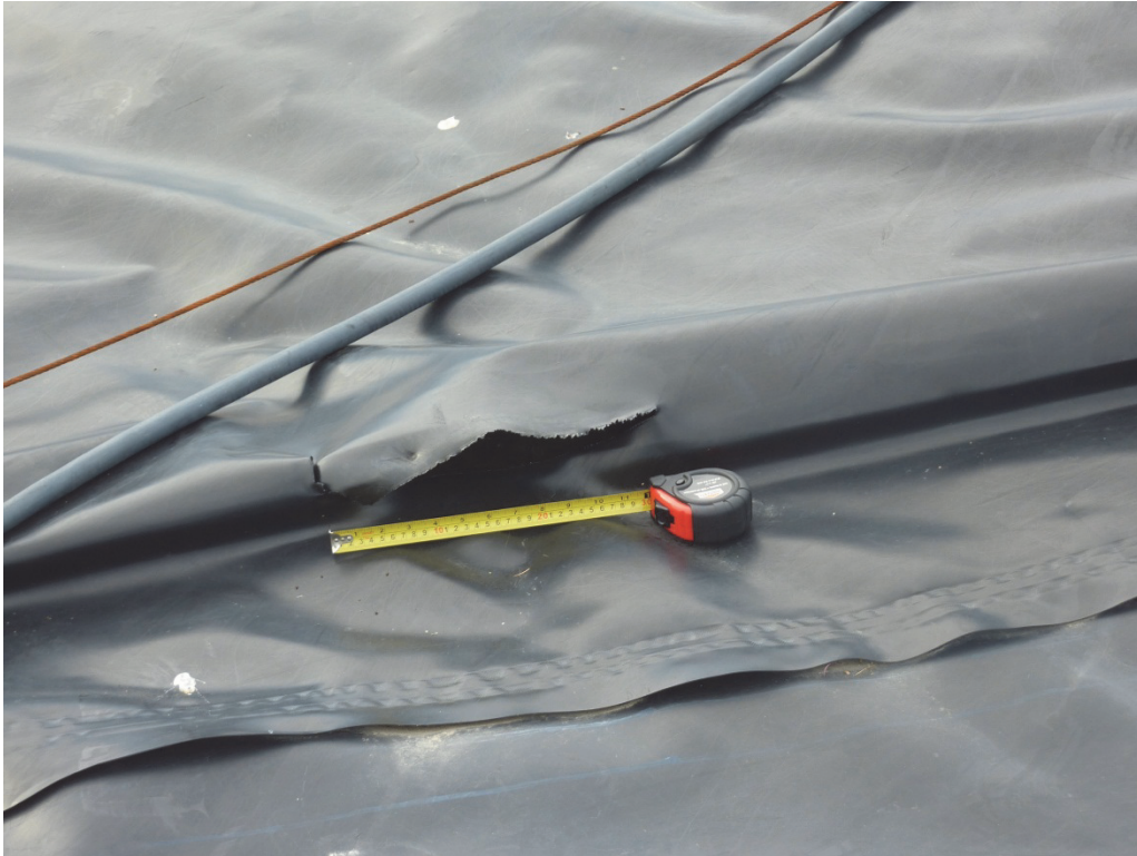
Photo III-13 - Tailings Pond – Close-up of small tear in geomembrane at SW corner.
