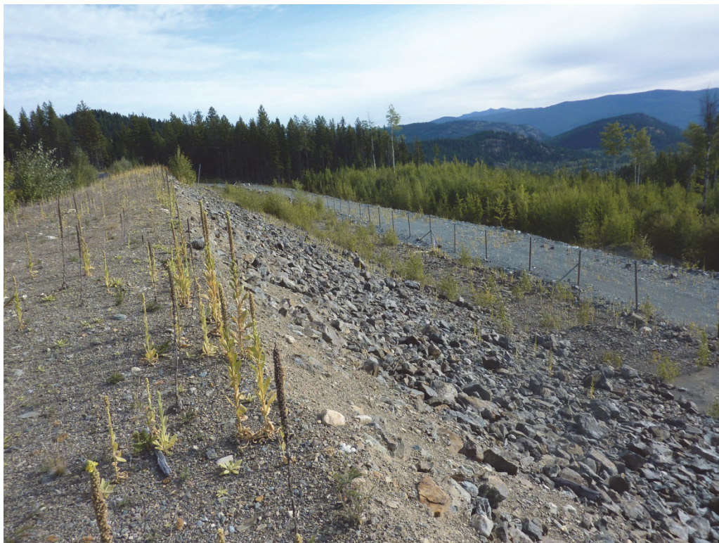
Photo III-10 – Tailings Pond – Dam Crest and Downstream Slope
