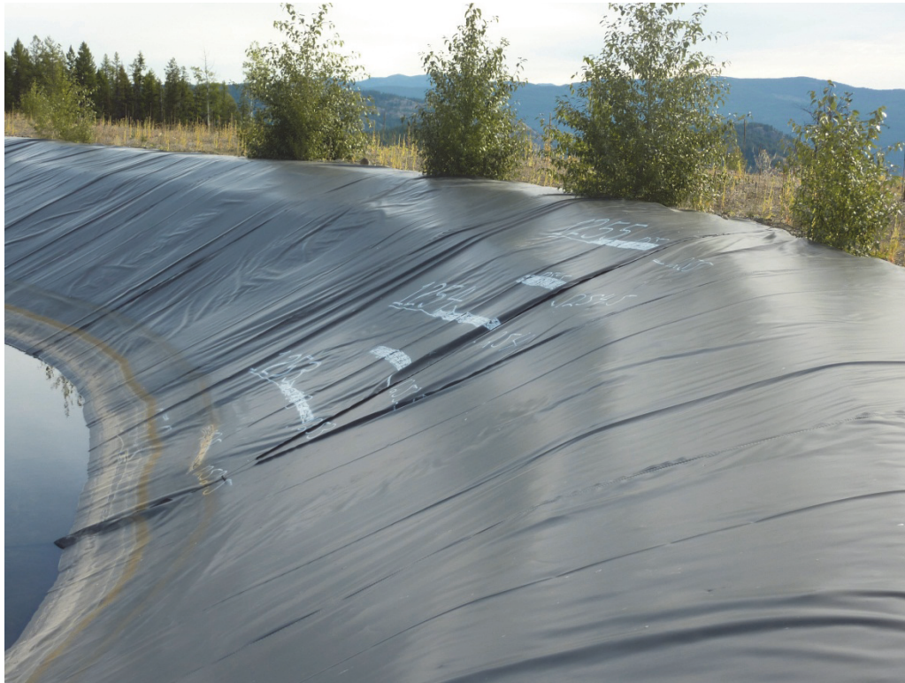
Photo III-15 – Tailings Pond – Reservoir Level Marks Spray Painted on Geomembrane Liner
