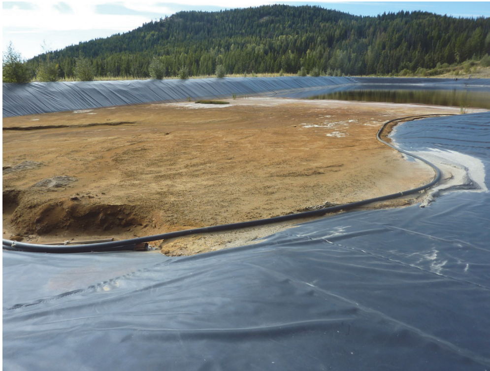
Photo III-11 – Tailings Pond – Geomembrane liner viewed from northeast corner looking southwest.
