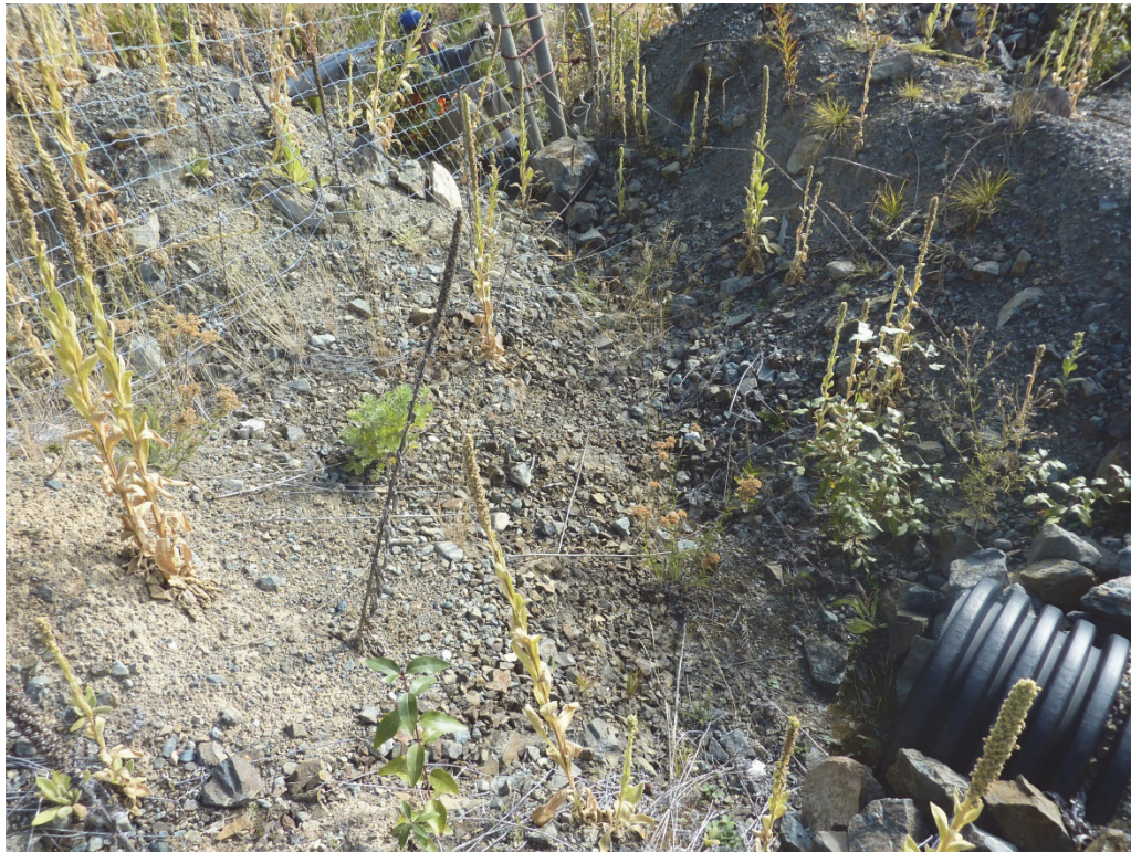
Photo III-9 – Tailings Pond – Bypass Channel at Northeast End of Dam Embankment – Inlet Culvert at Bottom of Photo
