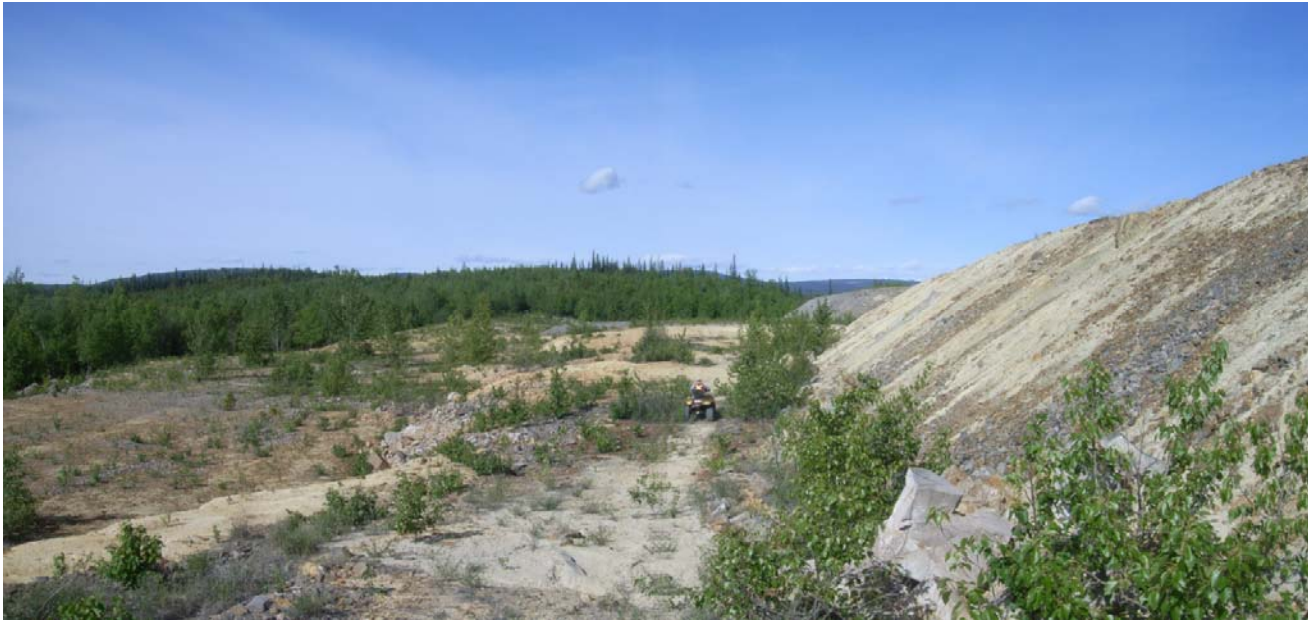
Photo D-11: View of the downstream slope of Dam 5, looking west. (11 June 2014)
