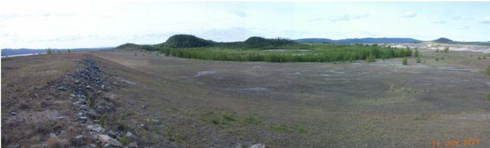
Photo D-2: View of upstream tailings beach and pond, looking south from the junction of Dams 2 and 4. Note that the dams were built to accommodate future tailings storage that did not happen. (11 June 2014)
