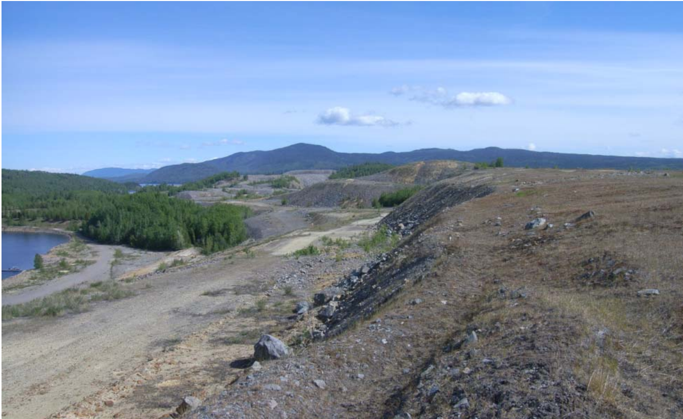
Photo D-10: View of the downstream slope of Dam 3, looking north-east. (11 June 2014)
