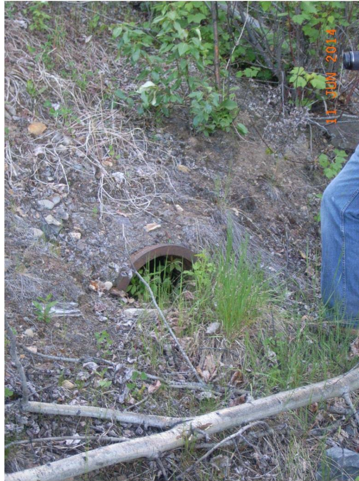
Photo C-8: View of a cast iron pipe located at the toe of the downstream slope of Dam 1, near the left abutment. This was a former decant pipe from the pond that had been decommissioned. There was no evidence of seepage around the pipe. Looking north-east from the toe of Dam 1. (11 June 2014)
