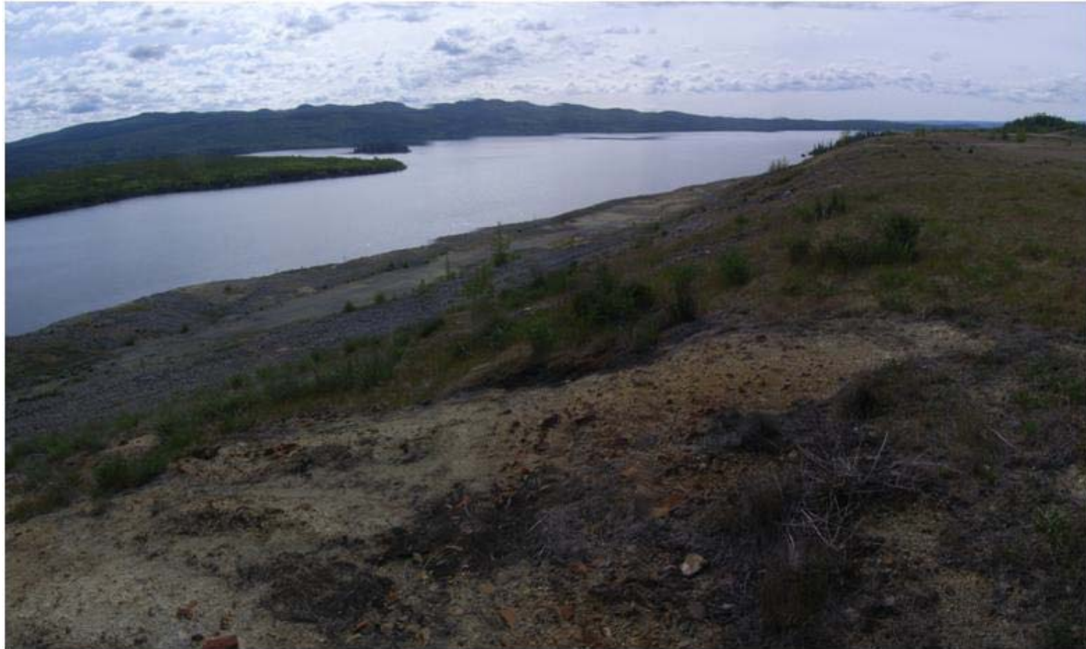
Photo D-6: View of the downstream slope of Dam 2, looking south-east from the junction of Dam 2 and 4. (11 June 2014)
