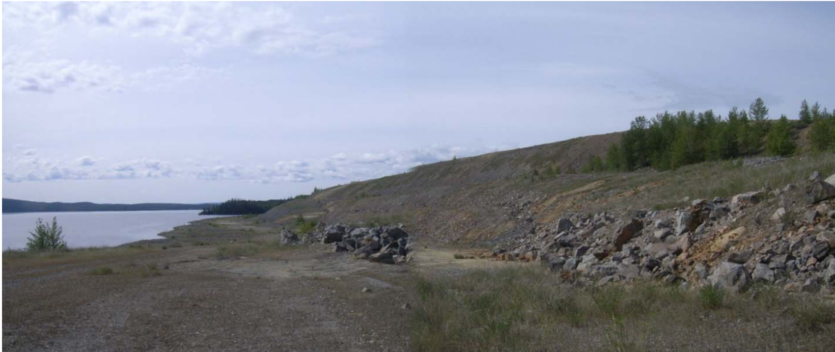
Photo D-7: View of the downstream slope of Dam 2, looking south-east along toe area of Dam 2. (11 June 2014)
