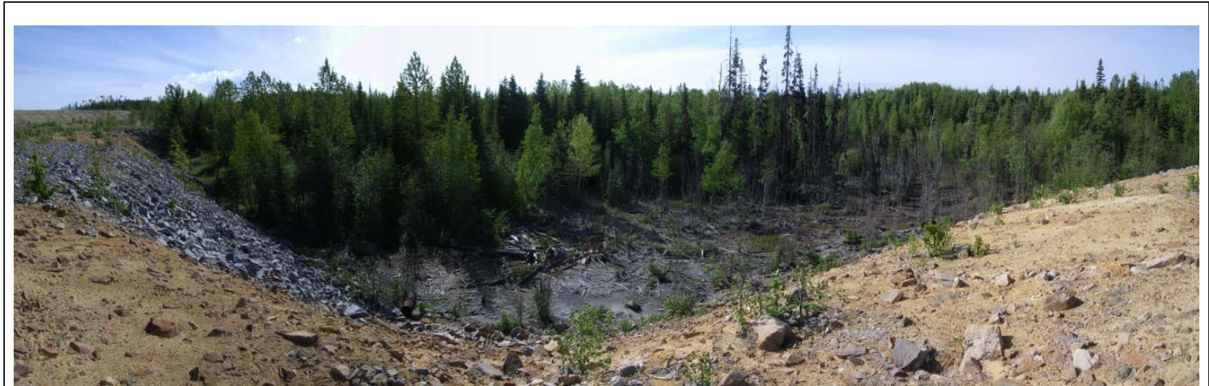
Photo D-12: View of the downstream toe of Dam 5, looking south. Some seepage evident, not a concern. (11 June 2014)
