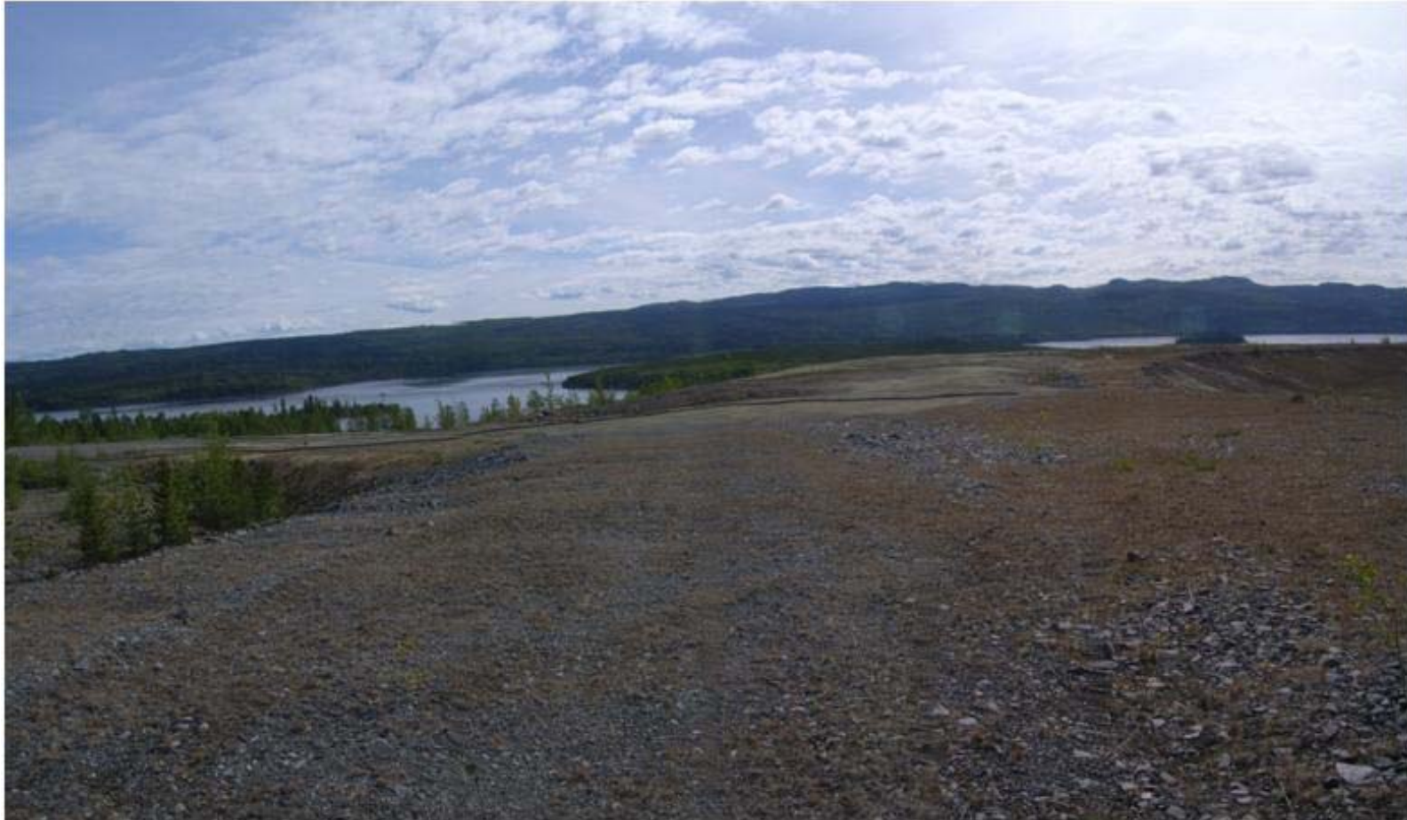
Photo D-3: View of the crest of Dams 4 and 2, near the junction with Dams 4 and 2. Looking east along the crest of Dam 4. (11 June 2014)
