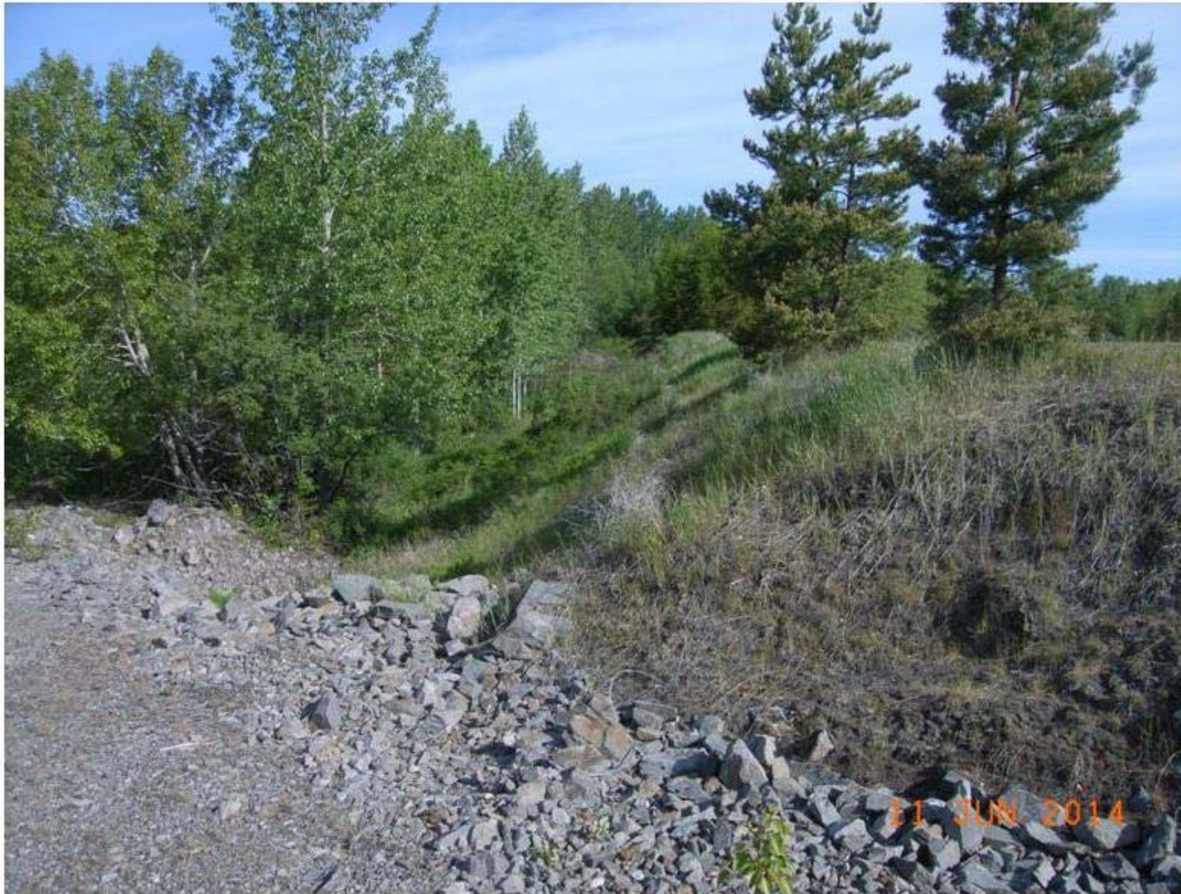
Photo C-6: View of the downstream discharge channel of the depression that could act as a spillway, looking north-west from the crest of Dam 1. (11 June 2014)
