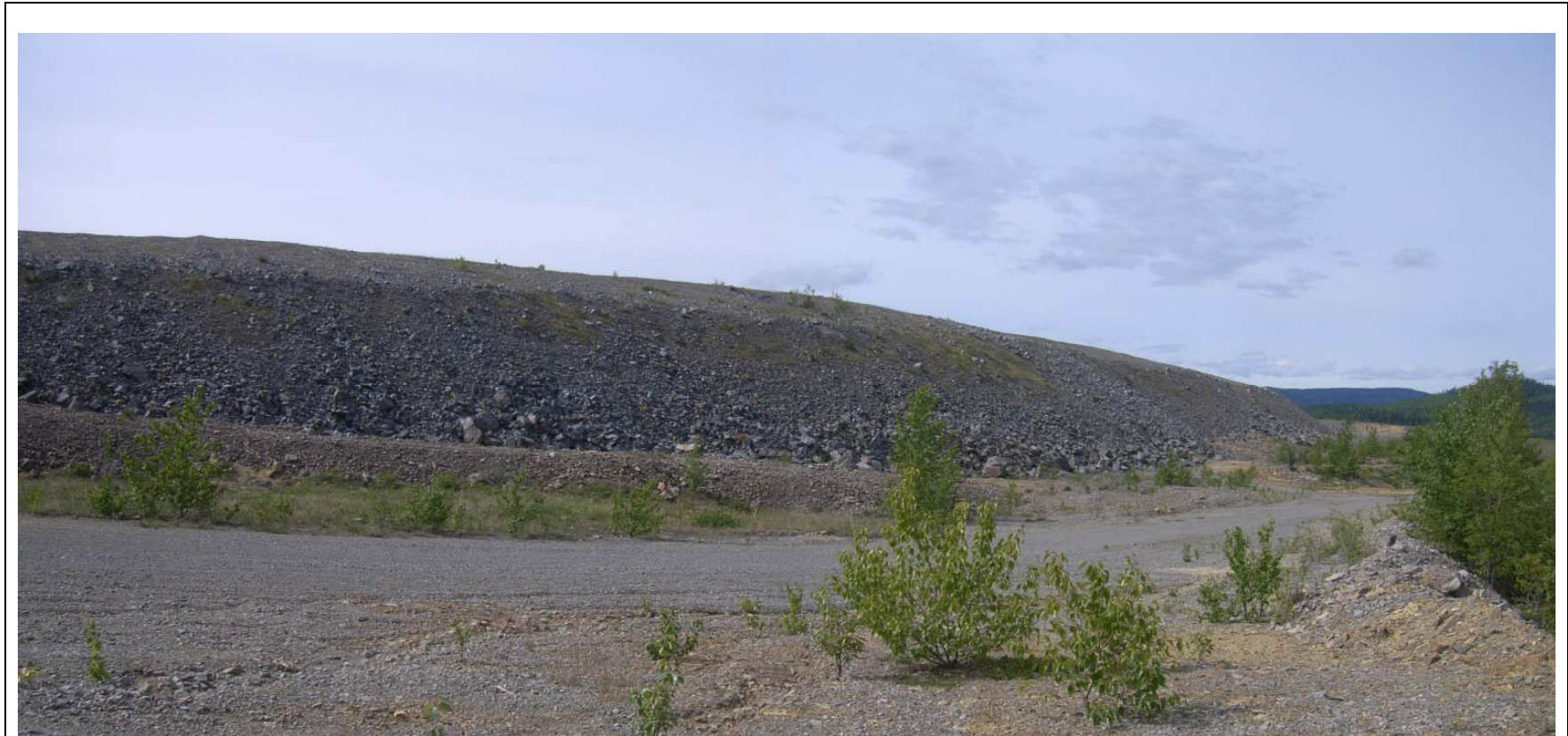
Photo D-8: View of the downstream slope of Dam 4, looking west from beyond the toe of the dam. (11 June 2014)
