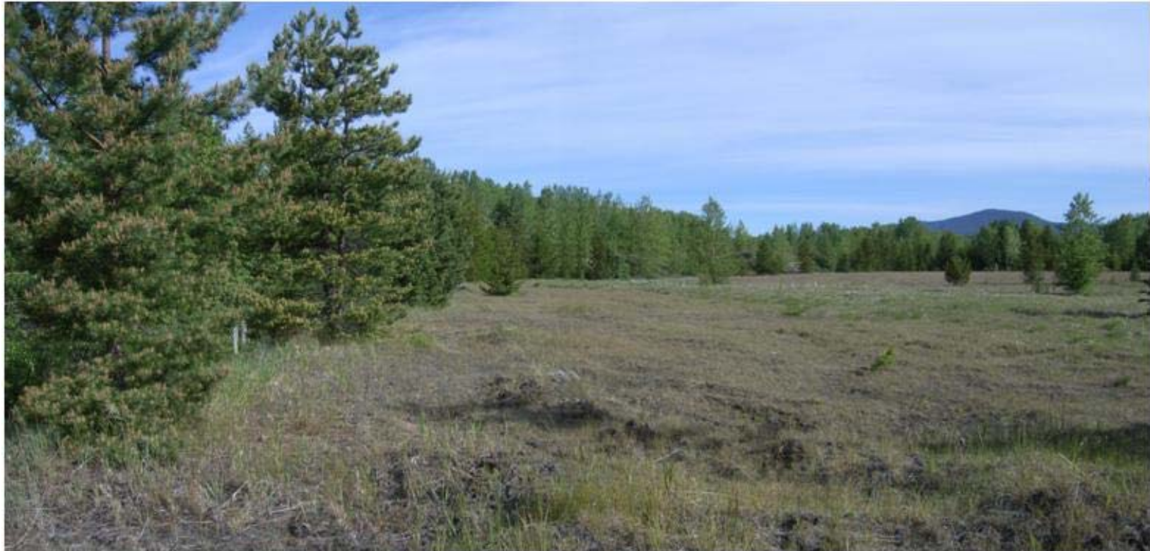
Photo C-3: View of the upstream beach for the segment of the dam that is oriented NW-SE. Looking north-west from about one third along the dam segment. The dam crest is on the left. The downstream slope of the dam is located on the west side of the photo but is heavily vegetated and difficult to see. (11 June 2014)
