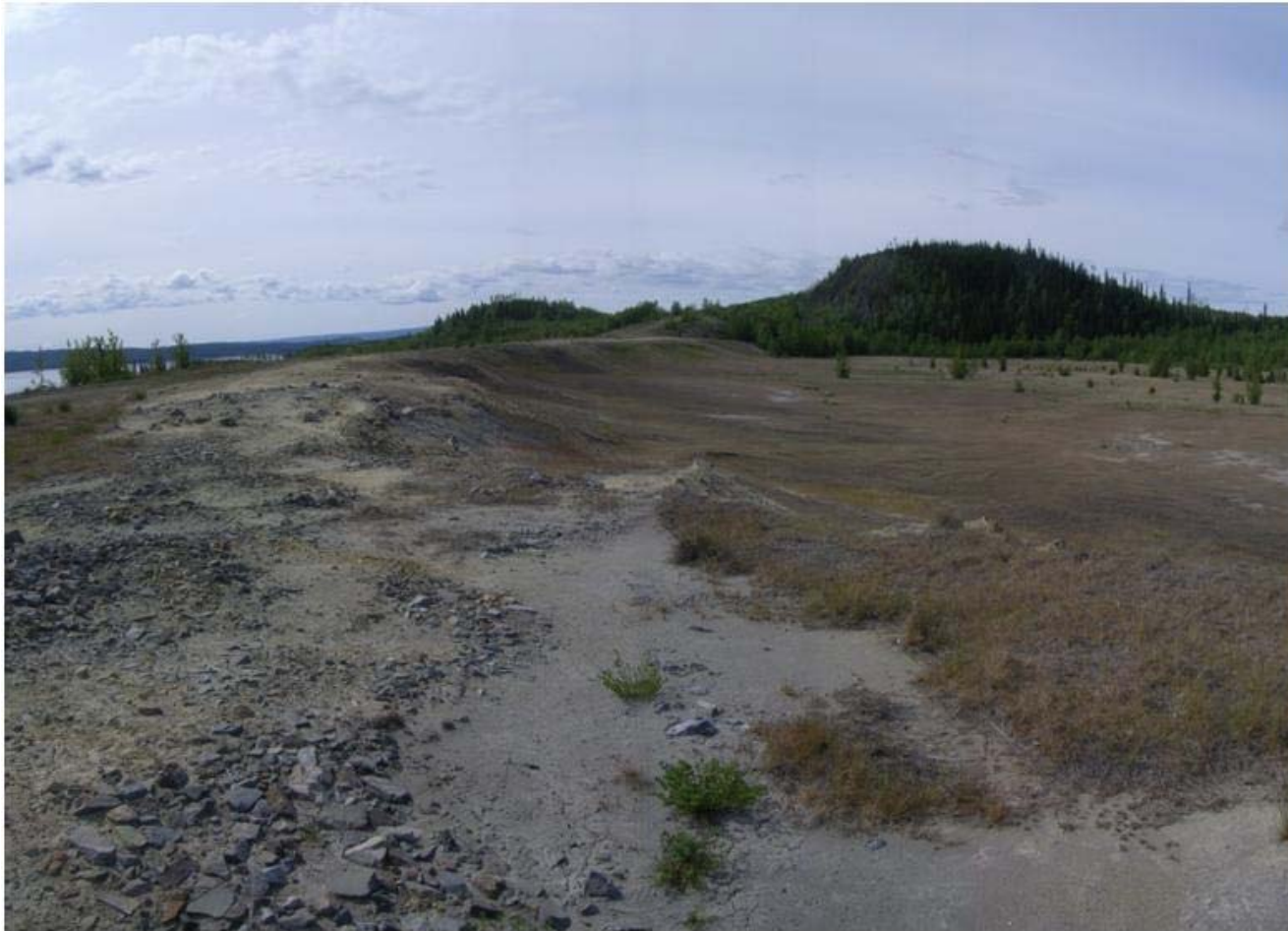
Photo D-1: View of Dam 2 crest and upstream tailings beach, looking south (toward right abutment) from the crest at the left end of Dam 2. (11 June 2014)
