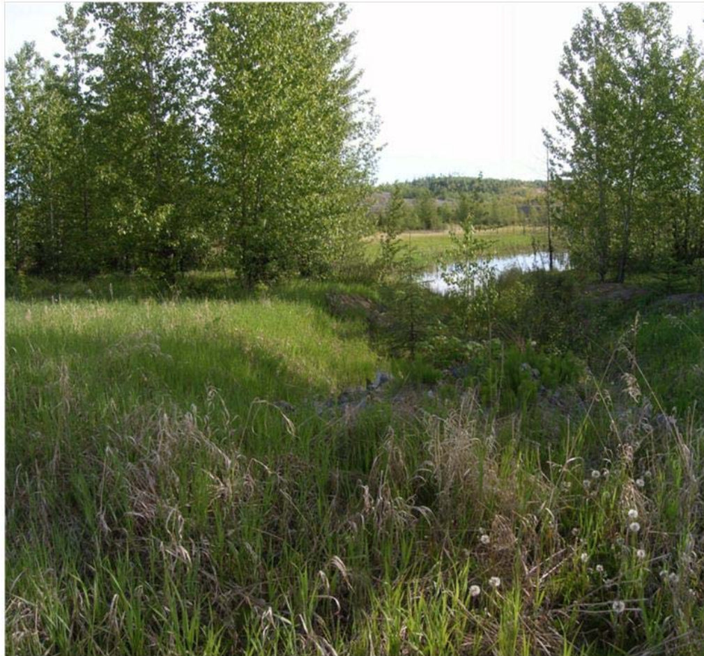
Photo C-2: View of the tailings beach and pond, looking east from the crest, near the north-west end of the segment that is oriented NW-SE. Note that tailings beach is well vegetated and pond is well away from the crest. (11 June 2014)
