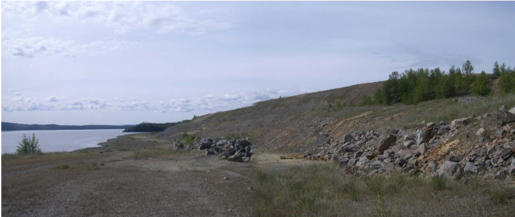
Photo D-13: View of the downstream slope of Dam 2, looking south-east along toe area of Dam 2. (11 June 2014)
