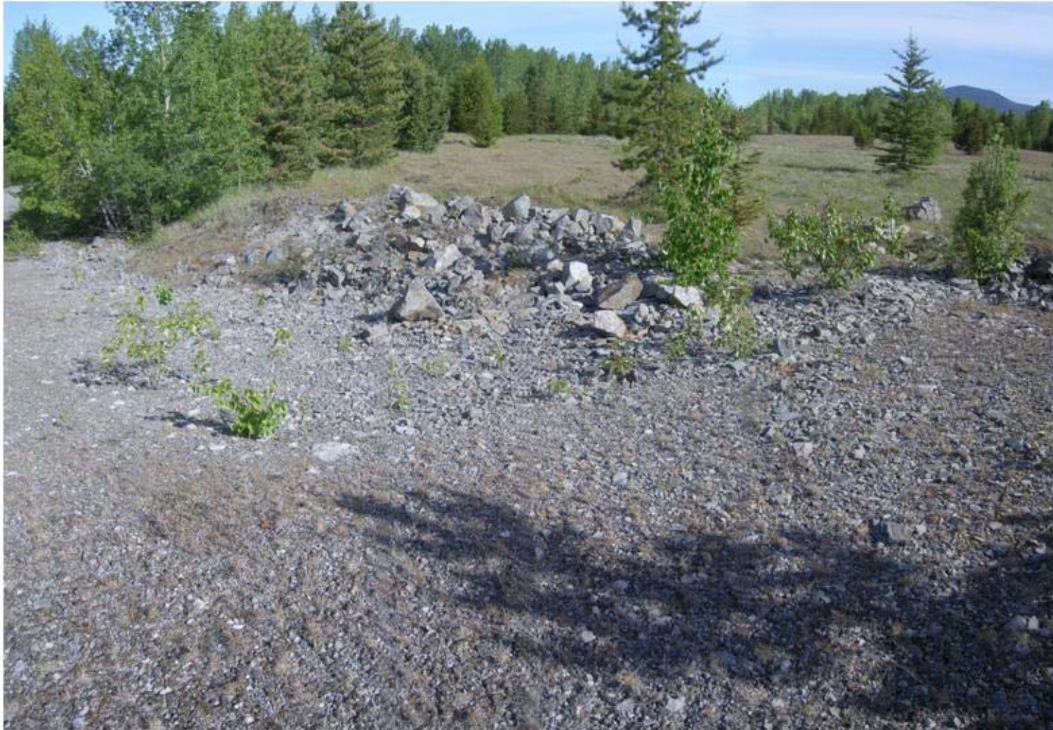
Photo C-5: View of the depression in central portion of Dam 1 that will act as a spillway. Looking north-west. According to Glencore, this feature was not intended to be a spillway, but it could act as such. (11 June 2014)
