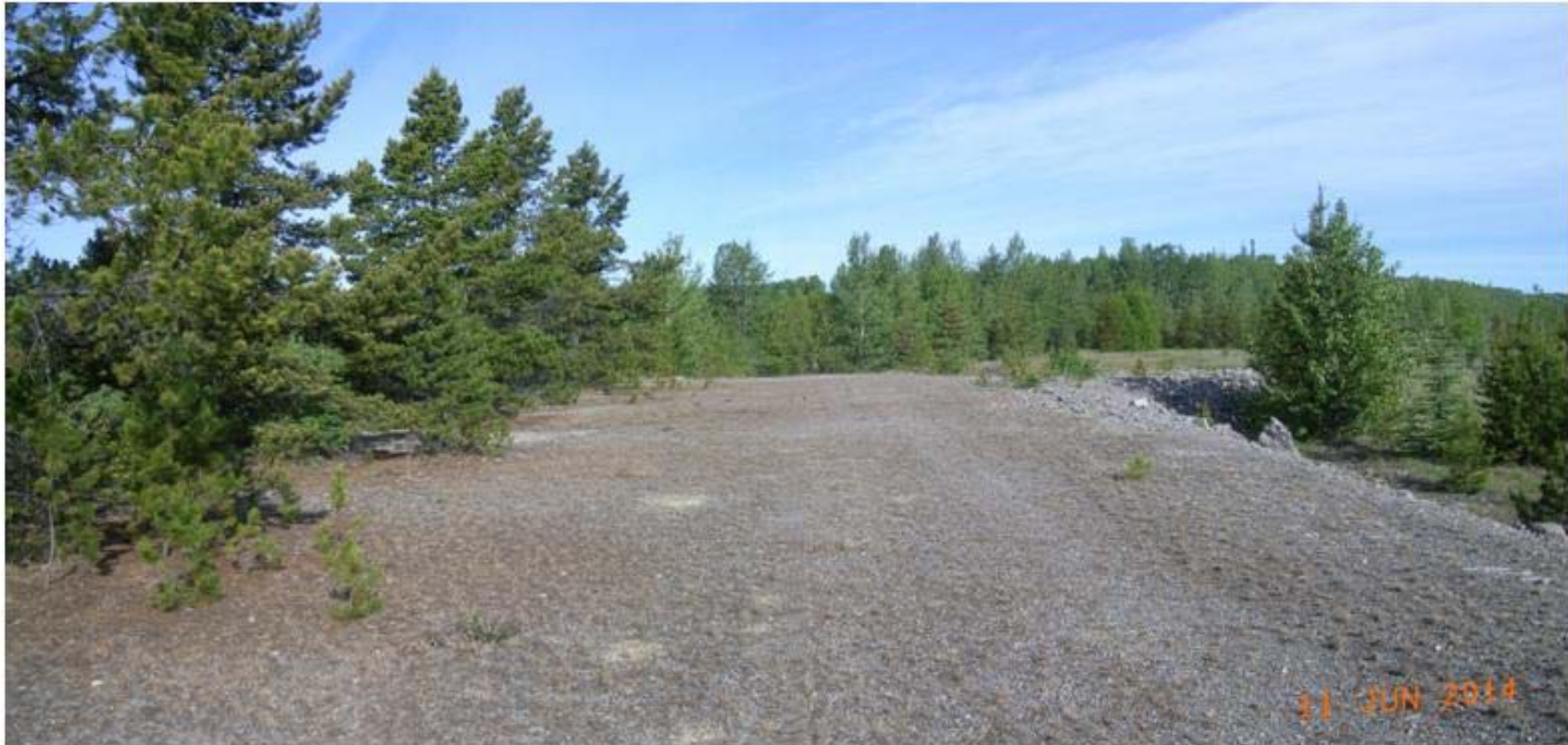
Photo C-4: View of the crest of Dam 1, looking north-west along the segment of the dam that is oriented NW-SE. In the background is a depression that will act as a spillway. See the next photo. (11 June 2014)
