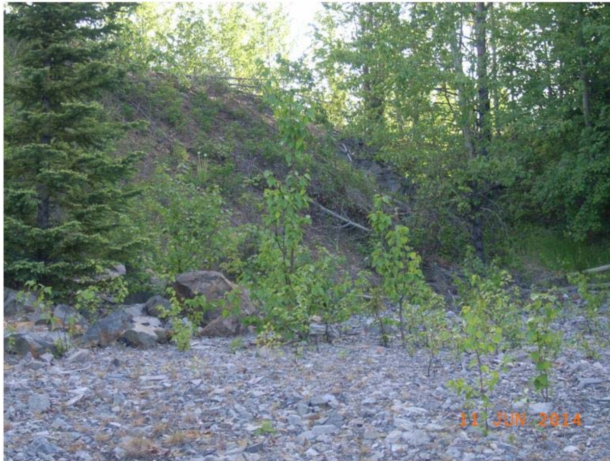
Photo C-7: View of the downstream slope at left abutment, looking north-east from beyond the toe of Dam 1. Note that the downstream slope of the dam is heavily vegetated, but it is not a concern. The actual spillway for the dam is located on the right side of the photo, note the depression, but it is covered in vegetation. (11 June 2014)
