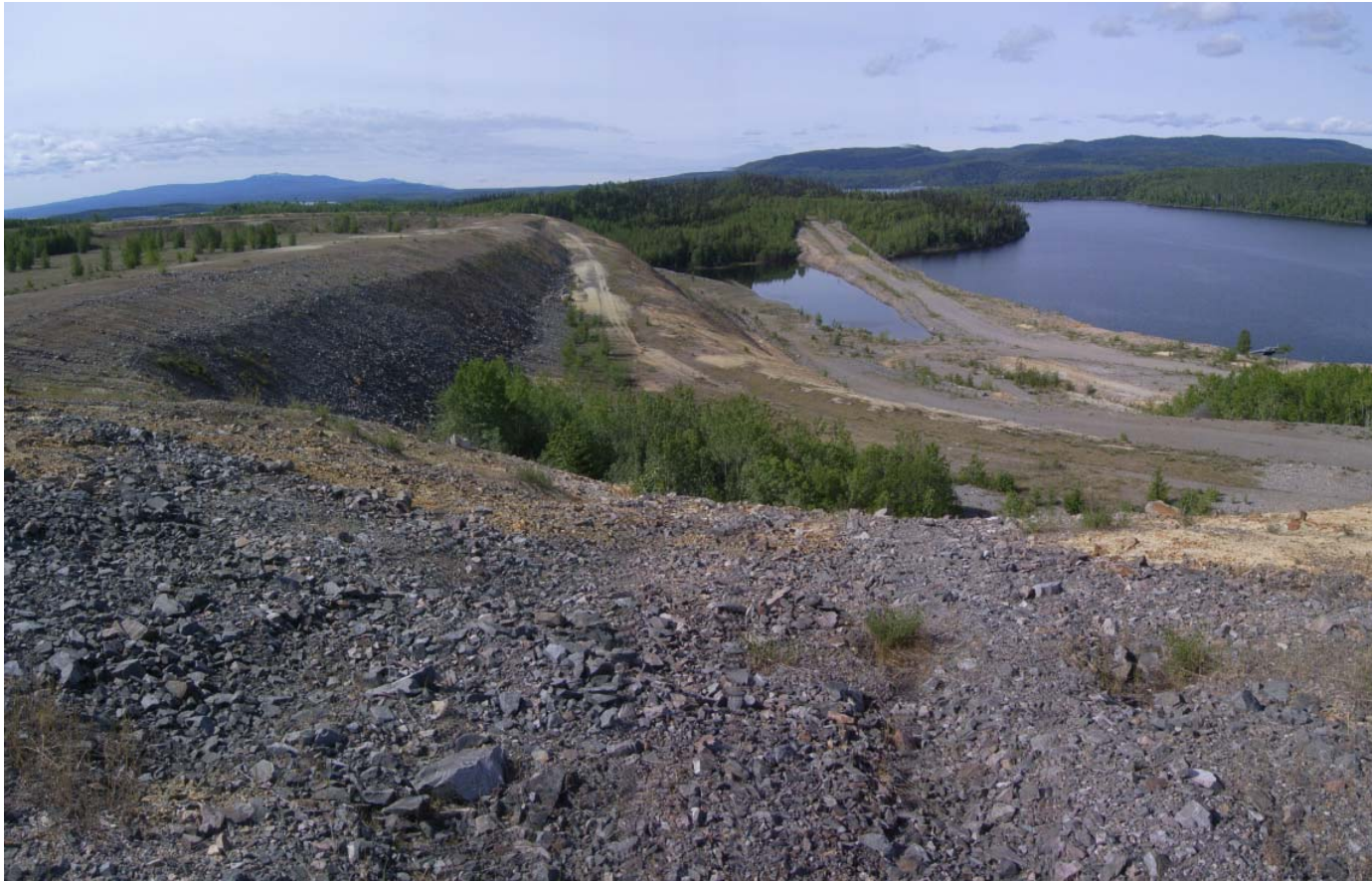
Photo D-9: View of the downstream slope of Dam 3, looking south-west. (11 June 2014)
