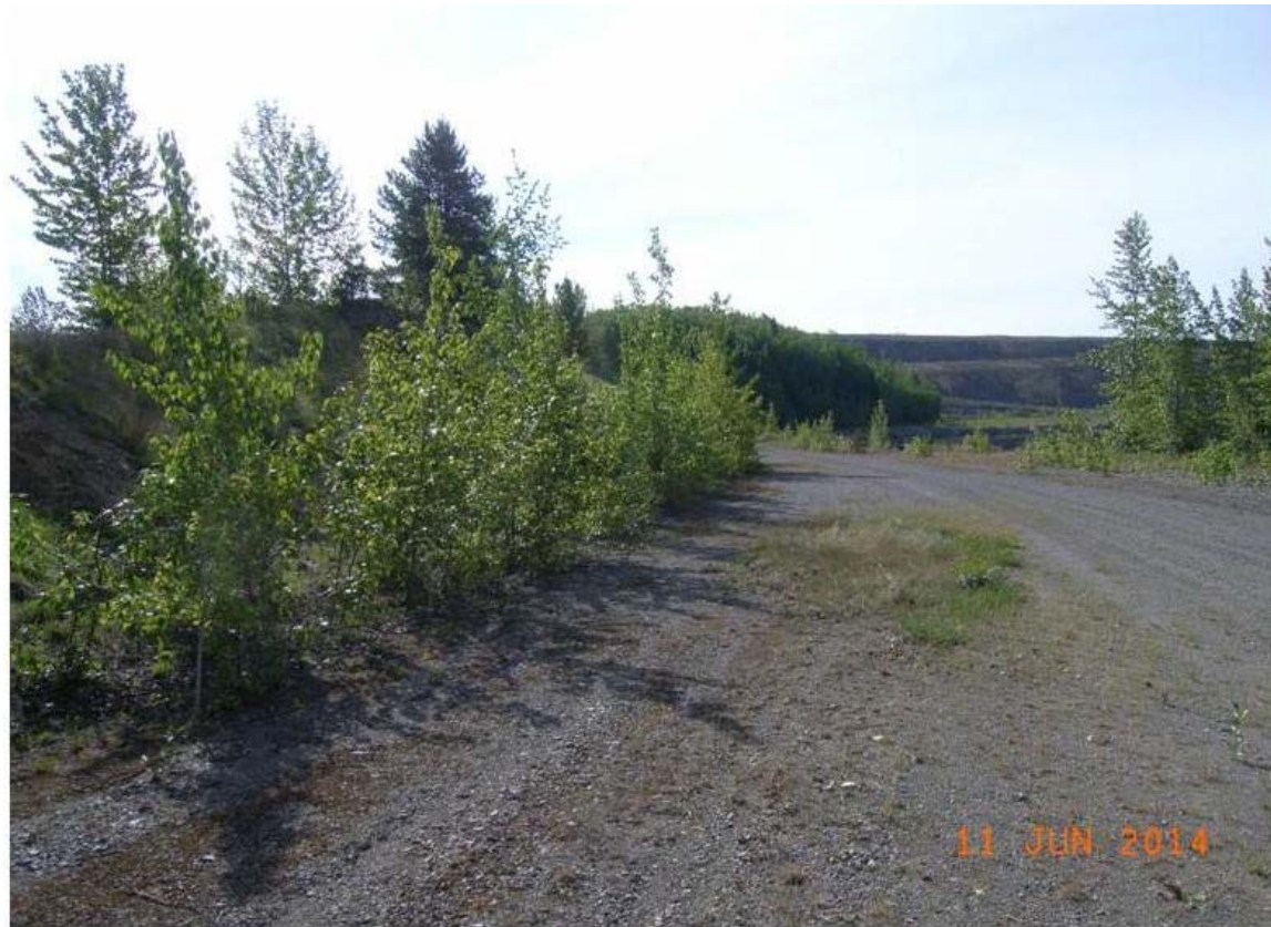
Photo C-9: View of the downstream slope of Dam 1, looking southeast along the NW-SE segment of the dam. (11 June 2014)
