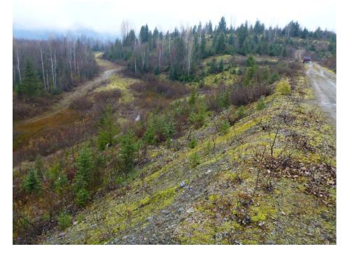
Photo 6 – Downstream slope, right abutment and toe area viewed from crest of West Dam. Photo taken from mid-point of dam, facing north northwest. Note bench at mid-slope on downstream slope of dam.
