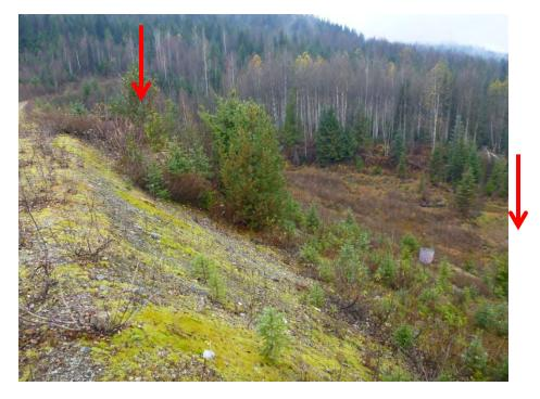
Photo 7 – Downstream slope and left abutment and toe area viewed from crest of West Dam. Photo taken from mid-point of dam, facing south southwest. Note bench at mid-slope on downstream slope of dam. Red arrows indicate piezometer locations on downstream slope.
