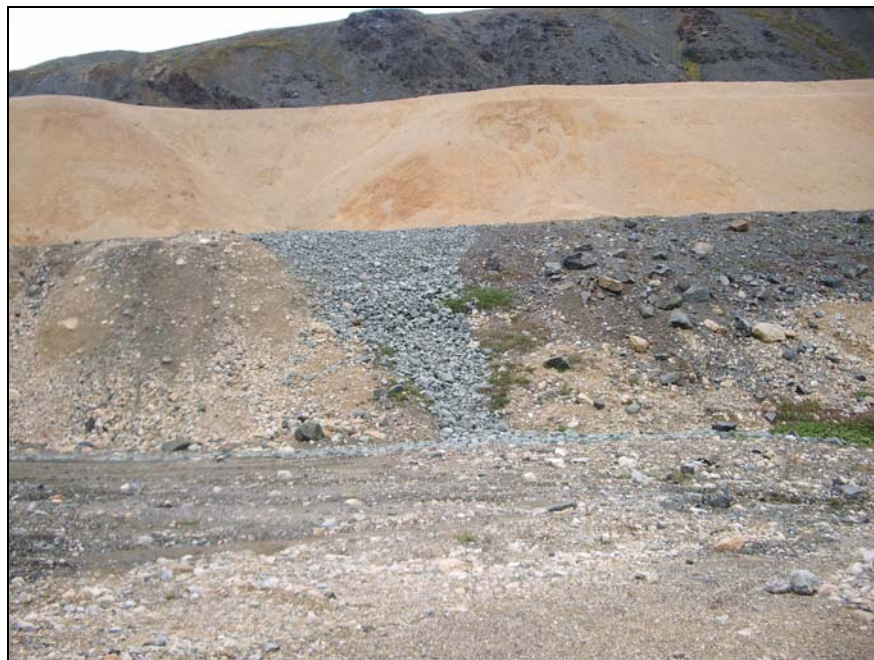
PHOTO 8 – Fleece Bowl Heap Leach Facility V-Notch Outlet Drain in Confining Embankment (Looking West)
