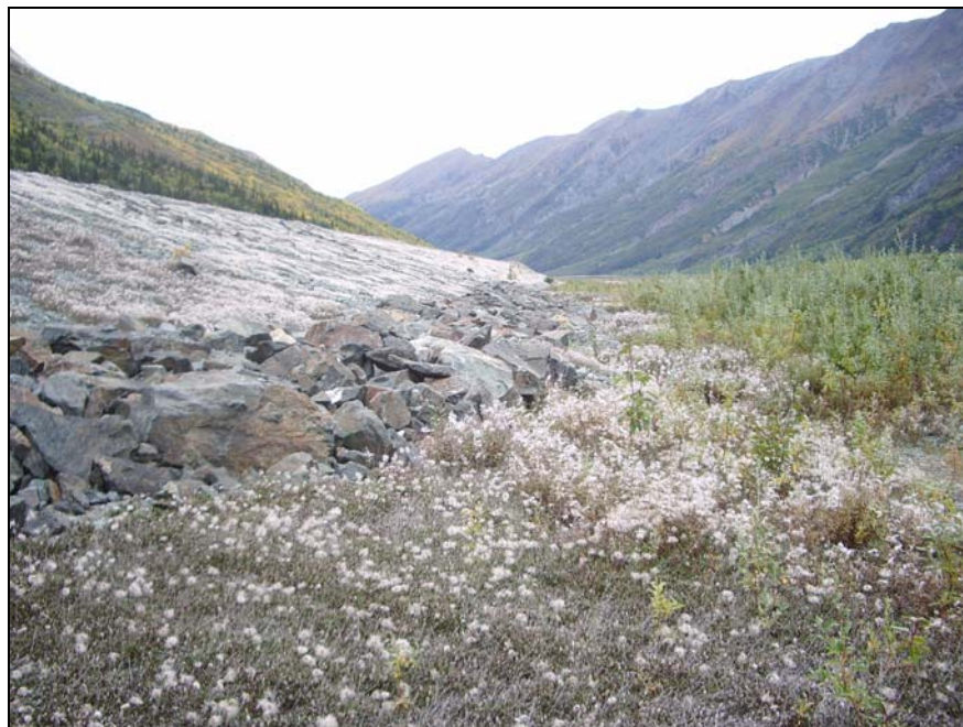
PHOTO 4 – Riprap Erosion Protection along Toe of Downstream TSF Embankment Slope (Looking East)
