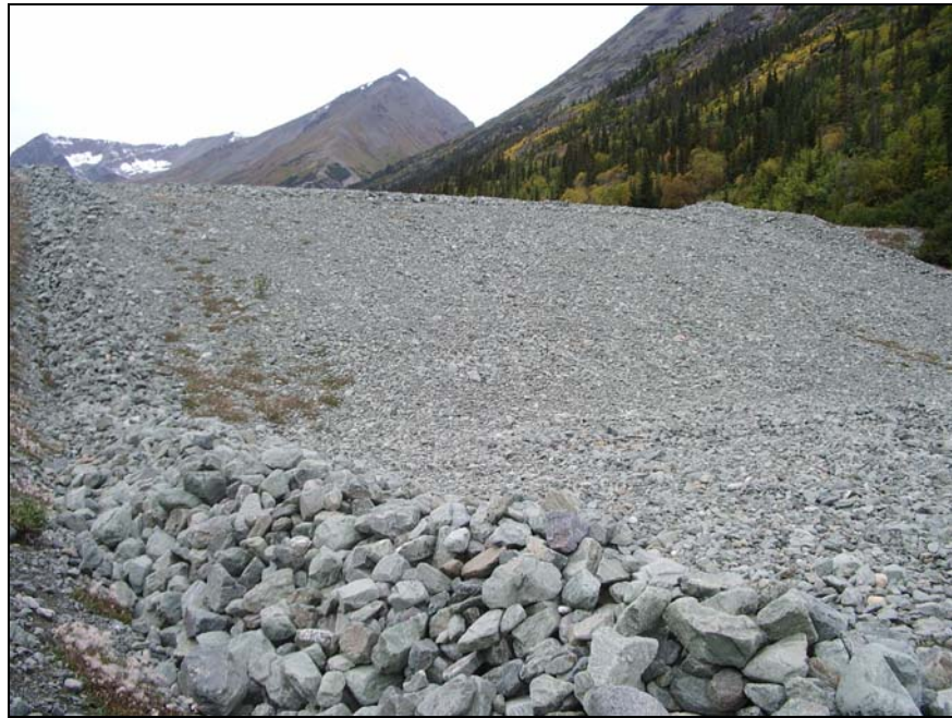
PHOTO 5 – Riprap Erosion Protection in TSF Spillway Channel (Looking West)
