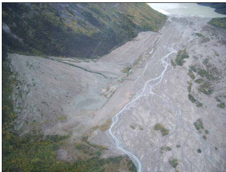
PHOTO 1 – Overview of Tailings Storage Facility (Looking East)
