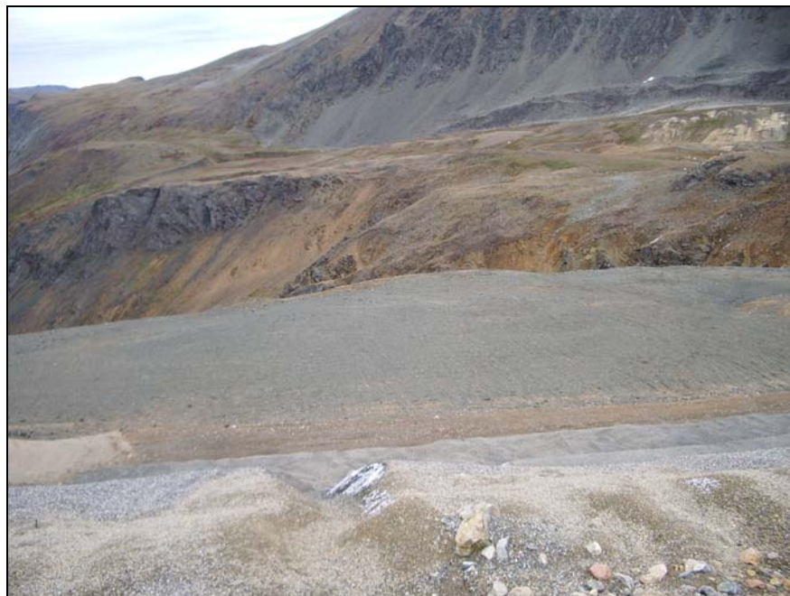
PHOTO 18 – Re-graded Totem Creek Events Pond Area (Looking Northeast)
