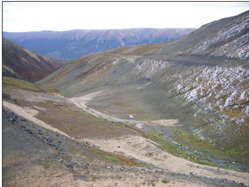
PHOTO 10 – Reclaimed Water Storage Dam Area (Looking East)
