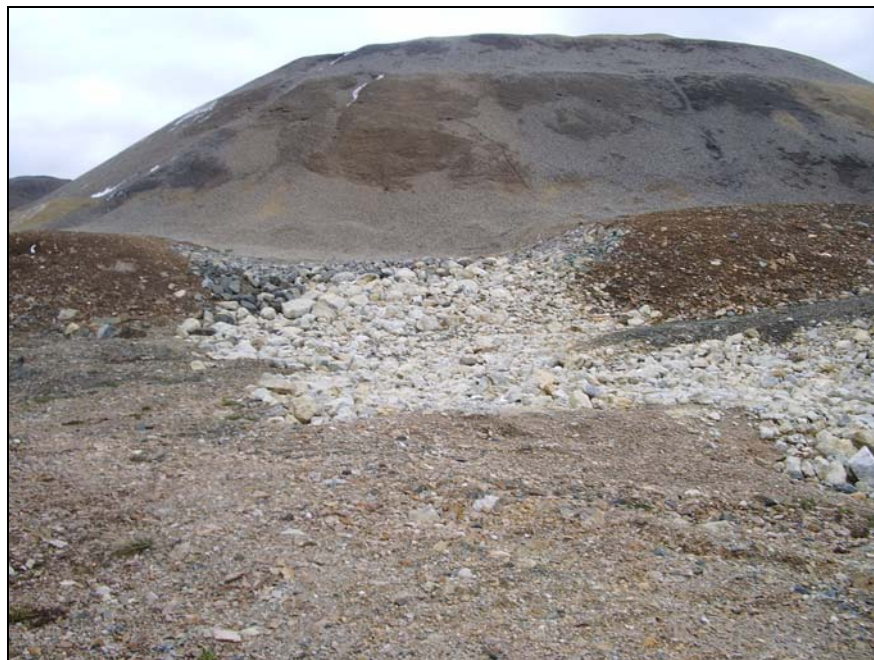
PHOTO 14 – Totem Creek Heap Leach Facility V-Notch Outlet Drain in Confining Embankment (Looking South)
