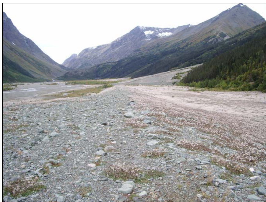
PHOTO 2 – Reclaimed Embankment Crest (Looking West)
