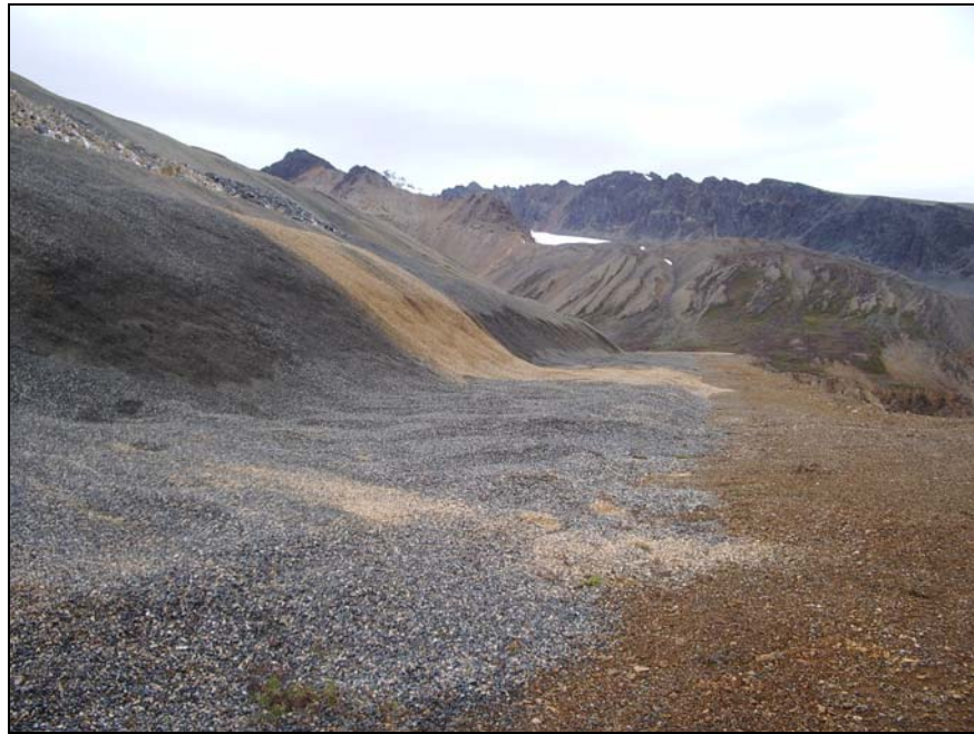
PHOTO 17 – Reclaimed Confining Embankment at Totem Creek Heap Leach Facility (Looking South)
