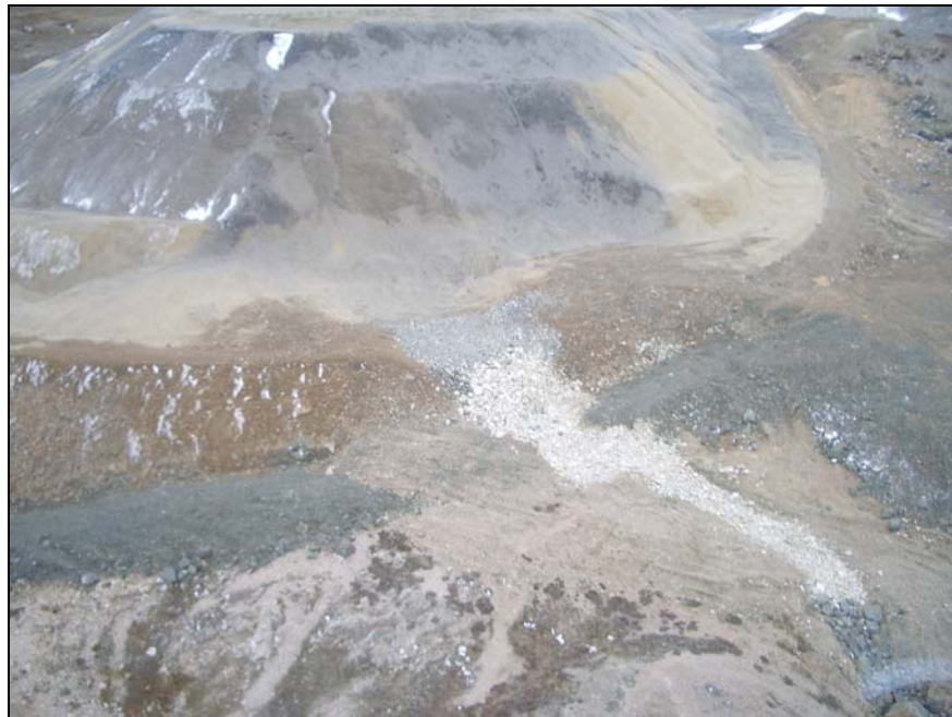
PHOTO 16 – Totem Creek Facility V-Notch Discharge Point into Existing Swale (Looking South)
