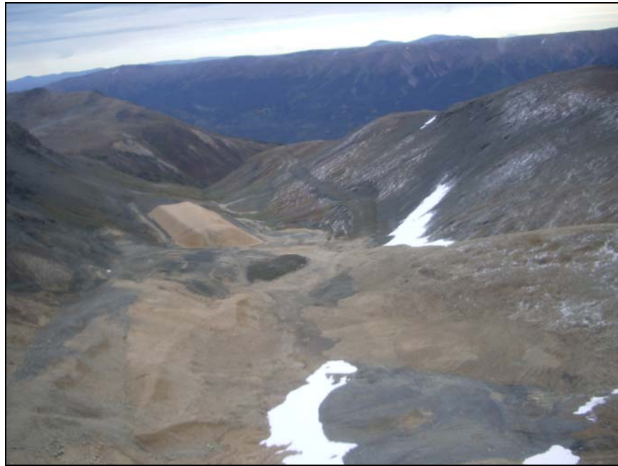
PHOTO 7 – Overview of Fleece Bowl Heap Leach Facility (Looking East)
