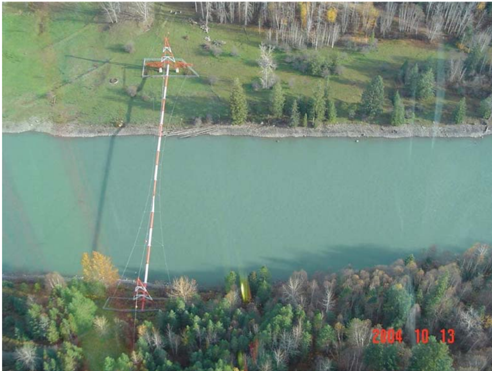
Photo II-21 Pipeline crossing on Quesnel River at eastern municipal boundary of City of Quesnel.
