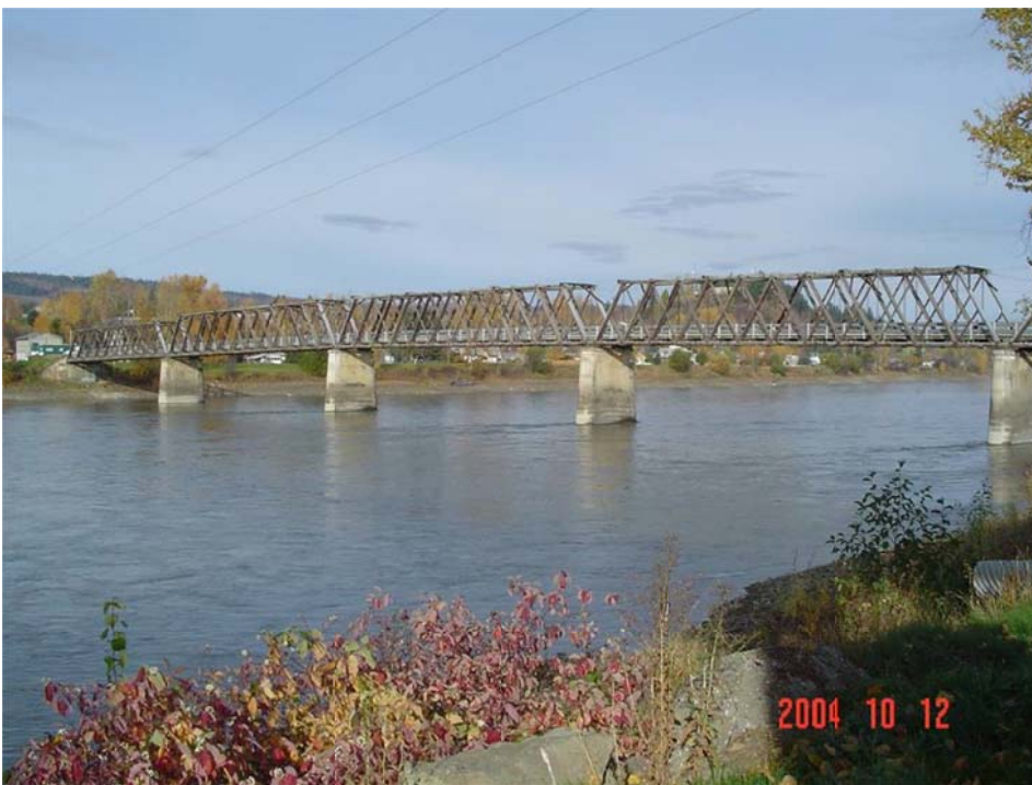
Photo II-36 Carson Ave. pedestrian bridge across Fraser River, looking upstream from left bank.
