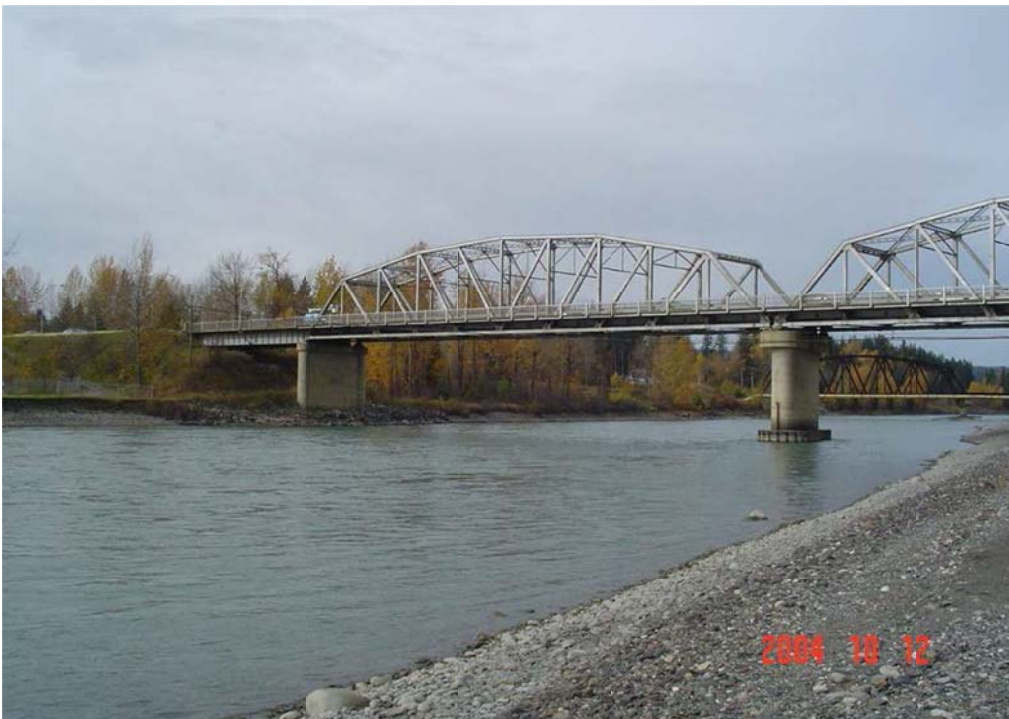
Photo II-30 Highway 97 bridge on Quesnel River, looking upstream from left bank.
