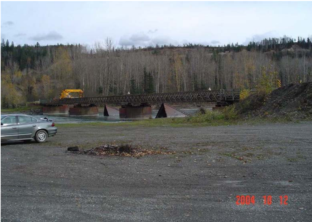
Photo II-15 Gravelle bridge across Quesnel River as seen from left bank.
