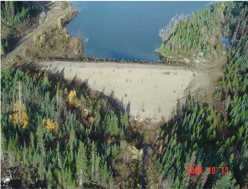
Photo II-3 East Saddle Dam as seen from downstream.
