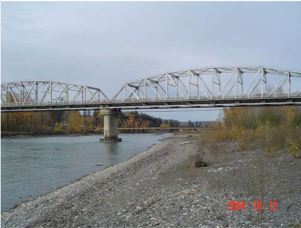
Photo II-31 Highway 97 bridge on Quesnel River, looking upstream from left bank.
