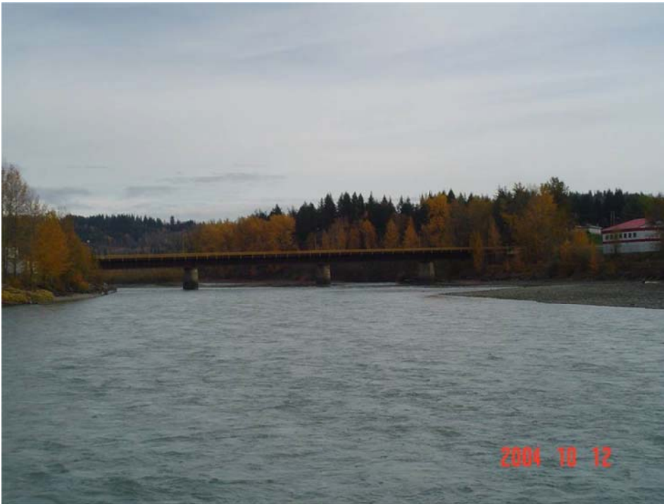
Photo II-33 Johnston Ave. bridge across the Quesnel River, looking upstream from right bank.
