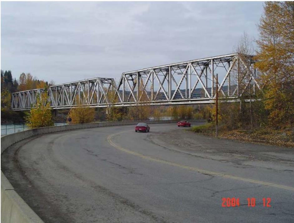
Photo II-35 Railway bridge at the mouth of the Quesnel River, as seen from the right bank of the river. Flow is left to right.
