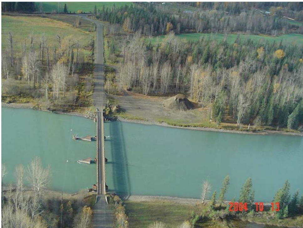
Photo II-14 Gravelle bridge across Quesnel River, as seen from right bank.
