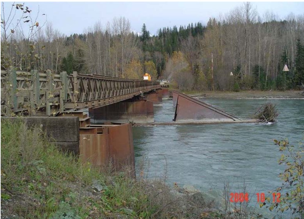
Photo II-16 Gravelle bridge as seen from left bank. Note triangular steel ice breakers upstream of bridge.
