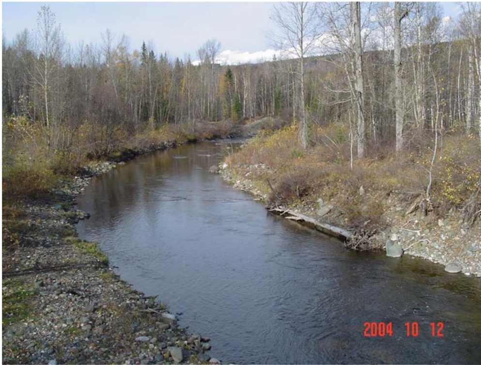
Photo II-11 Beaver Creek looking downstream from Beaver Creek bridge.
