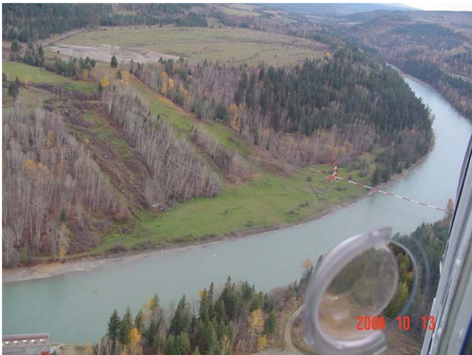
Photo II-22 Powerline and pipeline crossing on Quesnel River at eastern municipal boundary of City of Quesnel.
