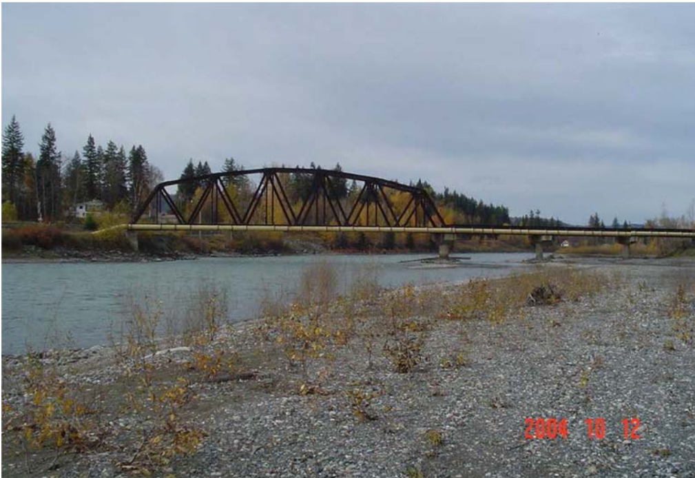
Photo II-29 Railway bridge across Quesnel River upstream of Highway 97, looking upstream from left bank. Note pipeline strung along the side of bridge.
