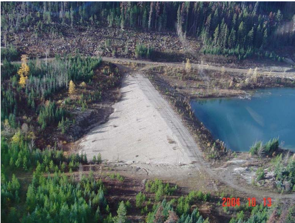
Photo II-4 East Saddle Dam as seen from north abutment.
