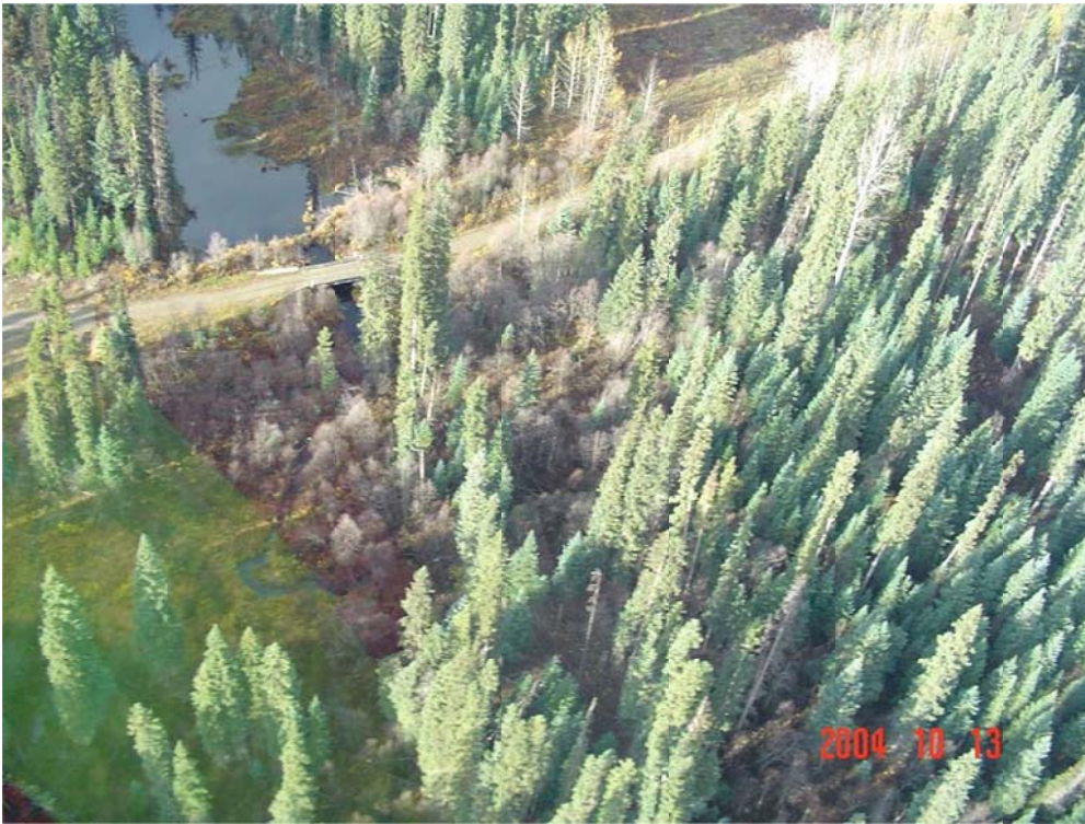
Photo II-39 Typical wooden bridge on local roads.
