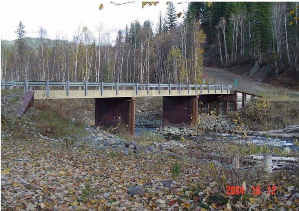
Photo 10 Beaver Creek bridge upstream of Beaver Creek and Quesnel River confluence, as seen from left bank.
