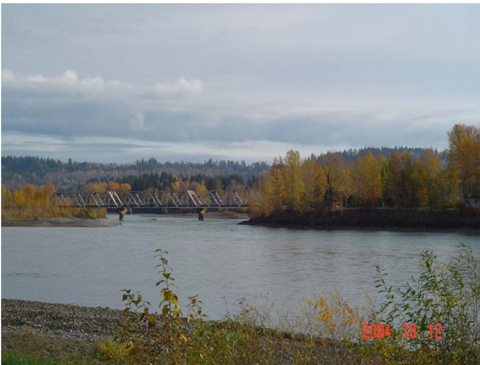
Photo II-34 Railway bridge across the mouth of the Quesnel River, as seen from right bank of Fraser River.
