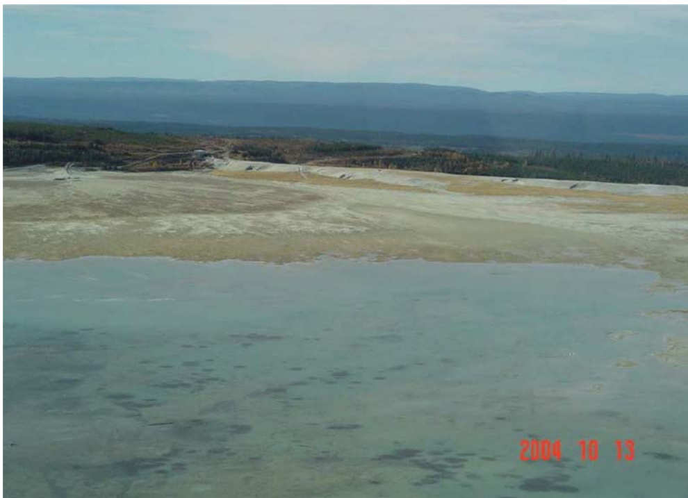
Photo II-2 Main Tailings Dam as seen from north side of tailings pond.
