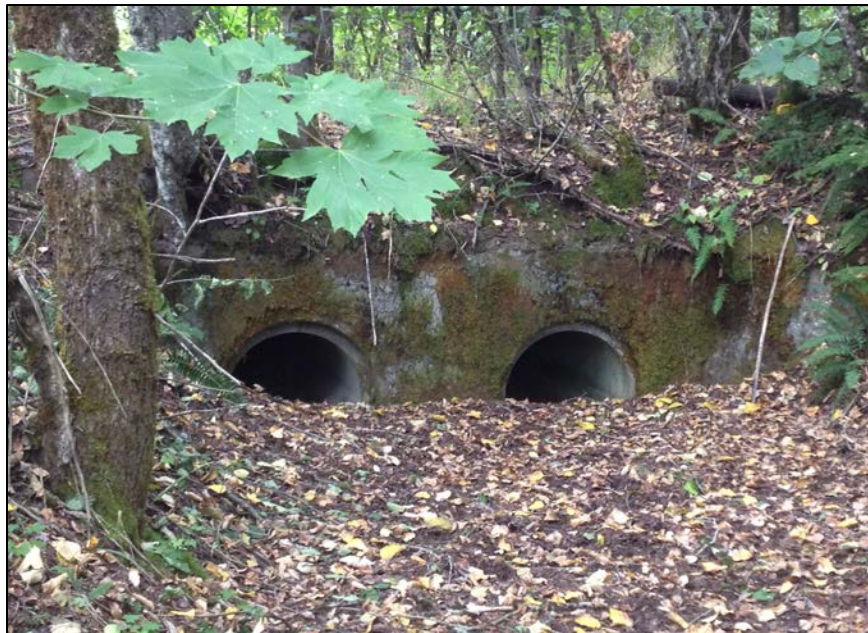
PHOTO 8 - Lower Tailings Pond - Concrete Decant Spillway Structure (looking downstream)
