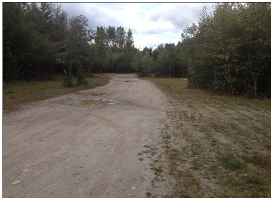
PHOTO 12 - Upper Tailings Pond - Access along capped and reclaimed tailings surface
