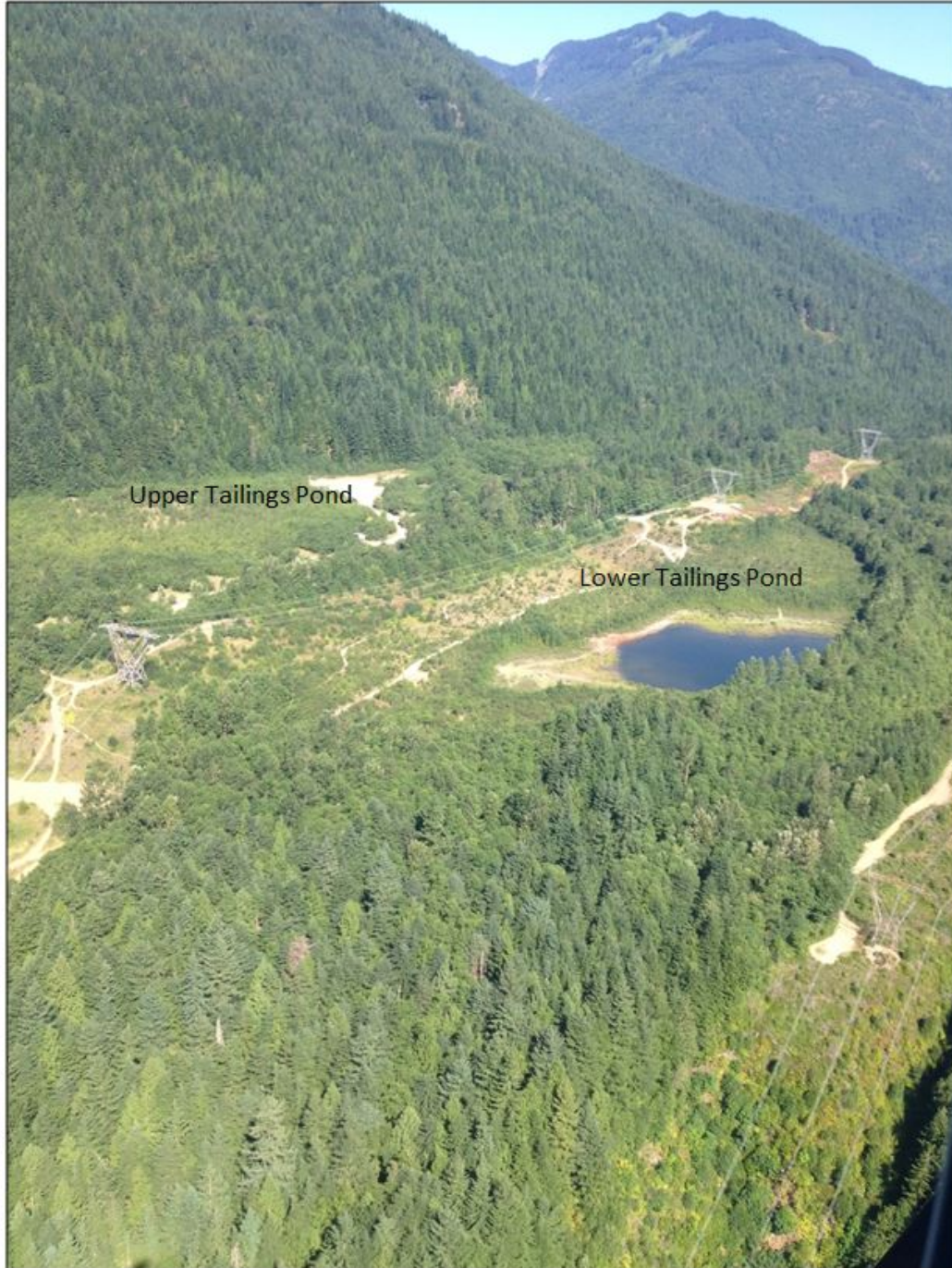
Figure 1.3 Aerial Photograph of the Tailings Facility (August 5, 2014)
