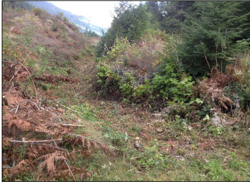
PHOTO 7 - Lower Tailings Pond - Channel Spillway (looking downstream)
