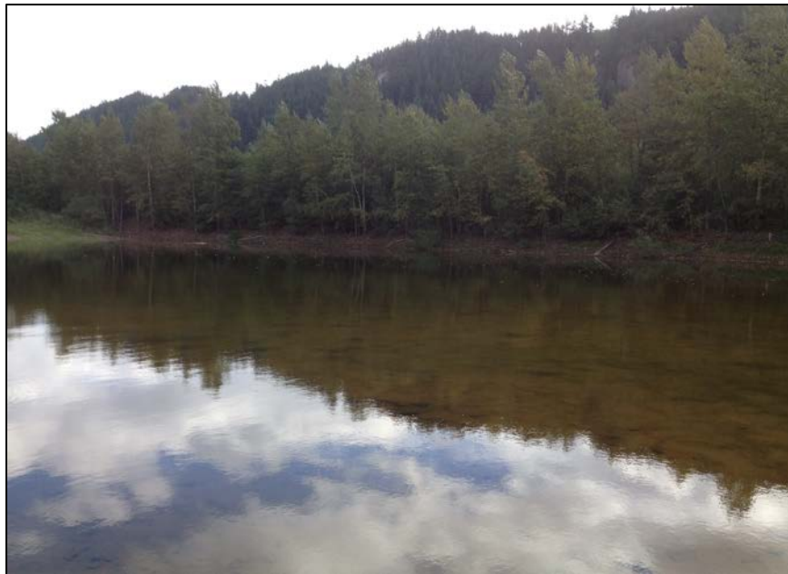
PHOTO 6 - Lower Tailings Pond - Water pond with eastern embankment behind (looking east)
