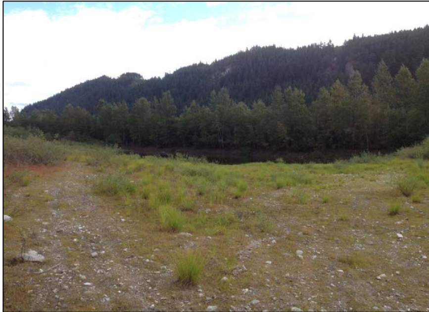
PHOTO 3 - Lower Tailings Pond - Capped tailings surface in foreground with water pond and eastern embankment behind (looking east)
