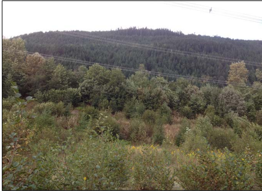
PHOTO 9 - Upper Tailings Pond - Downstream embankment slope (looking west)
