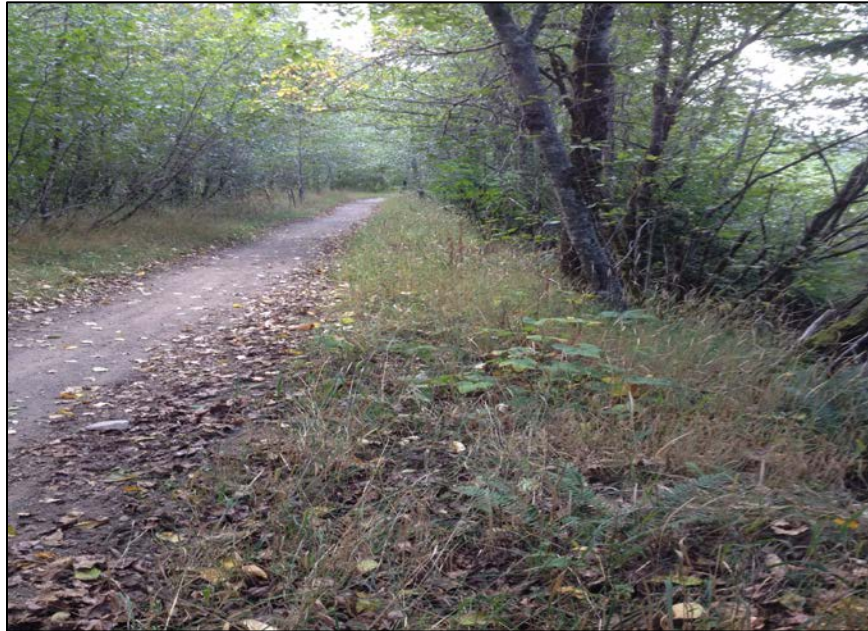
PHOTO 1 - Lower Tailings Pond - Embankment crest (looking south)
