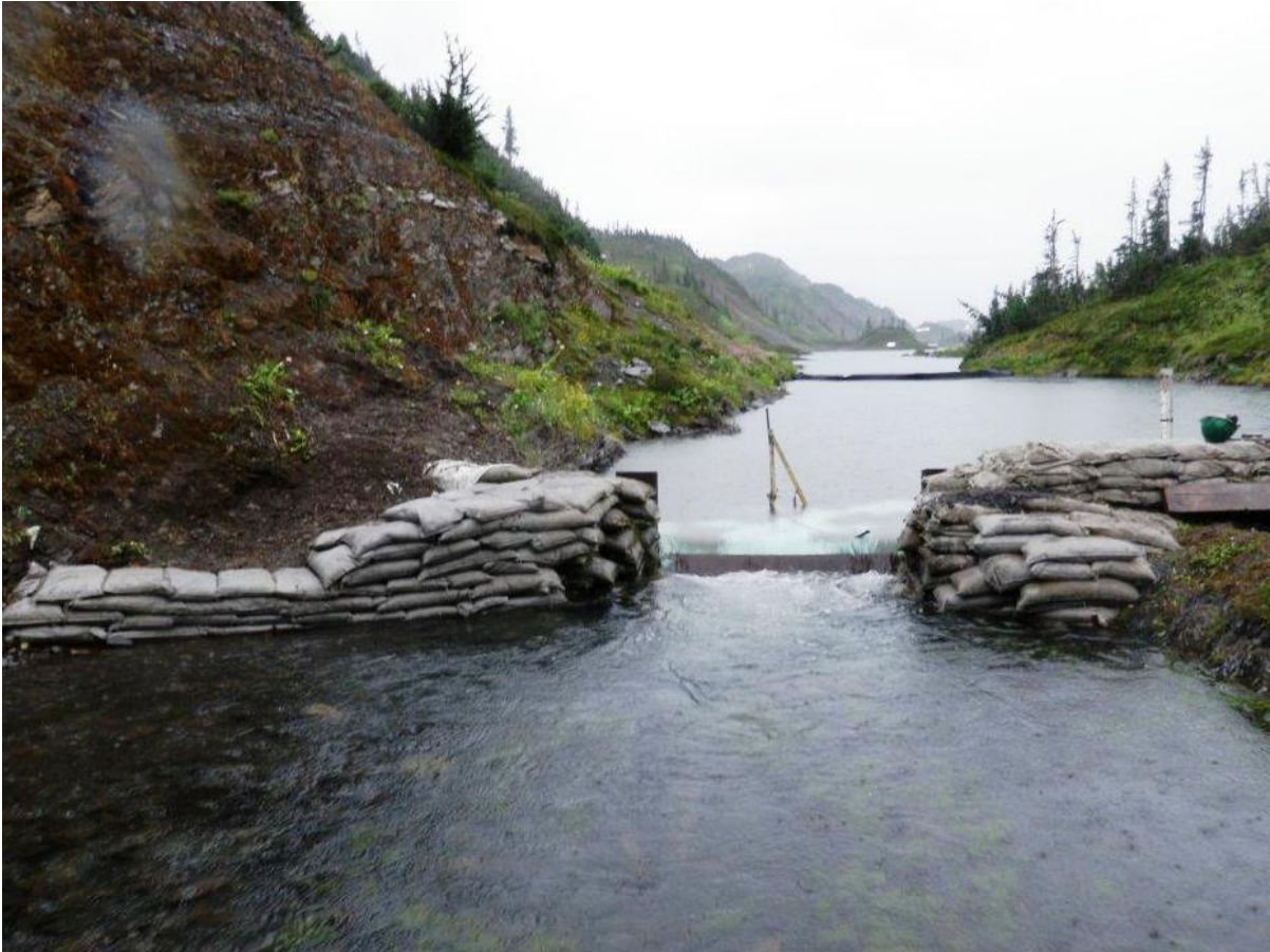
Figure 2. Outflow measurement weir at the northeast end of the Tom MacKay Lake TSF.
