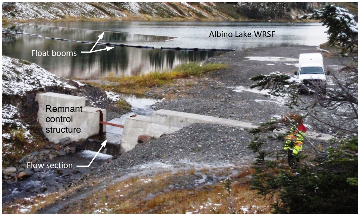
Figure 2. Remnant control structure at the south end of the Albino Lake WRSF.
