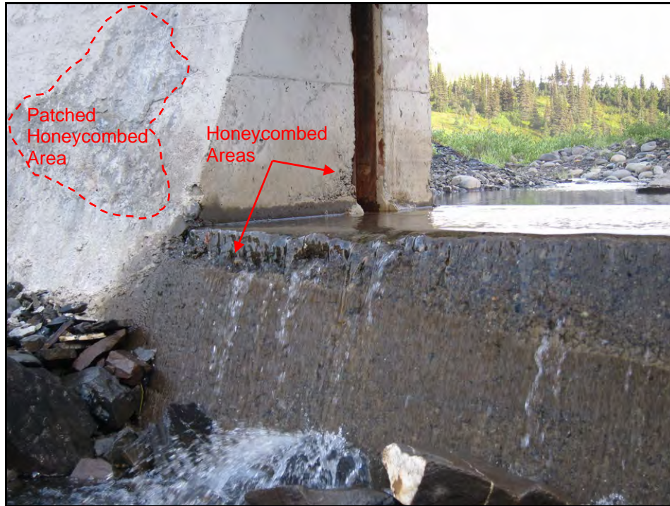
PHOTO 7 – Honeycombed areas below stop-log slot and next to steel stop-log guide.
