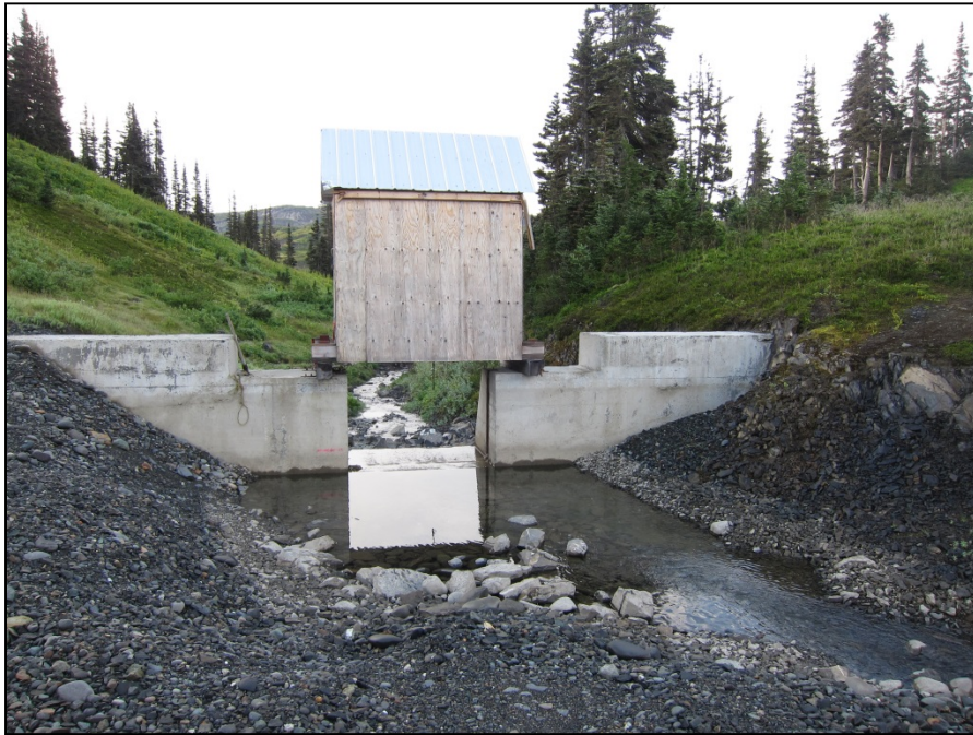
PHOTO 1 – Albino Lake Structure with Stop-Log Hoist Structure (2010).
