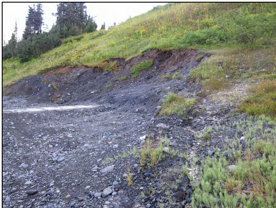
PHOTO 8 – Excavation on left abutment hill slope.
