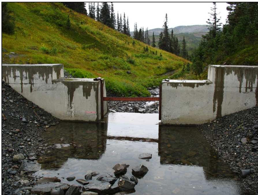
PHOTO 2 – Albino Lake Structure without Stop-Log Hoist Structure (2013).
