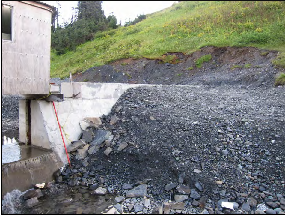
PHOTO 5 – Downstream left abutment (buried).
