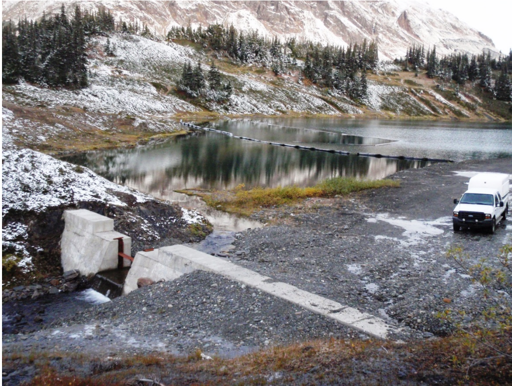
Albino Lake WRSF looking northwest over decommissioned control structure, with the concrete invert section approximately 160 mm below the lake water surface elevation.
