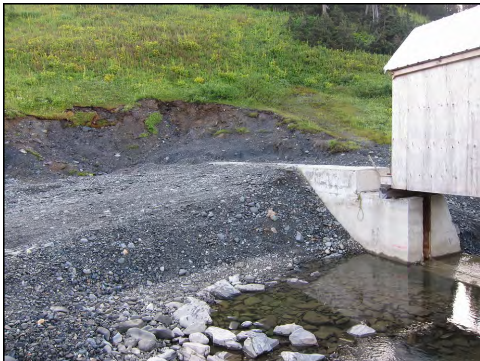
PHOTO 6 – Upstream left abutment (buried).
