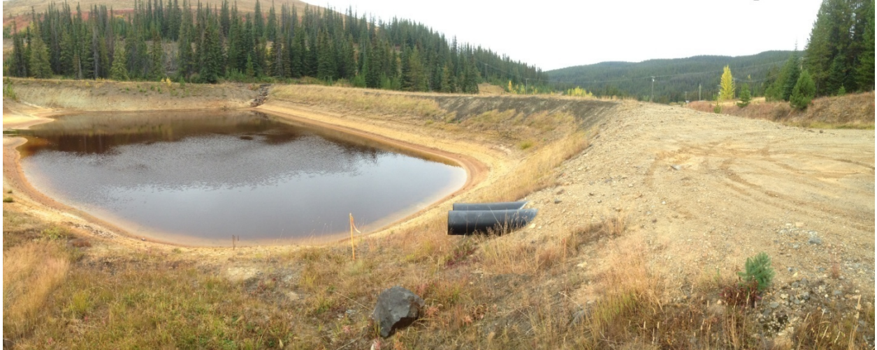
Photo 9: ARD Surge Pond, view of upstream slope and spillway inlet pipes. Taken 18 September 2014.
