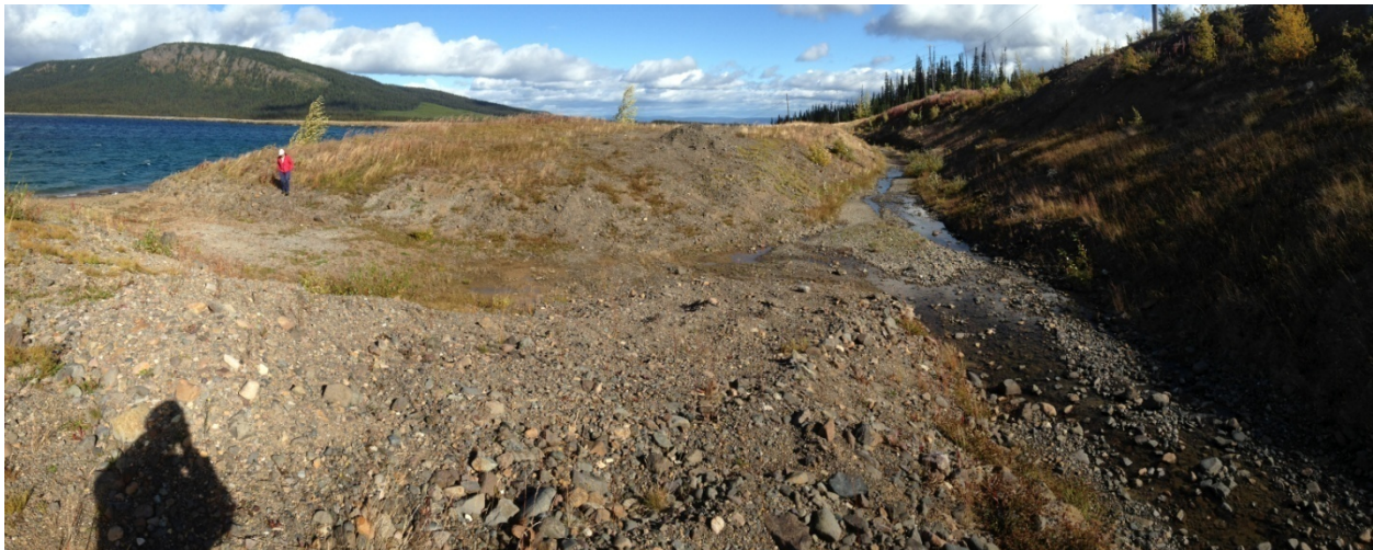
Photo 4: Tailings Impoundment spillway channel and outlet into Berzelius Diversion Channel. Taken 18 September 2014.
