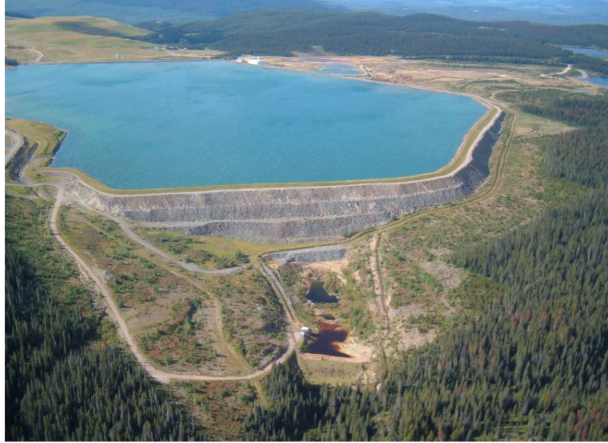
Photo 1: Aerial photograph of the Tailings Pond Dam No. 1 with Seepage Pond in foreground and treatment facilities in the background. Taken 29 August 2006.
