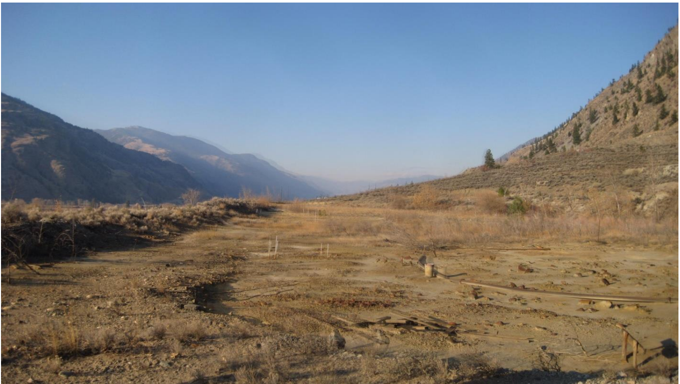
Photo 6. Tailings surface, taken from south dam crest looking north. Note standpipe piezometers.
