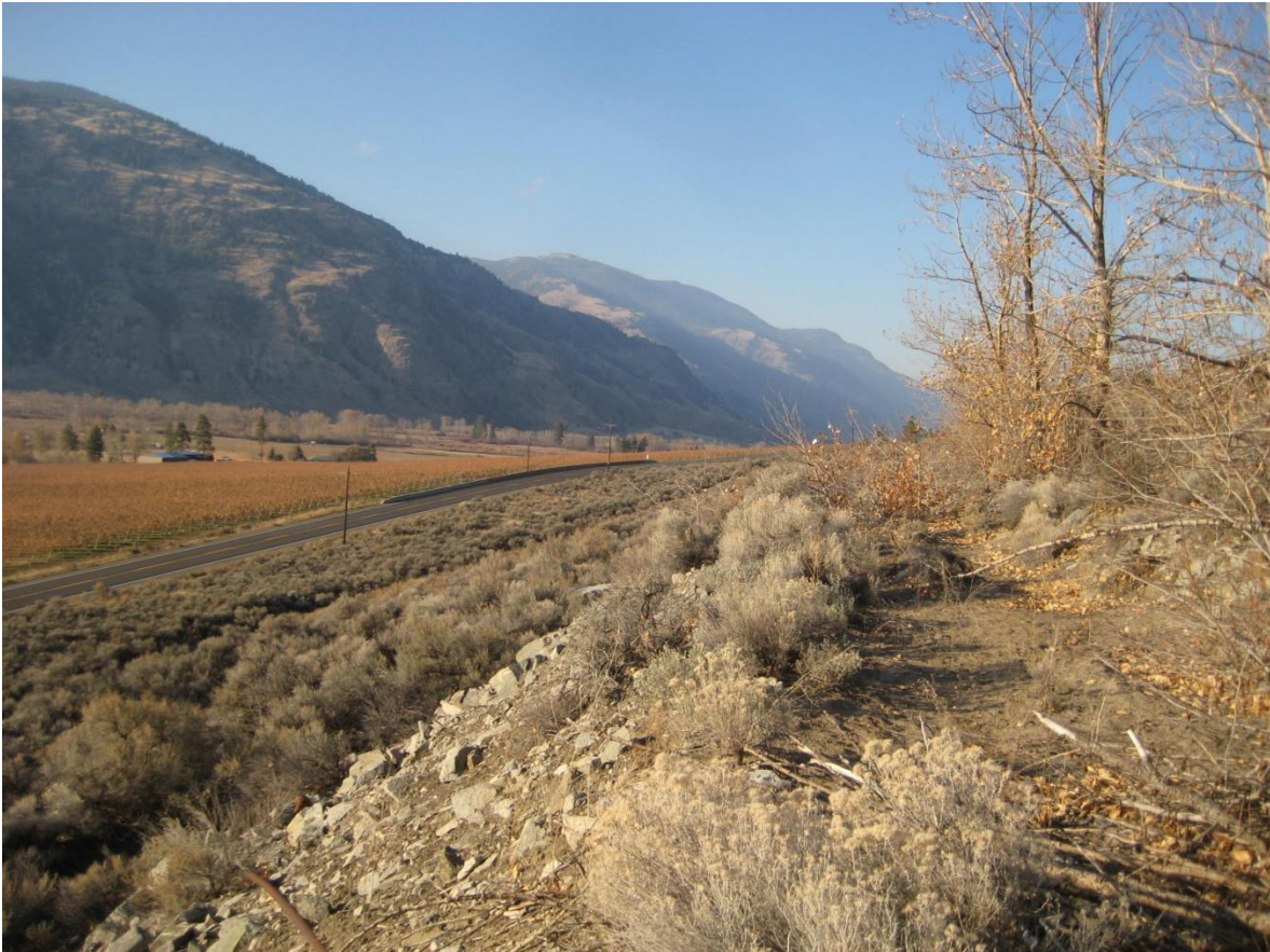
Photo 3. Downstream slope looking north. Highway 3 on left
