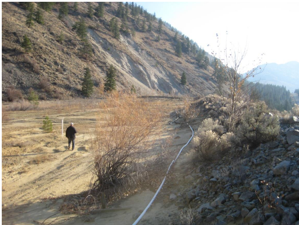
Photo 2. Crest of dam looking toward south abutment. Note standpipe piezometer on left
