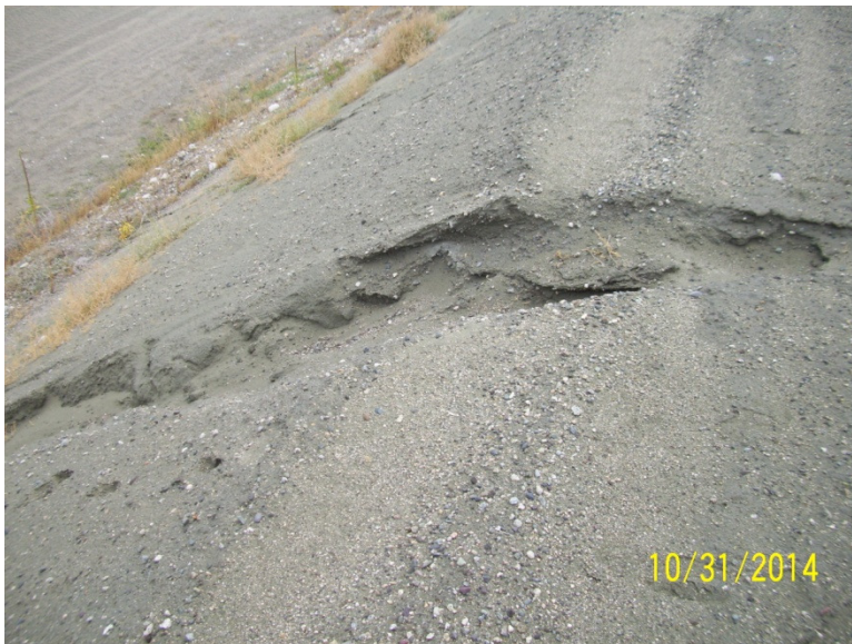
Photo 27 – West Tailings Facility (Dyke 4 Shoulder Erosion)
