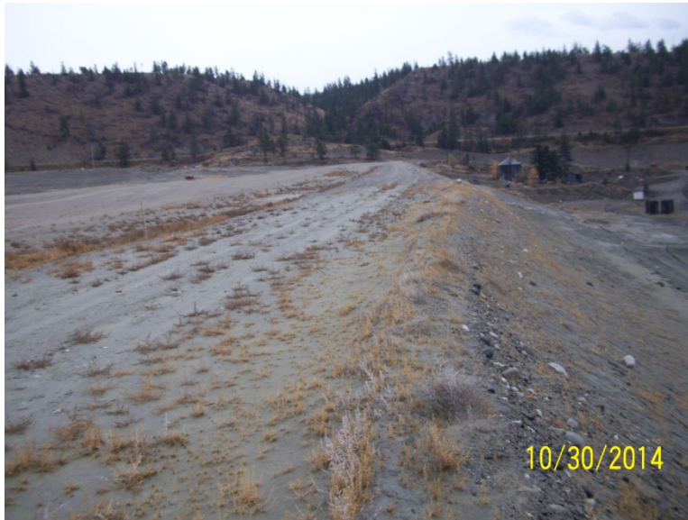
Photo 21 – Expanded Tailings Facility (Dyke 1)
