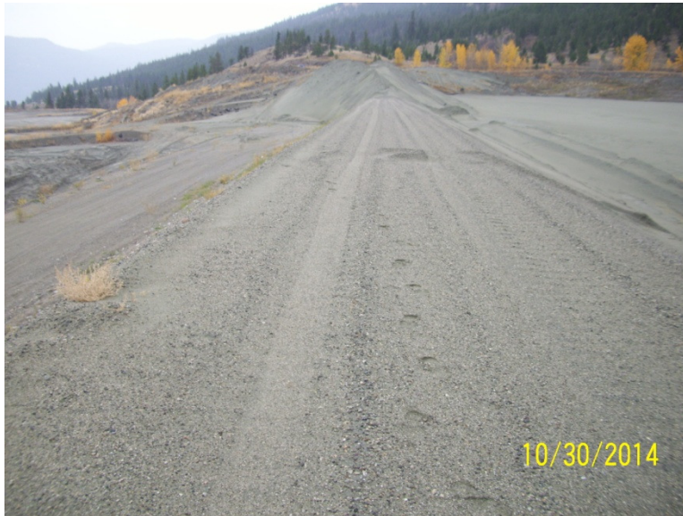
Photo 15 – West Tailings Facility (Dyke 4)
