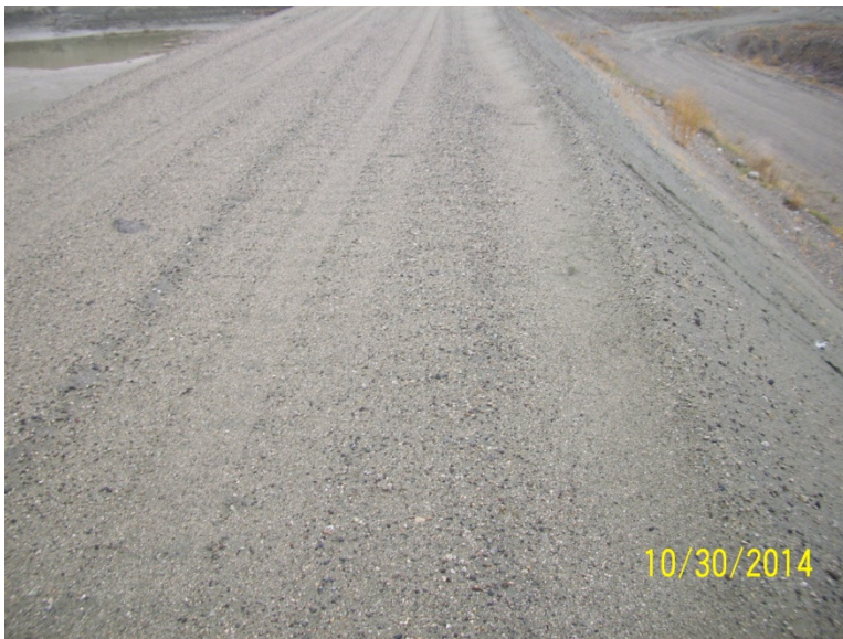
Photo 16 – West Tailings Facility (Dyke 4)
