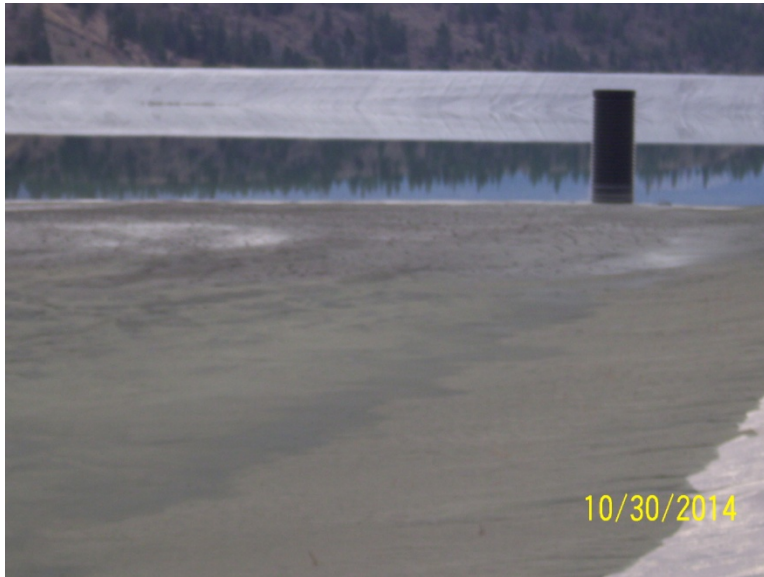
Photo 1 – Huldra Tailings Facility (Inside Pond)
