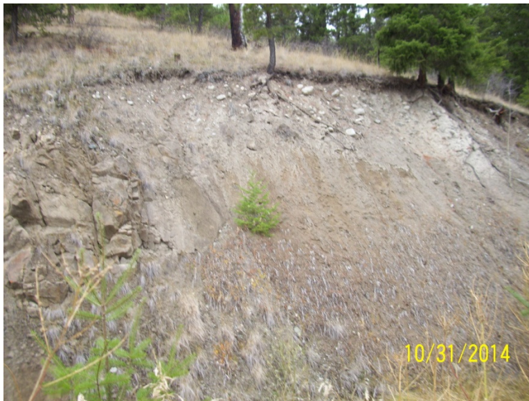
Photo 25 – Strumbles Creek Diversion Landslide
