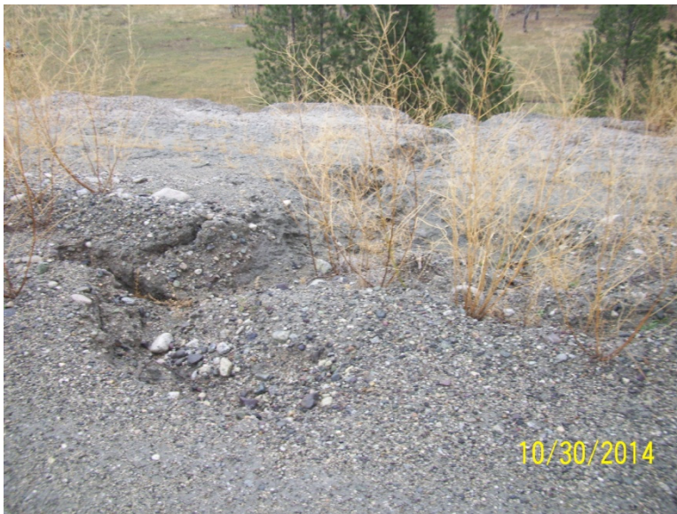
Photo 18 – Lower Tailings Facility (Erosion on Crest)
