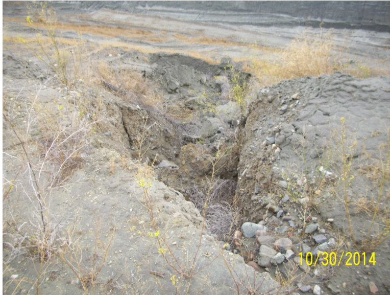
Photo 11 – Upper Tailings Facility (South Dam Downstream Gully)
