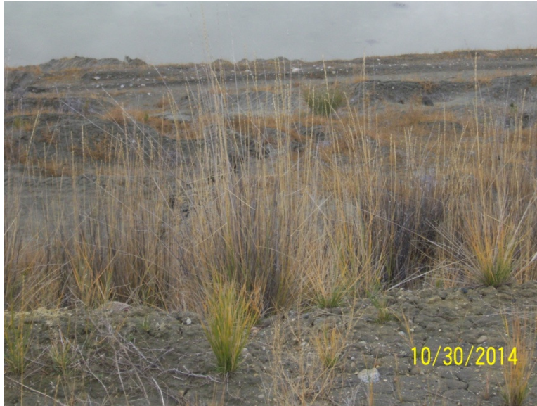
Photo 13 – Upper Tailings Facility (West Dam Downstream Vegetation)
