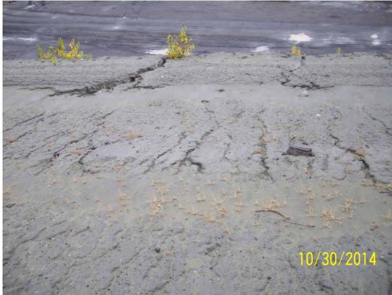
Photo 19 – Lower Tailings Facility (Downstream)
