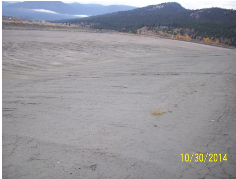
Photo 5 – Huldra Tailings Facility (Downstream Toe)
