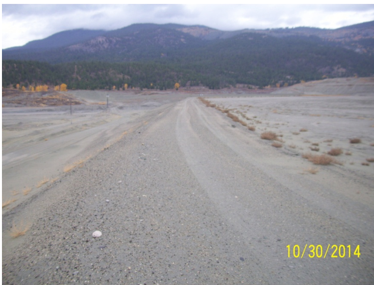
Photo 22 – Expanded Tailings Facility (Dyke 3)
