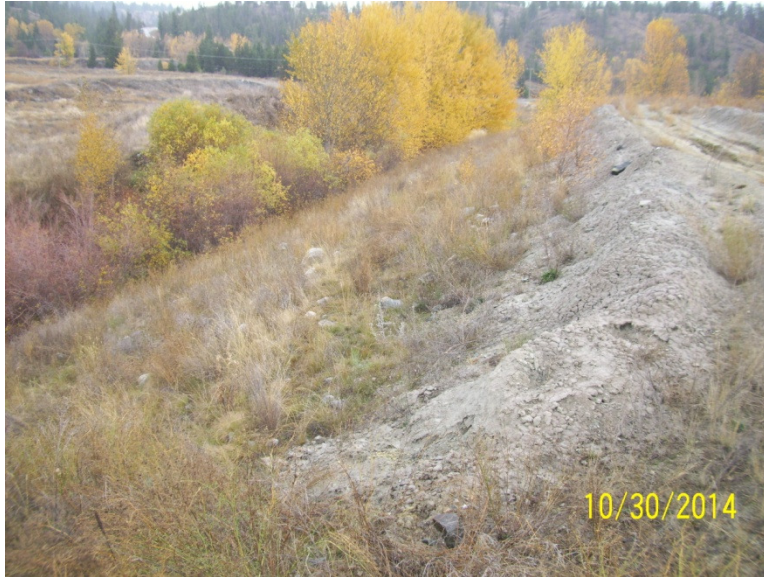
Photo 9 – Upper Tailings Facility (North Dam Downstream Vegetation)
