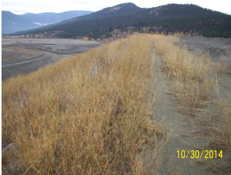
Photo 10 – Upper Tailings Facility (South Dam Crest)
