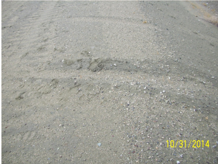
Photo 26 – West Tailings Facility (Dyke 4 Crest Erosion)
