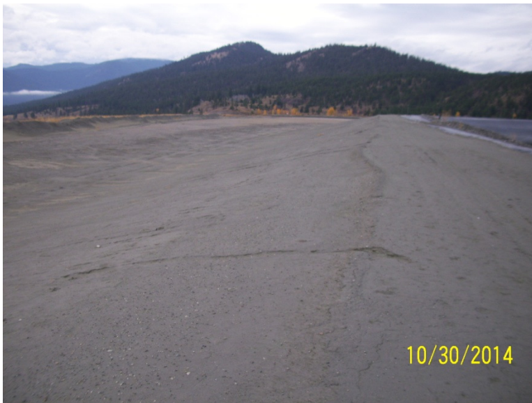
Photo 4 – Huldra Tailings Facility (Crest and downstream slope)
