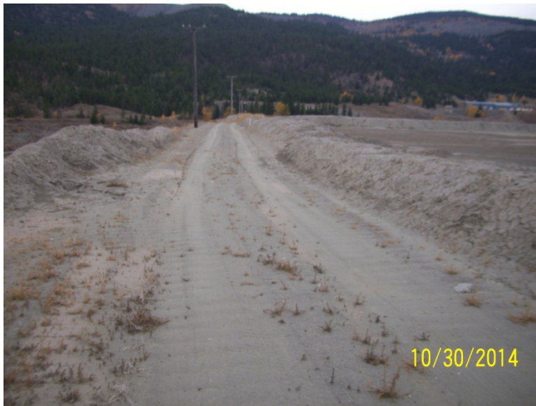
Photo 12 – Upper Tailings Facility (West Dam Crest)
