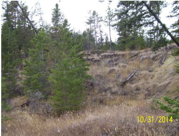
Photo 24 – Strumbles Creek Diversion Landslide
