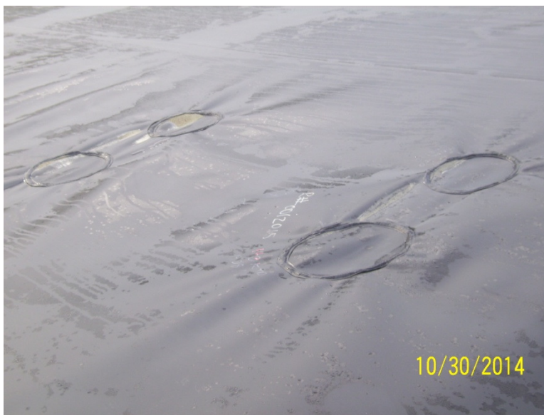
Photo 2 – Huldra Tailings Facility (Liner Repair)
