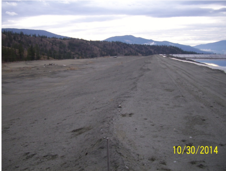
Photo 3 – Huldra Tailings Facility (Crest and downstream slope)
