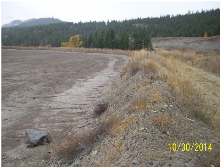
Photo 8 – Upper Tailings Facility (North Dam Upstream slope)
