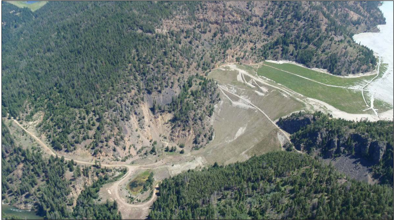
Figure 2.3: Aerial View of the West Dam Looking Northeast (July 2012)
