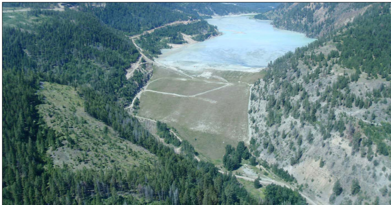
Figure 2.2: Aerial View of the East Dam Looking West (July 2012)
