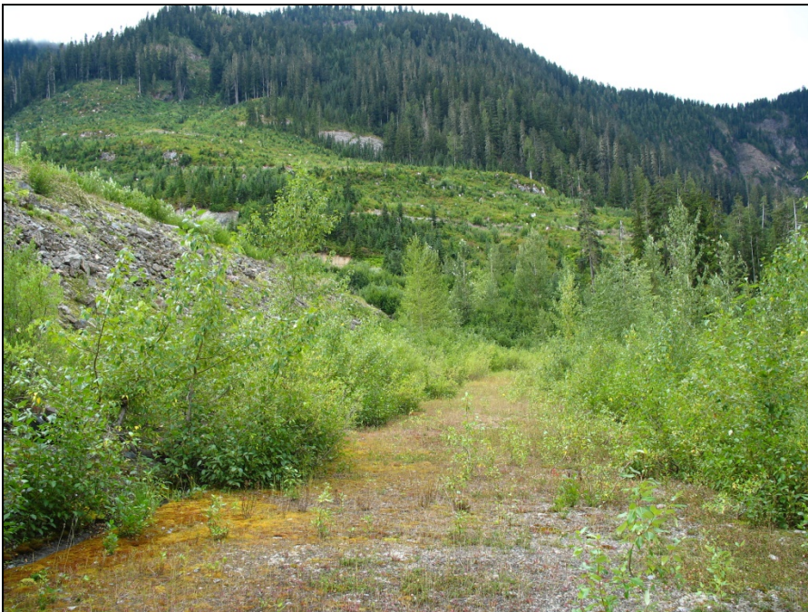
PHOTO 10 – Top of TSF downstream berm looking west.
