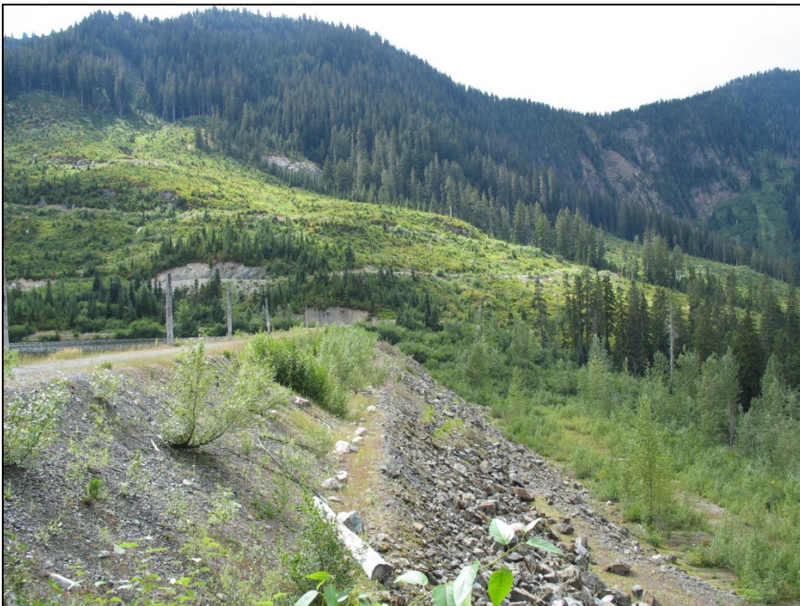
PHOTO 4 – TSF downstream slope looking west.
