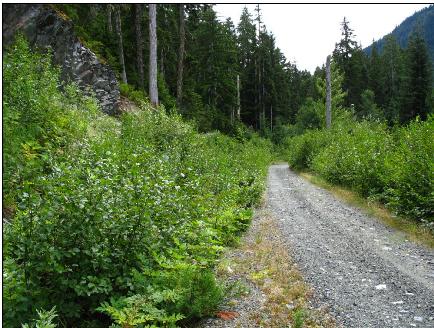
PHOTO 6 – Access road on east side of TSF. Diversion ditch on left side of access road.
