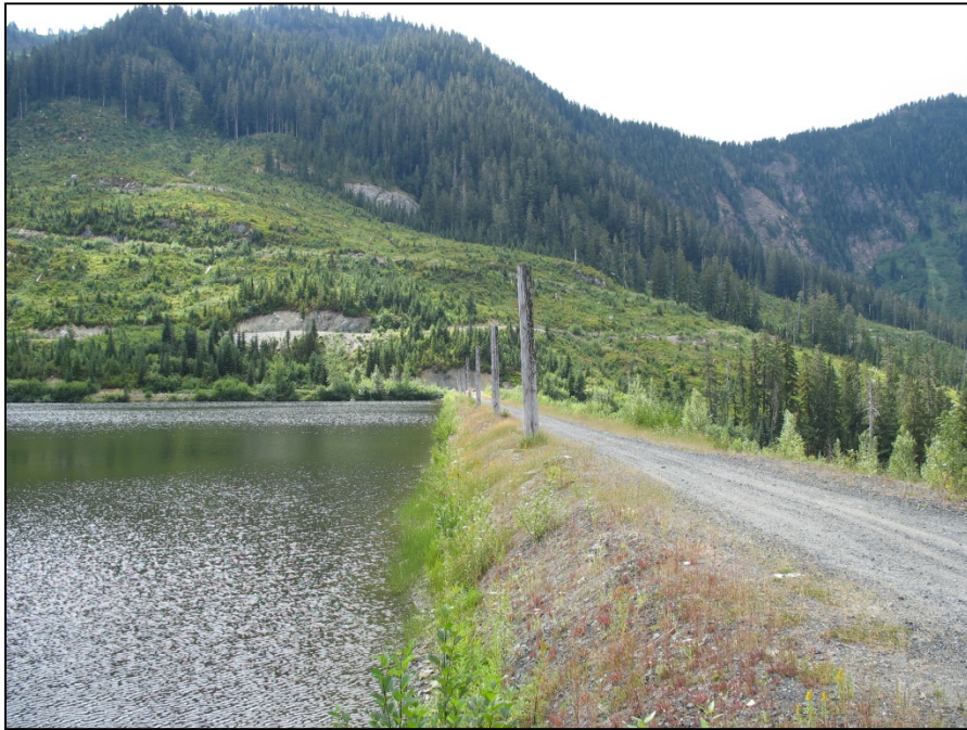
PHOTO 1 – Embankment crest looking west.
