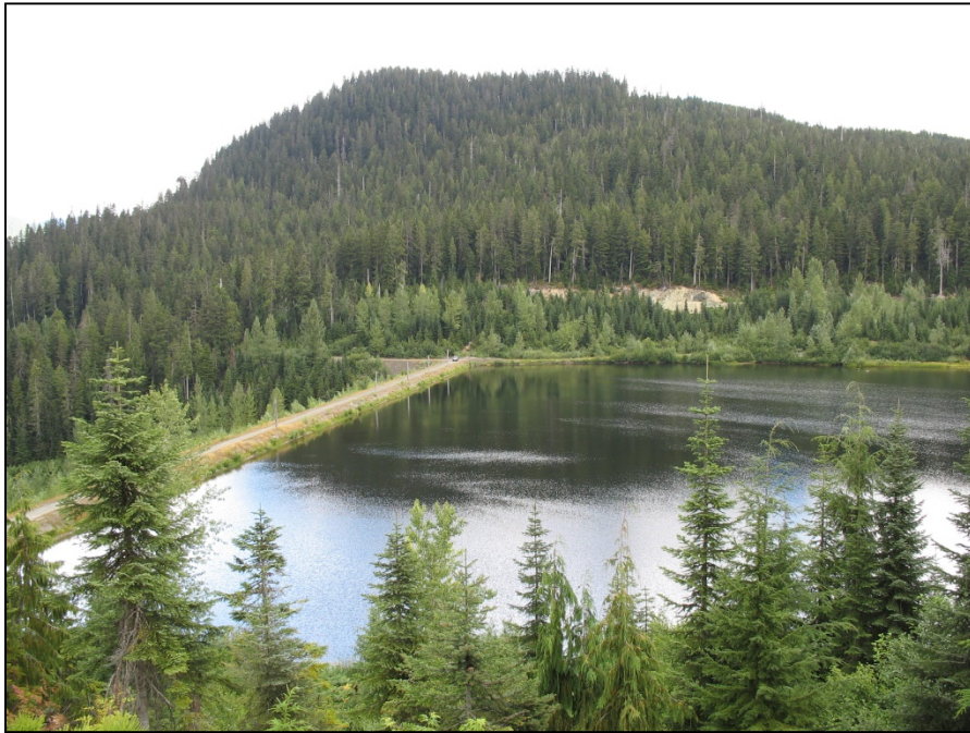
PHOTO 7 – TSF pond up against embankment. Looking East.
