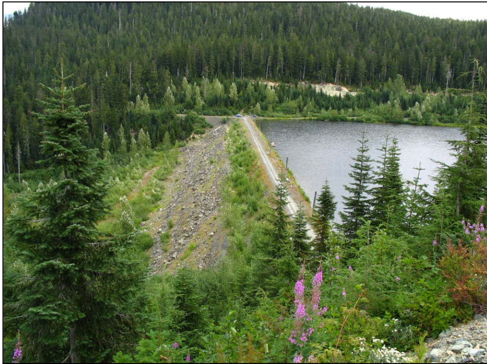
Figure 2.1 Photo of TSF from above Left Abutment
