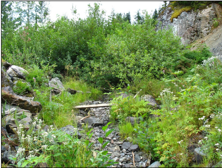
PHOTO 3 – TSF spillway channel looking upstream.
