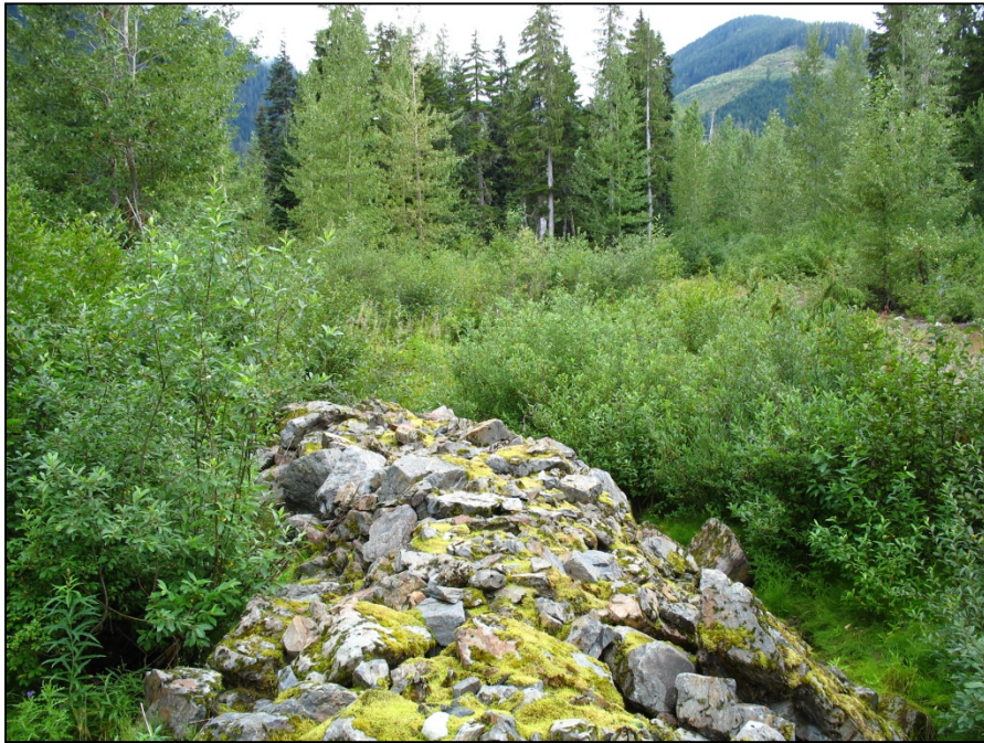
PHOTO 9 – Downstream rockfill finger drain.
