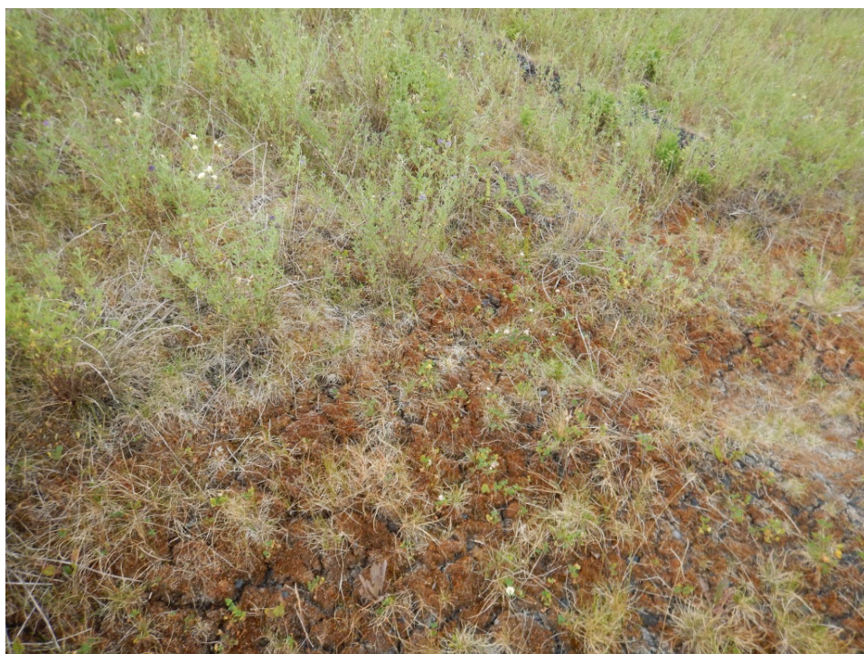
Photo I-9 Typical vegetation growth on downstream dam slopes. (TSF-2014-30)
