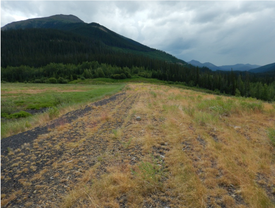
Photo I-4 Dam crest, looking north. (TSF-2014-09)
