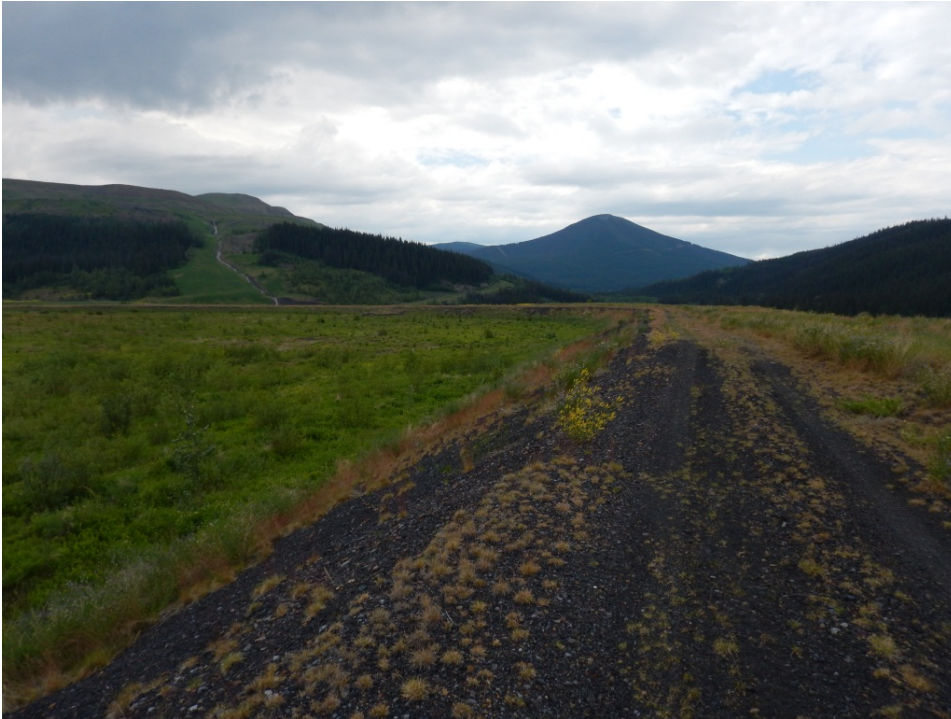
Photo I-2 Overview of dam crest and vegetated tailings surface, looking west. (TSF-2014-05)
