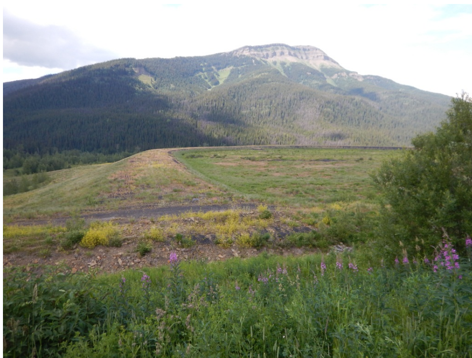
Photo I-8 West Dam overview with spillway channel in foreground, looking north. (TSF-2014-20)
