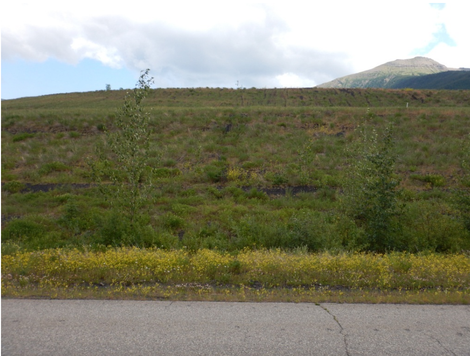
Photo I-17 Overview of downstream slope, looking east. (TSF-2014-24)
