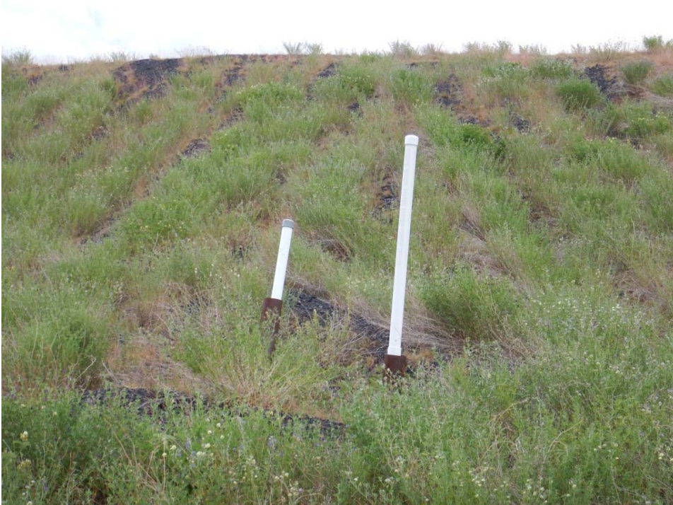
Photo I-11 Piezometer standpipes (no labels). Shallow rilling present (<1 m deep) in well vegetated downstream slope. (TSF-2014-02)
