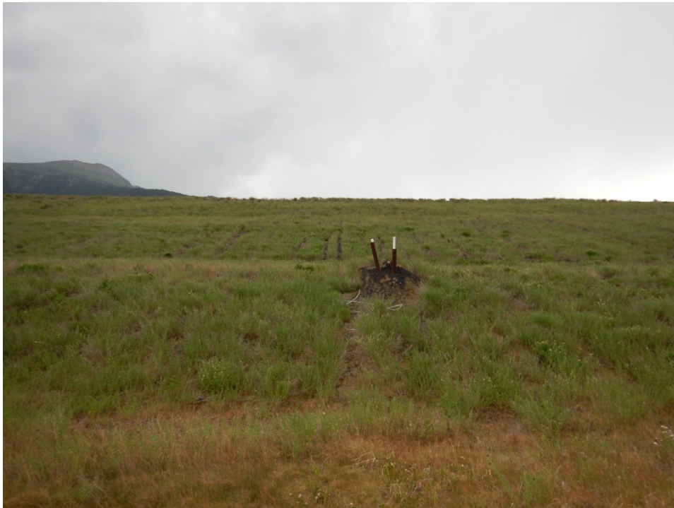
Photo I-13 Standpipe piezometers (PB-4 and PB-5) and overview of downstream slope, looking south. (TSF-2014-08)
