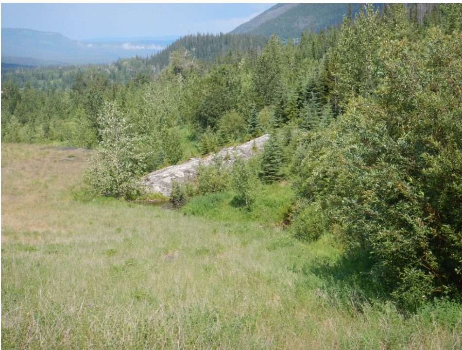
Photo I-19 East abutment downstream slope with mine road visible (light grey structure). Local surface water flows along contact between dam fill and native ground. The area is well vegetated and no visual sign of active significant erosion. (TSF-2014-15)
