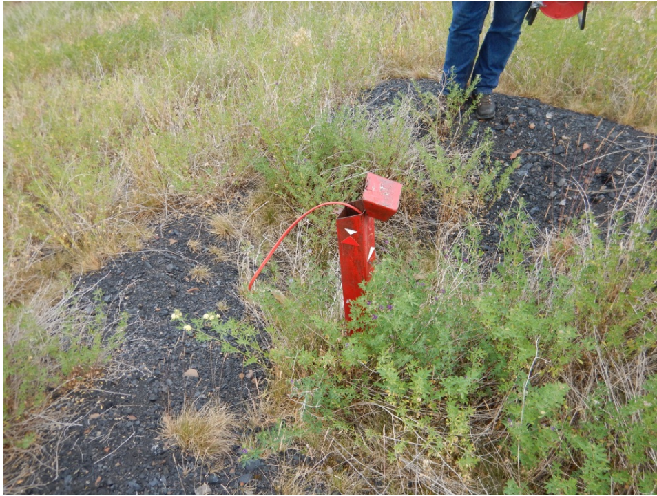
Photo I-12 Pneumatic piezometer (PC-4N). (TSF-2014-03)
