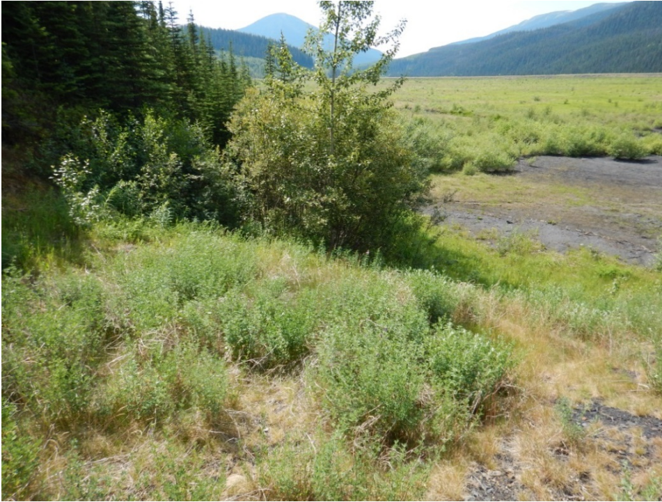
Photo I-20 East abutment upstream slope. (TSF-2014-15)
