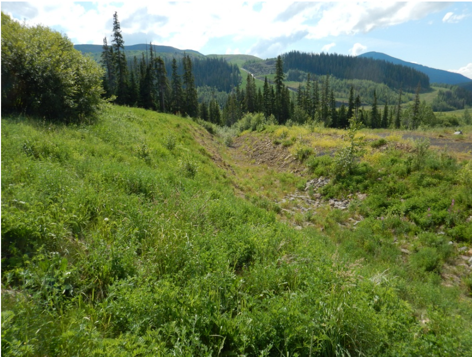
Photo I-7 Section of spillway channel that is excavated through tailings surface and dam crest at West Abutment. (TSF-2014-19)
