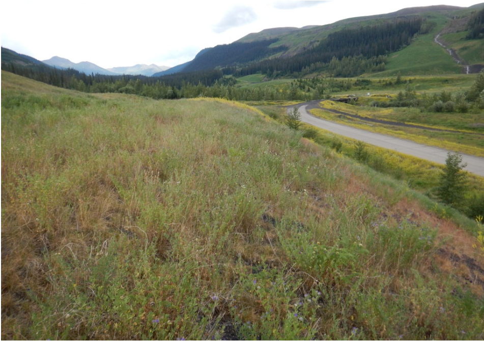
Photo I-18 Overview of downstream slope, looking west. (TSF-2014-24)
