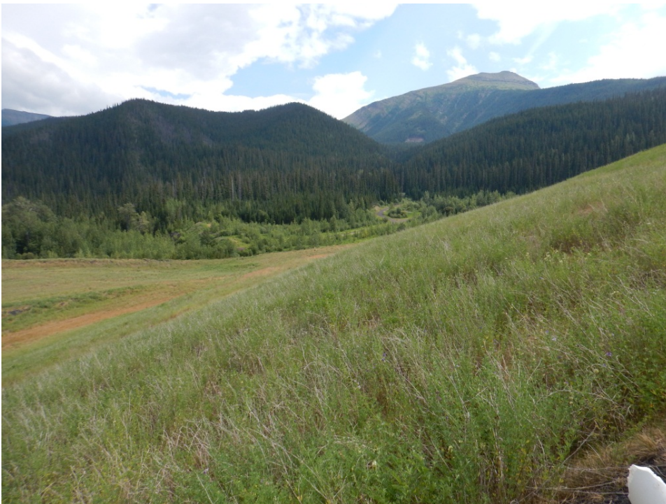
Photo I-15 Overview of downstream slope, looking south. (TSF-2014-10)
