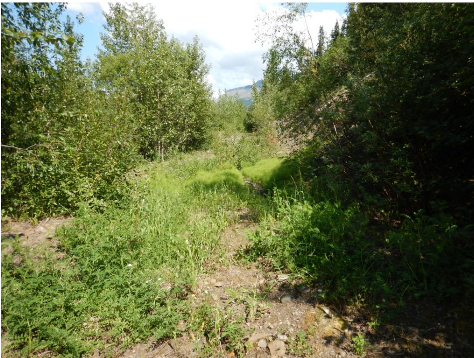
Photo I-21 Diversion channel upslope of impoundment. The diversion channel is so heavily overgrown it is difficult to identify in the field. (TSF-2014-18)
