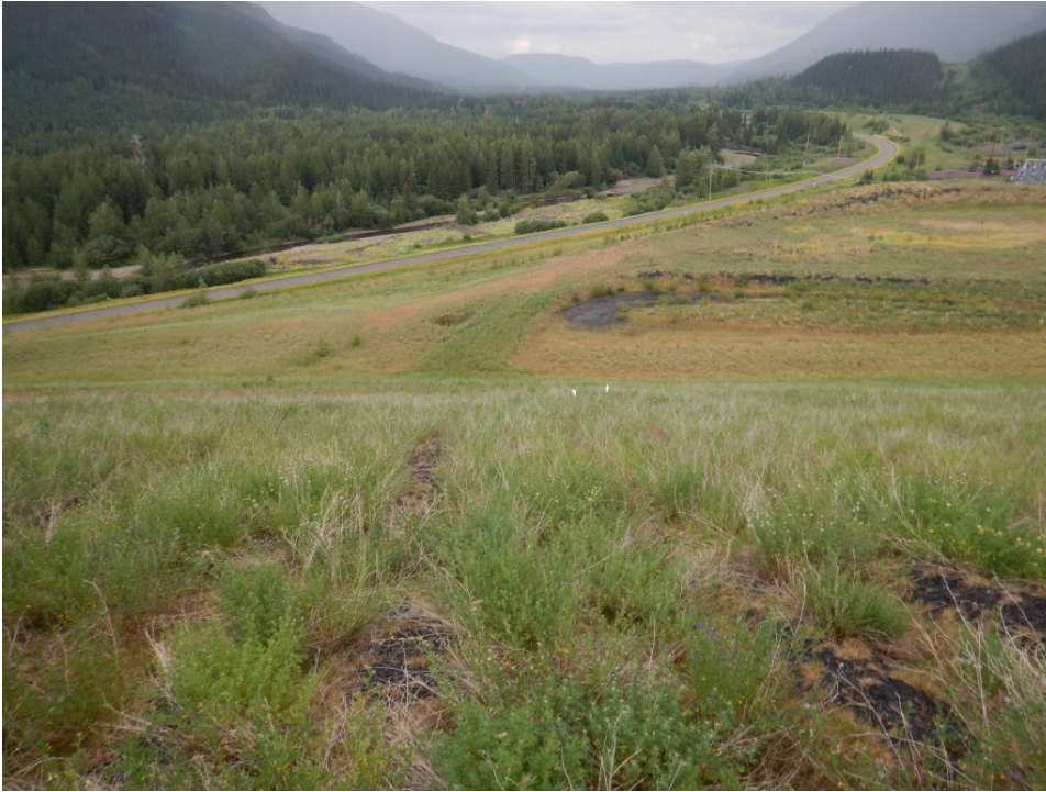
Photo I-16 Downstream slope and toe area, looking east. Reclaimed structure, appears to be a pond, visible at dam toe. (TSF-2014-09)
