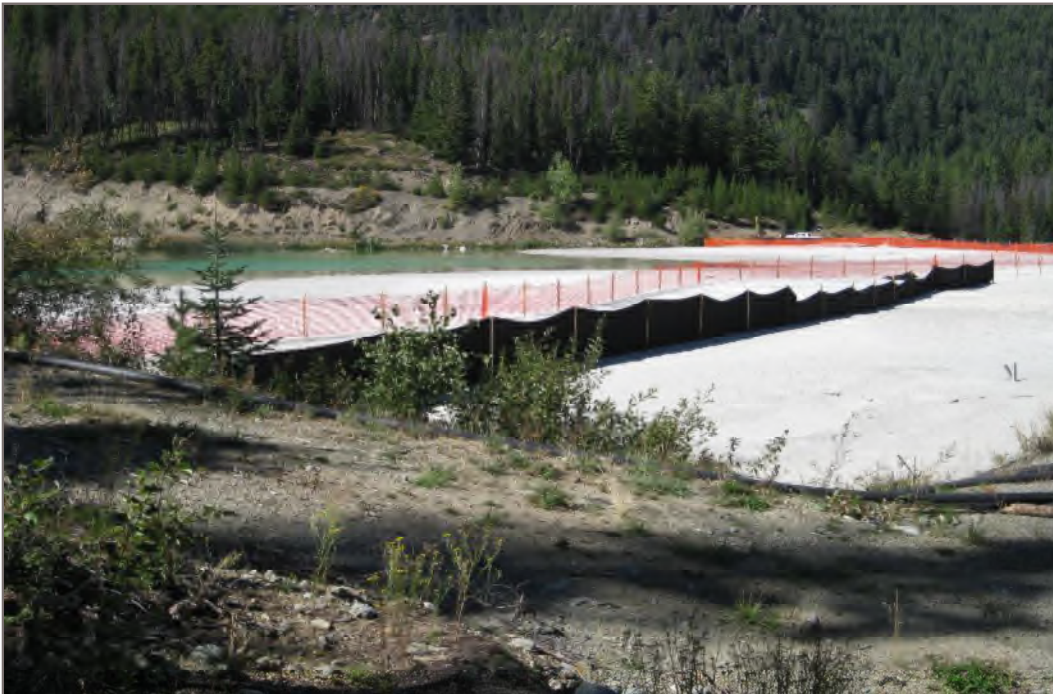
Photo 4: Tailings beach with wind fence, looking north from south abutment
