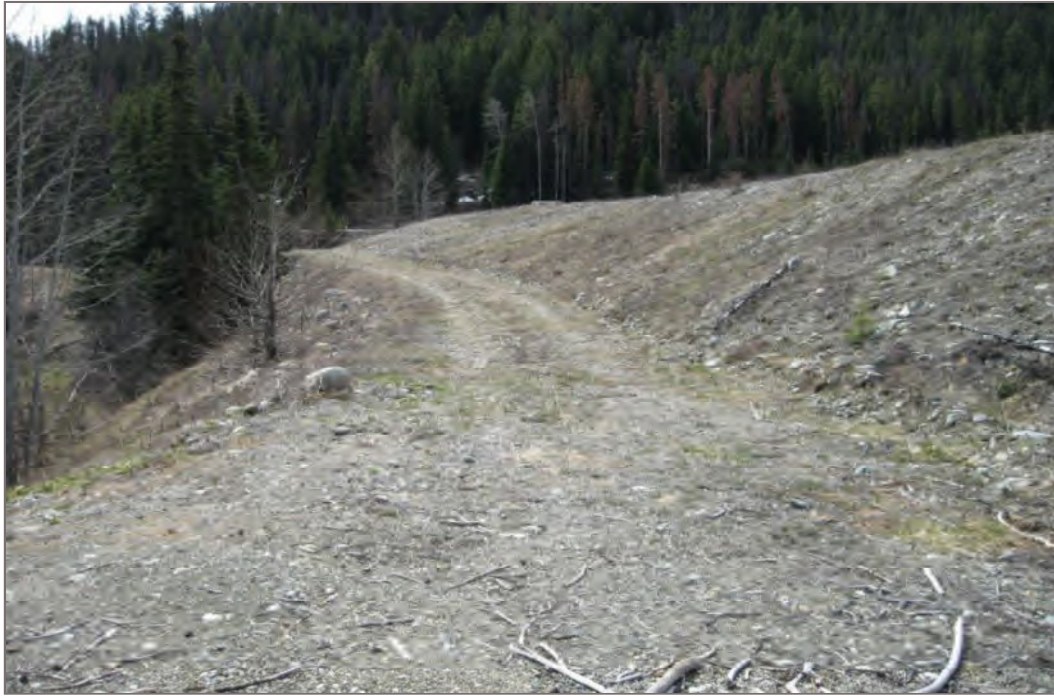
Photo 7: Downstream embankment bench, looking south – Note: variable batter slope
