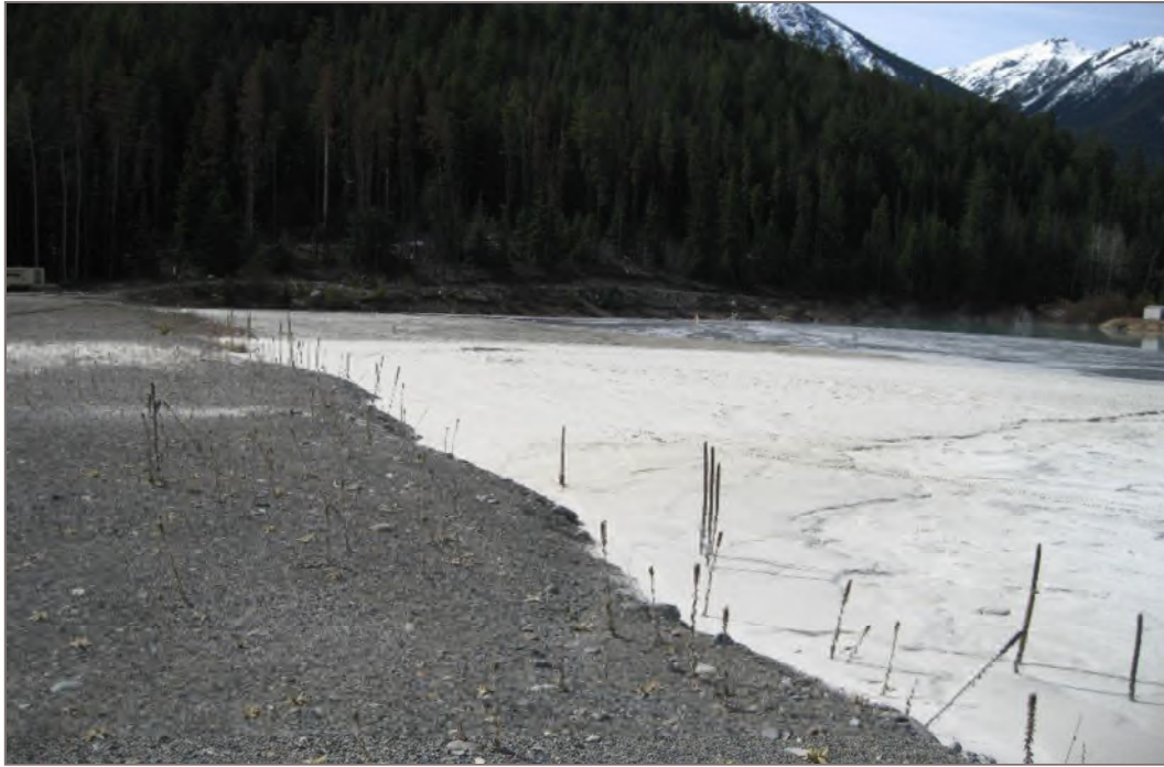
Photo 3: Embankment crest and beach development, looking toward south abutment
