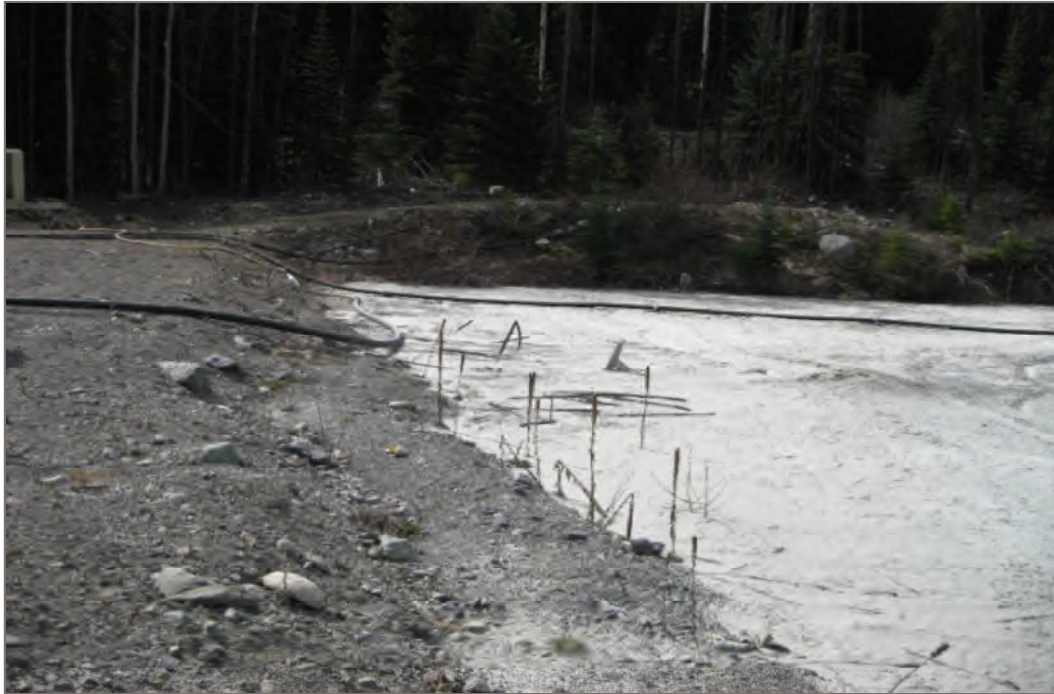
Photo 11: Tailings beach at south abutment
