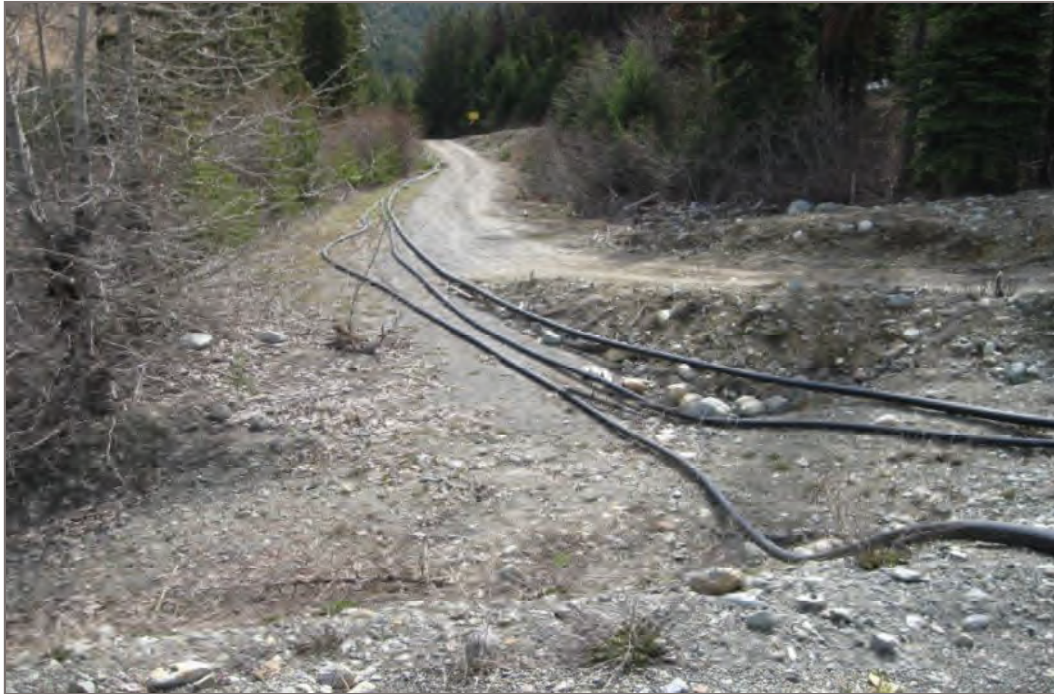
Photo 19: Tailings slurry line and underground water lines
