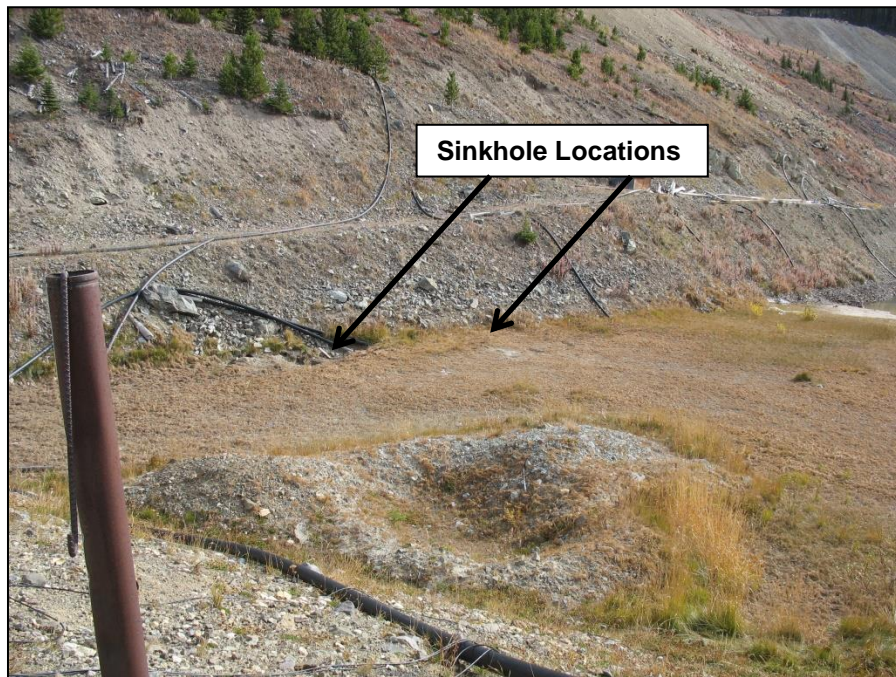
PHOTO 16 – Tailings beach near right abutment where sinkholes have been previously identified.
