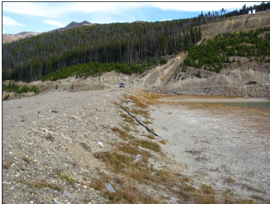
PHOTO 3 – View of tailings beach and upstream face of embankment looking east.
