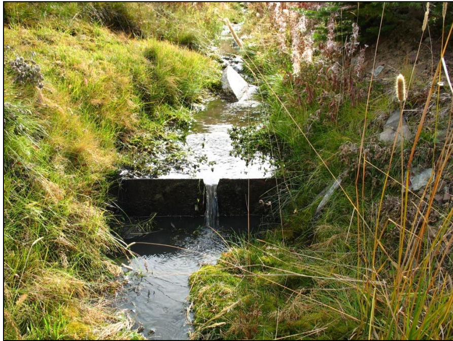
PHOTO 7 – View of flow through Weir 2 located on east side of TSF embankment.
