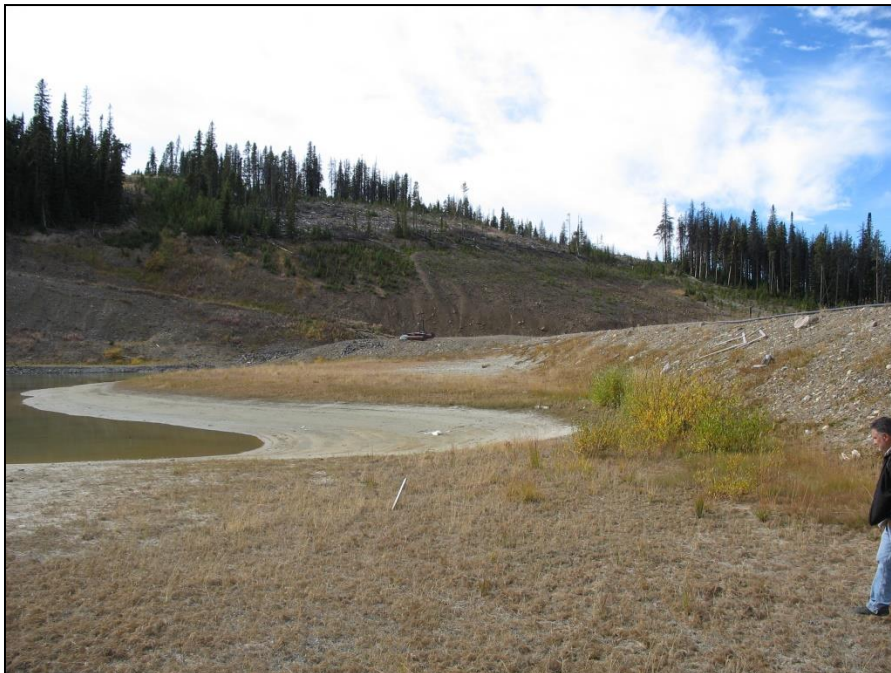
PHOTO 2 – View of tailings beach and upstream face of embankment looking west.
