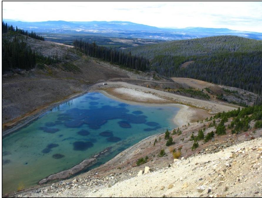
PHOTO 1 – View of tailings pond and embankment crest.
