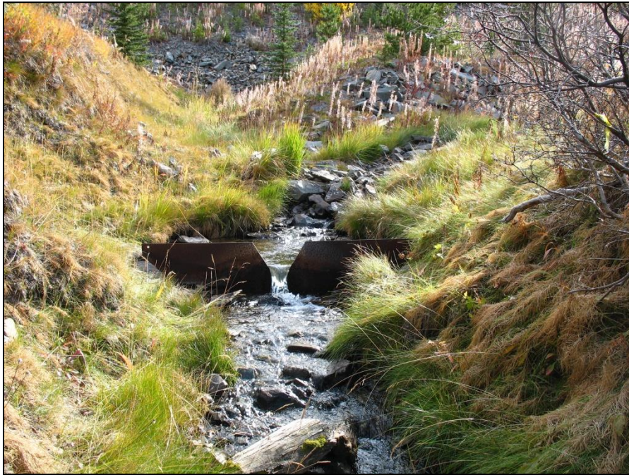
PHOTO 9 – View of flow through Lou Creek Weir located downstream of the Seepage Collection and Recycle Pond.
