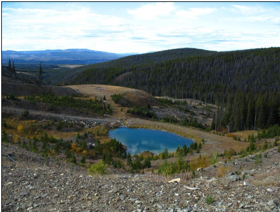
PHOTO 8 – View of Seepage Collection and Recycle Pond.
