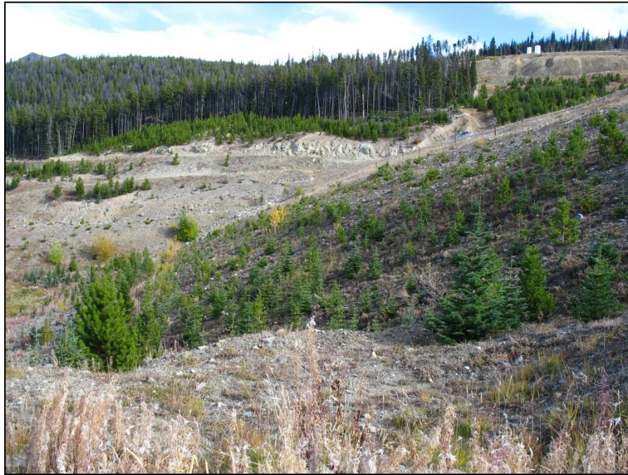
PHOTO 5 – View of tailings embankment downstream slope looking east.
