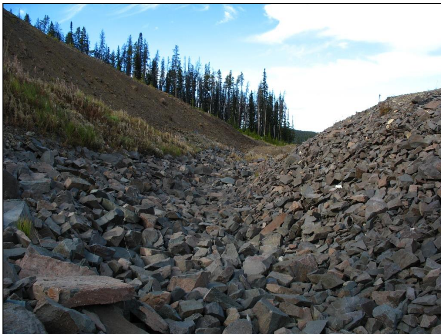
PHOTO 10 – View of spillway on left abutment looking downstream.
