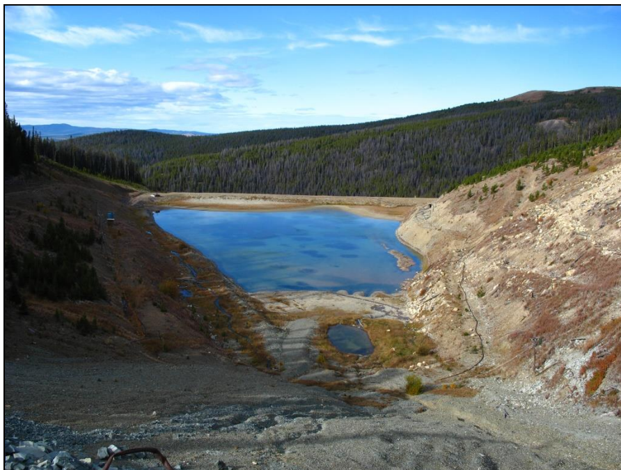
PHOTO 12 – View of Embankment Crest from south end of the facility.
