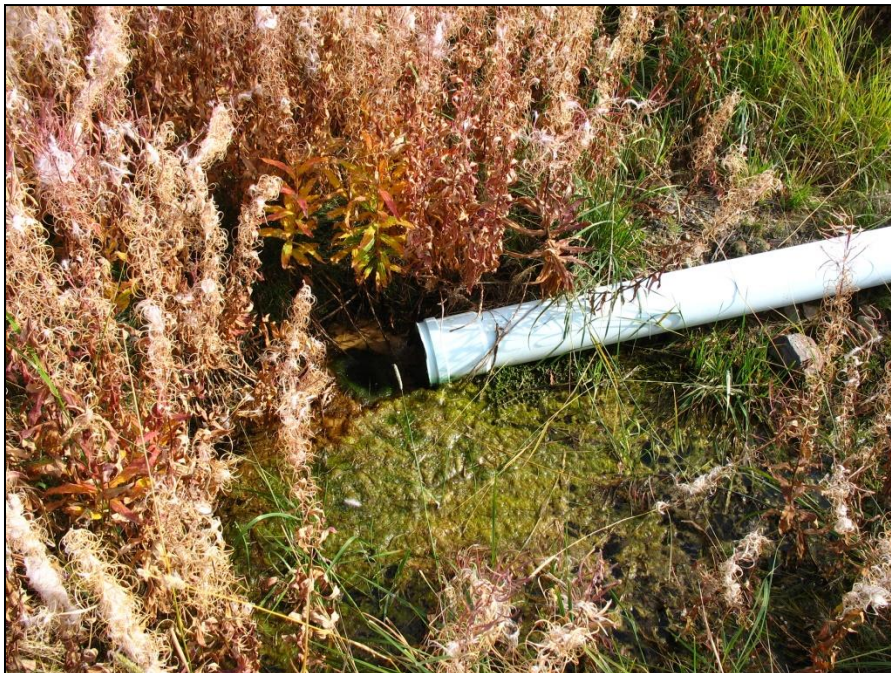
PHOTO 14 – Flow from upstream drain discharge pipe.
