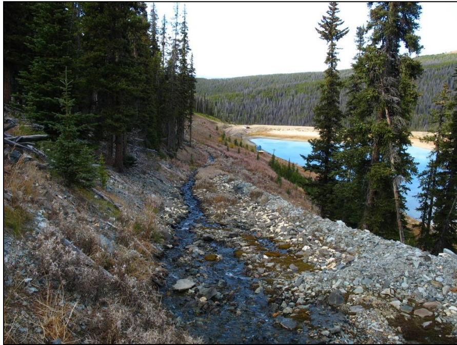
PHOTO 13 – South Diversion ditch looking downstream.
