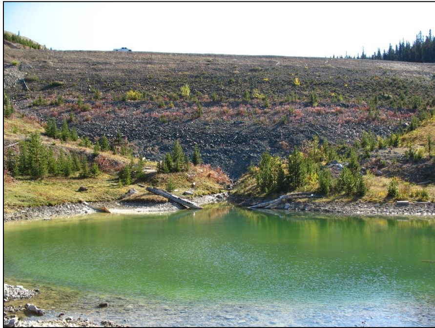
PHOTO 17 – Downstream slope of TSF embankment with Seepage Collection and Recycle Pond in foreground. Photo from 2012.
