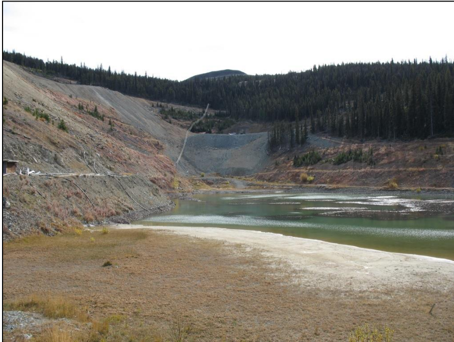
PHOTO 15 – TSF looking upstream from crest near right abutment.
