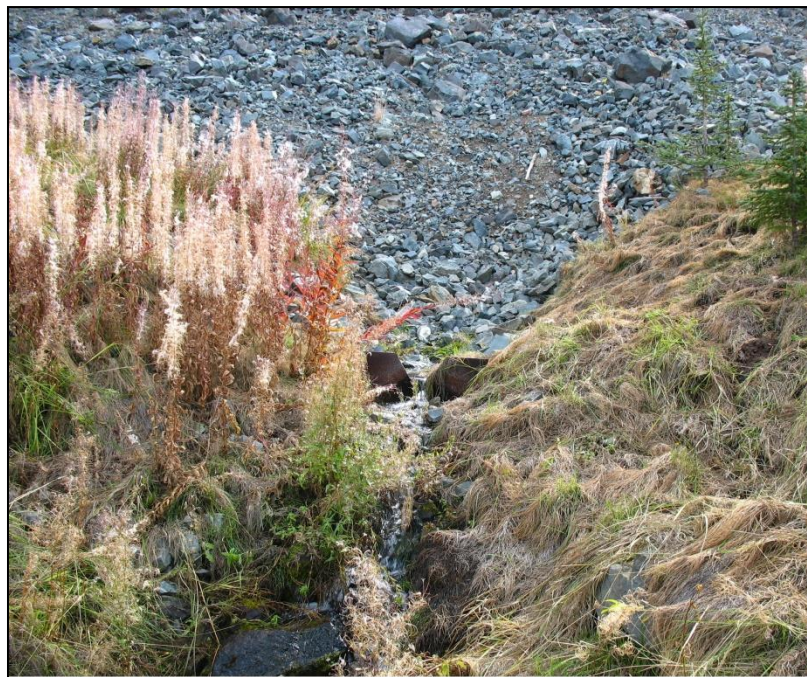
PHOTO 6 – View of flow through Weir 1 located downstream of TSF embankment.
