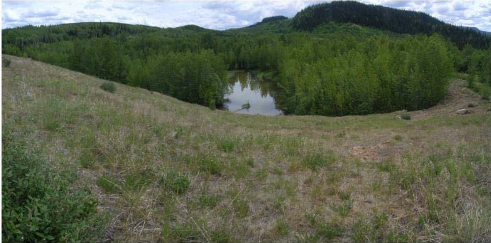
Photo C2-2: View of downstream slope and toe of Dam 2, looking south from about mid-way along its length. Water ponded at toe is not part of the seepage collection system. (11 June 2014)
