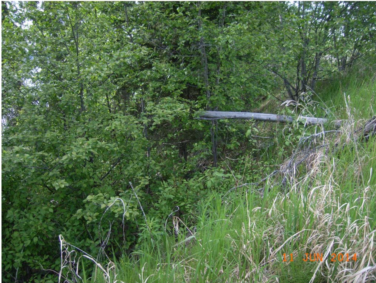
Photo D1-4: Close up view of CP1-3 downstream slope, looking north from south portion of the western segment of the dam. Note the downstream slope is heavily vegetated. (11 June 2014)
