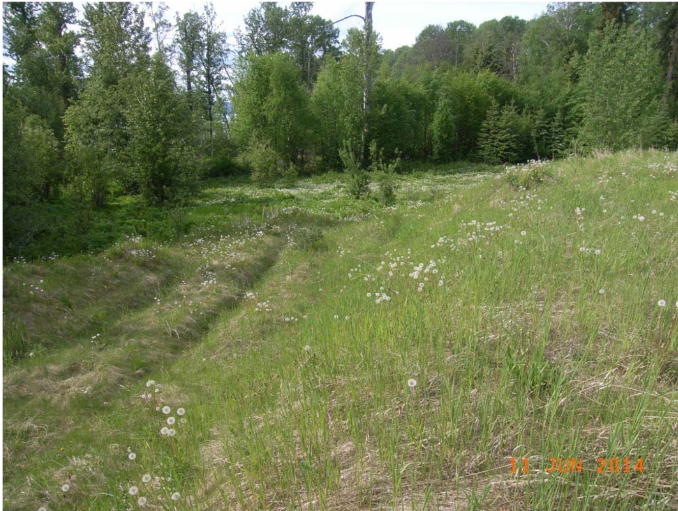
Photo D2-5: View of downstream slope and toe of CP1-5, west from the crest. Note there are no signs of adverse seepage. (11 June 2014)
