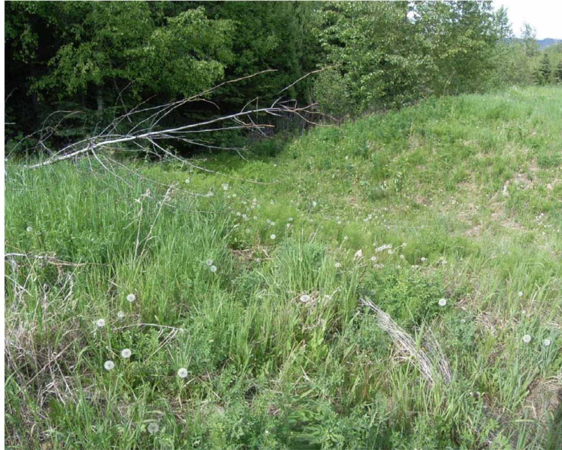
Photo D7-5: View of downstream slope of CP8 Dam, looking east from west end of north dam, note heavy vegetation (11 June 2014)
