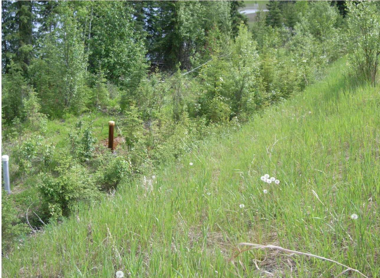
Photo D5-3: View of downstream toe of CP5 Dam, showing monitoring wells. Along east toe of the dam, looking southeast Note that one of the wells has water flowing over the top of the well casing. (11 June 2014)
