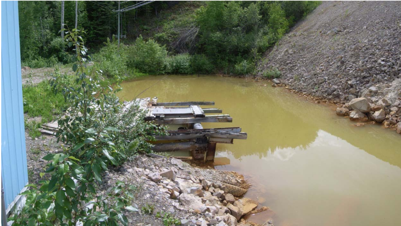
Photo D3-3: The wooden frame is around pipes that discharge water to the environment when the water is high enough to flow through them. . (11 June 2014)
