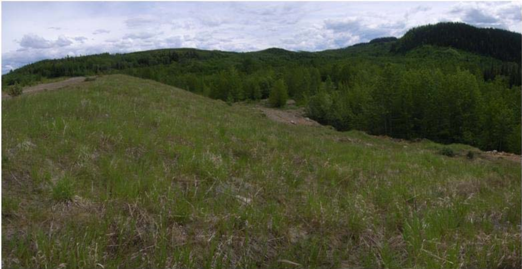
Photo C2-1: View of downstream slope of Dam 2, looking east from west end of the dam. Note the slope is well vegetated. (11 June 2014)
