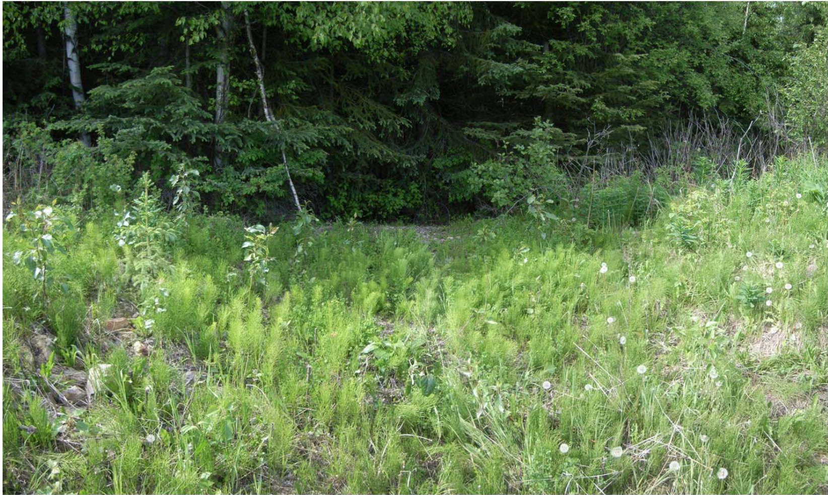
Photo D7-4: View of CP8 spillway, looking north from the crest along the spillway located mid-way along the north dam. Note lack of erosion protection in the spillway. (11 June 2014)
