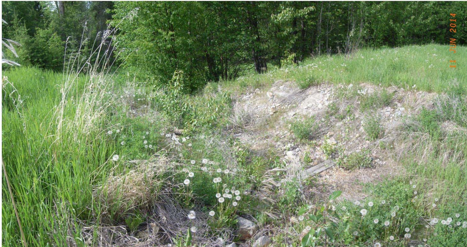
Photo D2-2: View of CP1-5 spillway, looking north from crest of the dam. Note small and irregular size of the erosion protection. (11 June 2014)
