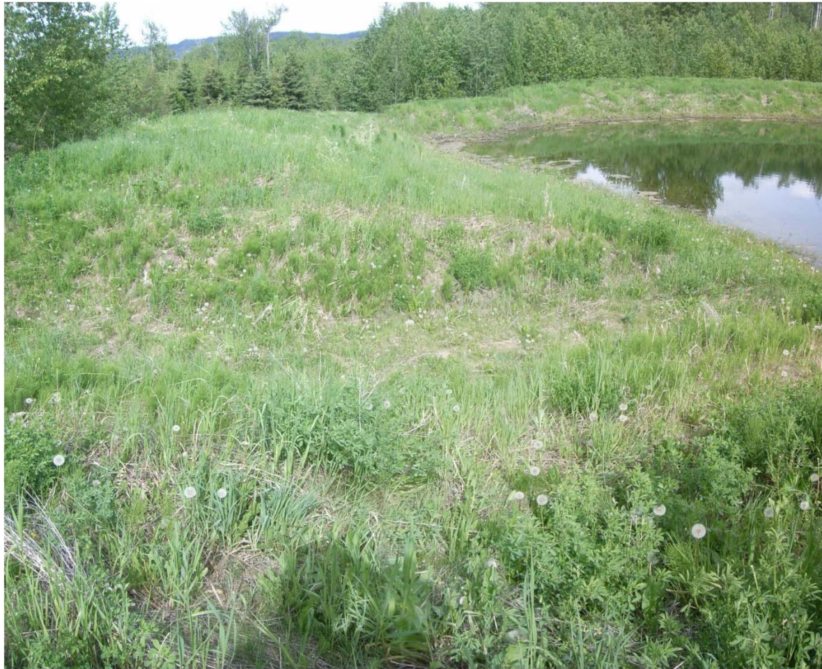
Photo D7-3: View of crest of CP8 Dam, looking east from west end of the north dam. Note spillway in the foreground and low area of the crest in the background. (11 June 2014)
