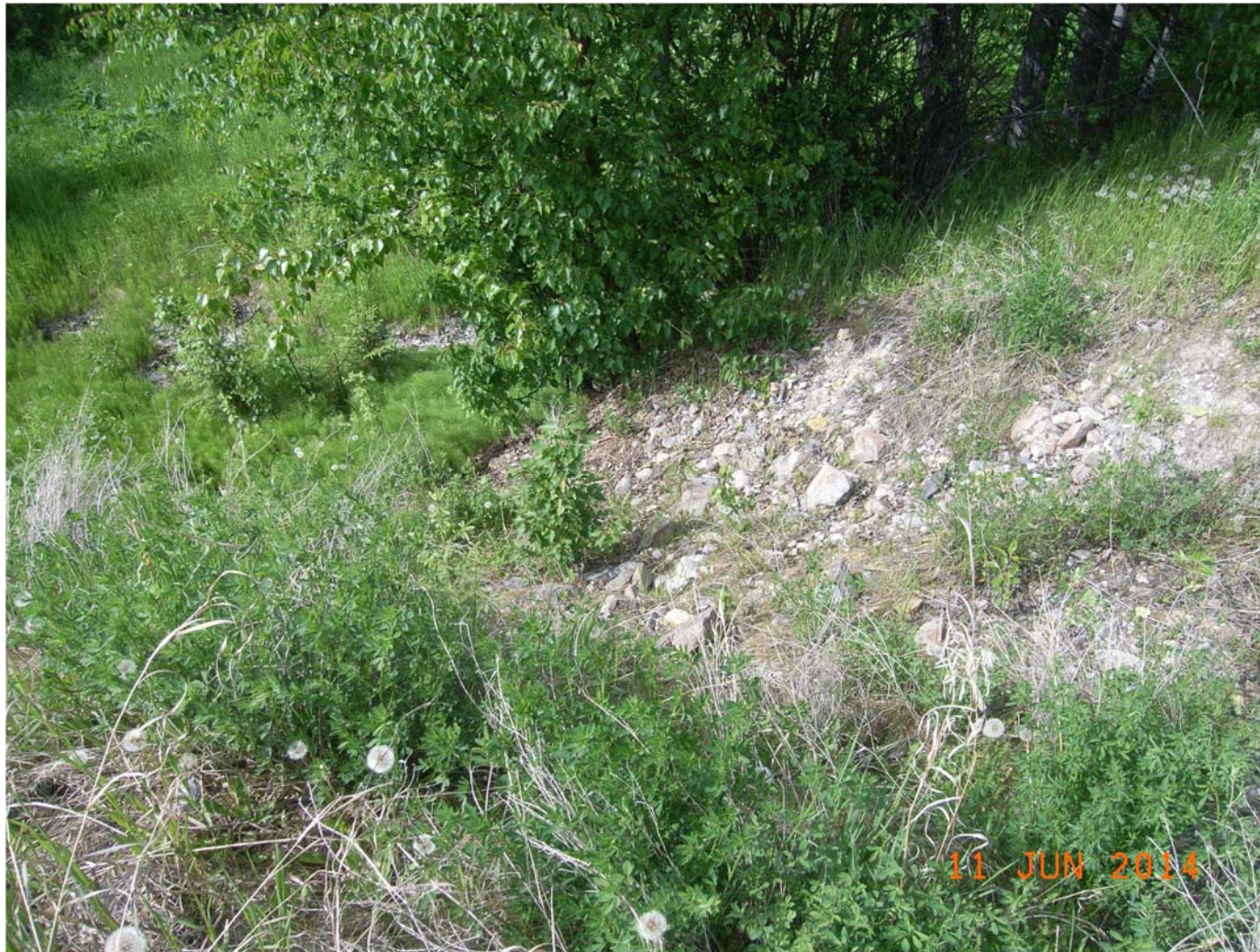
Photo D2-3: View of downstream end of spillway at CP1-5, looking north west from within the spillway. Note small size of the erosion protection (11 June 2014)
