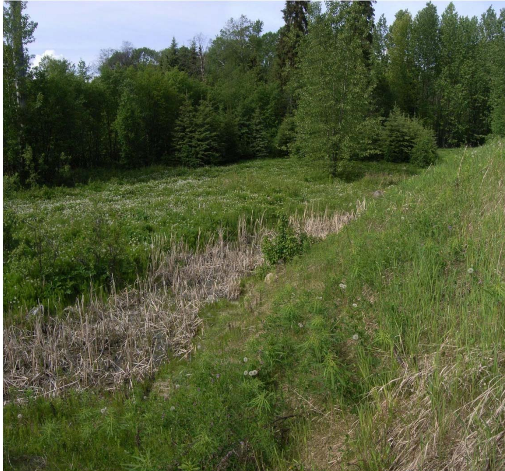
Photo D2-6: View of downstream slope and toe of CP1-5, north from crest of west segment. Note there are no signs of adverse seepage. (11 June 2014)
