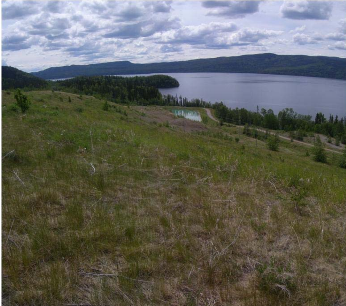
Photo C1-8: View of downstream slope and toe of Dam 1, looking south from about midway along the dam crest. Note good vegetation and CP1-3 in the background. (11 June 2014)
