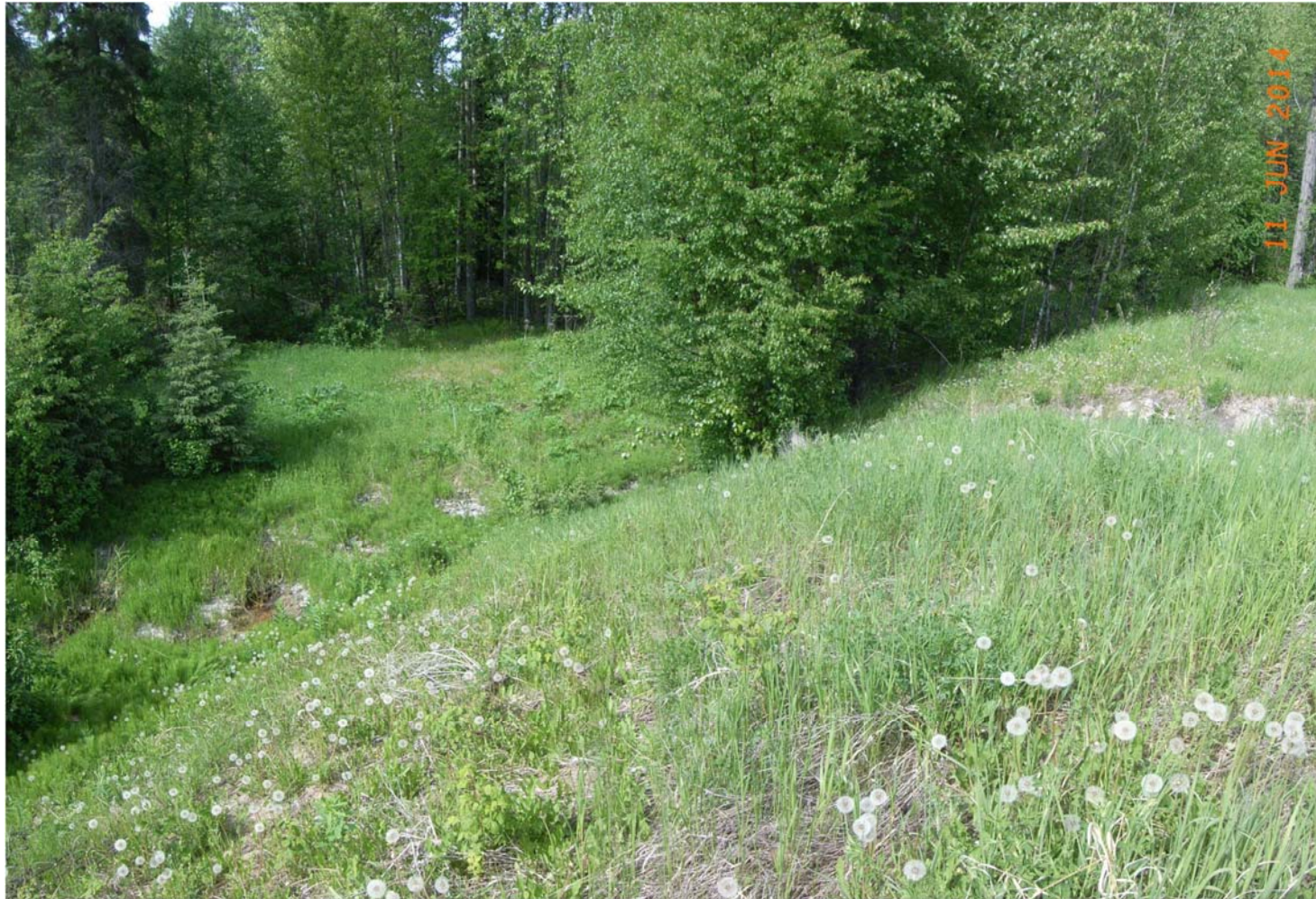
Photo D2-4: View of downstream slope and toe of CP1-5, looking north from crest of west segment. Note there are no signs of adverse seepage. (11 June 2014)
