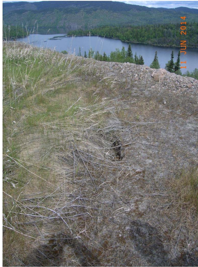
Photo C3-5: Close up view of sinkhole on the downstream side of the crest. Note that this area is a topographic low where water can accumulate and flow downward into the rockfill shell of the dam. The sinkhole has formed in the soil cover material over the rockfill. (11 June 2014)
