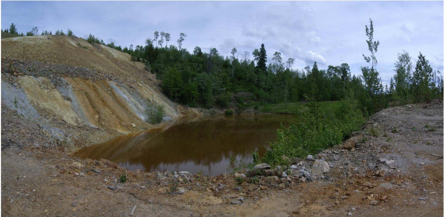
Photo C7-2: View of downstream slope of Dam 7, on the left side of Collection Pond CP7-1, looking east from the west end of the CP7-1 pond. This was an area where there was a concern with respect to erosion on the downstream slope noted in the 2013 DSI. There was no significant change from 2013. (11 June 2014)
