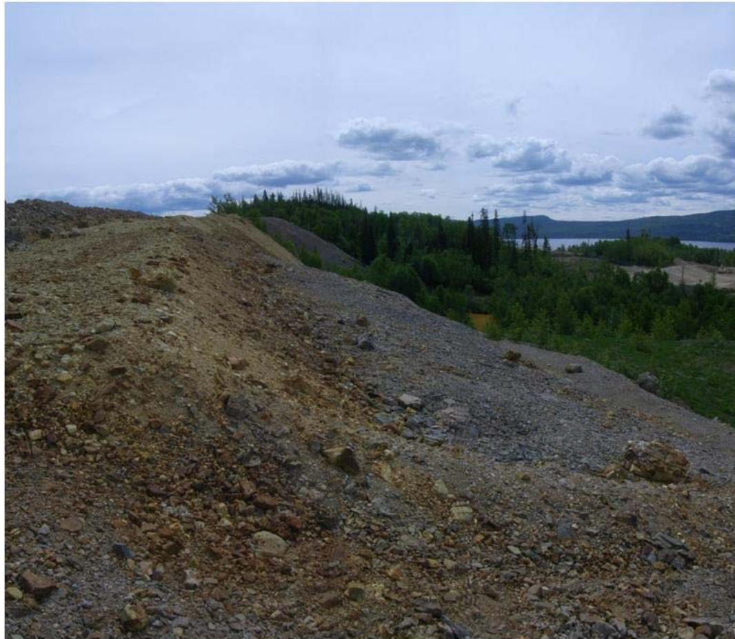
Photo C1-4: View of downstream slope of Dam 1, looking south from north end of the dam. Note the slope showing rockfill comprising dam shell. (11 June 2014)
