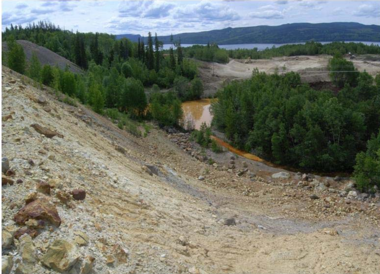
Photo C1-6: View of downstream slope and toe of Dam 1, looking south from north end of the dam. Note CP1-5 in the background. (11 June 2014)
