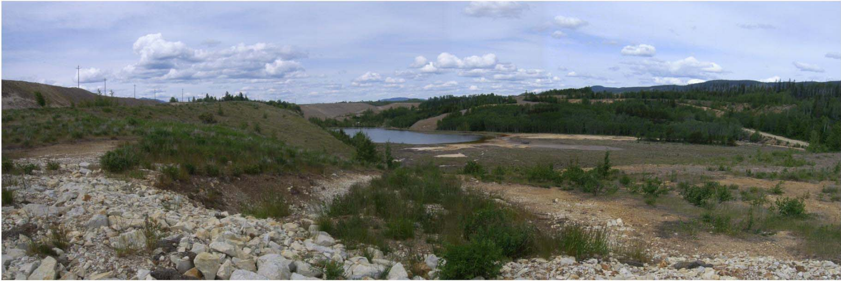
Photo C5-1: View of downstream slope and toe of Dam 5, looking northeast from the downstream slope of Dam 5. Note tailings beyond the toe of Dam 5 as part of Tailings Pond Expansion area. (11 June 2014)
