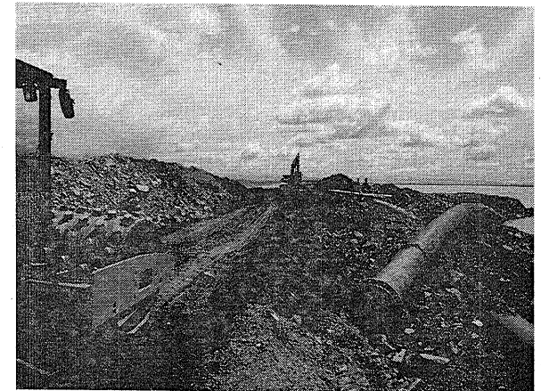
Photo 6: Till compaction at perimeter pipe crossing on May 28th
