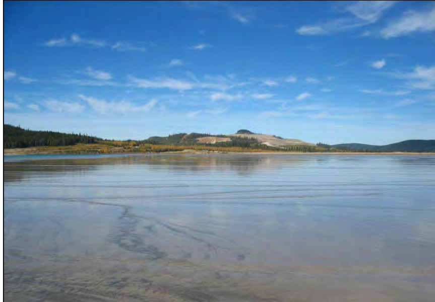
PHOTO 11 – Tailings Beach, From Main Embankment looking towards Perimeter Embankment.
