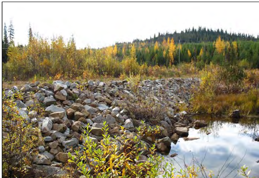
PHOTO 16 – South Bootjack Dam.
