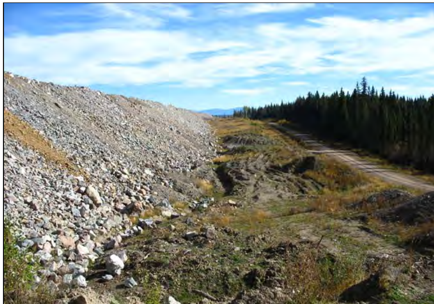
PHOTO 12 – Downstream Slope of South Embankment.
