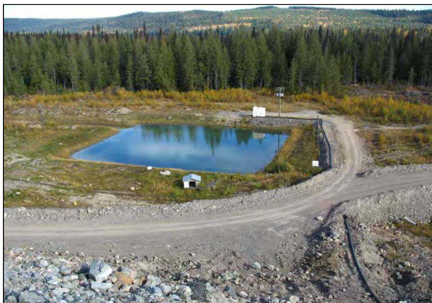
PHOTO 2 – Perimeter Embankment Seepage Collection and Recycle Pond.
