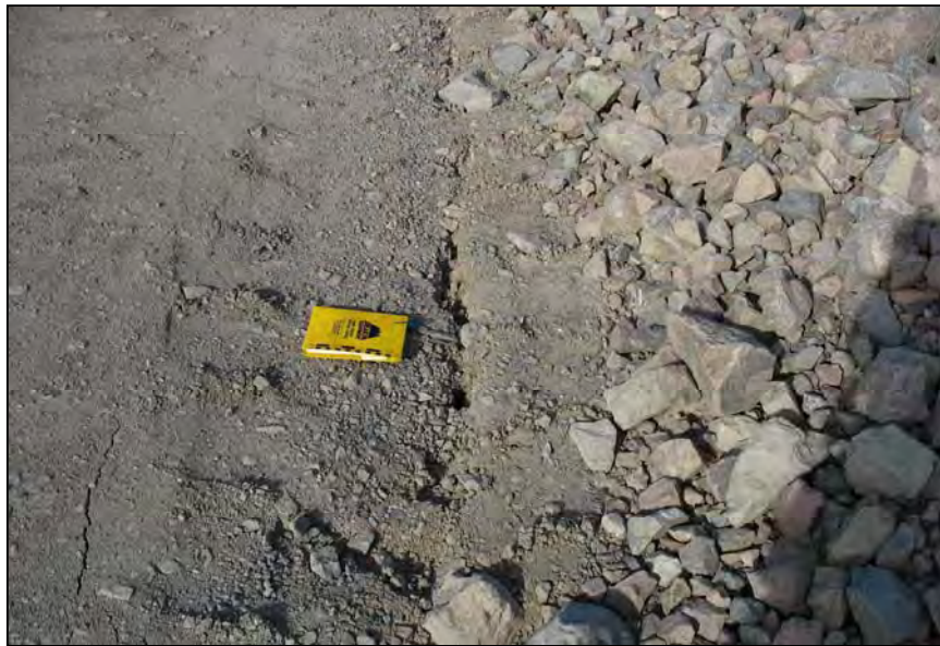
PHOTO 6 – Tension Crack at the Perimeter Embankment.
