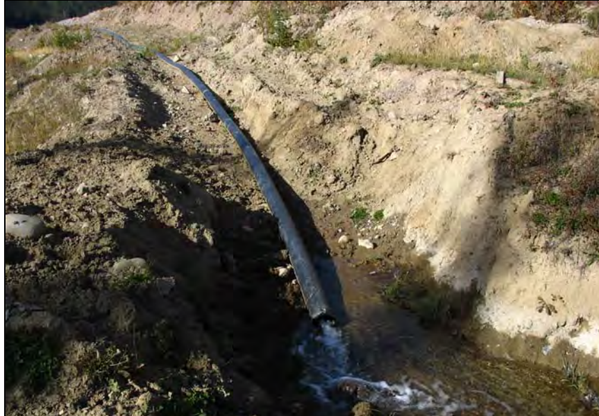
PHOTO 15 – South Embankment Upstream Toe Drain flow.
