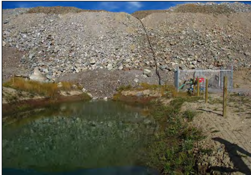
PHOTO 14 – South Embankment Seepage Collection and Recycle Pond.
