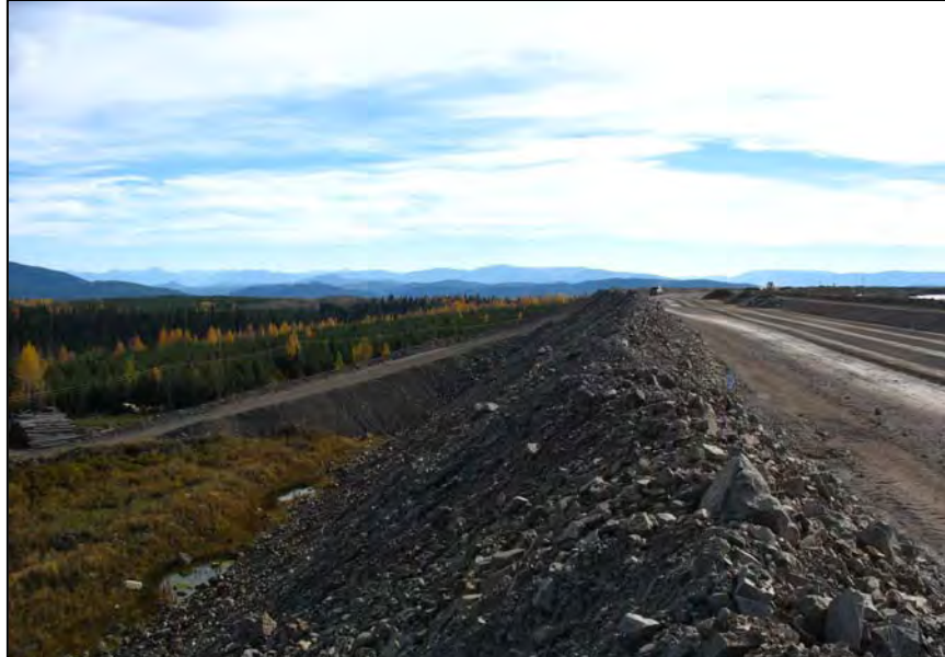
PHOTO 5 – Tension Crack Location at the Perimeter Embankment.
