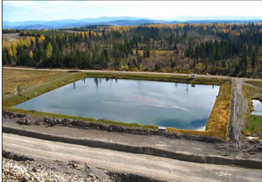
PHOTO 9 – Main Embankment Seepage Collection and Recycle Pond.
