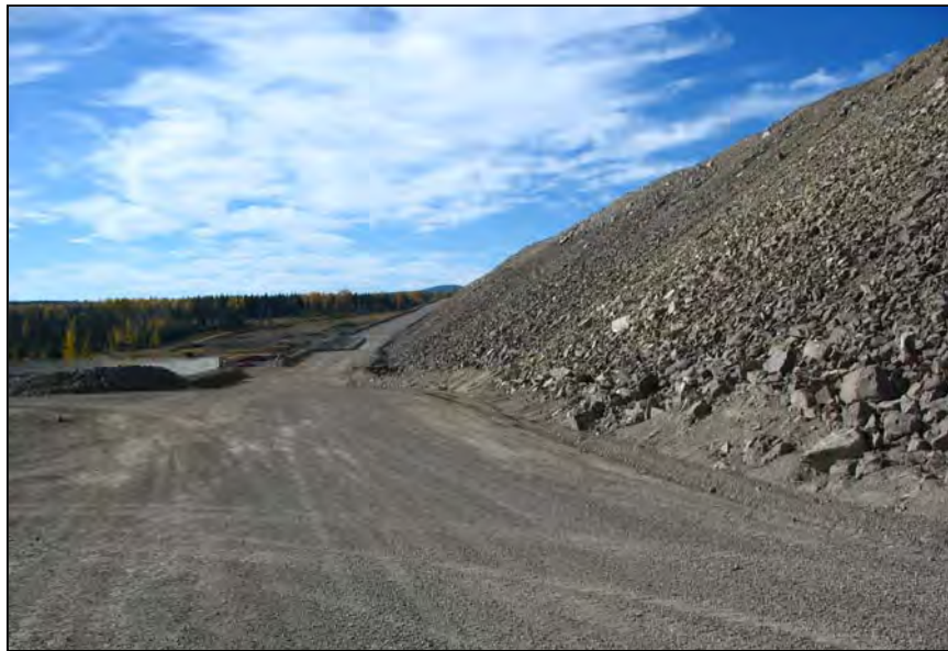
PHOTO 8 – Downstream Slope of Main Embankment.
