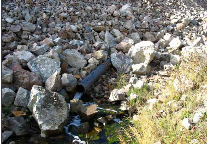
PHOTO 3 – Perimeter Embankment Toe Drain Flow.
