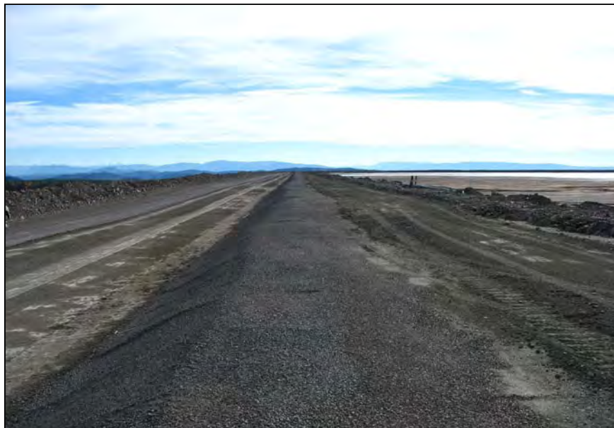
PHOTO 1 – Perimeter Embankment Crest.
