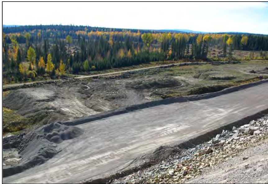
PHOTO 10 – Main Embankment Buttress.
