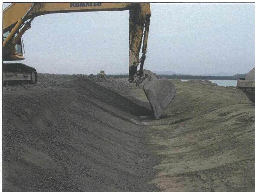
PHOTO 17 – Using a hoe to move the Zone F filter material into its final position.
