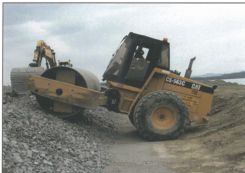
PHOTO 18 – Compacting the modified design Zone T. This new design is much faster and easier to compact.
