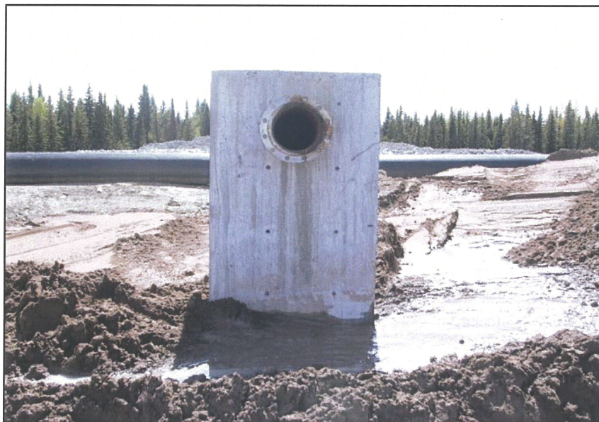
PHOTO 28 – South Embankment toe drain concrete encasement.
