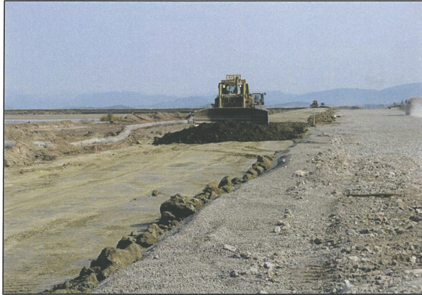
PHOTO 7 – Adding the 777's allowed for a second 'dozer roller team effectively doubling the till production rate
