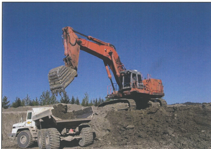
PHOTO 4 – Removing Till (Zone S) from Borrow Area 2
