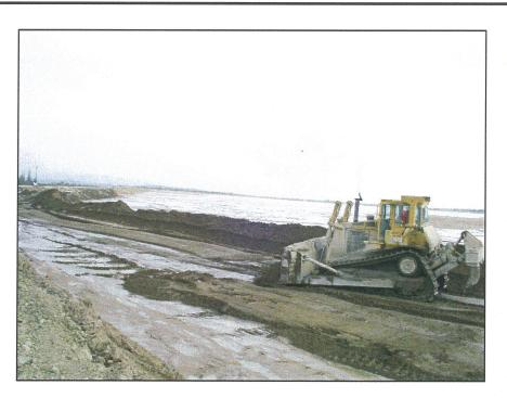
PHOTO 15 - Sand Cell on the Perimeter Embankment.
