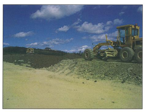
**PHOTO 22** – Placing till on the Perimeter Embankment.
