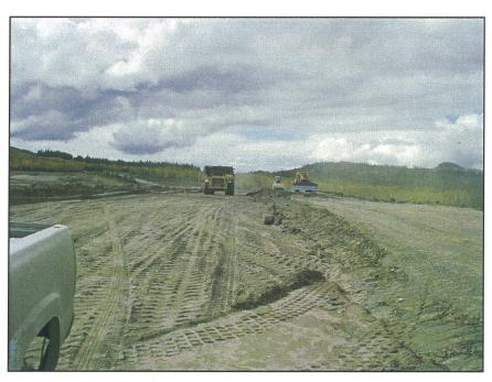
**PHOTO 19** – Placing sand from the Cyclone sand stock pile on the Perimeter Embankment as Zone U.
