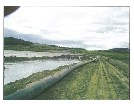
**PHOTO 16** – Sand cell on the Perimeter Embankment. Tailings are discharged at the far end and exit into the TSF through culverts installed at the opposite end of the cell.
