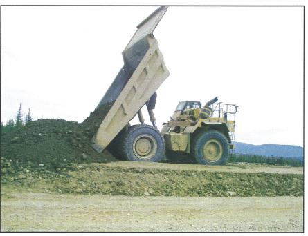
**PHOTO 28** – Placing Zone S material with a 777 haul truck on the Perimeter Embankment.
