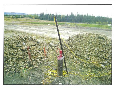
**PHOTO 33** – A "poorboy" was used to ensure that there were no "pinch points" in the inclinometers.
