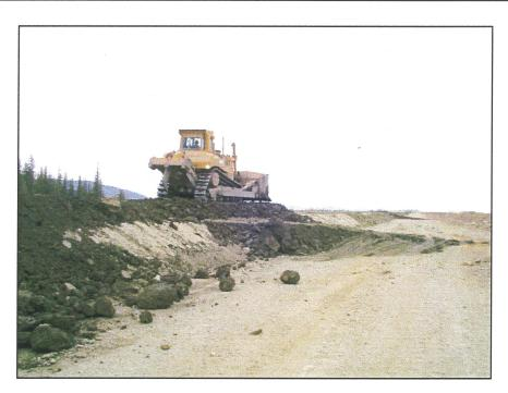
**PHOTO 27** –Till ramps were set up to minimize the traffic on the Zone S material with the 777 haul trucks.
