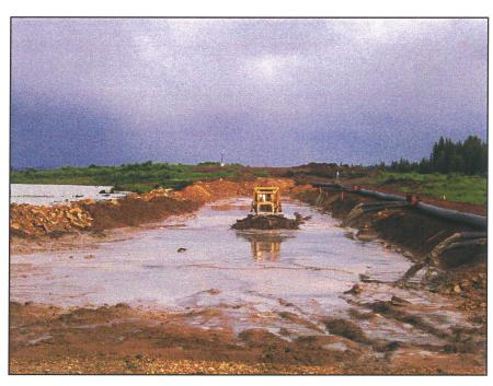
**PHOTO 11** – Using a dozer in the sand cell at the South Embankment to distribute and compact the tailings sand.
