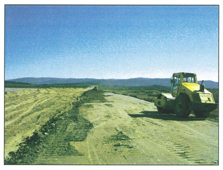
**PHOTO 24** – The vibratory smooth drum compacting Zone S material on the Main Embankment.
