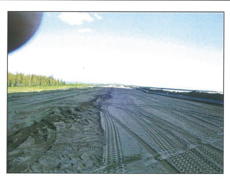
PHOTO 17 - Comleted sand cell on the Perimeter Embankment.
