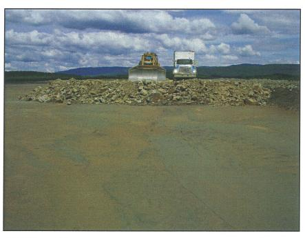
PHOTO 5 - CBL placement on the tailings beach at the Main Embankment.
