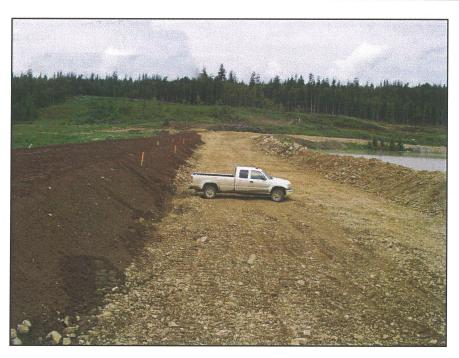
PHOTO 7 – South Embankment after the Stage 4 CBL was placed.
