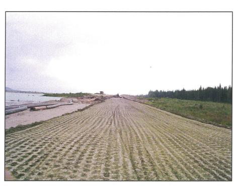
**PHOTO 21** – Scarifying the Zone S material at the South Embankment with a sheepsfoot prior to placing the next lift.
