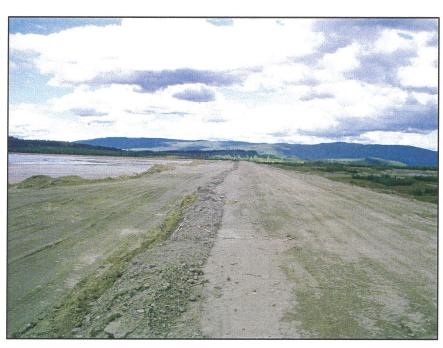
**PHOTO 31** – Completed Zone U and Zone S lift on the Main Embankment.
