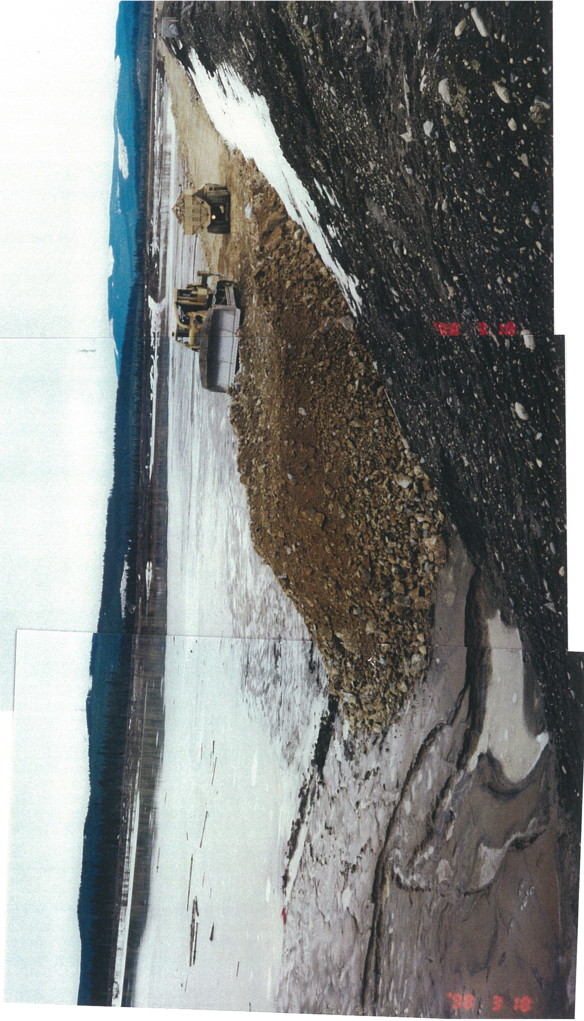
Photo No. 5: Placement of Coarse Bearing Layer (Zone CBL) on Tailings at Main Embankment, March 18, 1998.
