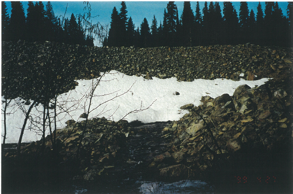
Photo No. 11: Bootjack Creek Culvert. Downstream side.
