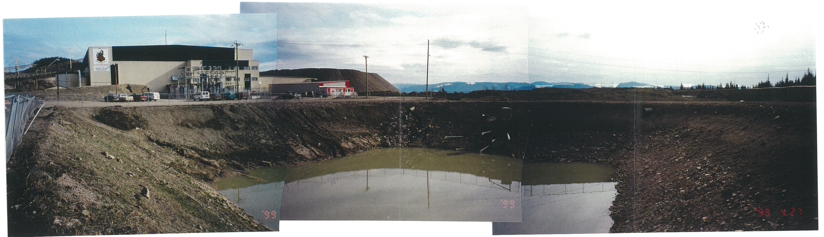
Photo No. 20: Millsite Sump. Note low water level and stable inner slopes.
