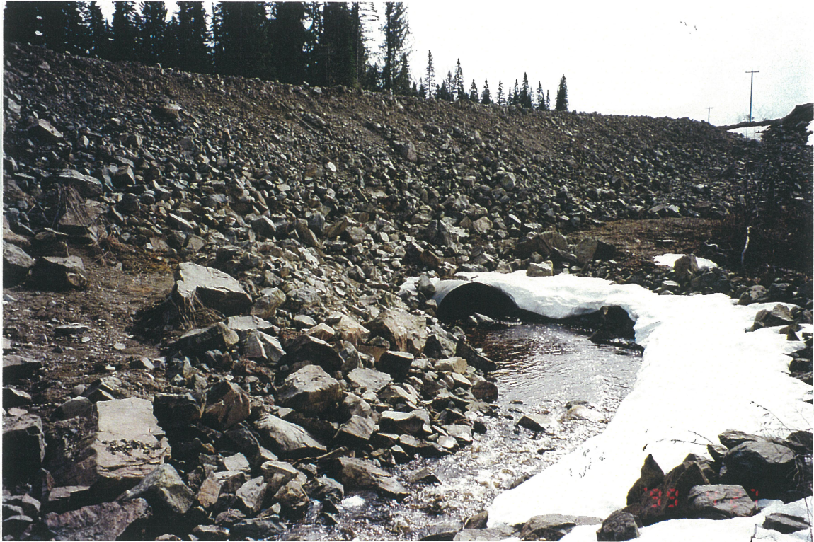
Photo No. 10: Bootjack Creek Culvert. Upstream side.
