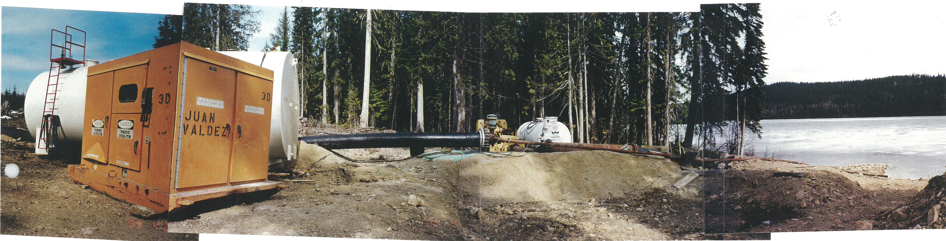
Photo No. 19: Polley Lake Pumping System. Intake Area. Note float on Polley Lake. Float is attached to the intake.
