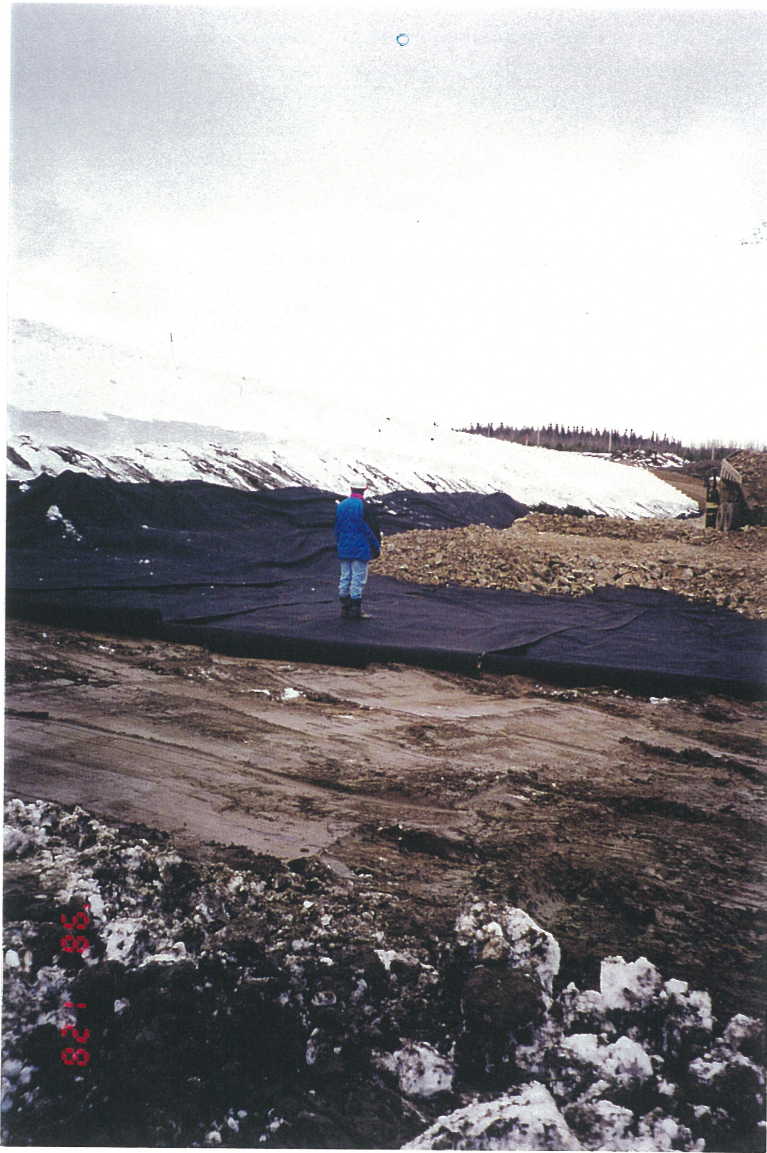
Photo No. 3: Prepared foundation at Perimeter Embankment with Type 2 Geotextile Filter Fabric layer between Transition Zone Material (Zone T) and Foundation Soil, January 28, 1998.
