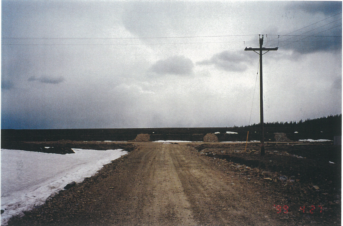
Photo No. 6: Perimeter Embankment. Looking upstream from access road on east side of Seepage Collection Pond. Note Outlet Drains going up face of embankment.
