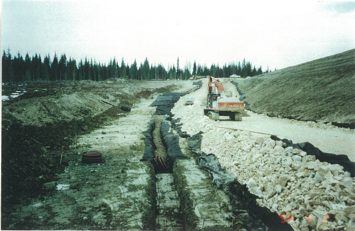
Photo No. 1: Installing Foundation Drain FD-5 at Main Embankment, April 2, 1998.
