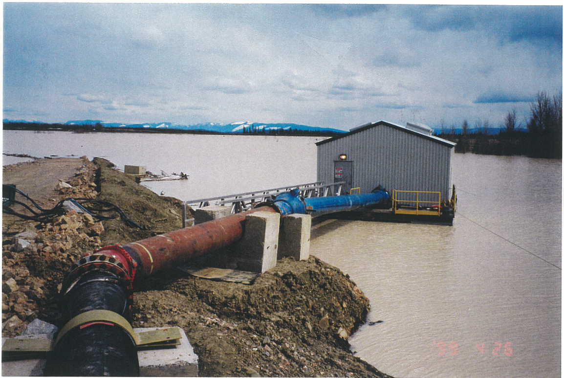
Photo No. 14: Reclaim Pipeline System. Reclaim Barge and Channel. Note 35 degree elbow added and barge alignment changed.
