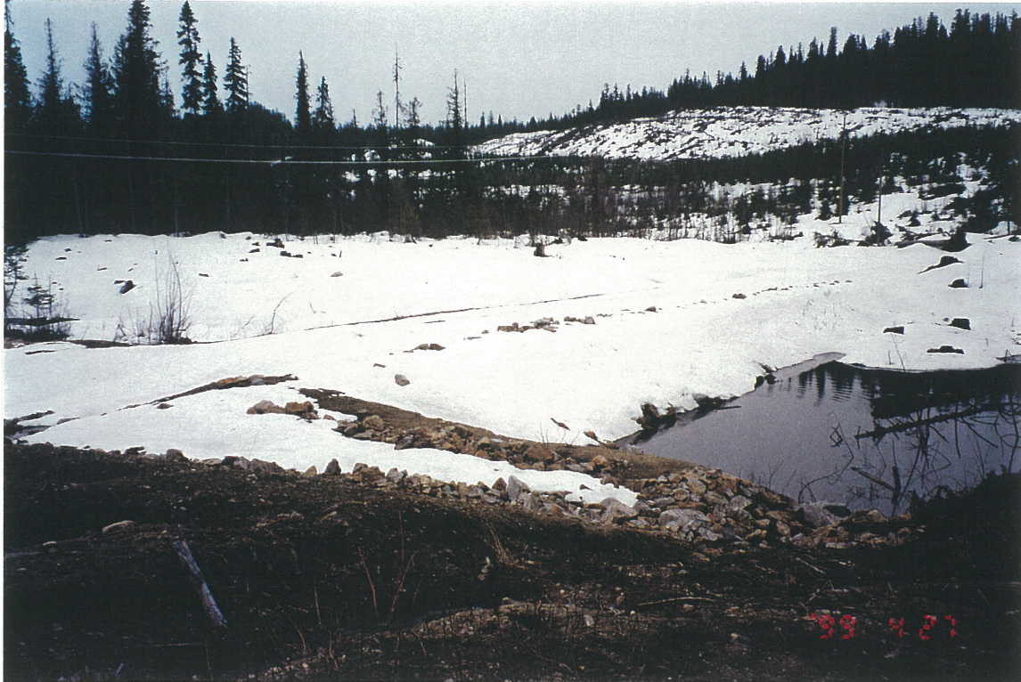
Photo No. 22: South Bootjack Dam. View of upstream face of embankment, looking northwest. Ponded water is now seeping through old dam back into Bootjack Lake.
