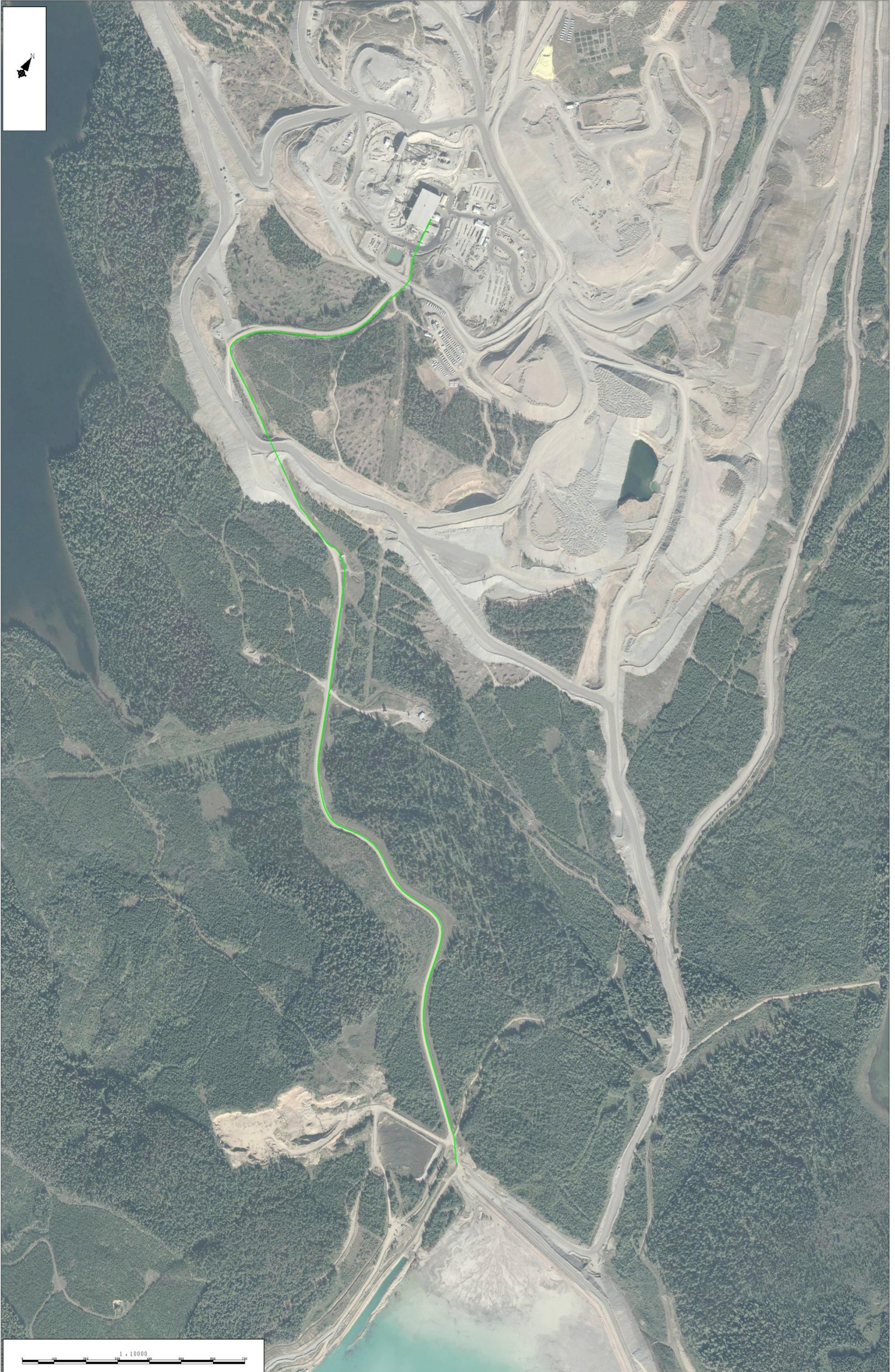
Figure 4.2.1.1 - Tailings Line Mill to TSF
