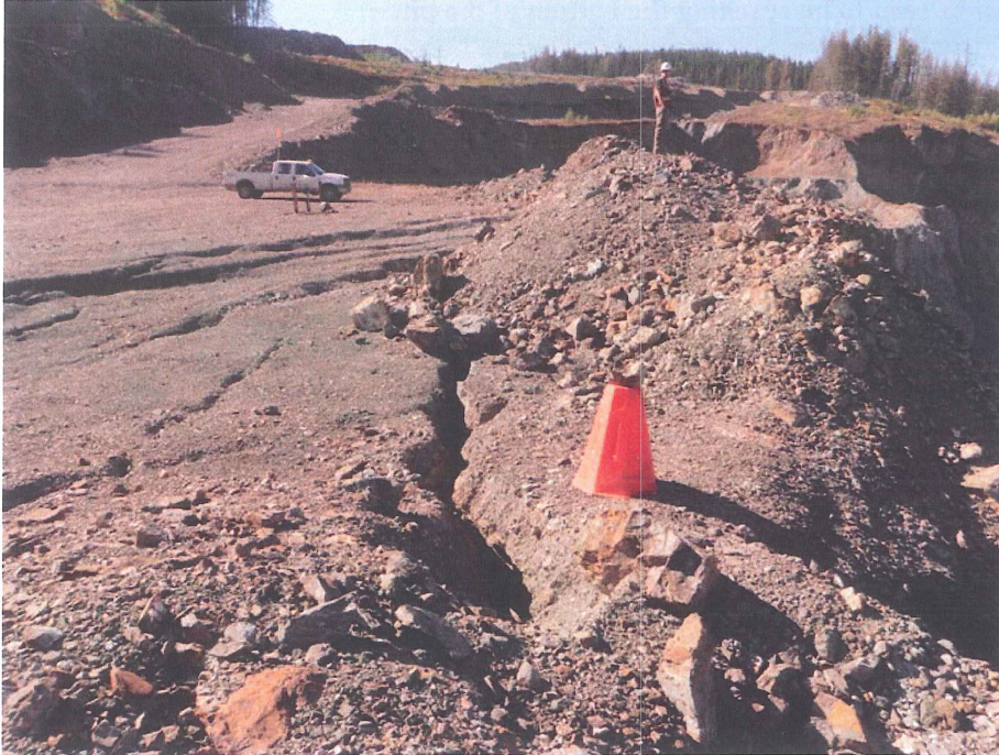
Photo 2: Tension Cracks and slump on western crest of Wight Pit above underground infrastructure
