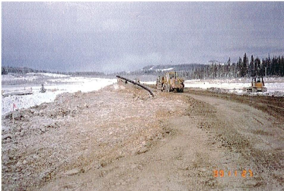
**Photo No. 6:** Perimeter Embankment upstream toe drain (to be installed later) will tie into the exposed pipe.
