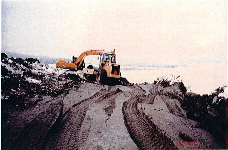
**Photo No. 12:** Backfilling basin liner trench.
