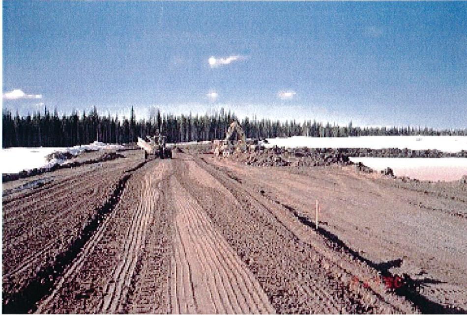
**Photo No. 14:** Mechanical placement of cycloned sand in the upstream fill of the Main Embankment.
