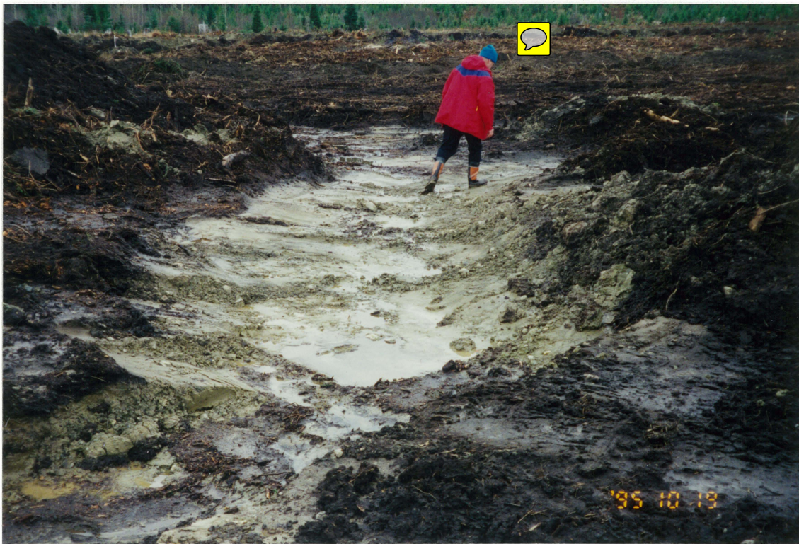
Photo 5 - Glacial till surface exposed by removing organic overburden. The exposed surface is slippery. Prior to placing and fill the surface must be scarified.
