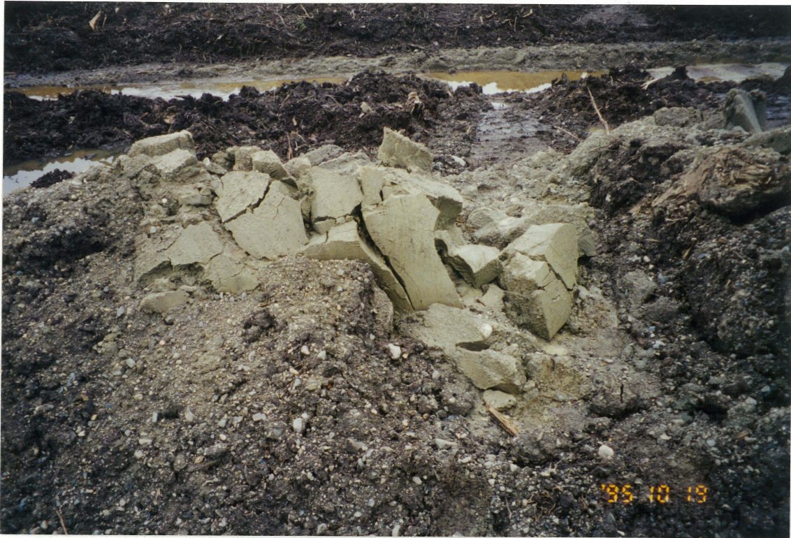
Photo 4 - Excavated medium dense glacial lacustrine clayey sandy silt. This material has medium strength, low permeability and medium-low compressibility.
