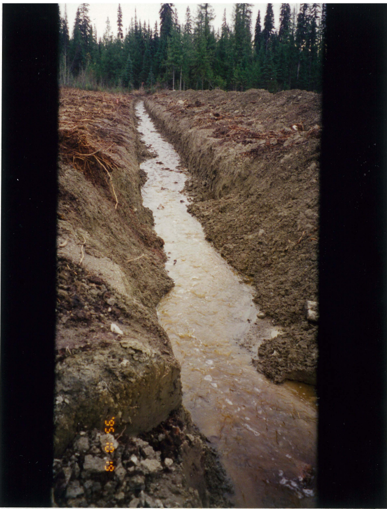
Photo 2 - Ditch excavated to contain a small creek across the site. The southern portion of the ditch is in medium dense to dense glacial till and the southern portion is in glacial lacustrine soils. Note the transition from stable side slopes to ravelling slopes. Easterly end of the dam.
