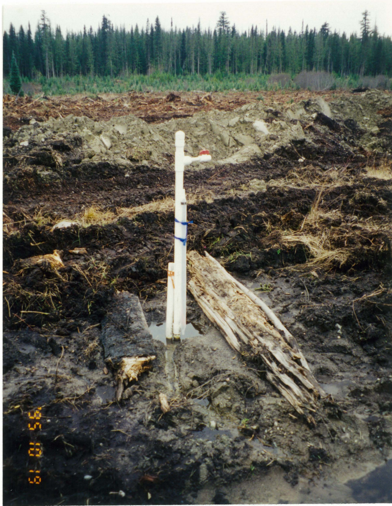
Photo 6 - Piezometer installed with water sampling capability. Toe area of the main dam.
