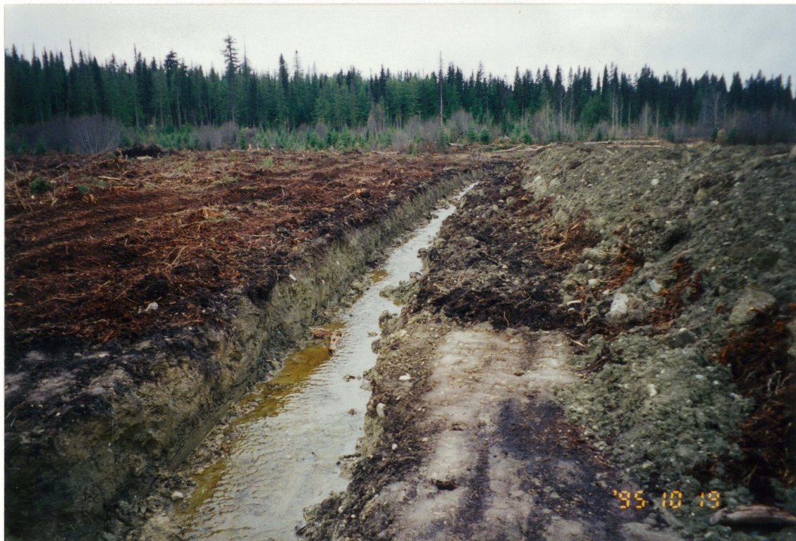
Photo 3 - Looking North along the westerly portion of the dam site. Drainage ditch in glacial till.
